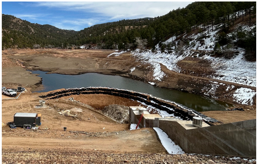
34 – View of drained reservoir, cofferdam, bypass pumping arrangement, and intake structure
