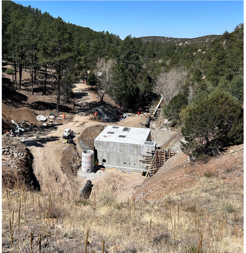
35 – Construction of the new Nichols valve vault
