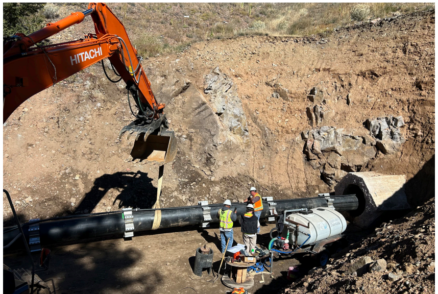
33 – Installation of new HDPE pipe within existing outlet conduit
