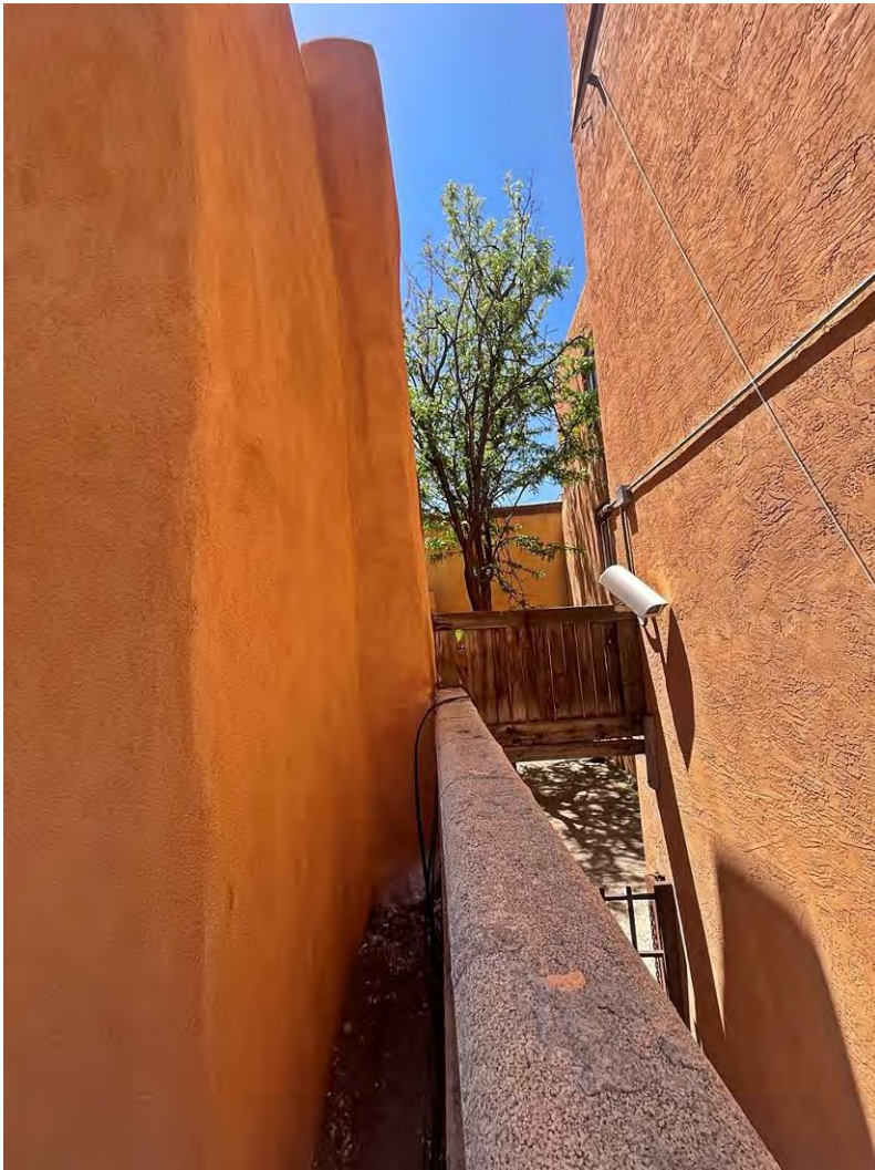
Photo 12: Back building, west elevation at left; Petroleum Building at right. Camera facing south.
