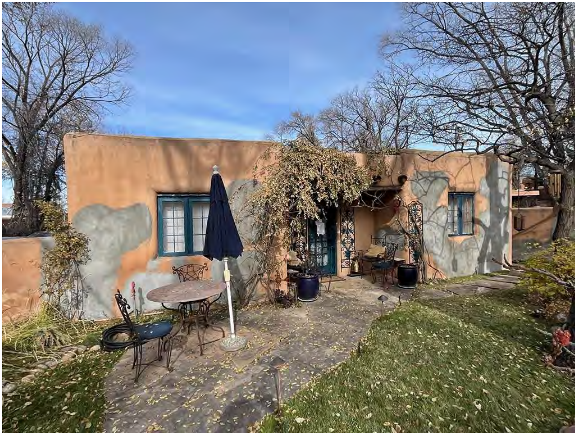
Photo 2: South (front) elevation. Camera facing northeast.
