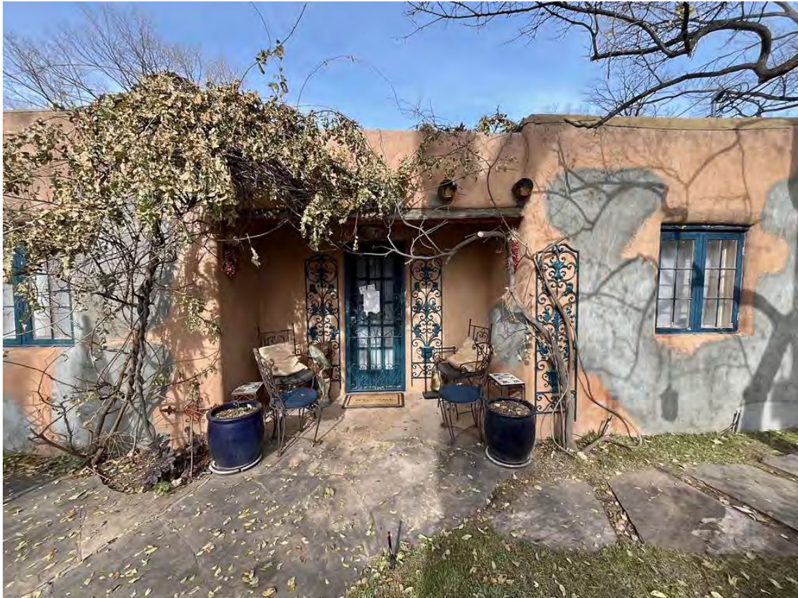
Photo 4: South (front) elevation. Recessed portal. Camera facing north.
