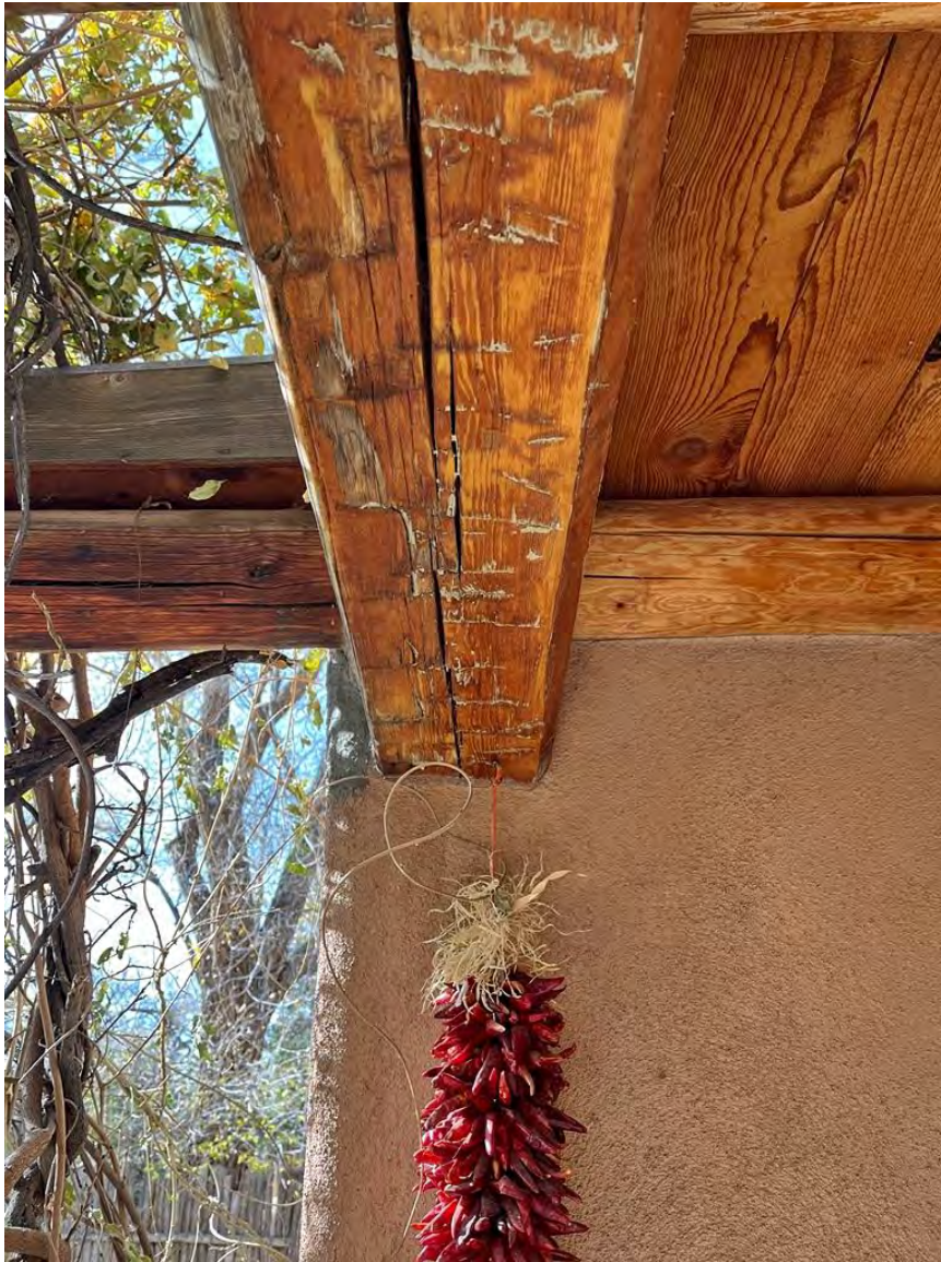
Photo 5: South (front) elevation. Recessed portal decking and beam. Camera facing up.
