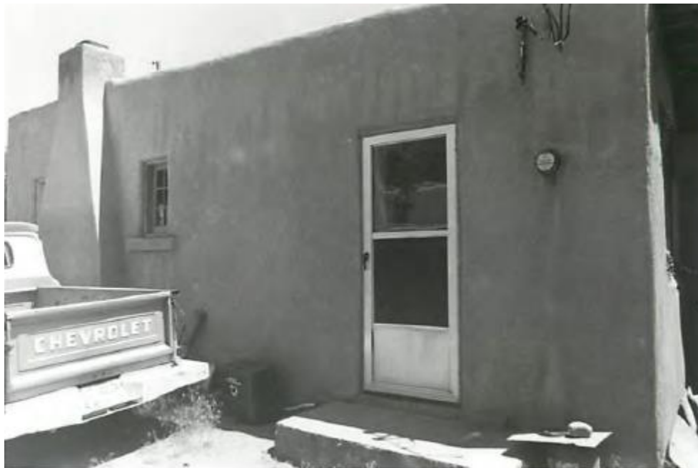
#24 east portion of north elevation
