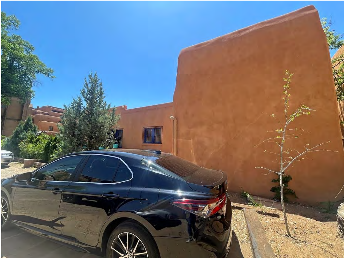
Photo 11: Back building, north elevation. Camera facing southeast.
