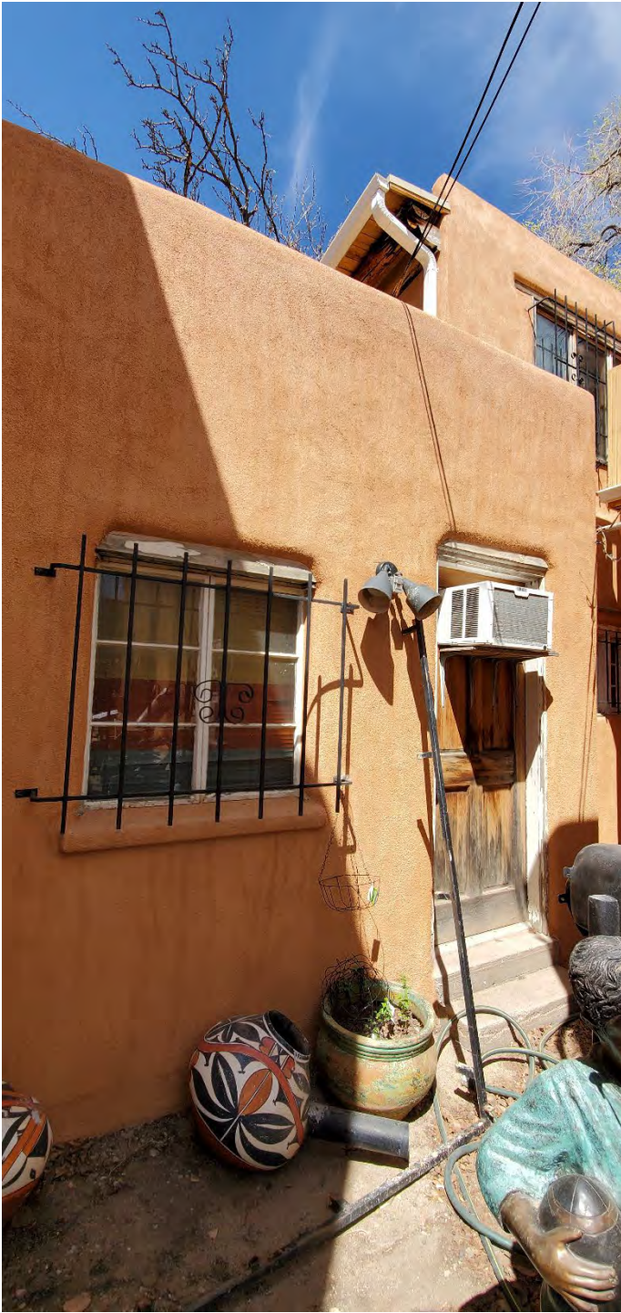
EXISTING EAST ELEVATION REAR SOUTH PORTION OF THE BUILDING (BEFORE FIRE DAMAGE)
