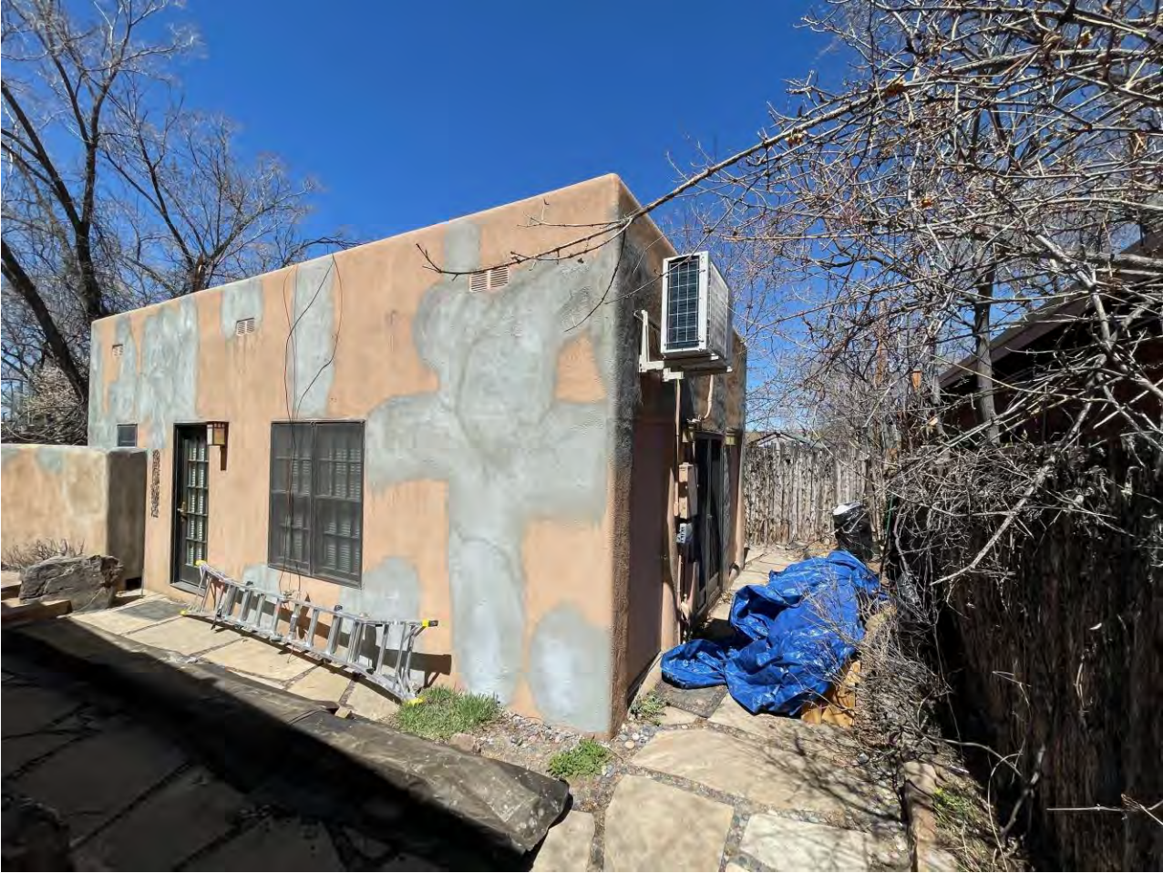
925 Casita Southeast Elevation at Courtyard
