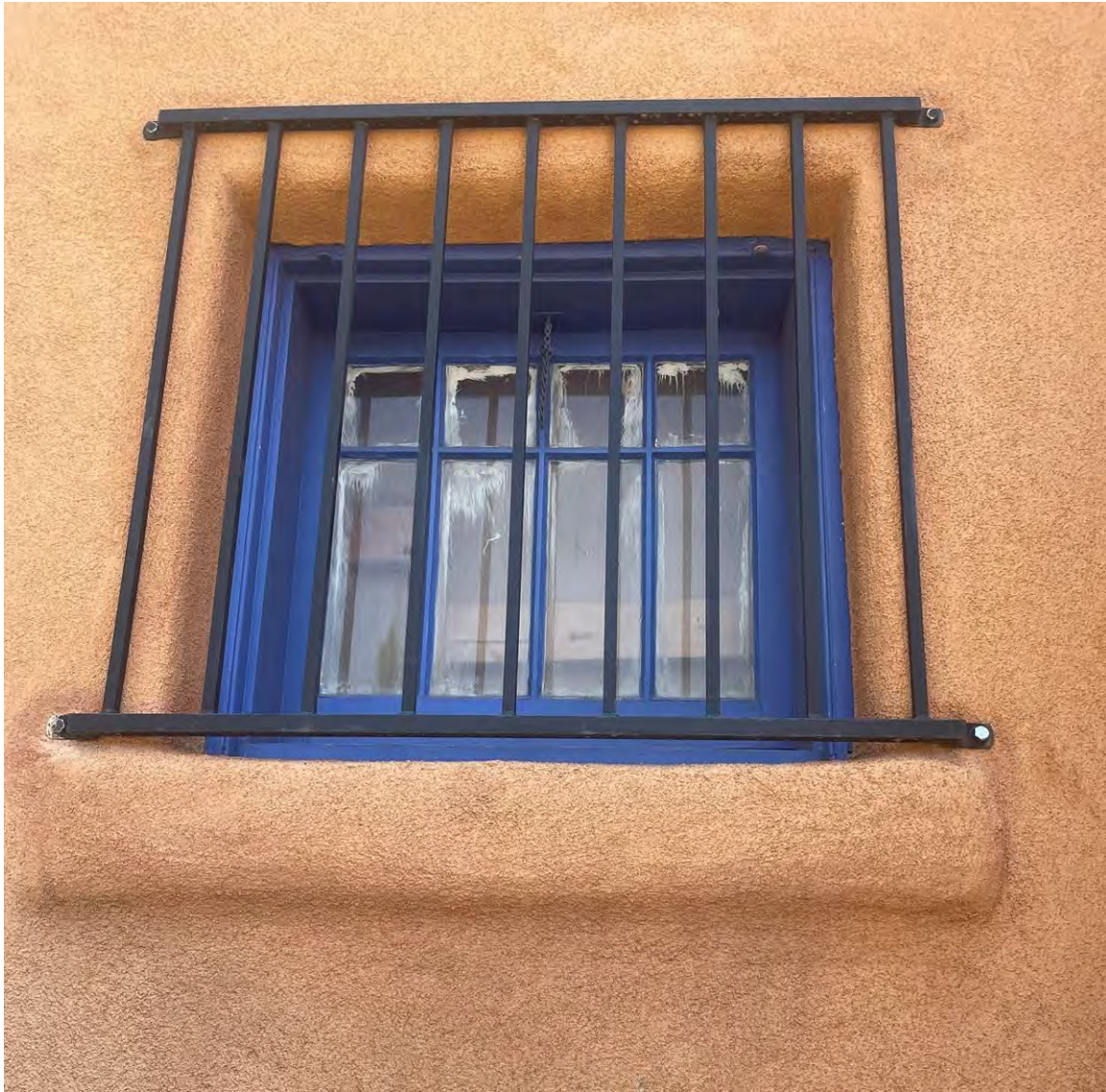
Photo 4: North elevation. Window #1. Camera facing up.
