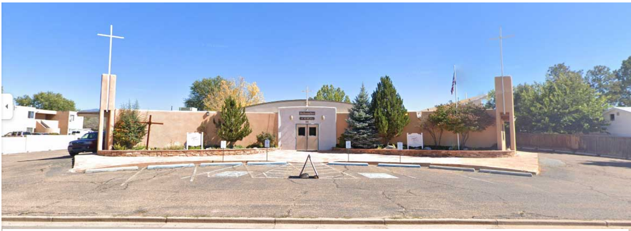
Figure 6 – Front of Existing Grace Community Church
