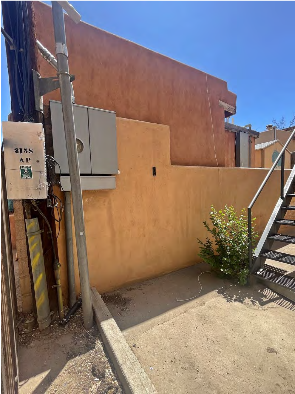
Photo 4: West elevation. Camera facing southeast.
