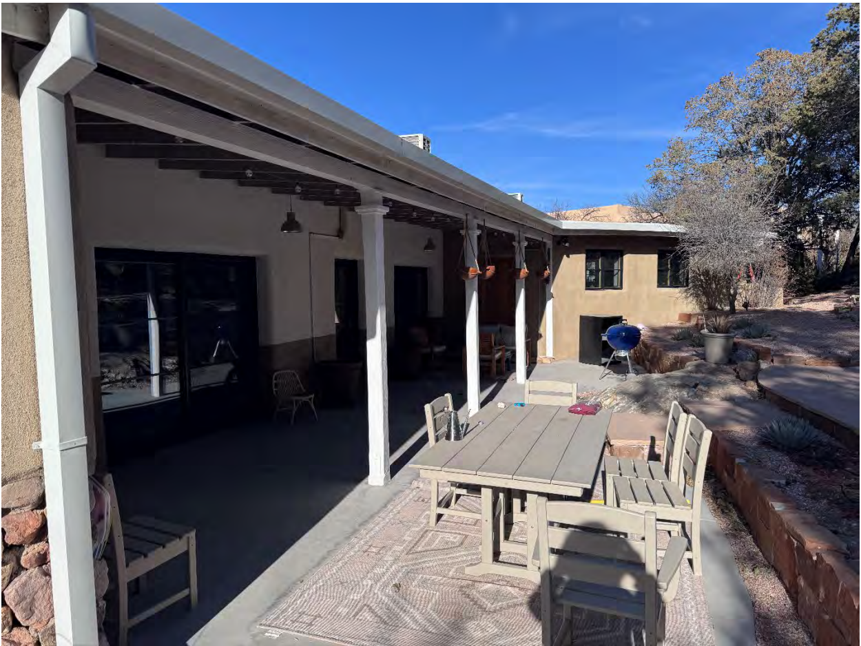
South elevation portal detail.
