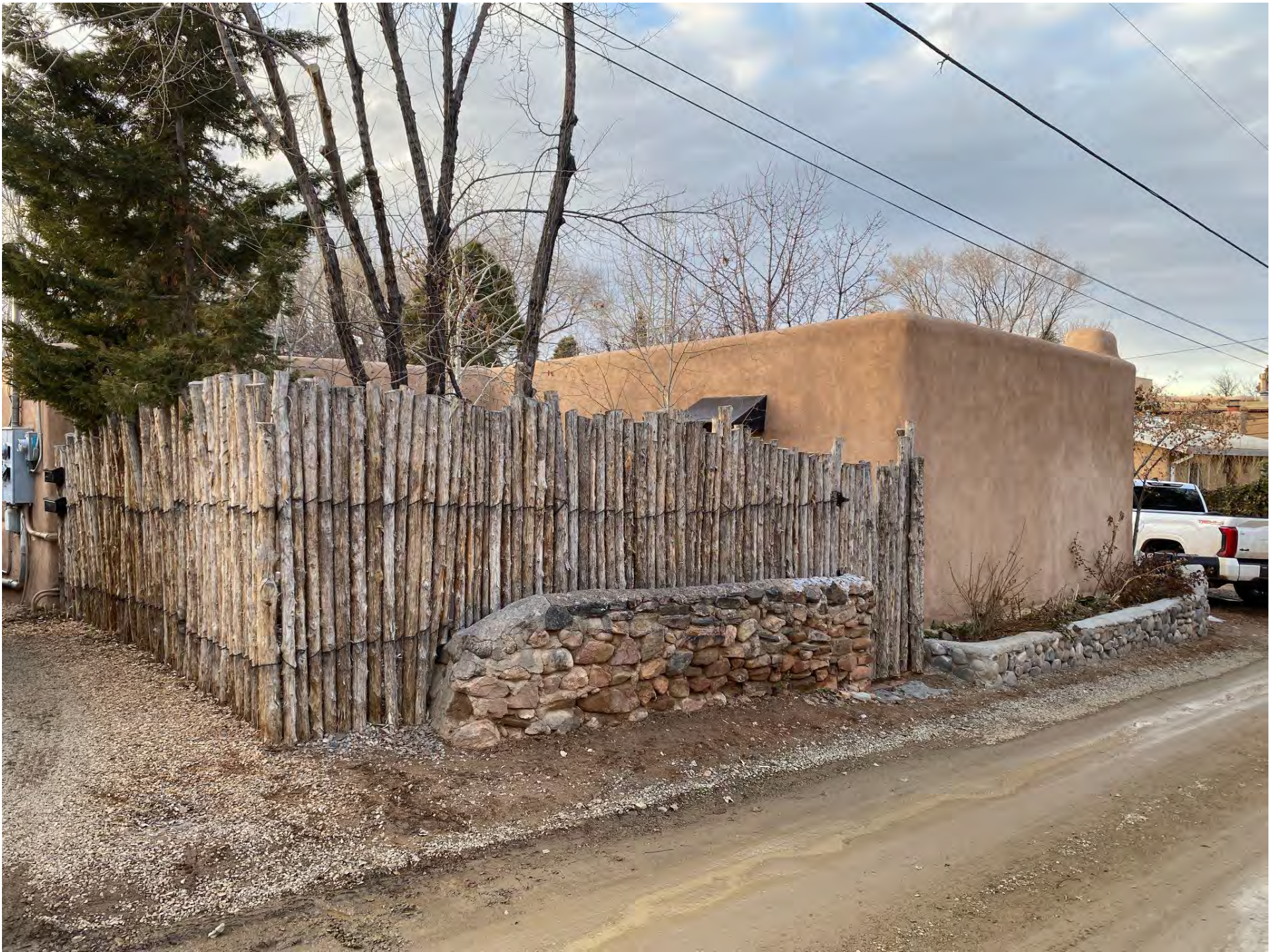
512 Abeyta Street Santa Fe, NM 87505- South East Elevation
