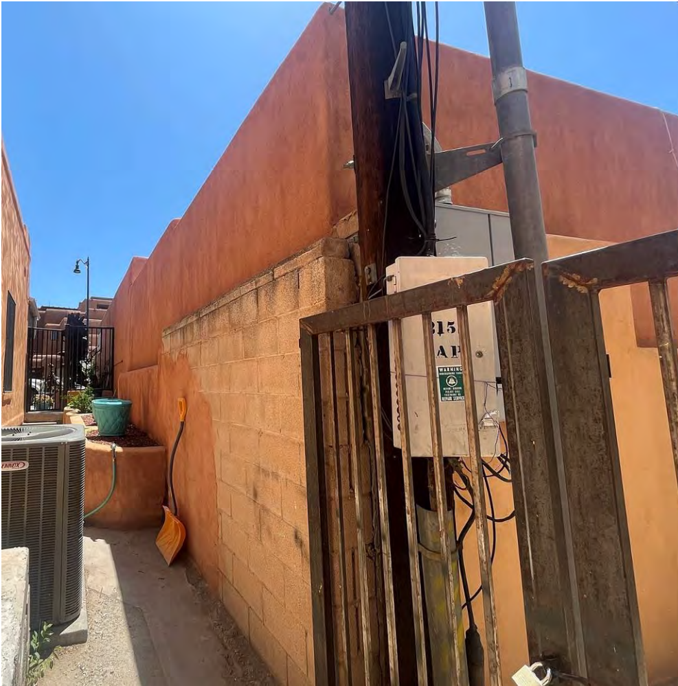
Photo 2: North elevation. Camera facing southeast.
