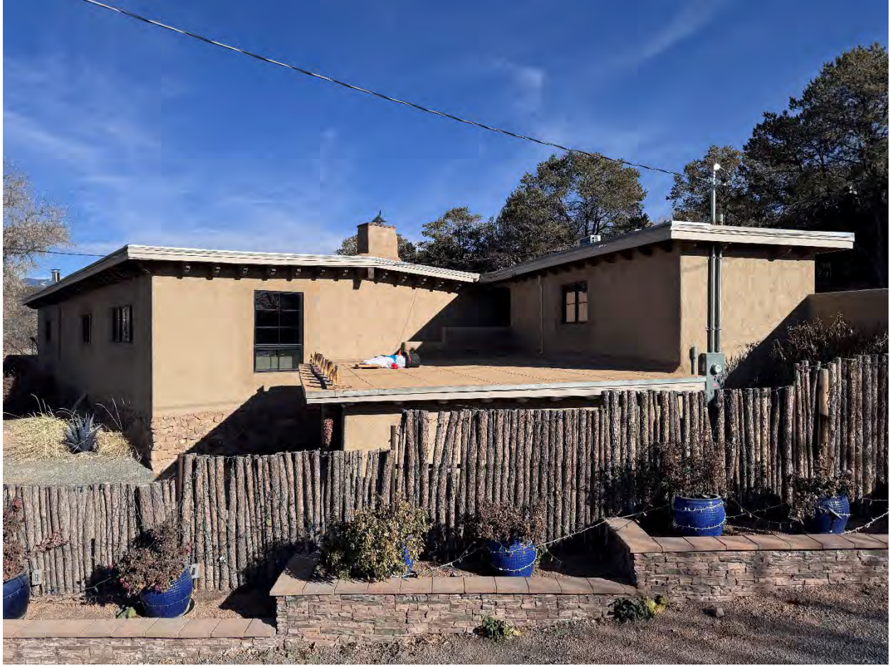
West and north (front) elevations of house and carport.
