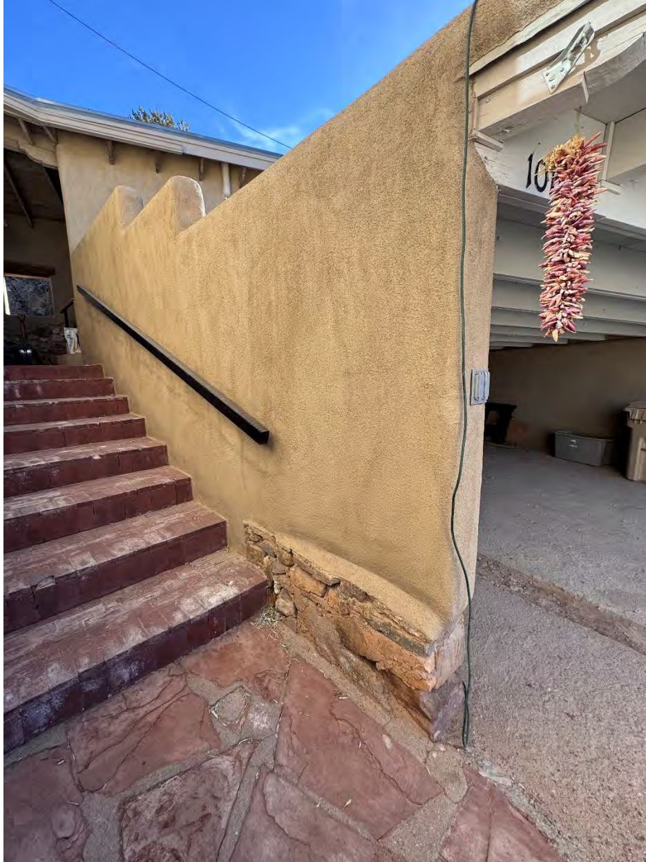
Detail of entry stairs, east elevation of carport.
