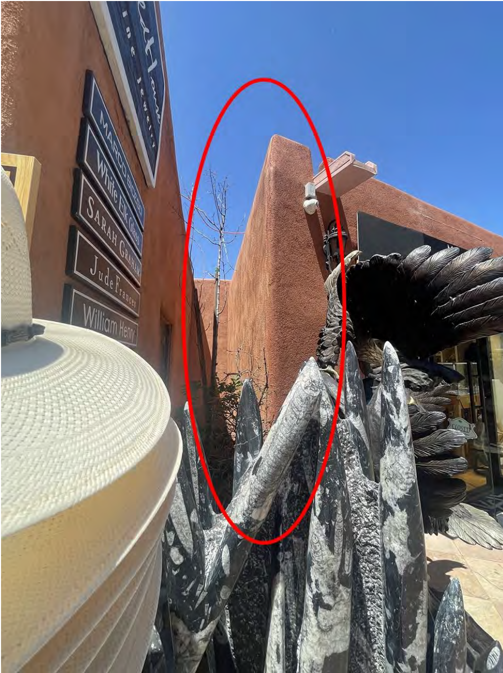
Photo 3: South elevation. Camera facing northwest.
