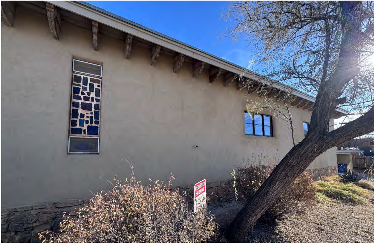
Front (north) elevation with stained-glass window.
