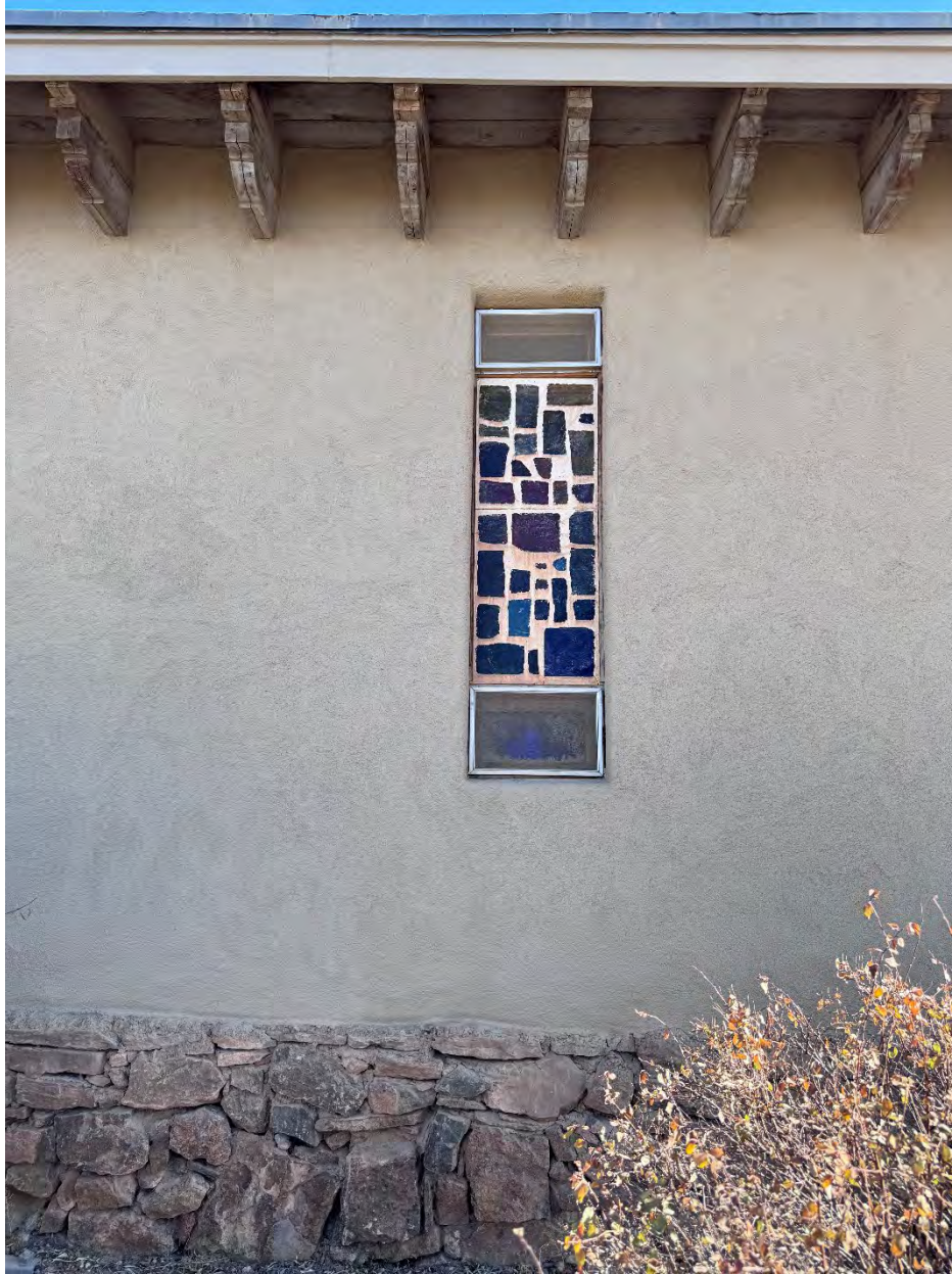
Detail of stained-glass window, front (north) elevation.
