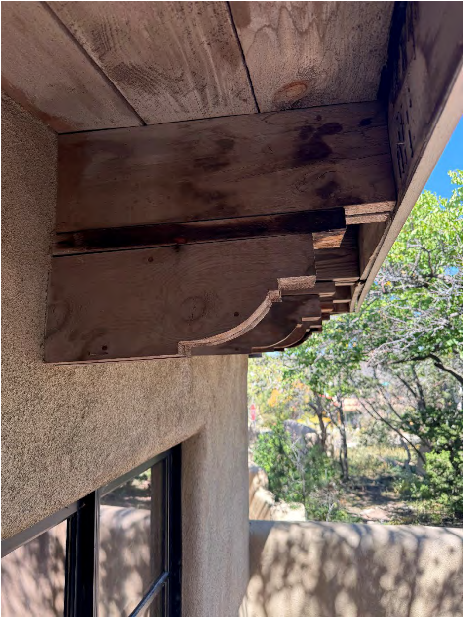
Detail of decorative corbelled brackets.
