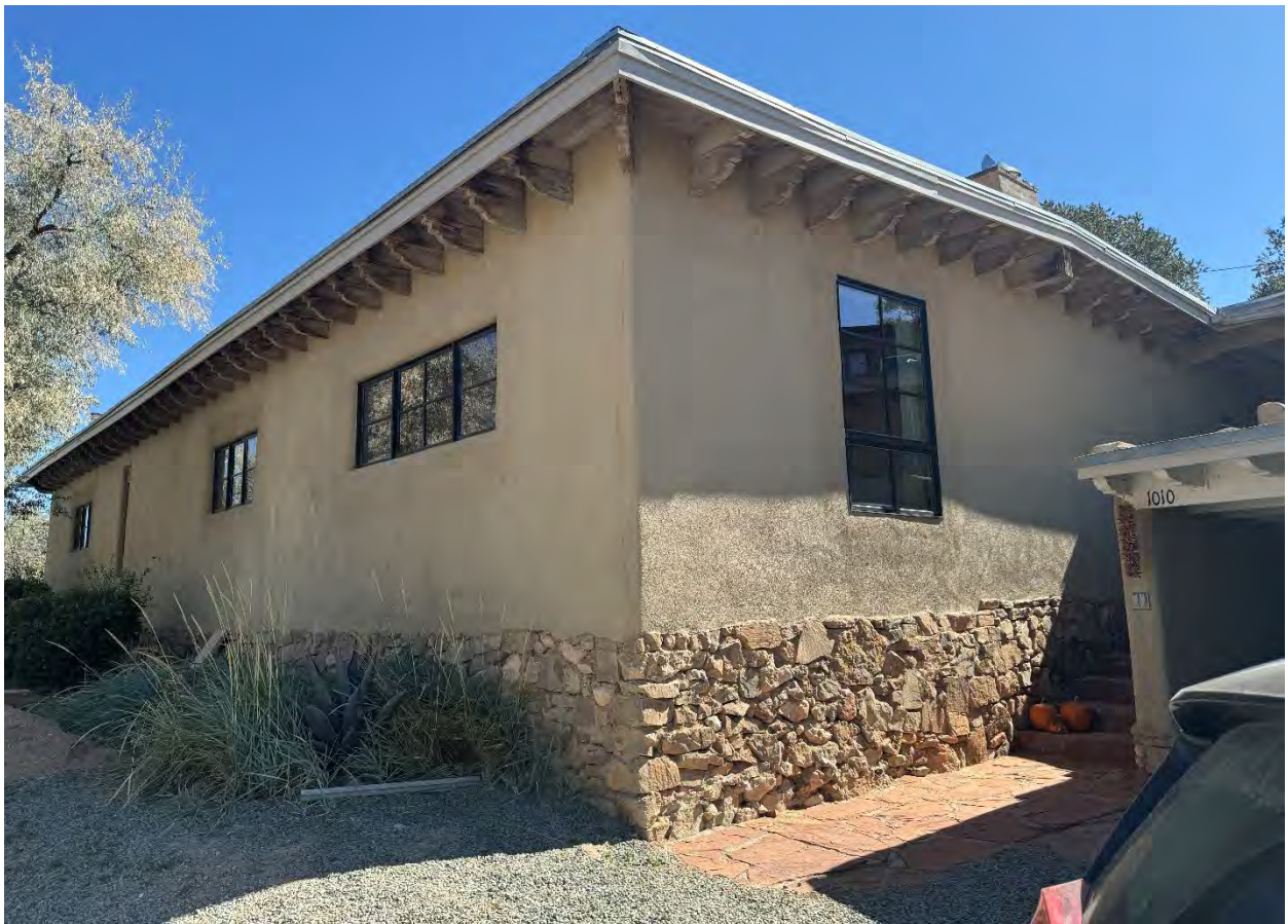
Front (north) and west elevations.
