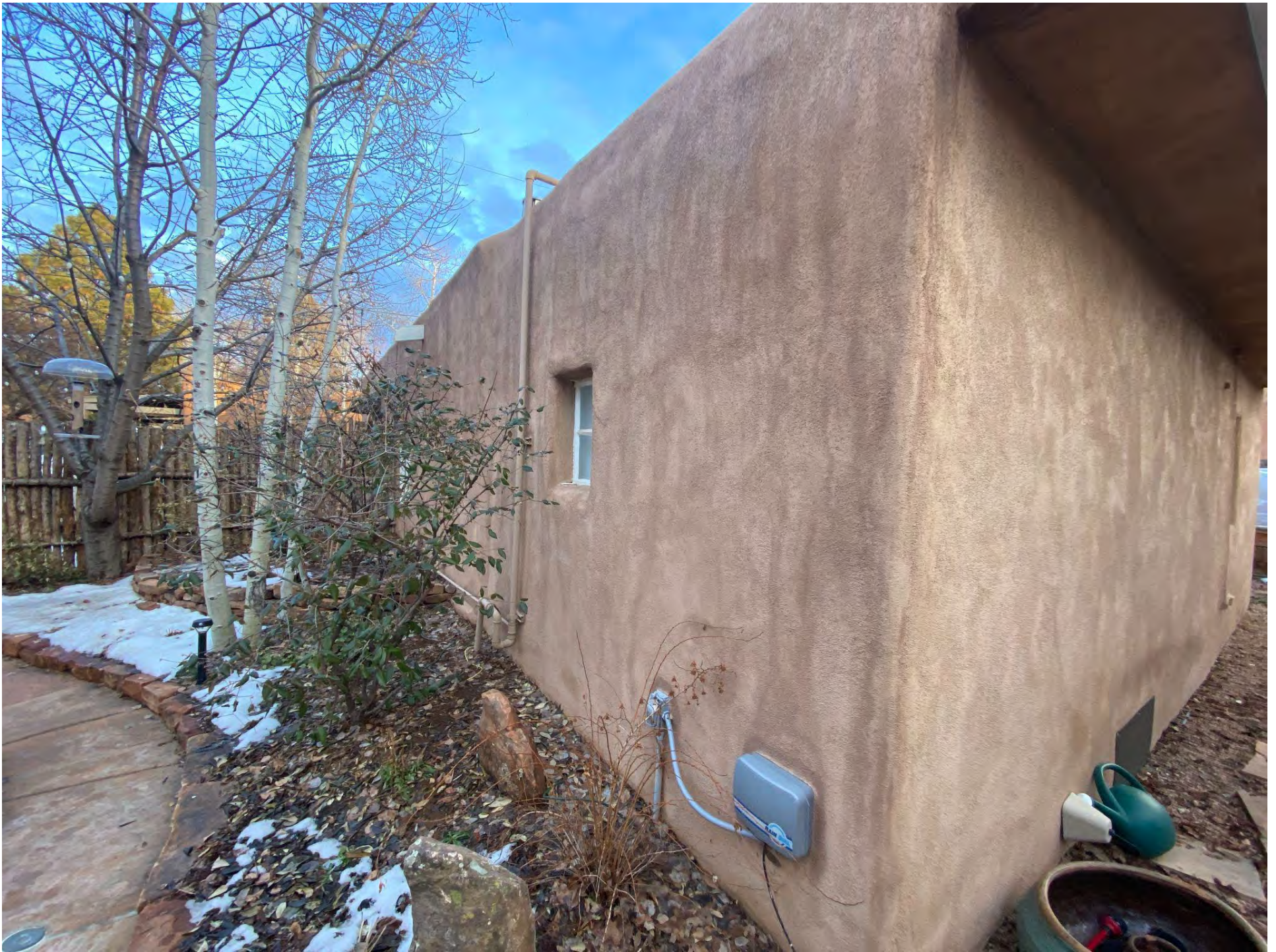
512 Abeyta Street Santa Fe, NM 87505- South Elevation
