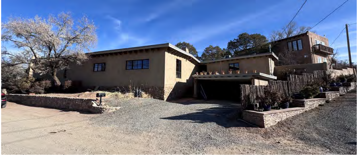
Front (north) and west elevations.
