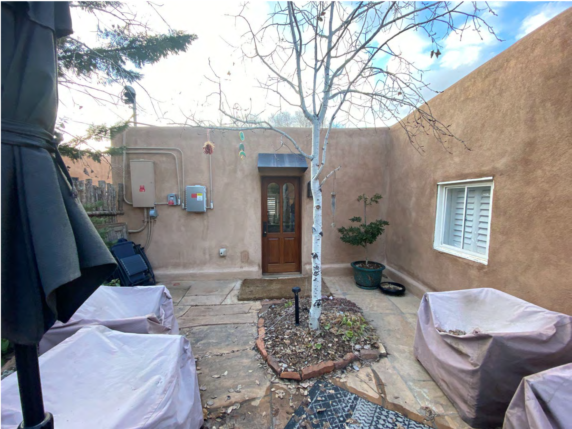
512 Abeyta Street Santa Fe, NM 87505- East Elevation
