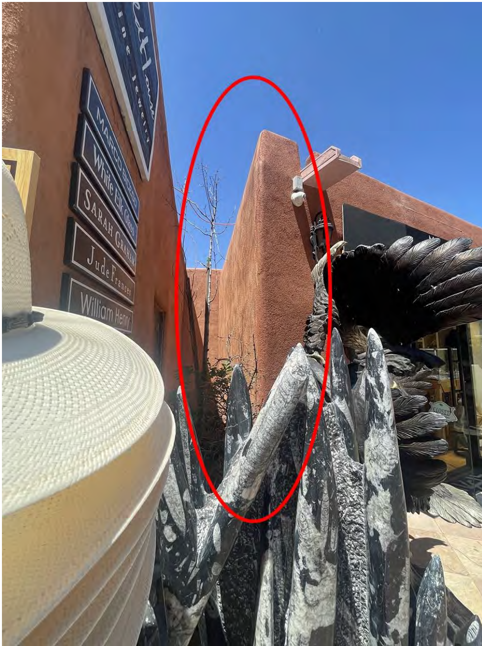
Photo 3: South elevation. Camera facing northwest.
