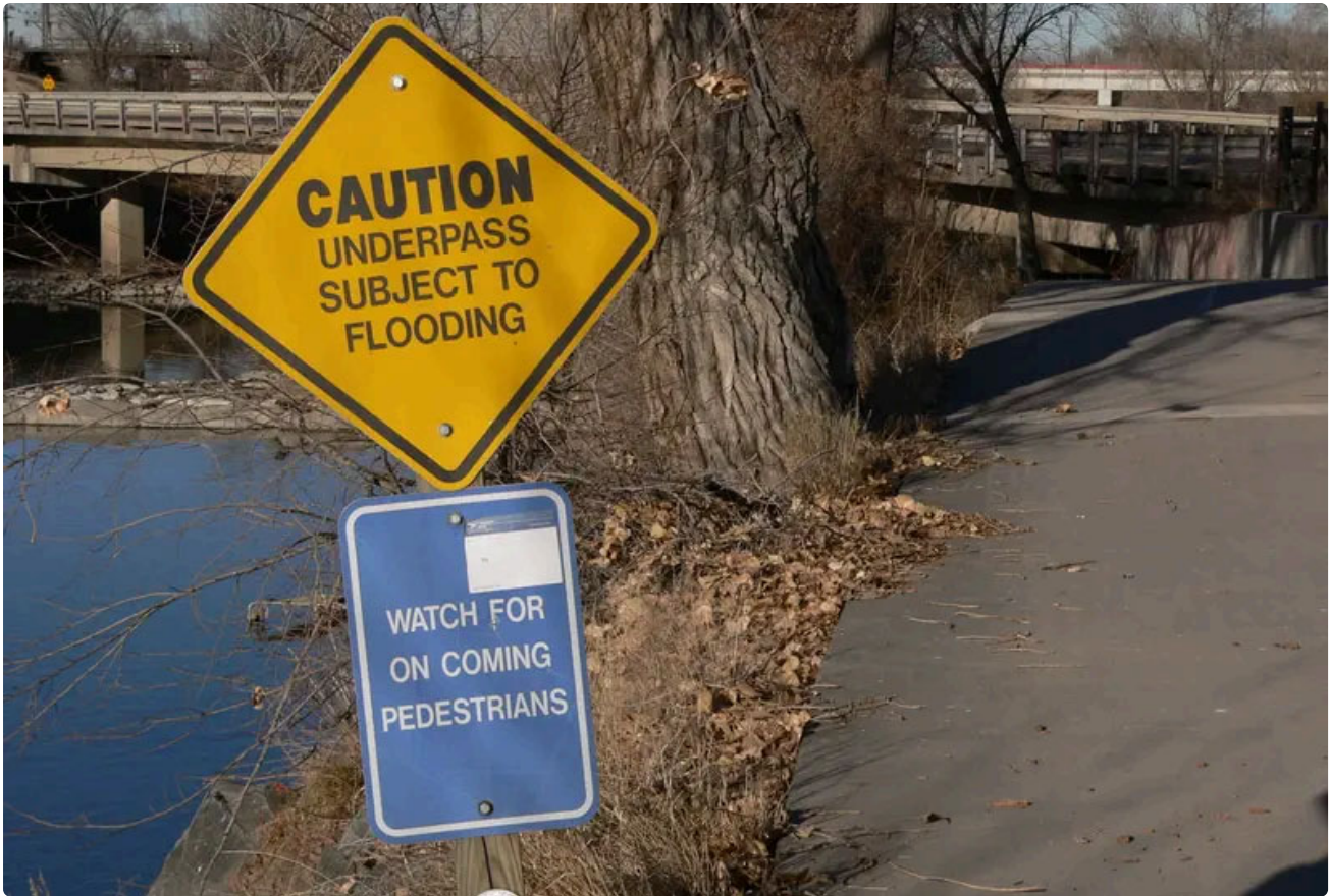
( https://optimise2.assets-servd.host/material-civet/production/images/15-P1160799.JPG?w=800&h=540&auto=compress%2Cformat&fit=crop&dm=1620062402&s=f29de8512dd681af3e39b7969a251a99 ) Sign at curving trail underpass warning cyclists along Cherry Creek Trail, Denver, CO
