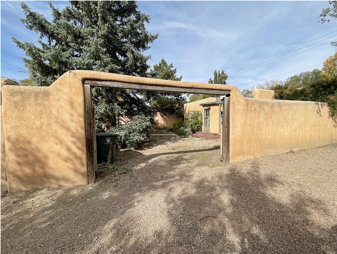
Photo 12: Alley wall. Camera facing northeast.
