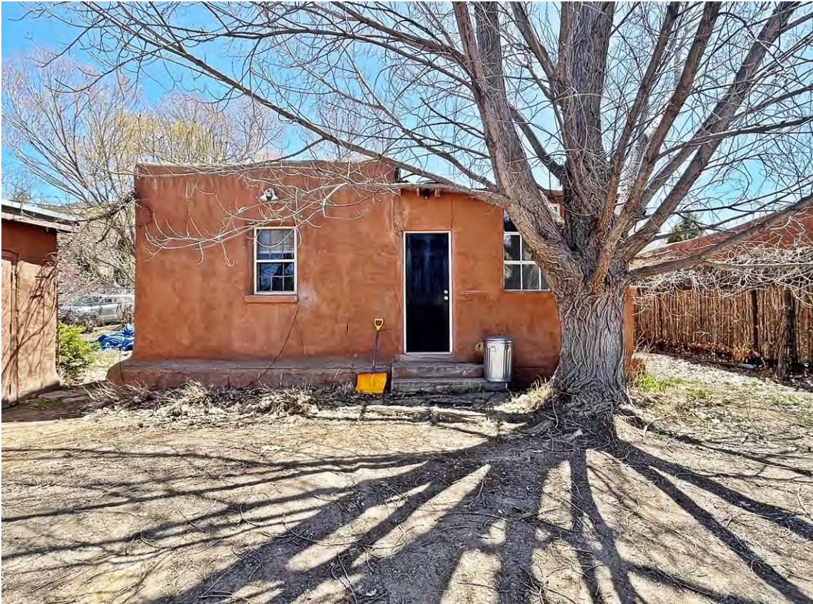
Photo 5: North elevation. Camera facing south.
