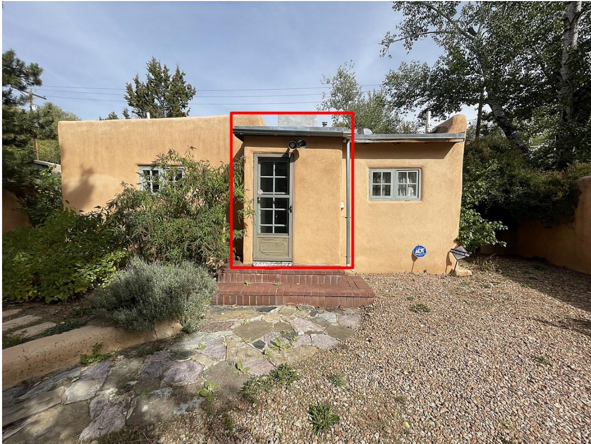
Photo 8: West elevation. Enclosed porch highlighted. Camera facing northeast.
