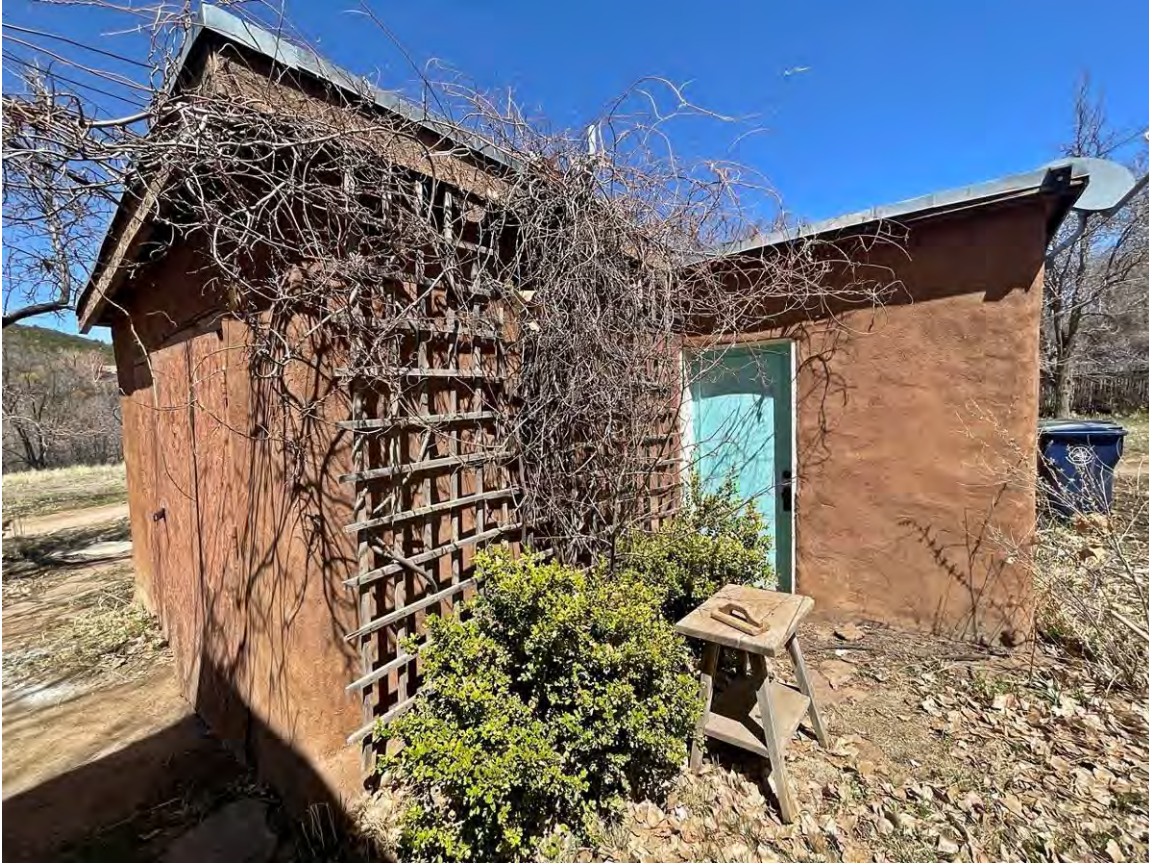
Photo 9: West elevation. Camera facing northeast.
