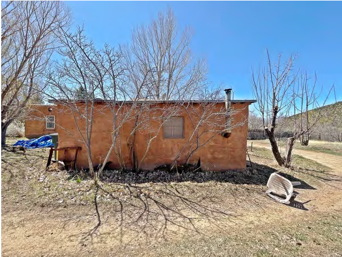
Photo 11: East elevation. Camera facing west.
