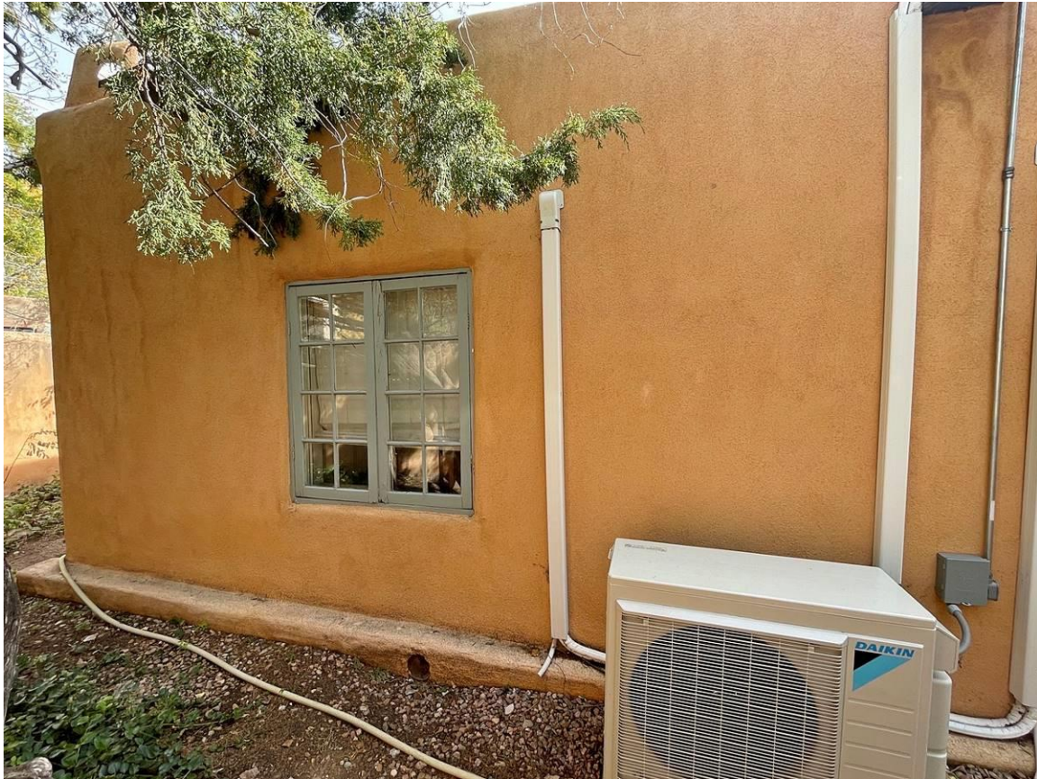
Photo 11: North elevation, northeast corner. Camera facing southeast.
