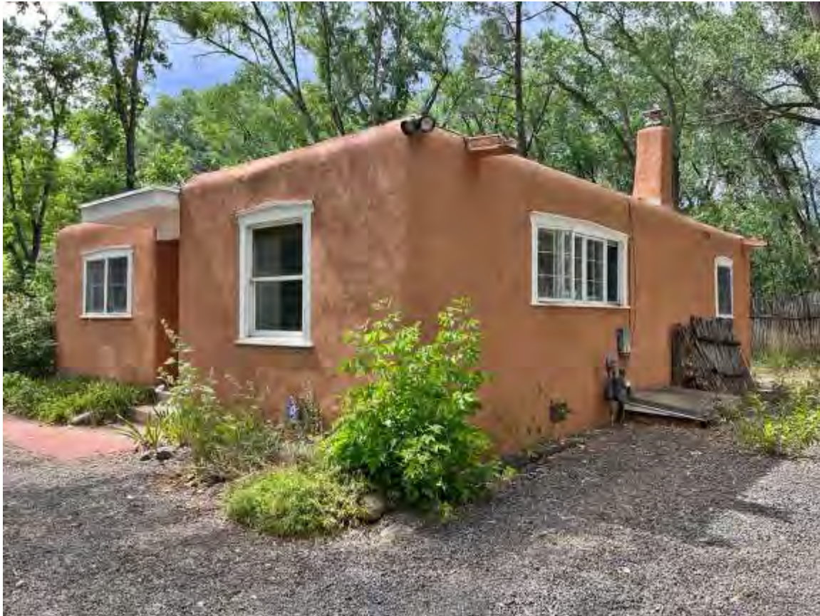
Photo 7: South and east elevations. Camera facing northwest.
