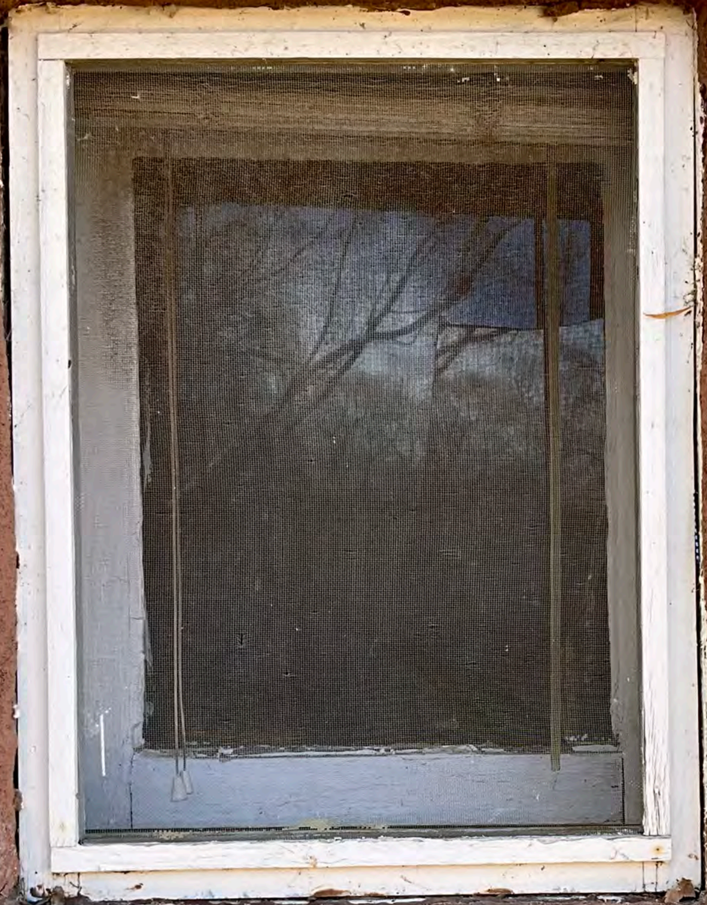
East Elevation Window C
