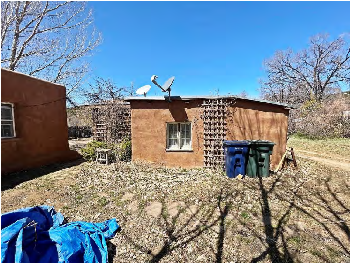
Photo 12: South elevation. Camera facing north.
