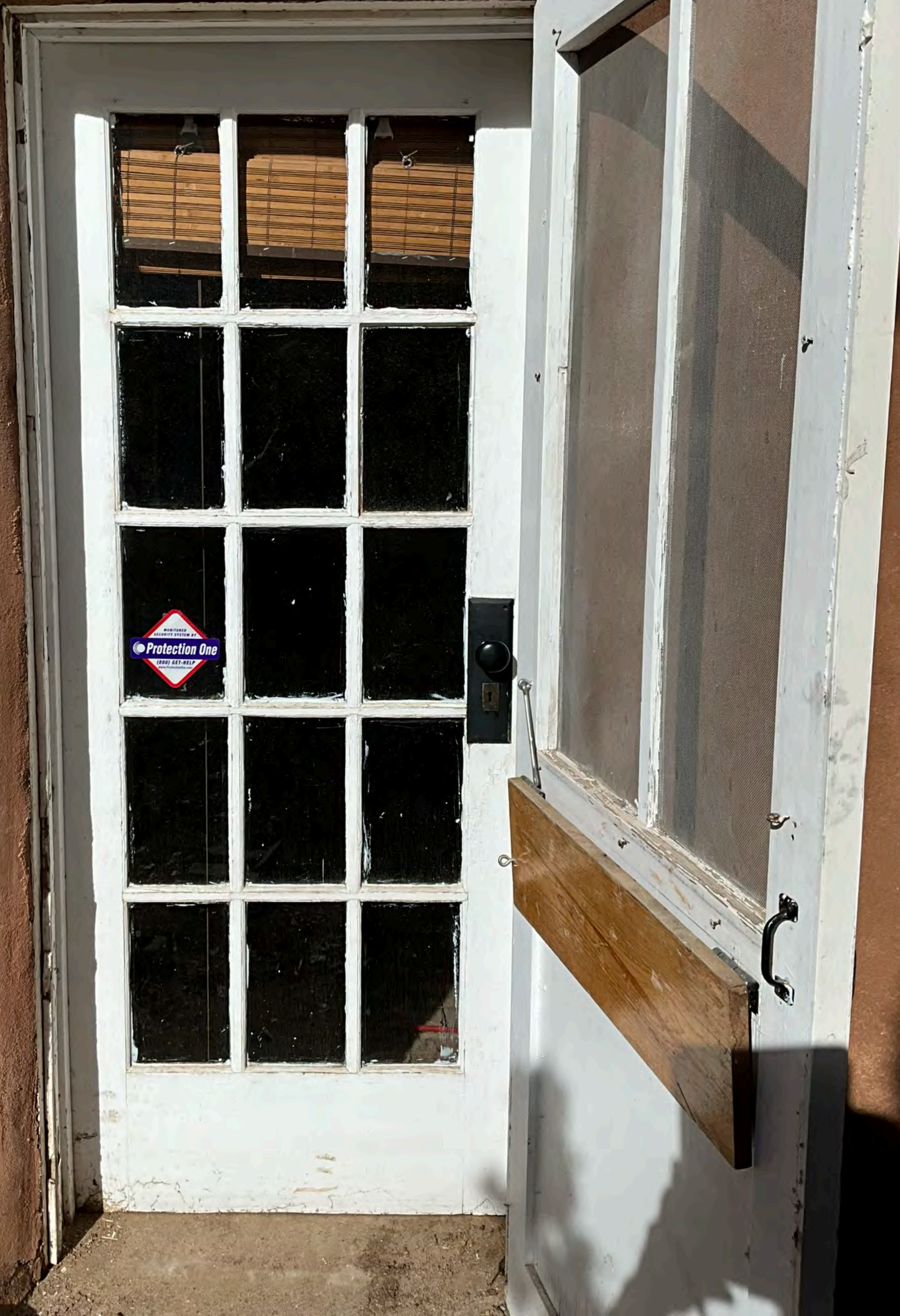
South Elevation Door #1
