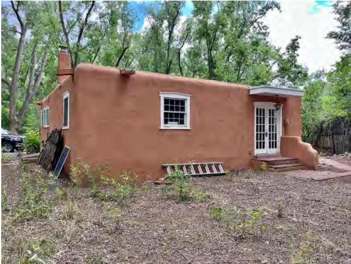
Photo 9. North elevation. Camera facing southwest.
