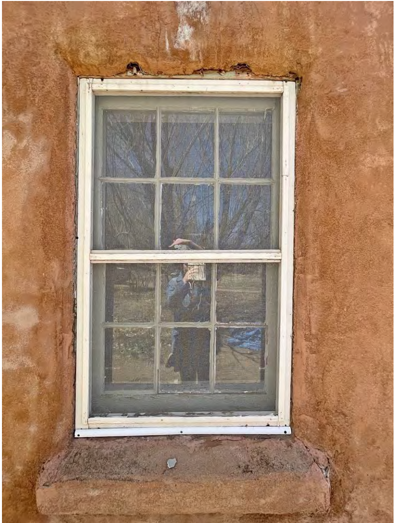
Photo 3: Typical window with extended sill. East elevation. Camera facing west.
