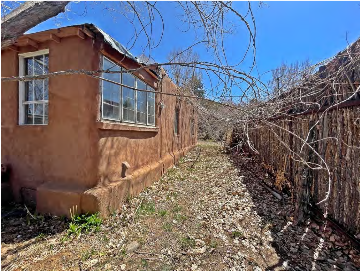
Photo 7: West elevation. Camera facing southeast.
