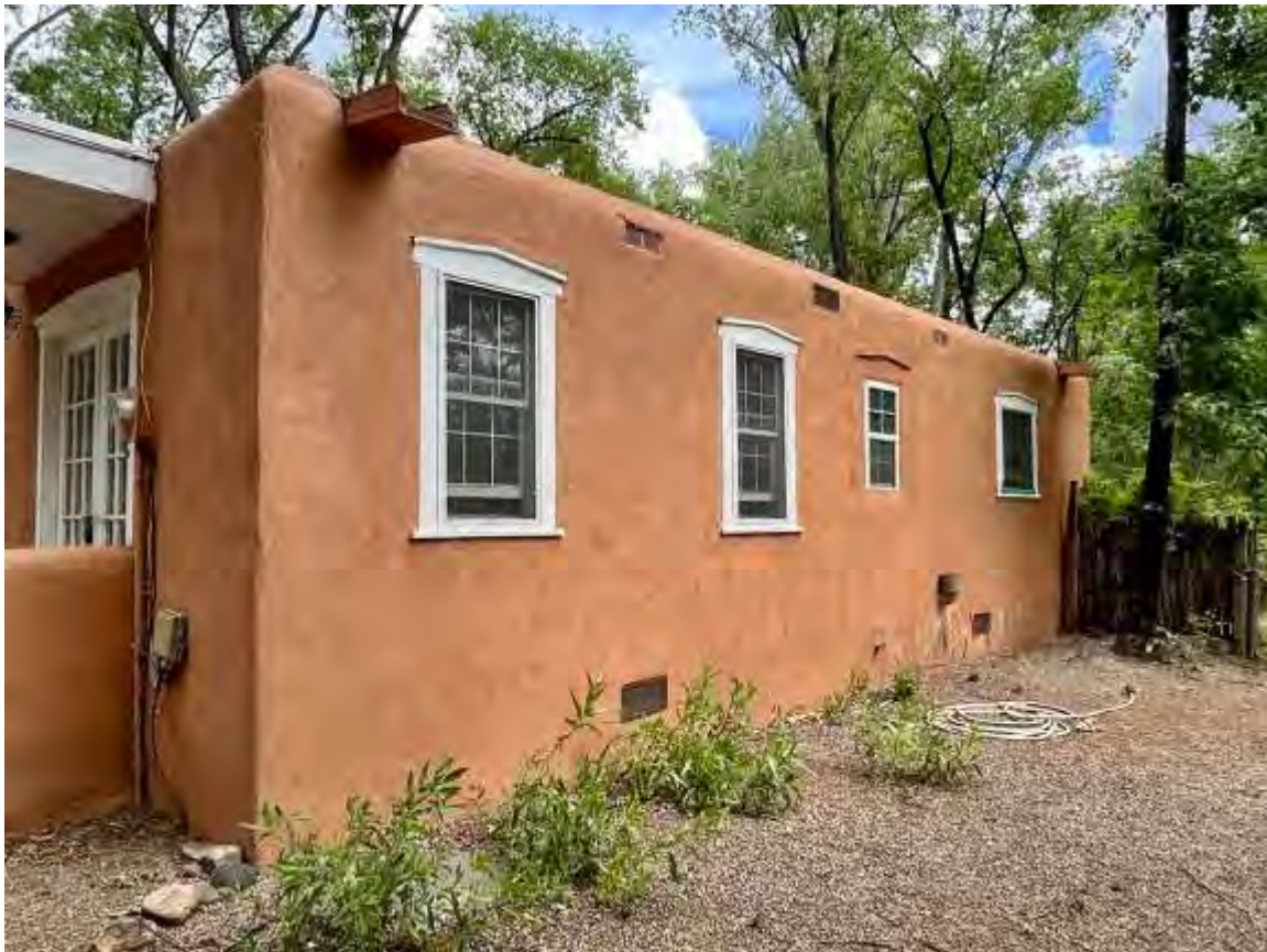
Photo 10: West elevation. Camera facing southeast.
