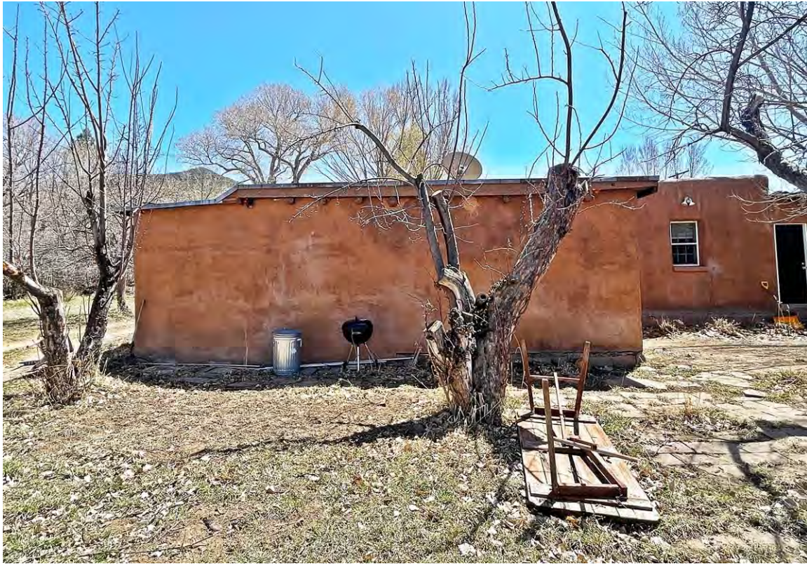
Photo 10: North elevation. Camera facing south.
