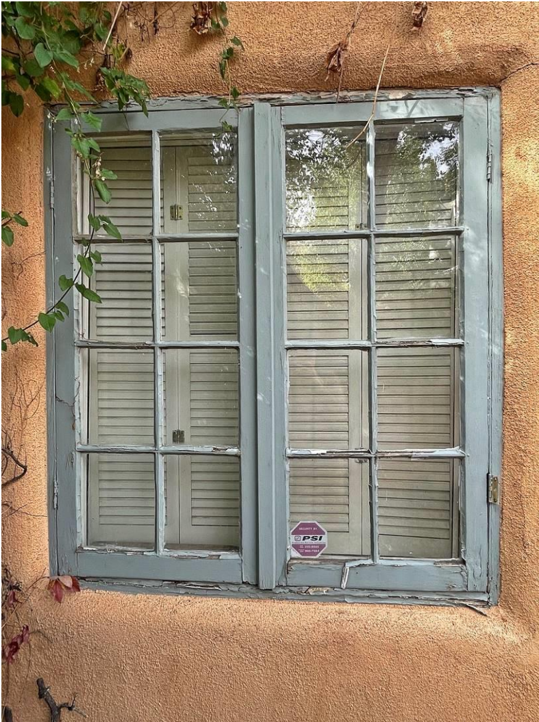
Photo 6: South elevation. Older casement window.
