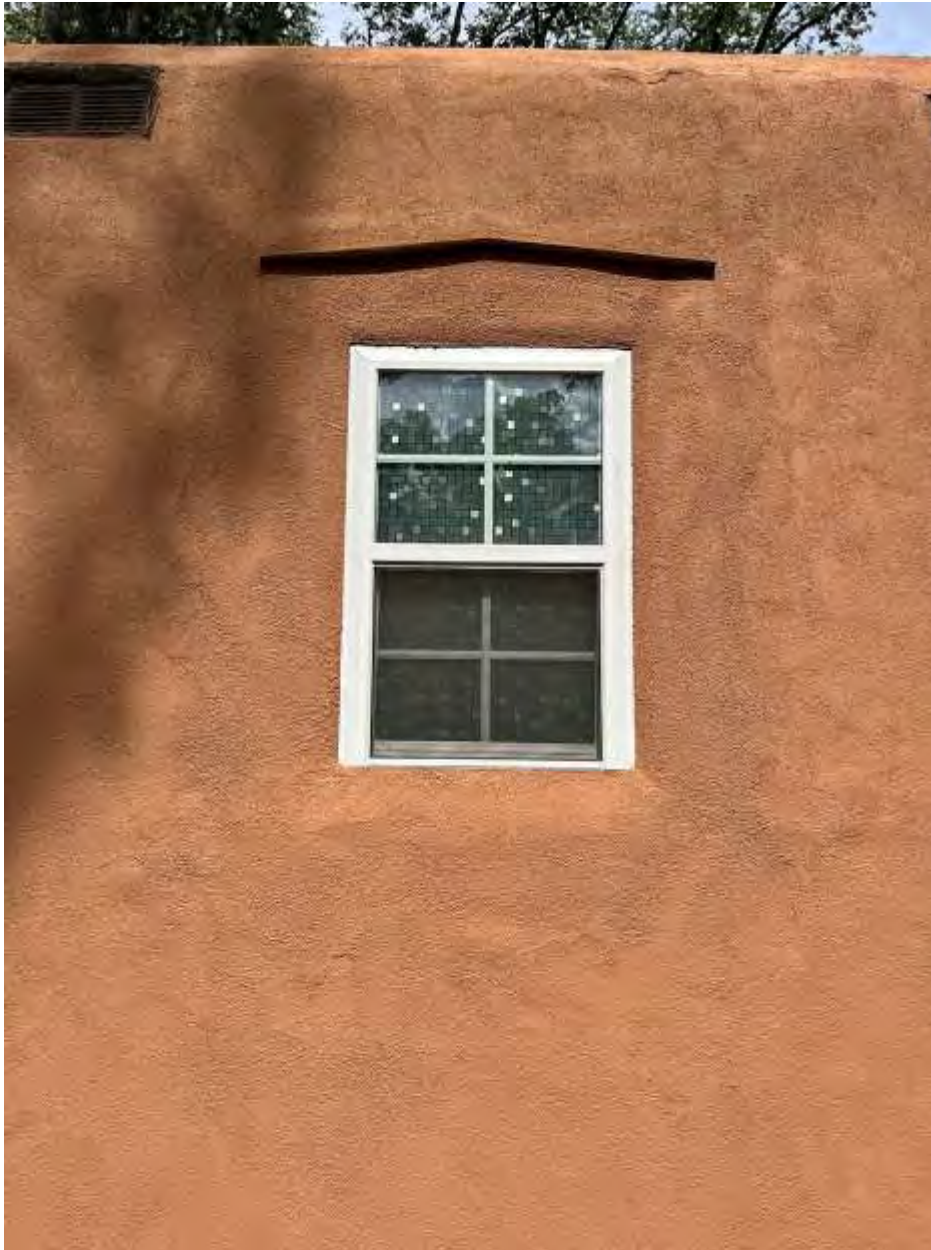
Photo 11: West elevation, replacement window at bathroom. Camera facing east.
