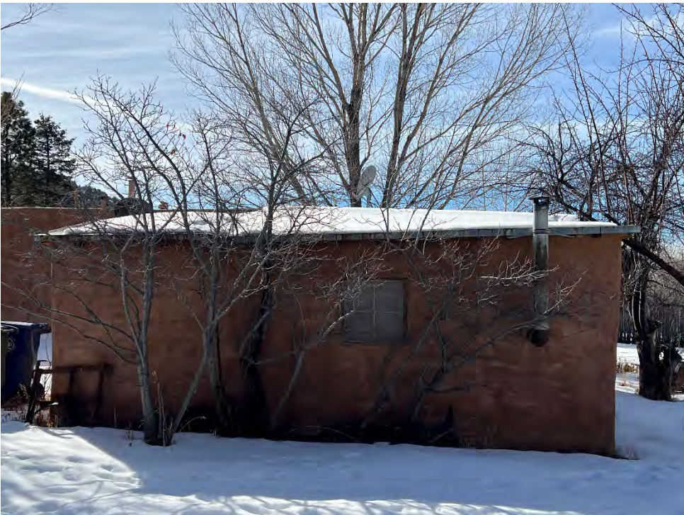
East Side – Shed / Garage Elevation
