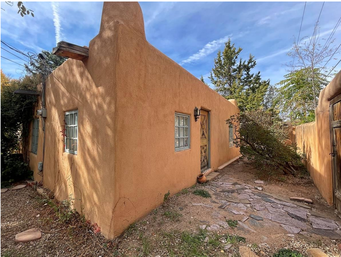
Photo 2: East oblique angle. Camera facing northwest.
