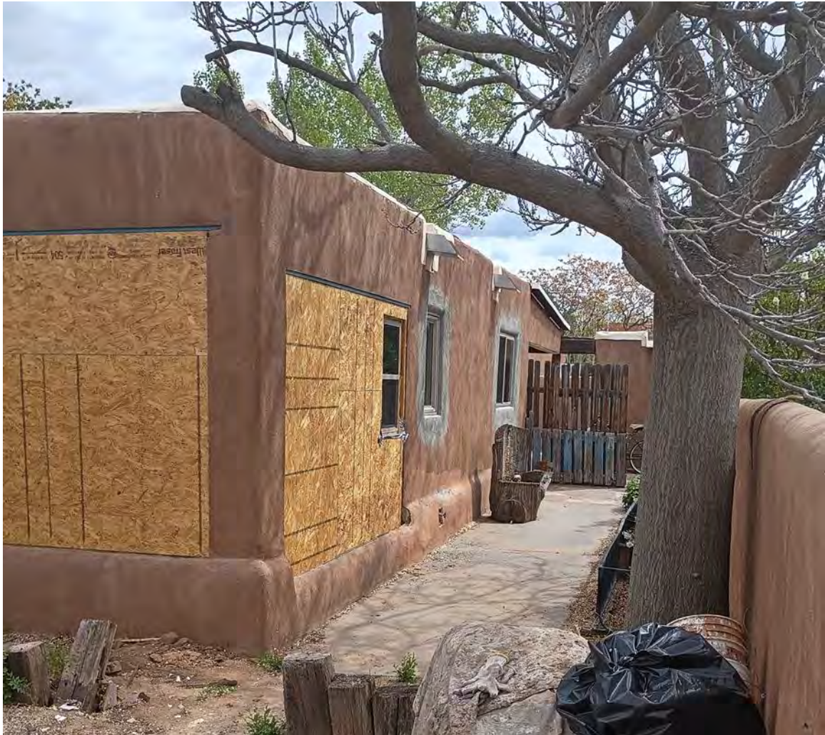
Photo 10: West elevation. Camera facing southeast.
