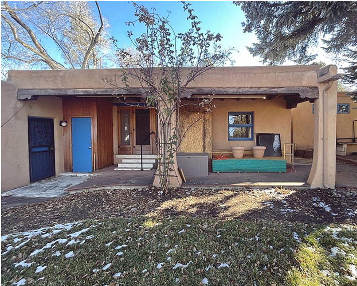
Photo 11: West elevation. Portal erected in 1958. Camera facing east.
