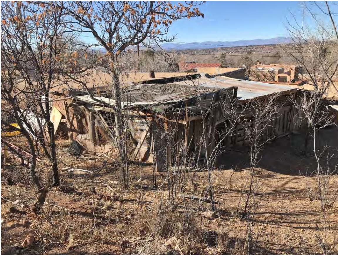
Photo 12: Shed, east elevation. Camera facing northwest.
