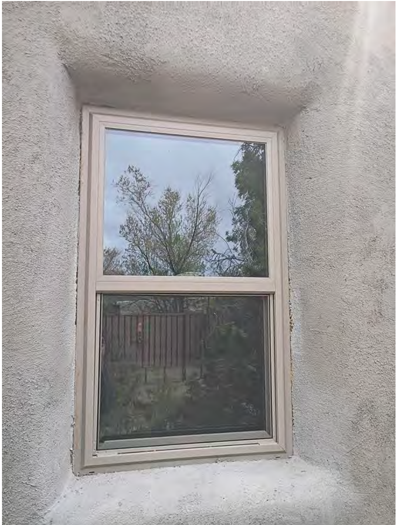
Photo 8: North façade, replaced window. Camera facing southwest.
