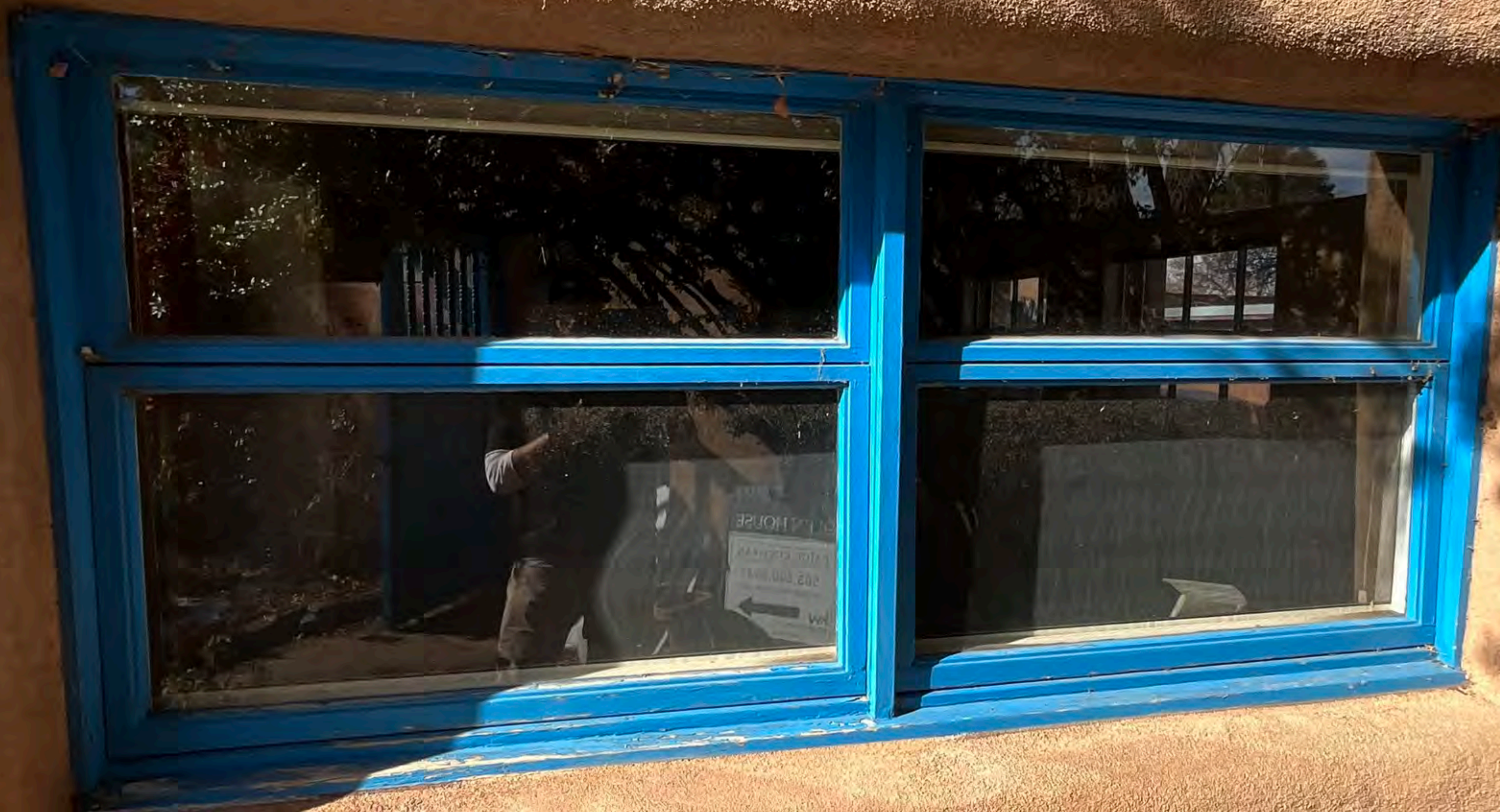
East Elevation Window W14
