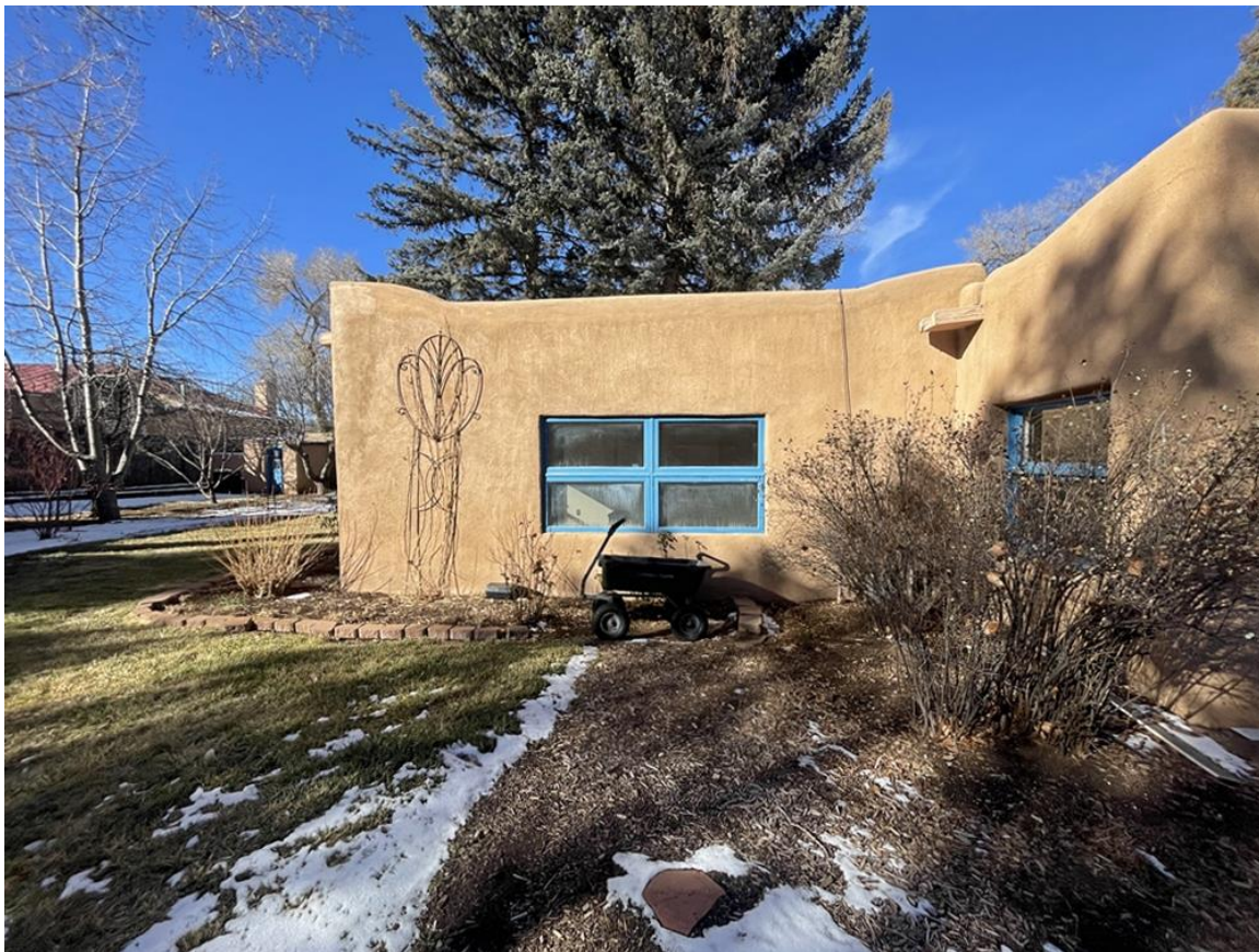
Photo 7: East elevation. 1992-93 addition. Camera facing west.
