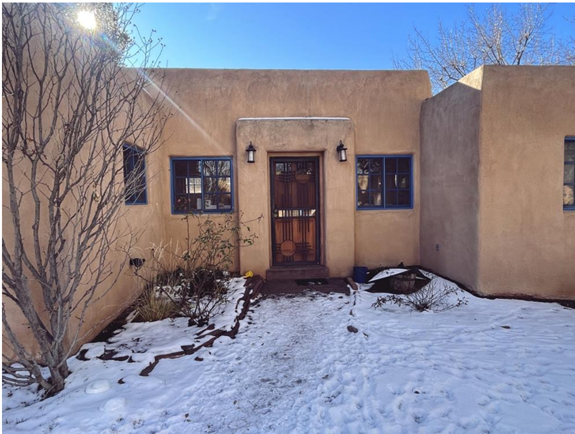
Photo 18: 1992-93 Guesthouse. North elevation. Camera facing south.
