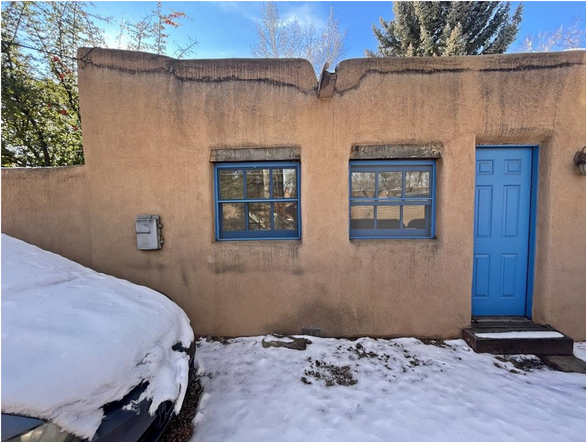
Photo 14: North elevation. Change of fenestration after 1992. Camera facing south.
