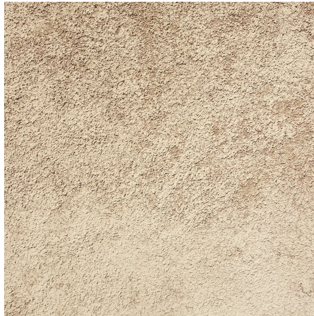
Historic House Existing Stucco Repair
