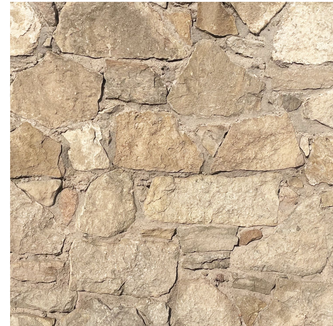
Historic Existing Stone Wall
