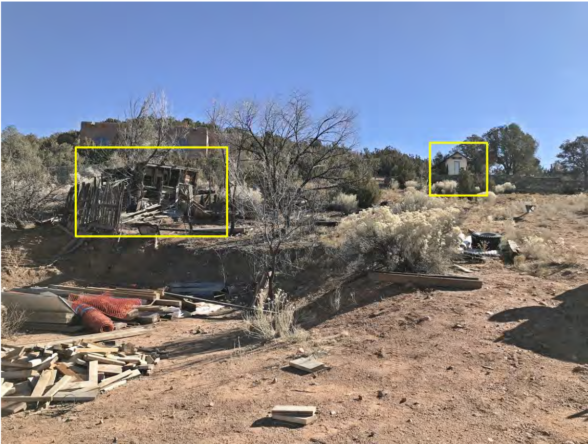
Photo 2: Deteriorating structure and capilla on separate property. Camera facing southeast.
