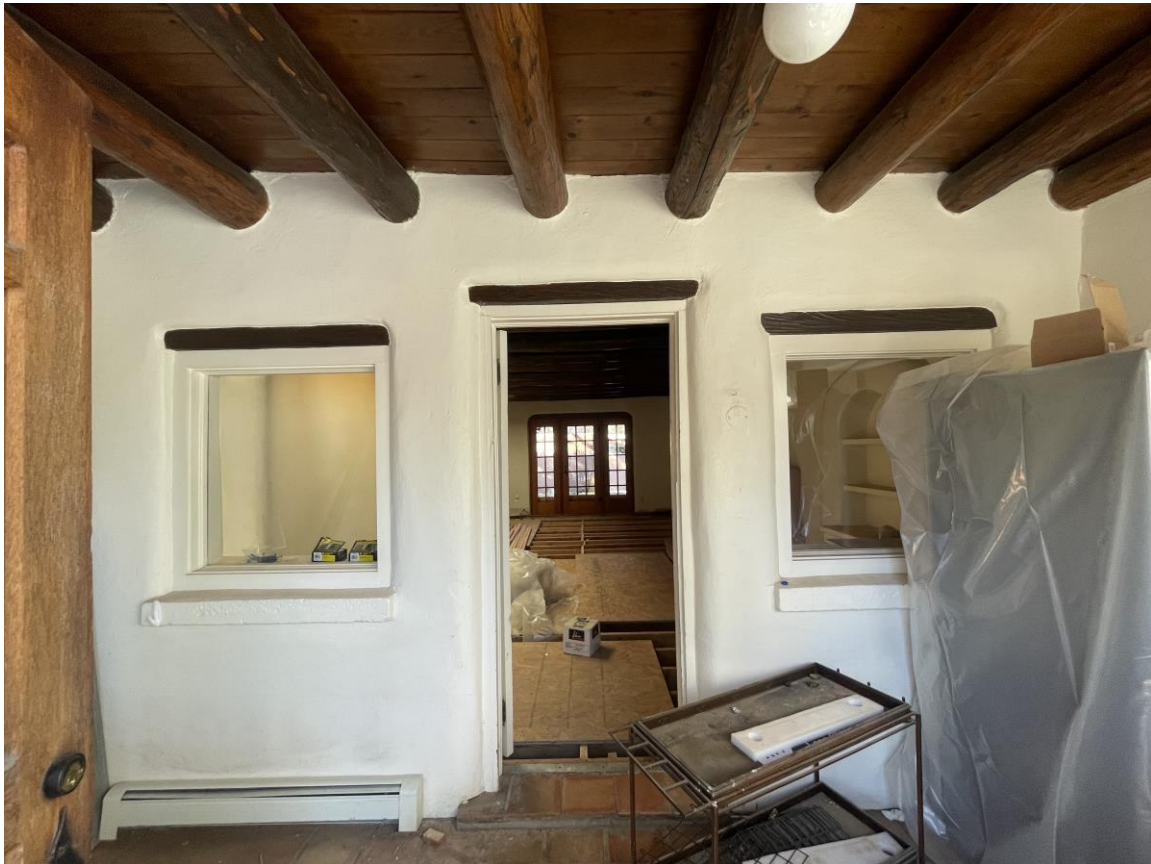
Photo 4: East Elevation. Interior of east entry hall. Camera facing west.
