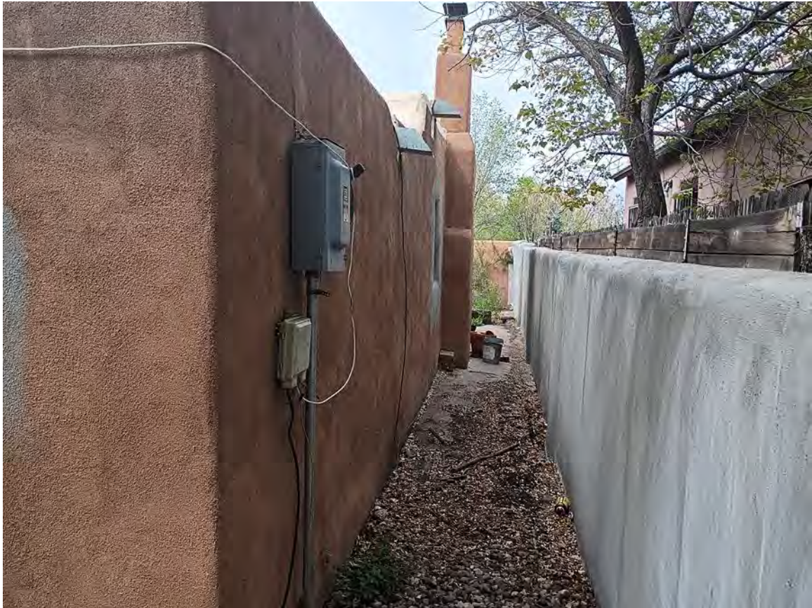
Photo 15: East elevation. Camera facing north.
