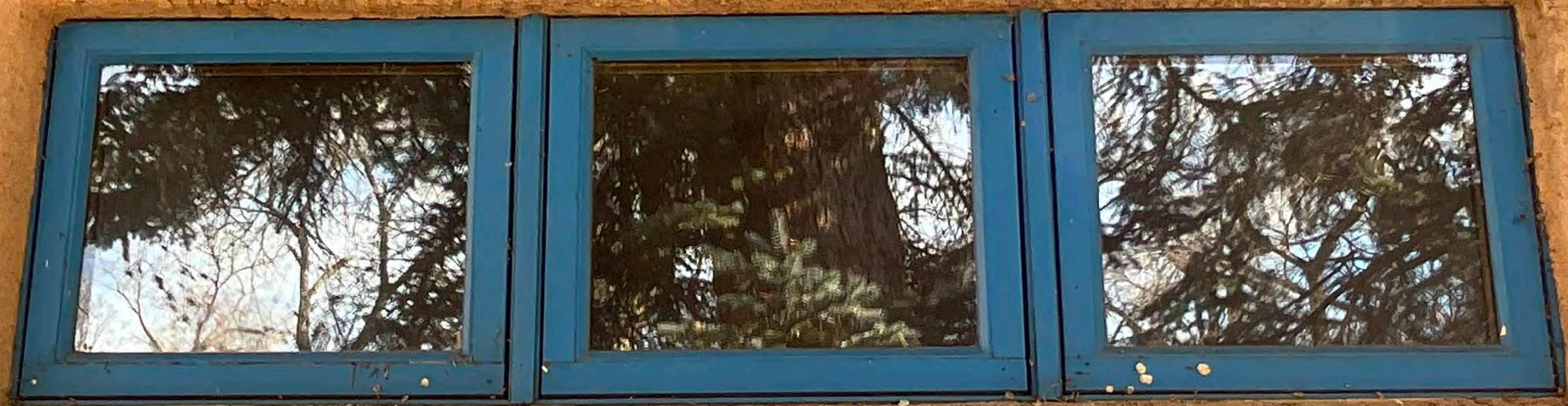
West Elevation Window W06
