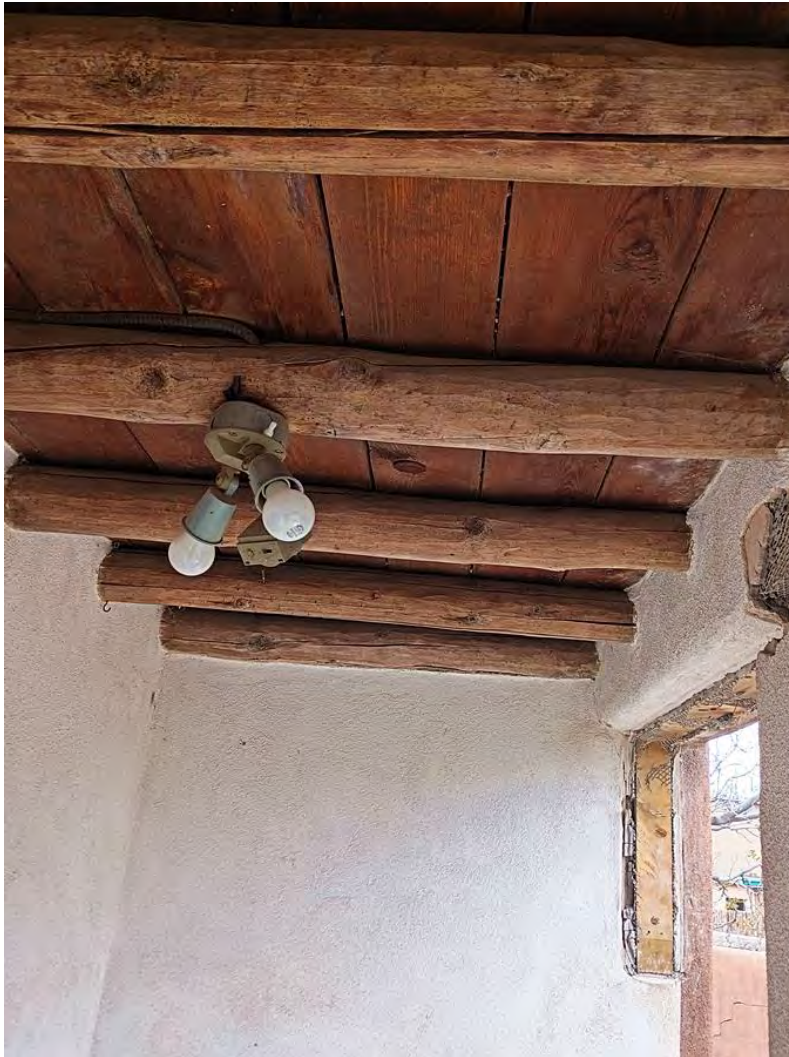
Photo 4: North façade entry portal, decking. Camera facing up.
