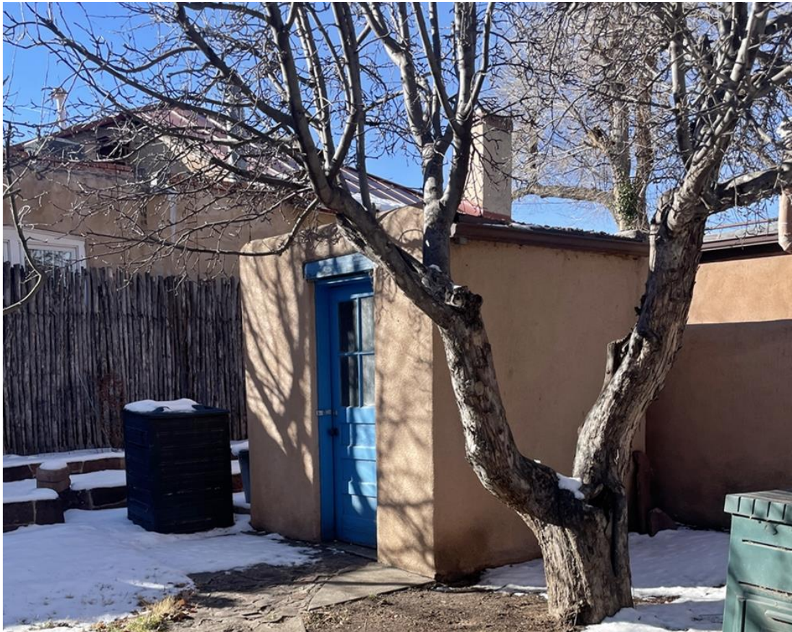
Photo 19: Shed. Camera facing southwest.
