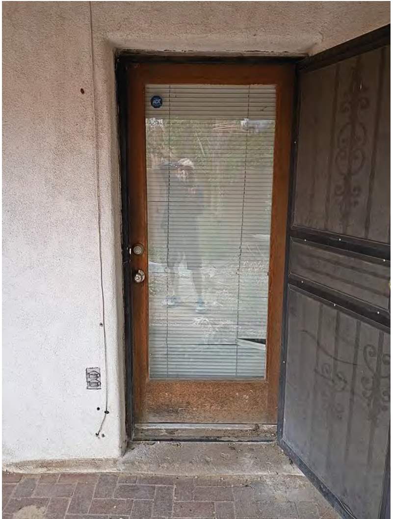
Photo 15: South elevation entry door. Camera facing north.
