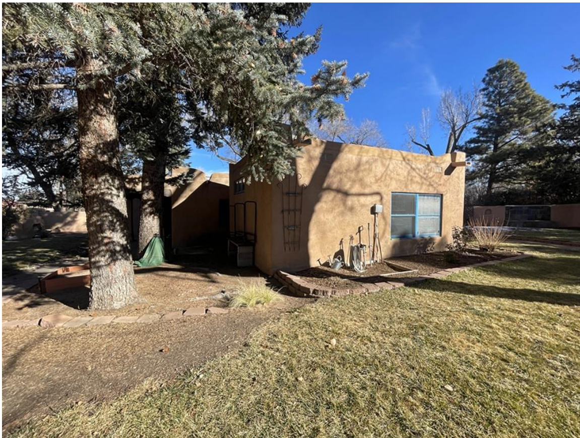
Photo 8: South elevation. 1992-93 addition. Camera facing northeast.
