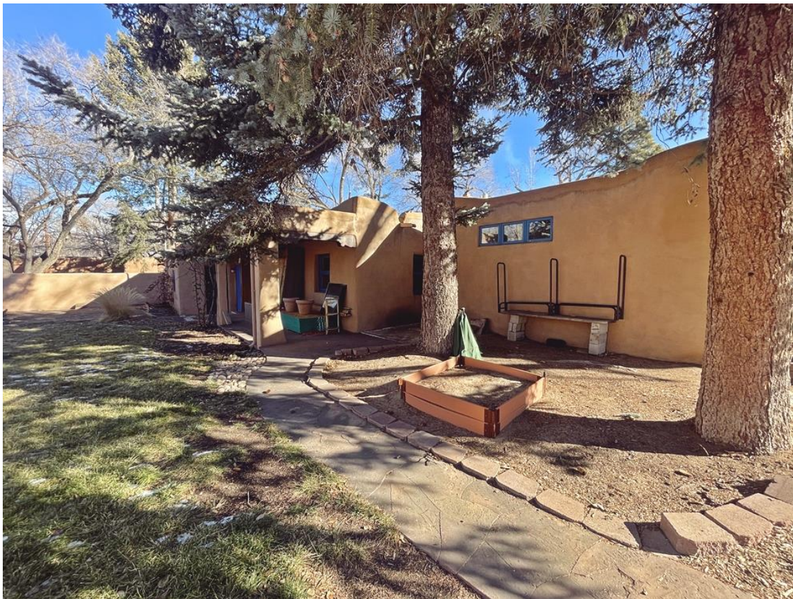
Photo 9: West elevation. 1929-30 addition at right. Camera facing northeast.
