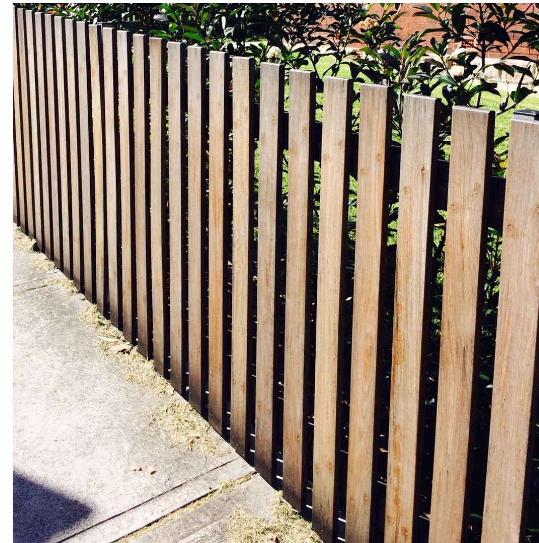
Wood Picket Fence & Guardrail
