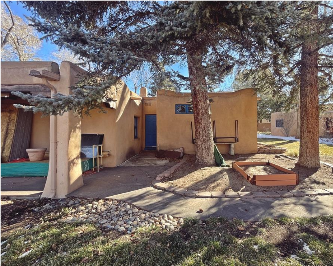
Photo 10: West elevation. Passageway between original building and 1992-93 addition. Camera facing east.
