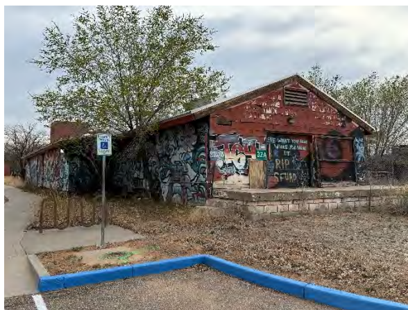
Brunn's Barracks Building
