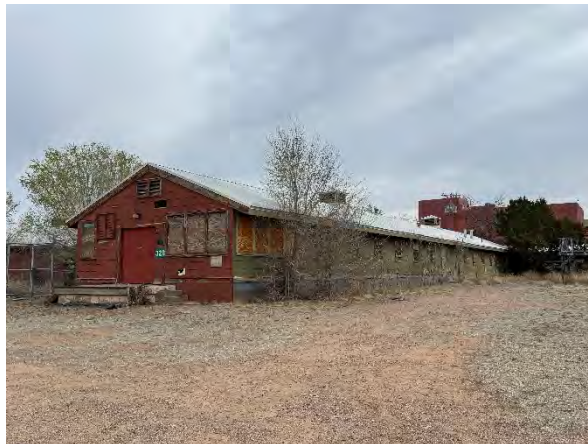
Brunn's Barracks Building
