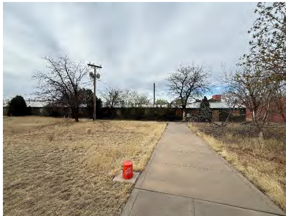
Brunn's Barracks Building
