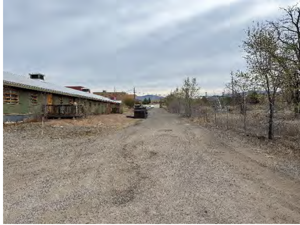
Brunn's Barracks Building
