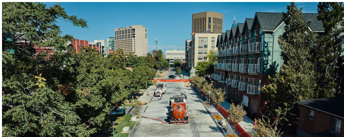
Rebuild Old Boise Blocks project: Grove Street in Boise between 4th Street and 5th Street, looking west.
