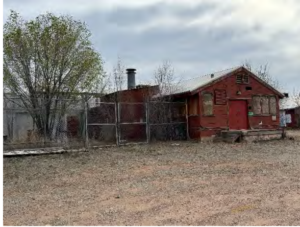
Brunn's Barracks Building
