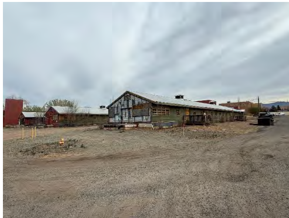
Brunn's Barracks Building
