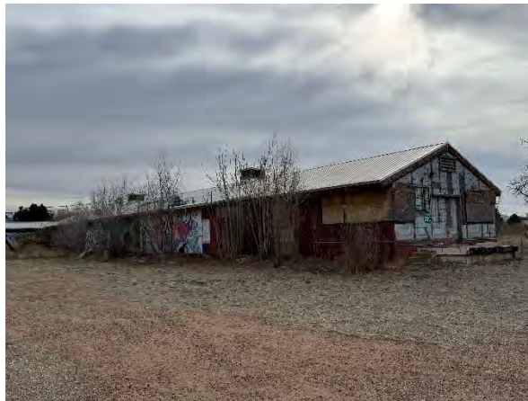
Brunn's Barracks Building
