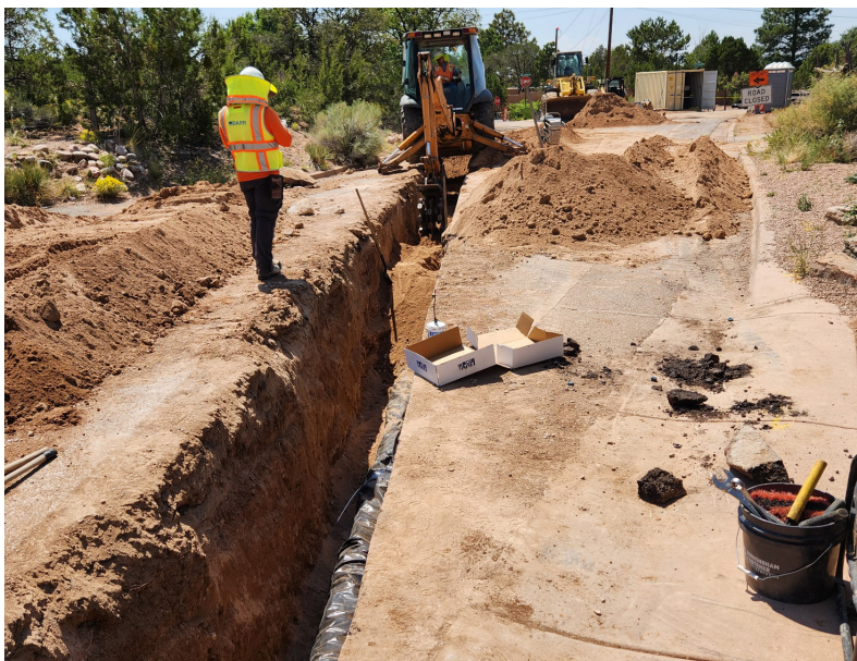
> Contractor replacing pipe on Garcia Street as part of the priority line replacement project.
