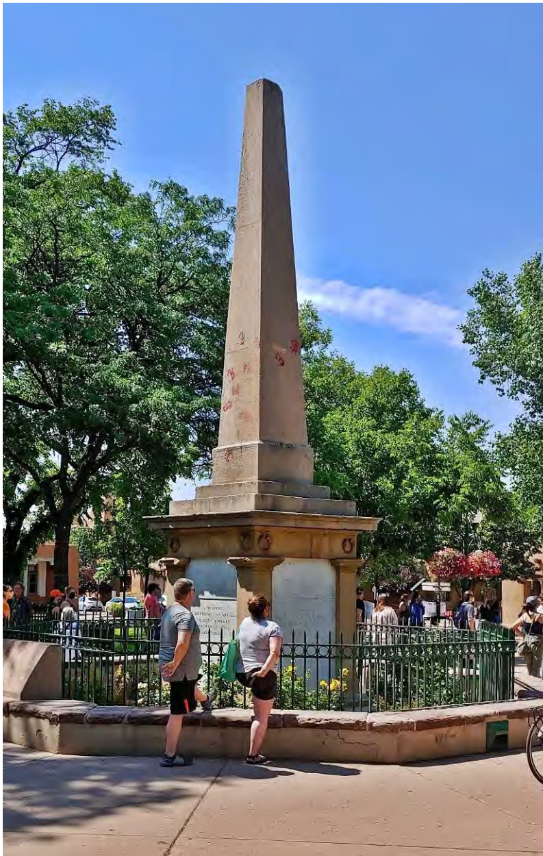
Photo 11: South and east elevations. Camera facing northwest. June 20, 2020.
