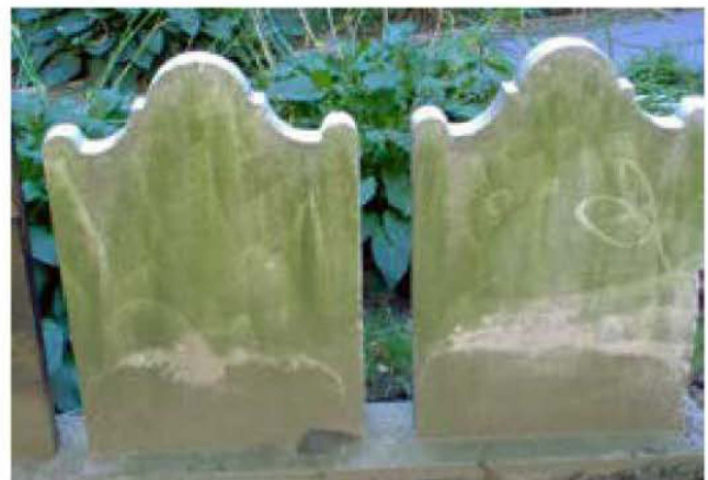
Figure 14. High-pressure water washing can damage grave markers. The photograph shows "wand marks" on the headstones produced by inappropriate pressure washing. Photo: Jason Church.
