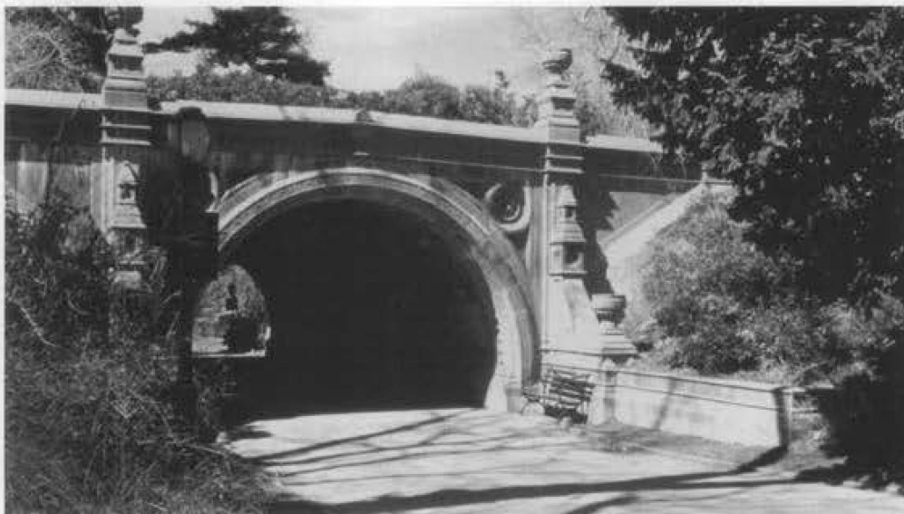
Figure 5. Constructed in 1868 of Beton Coignet, the Cleft Ridge Span in New York City's Prospect Park is one of the earliest extant cast stone structures in the United States.
