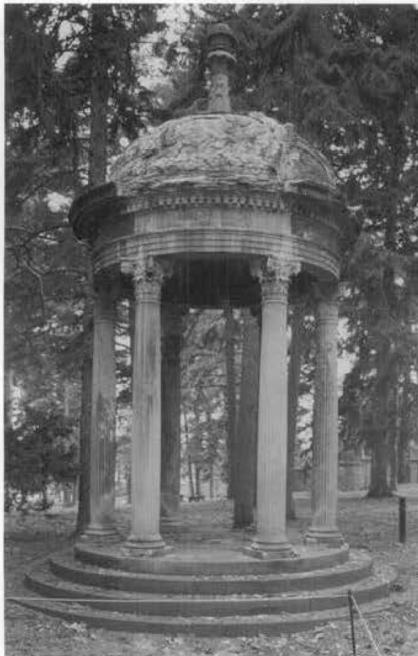
Figure 10. Scaling of cast stone units signals problems with the cementing mix and method of manufacture. Serious deterioration of cast stone, such as this, warrants replacement.
