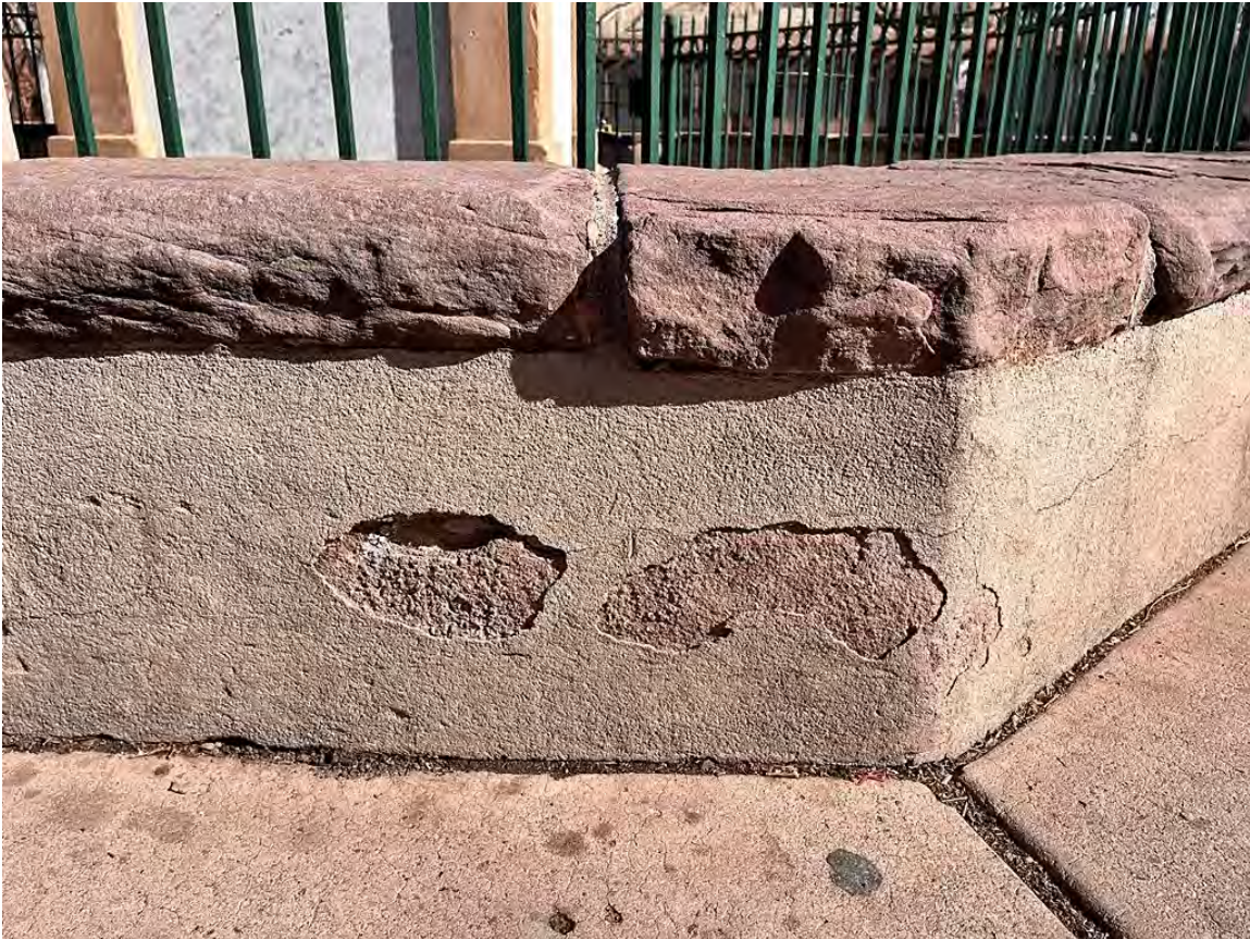
Photo 4: Seating wall. South elevation. Camera facing north. March 14, 2025.
