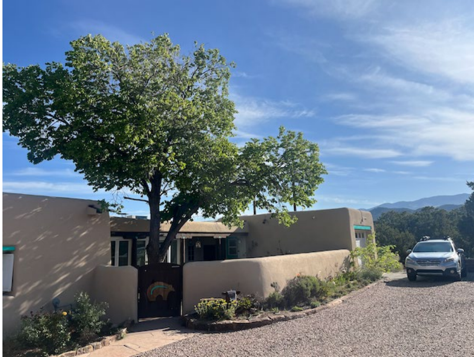
View of west side of garage. Two windows are proposed on this façade.
