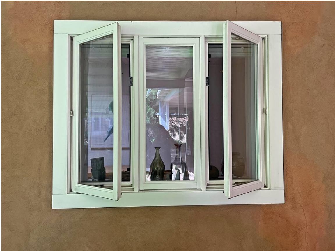
Photo 12: Wing. East elevation. Fenestration. Camera facing west.
