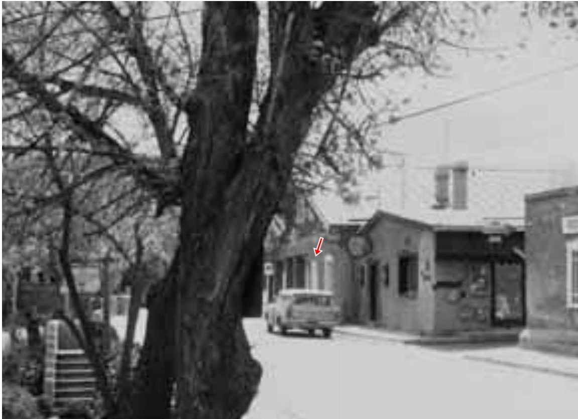
Figure 11: Crop and blowup of 1983 photograph showing presence of west door or window (arrow).
