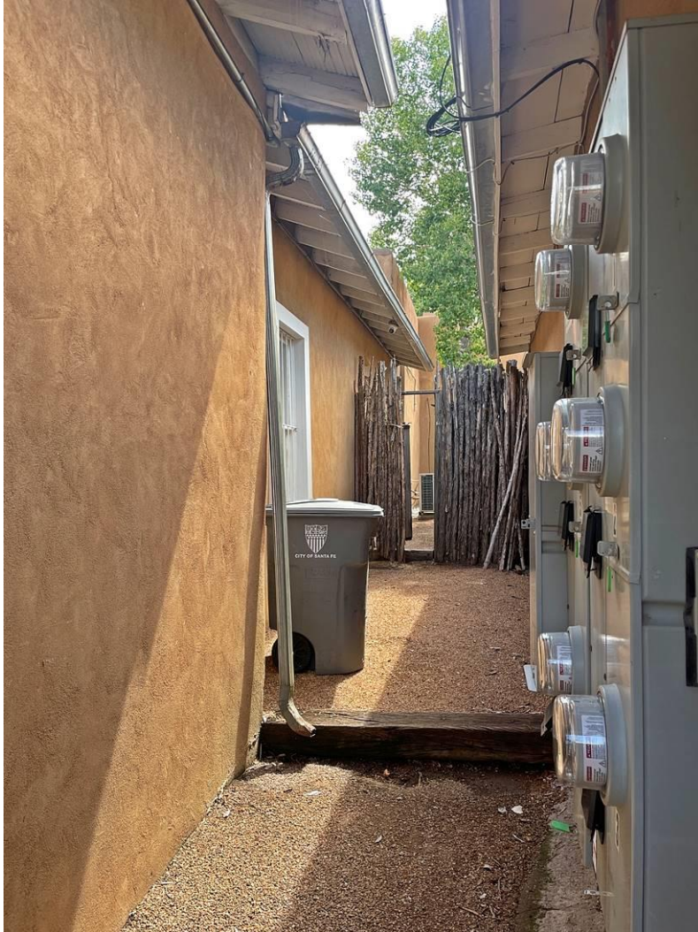
Photo 9: West elevation. Camera facing south.
