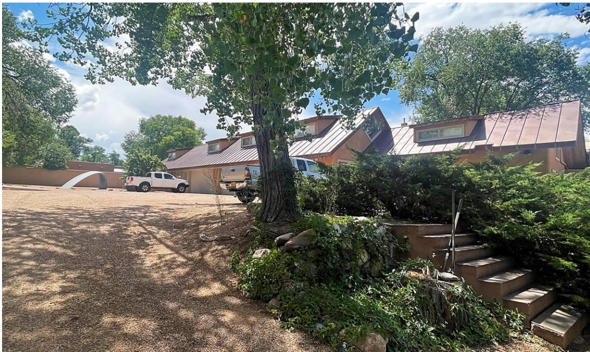
Photo 2: 1980s Back Building. Camera facing southwest.
