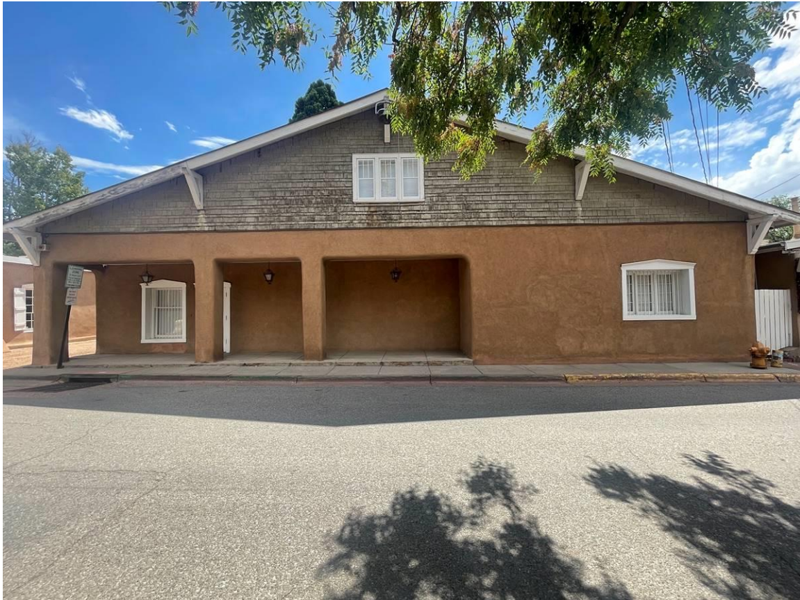
Photo 3: Front Building. North façade. Camera facing south.
