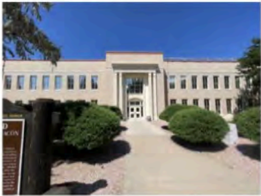
30. Bataan Memorial Building - 1/8" bullnose
