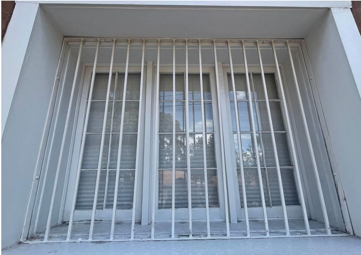
Photo 4: North elevation. West window. Camera facing up.
