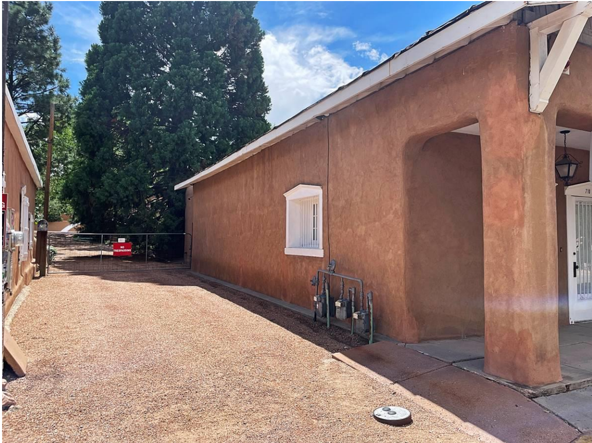
Photo 6: East elevation. Camera facing southwest.
