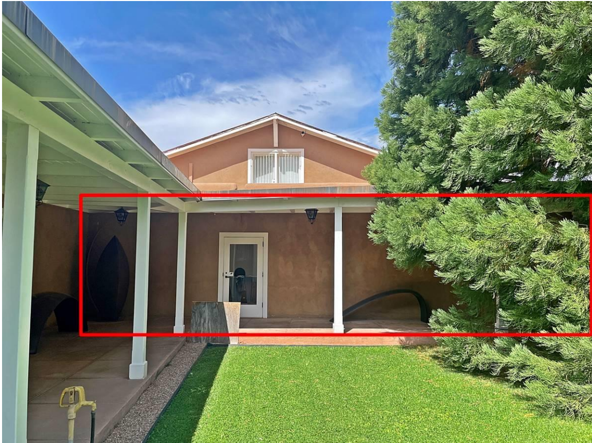
Photo 8: South elevation. c.1967 addition highlighted. Camera facing north.
