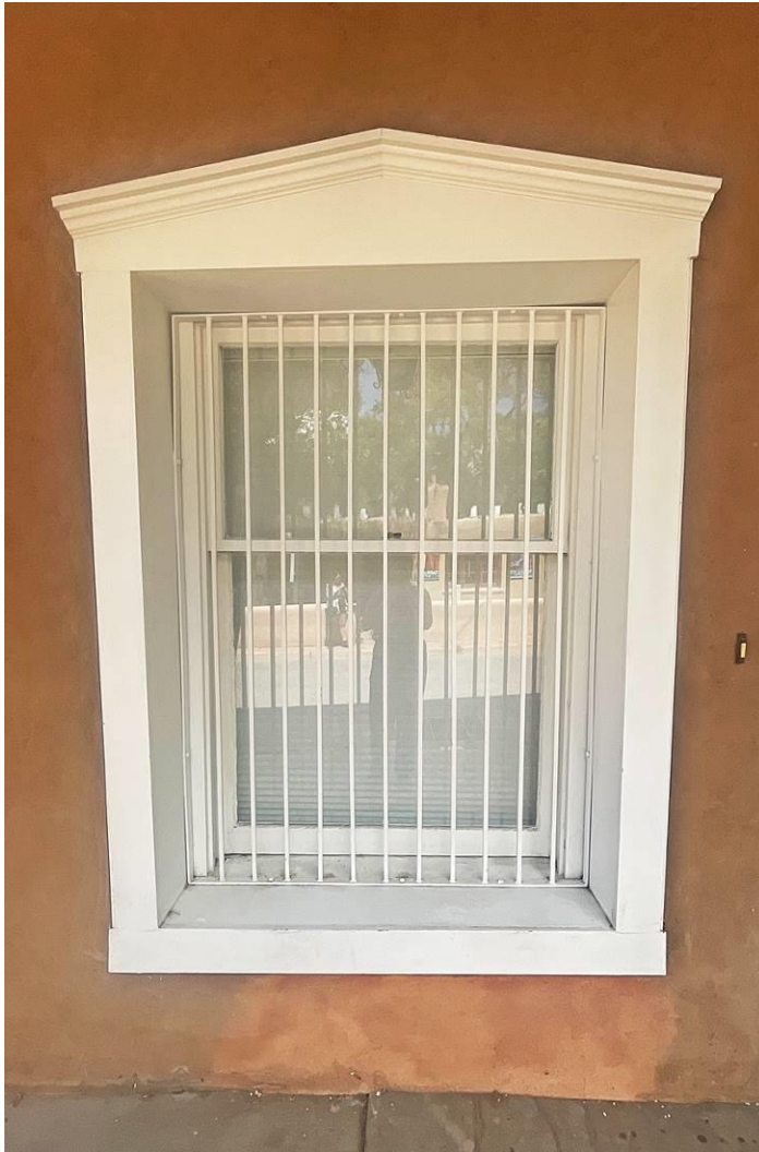
Photo 5: North elevation. East window. Camera facing south.
