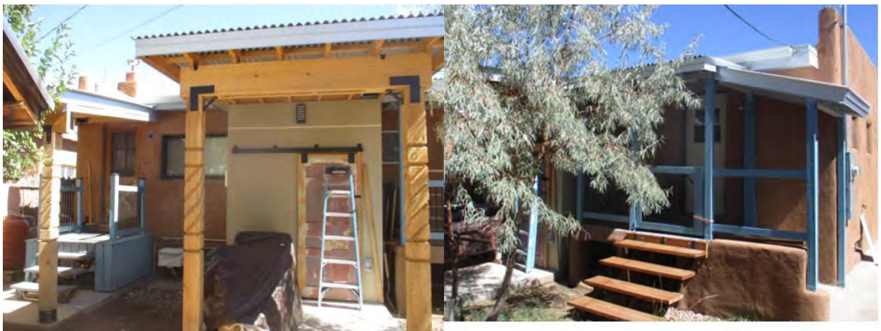
Figure 3: Image of the three constructed portals on the west elevation.
