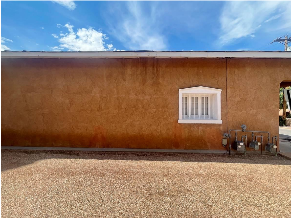
Photo 7: East elevation. Camera facing west.
