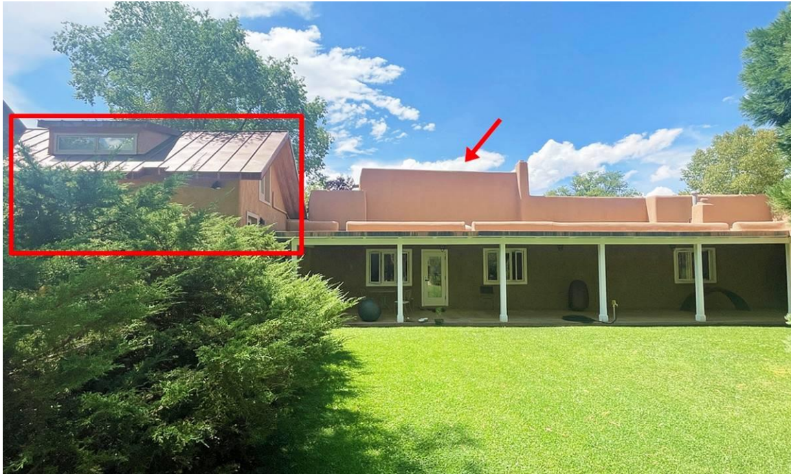
Photo 10: Wing. East elevation. 1980s building (highlighted); parapets of adjoining properties (arrow). Camera facing northwest.
