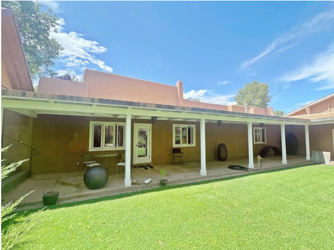
Photo 11: Wing. East elevation. Camera facing northwest.
