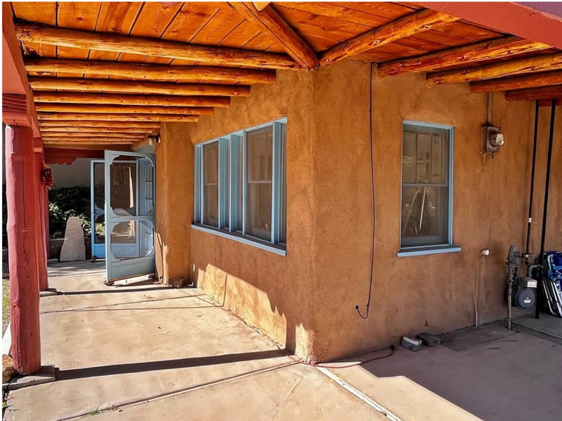
Photo 7: Southeast corner. Camera facing northwest.
