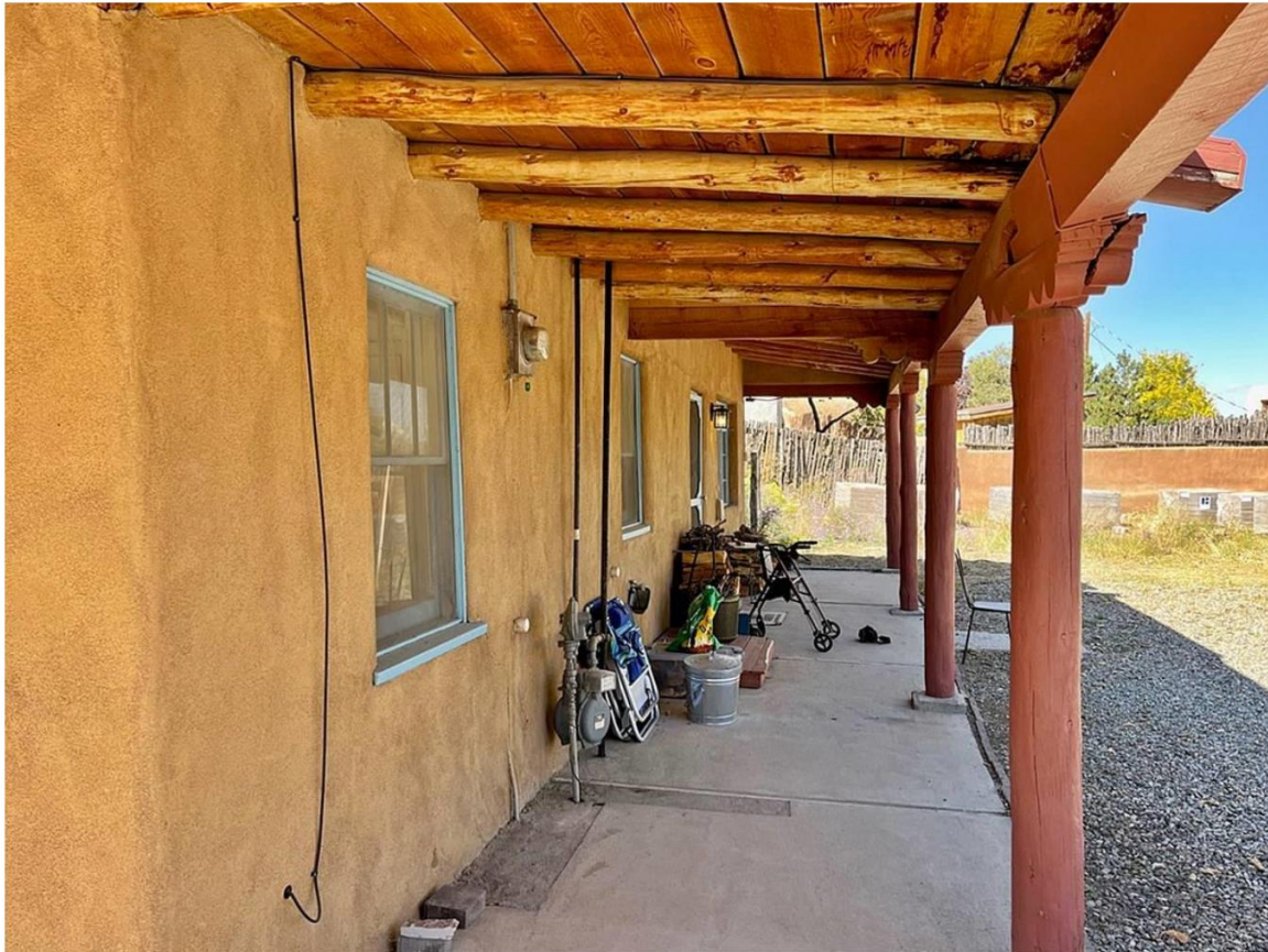
Photo 8: East elevation. Camera facing north.
