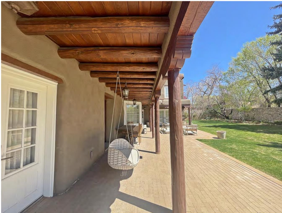
Photo 10: South elevation – portal. Camera facing east.
