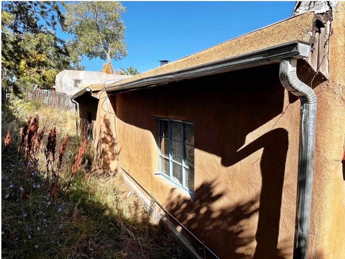
Photo 14: West elevation. Camera facing north.
