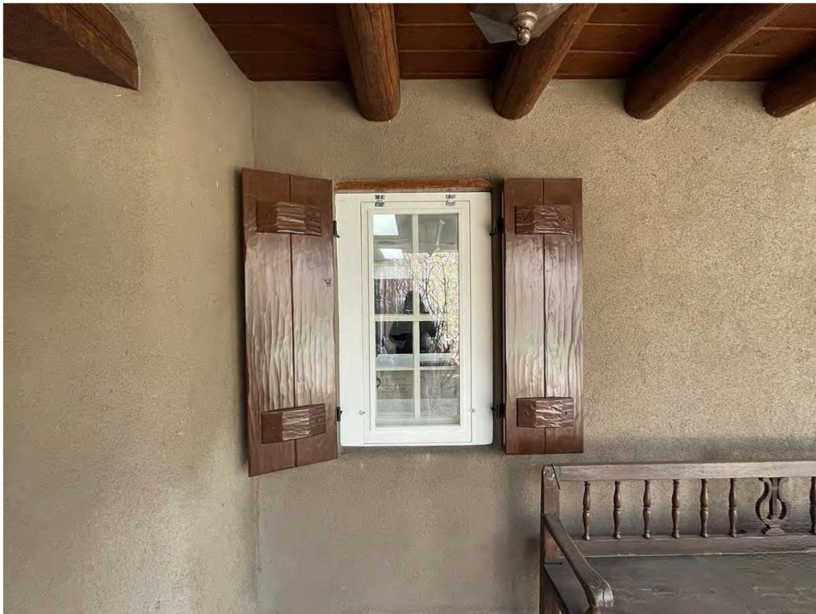
Photo 5: East elevation – window at portal. Camera facing west.
