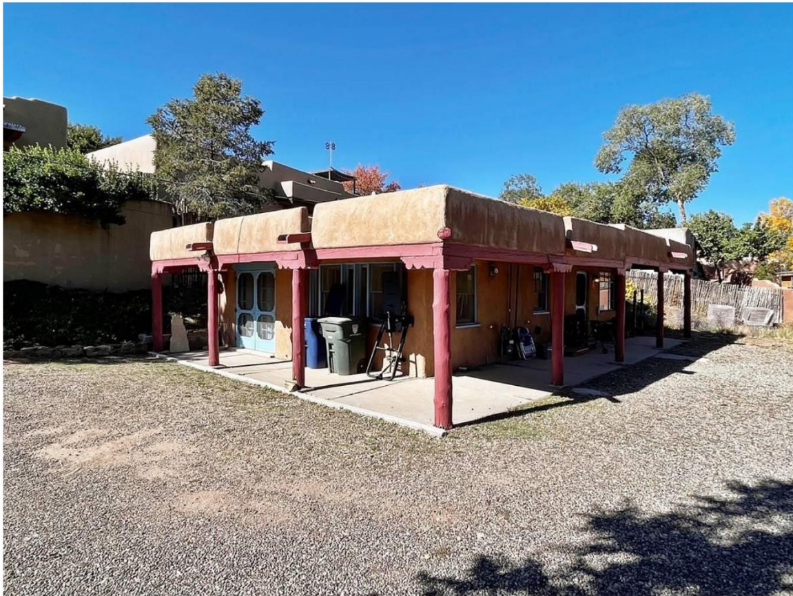
Photo 2: South and east elevations. Camera facing northwest.
