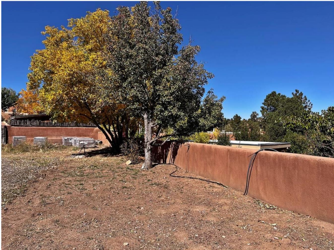
Photo 15: East yard wall. Camera facing northeast.
