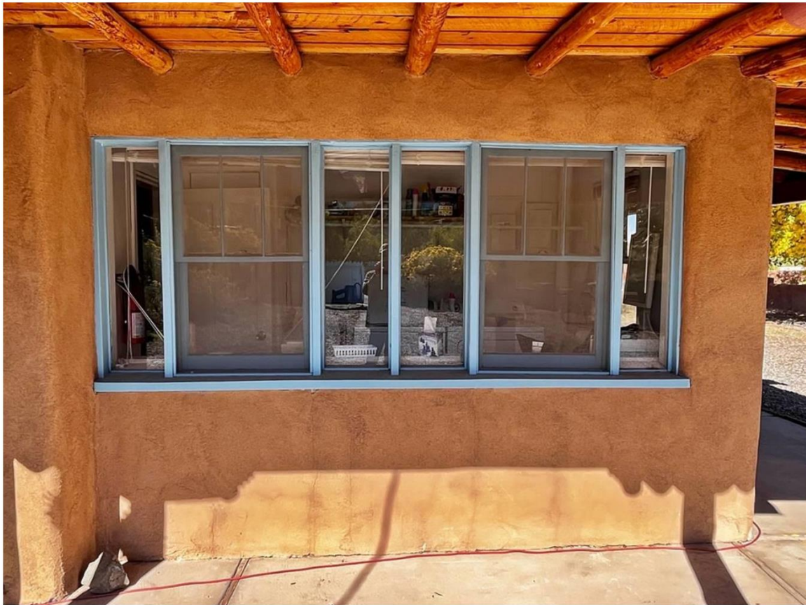
Photo 5: South elevation. Combination at laundry room. Camera facing north.
