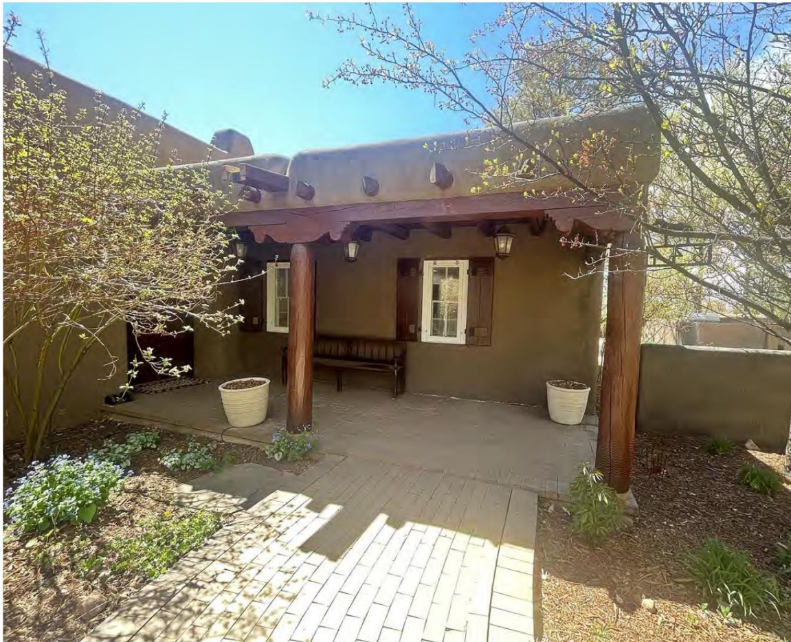
Photo 4: East elevation – entry portal. Camera facing southwest.
