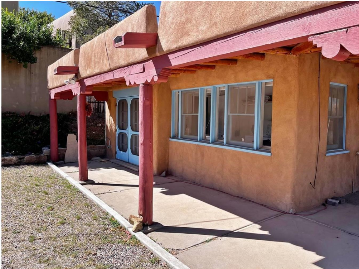
Photo 3: South elevation. Camera facing northwest.
