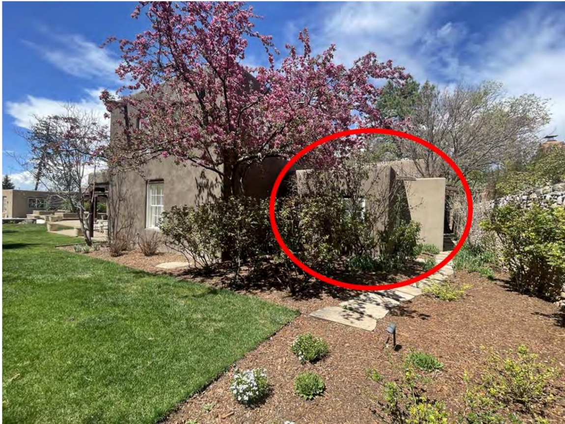
Photo 14: South elevation – 2012 bathroom addition. Camera facing northwest.
