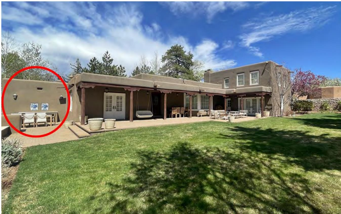
Photo 9: South elevation. Circled area indicates removal of fenestration. Camera facing northeast.
