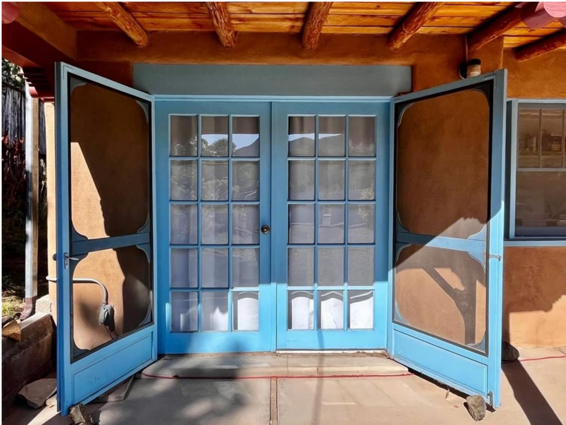
Photo 4: South elevation. Double doors at dining area. Camera facing north.
