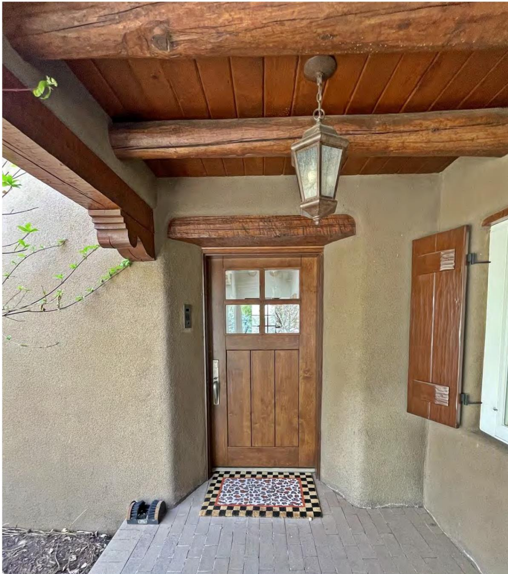
Photo 6: North elevation – entry door. Camera facing south.
