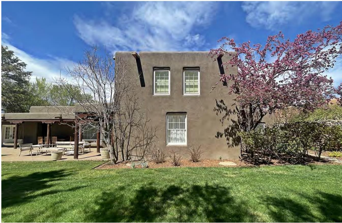
Photo 12: South elevation – bedroom suite. Camera facing north.
