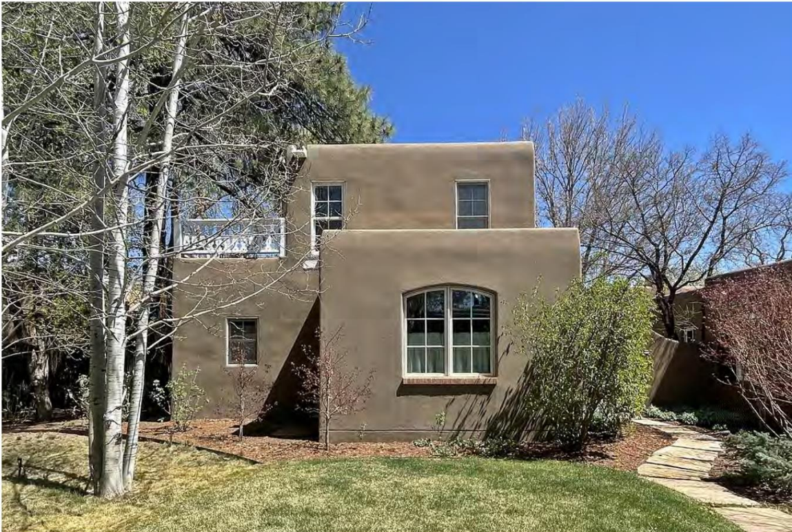
Photo 15: West elevation. Camera facing east.
