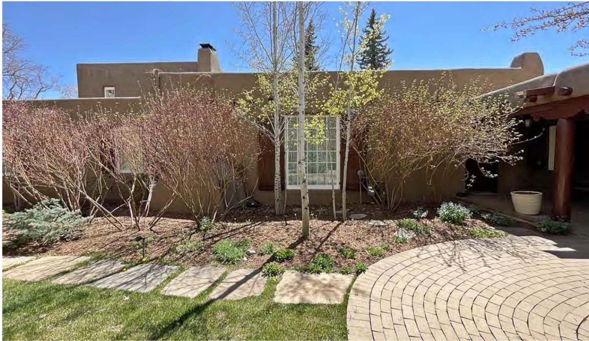
Photo 7: North elevation – 30-light window at living room. Camera facing south.
