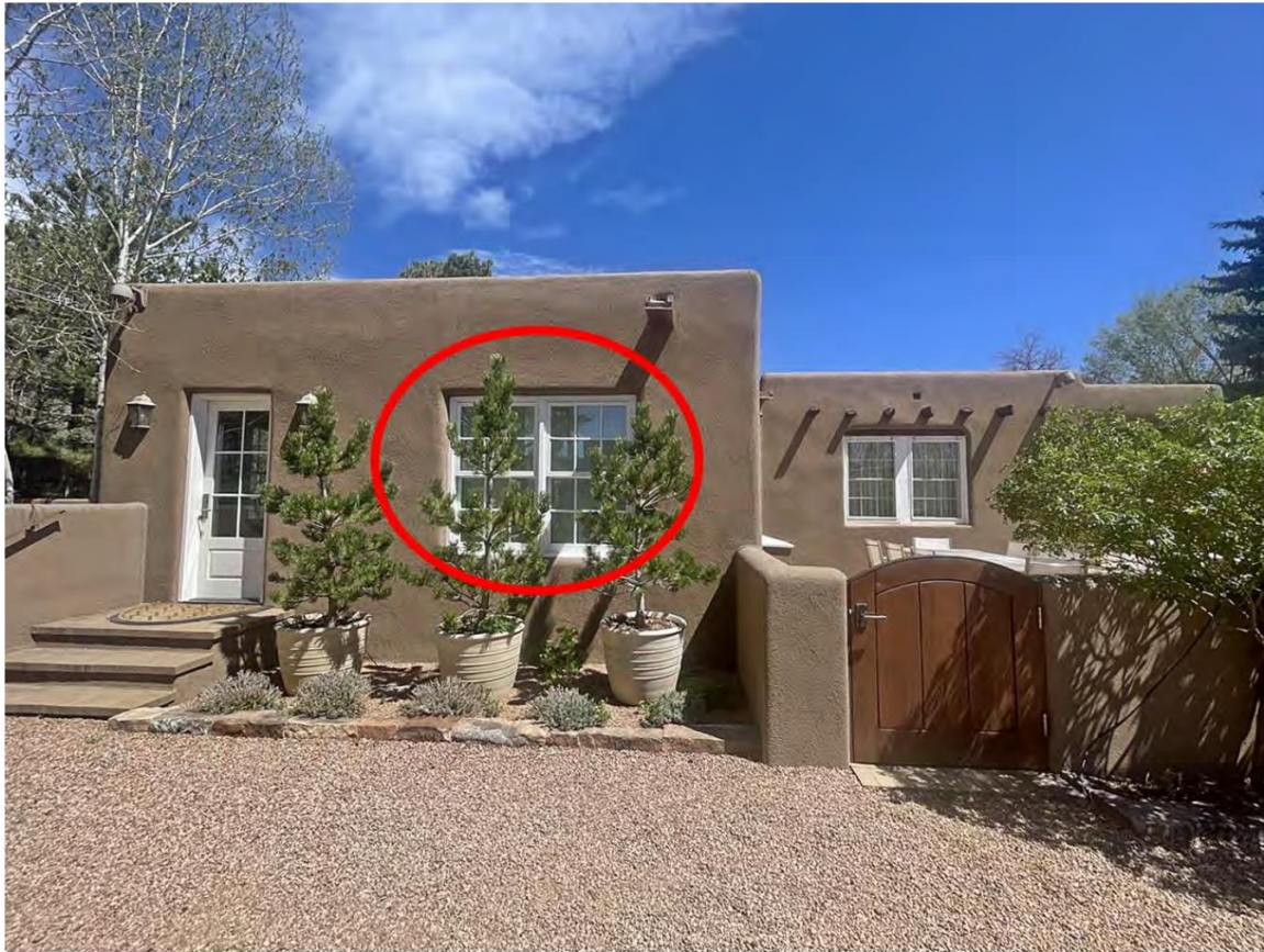
Photo 13: West elevation – enlarged window opening. Camera facing east.
