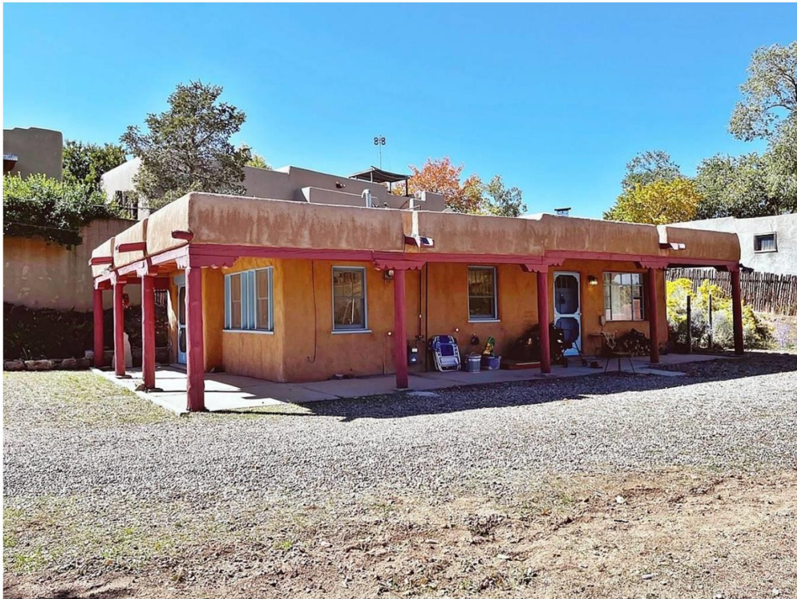
Photo 6: East elevation. Camera facing northwest.
