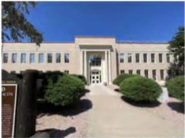
30. Bataan Memorial Building - 1/8" bullnose
