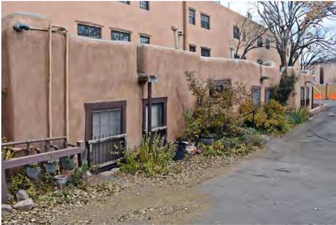
Photo 2: Partial south elevation. Camera facing northeast.
