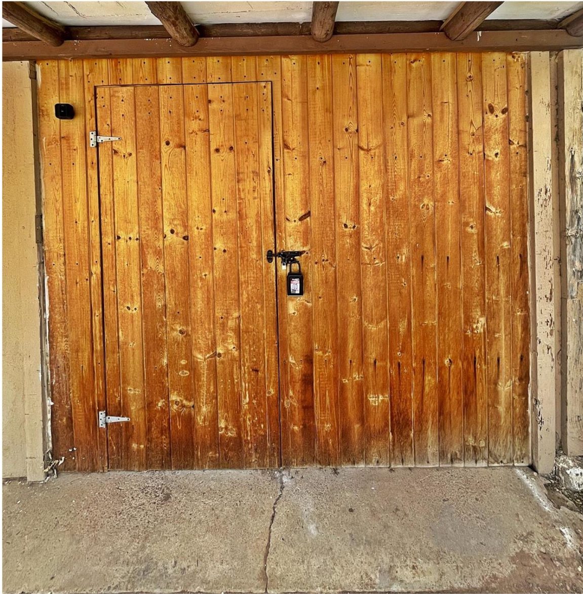
Photo 4: Garage door. Camera facing east.
