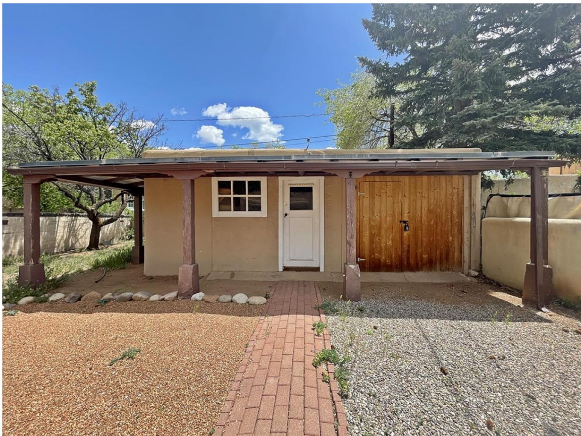
Photo 2: West elevation and setting. Camera facing east.
