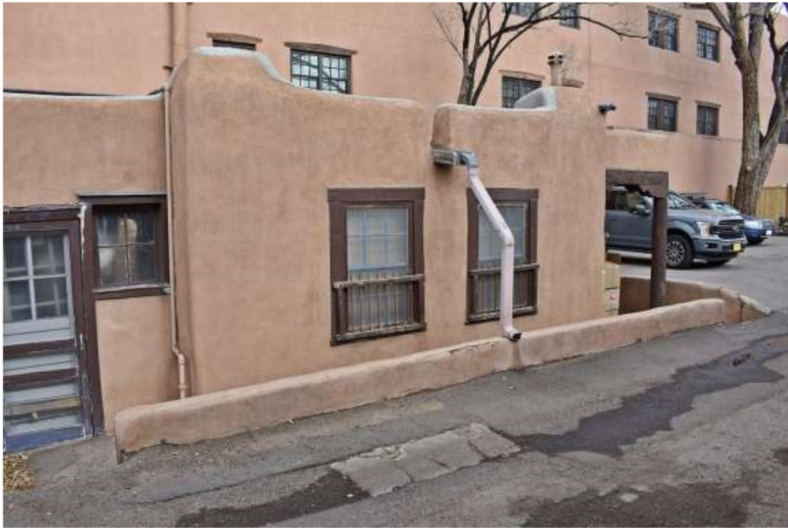
Photo 7: South elevation, Section 4. Camera facing northeast.
