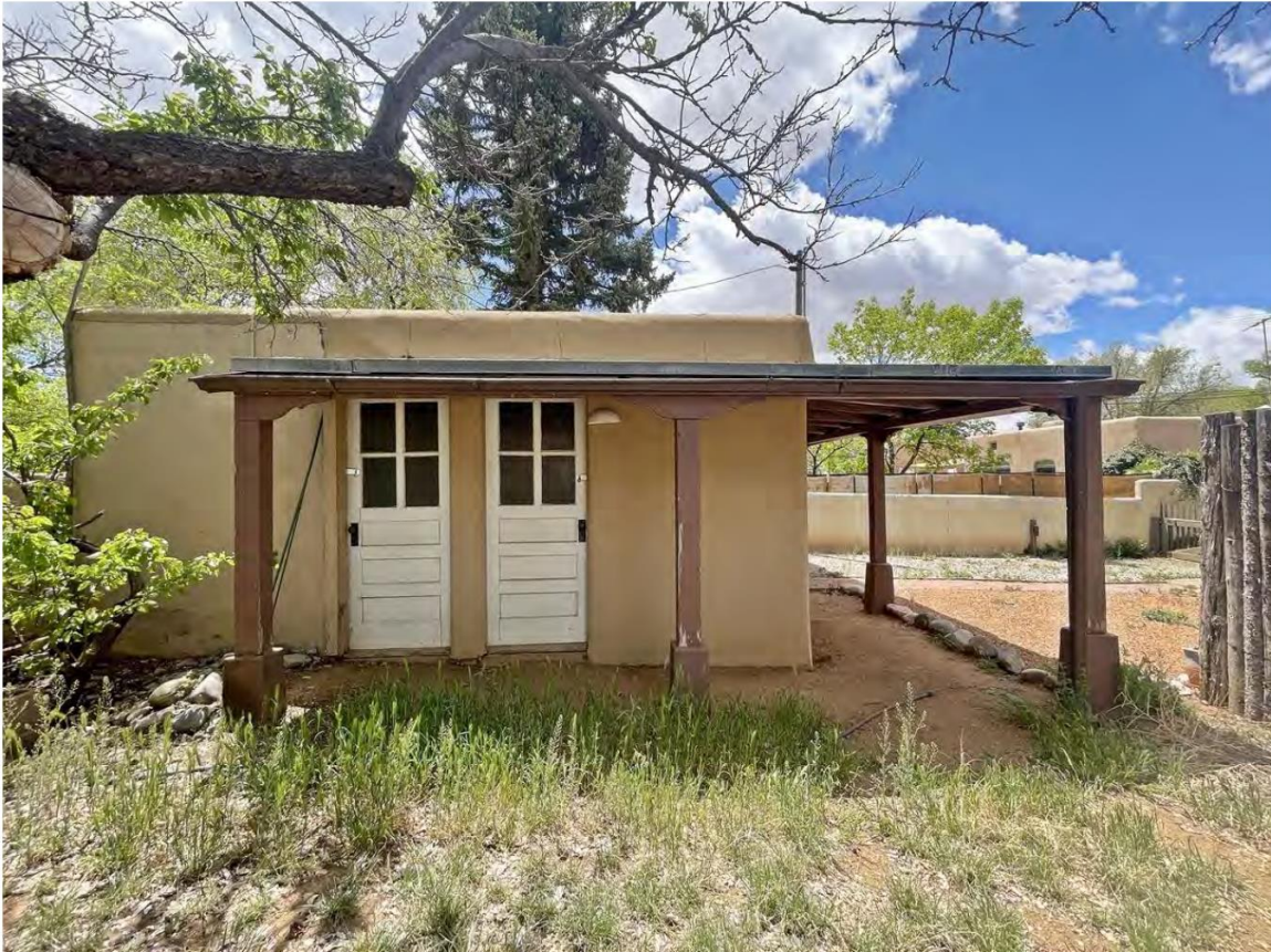
Photo 6: North elevation. Camera facing southwest.
