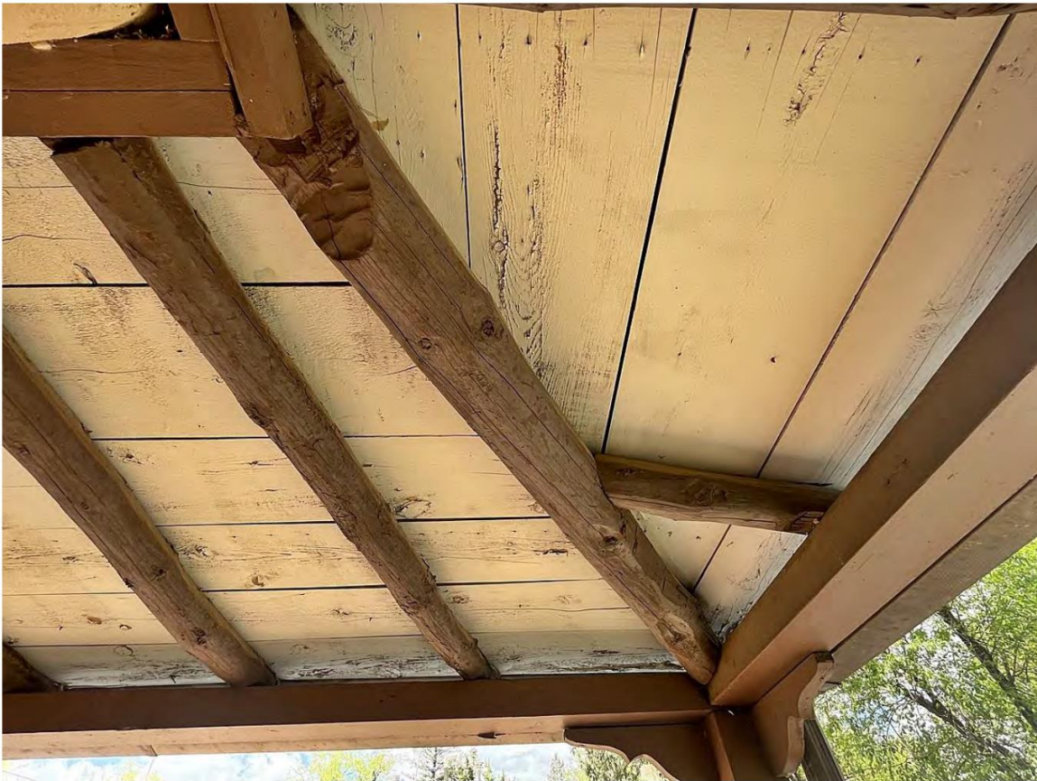
Photo 9: Roof decking, northwest corner. Camera facing up.
