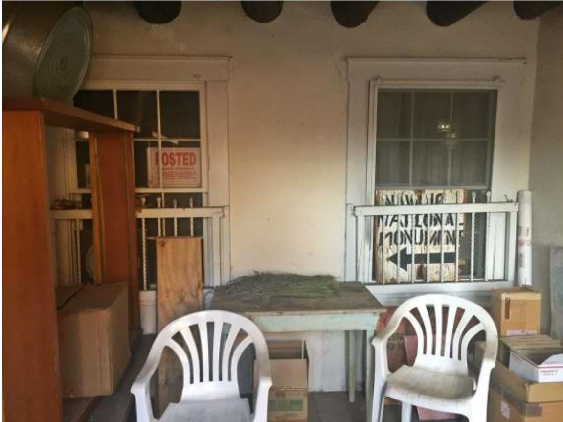
Photo 5: South elevation, Section 2, portal. Camera facing north. November 17, 2020.
