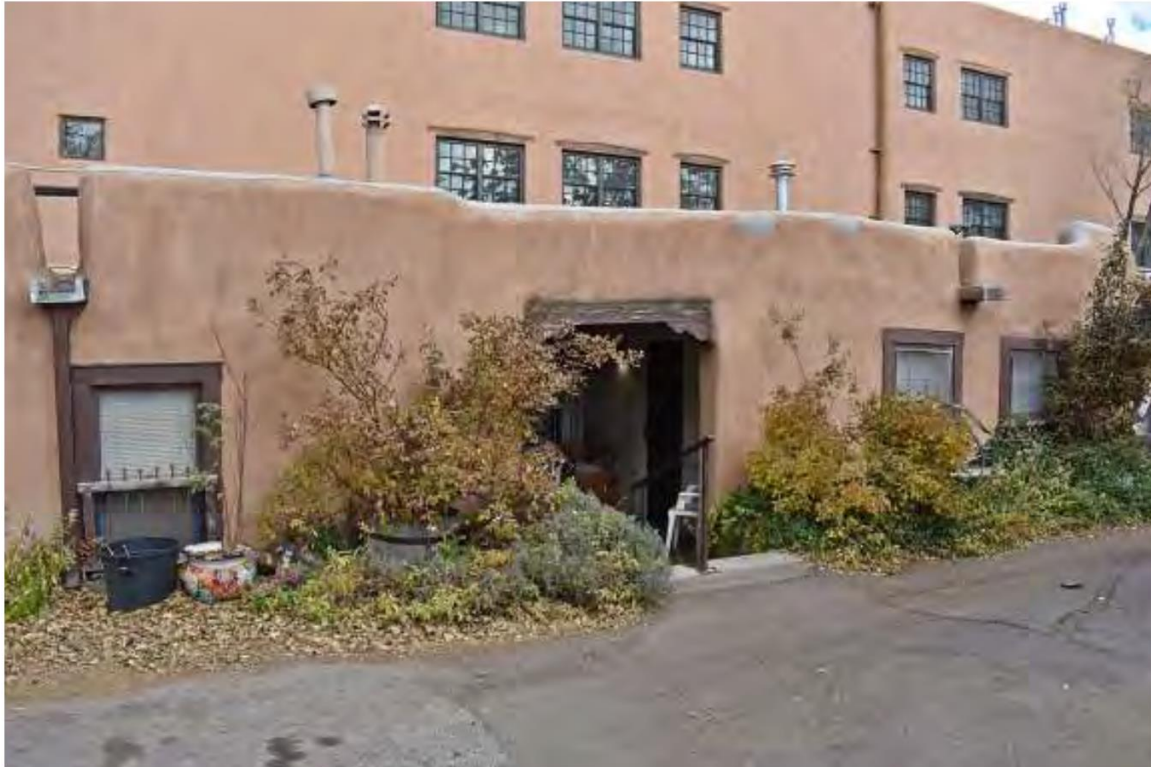
Photo 4: South elevation, Section 2. Camera facing northeast.
