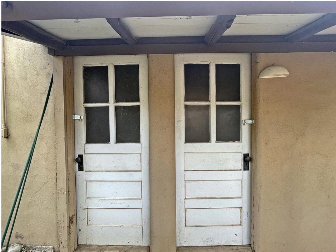
Photo 7: North elevation entry doors. Camera facing south.
