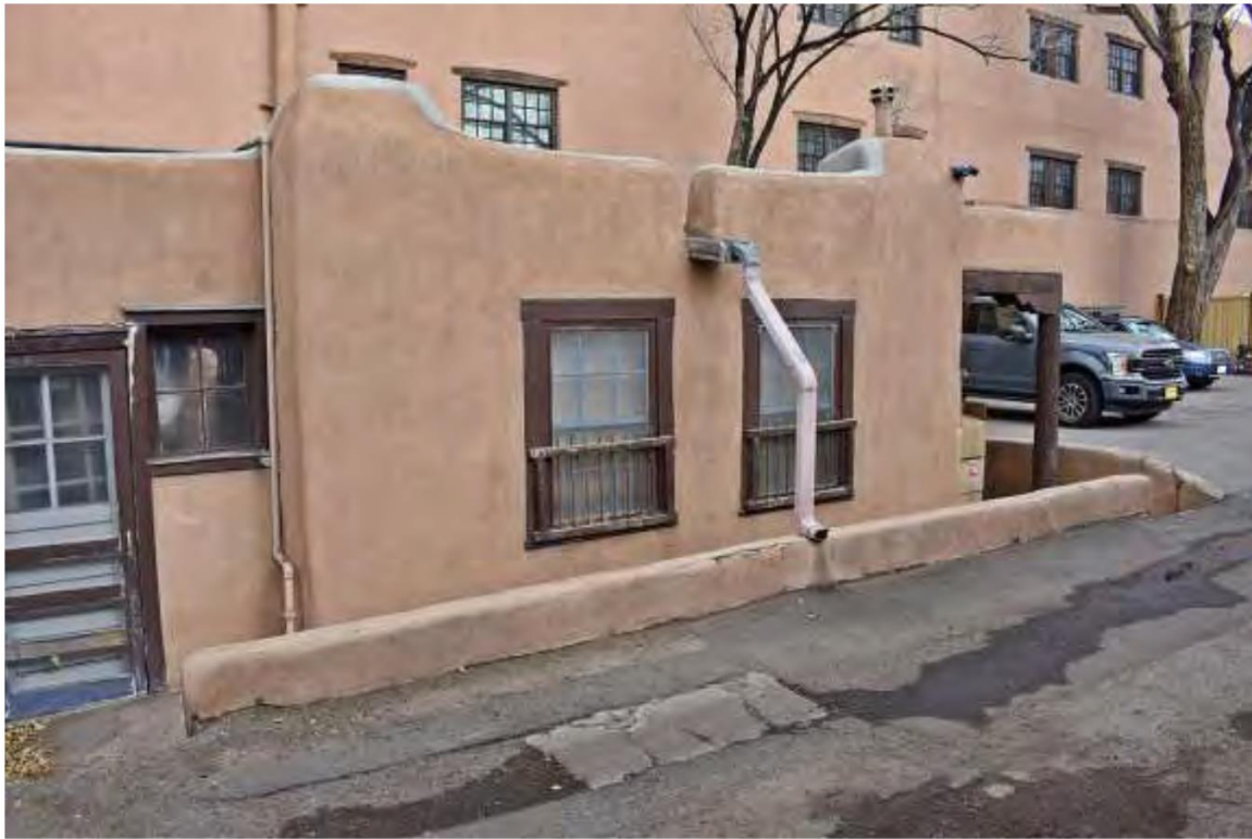
Photo 7: South elevation, Section 4. Camera facing northeast.
