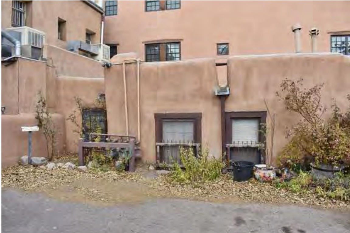
Photo 3 South elevation, Section 1. Camera facing northwest.
