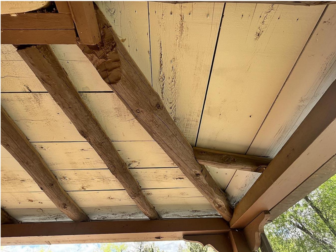
Photo 9: Roof decking, northwest corner. Camera facing up.
