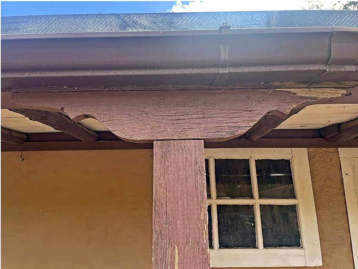
Photo 8: West elevation, faux corbel. Camera facing up.
