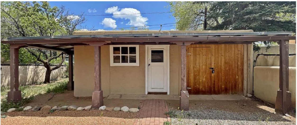
Figure 2: The accessory structure west facade
