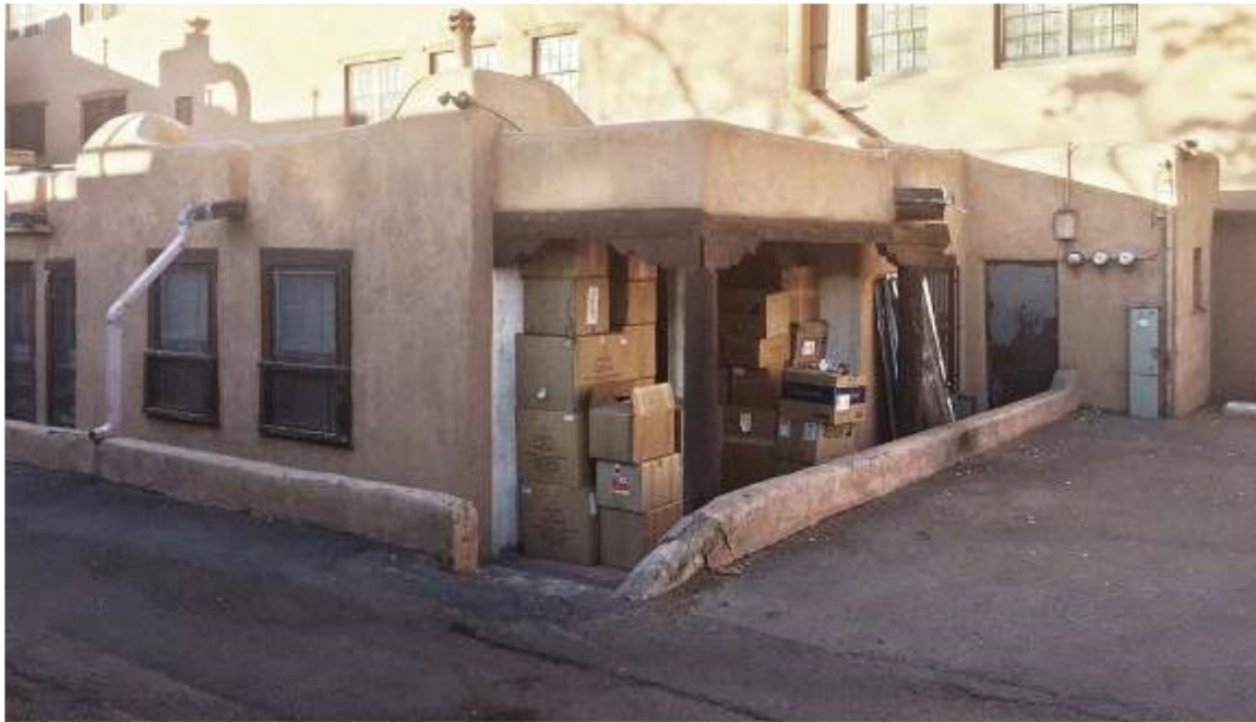
Photo 8: East elevation. Camera facing northwest.
