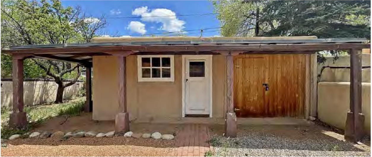
Figure 2: The accessory structure west facade
