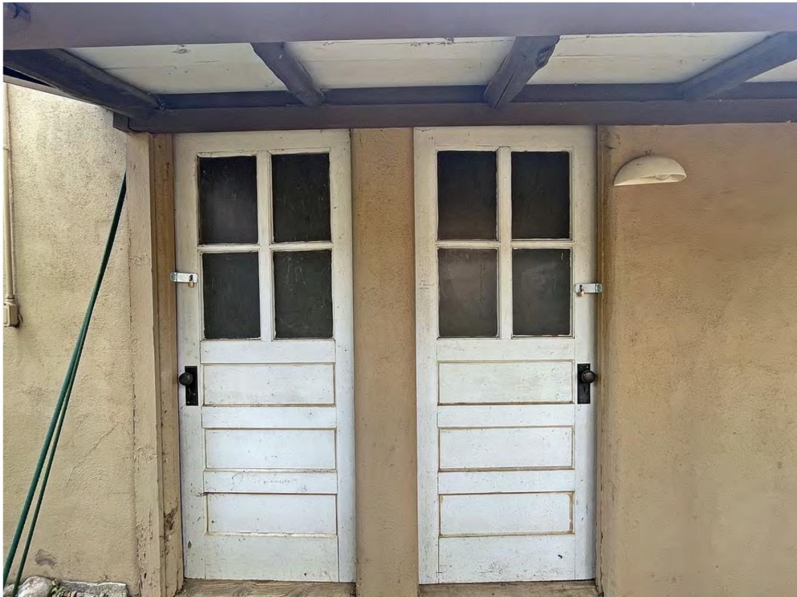
Photo 7: North elevation entry doors. Camera facing south.
