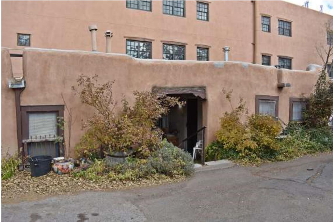
Photo 4: South elevation, Section 2. Camera facing northeast.
