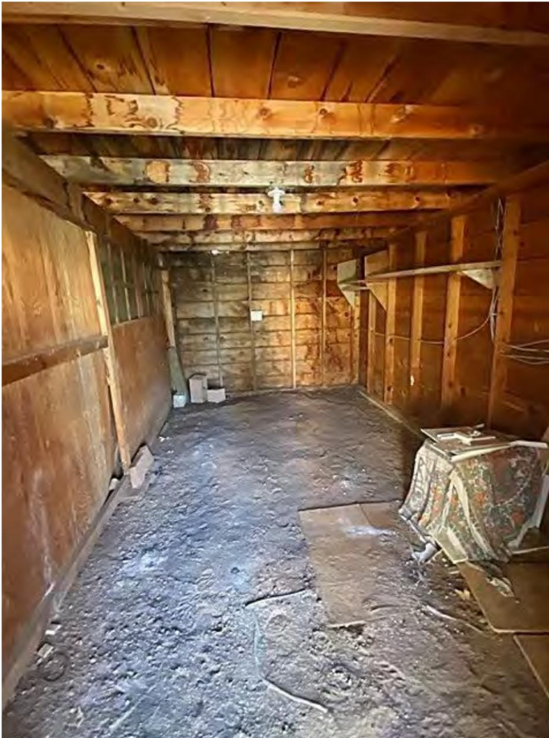
Photo 3: Garage section. Camera facing east. Marc Natkin, May 2024.
