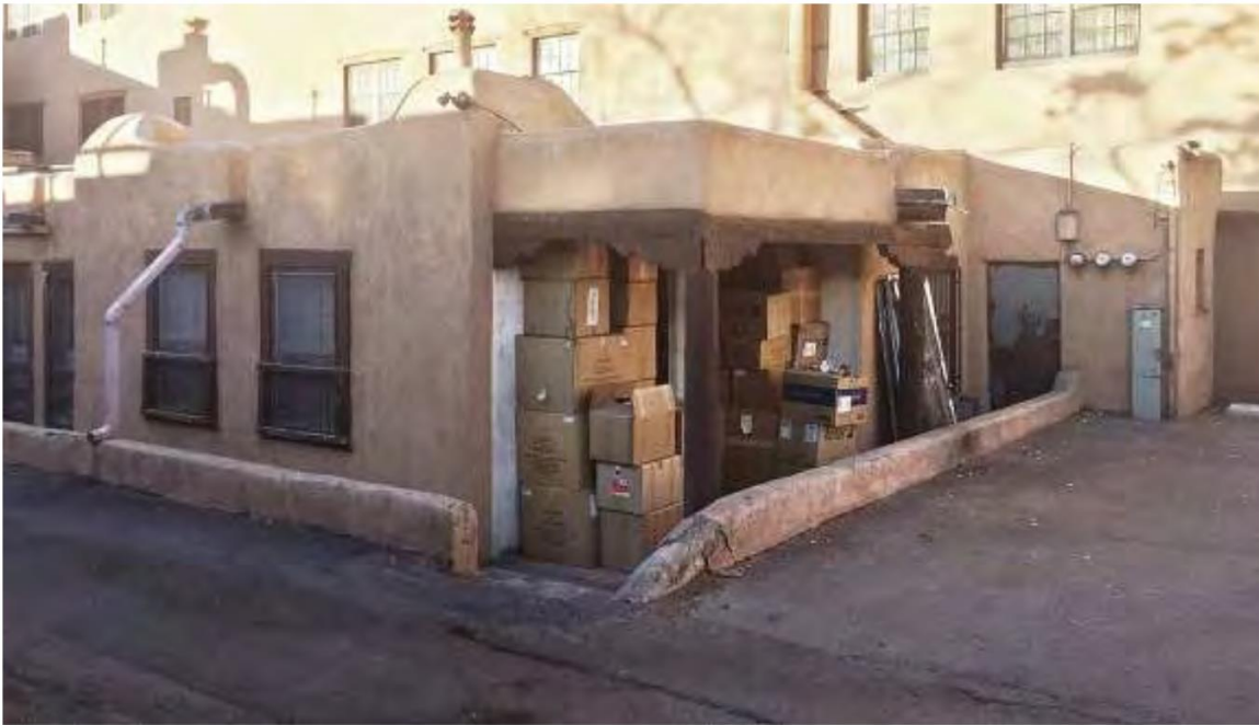
Photo 8: East elevation. Camera facing northwest.
