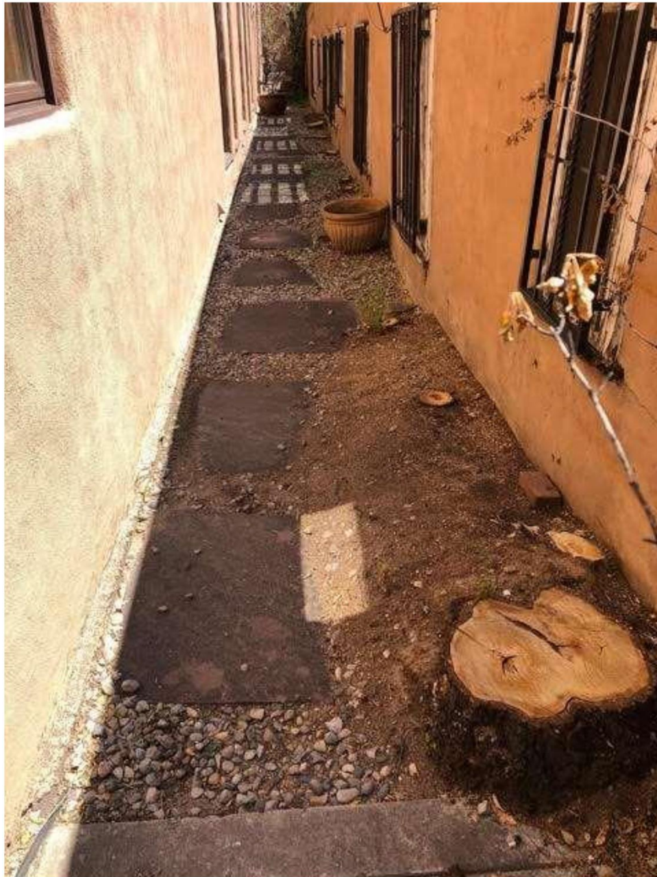
Photo 9: North elevation (right). Camera facing east. Carlos Kinsey, August 28, 2020.
