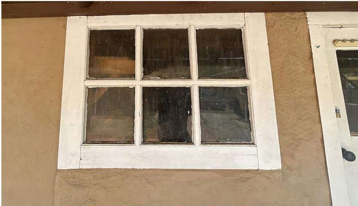
Photo 5: West elevation, window. Camera facing up.
