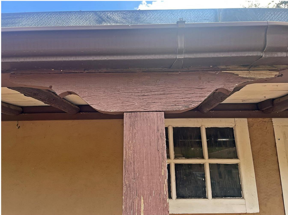
Photo 8: West elevation, faux corbel. Camera facing up.
