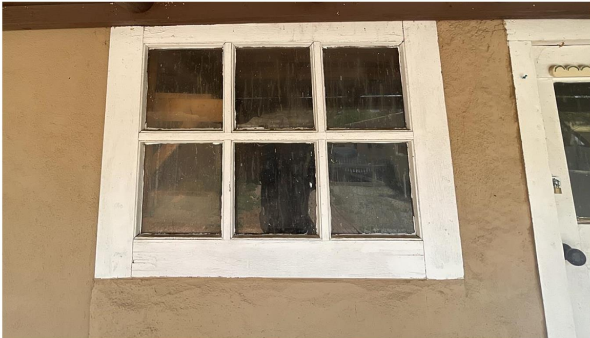
Photo 5: West elevation, window. Camera facing up.
