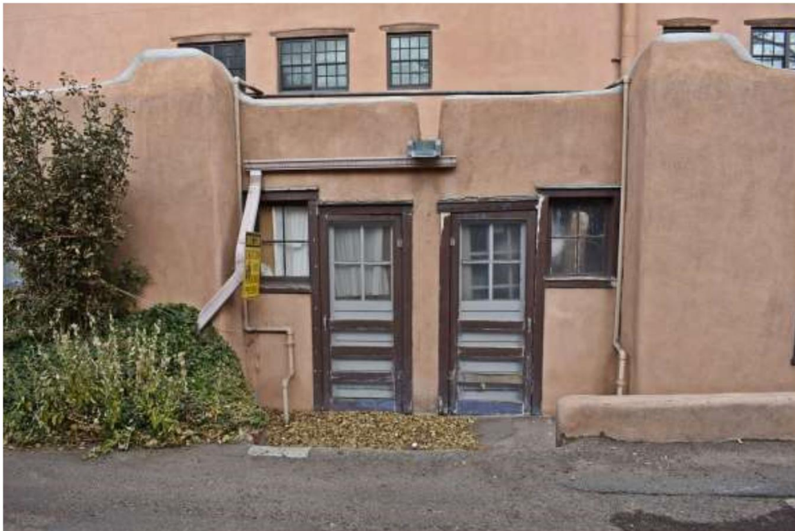
Photo 6: South elevation, Section 3. Camera facing north.
