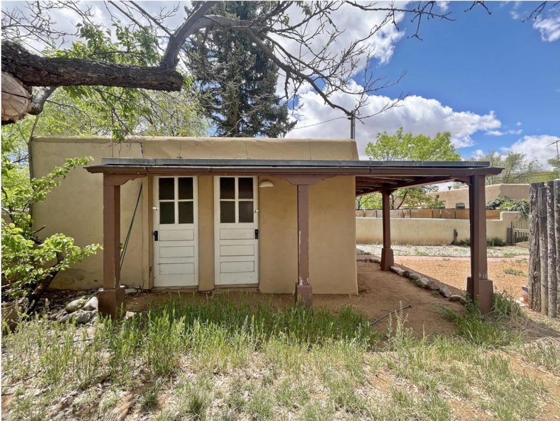
Photo 6: North elevation. Camera facing southwest.
