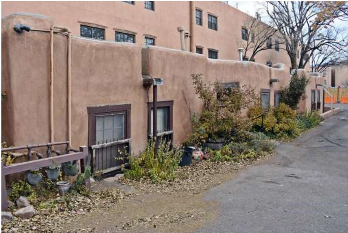
Photo 2: Partial south elevation. Camera facing northeast.
