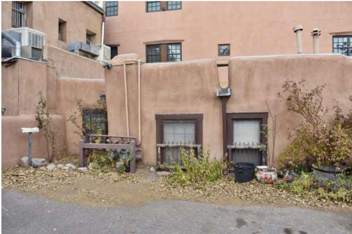
Photo 3 South elevation, Section 1. Camera facing northwest.
