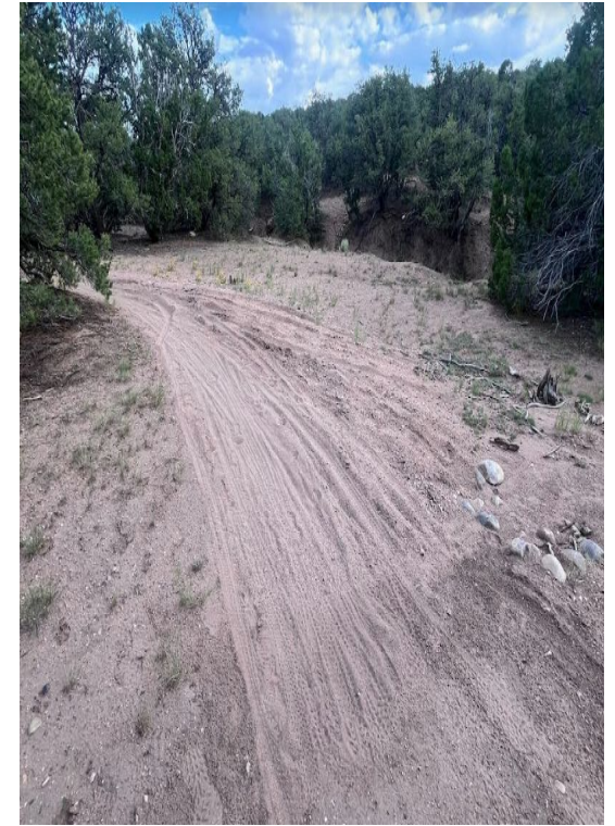
Washed out section with deep sand.
