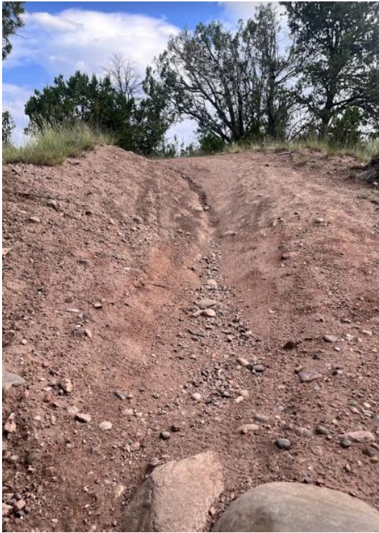
Arroyo crossing that's deep and difficult to cross.
