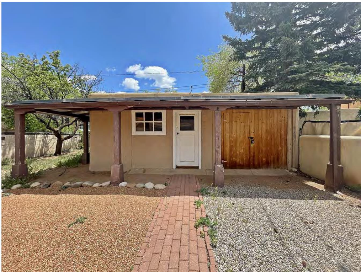
Photo 2: West elevation and setting. Camera facing east.
