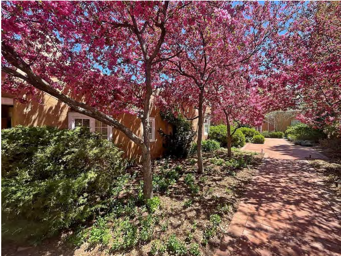
Photo 6: South elevation and walkway. Camera facing east.
