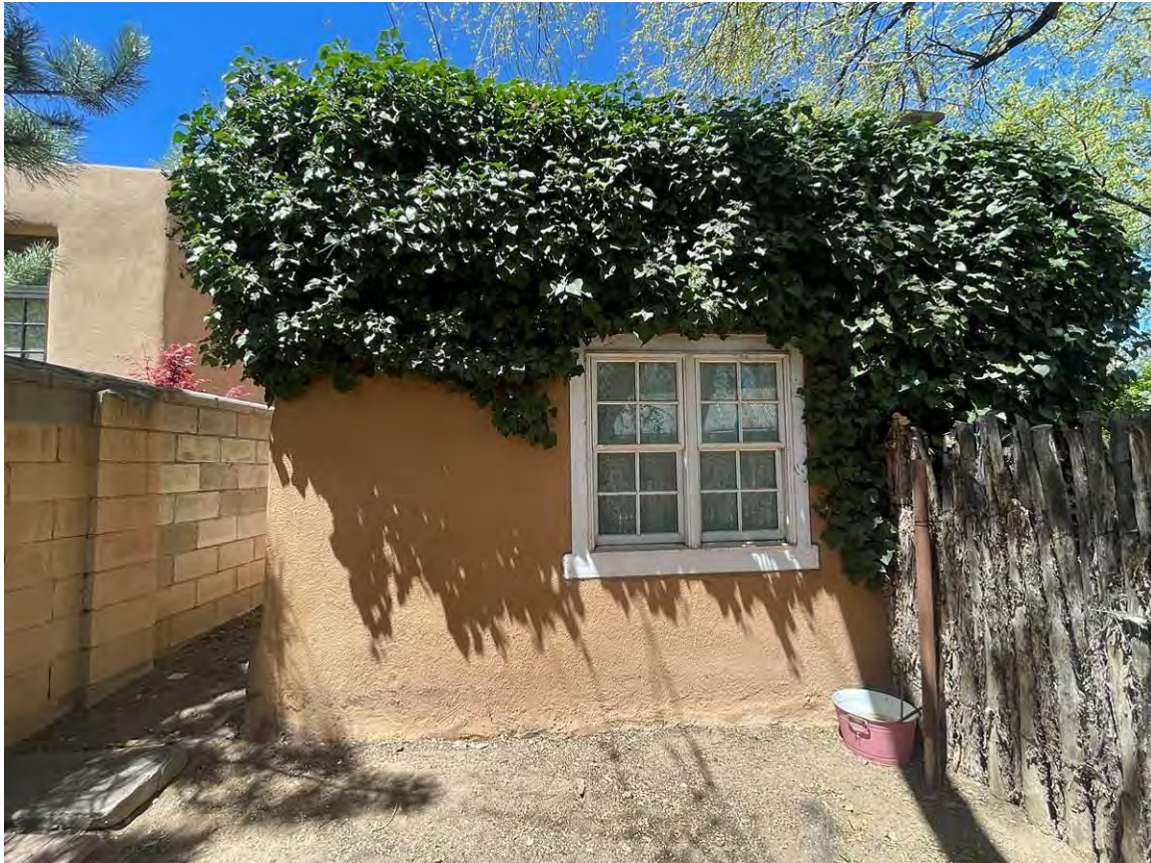
Photo 27: East elevation. Camera facing west.
