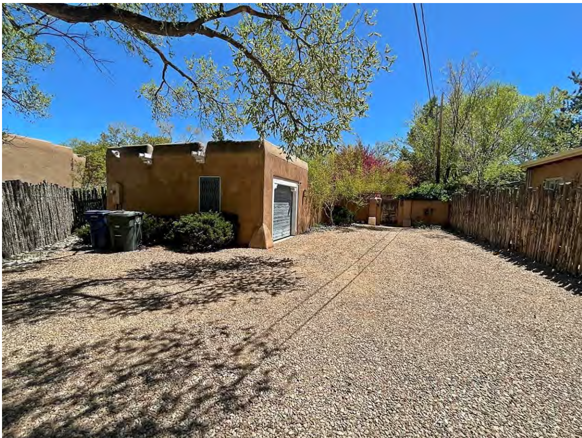
Photo 2: View from entry to non-historic garage. Camera facing east.
