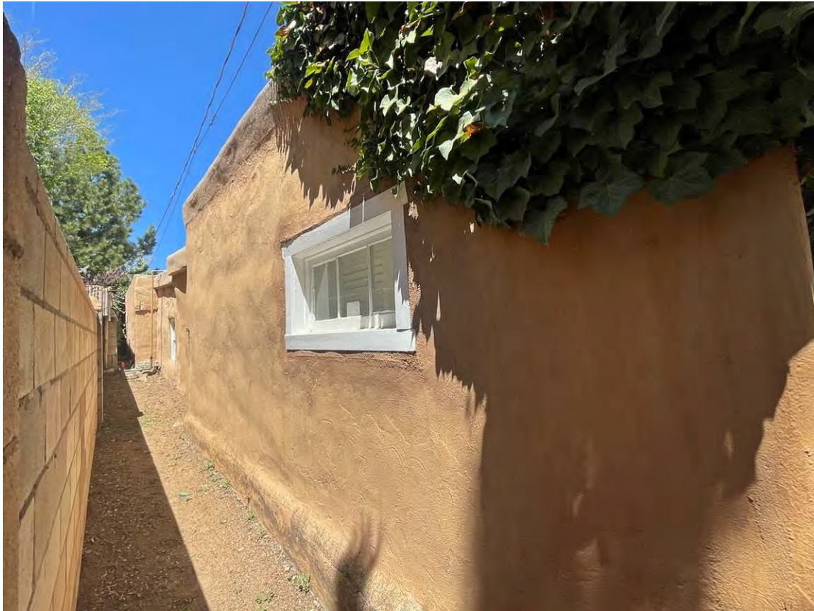
Photo 28: South elevation, east end. Camera facing northwest.
