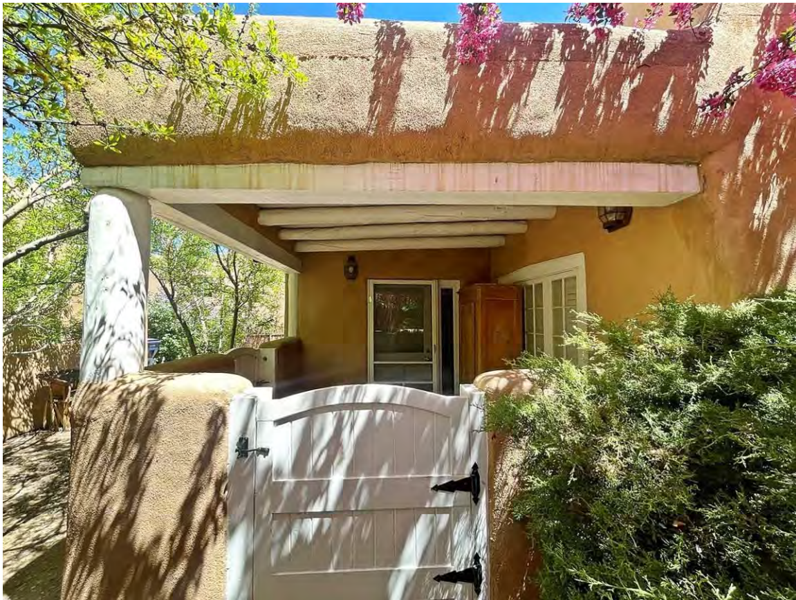
Photo 4: South elevation, altered 1976 portal. Camera facing north.
