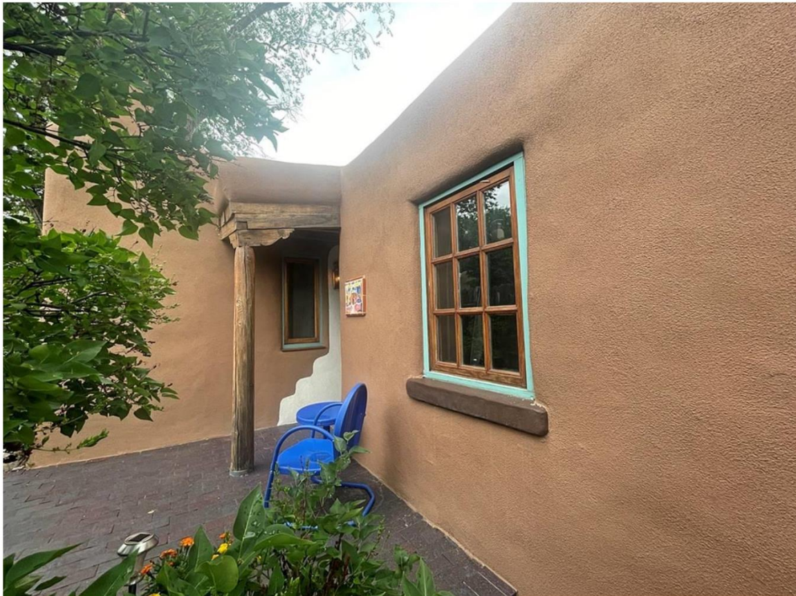
Photo 9: South elevation oblique, east of entrance. Camera facing northwest. June 22, 2024.
