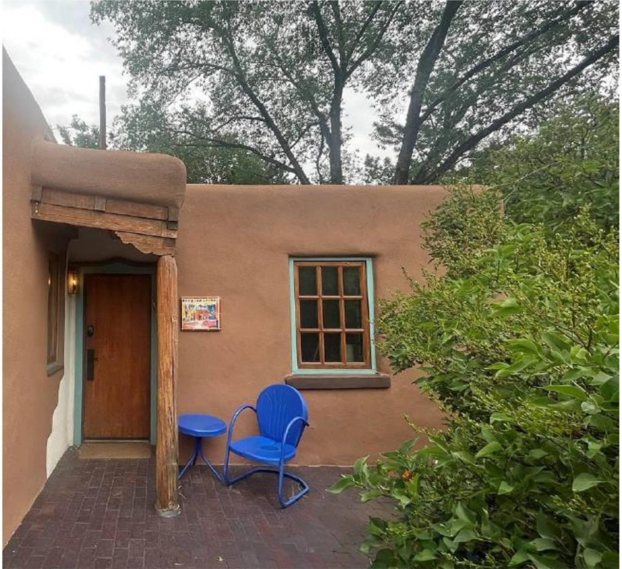
Figure 2: South and East facades at main entrance
