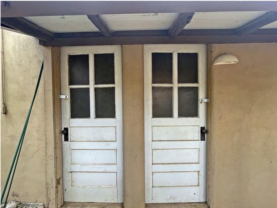
Photo 7: North elevation entry doors. Camera facing south.
