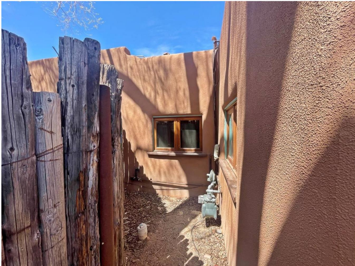
Photo 7: South elevation, west end. Camera facing north. April 20, 2024.
