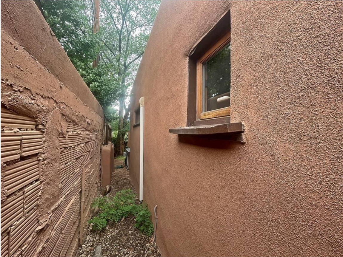
Photo 12: North elevation oblique. Camera facing east.
