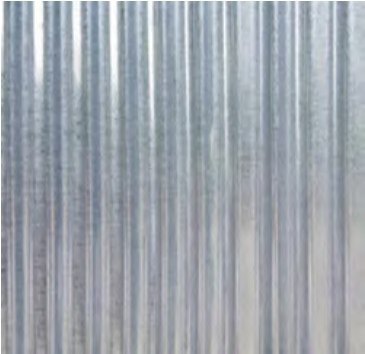
Pitched Roof Locations: Corrugated Galvanized Sheet Metal
