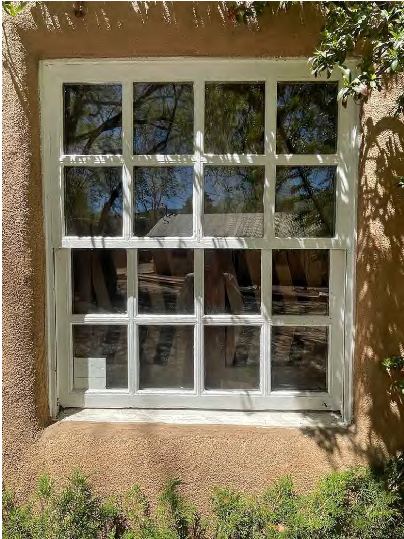
Photo 14: East elevation, 1980s window. Camera facing west.
