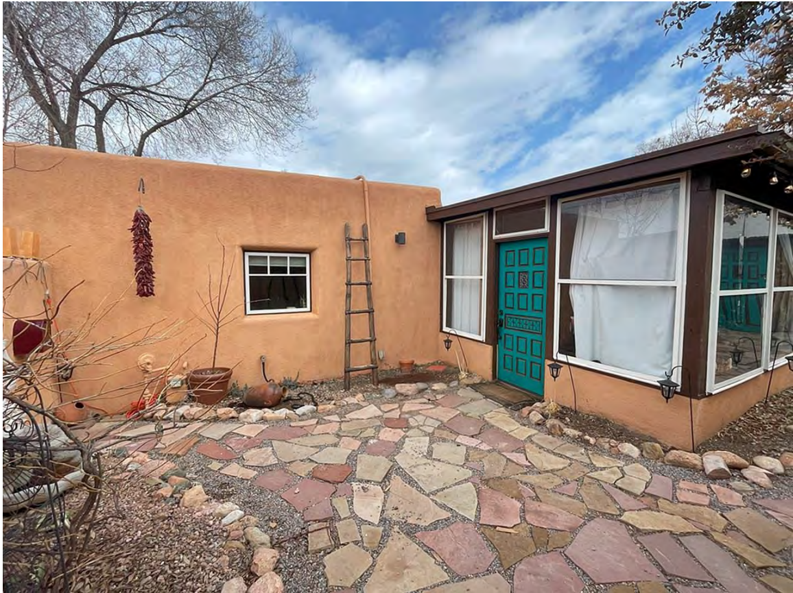
Photo 6: South elevation and sunroom. Camera facing northeast.
