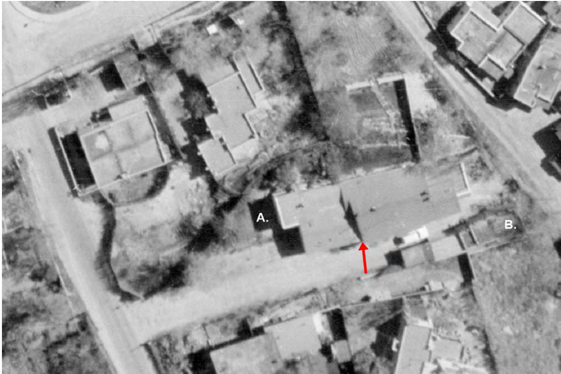
Figure 15: May 11, 1973, aerial photograph. A. Main house; B. Guesthouse. The arrow indicates that dwellings have been joined together.
