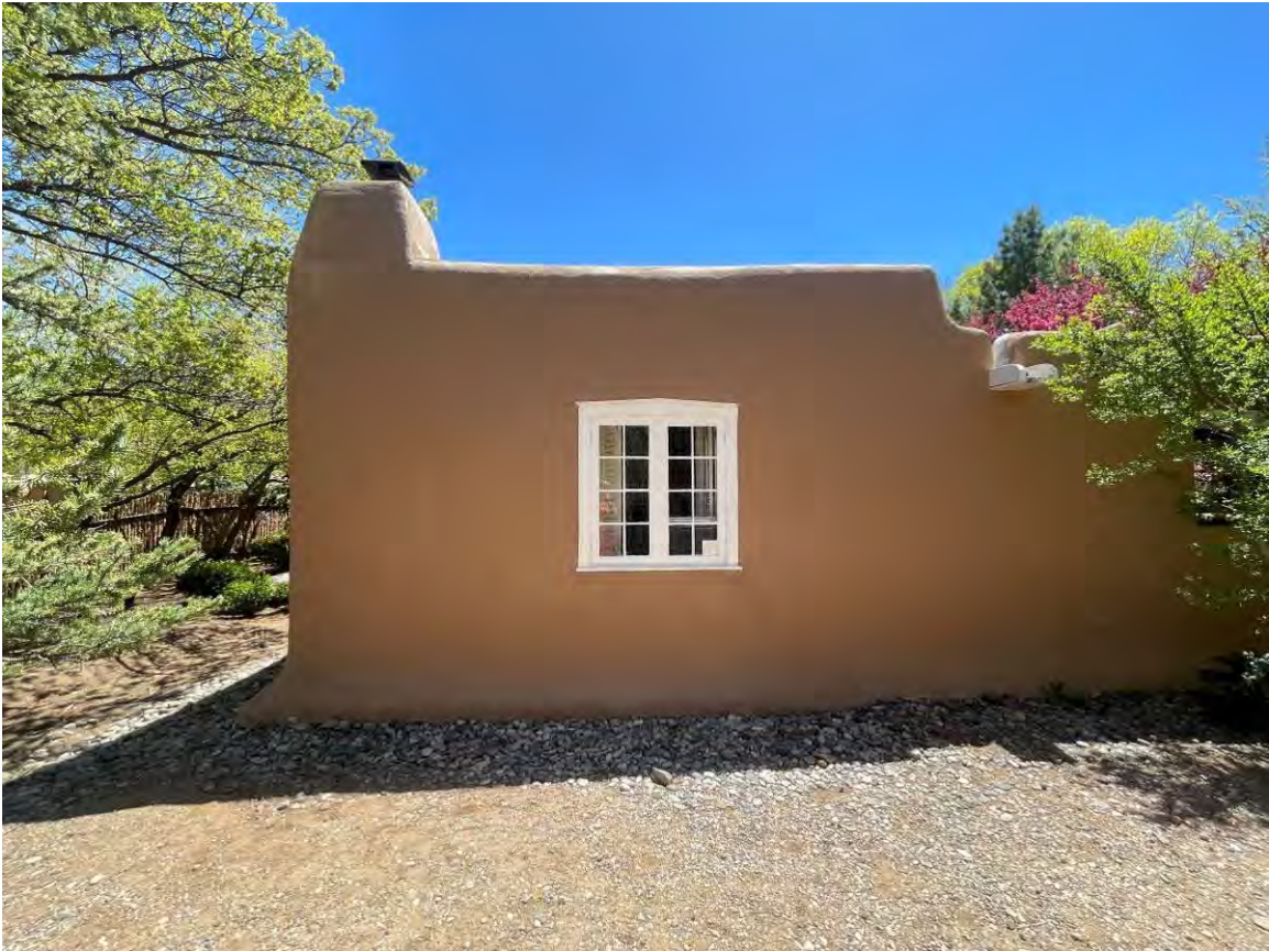
Photo 5: West elevation, unaltered section. Camera facing east.
