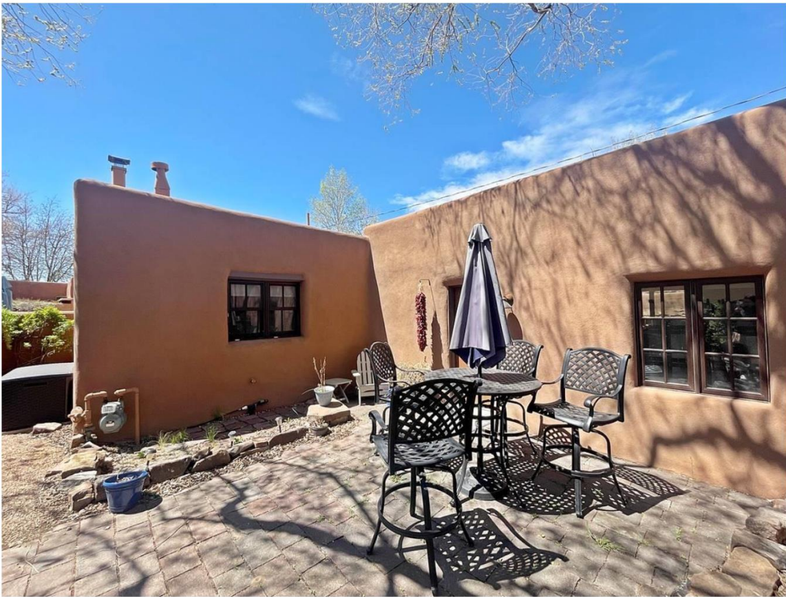
Photo 13: East and south elevation oblique. Camera facing northwest. April 20, 2024.
