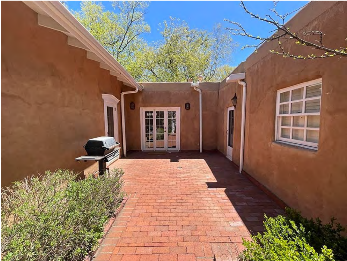
Photo 11: South elevation (left), non-historic connector (center), guesthouse (right). Camera facing east.
