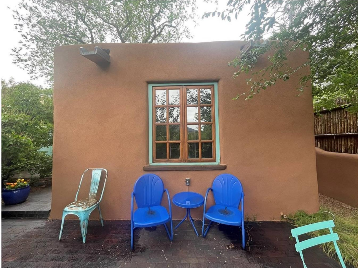
Photo 10: East elevation. Camera facing west.
