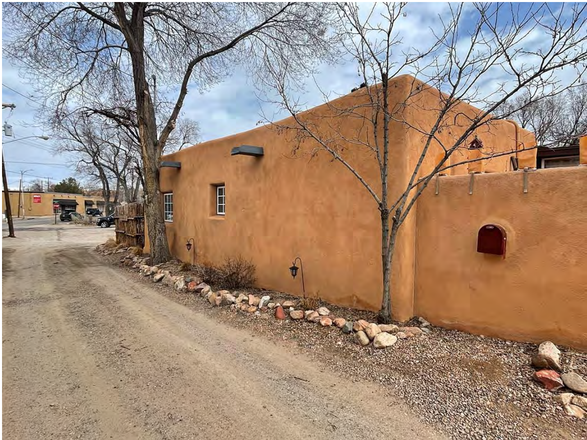
Photo 5: West and south elevation. Camera facing northeast. Note wall is non-historic.
