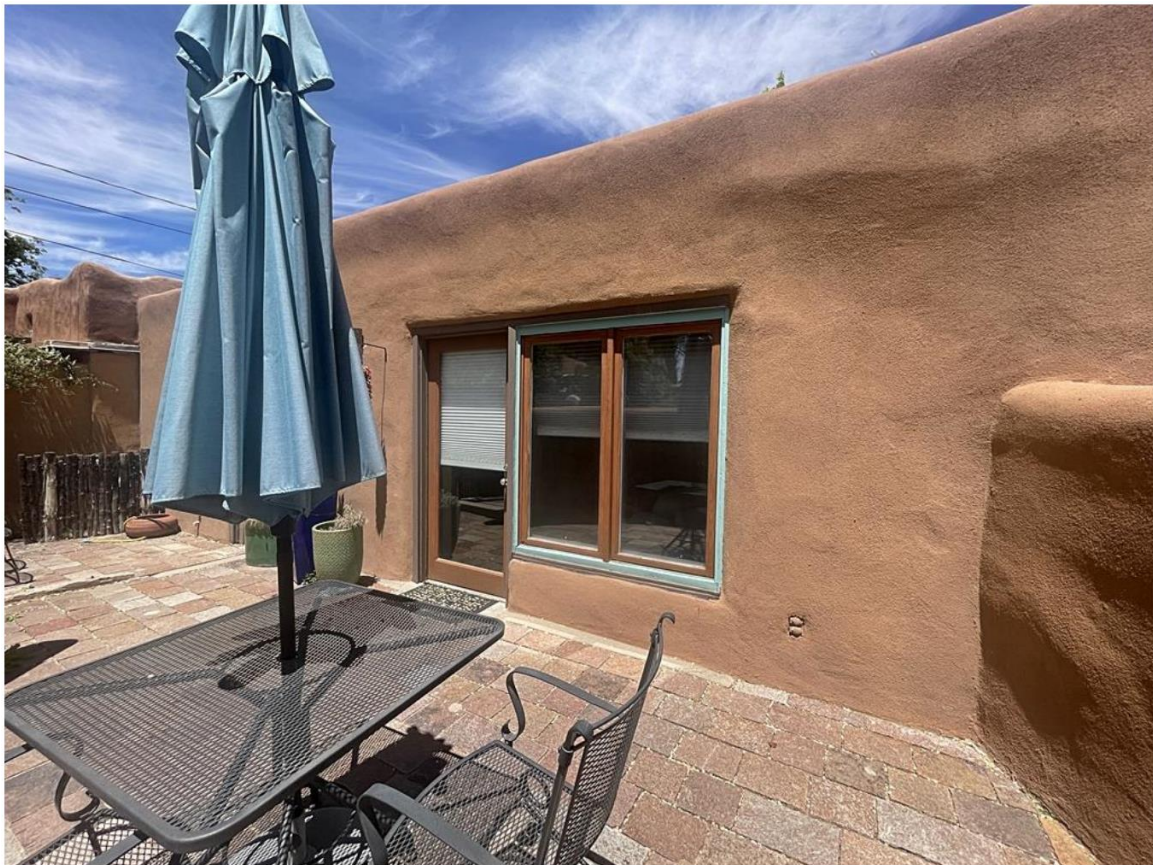
Photo 18: South elevation, oblique. Camera facing northwest. May 20, 2024.
