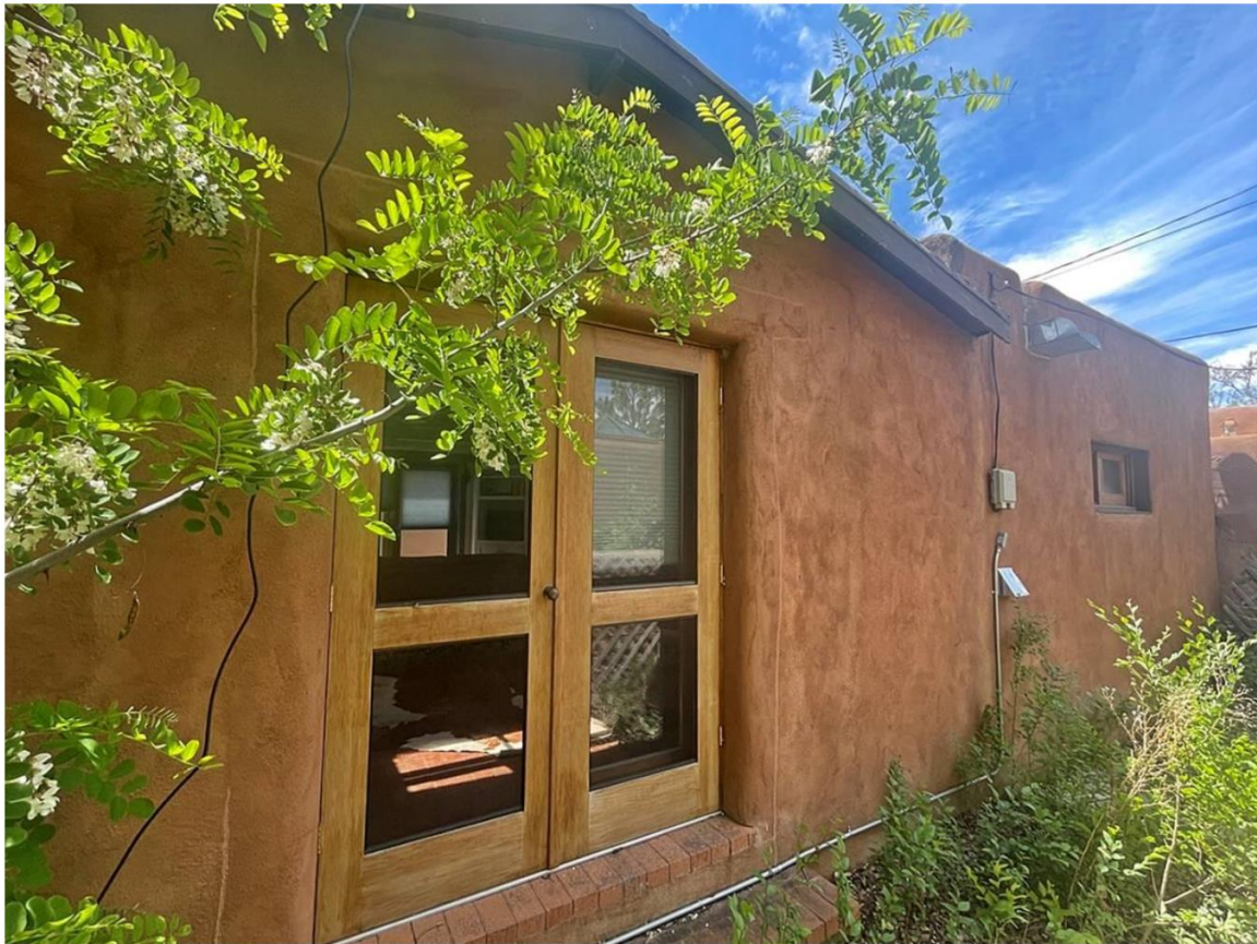
Photo 21: North elevation, oblique. Camera facing southwest. May 20, 2024.
