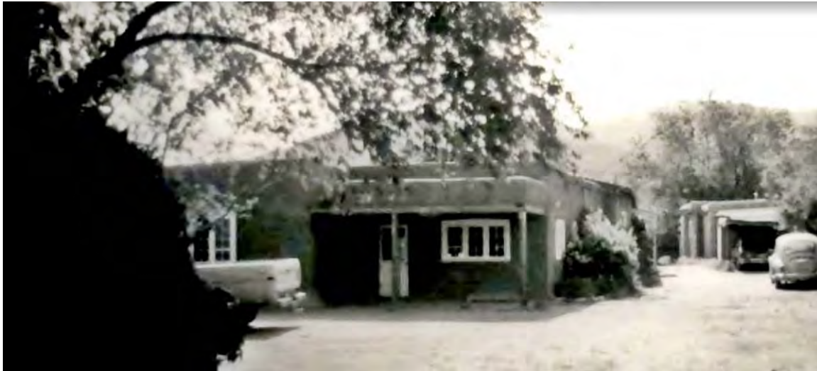
Figure 2: March 6, 1983, HBI survey photograph. Michael Belshaw. West side of building complex. Camera facing east. Courtesy NMCRIIS.
