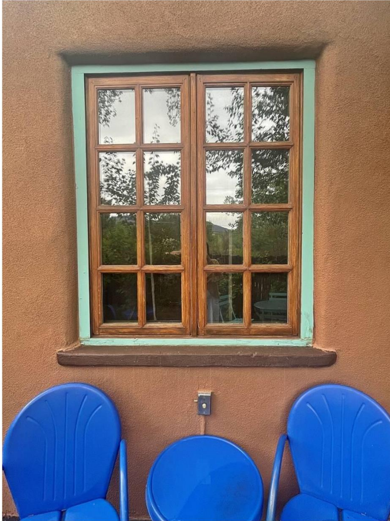
Photo 11: East elevation window. Camera facing west.
