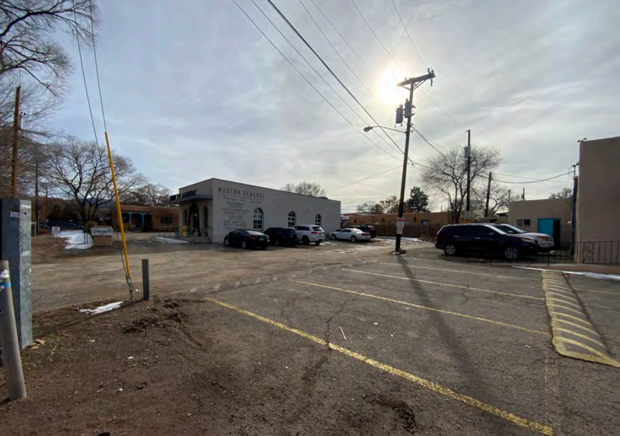
VIEW OF NORTHERN WALL FROM CERILLOS
