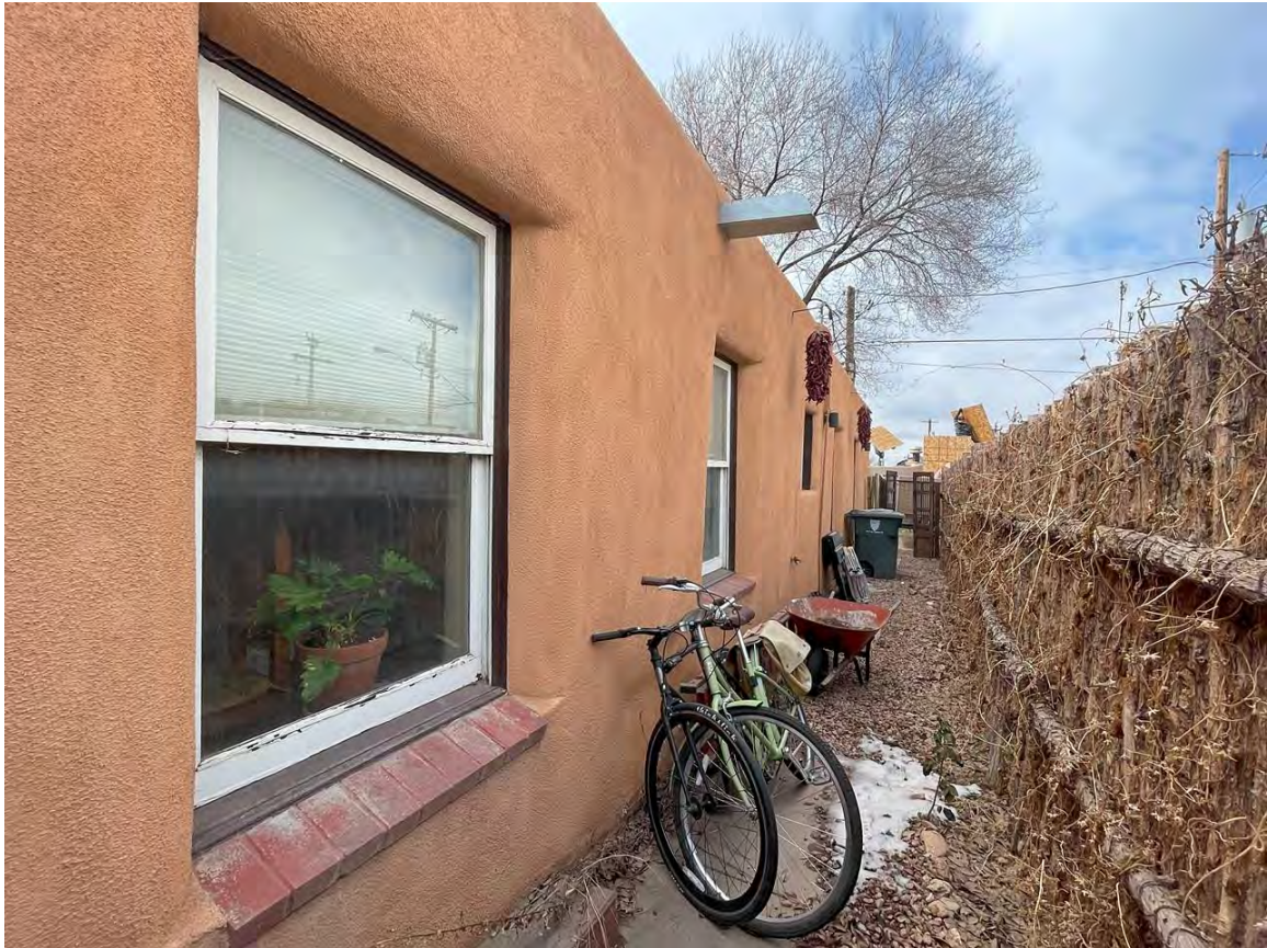
Photo 3: North elevation. Camera facing southwest.
