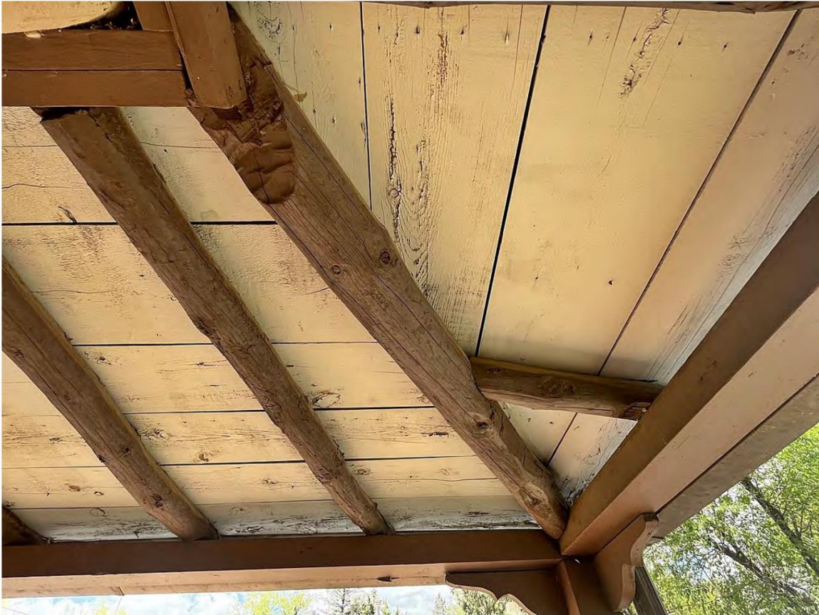
Photo 9: Roof decking, northwest corner. Camera facing up.
