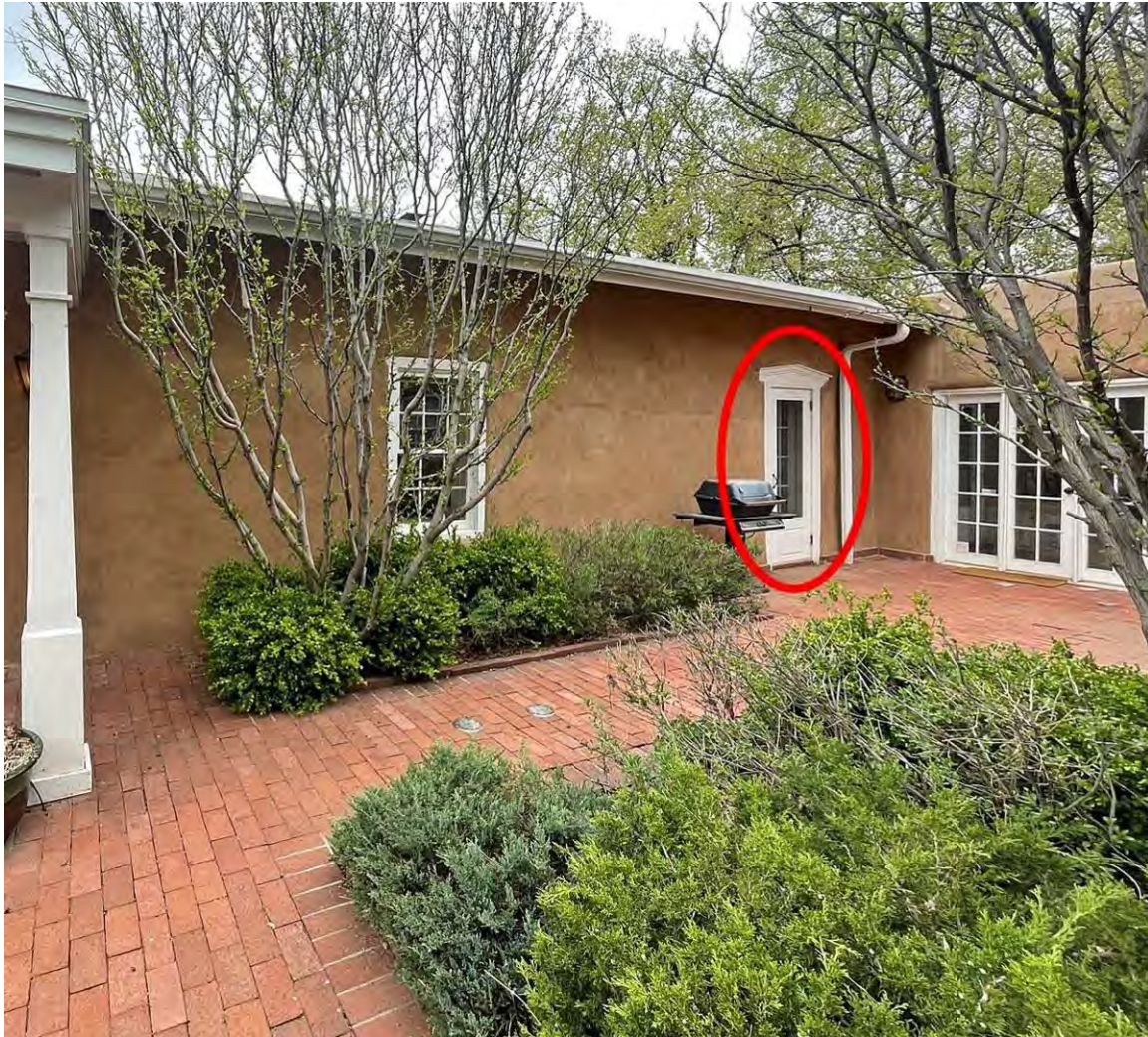
Photo 12: South elevation, east end. 1990s door circled. Camera facing northeast. May 4, 2024.
