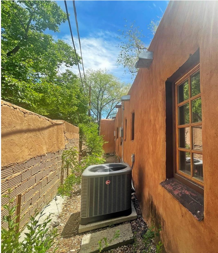
Photo 17: North elevation, oblique. Camera facing east. May 20, 2024.
