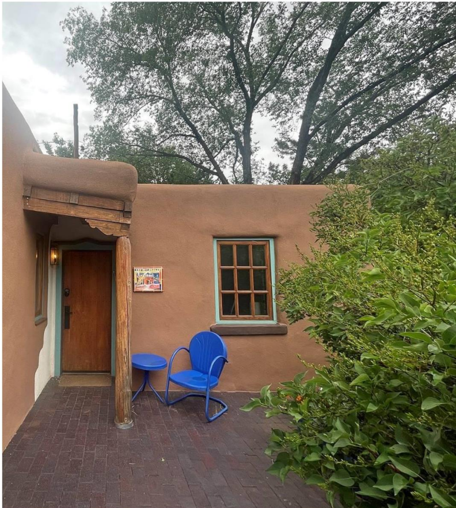
Photo 8: South elevation, entry. Camera facing north. June 22, 2024.
