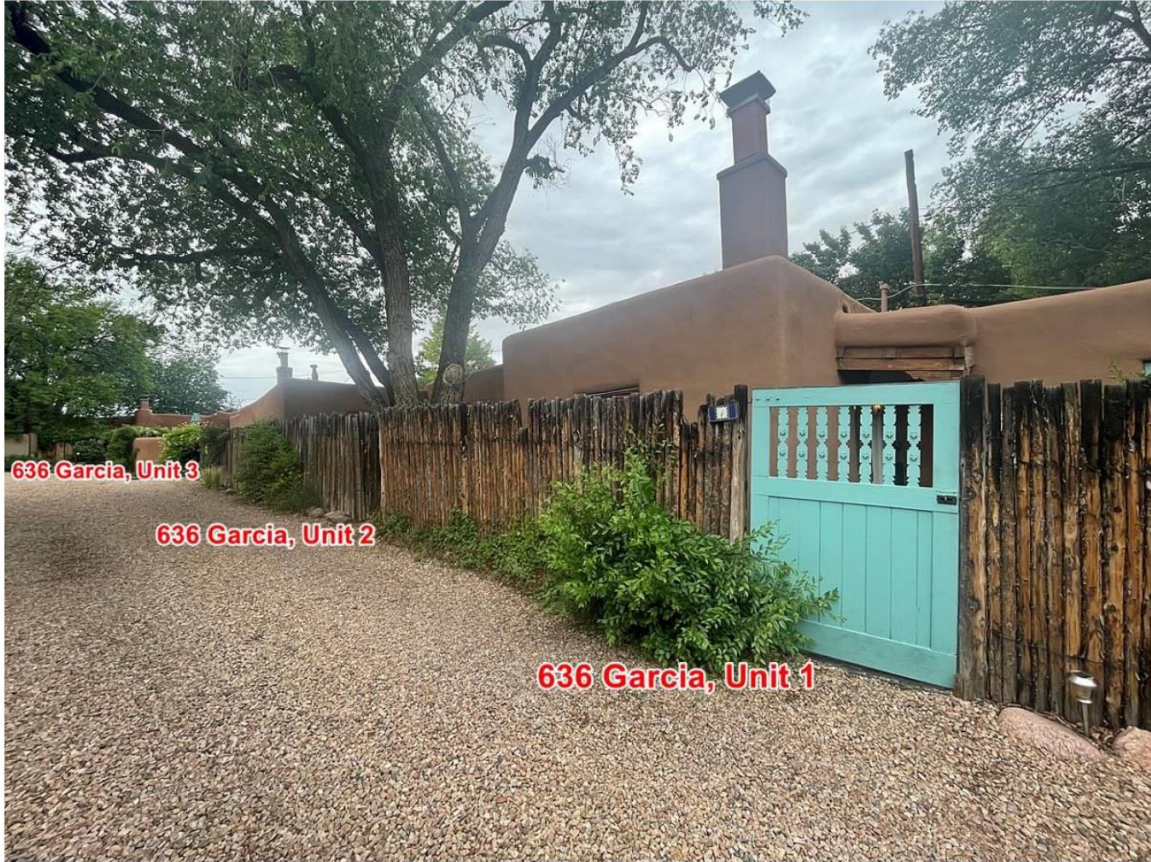
Photo 4: Units 1, 2, and 3. Camera facing northwest. June 22, 2024.
