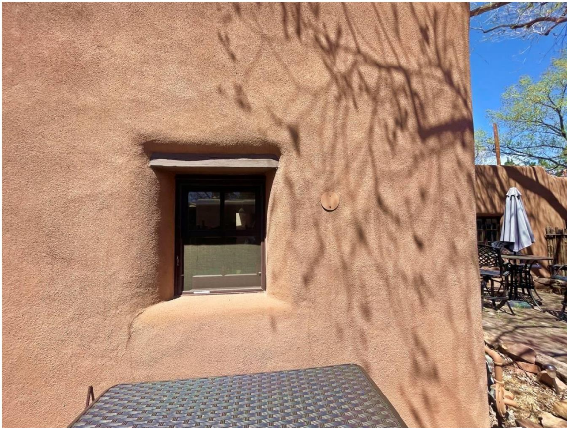
Photo 15: South elevation. Window at kitchen. Camera facing north. April 20, 2024.
