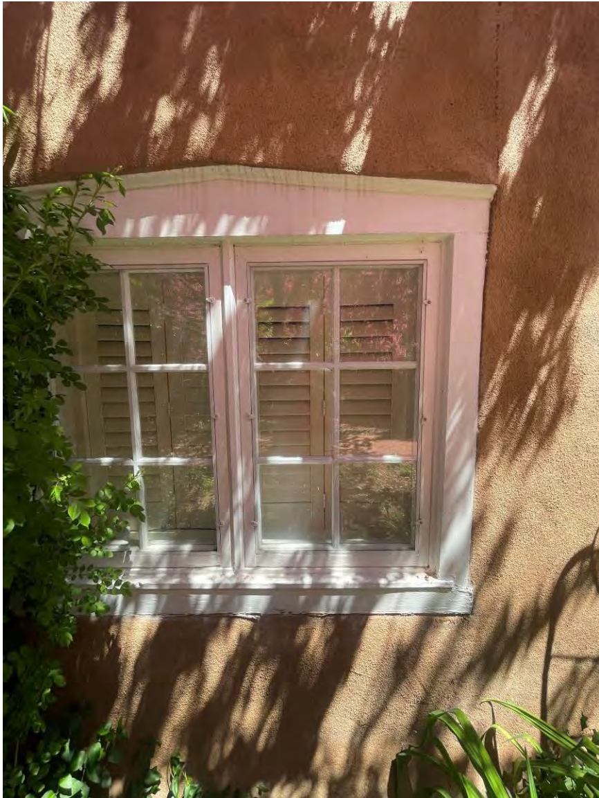
Photo 8: South elevation, older window. Camera facing north.
