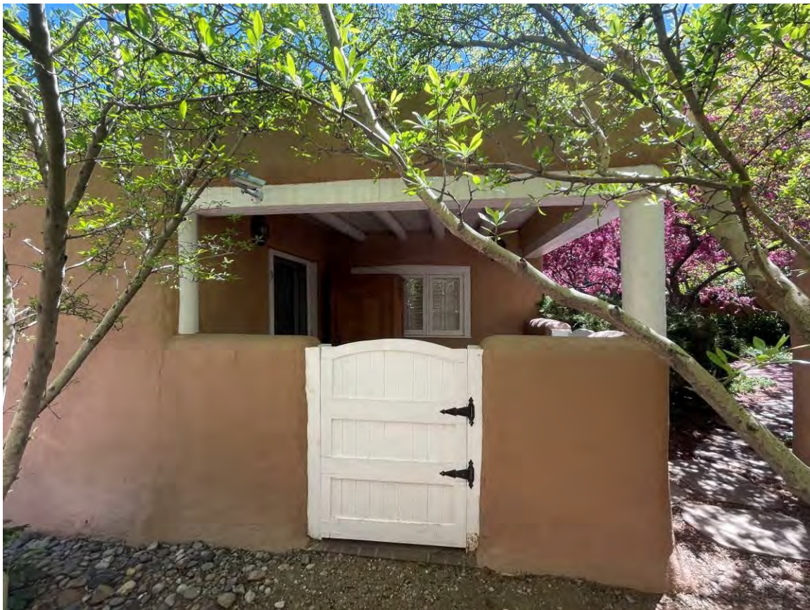
Photo 3: West elevation, altered 1976 portal. Camera facing east.
