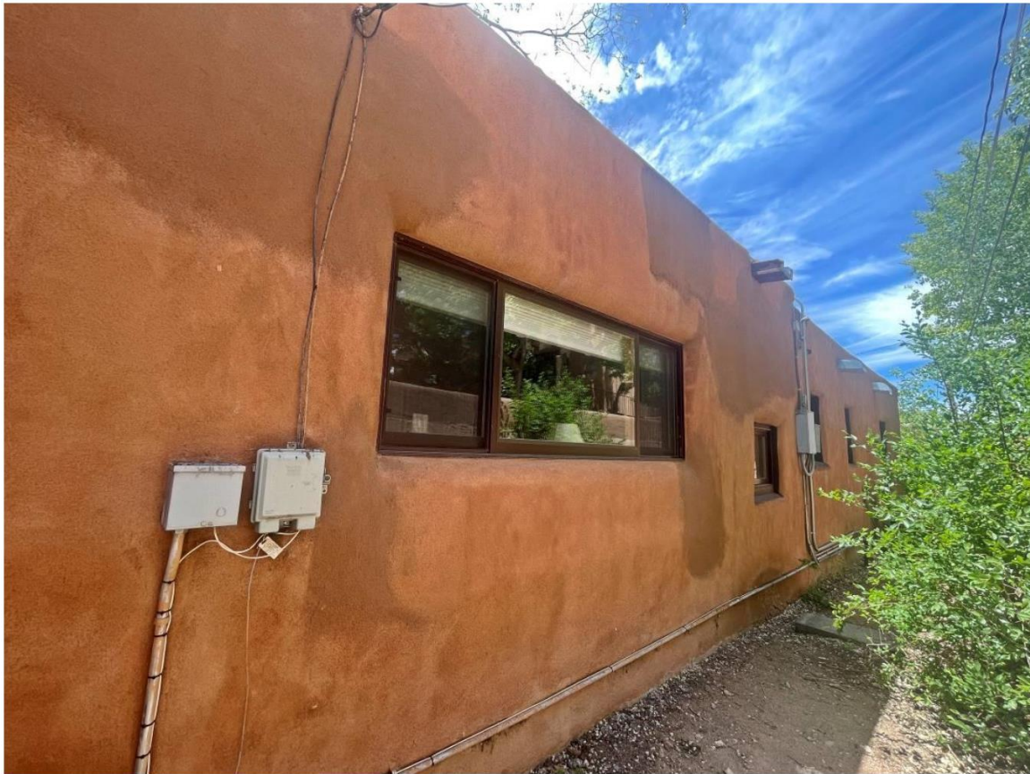
Photo 16: North elevation, oblique. Camera facing southwest. May 20, 2024.
