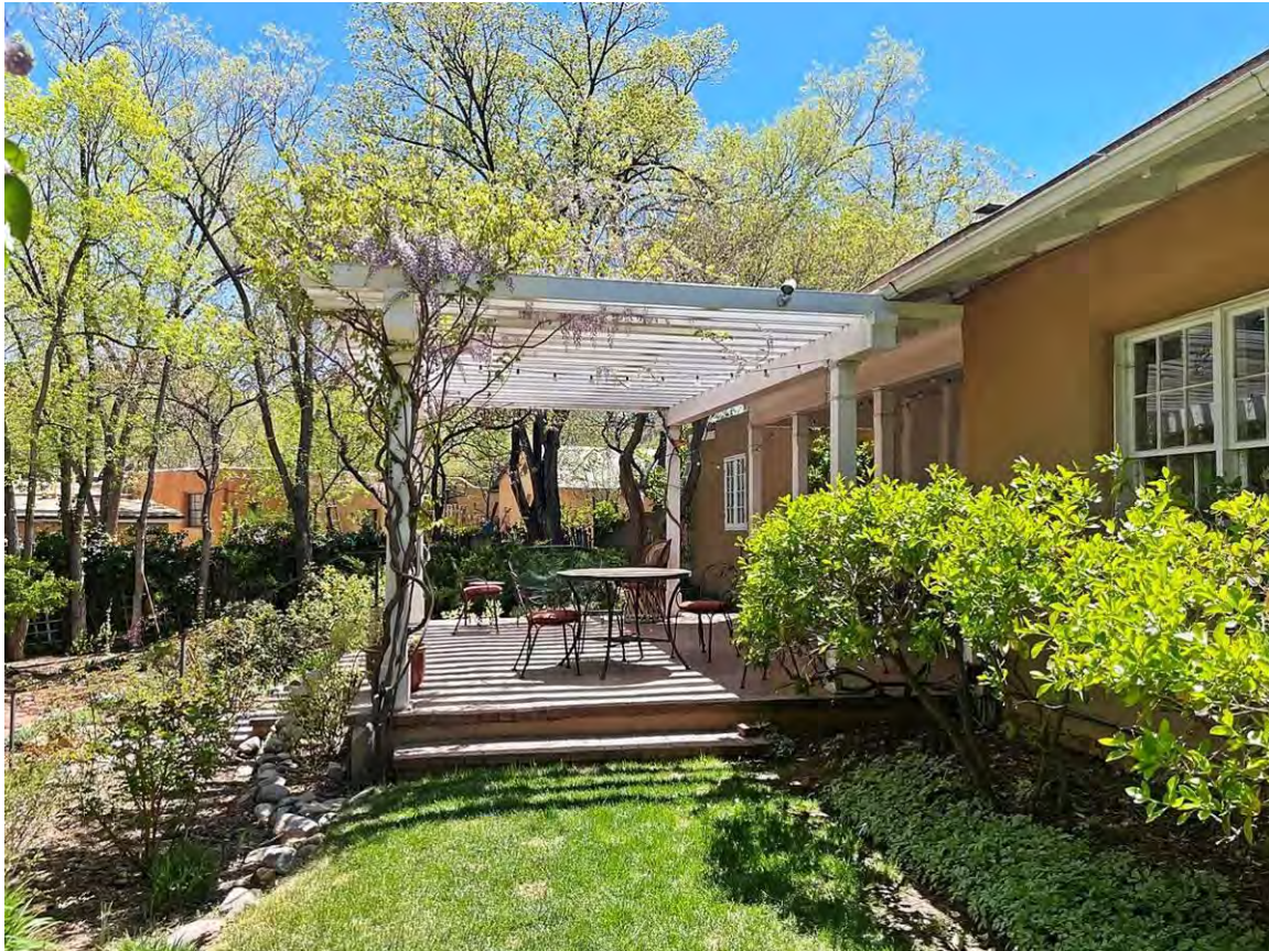
Photo 20: North elevation, ramada shade structure. Camera facing east.
