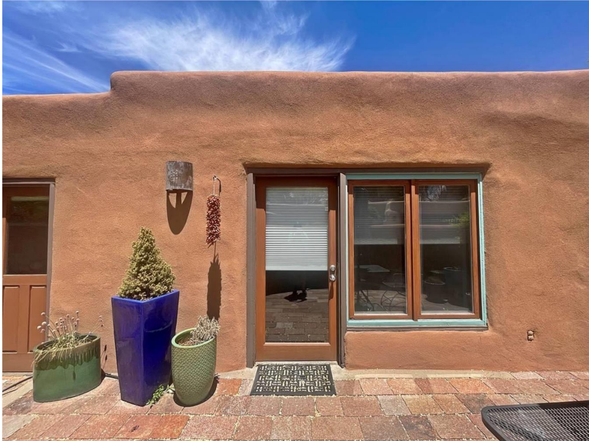
Photo 19: South elevation, east section. Camera facing north. May 20, 2024.
