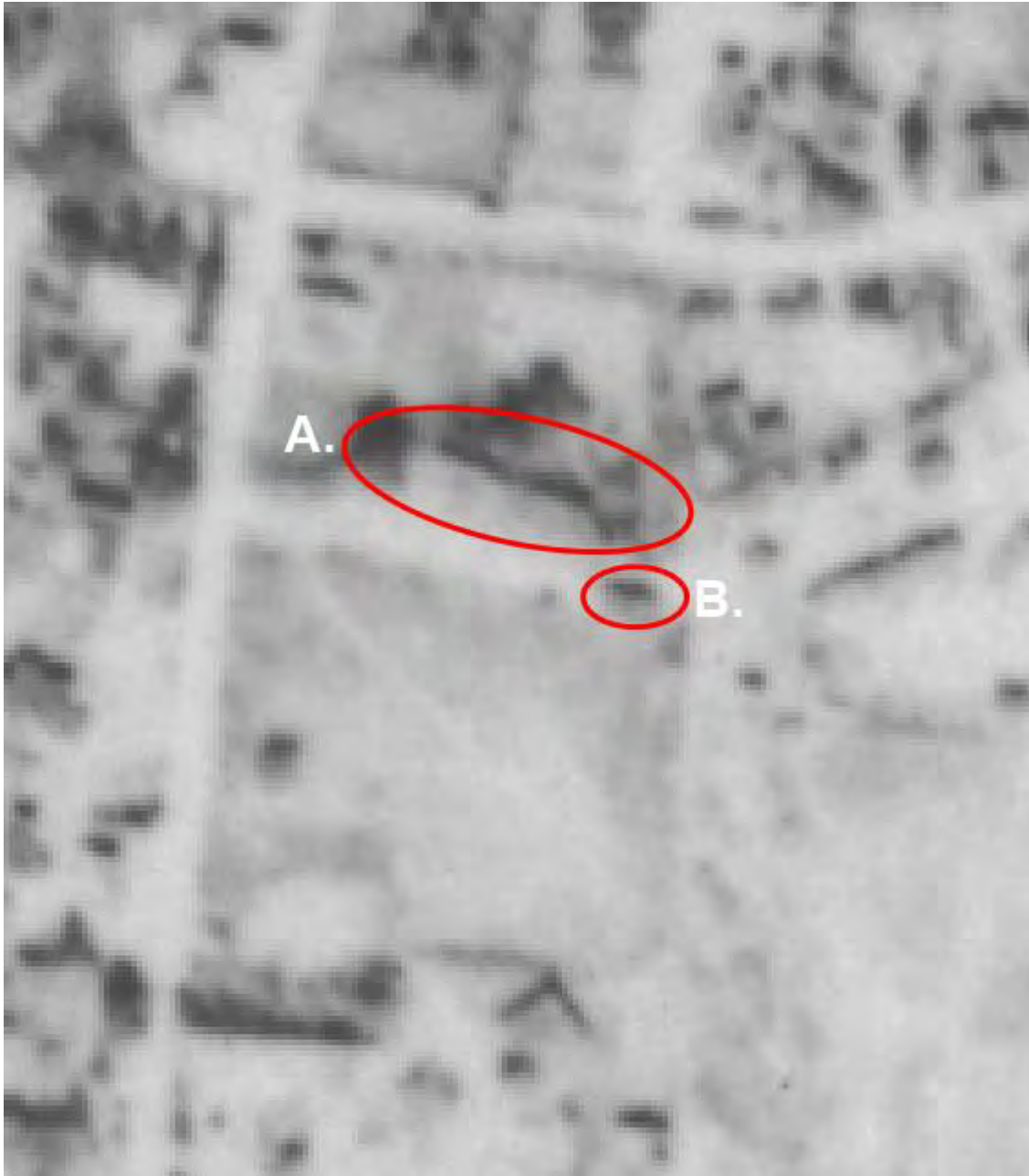
Figure 13: October 25, 1948, aerial photograph. A. Main house; B. Guesthouse.
