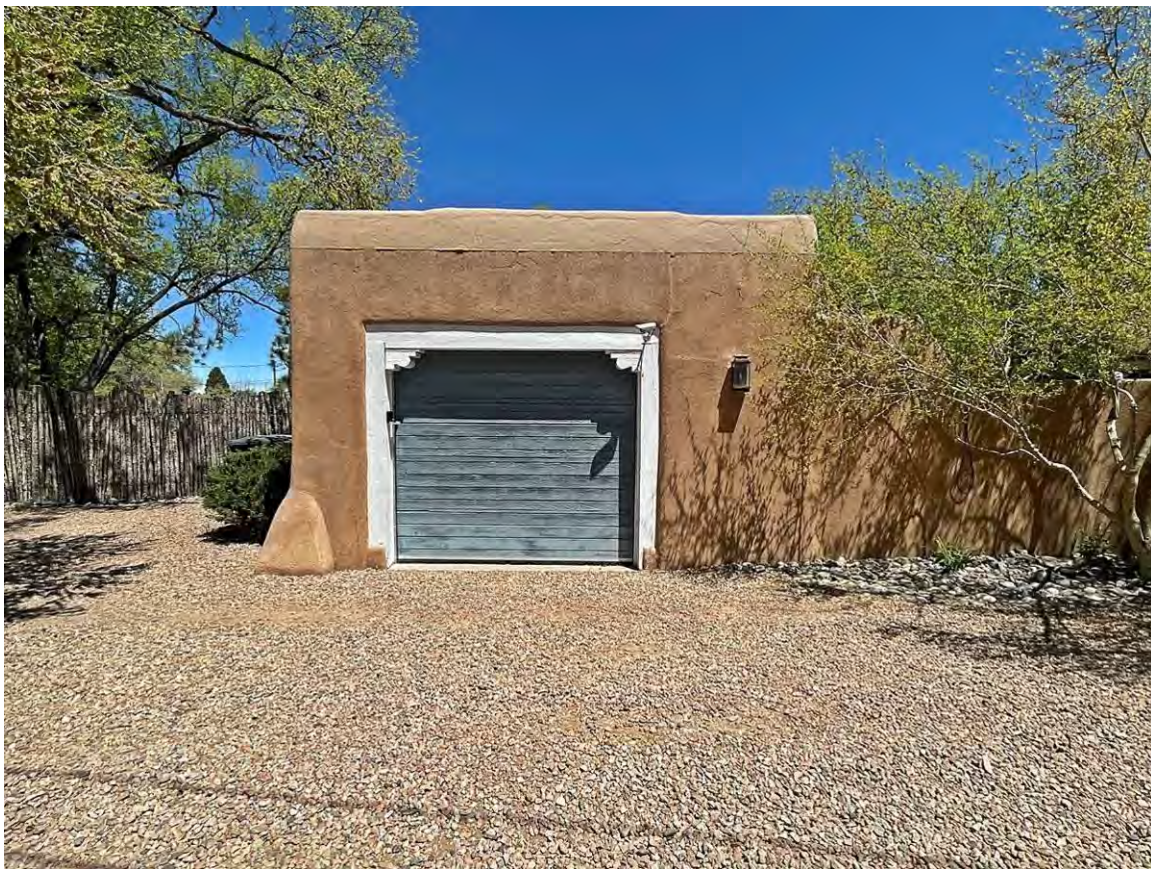
Photo 30: South elevation. Camera facing north.
