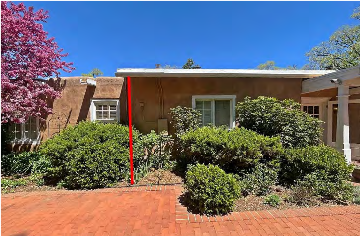
Photo 9: South elevation, where flat roof section meets gabled section. Camera facing north.
