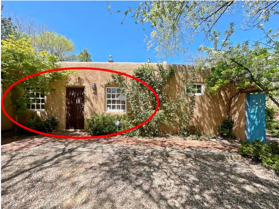
Photo 13: East elevation. New fenestration circled. Camera facing west.
