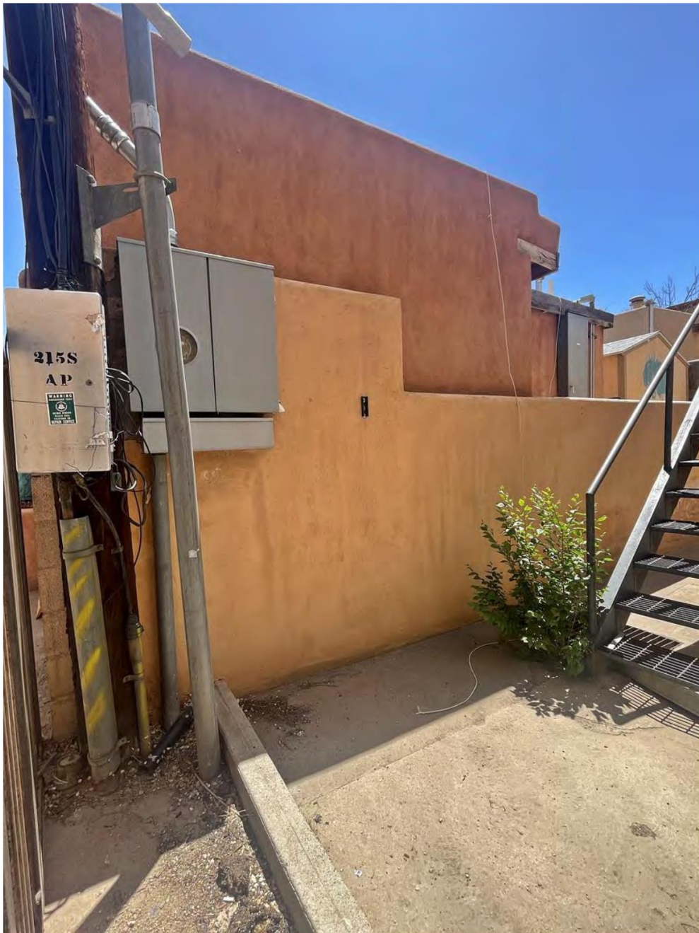
Photo 4: West elevation. Camera facing southeast.
