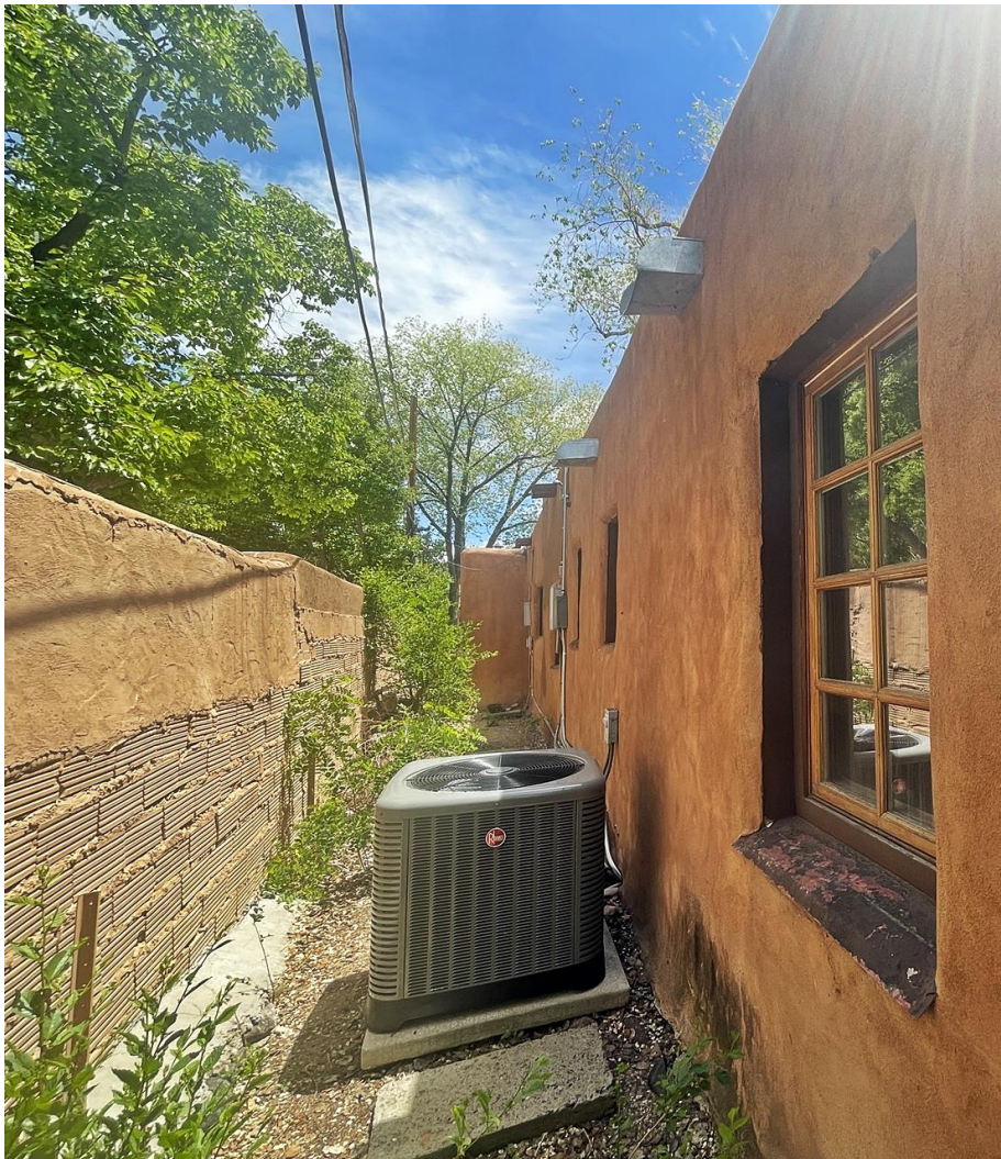
Photo 5: North elevation, oblique. Camera facing east. May 20, 2024.
