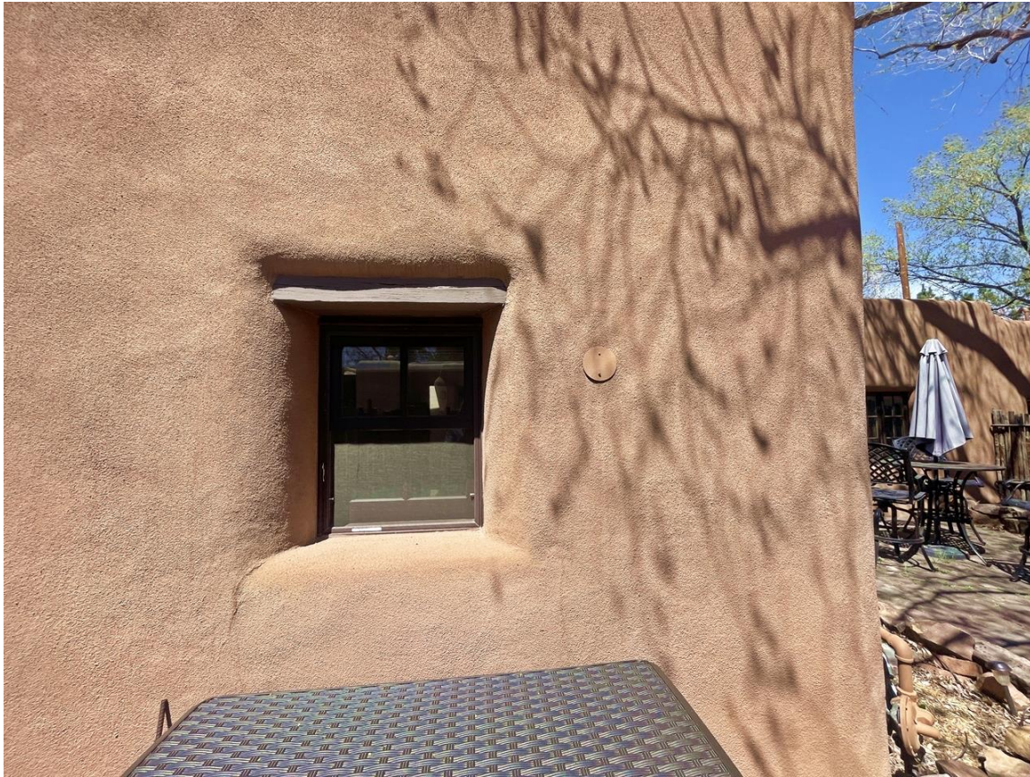
Photo 4: South elevation. Window at kitchen. Camera facing north.
