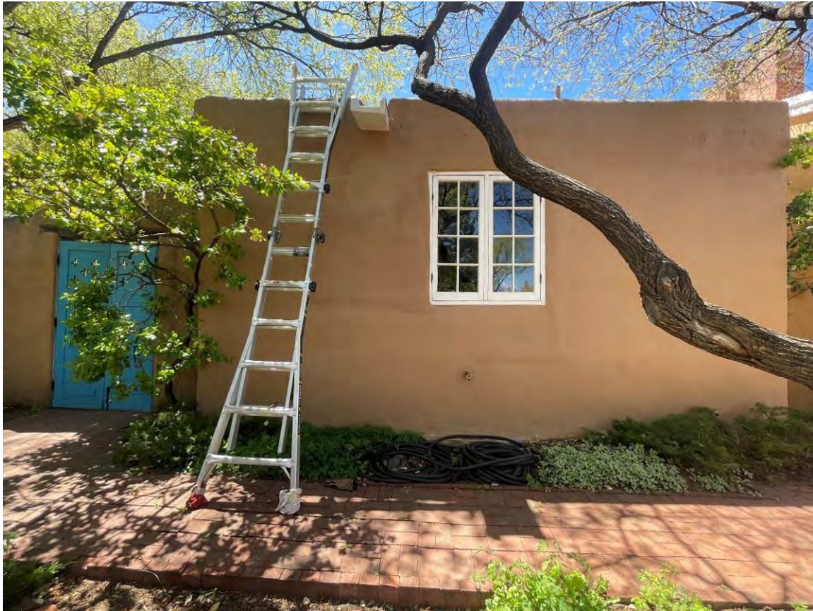
Photo 17: North elevation, kitchen addition. Camera facing south.
