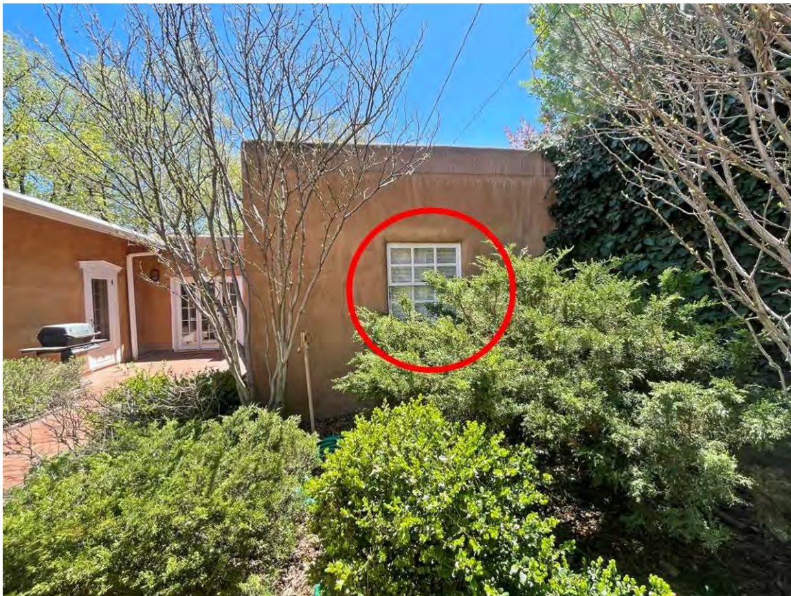
Photo 24: West elevation, altered window circled. Camera facing east.
