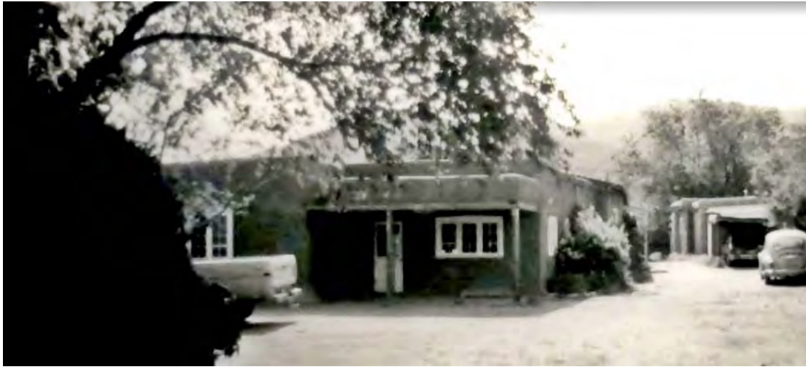
Figure 2: March 6, 1983, HBI survey photograph. Michael Belshaw. West side of building complex. Camera facing east. Courtesy NMCRIIS.
