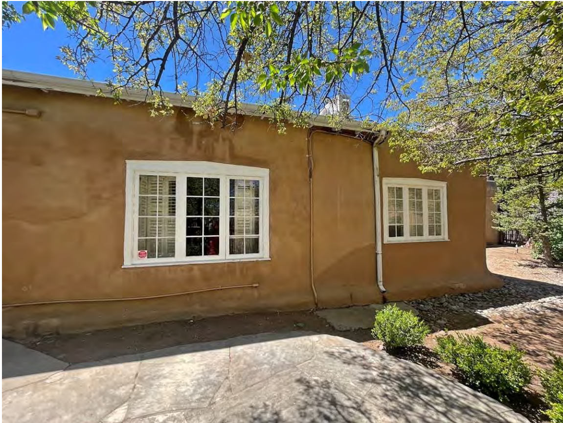
Photo 22: North elevation, west end. Camera facing southwest.
