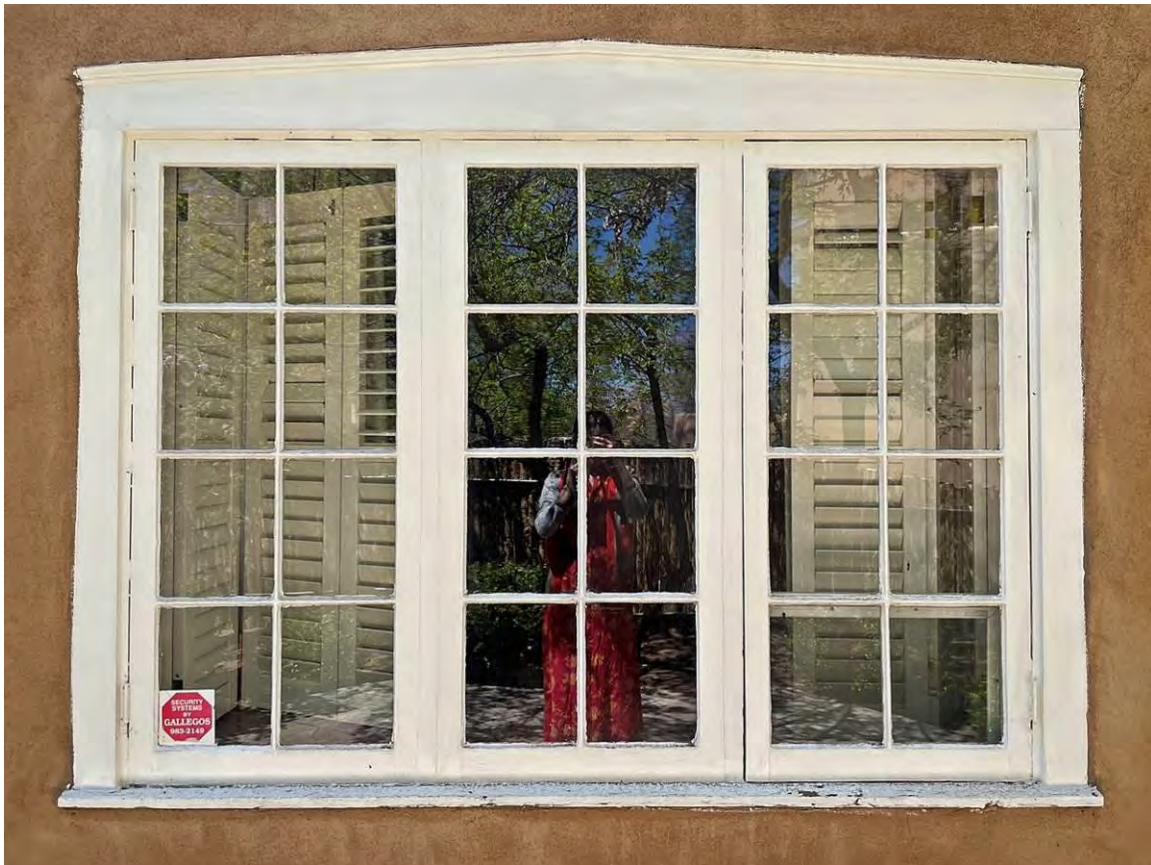
Photo 23: North elevation, detail of older window. Camera facing south.
