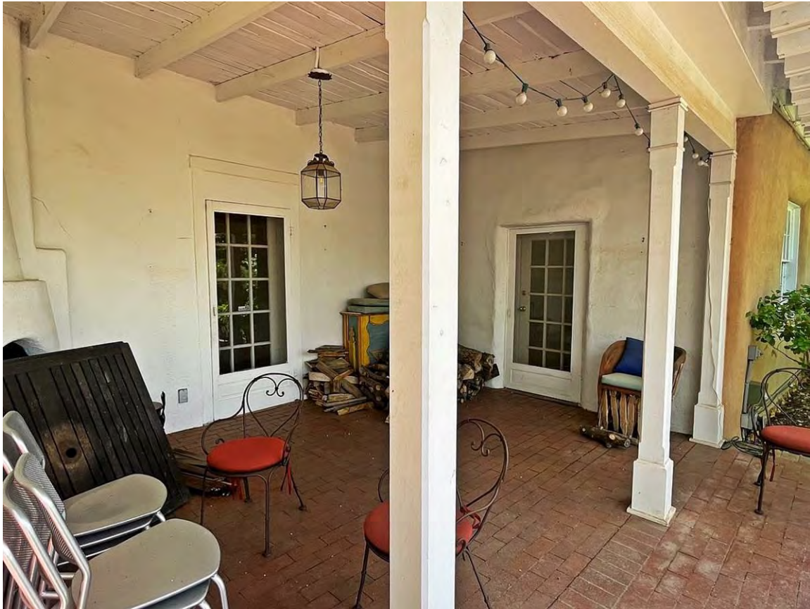
Photo 19: North elevation, portal. Camera facing southwest.
