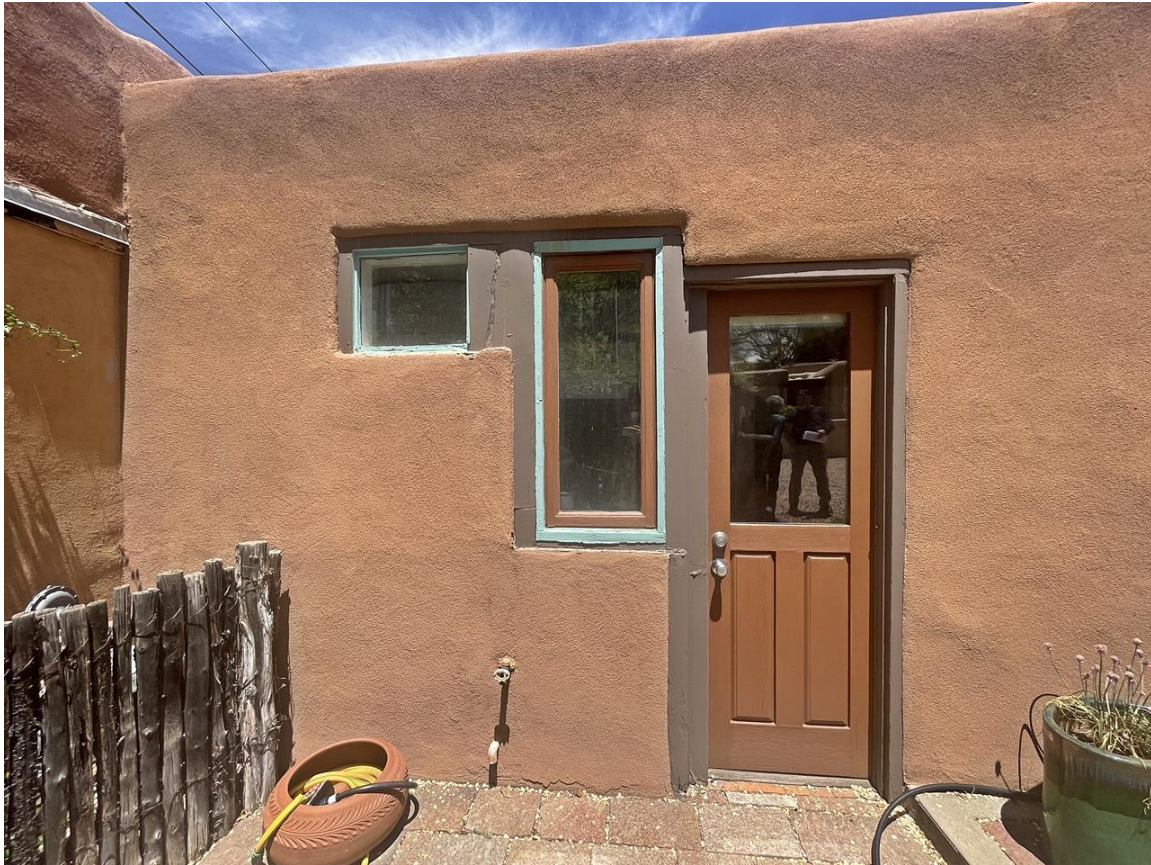
Photo 8: South elevation, west section. Camera facing northwest. May 20, 2024.
