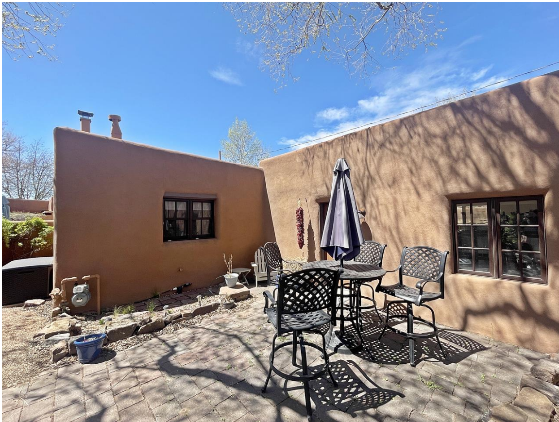
Photo 2: East and south elevation oblique. Camera facing northwest. April 20, 2024.
