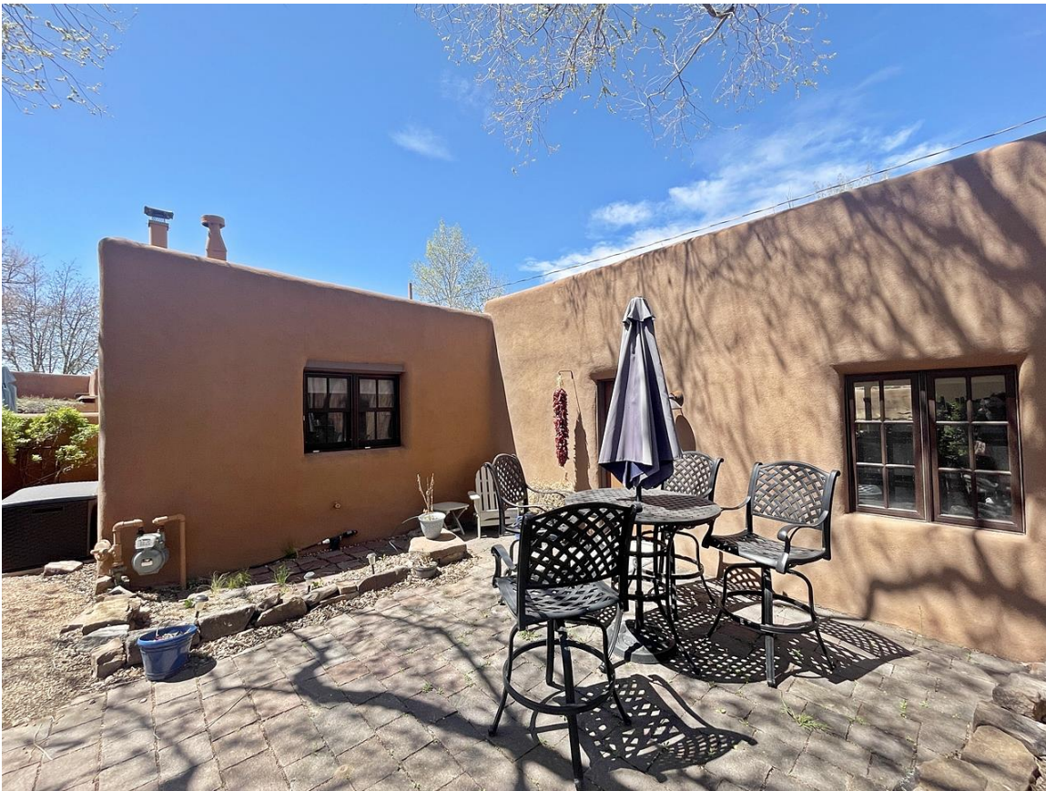
Photo 2: East and south elevation oblique. Camera facing northwest.
