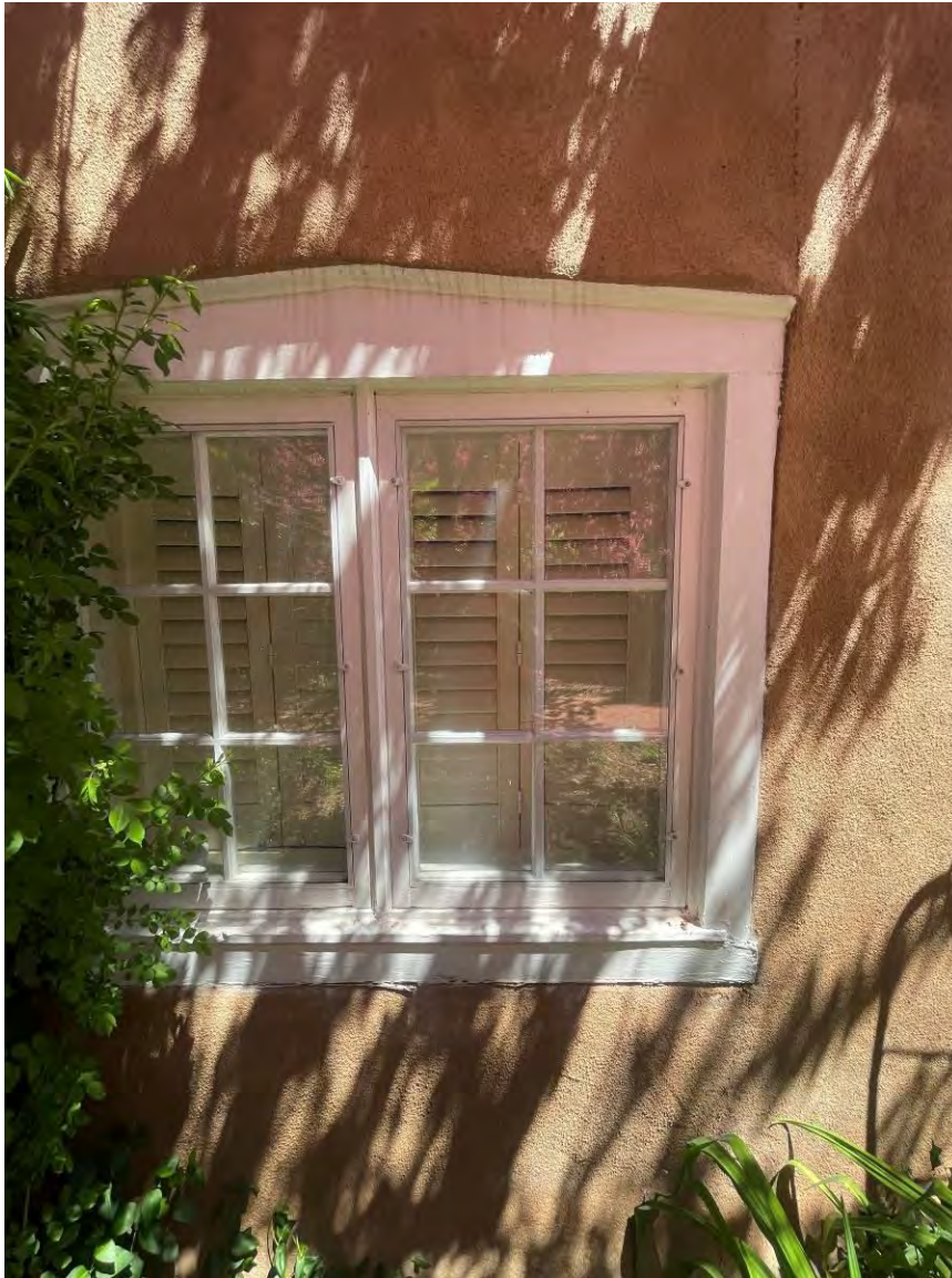
Photo 8: South elevation, older window. Camera facing north.
