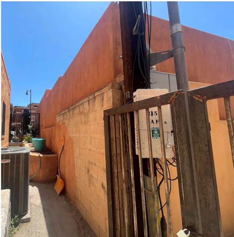
Photo 2: North elevation. Camera facing southeast.
