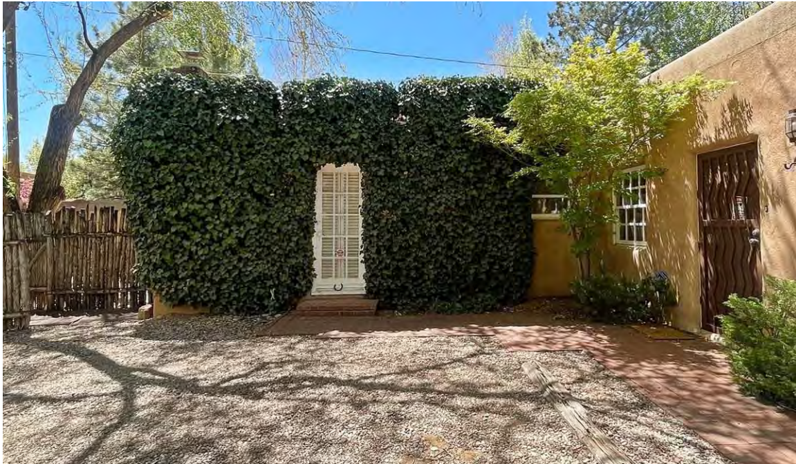
Photo 26: North elevation, representing Severino Vigil home.
