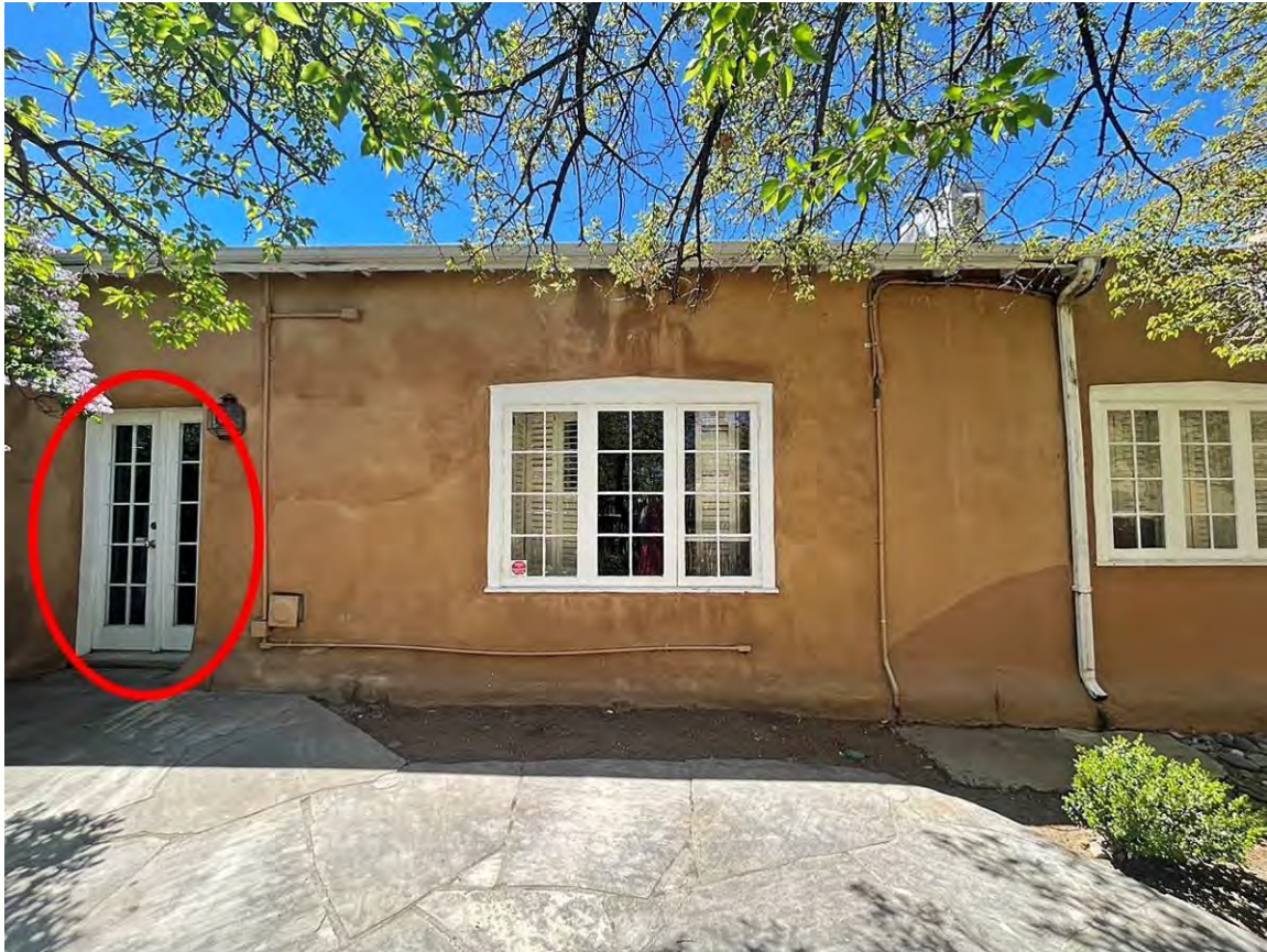
Photo 21: North elevation 1990s door circled. Camera facing southeast.
