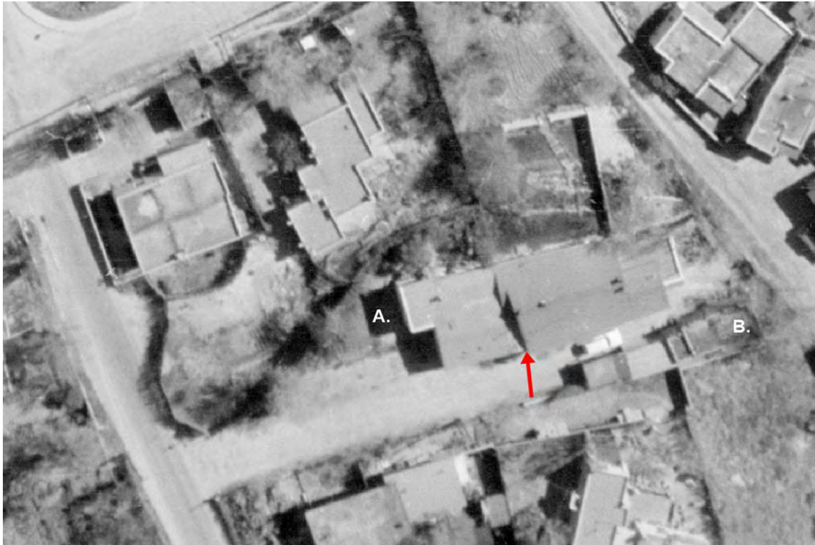
Figure 15: May 11, 1973, aerial photograph. A. Main house; B. Guesthouse. The arrow indicates that dwellings have been joined together.
