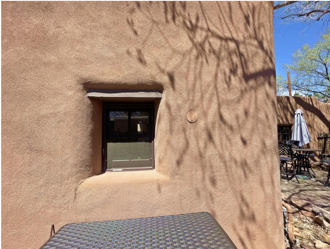
Photo 4: South elevation. Window at kitchen. Camera facing north. April 20, 2024.
