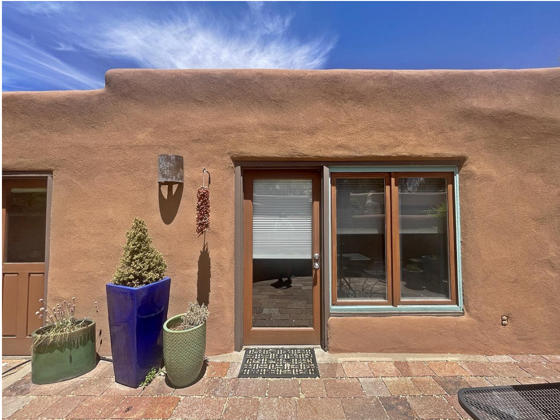
Photo 7: South elevation, east section. Camera facing north. May 20, 2024.
