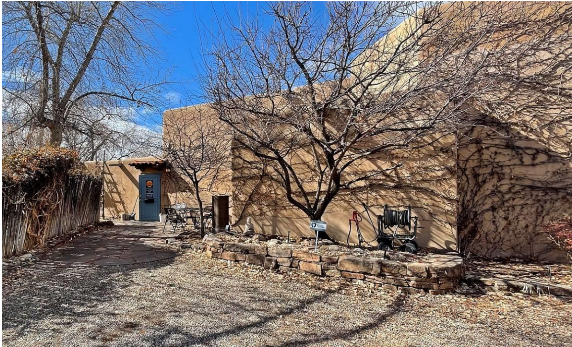
Photo 8: East elevation. Camera facing southwest.
