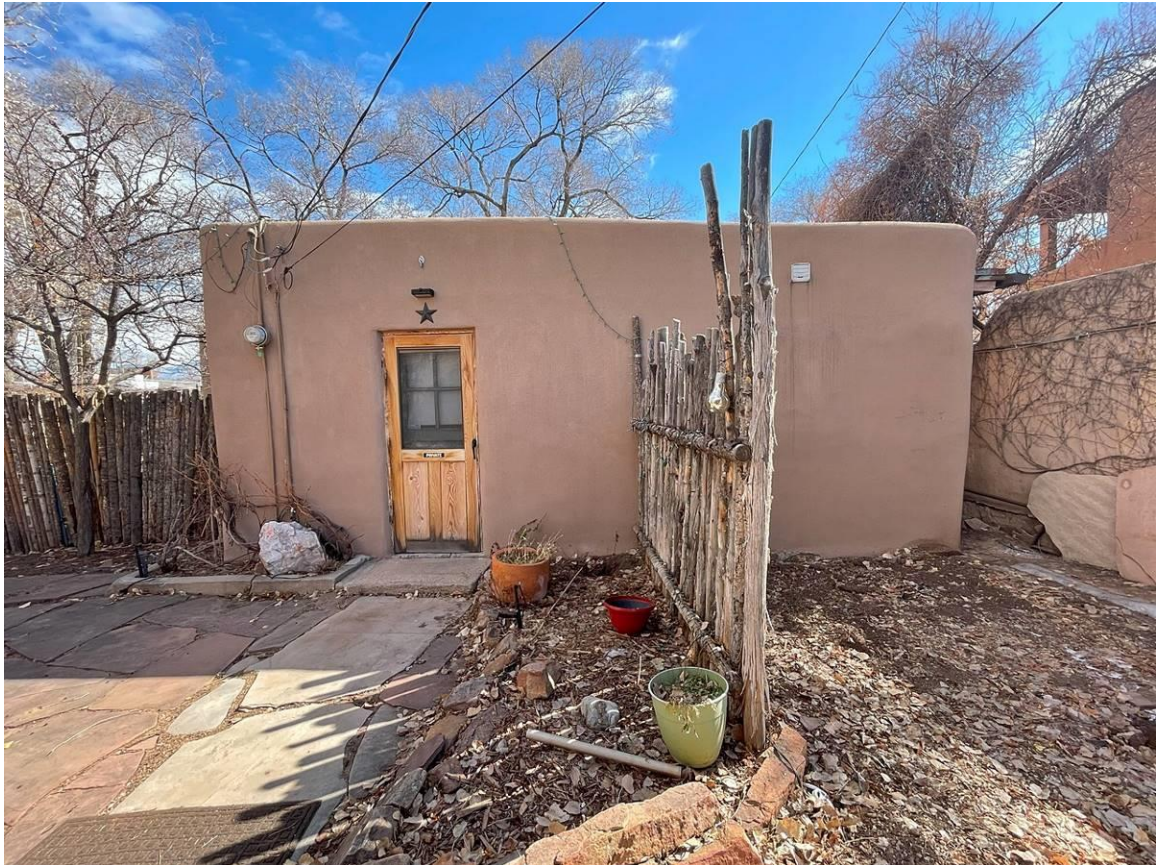
Photo 5: West elevation. Camera facing east.
