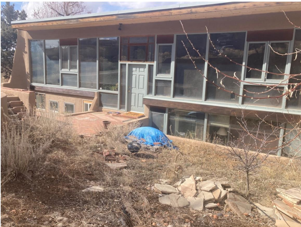
1072 Camino San Acacio, South elevation. View from private yard. No proposed changes.
