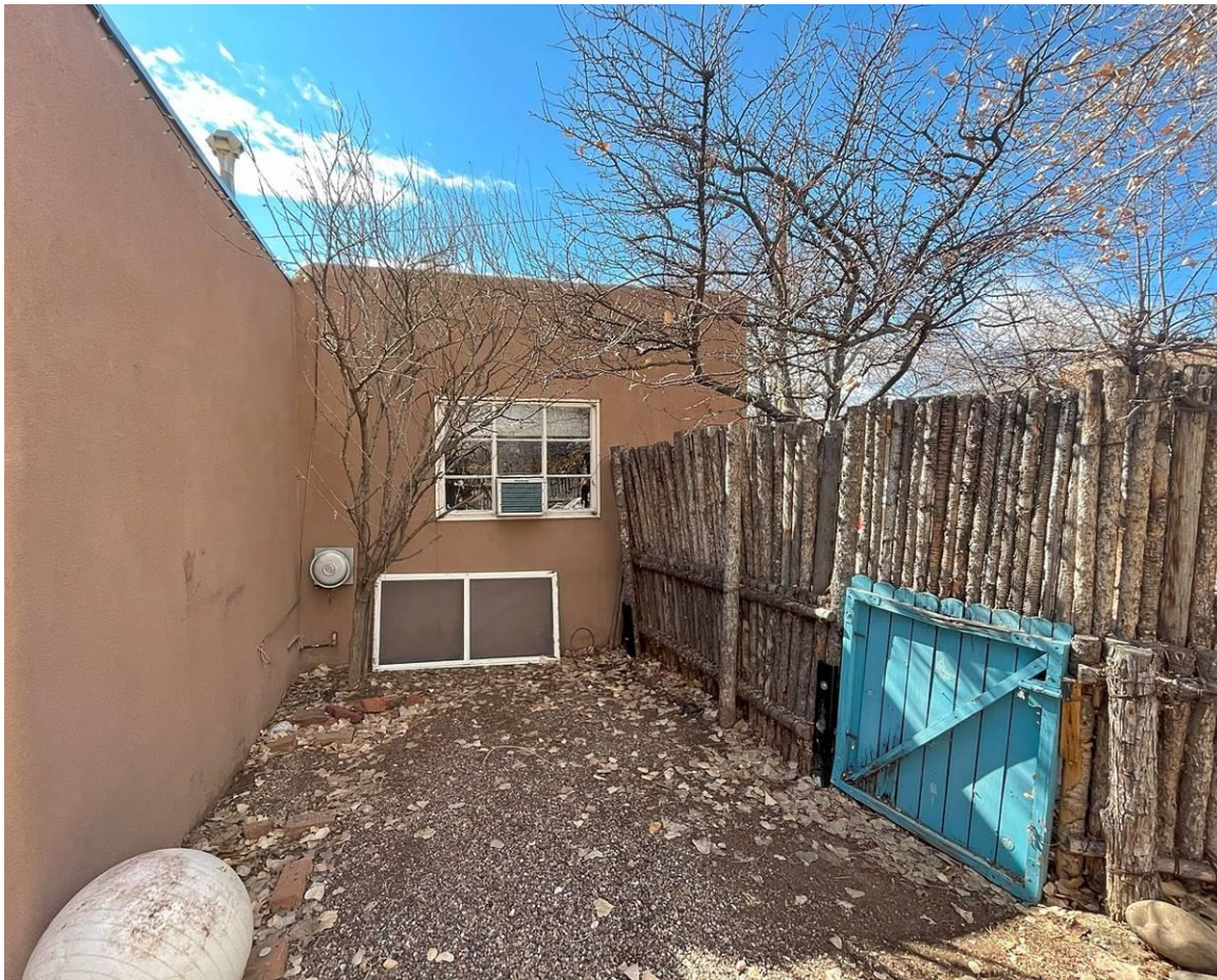
Photo 4: West and north elevations. Camera facing south.
