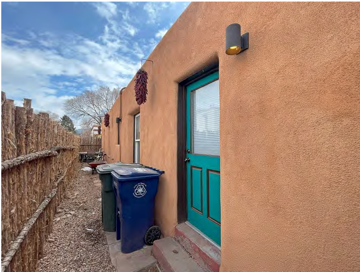
Photo 2: West elevation. Camera facing east.
