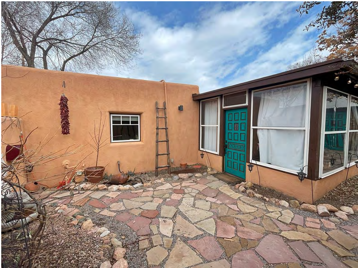
Photo 6: South elevation and sunroom. Camera facing northeast.
