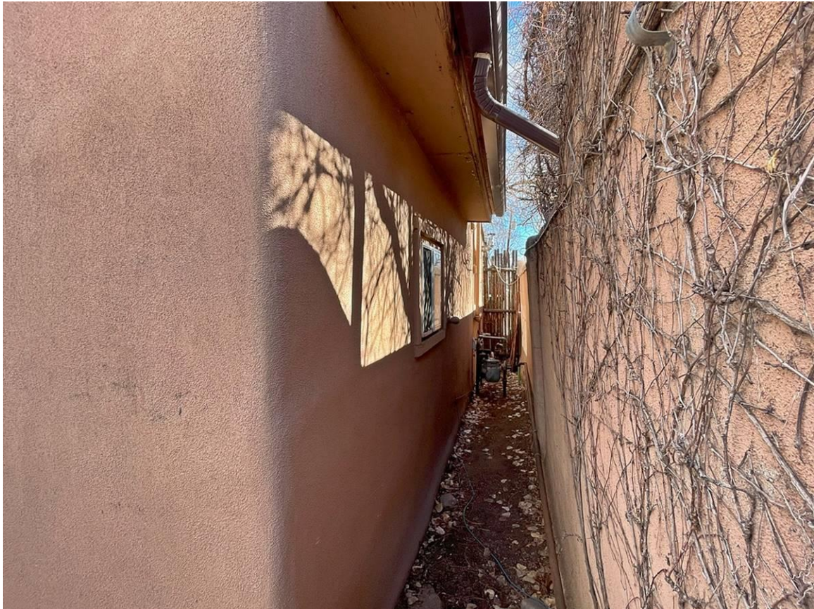
Photo 6: South elevation. Camera facing east.
