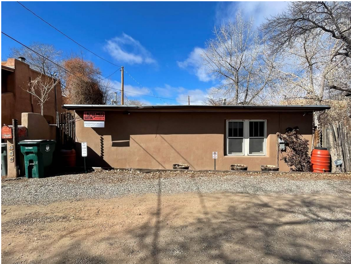
Photo 2: East elevation. Camera facing west.
