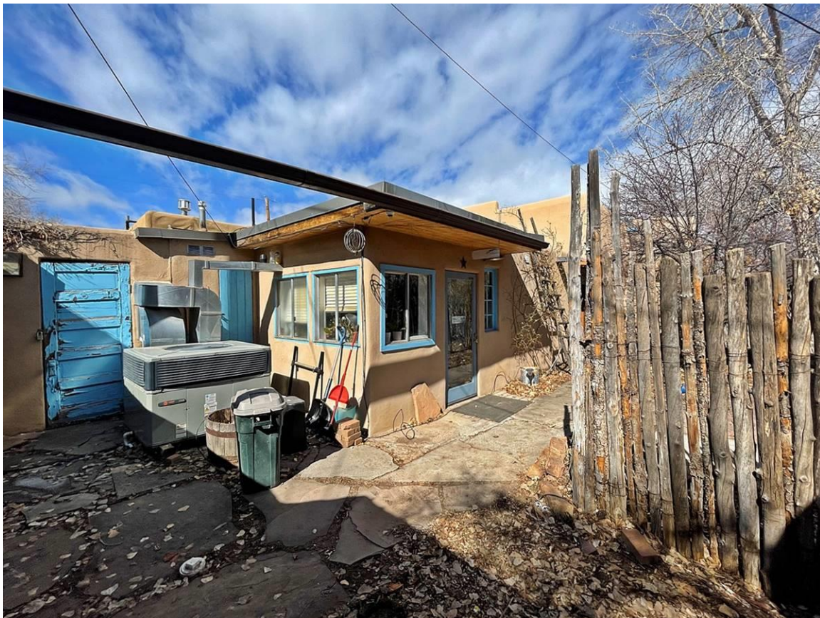
Photo 7: Southeast corner. Camera facing northwest.
