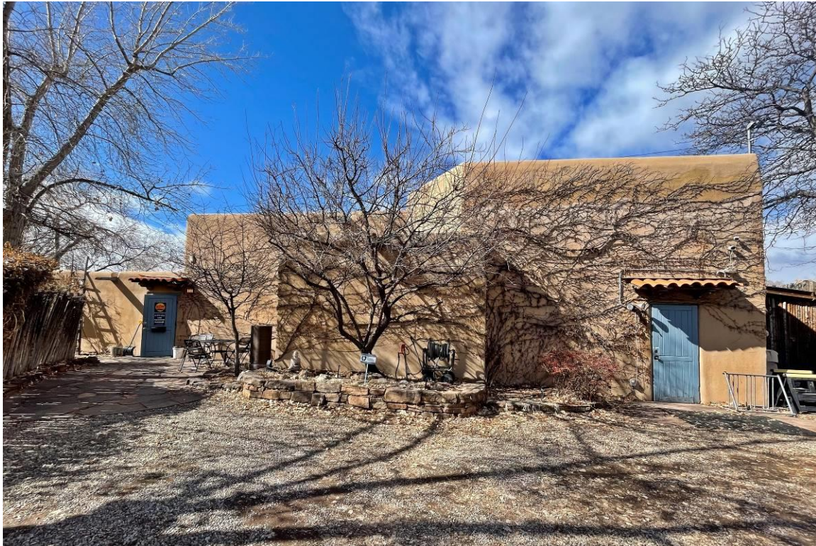
Photo 9: East elevation. Camera facing west.
