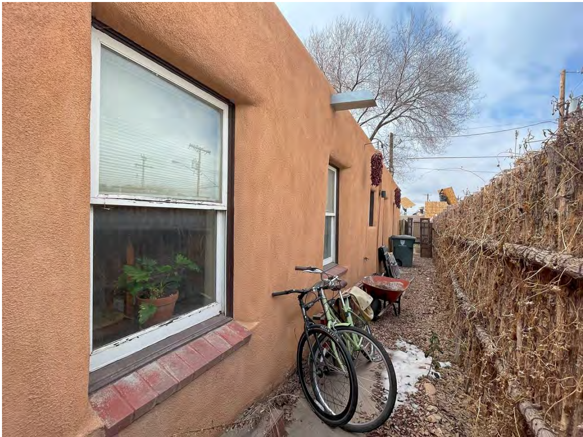
Photo 3: North elevation. Camera facing southwest.
