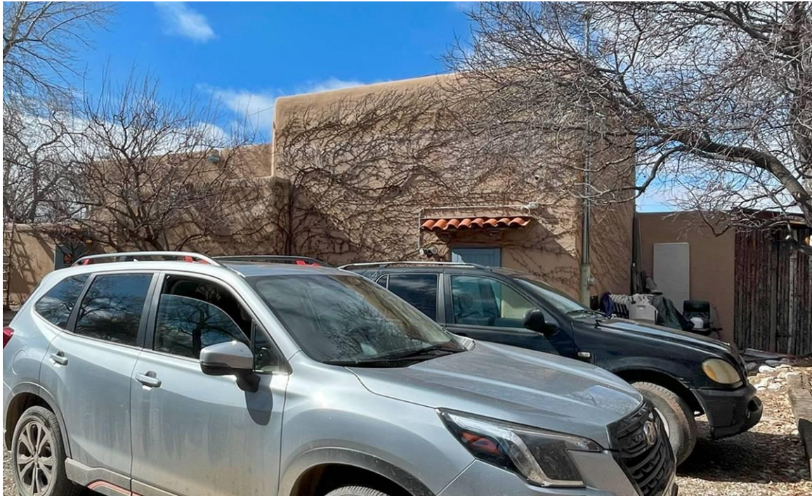
Photo 10: East elevation. Camera facing southwest.
