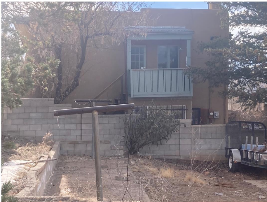
1072 Camino San Acacio, East elevation of main house. No proposed changes.
