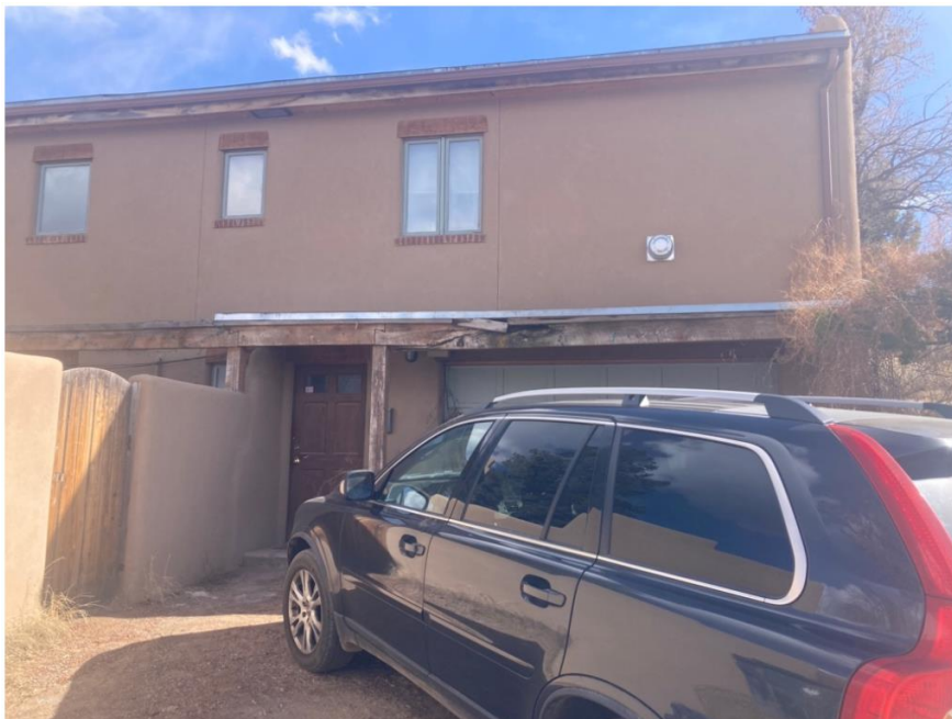
1072 Camino San Acacio, North elevation (right side). View from driveway (access road). 79 sf addition will be visible here, replacing right (west) end of wooden trellis. Yard-wall and gate will move out 10 feet and this parking area will reduce from two spaces to one.
