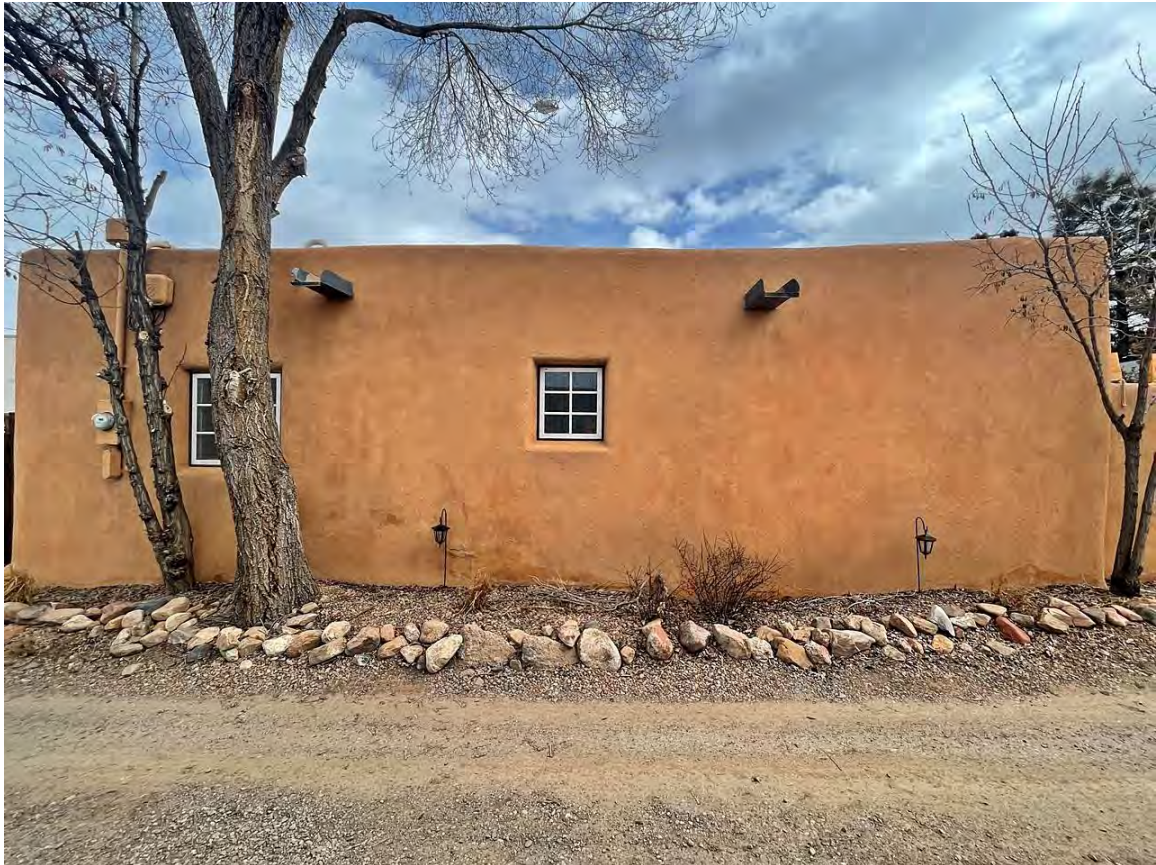
Photo 4: West elevation. Camera facing east.
