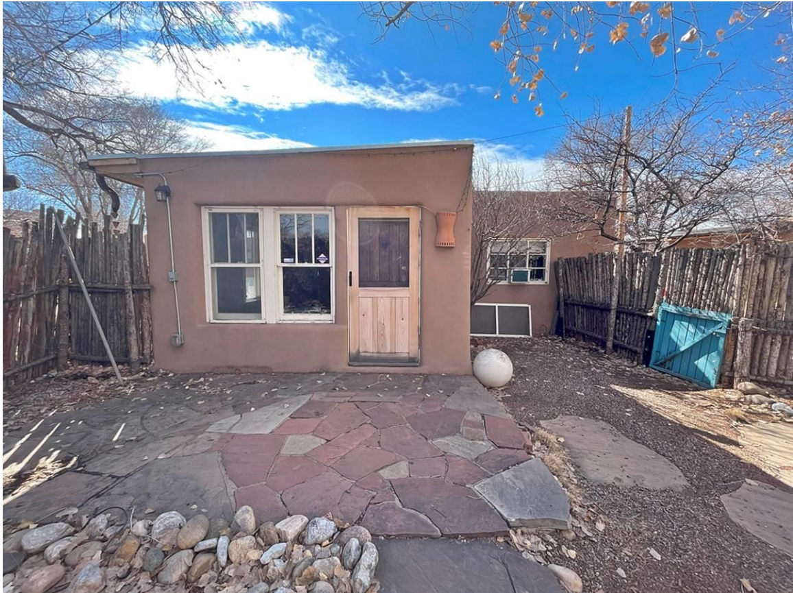
Photo 3: North elevation. Camera facing south.
