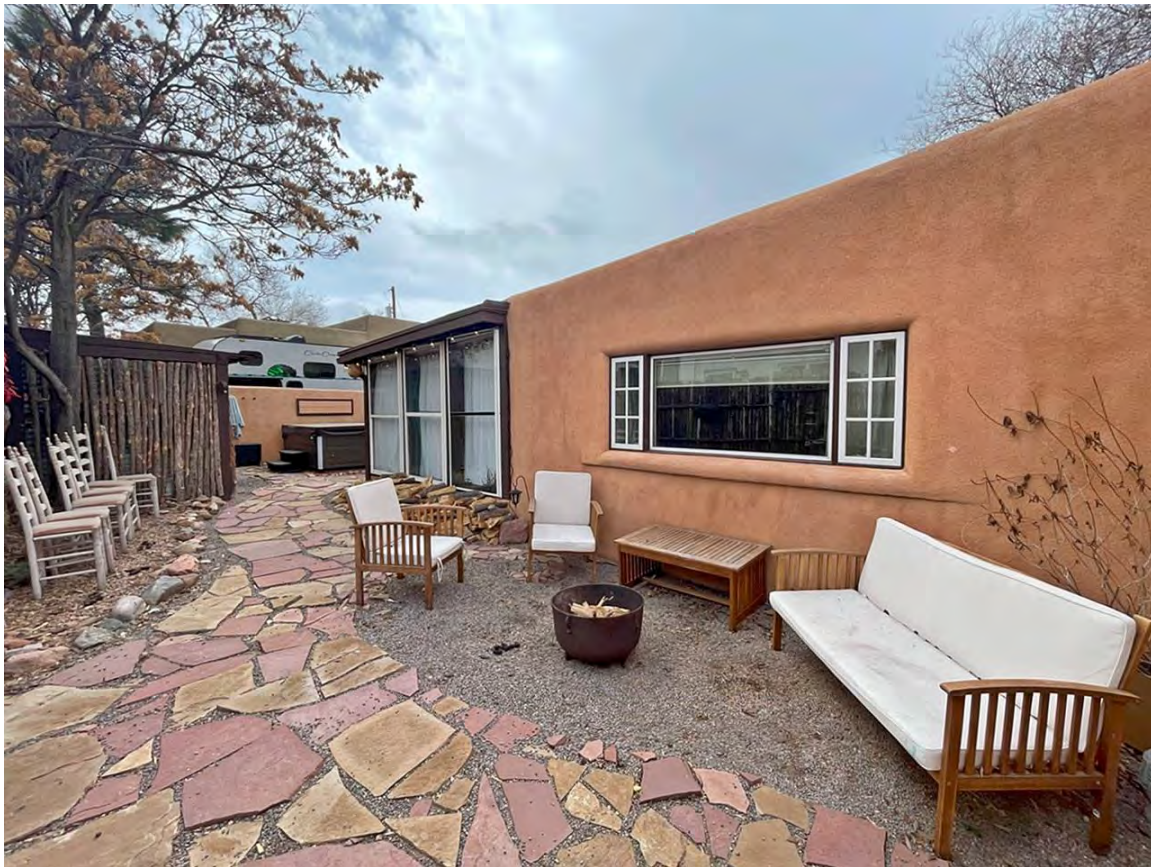
Photo 8: East elevation. Camera facing southwest.
