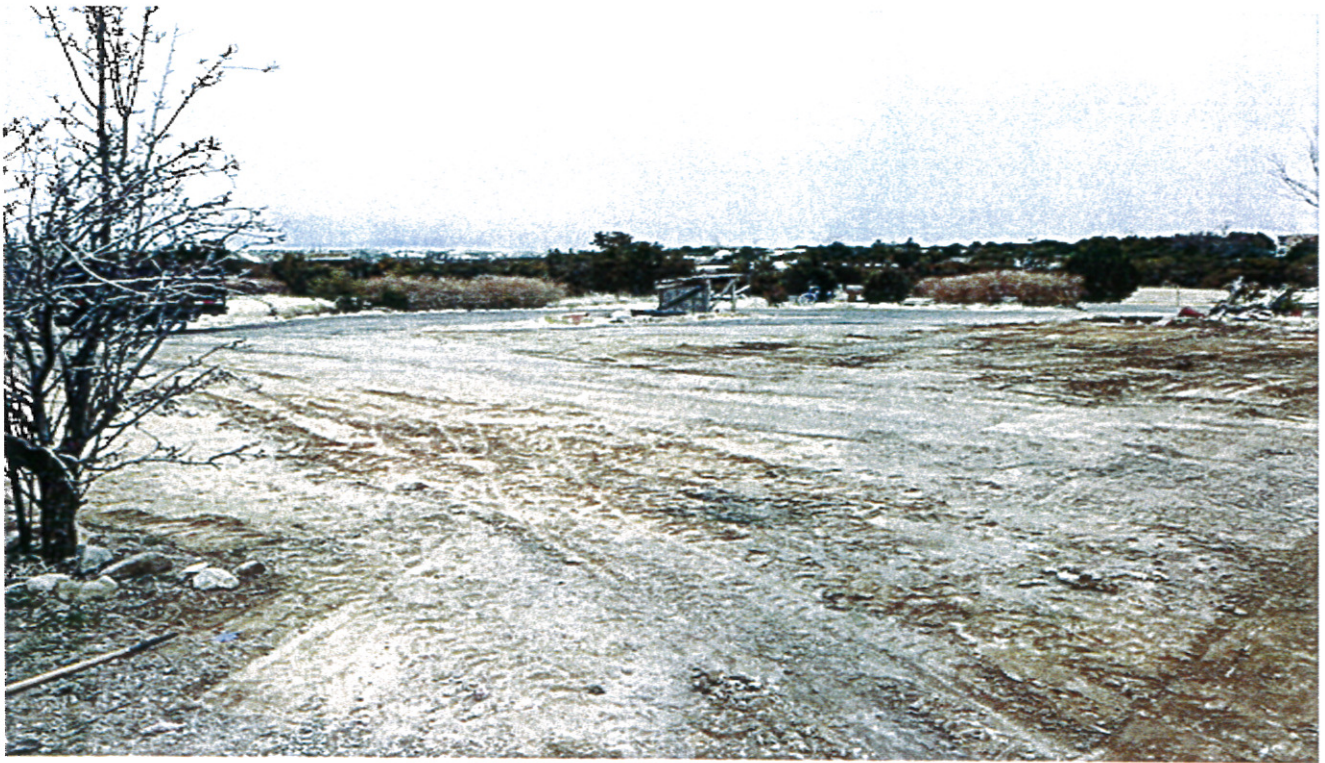
Photo No. 3 View of property after the house demolition. Photo taken 3/8/24.
