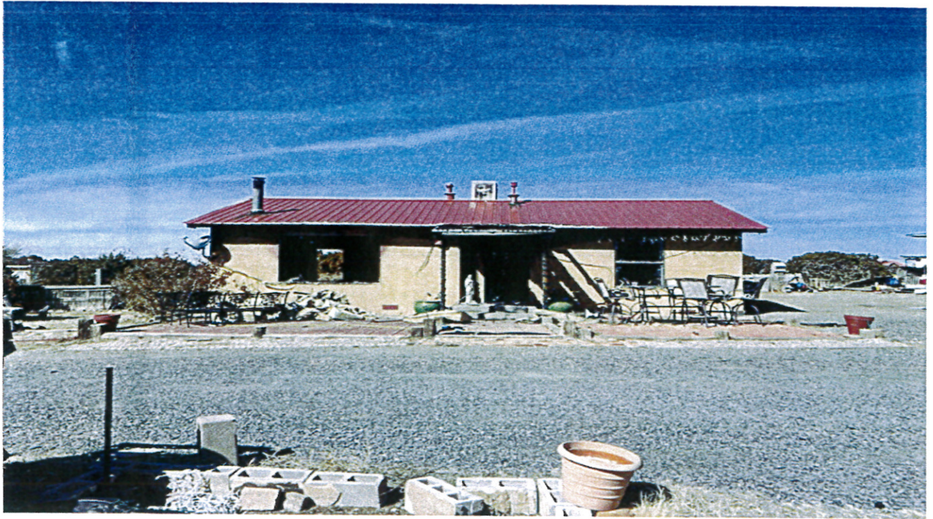
Photo No. 1 Front view of burnt house. Photo taken 2/20/24.
