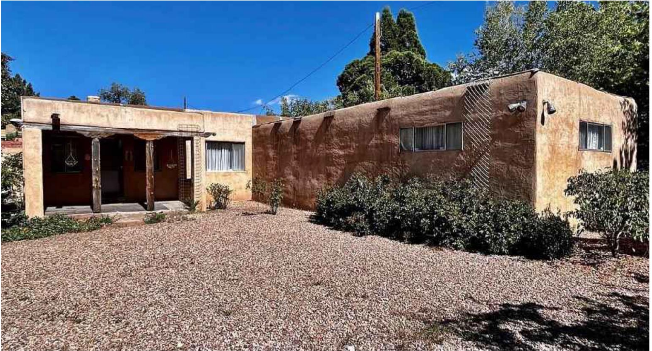
HOUSE SOUTH AND PARTIAL WEST ELEVATION
