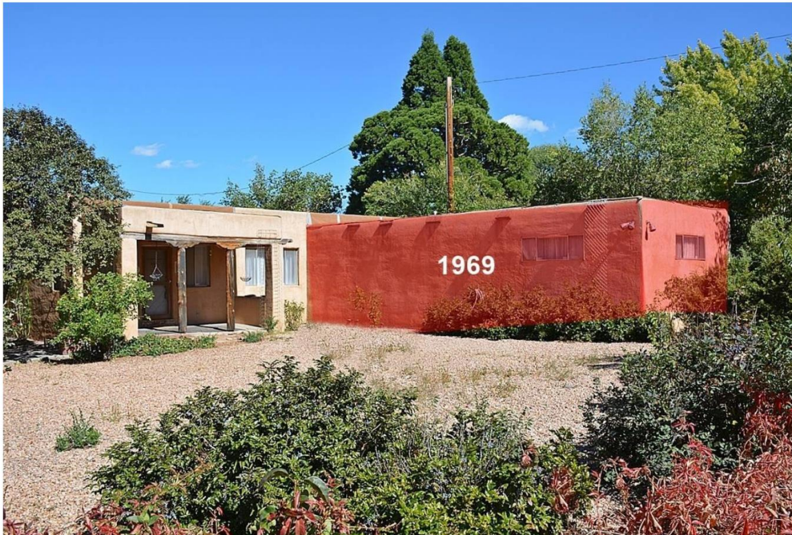
Photo 2: Original Older House, with 1969 Bedroom Wing Addition. Camera facing northeast.
