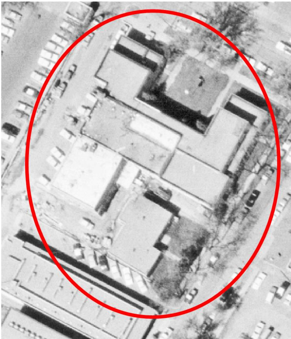
Figure 9: 1958 aerial photograph. Note the original window pattern across the east elevation.
