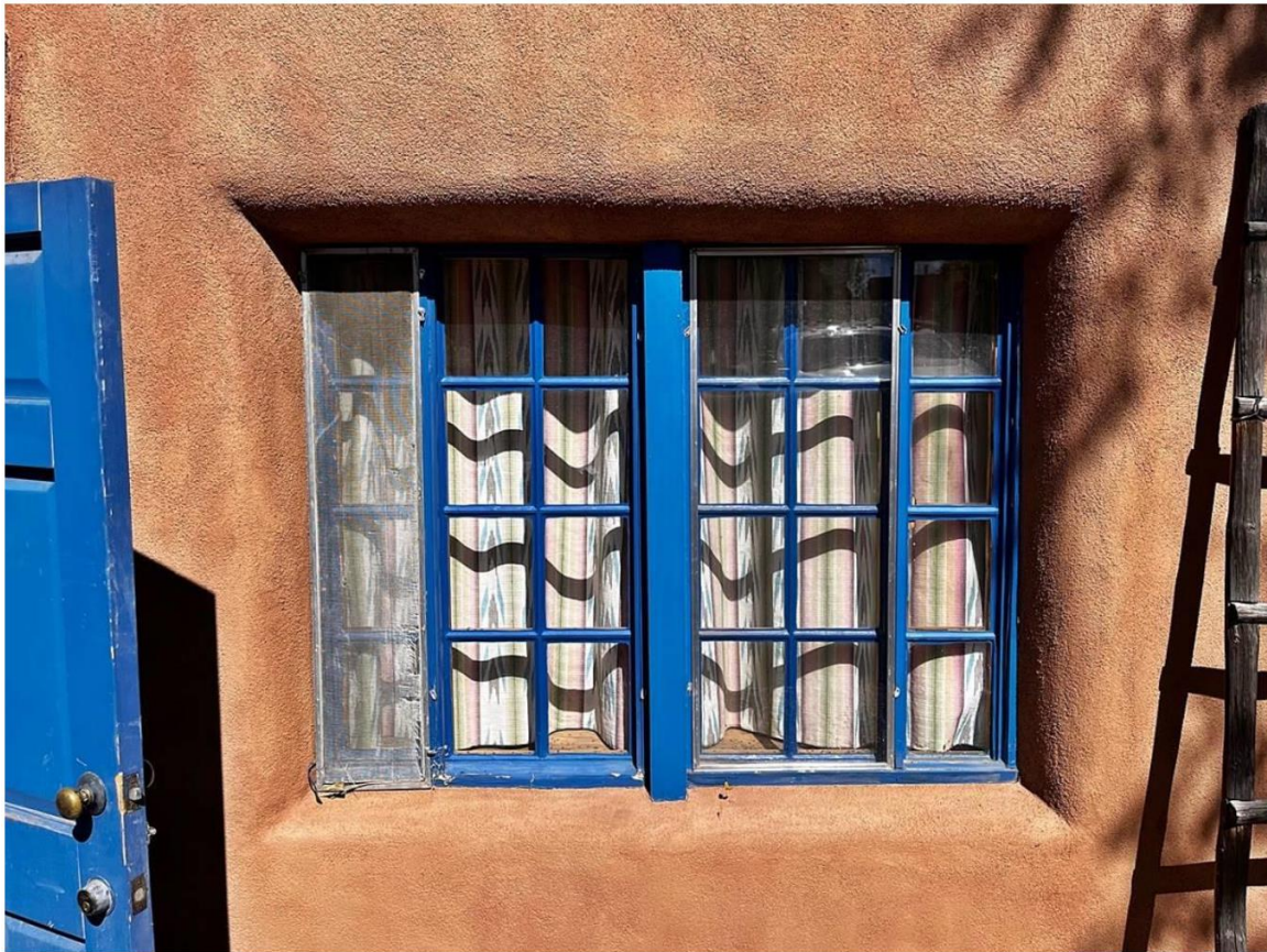
Photo 8: South elevation. Window at sala/living room area. Camera facing north.
