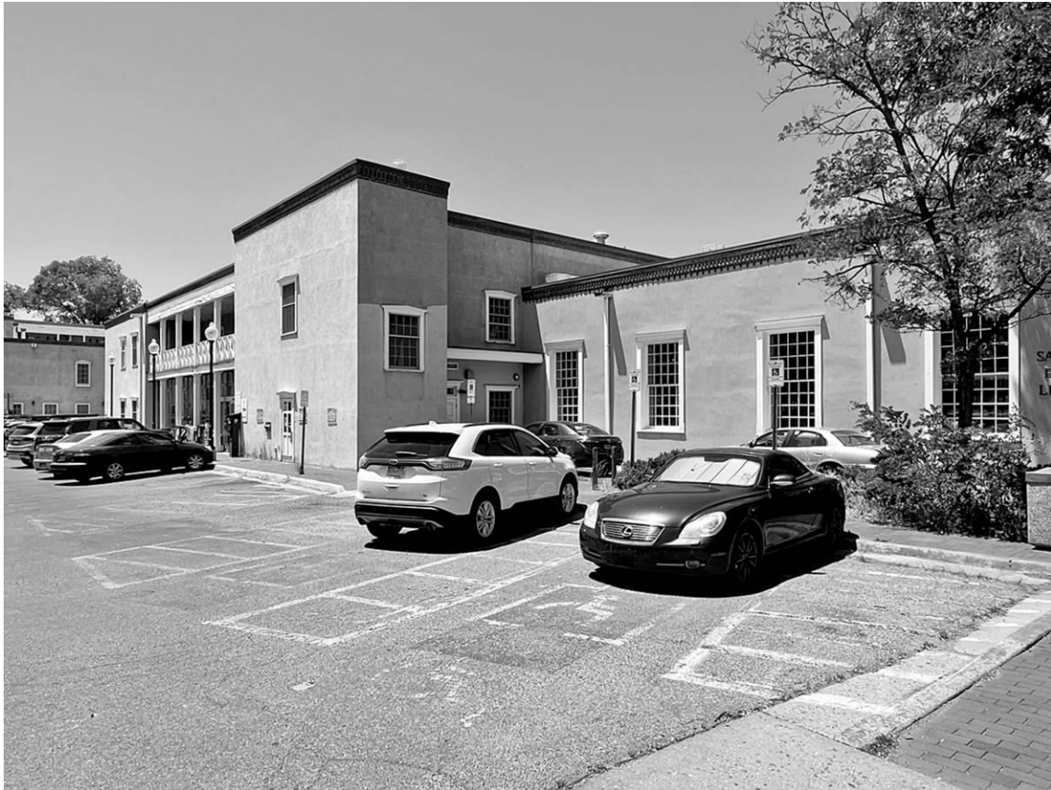
Photo 14. East elevation. Area left of white area is 1980s construction. Camera facing southwest.
