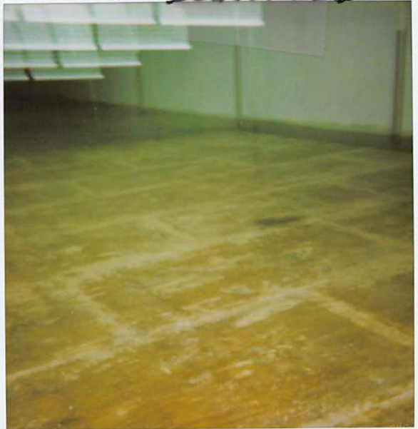
58 E. SAN FRANCISCO 1ST FLOOR WOOD SHEATHING 10/26/00
