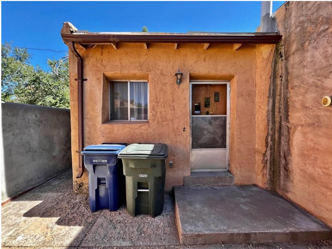
Photo 5: Old House. West elevation entry. Camera facing east.
