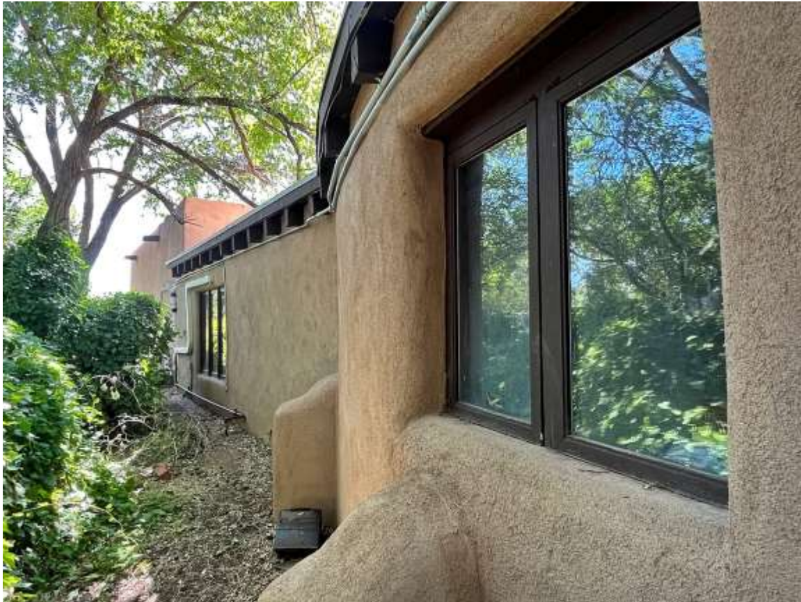
Photo 8: Former studio, guesthouse, and addition. Camera facing northeast.
