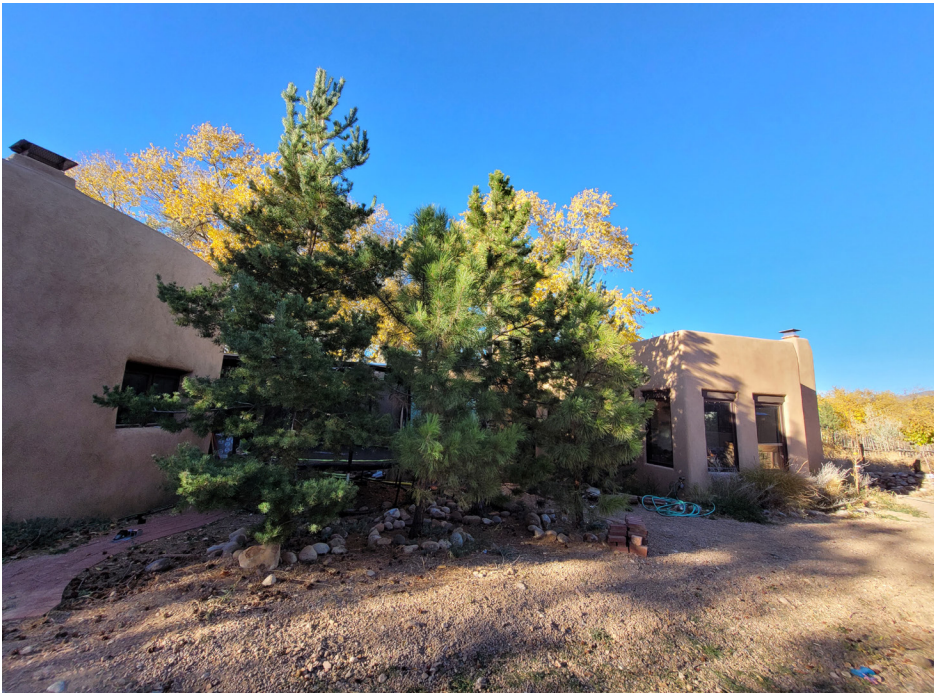
1047 A Camino San Acacio- Partial South Elevation
