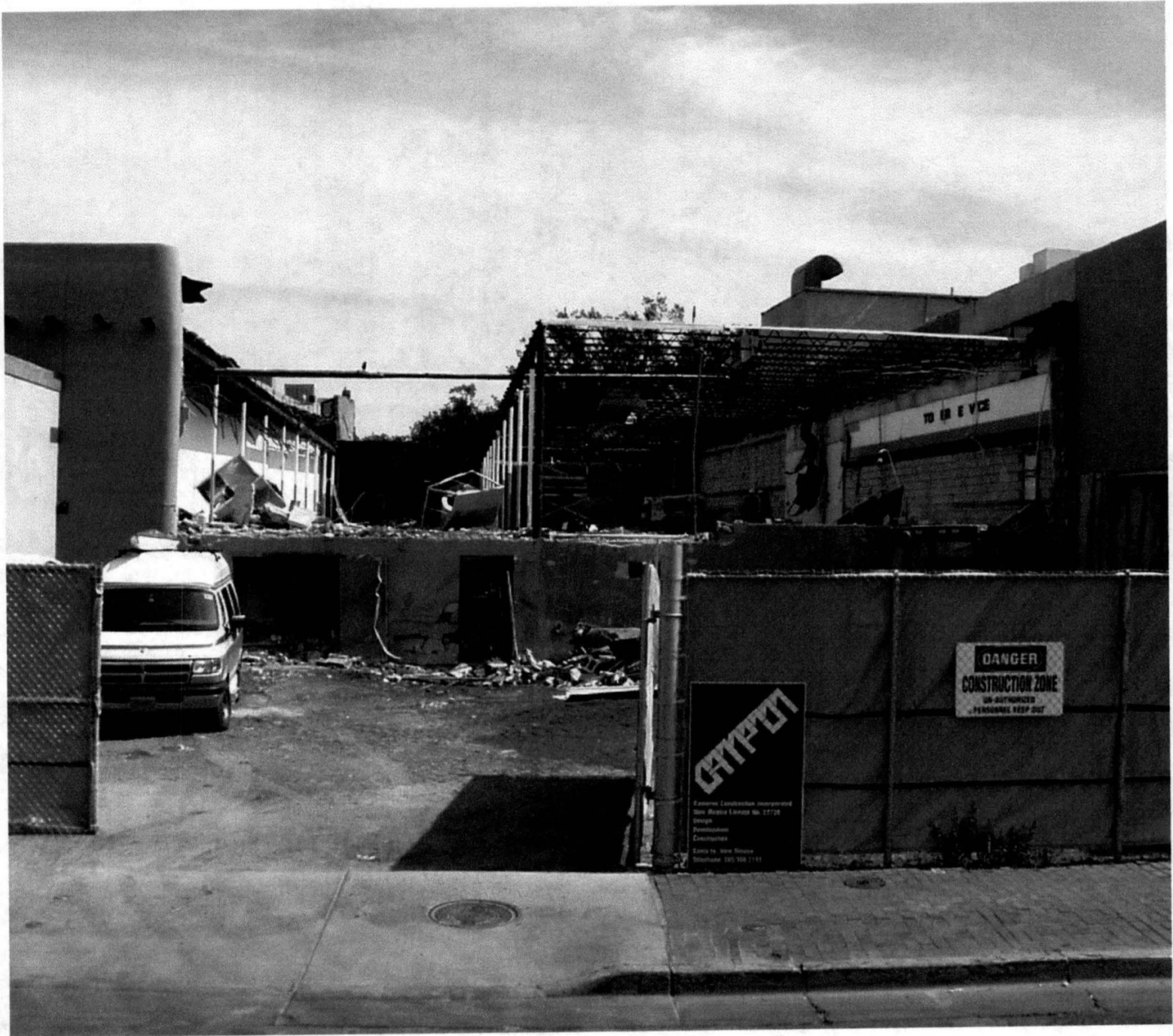
WATER STREET @ PROJECT SITE
