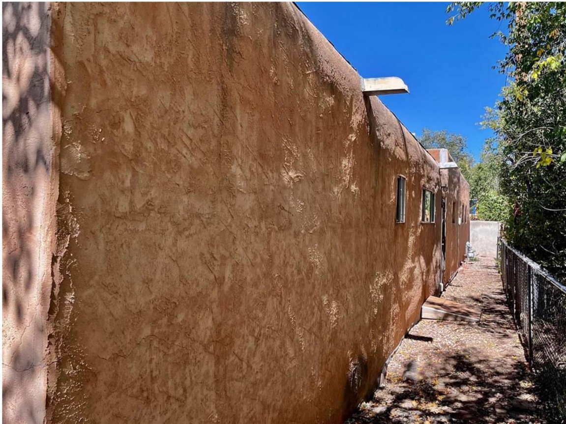
Photo 13: East elevation. Camera facing northwest.
