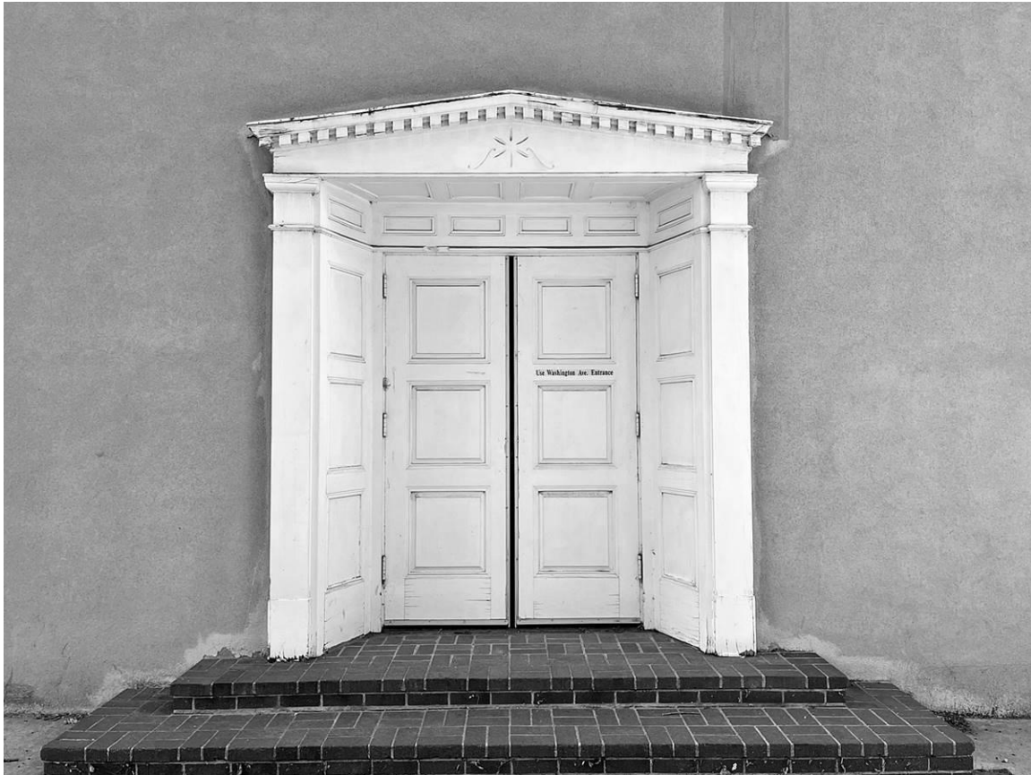
Photo 11: North elevation, former entrance to City Council Chamber. Camera facing south.
