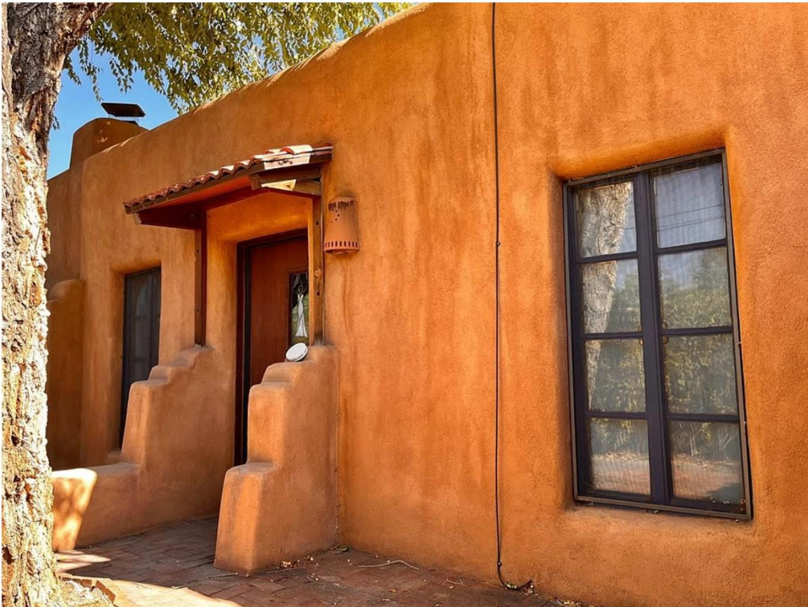
Photo 3: West elevation. Camera facing northeast.
