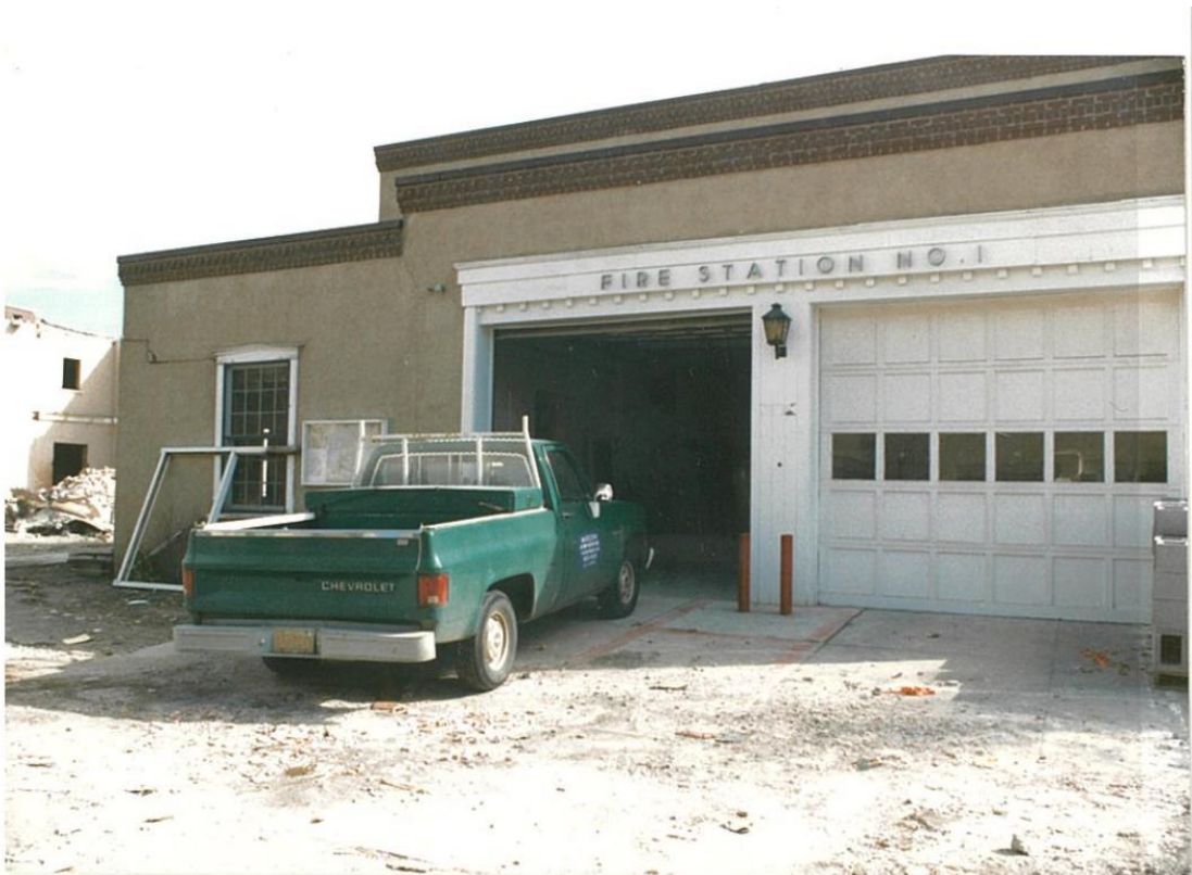
Figure 11: Extant fire station bays. Note on left, the building's center block has been mostly removed. Construction photographs, November 11, 1985. Courtesy City of Santa Fe.
