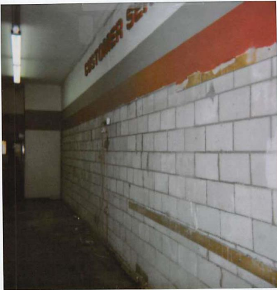
58 E. SAN FRANCISCO 10/26/00 1st Floor wall
