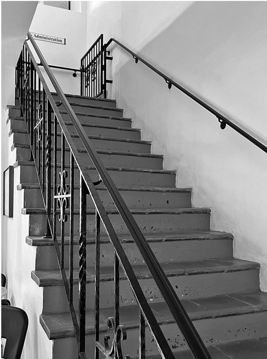
Photo 26: Original 1937 staircase. Camera facing up.
