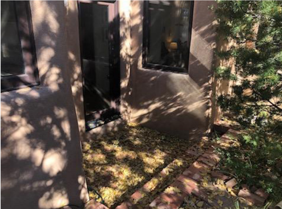
1047 A Camino San Acacio- South Elevation at 2018 Addition Entrance
