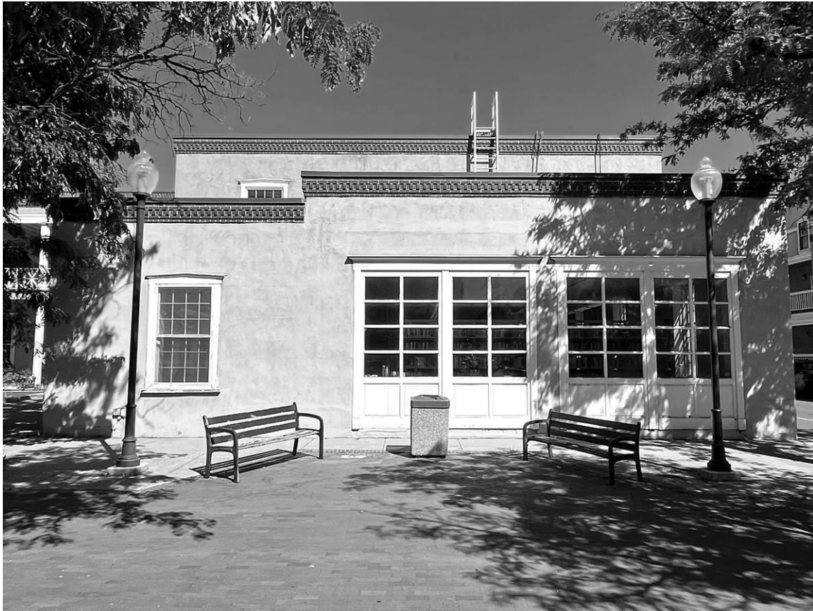
Photo 6: West (front) façade, south wing, former fire station bays. Camera facing east.
