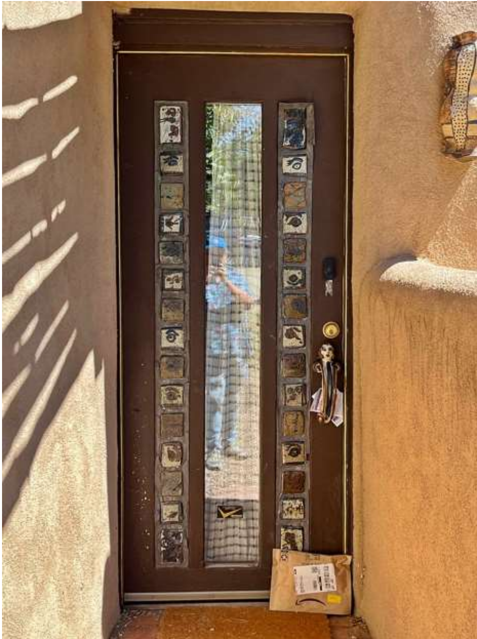
Photo 3: Front entry. Camera facing northeast.
