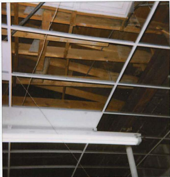
58 E. SAN FRANCISCO 10/26/00 1ST Floor Ceiling assy WOOD FRAME
