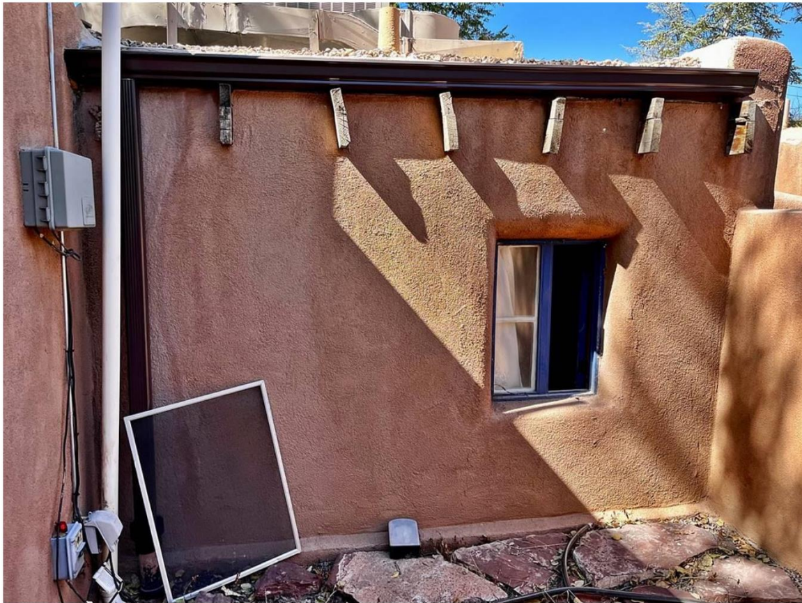
Photo 13: East elevation. Bathroom. Camera facing northwest.
