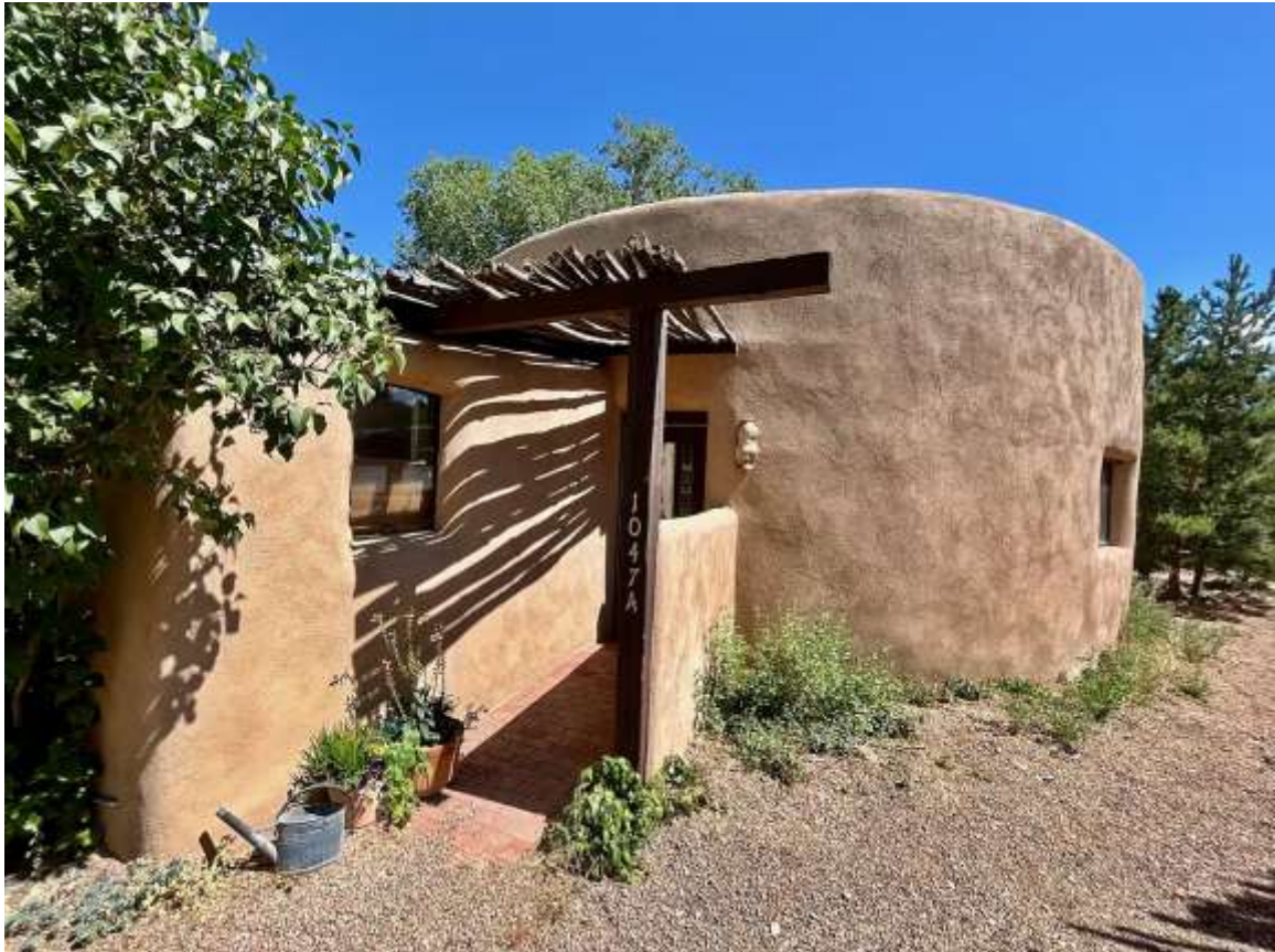
Photo 4: Front entry. Camera facing northeast.
