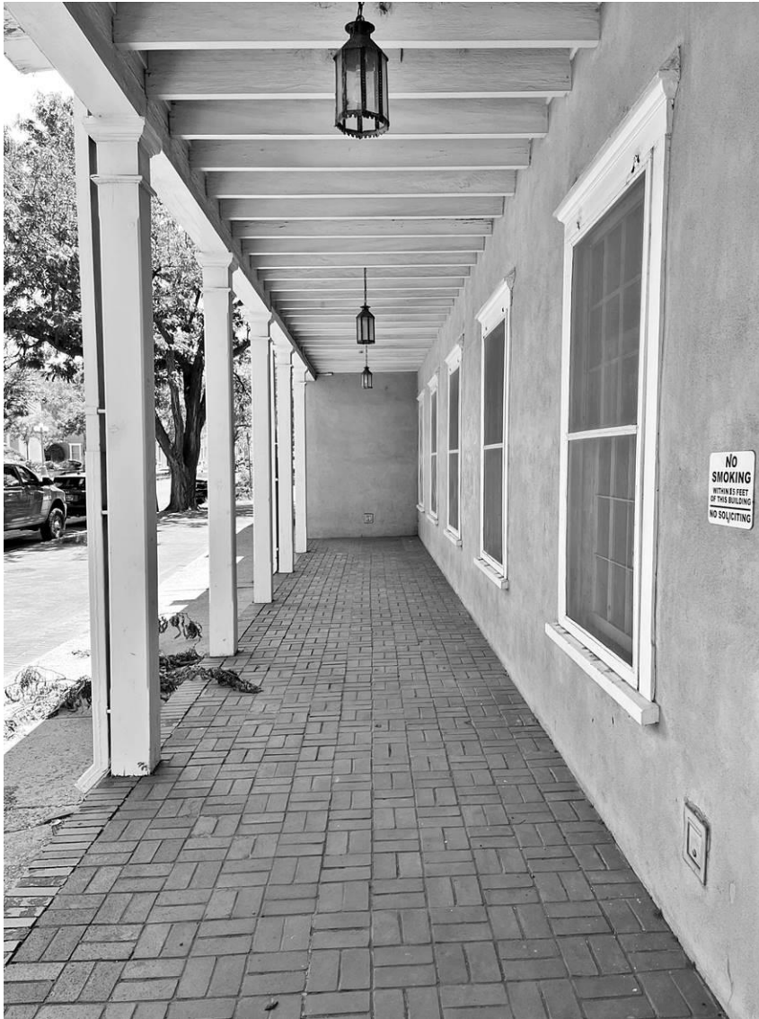
Photo 8: North elevation, portico. Camera facing east.
