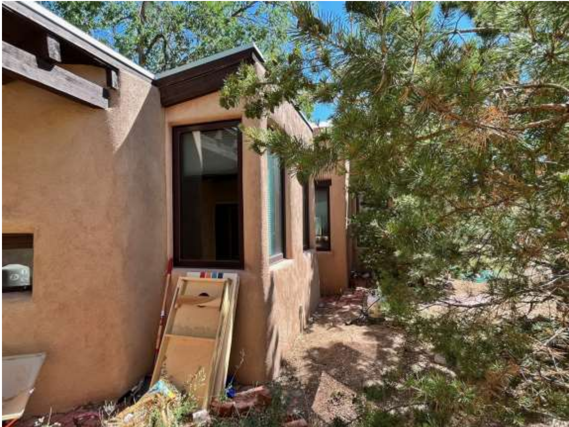
Photo 12: Guesthouse, former sleeping area. Camera facing northeast.
