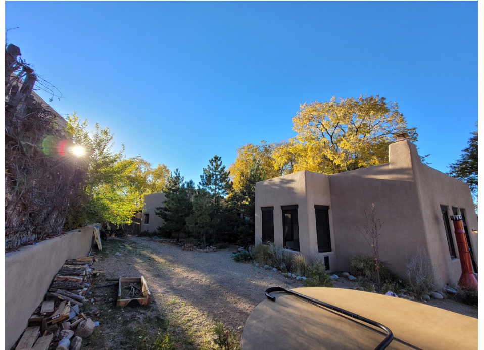
1047 A Camino San Acacio- South East Corner
