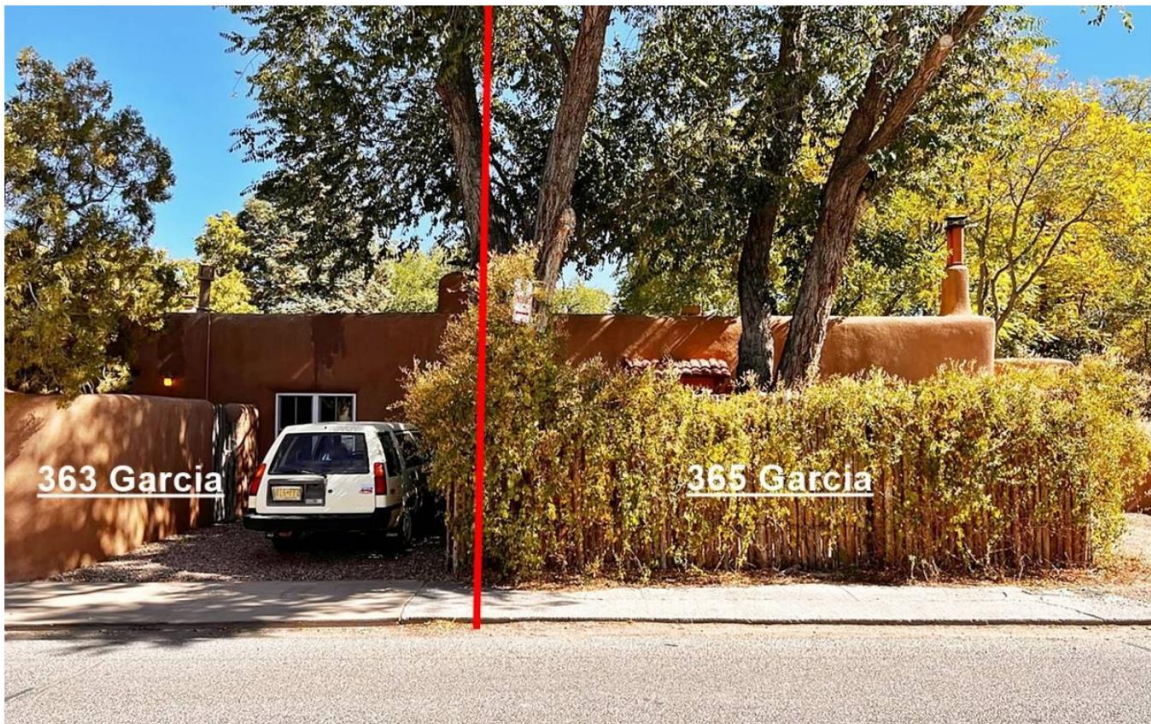
Photo 2: 363 and 365 Garcia Street. Street view. Camera facing east.
