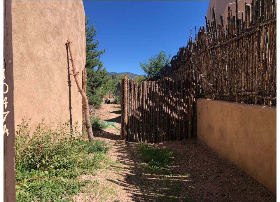
1047 A Camino San Acacio- Looking East at Yard Gate
