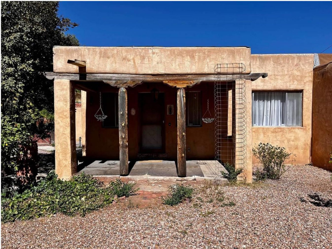
Photo 4: South elevation entry portal. Camera facing north.
