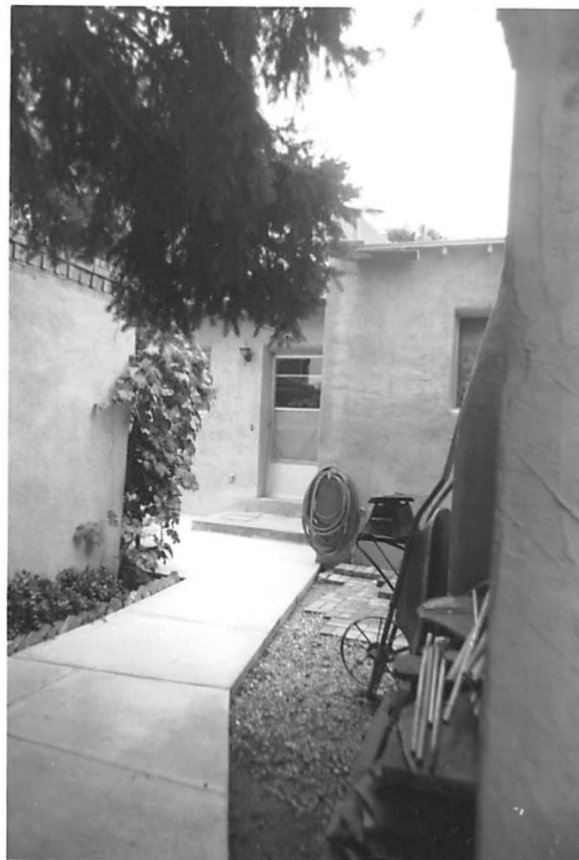
#15 west facade of north wing
