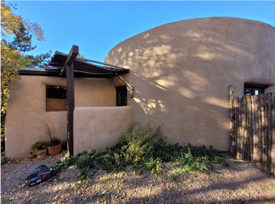
1047 A Camino San Acacio- South Elevation from South West Corner
