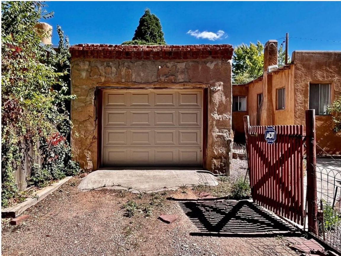
Photo 19: Garage. West elevation. Camera facing east.
