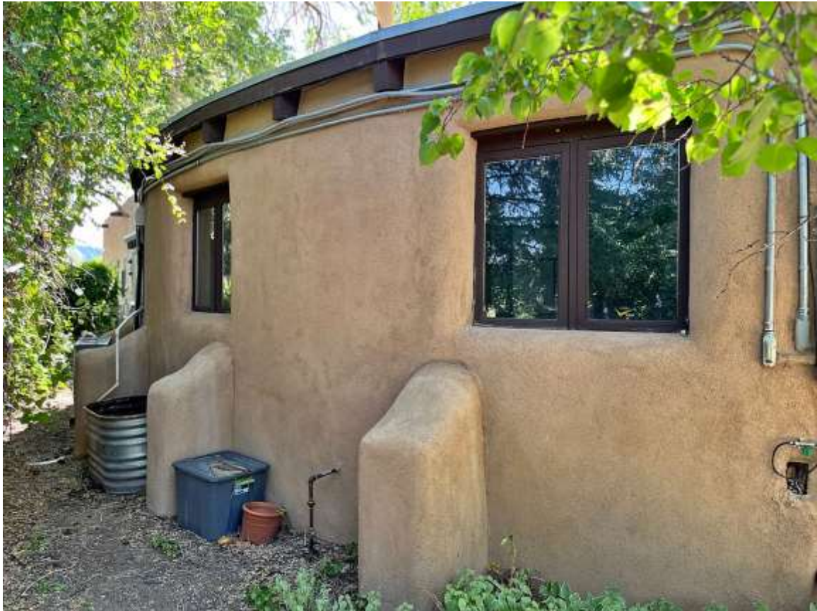
Photo 7: Former studio area. Camera facing east.
