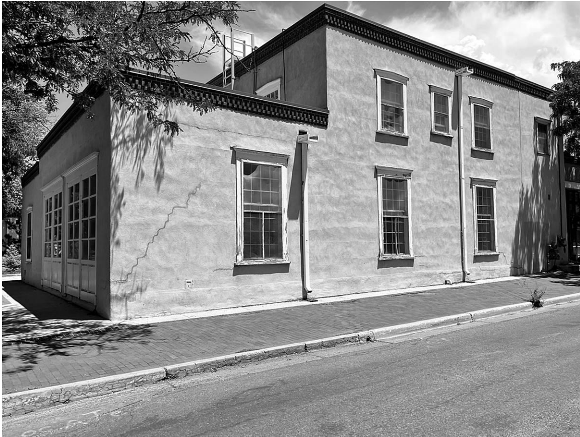
Photo 20: East elevation, southwest corner, representing original construction. Camera facing northeast.
