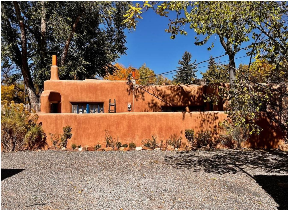
Photo 15: South property/yard wall. Camera facing north.
