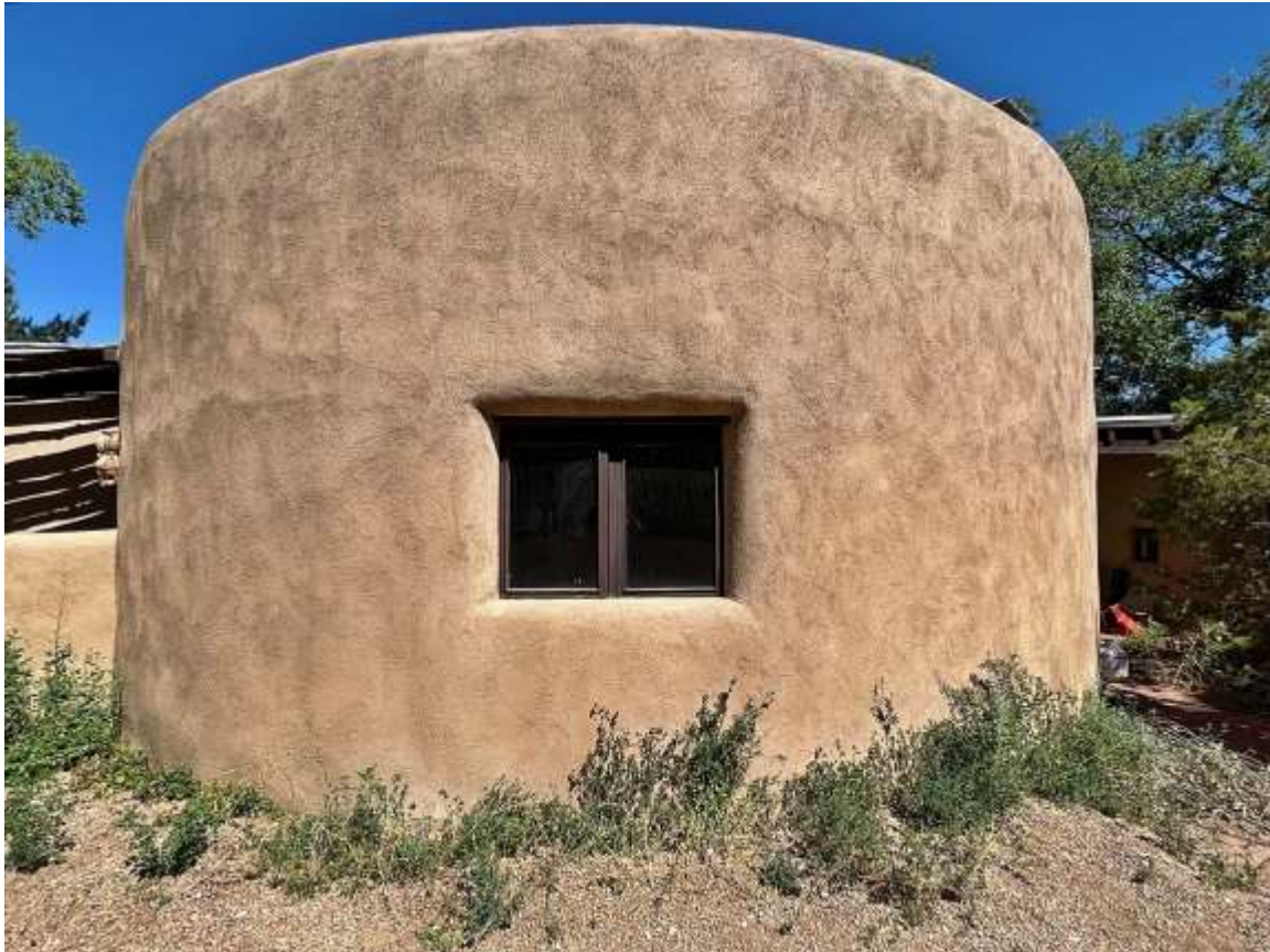
Photo 9: South side. Camera facing north.
