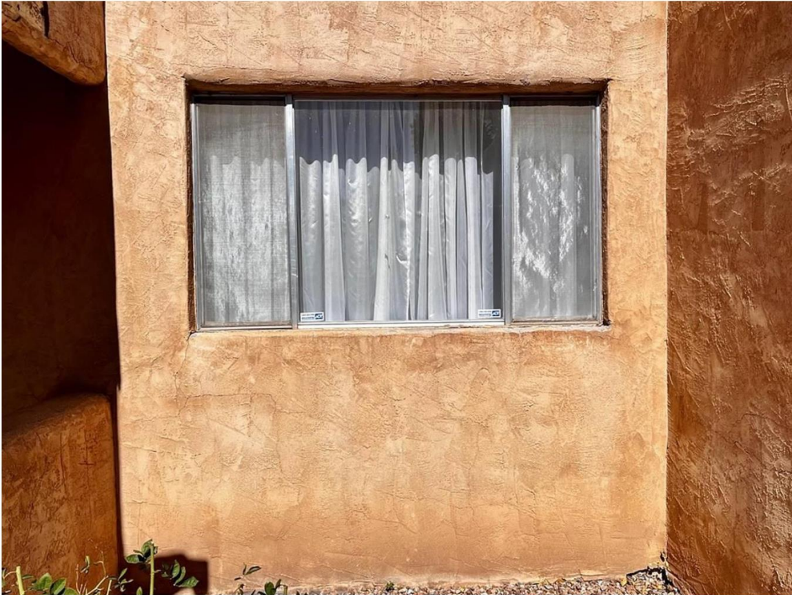
Photo 11: Older House. South elevation living room window. Camera facing north.
