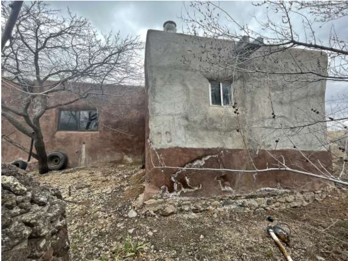
Photo 5: East elevation, bathroom bump-out at right. Camera facing southwest.
