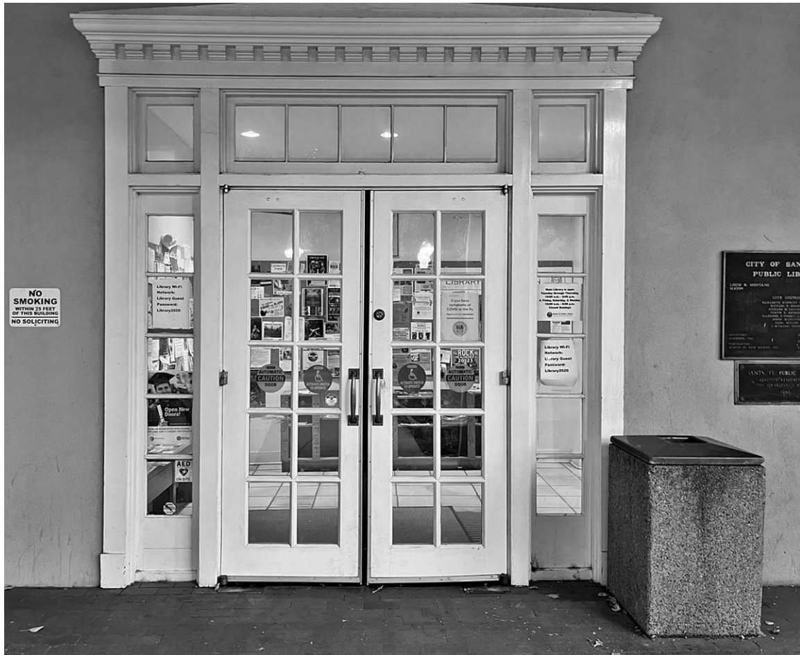
Photo 4: West (front) façade, north entry. Camera facing east.
