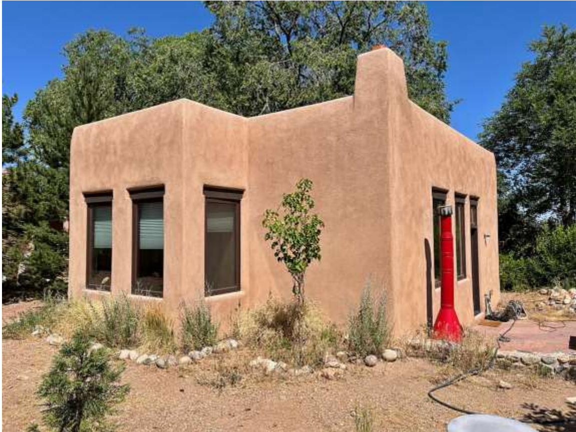
Photo 14: Addition, south and east elevations. Camera facing northwest.
