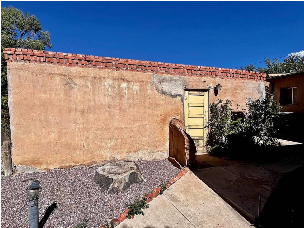
Photo 20: Garage. South elevation. Camera facing northeast.
