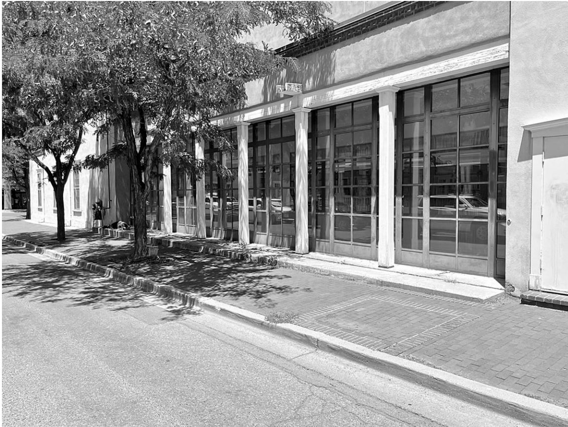
Photo 19. South elevation. Area at center is 1980s construction. Camera facing northwest.
