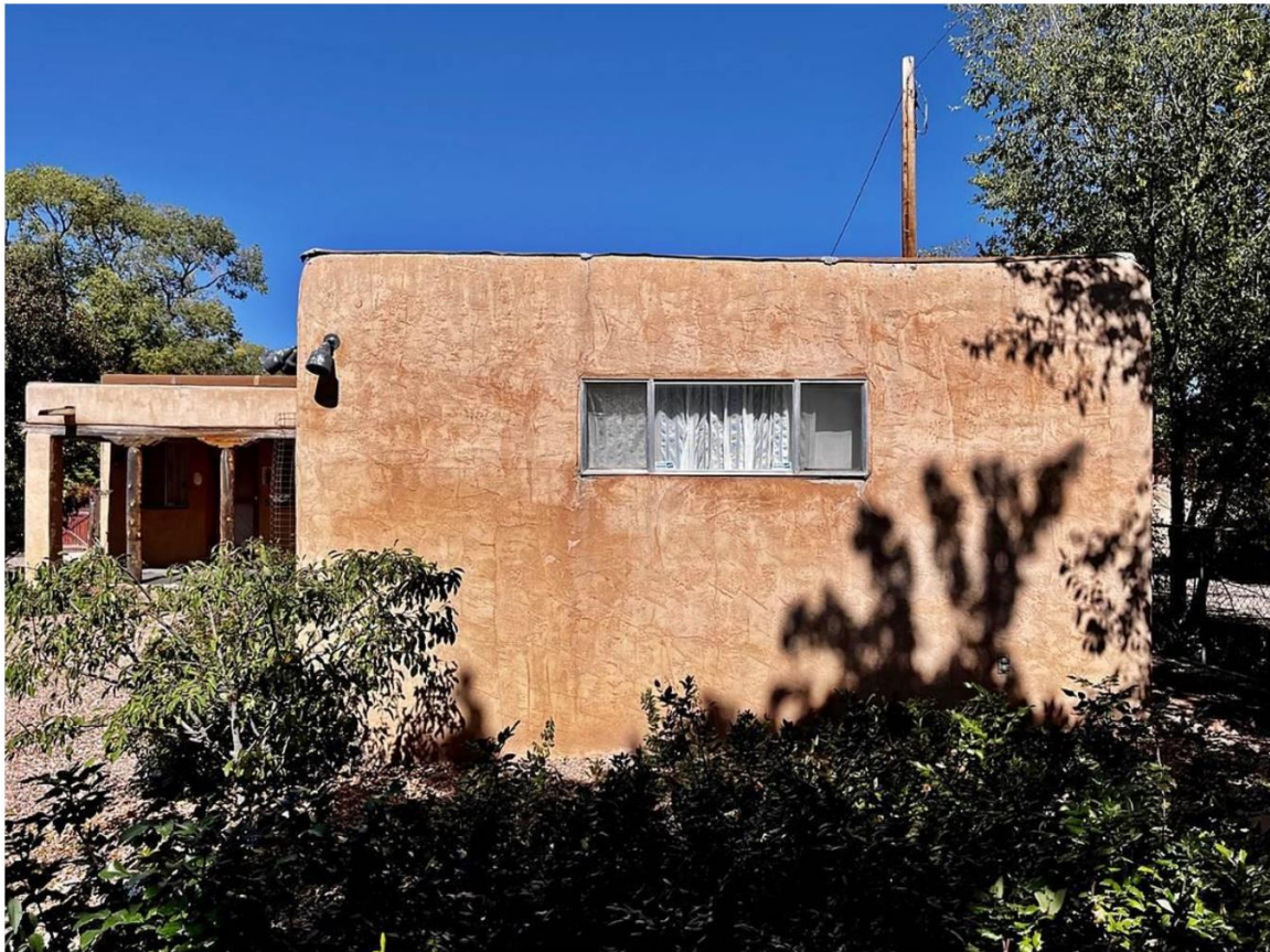
Photo 12: Bedroom Wing Addition. South elevation. Camera facing north.
