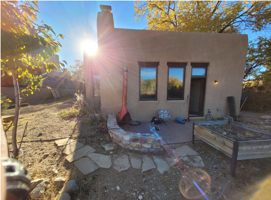
1047 A Camino San Acacio- East Elevation
