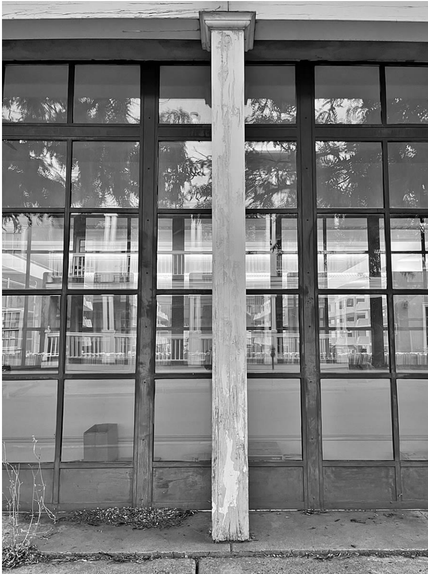
Photo 17: East elevation, window and wall post. Camera facing west.
