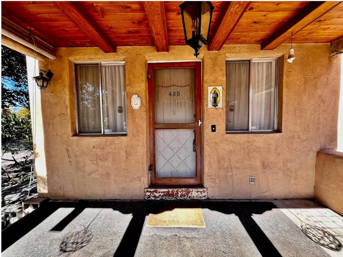
Photo 10: Older House. South elevation entry portal. Camera facing north.
