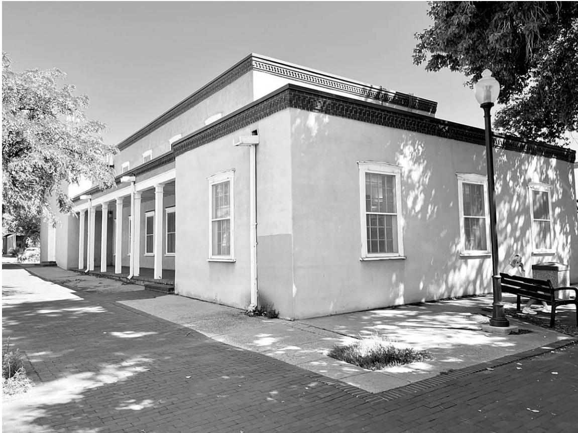
Photo 7: West (front) façade, north wing and north elevation. Camera facing northeast.
