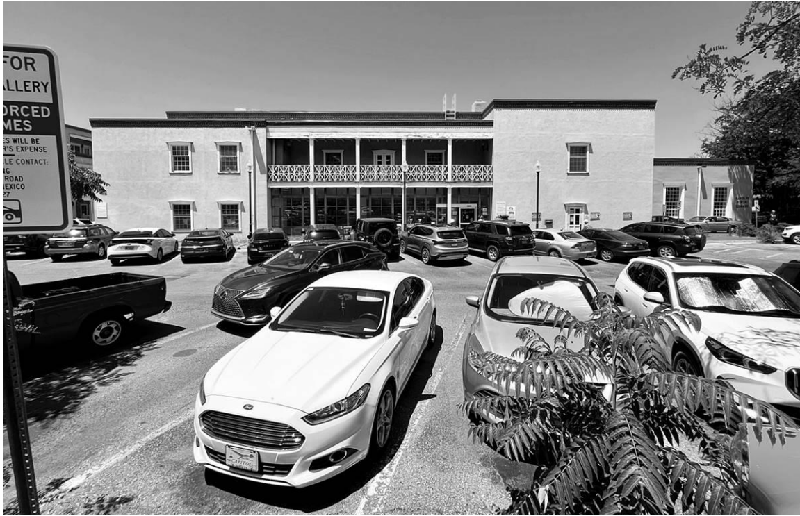
Photo 15: East elevation. Two-story center block represents 1980s construction. Camera facing west.
