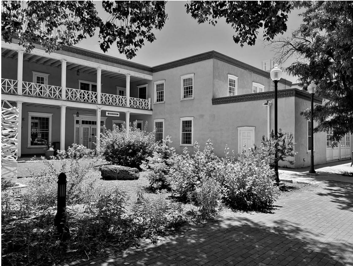
Photo 5: West (front) façade, south wing. Camera facing southeast.
