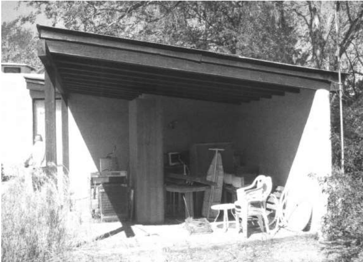
Figure 7: Carport demolished for addition. Courtesy Martinez Architecture Studio PC.
