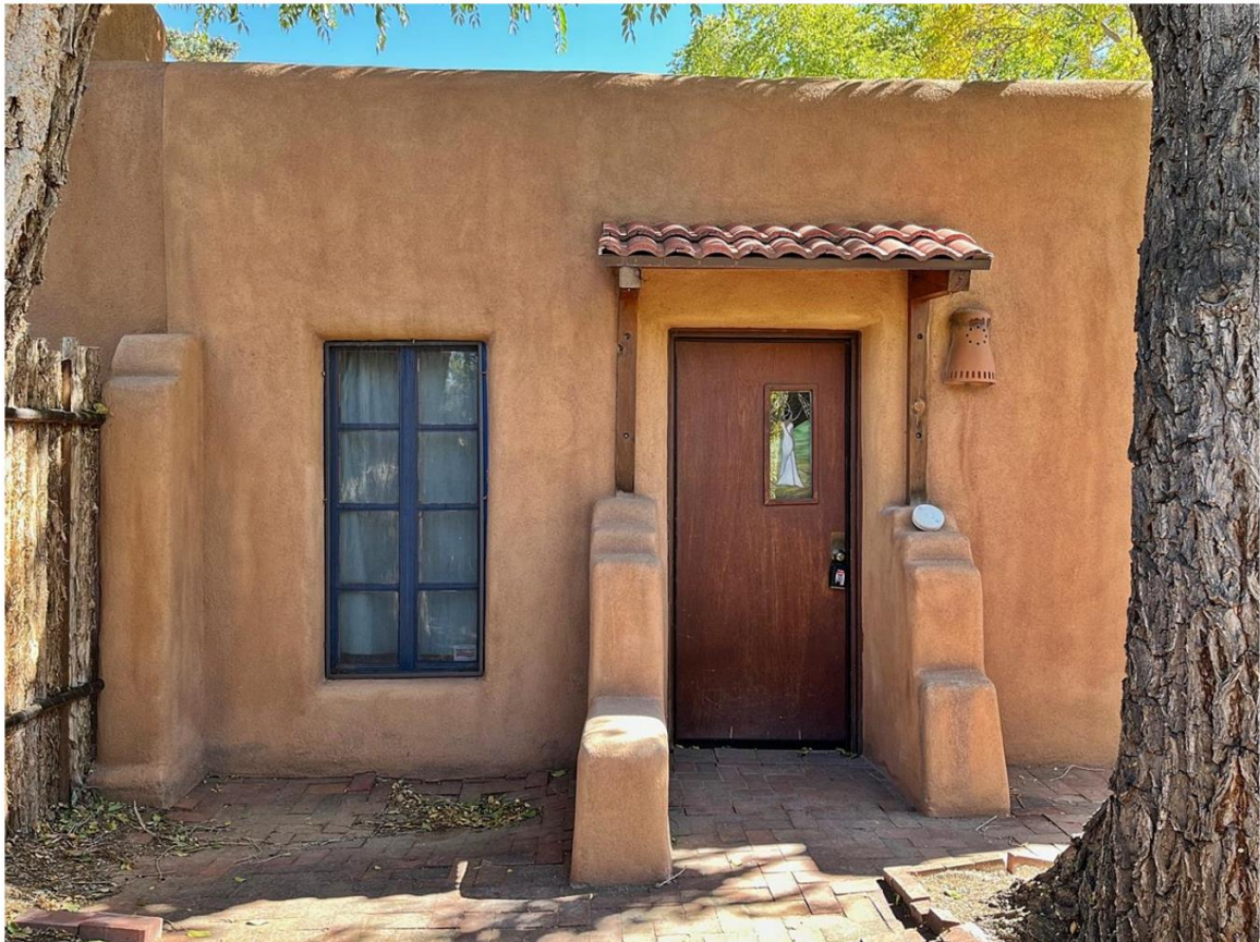
Photo 4: West elevation. North end where house shares a wall with 363 Garcia. Camera facing east.
