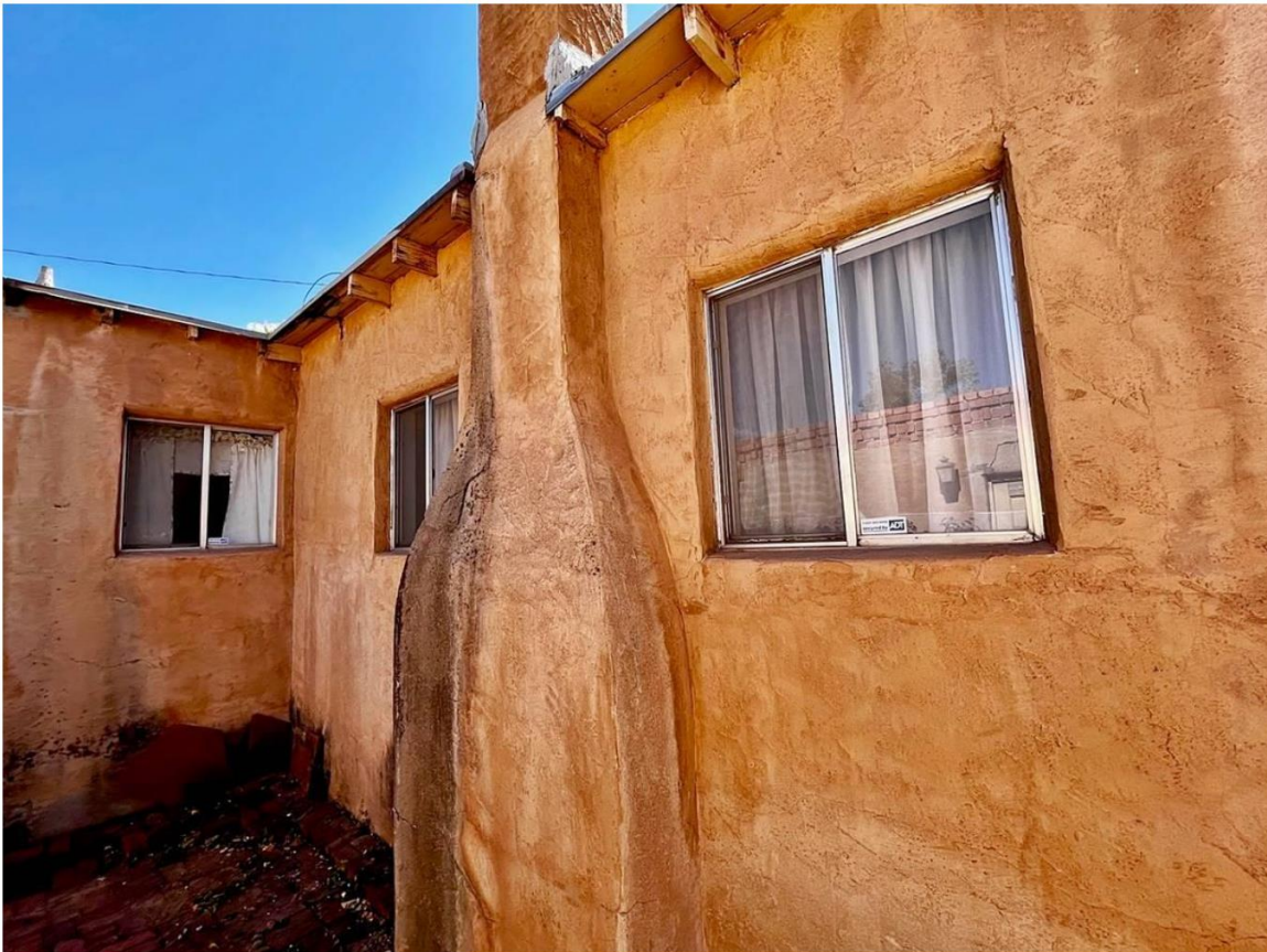
Photo 7: Older House. North elevation. Camera facing southeast.
