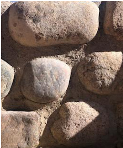
Site-Collected Rock for wall base and site retaining walls
