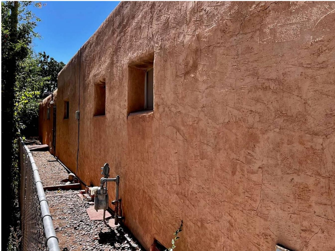
Photo 16: East elevation. Camera facing southwest.
