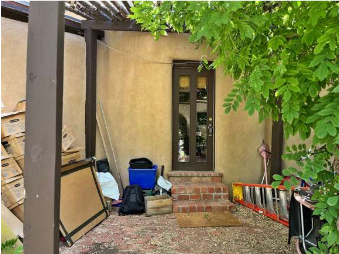
Photo 6: Back entrance. Camera facing southeast.
