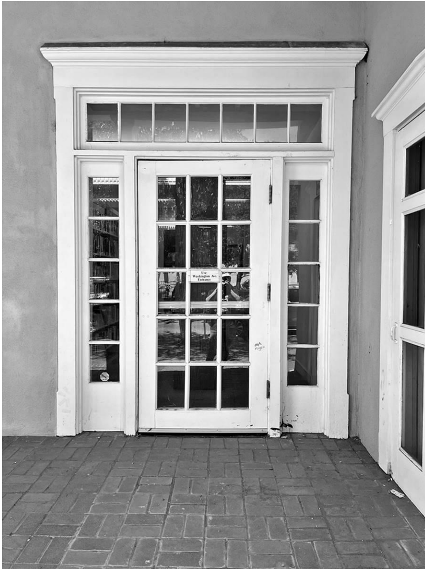
Photo 9: North elevation, entry. Camera facing south.
