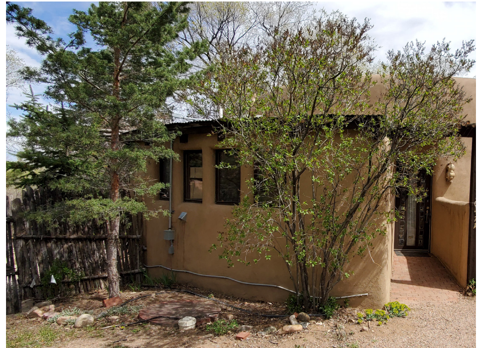
1047 A Camino San Acacio- West Elevation at Laundry/ 2nd Front Door
