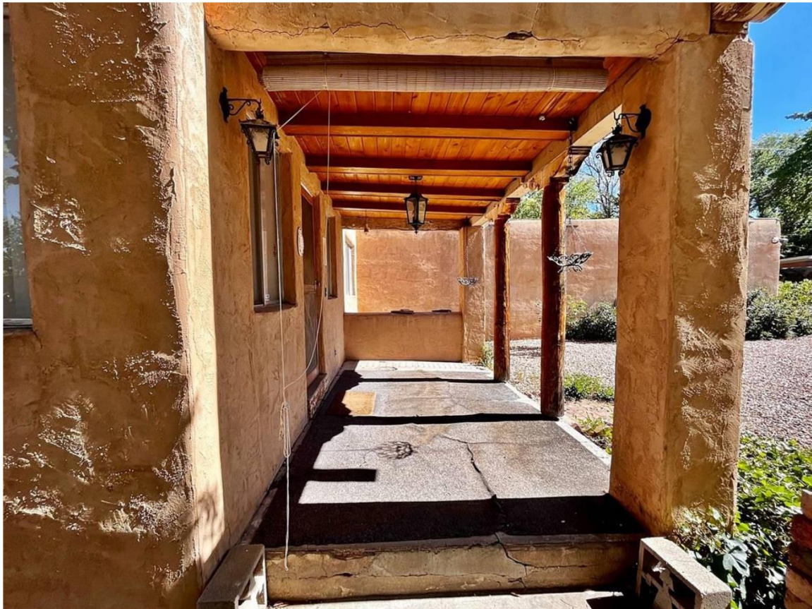
Photo 9: Older House. South elevation entry portal. Camera facing east.
