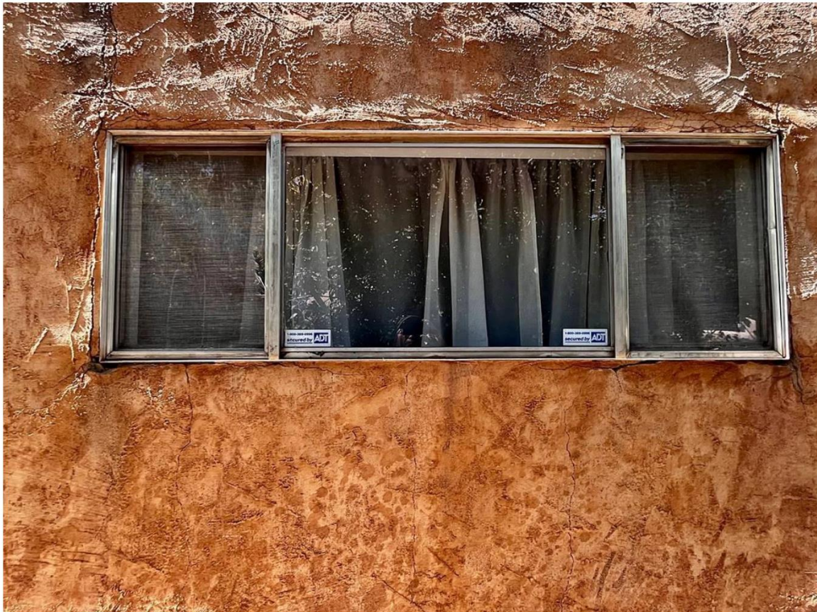
Photo 14: East elevation at Bedroom Wing Addition. Camera facing west.
