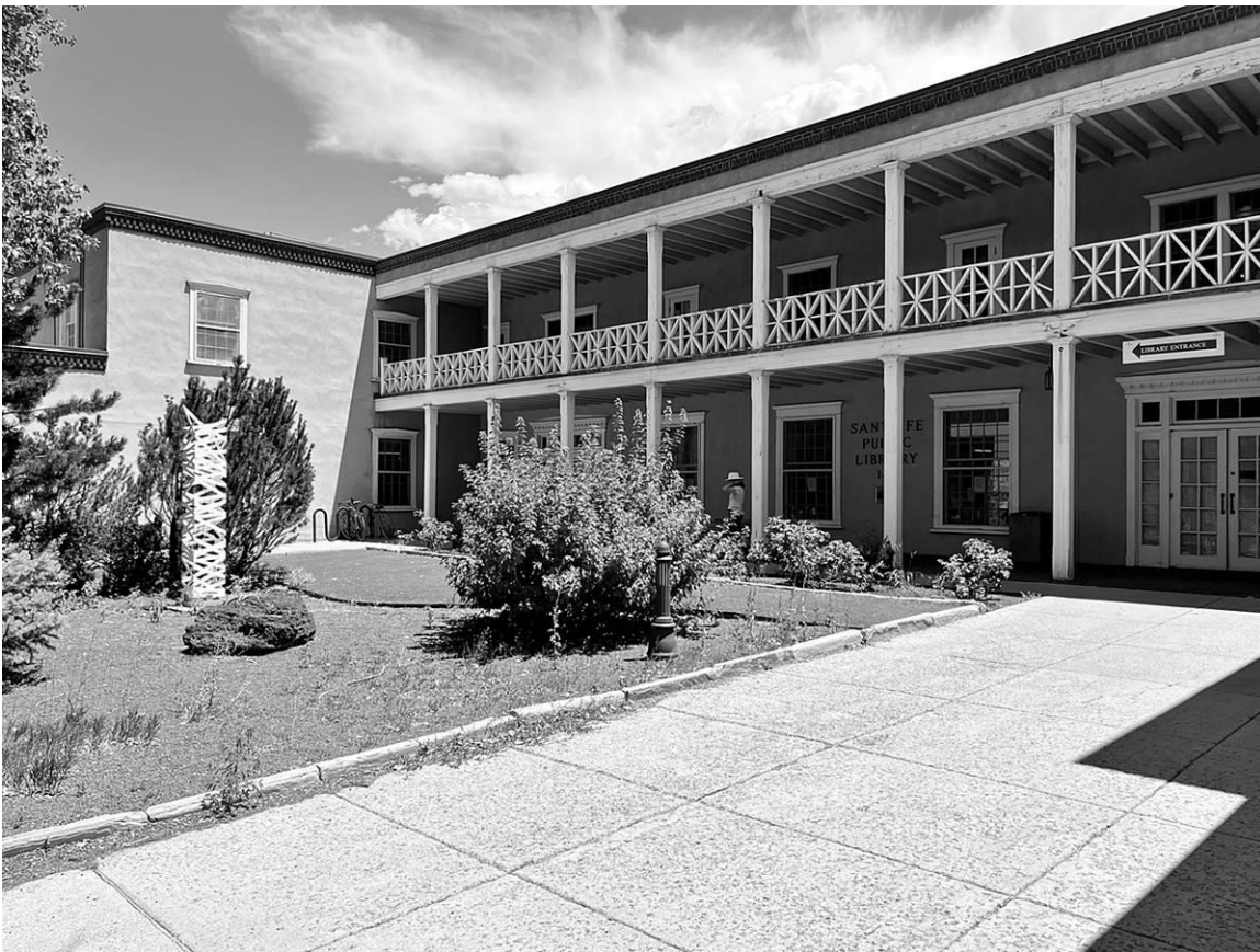
Photo 2: West (front) façade. Camera facing northeast.
