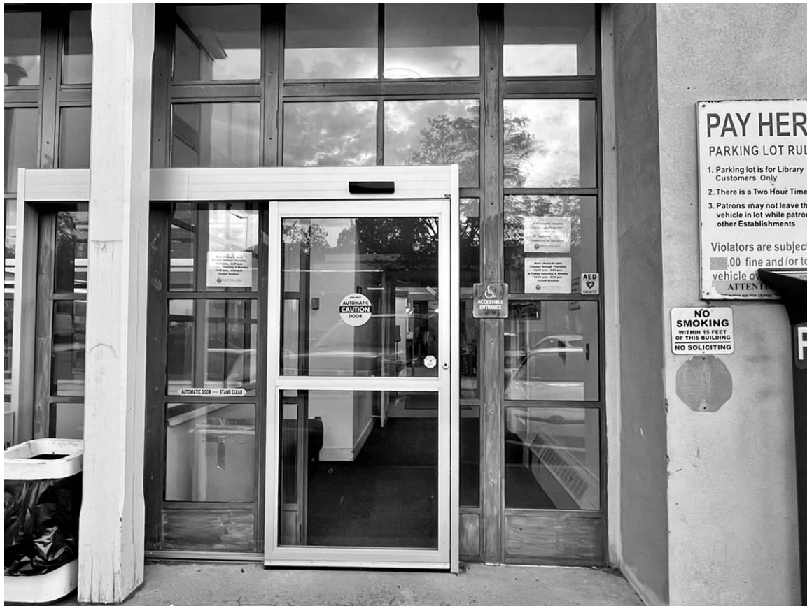
Photo 16: East elevation window wall and entry. Camera facing west.
