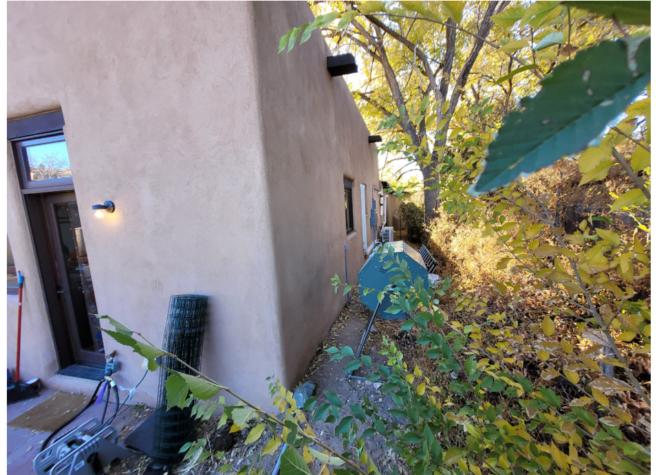
1047 A Camino San Acacio- North East Corner
