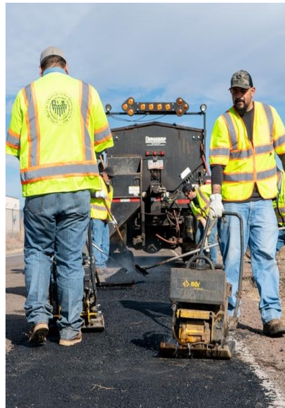
Streets and Drainage Maintenance
