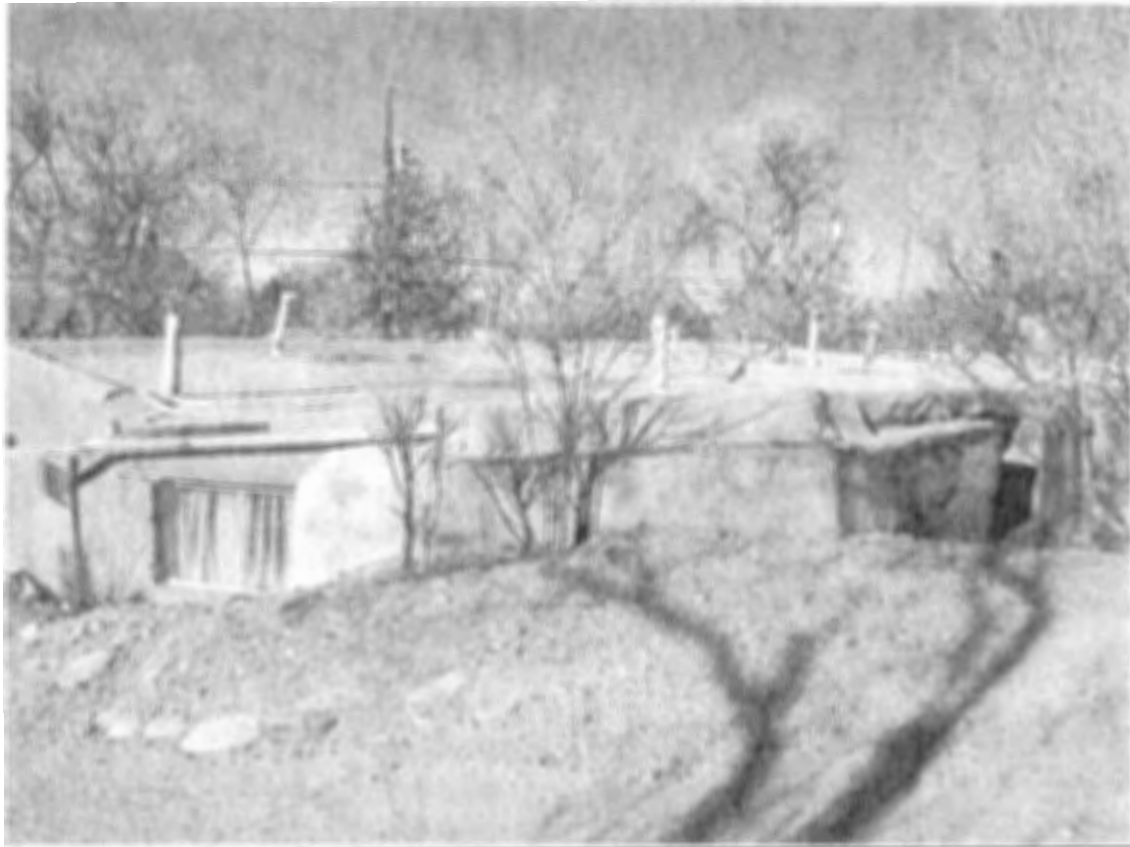
Photo 8: East end of north elevation, facing southeast.
