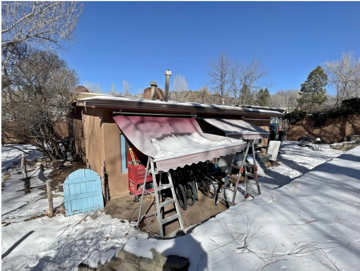
Photo 7: South elevation. Camera facing northeast.
