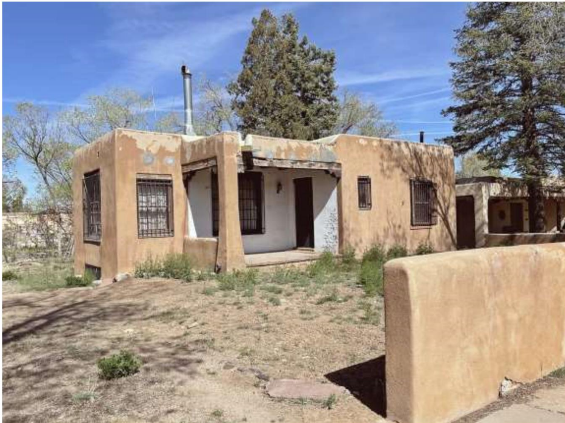
Photo 2: East elevation. Camera facing northwest.
