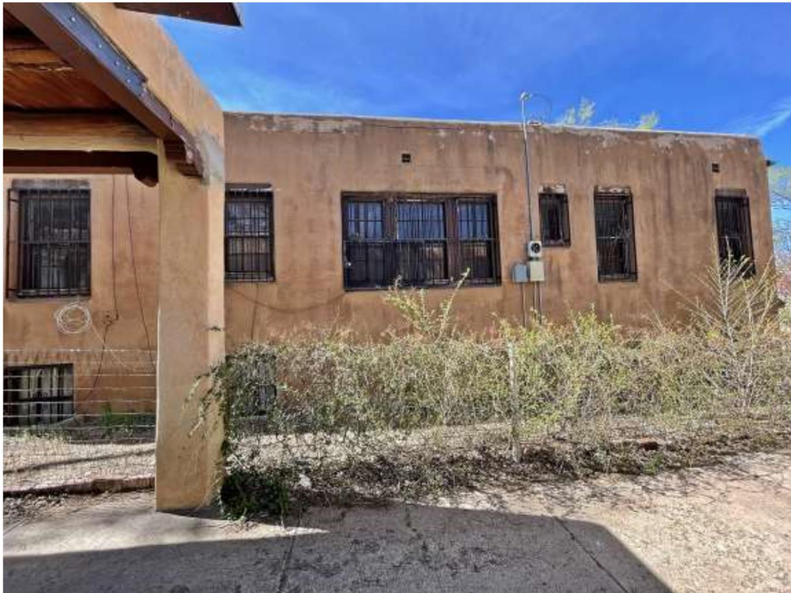
Photo 9: North elevation as viewed neighboring property. Camera facing south.
