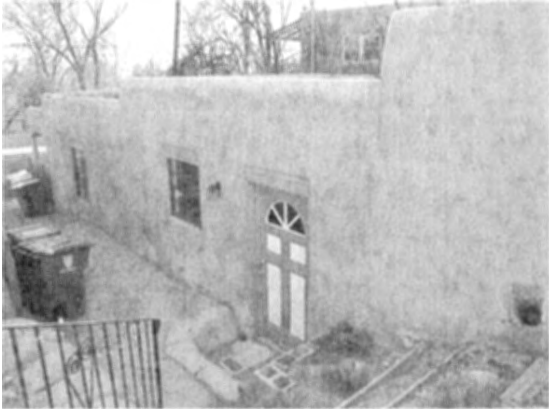
Photo 4: East elevation, facing southwest.
