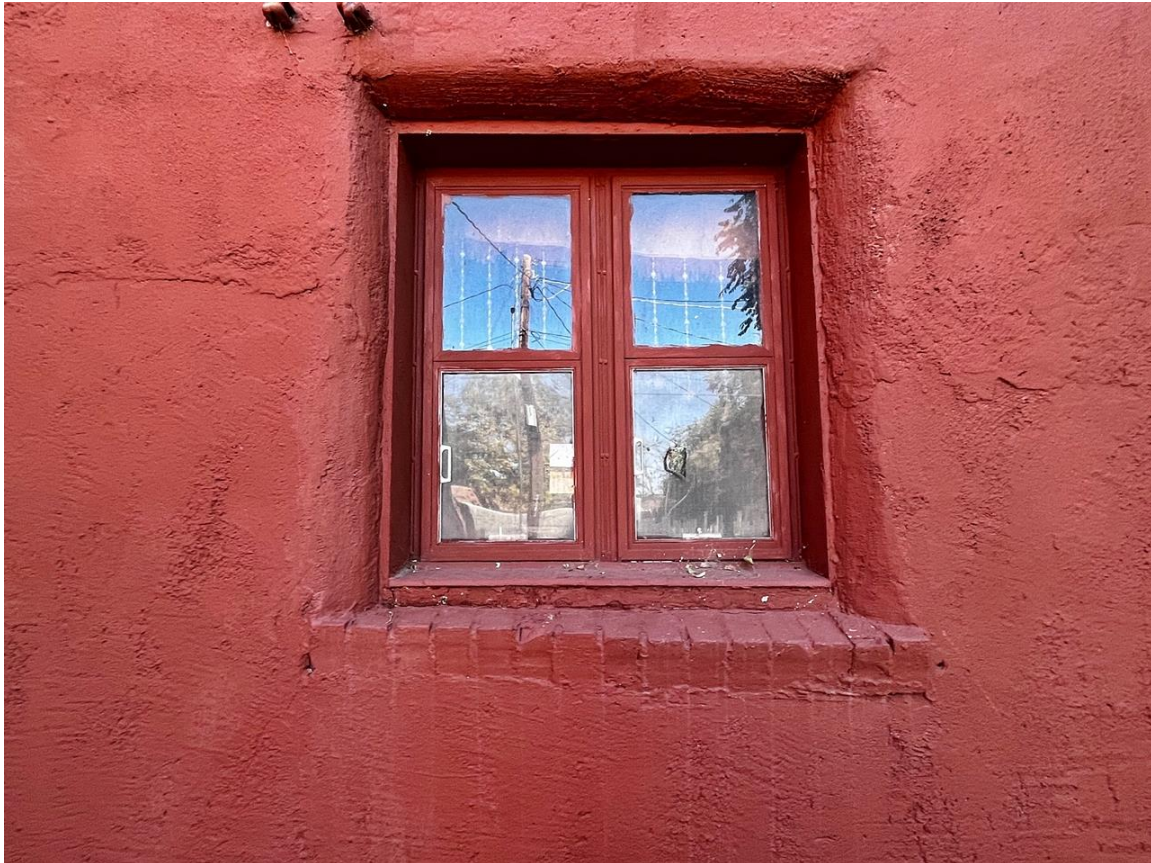
Photo 5: North elevation of foot of L. Camera facing south.
