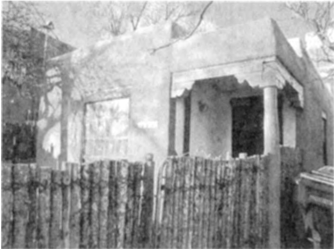
Photo 2: South (front) elevation, facing northwest.
