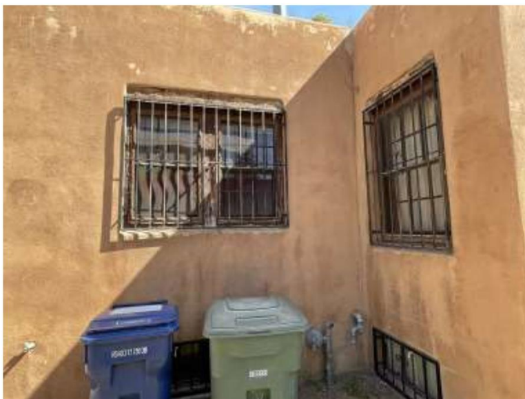
Photo 4: Windows. Top, window at portal; bottom, grouped windows at living room and kitchen.
