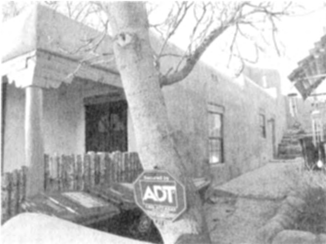
Photo 3: East elevation, facing northwest.
