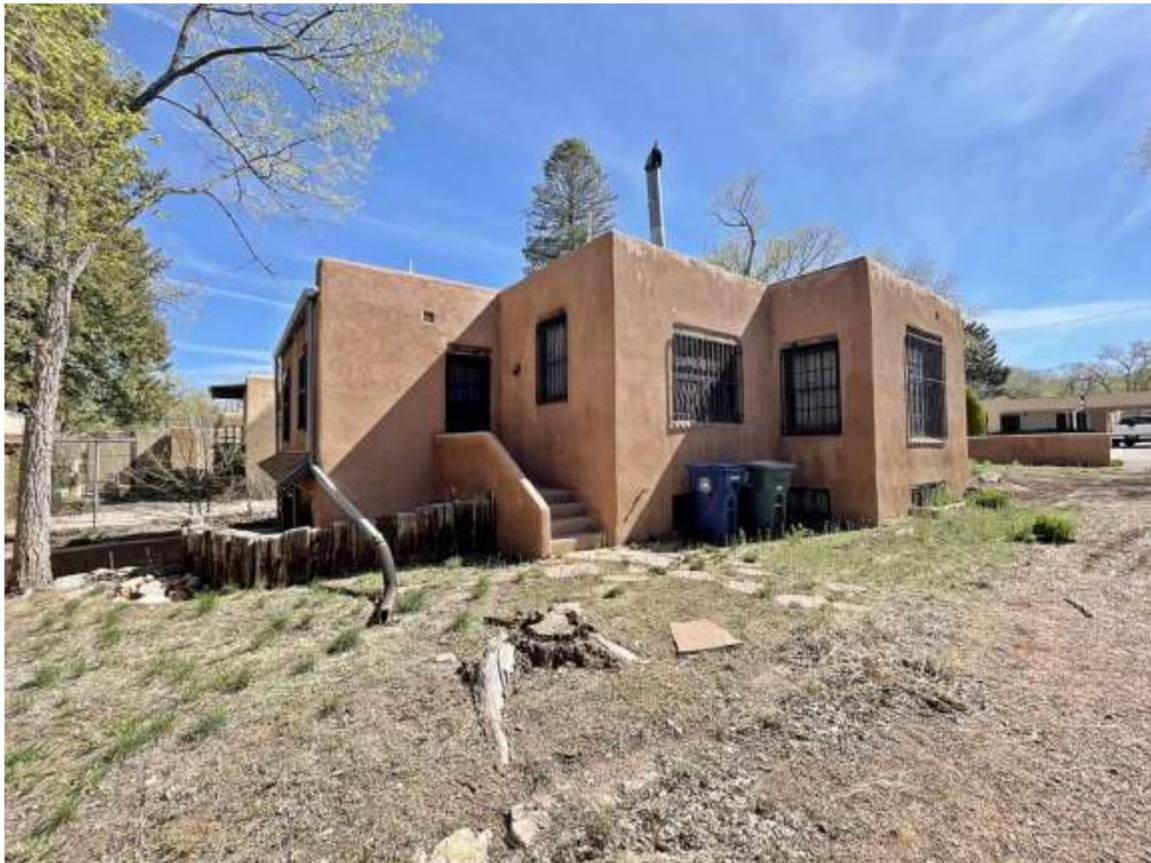
Photo 6: South elevation. Camera facing northeast.
