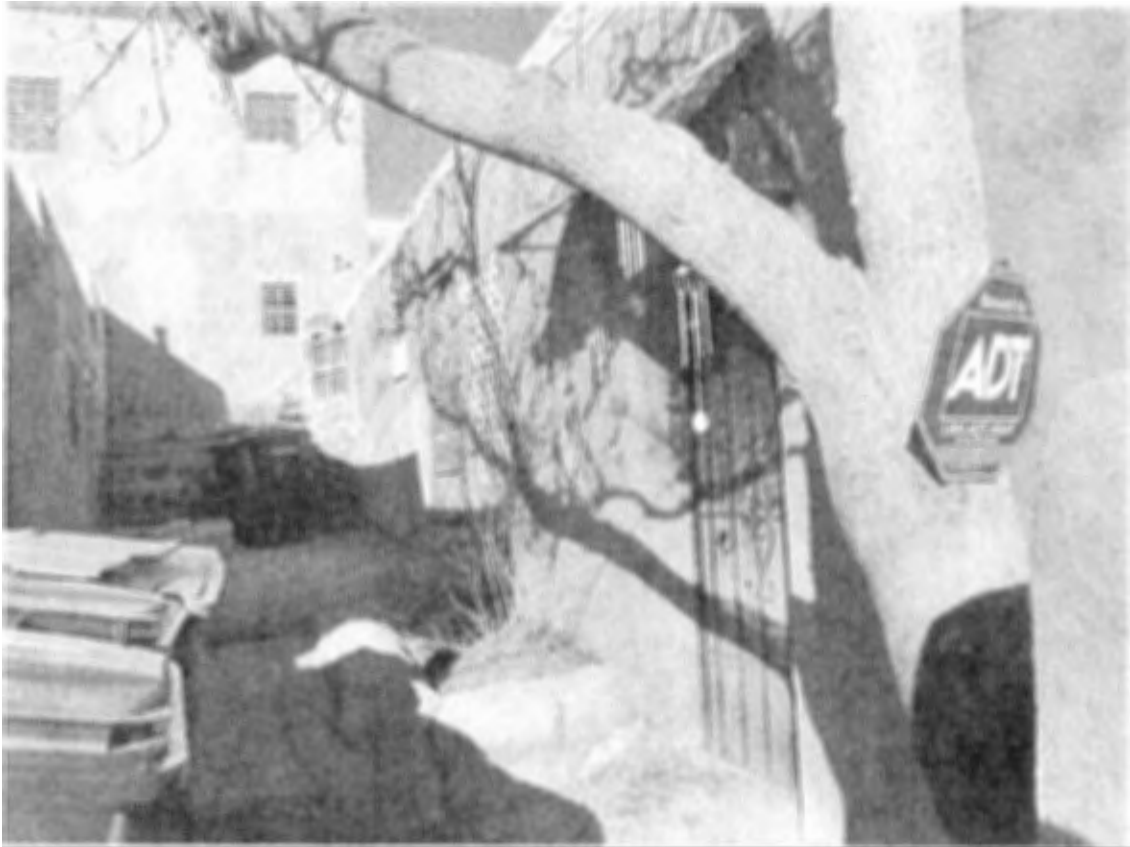
Photo 3: west elevation, facing north.
