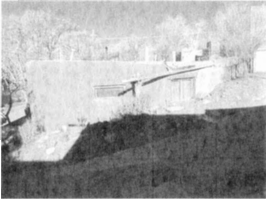
Photo 2: East elevation, facing northwest.
