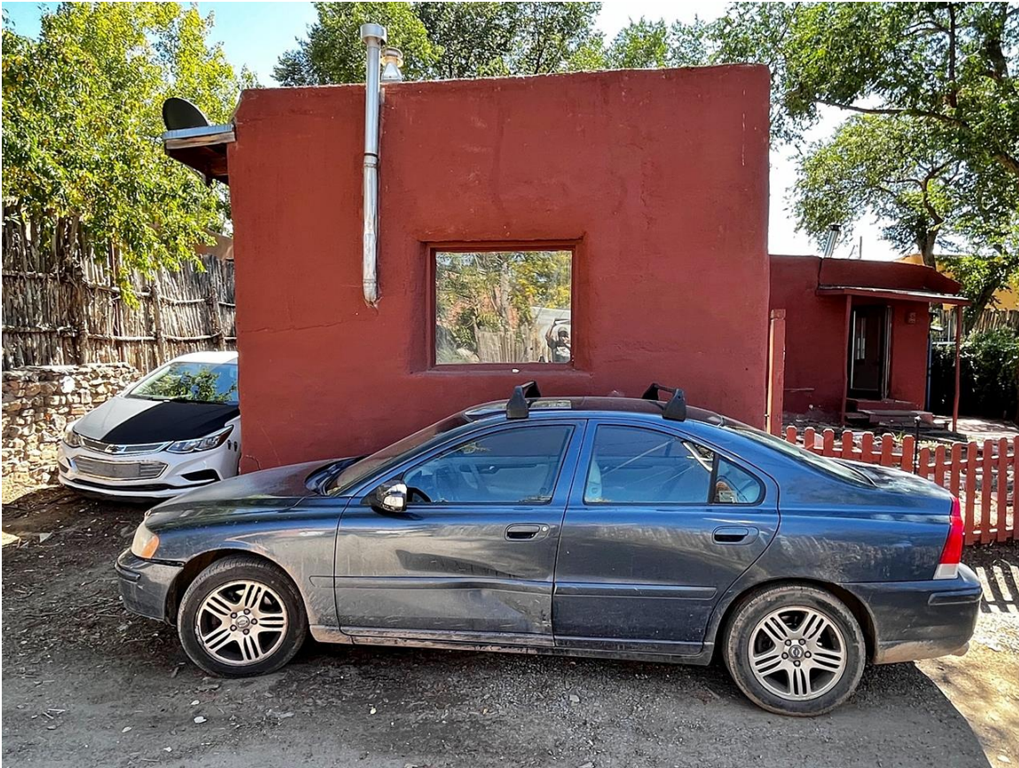
Photo 2: North elevation, older portion of building. Camera facing south.
