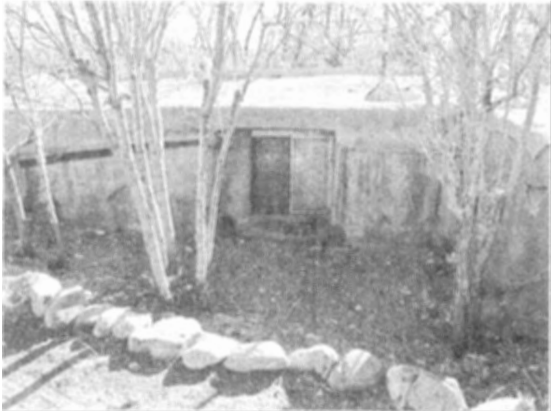
Photo 7: Middle section of north elevation, facing south.
