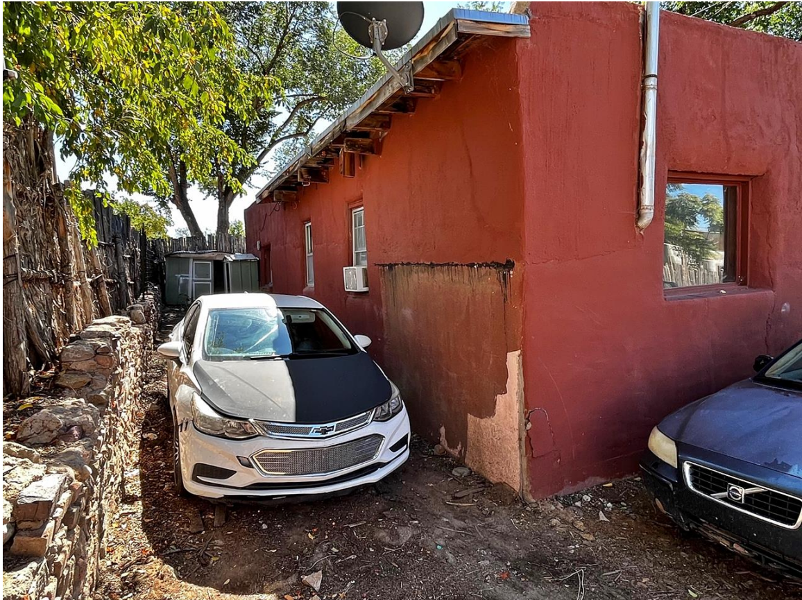
Photo 14: East elevation. Camera facing southwest.
