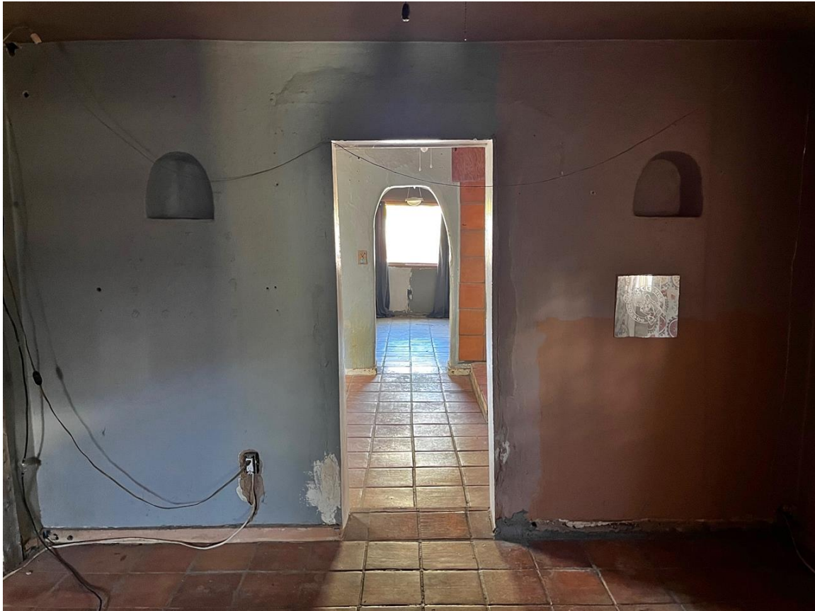
Photo 18: South room. Camera facing north.
