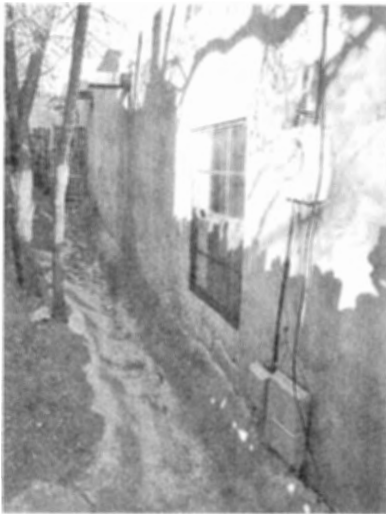
Photo 5: West elevation, facing north.
