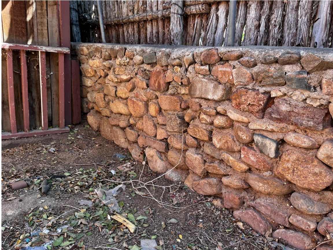
Photo 23: South property wall. Camera facing southeast.
