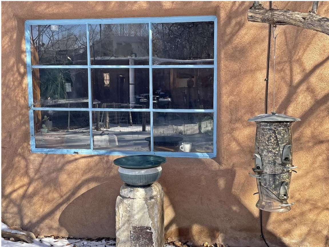
Photo 6: West elevation. Example of nine-light window. Camera facing northeast.
