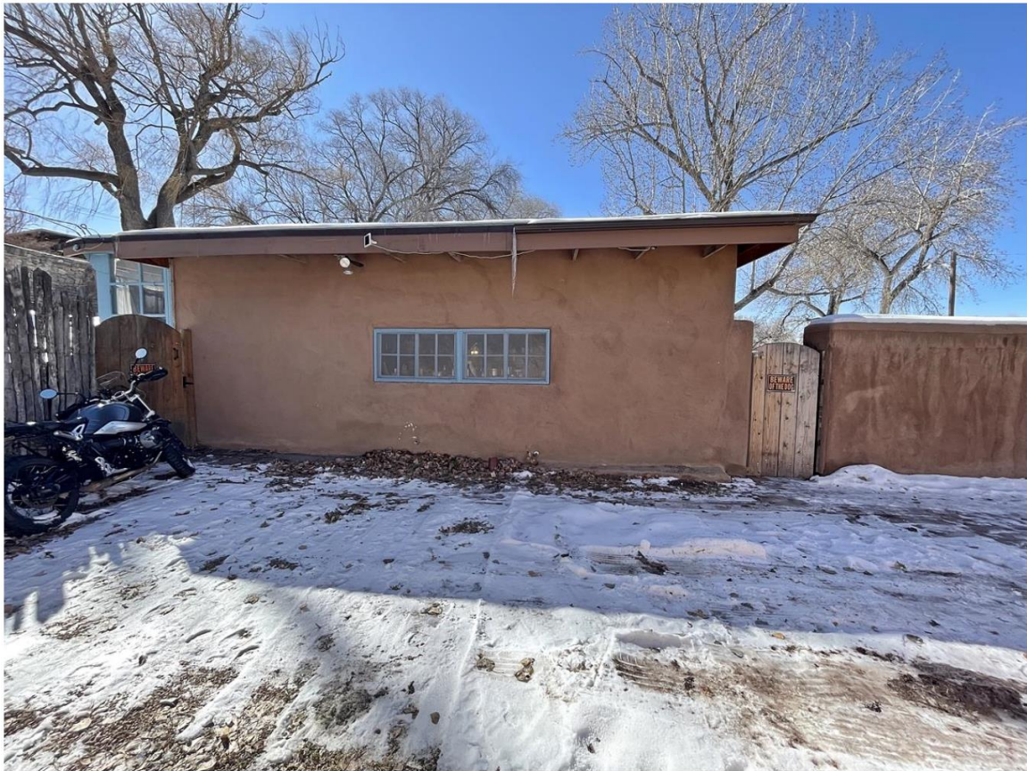
Photo 11: East elevation. Camera facing southwest.
