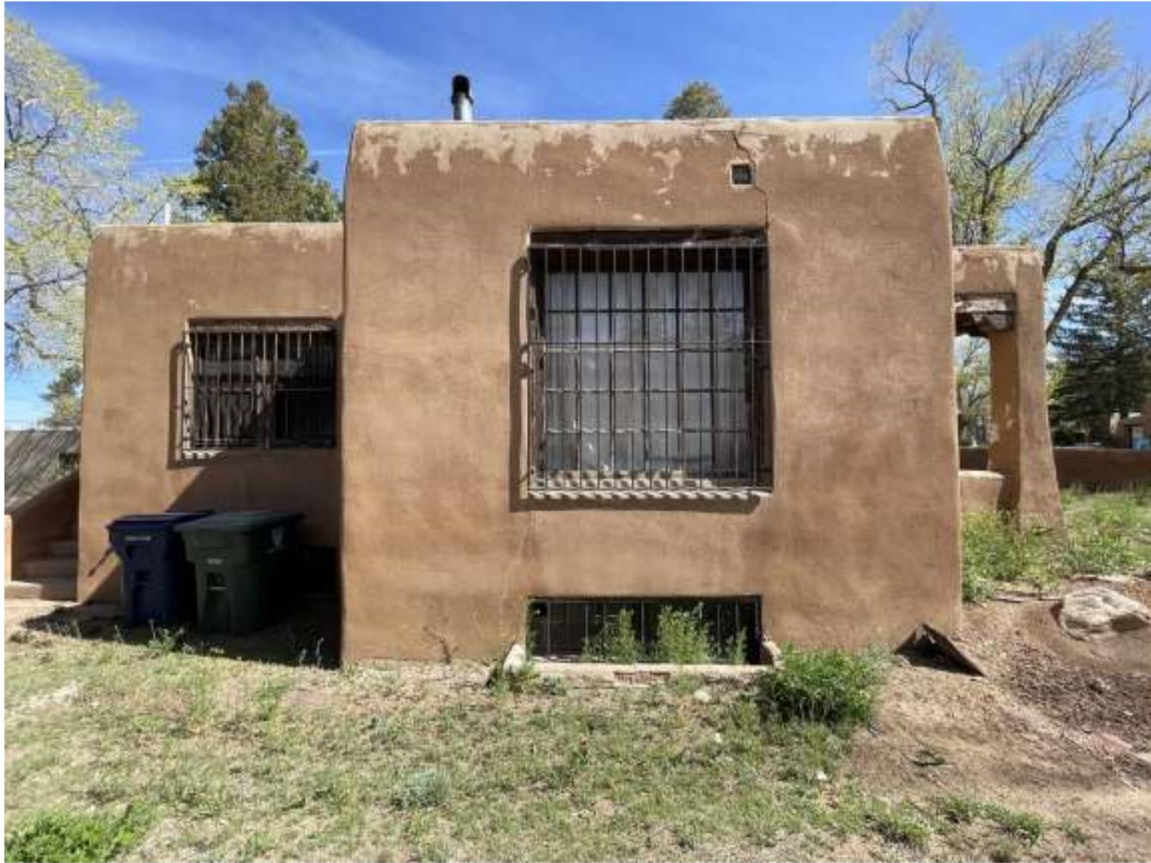
Photo 5: South elevation. Living room (right), kitchen (left). Camera facing north.
