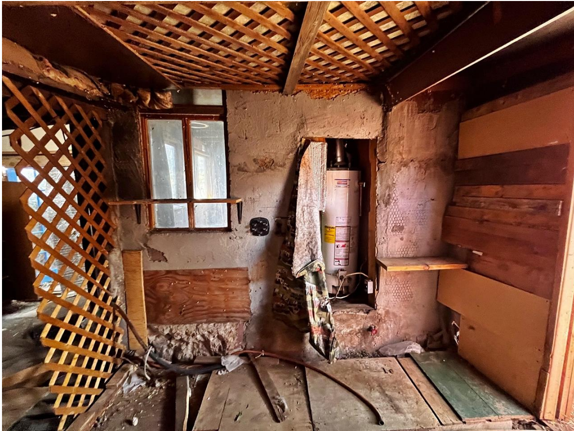
Photo 9: South elevation of post-1978 addition. Camera facing north.
