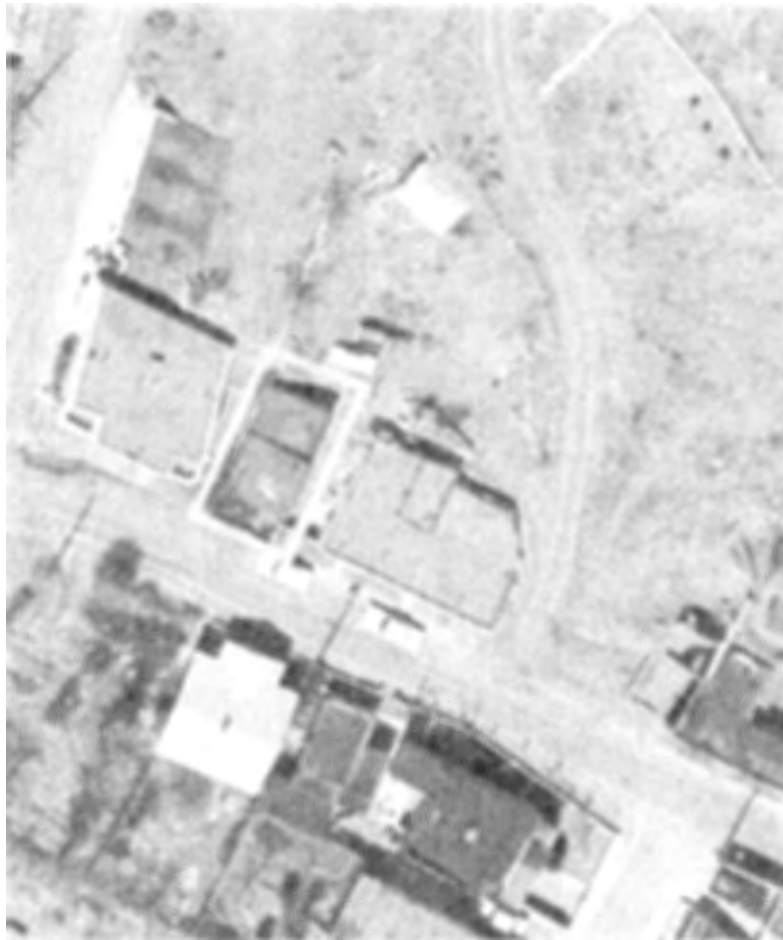
Figure 5: Portion February 27, 1969 aerial photograph showing rear addition and shed roof of older section. Courtesy New Mexico Department of Transportation.
