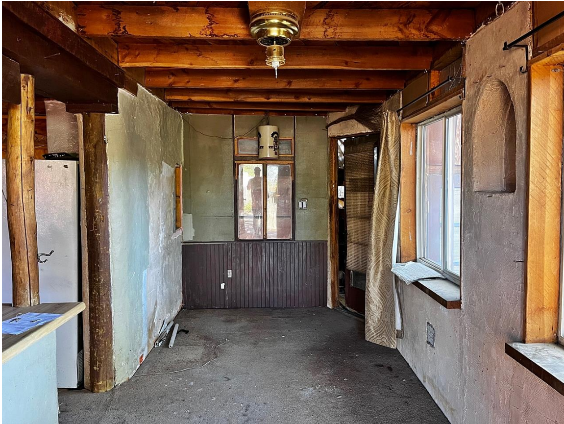
Photo 15: Post-1978 porch enclosure. Camera facing south.
