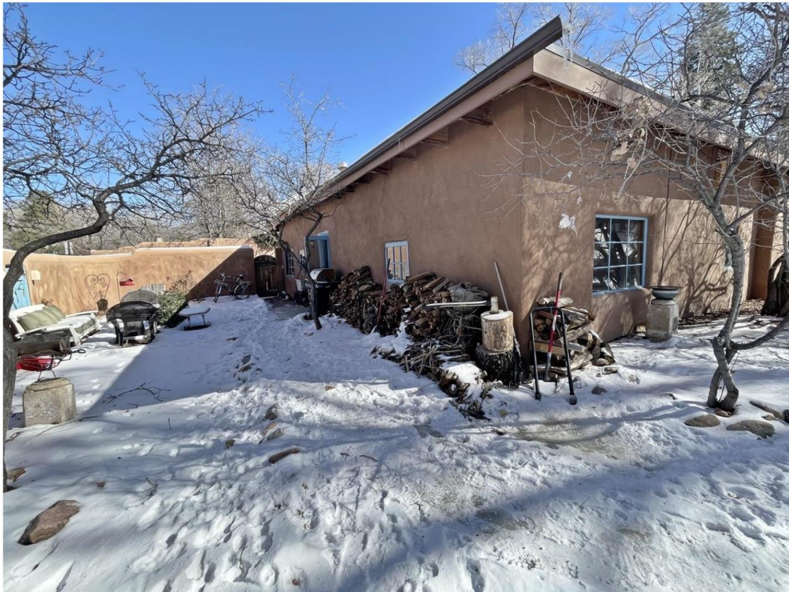
Photo 4: North and partial west elevations. Camera facing southeast.
