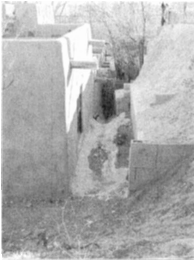
Photo 6: West elevation, facing south.
