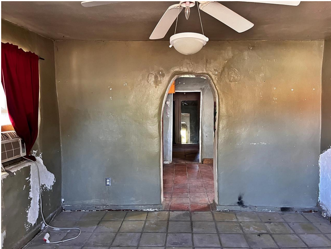
Photo 20: North room. Camera facing south.
