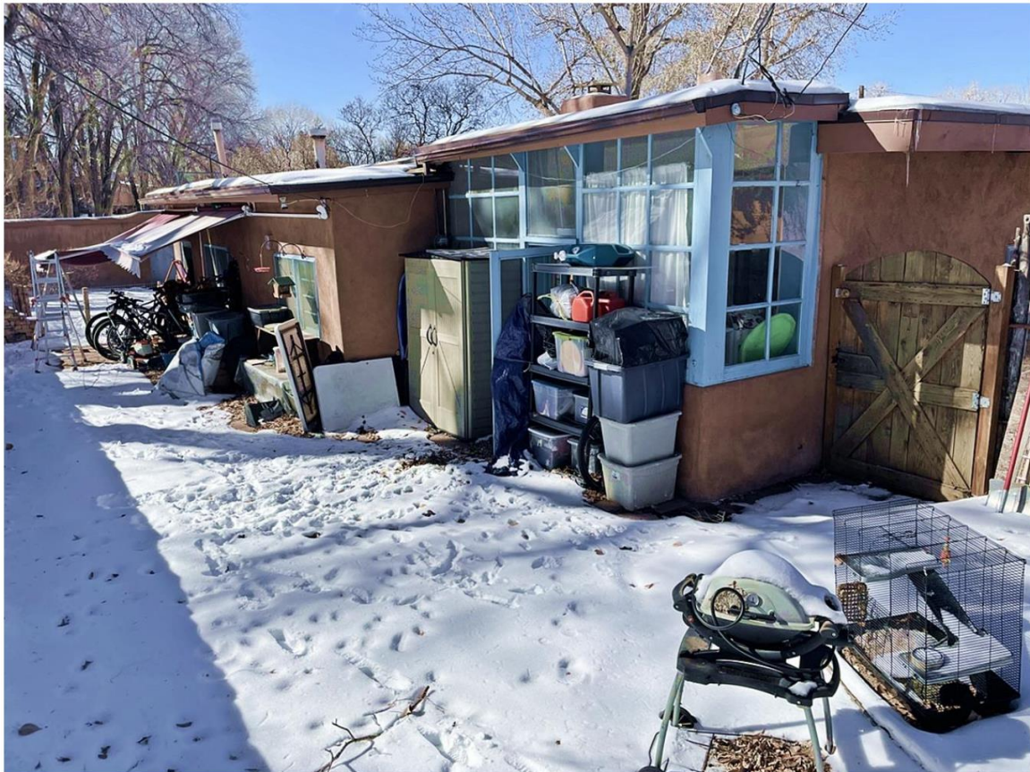
Photo 8: South elevation. Sun Room at right. Camera facing northwest.
