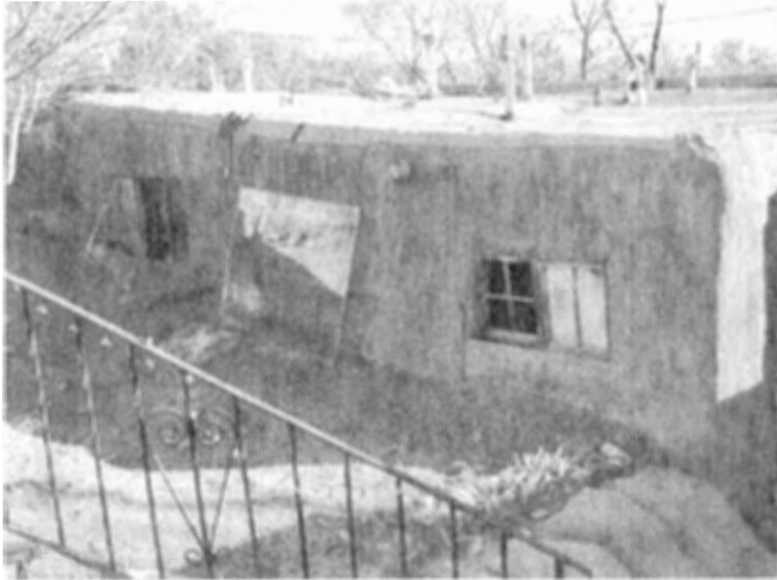
Photo 6: West end of north elevation, facing southeast.
