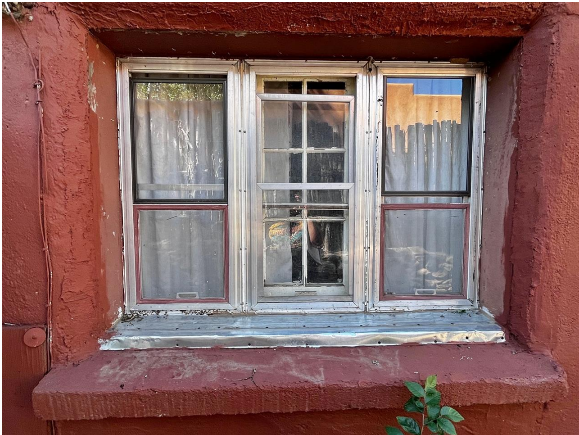
Photo 12: East elevation. Window at south room. Camera facing west.
