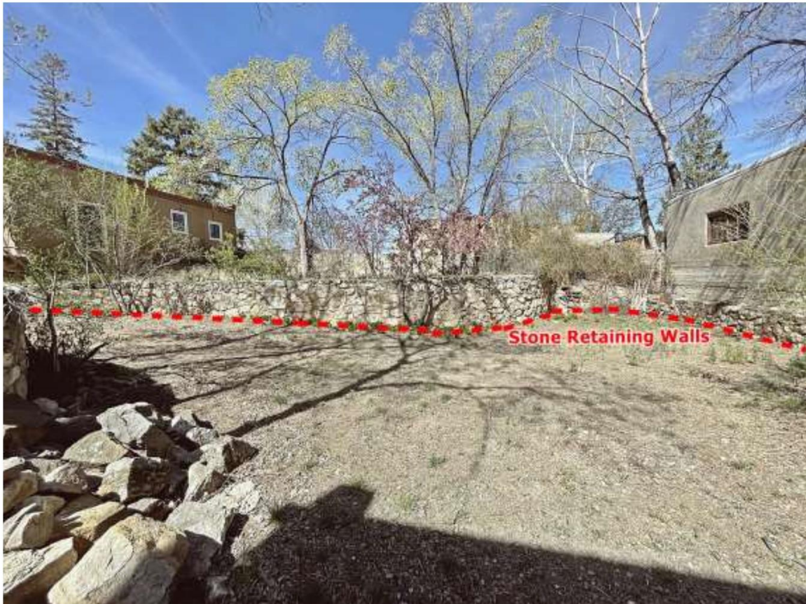
Photo 10: Perimeter stone retaining walls. Camera facing south.
