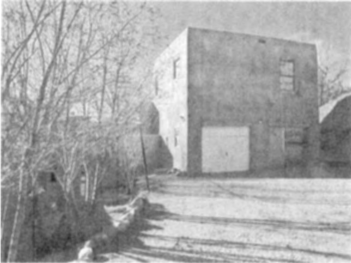
Photo 7: South and east elevations of two-story portion, facing northwest.
