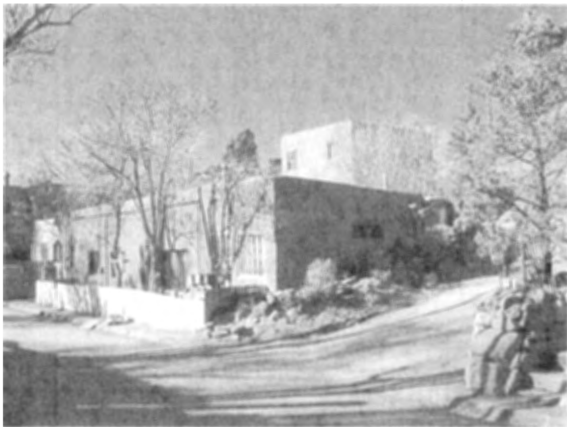
Photo 1: South and east elevations, facing northwest. Two-story portion of 367 ½ Hillside visible in background.
