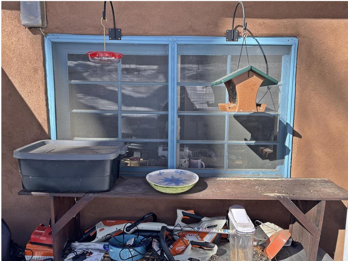
Photo 9: South elevation. West section. Windows. Camera facing northwest.
