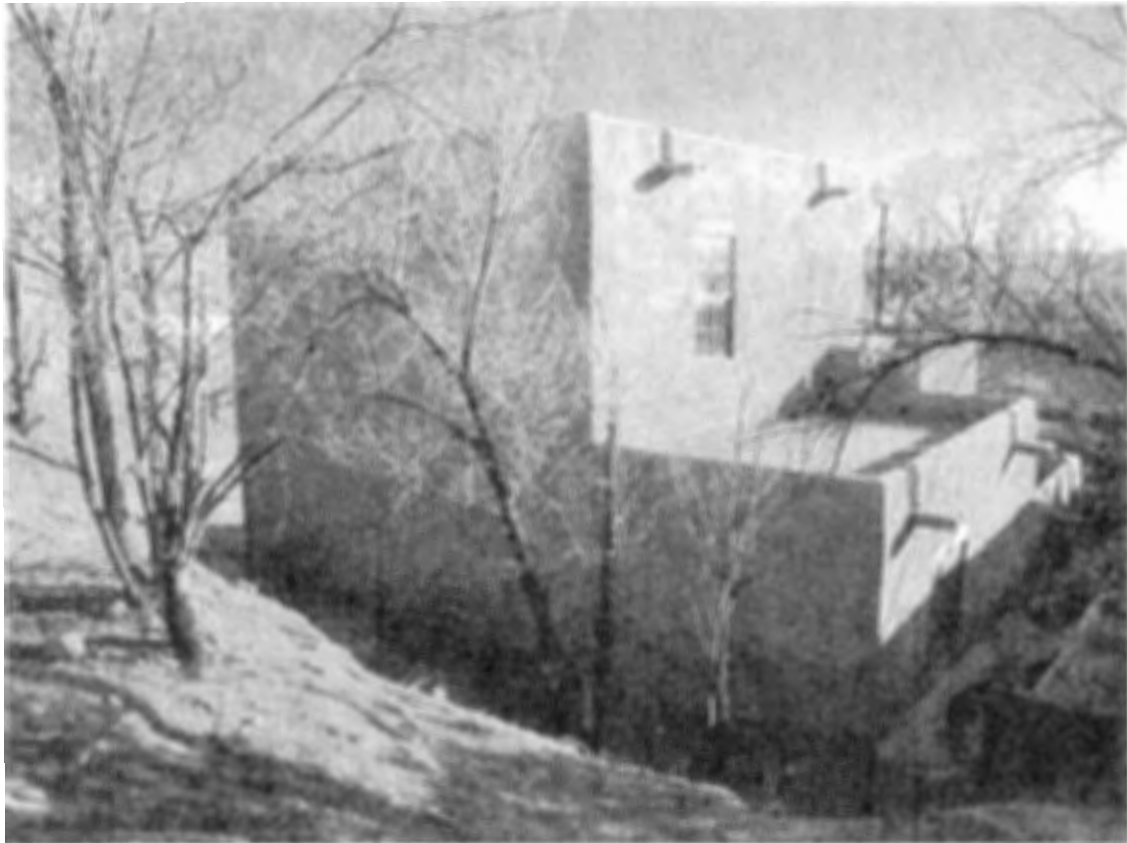
Photo 8: North and west elevations two-story portion, facing southeast.
