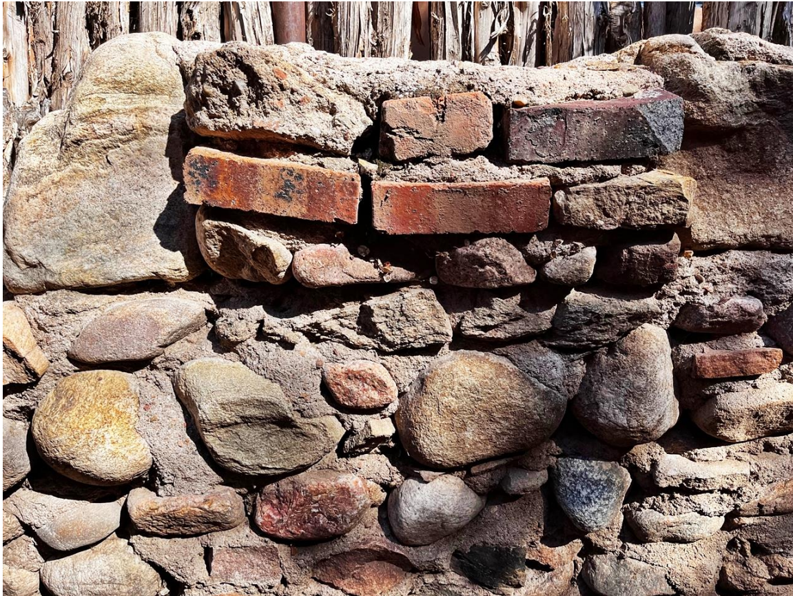
Photo 22: East property wall, detail. Camera facing east.
