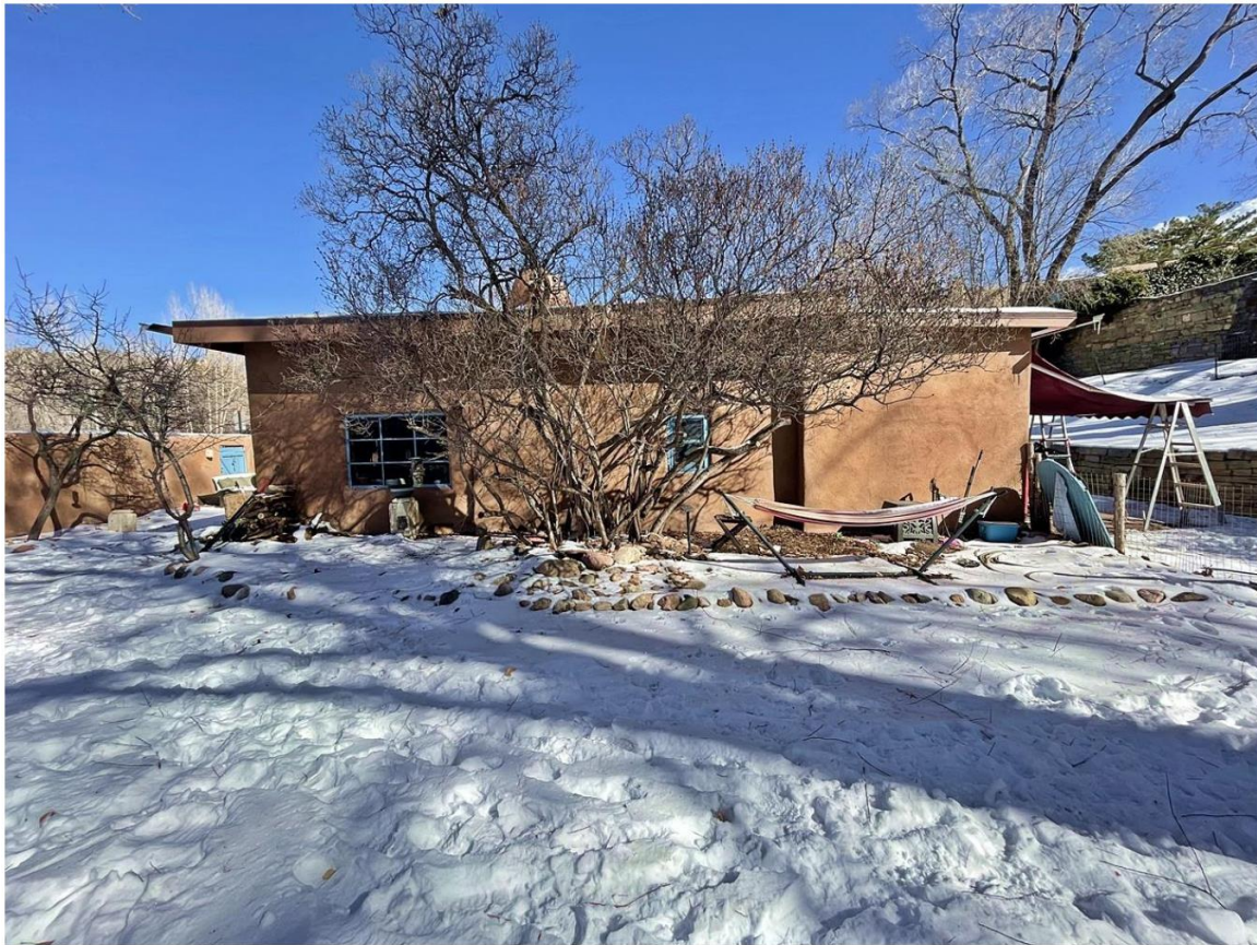
Photo 5: West elevation. Camera facing northeast.
