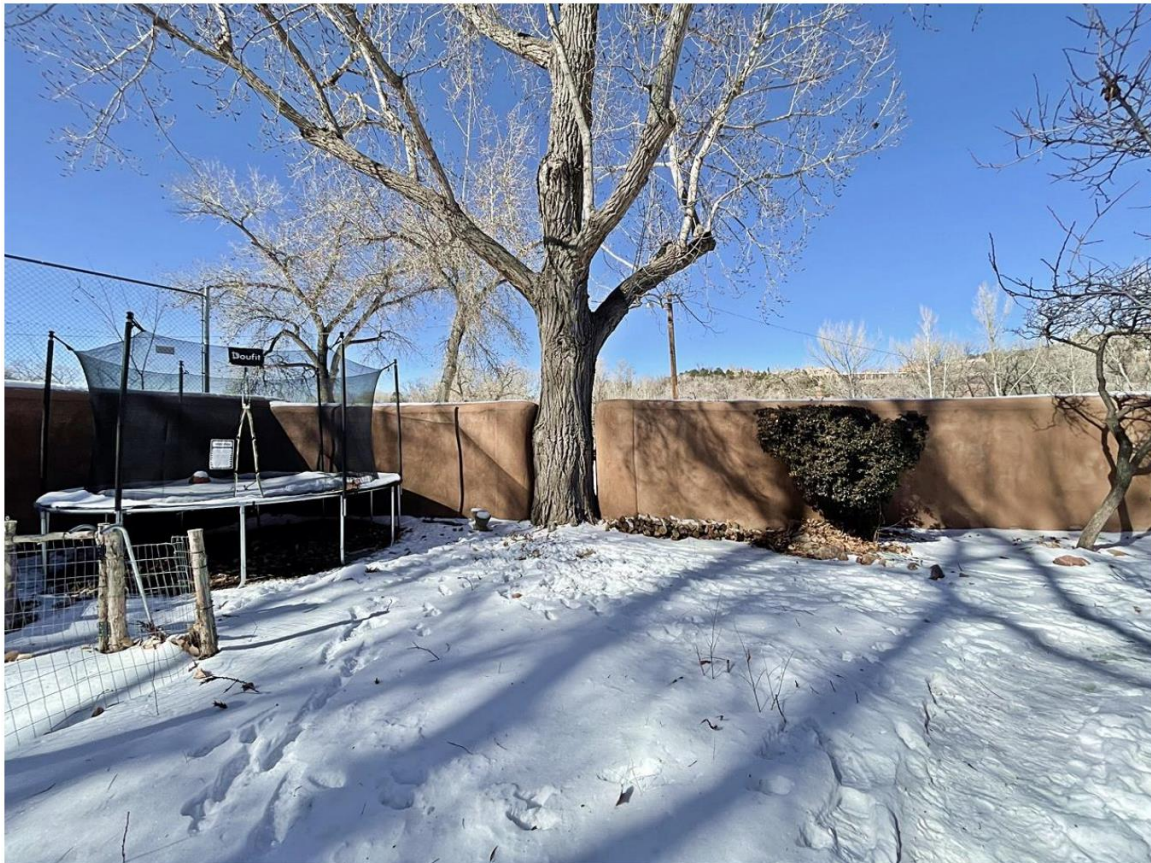
Photo 12: Perimeter Wall. Camera facing northwest.
