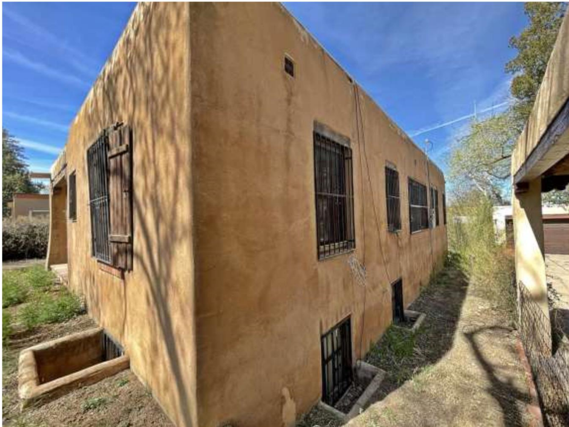
Photo 7: North elevation oblique. Camera facing southwest. Notice window wells on both elevations and tall basement windows on the north side.
