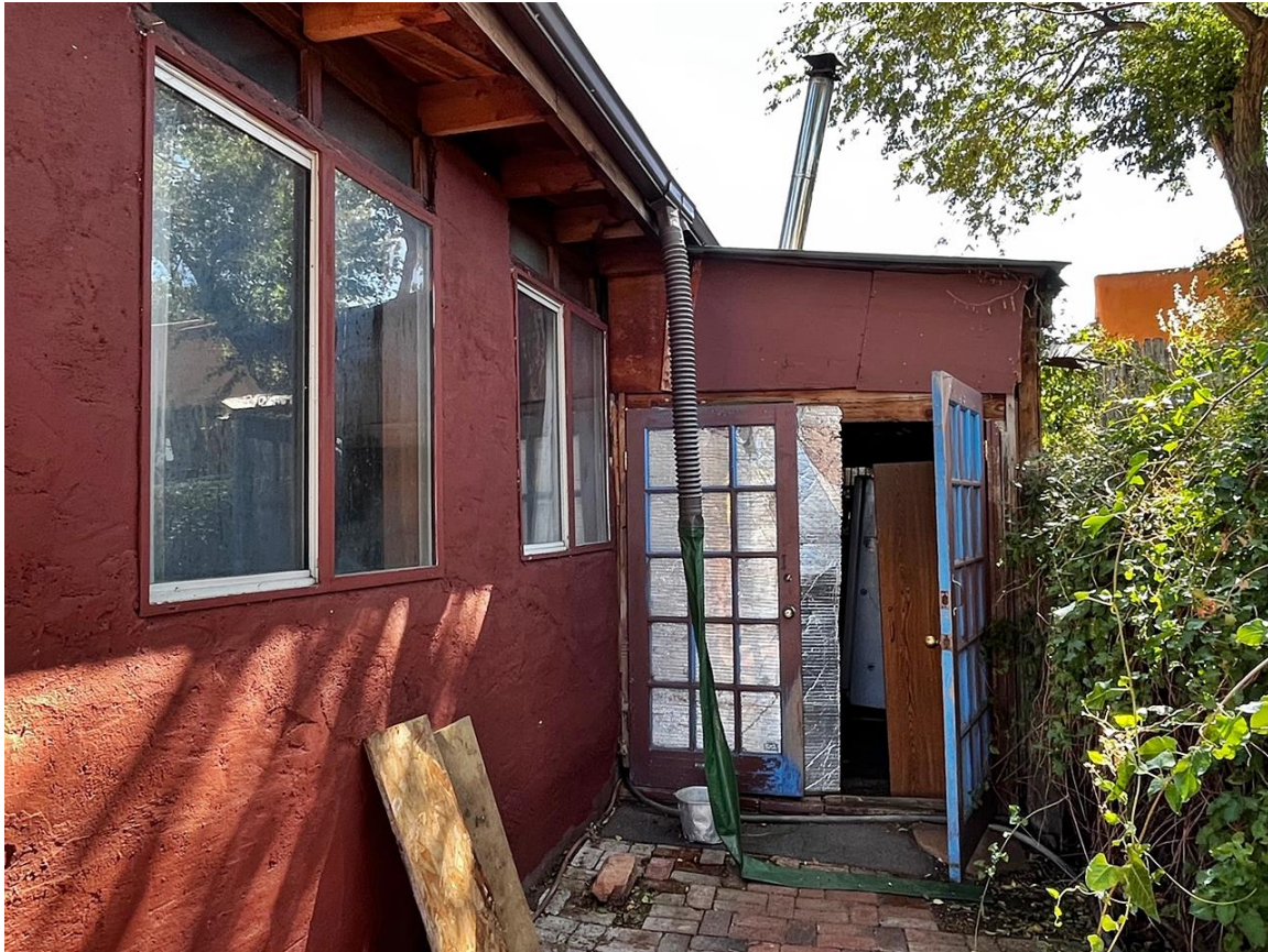
Photo 7: West elevation post-1978 porch enclosure (left); shanty (center). Camera facing south.
