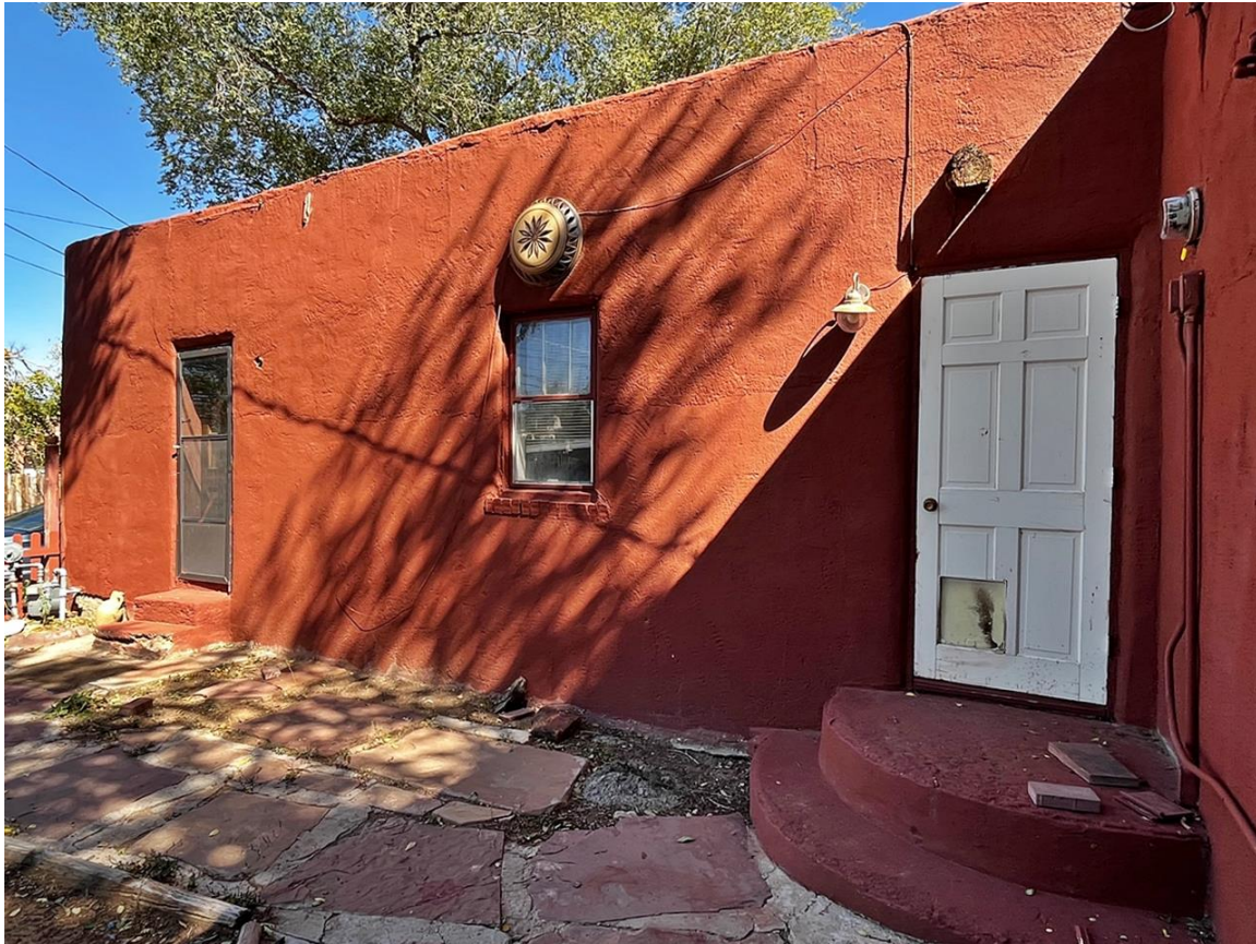
Photo 4: West elevation of older portion of building. Camera facing northeast.
