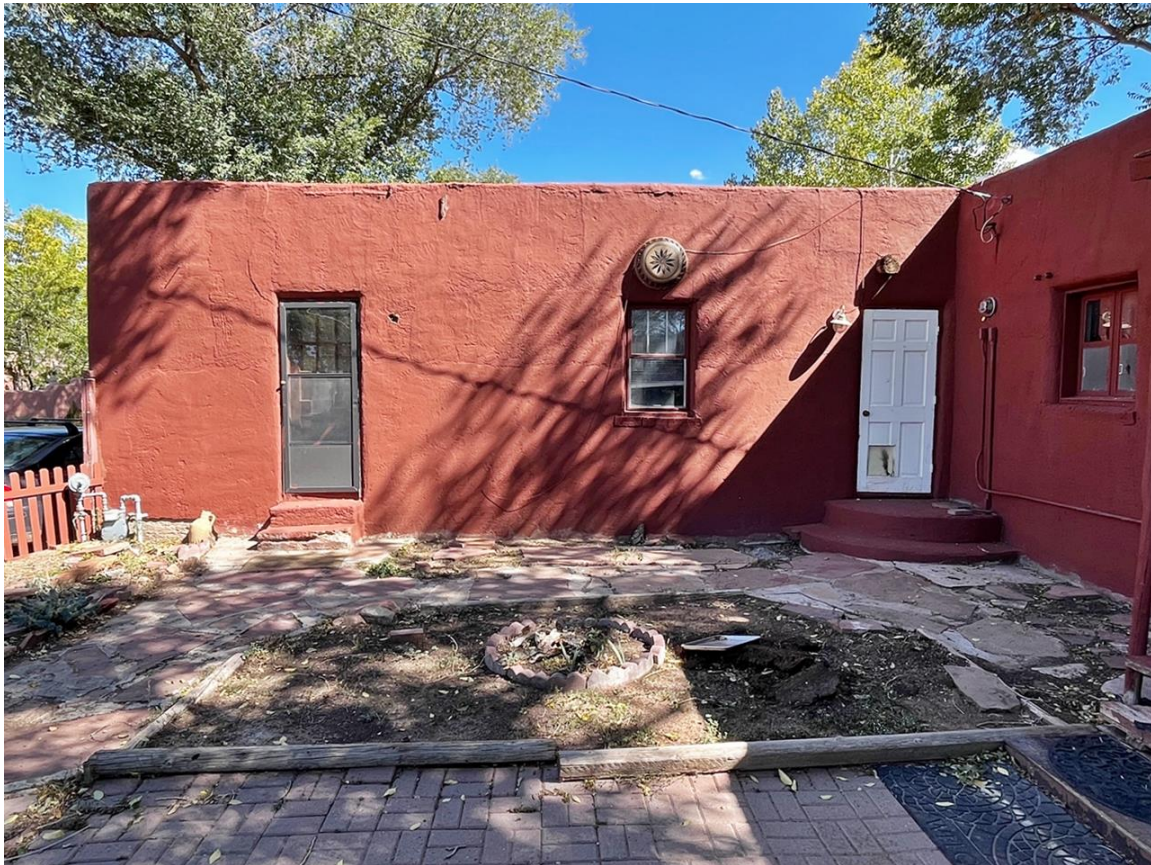
Photo 3: West elevation of older portion of building. Camera facing east.
