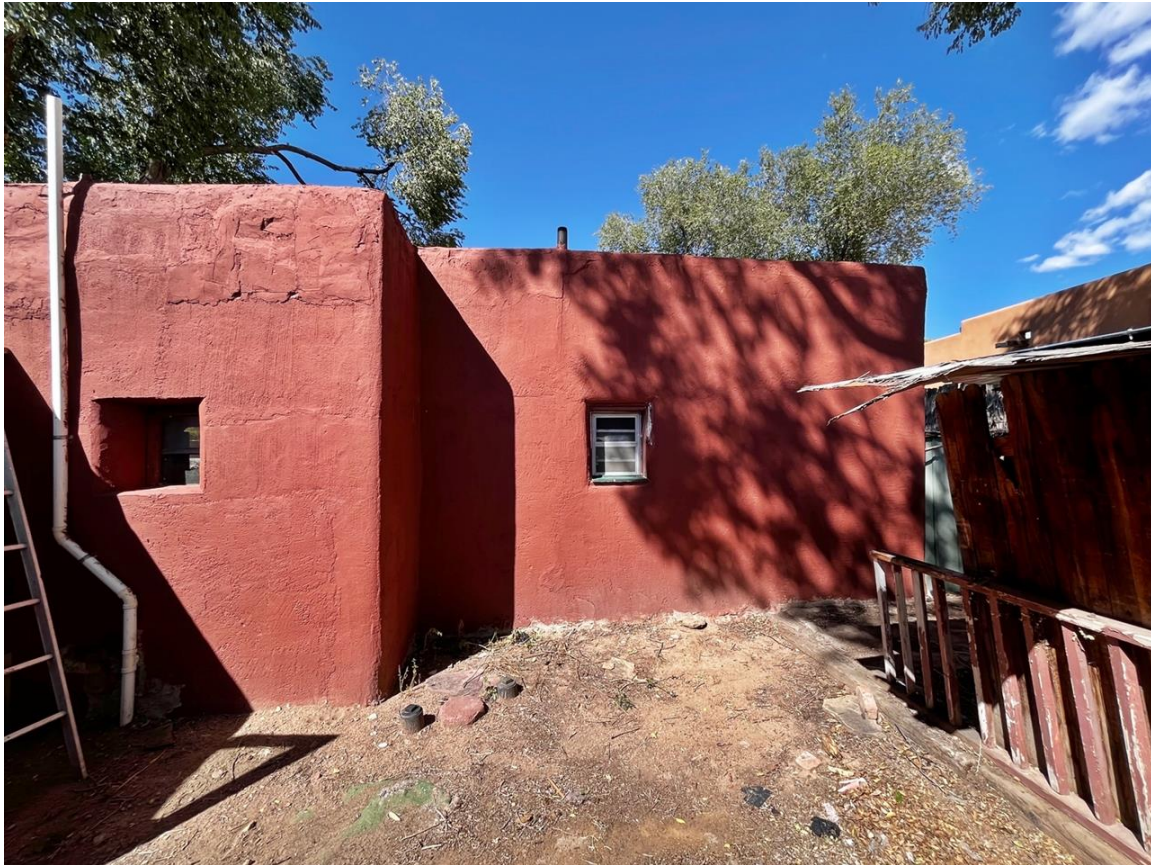
Photo 10: South elevation; kitchen (left); bathroom (right). Camera facing north.
