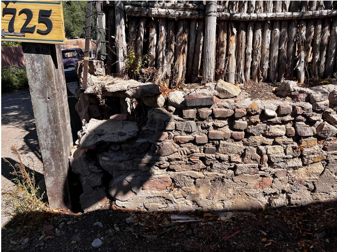
Photo 21: East property wall. Camera facing east.
