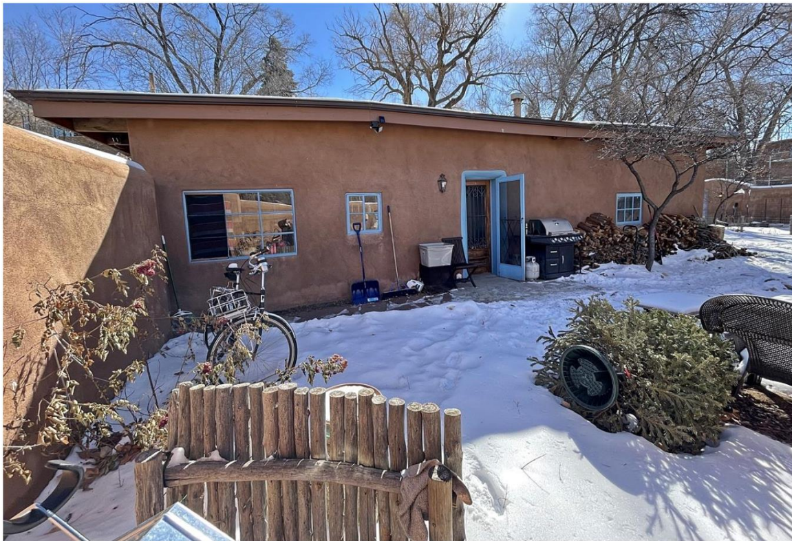
Photo 2: Front (north) façade. Camera facing southwest.
