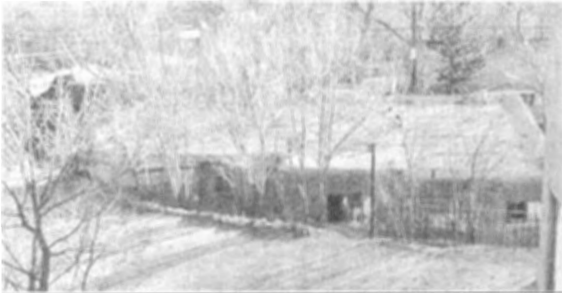
Photo 5: North elevation, facing south.
