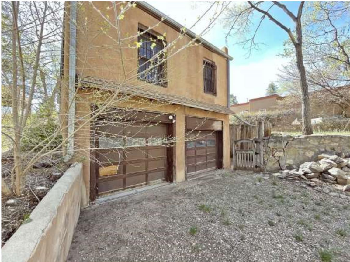
Photo 7: West elevation. Camera facing southeast.
