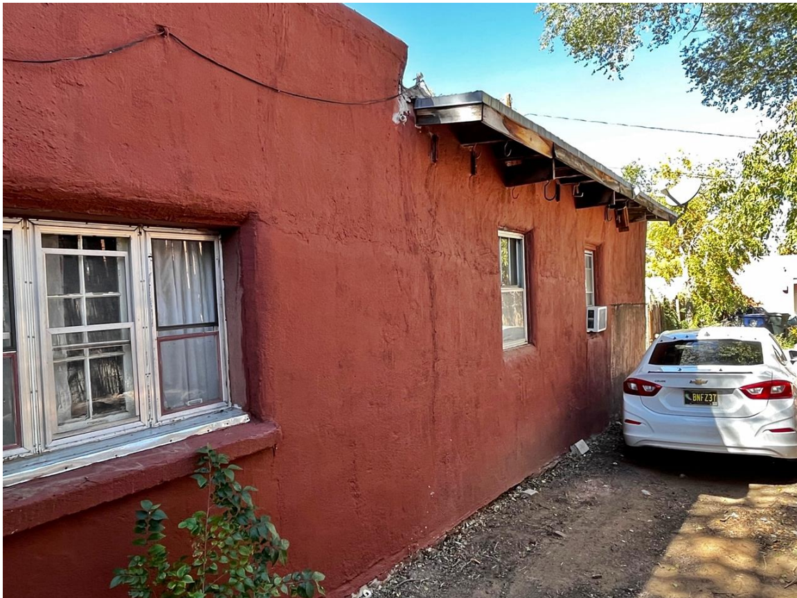
Photo 11: Partial east elevation. Camera facing northwest. Note change in parapet height and window pattern and placement.
