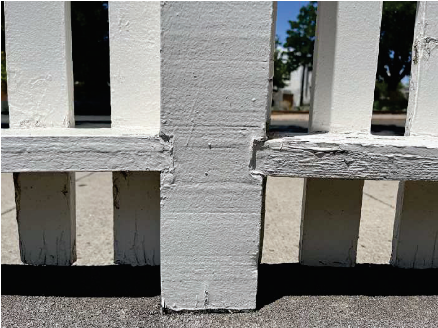
Figure 5: Dado connection. July 25, 2023, John W. Murphey.
