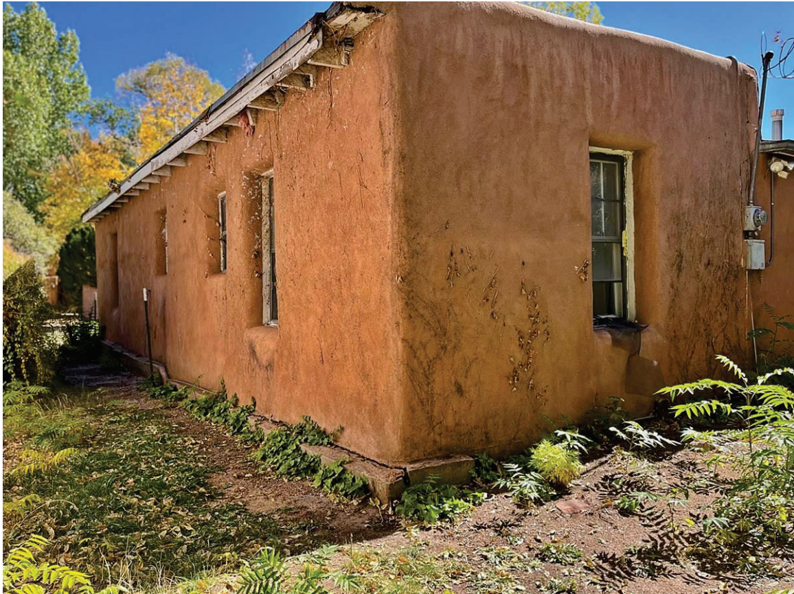
Photo 13: North and west elevations of Bedroom Wing. Camera facing northeast.
