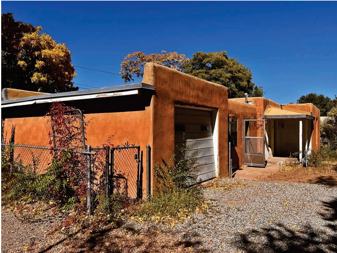
Photo 3: East façade, Garage (c.1966-1973). Camera facing northeast.
