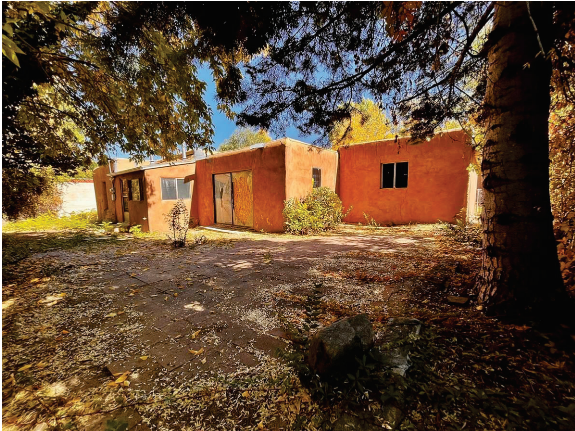
Photo 16: Full west elevation. Camera facing northeast.
