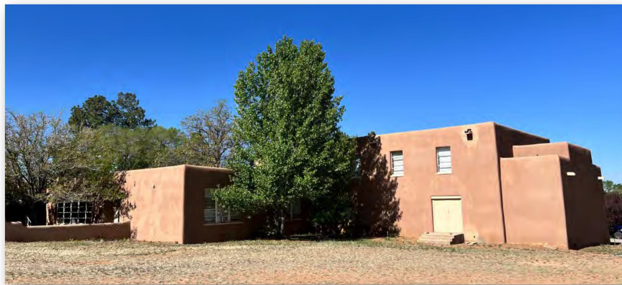
Fatima Building East Elevation (north side)
