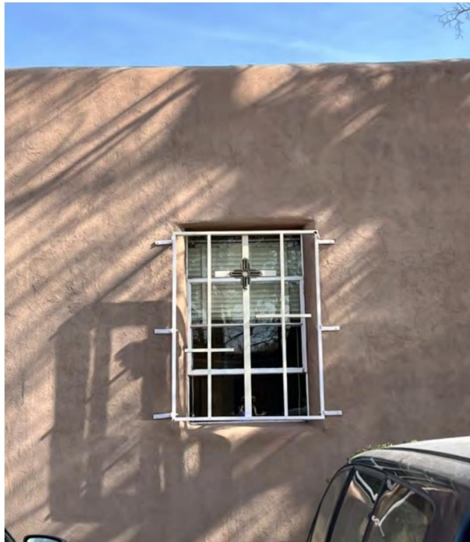
Figure 7. Security Bars at South
