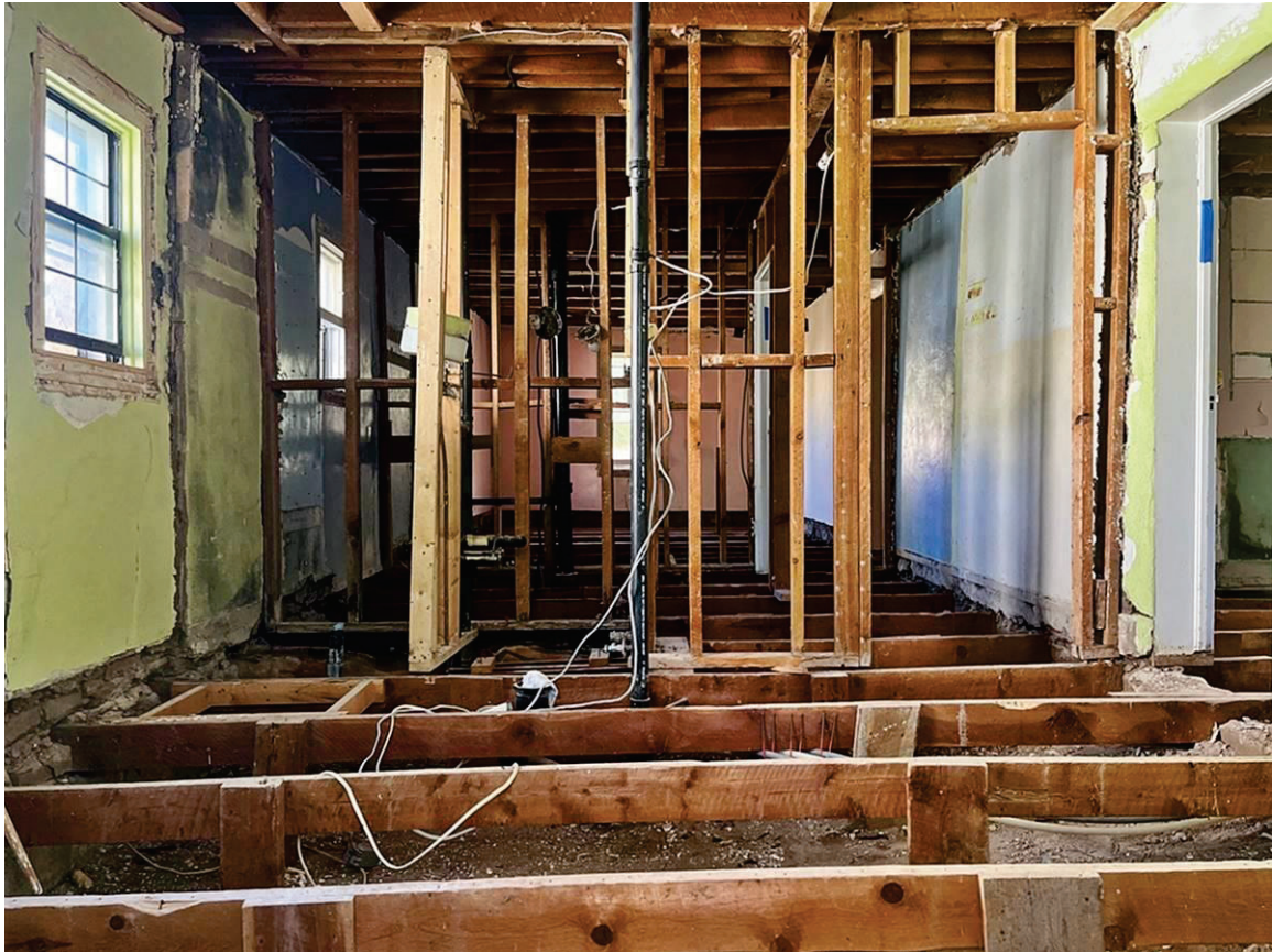
Photo 15: Bedroom Wing interior. Camera facing east.
