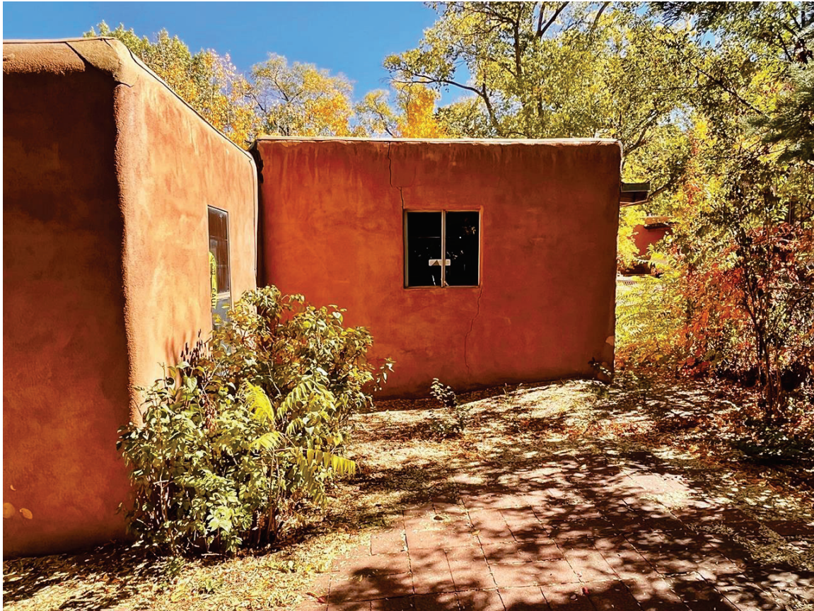
Photo 20: West elevation, Garage (c.1966-1973). Camera facing east.
