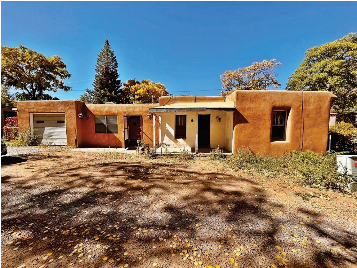
Photo 2: Full east façade. Camera facing southwest.
