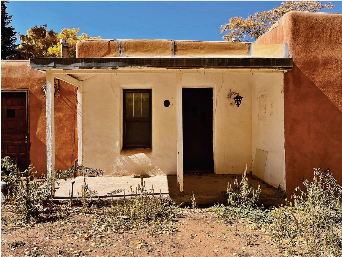
Photo 6: East façade, Porch (c.1966-1973). Camera facing west.
