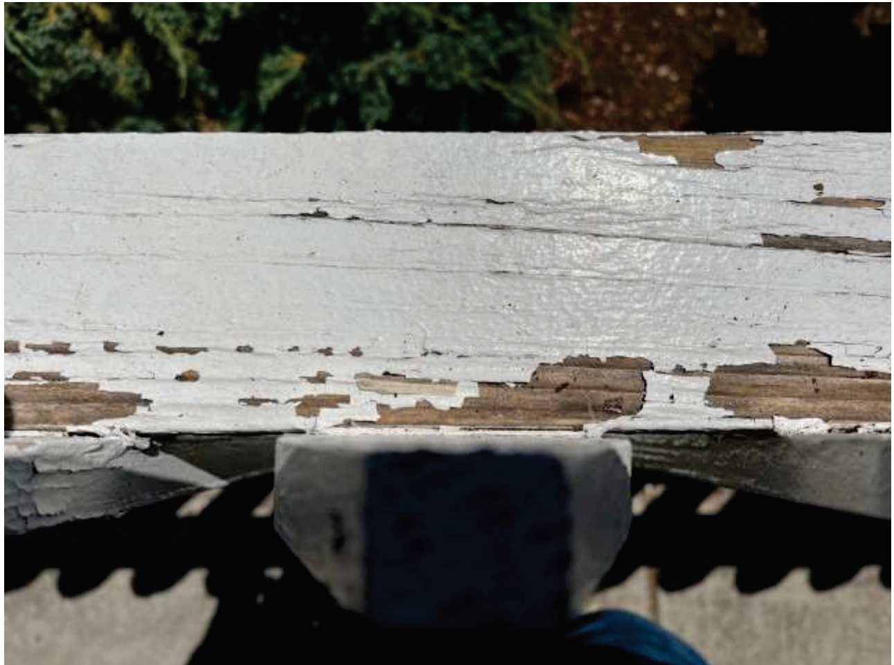
Figure 7: Top rail with only one layer of paint. July 25, 2023, John W. Murphey.
