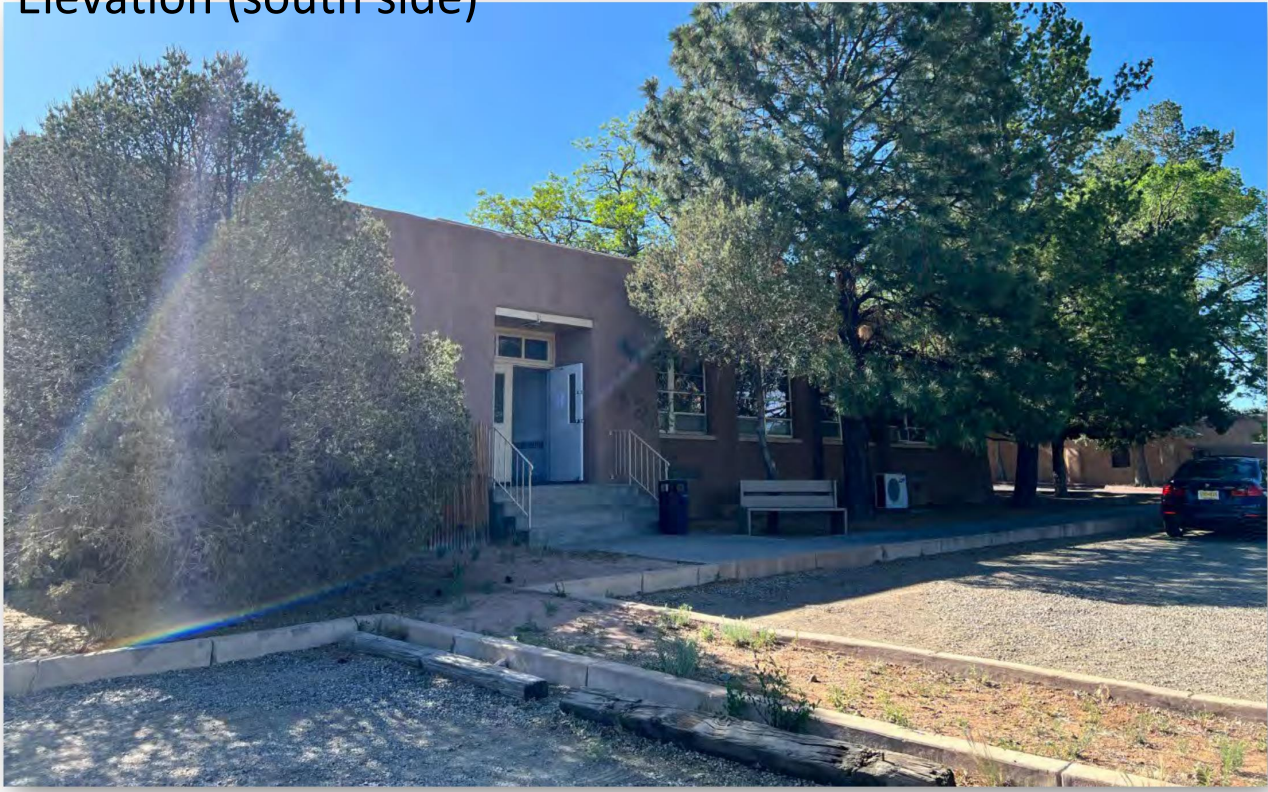
Fatima Building West Elevation (south side)
