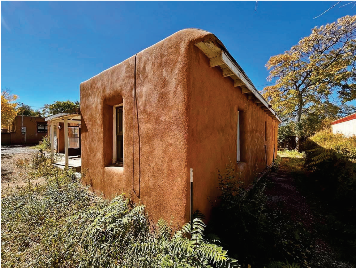
Photo 12: East and north elevations of Bedroom Wing. Camera facing southeast.
