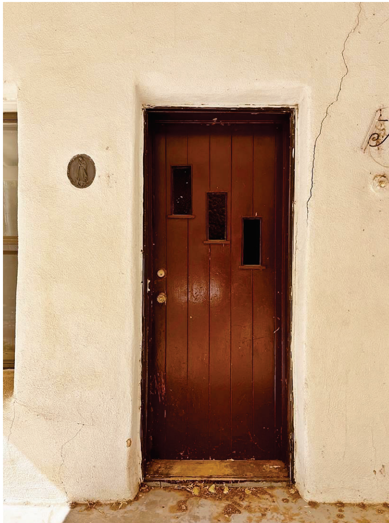
Photo 8: East façade, entry. Camera facing west.
