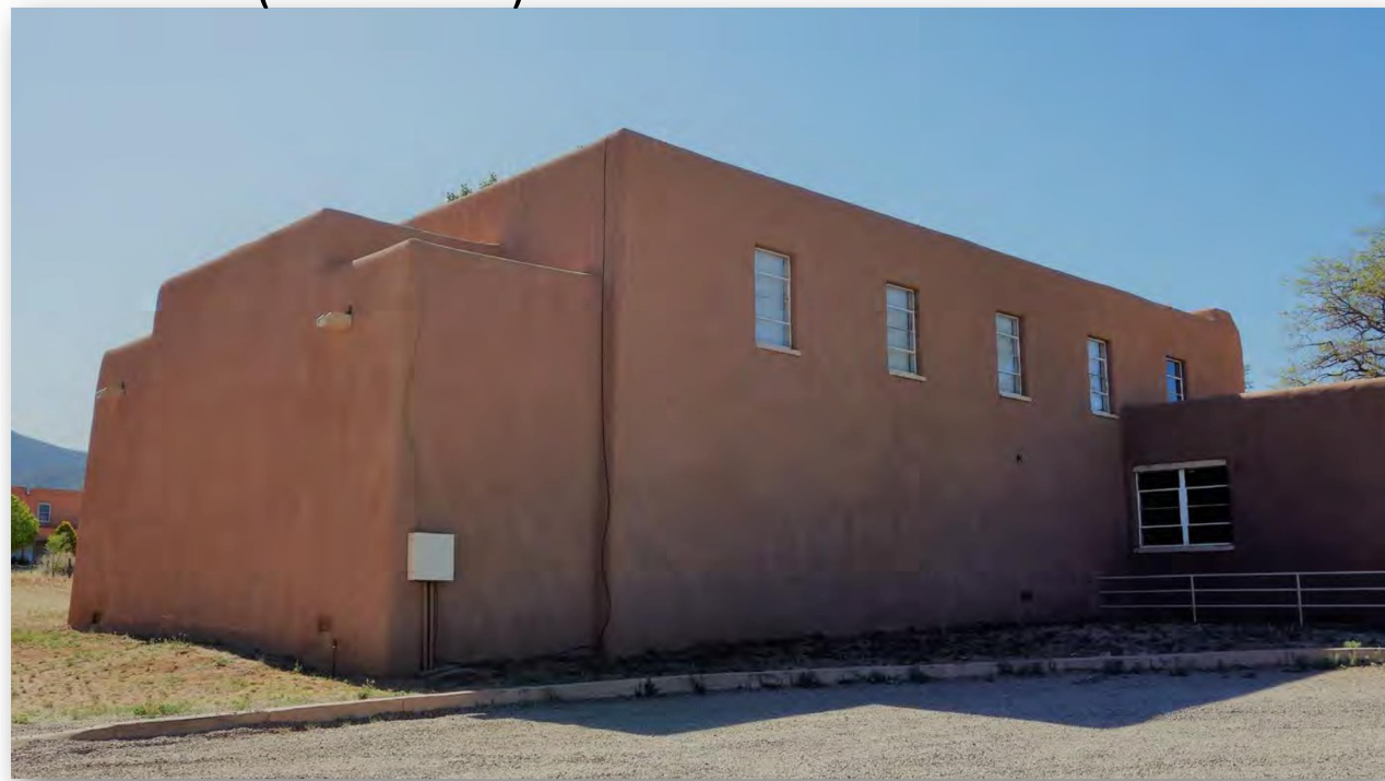
Fatima Building West Elevation (north side)
