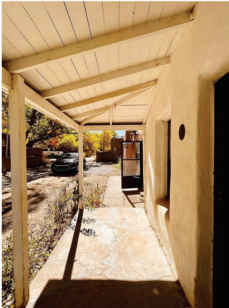
Photo 7: Porch, decking. Camera facing south.
