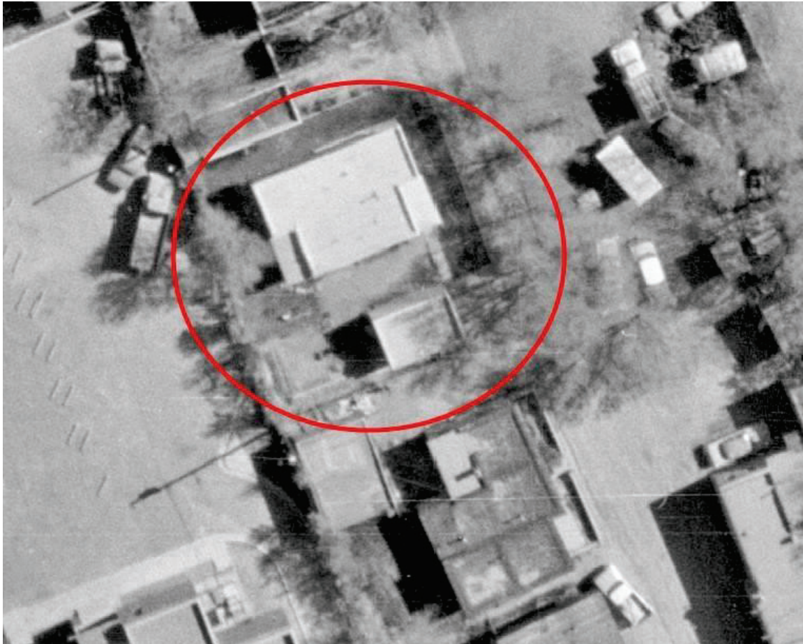
Figure 7: May 11, 1973, aerial photograph. Note presence of Laundry Room, Porch, and freestanding Garage. Note absence of Family Room.
