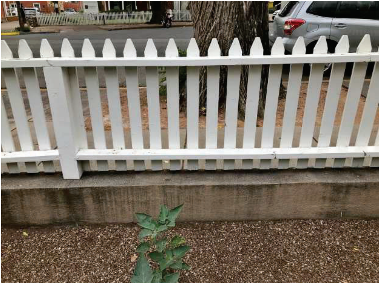
Figure 5: Concrete curb or base. July 2, 2021, John W. Murphey.
