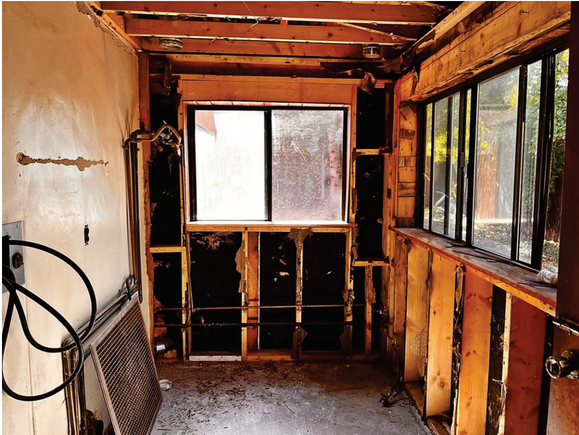
Photo 18: Laundry Room interior. Camera facing south.
