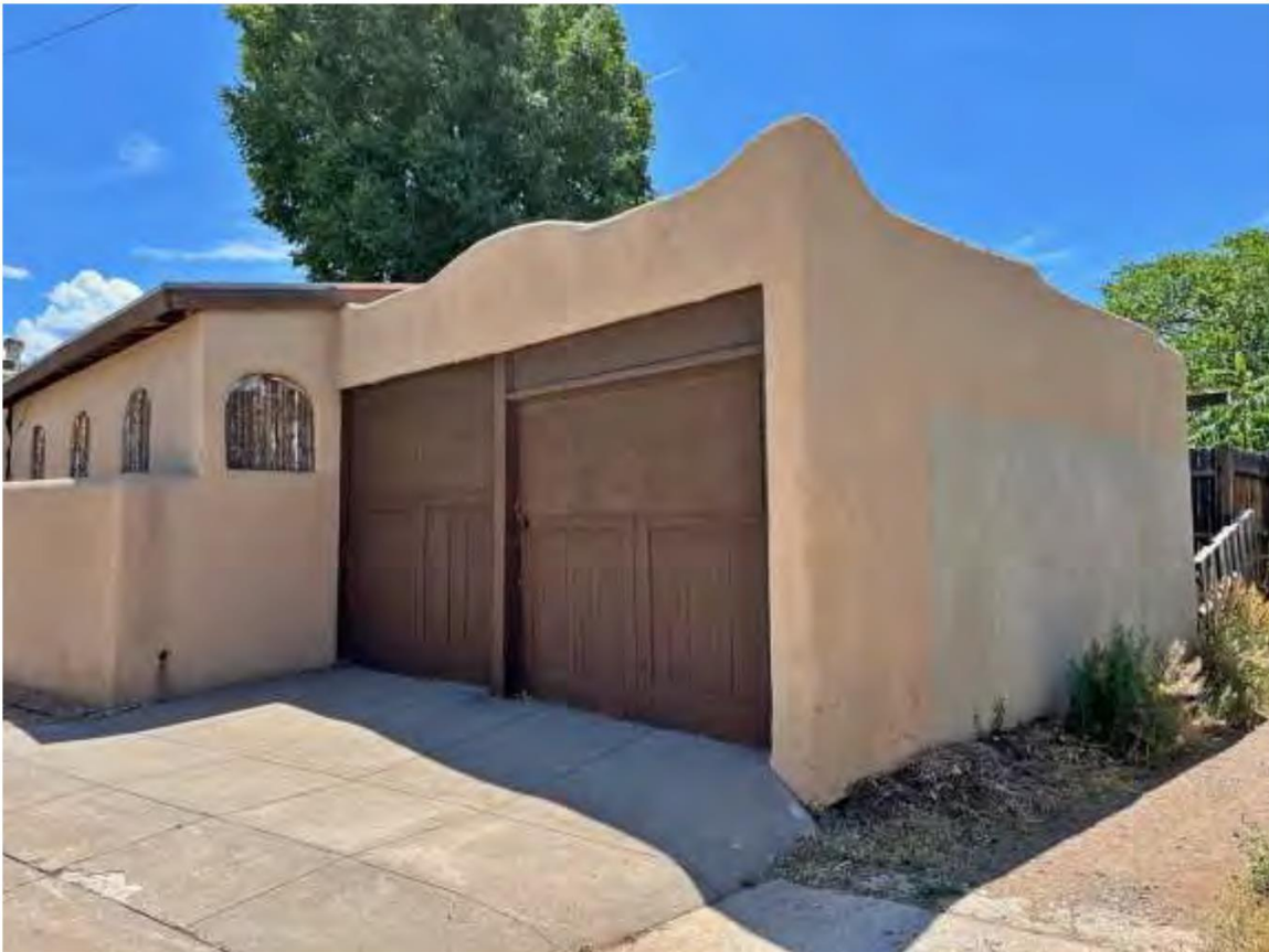
Photo 12: Garage, north and west elevations. Camera facing southeast.
