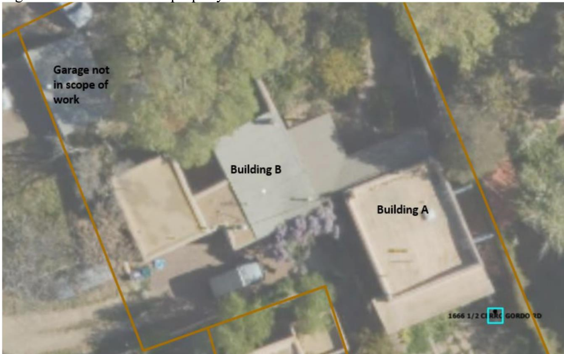
Figure 2: Structures of the property:
