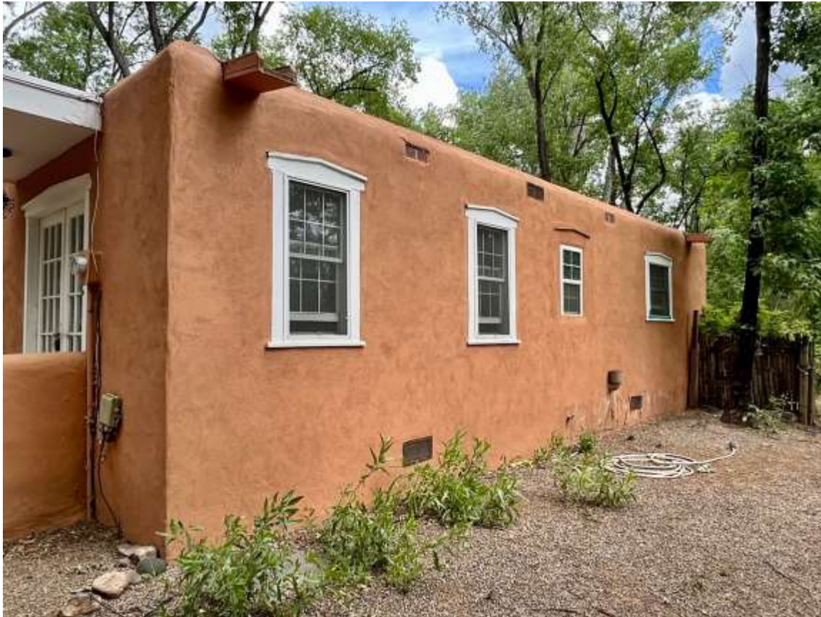
Photo 10: West elevation. Camera facing southeast.
