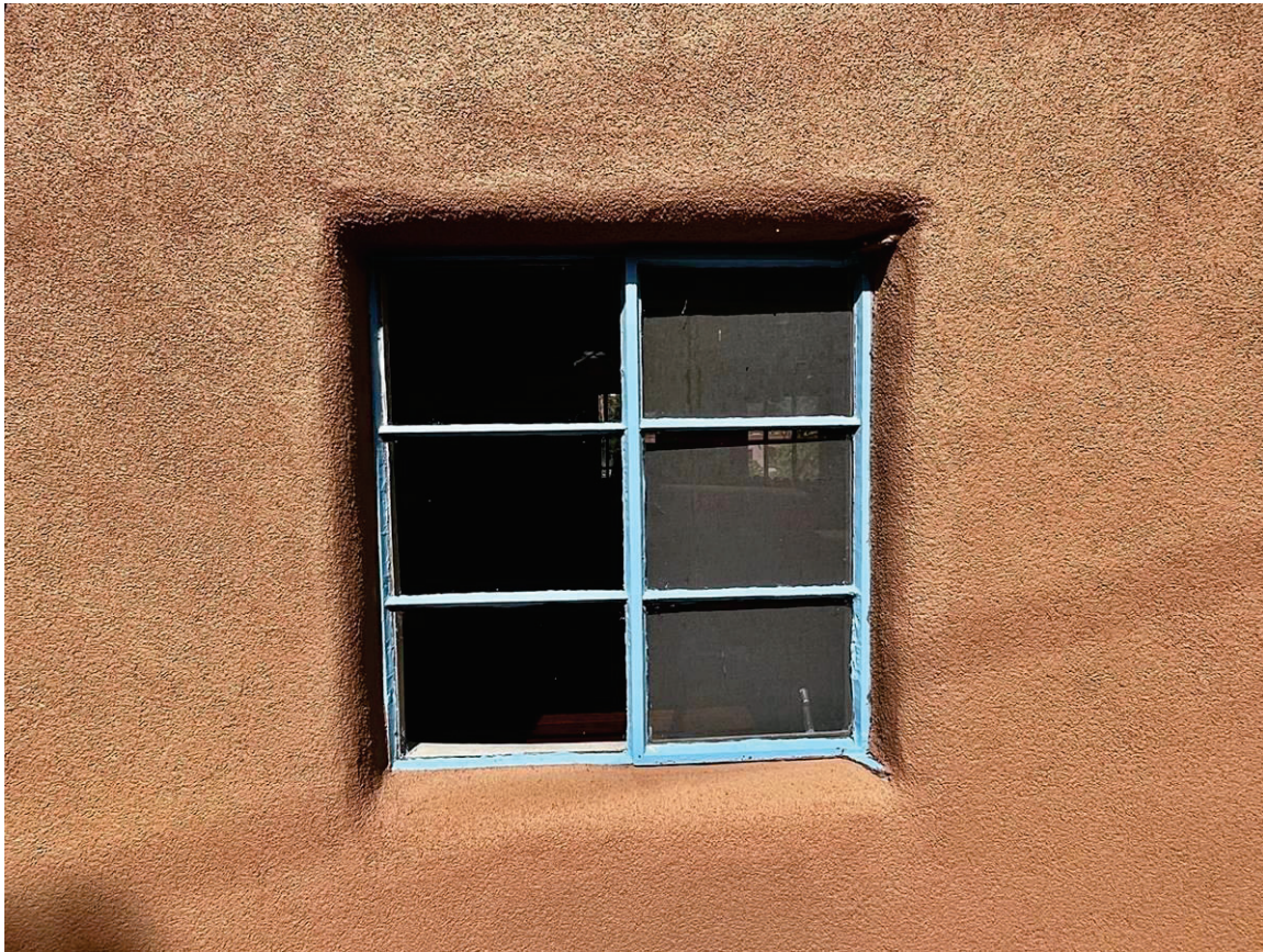
Photo 13: South elevation. Casement window at living room. Camera facing north. October 4, 2023, JWM.
