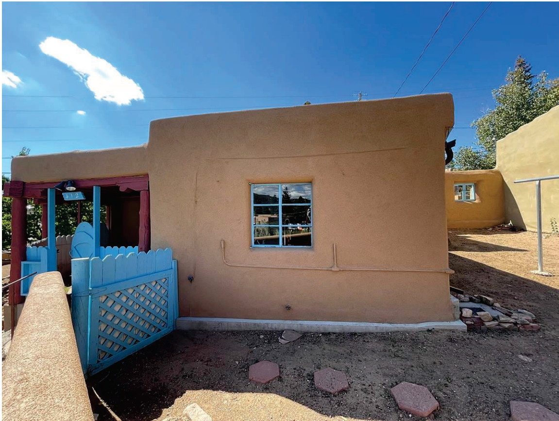
Photo 9: North elevation. Camera facing southwest. September 21, 2023, GC.
