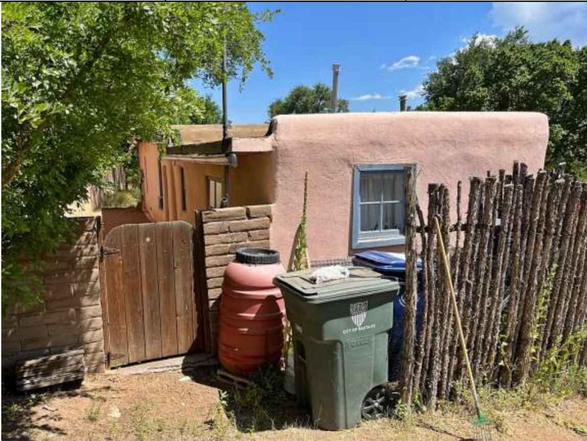
Photo 10: South elevation, assumed addition. Camera facing northeast.
