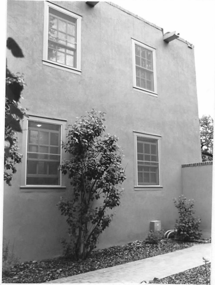
#7 south part of west elevation
