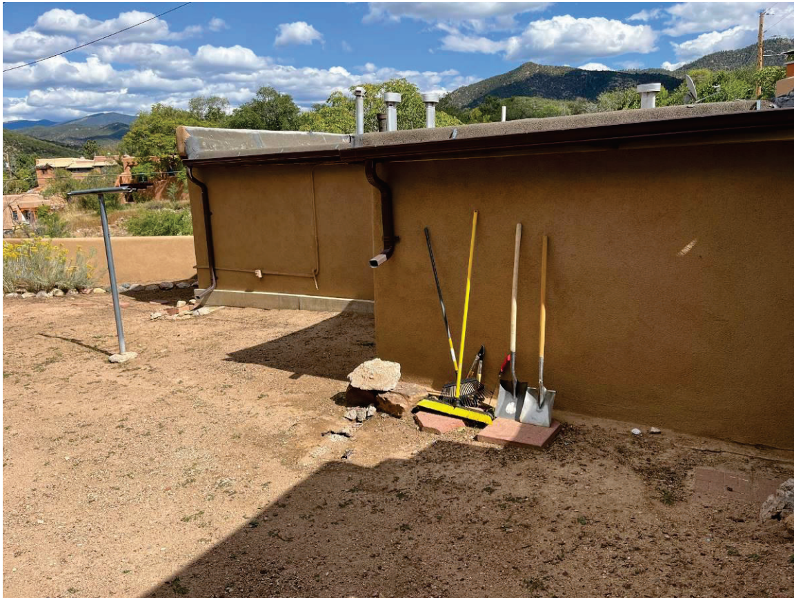
Photo 11: West elevation. Closet addition at right. Camera facing northeast. October 4, 2023, JWM.
