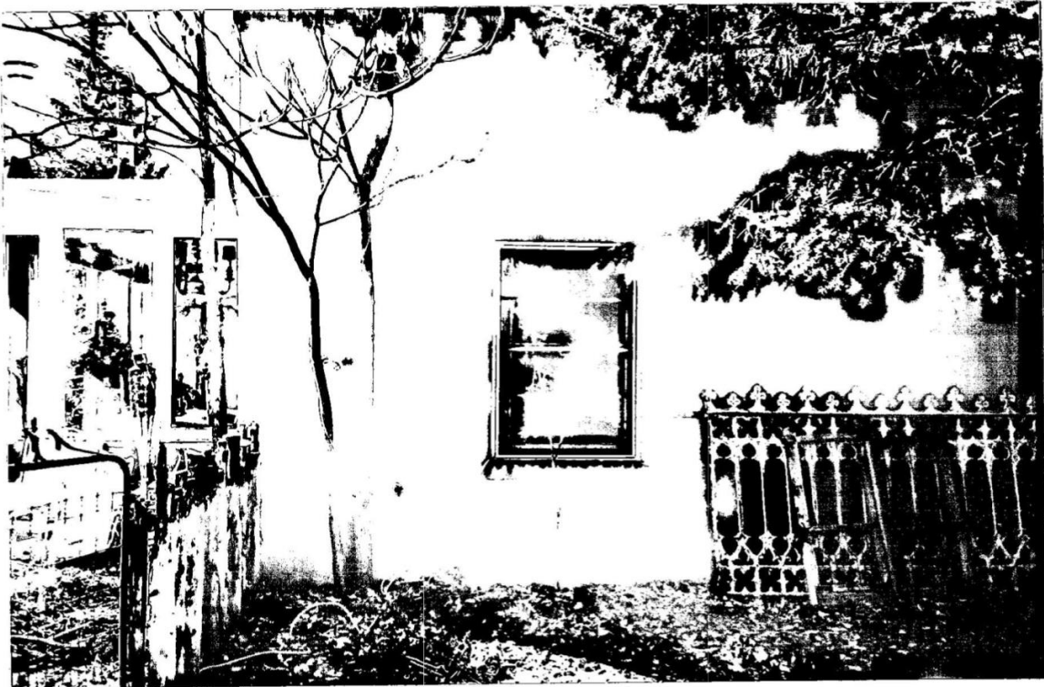
East elevation, south end & sun porch
