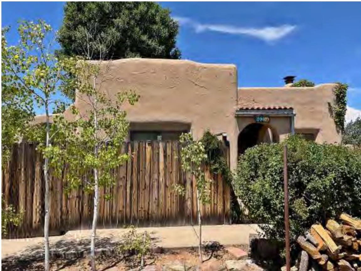
Photo 3: Front (east) façade. Camera facing west.
