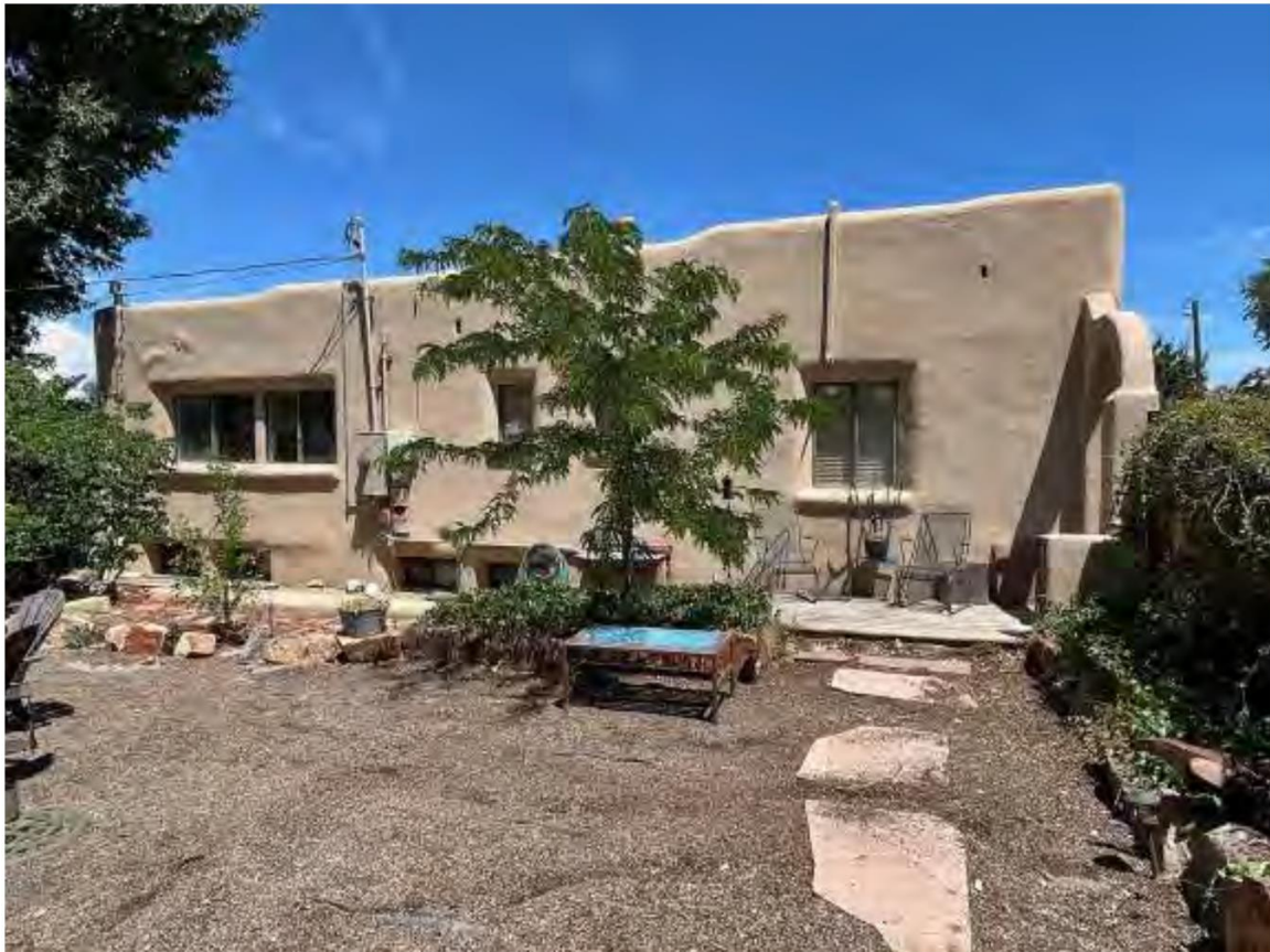
Photo 9: South elevation. Camera facing northwest.
