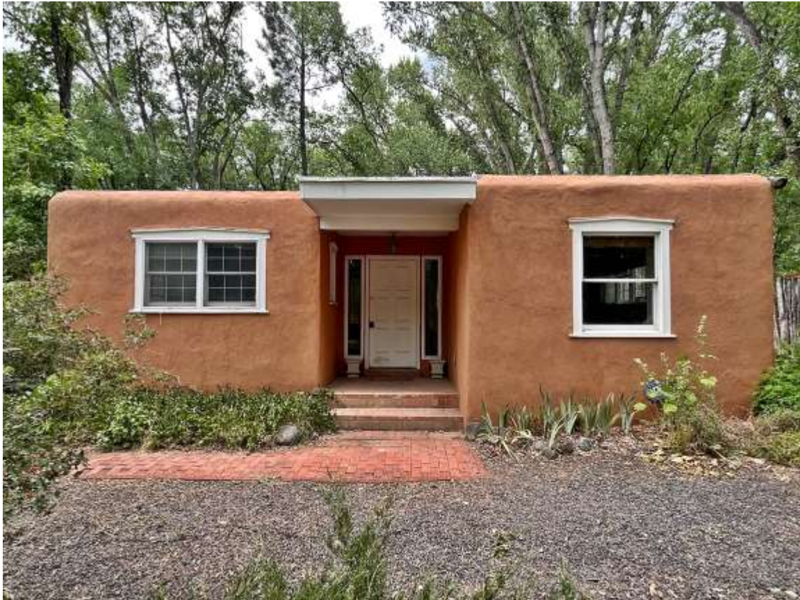
Photo 3: South (front) façade. Camera facing north.
