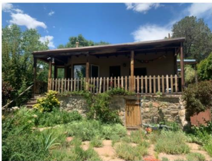
(3) South Façade of 696 s.f. Casita Showing Root Cellar and portal
