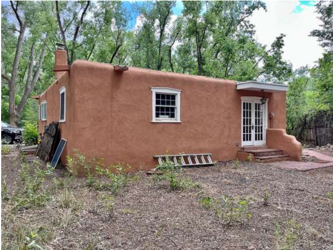
Photo 9. North elevation. Camera facing southwest.
