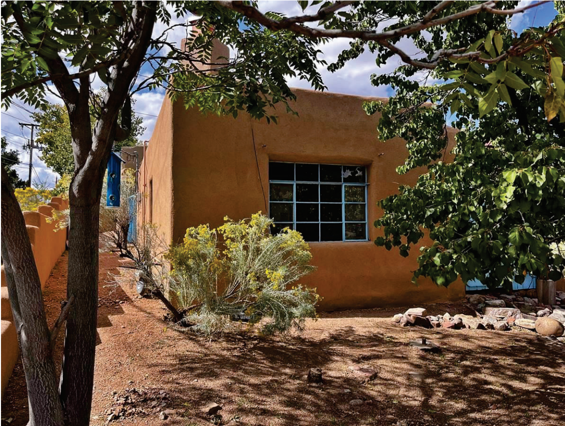
Photo 3: East elevation, living room window. Camera facing northwest. October 4, 2023, JWM.
