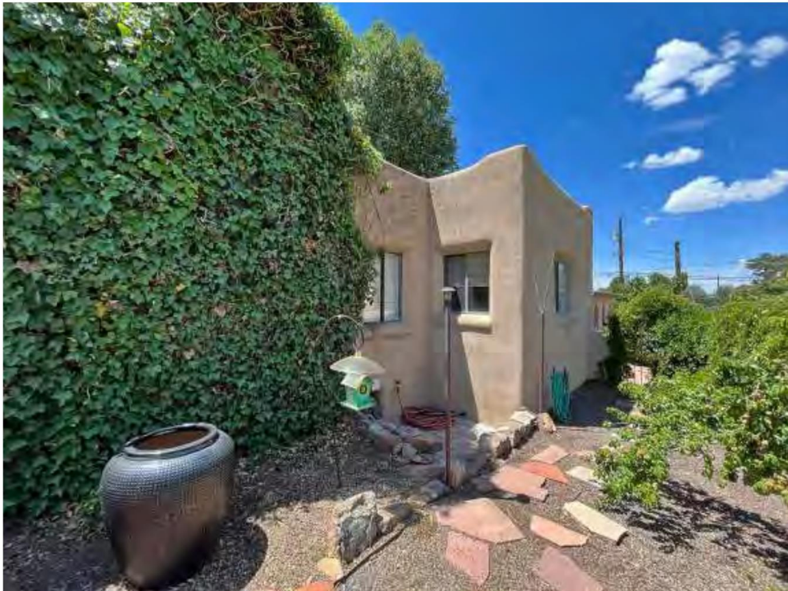
Photo 6: North elevation. Camera facing southeast.
