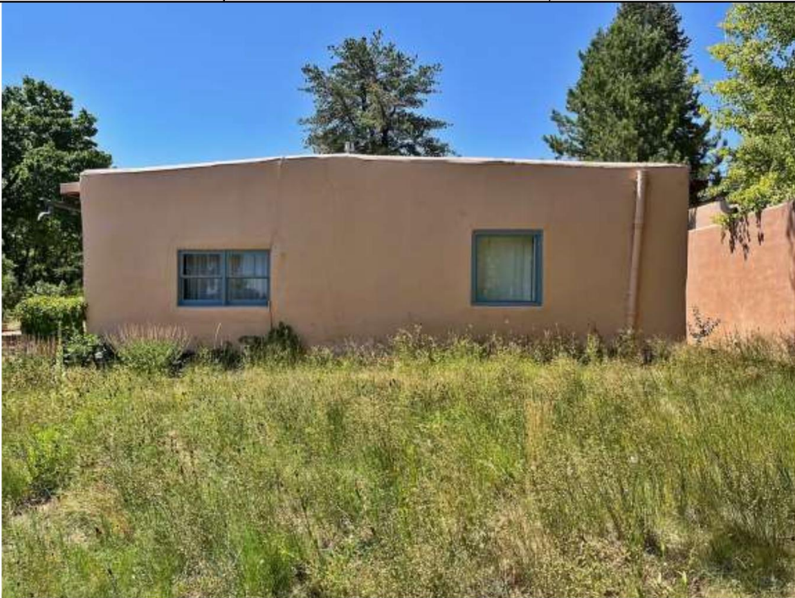
Photo 11: North elevation. Camera facing south.
