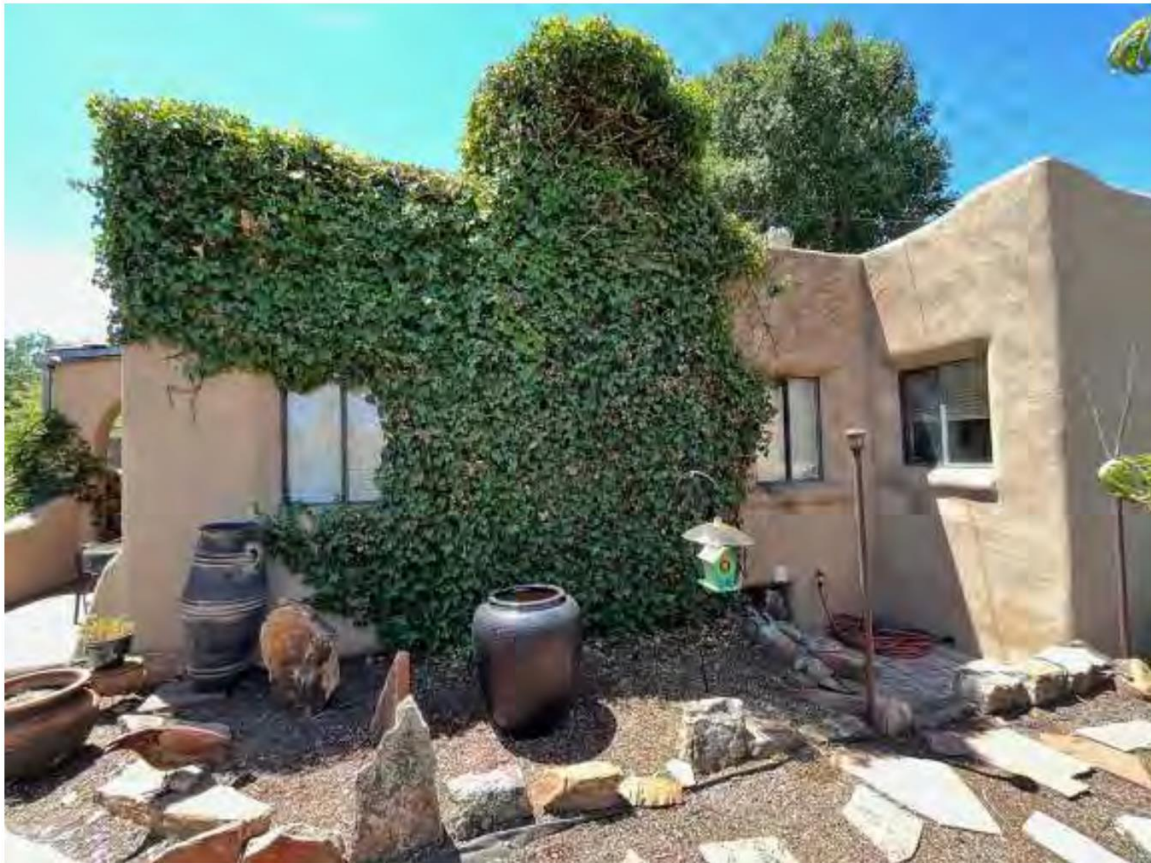
Photo 5: North elevation. Camera facing southwest.
