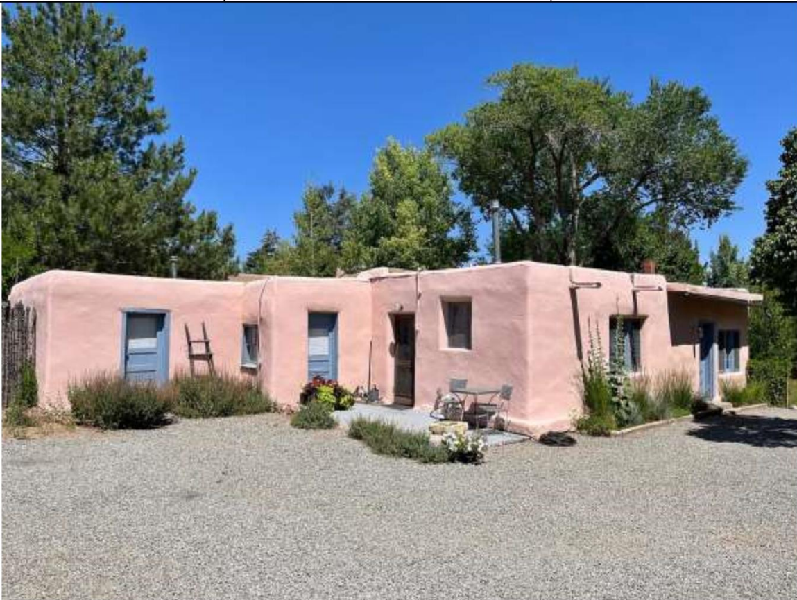
Photo 3: East elevation. Camera facing northwest.
