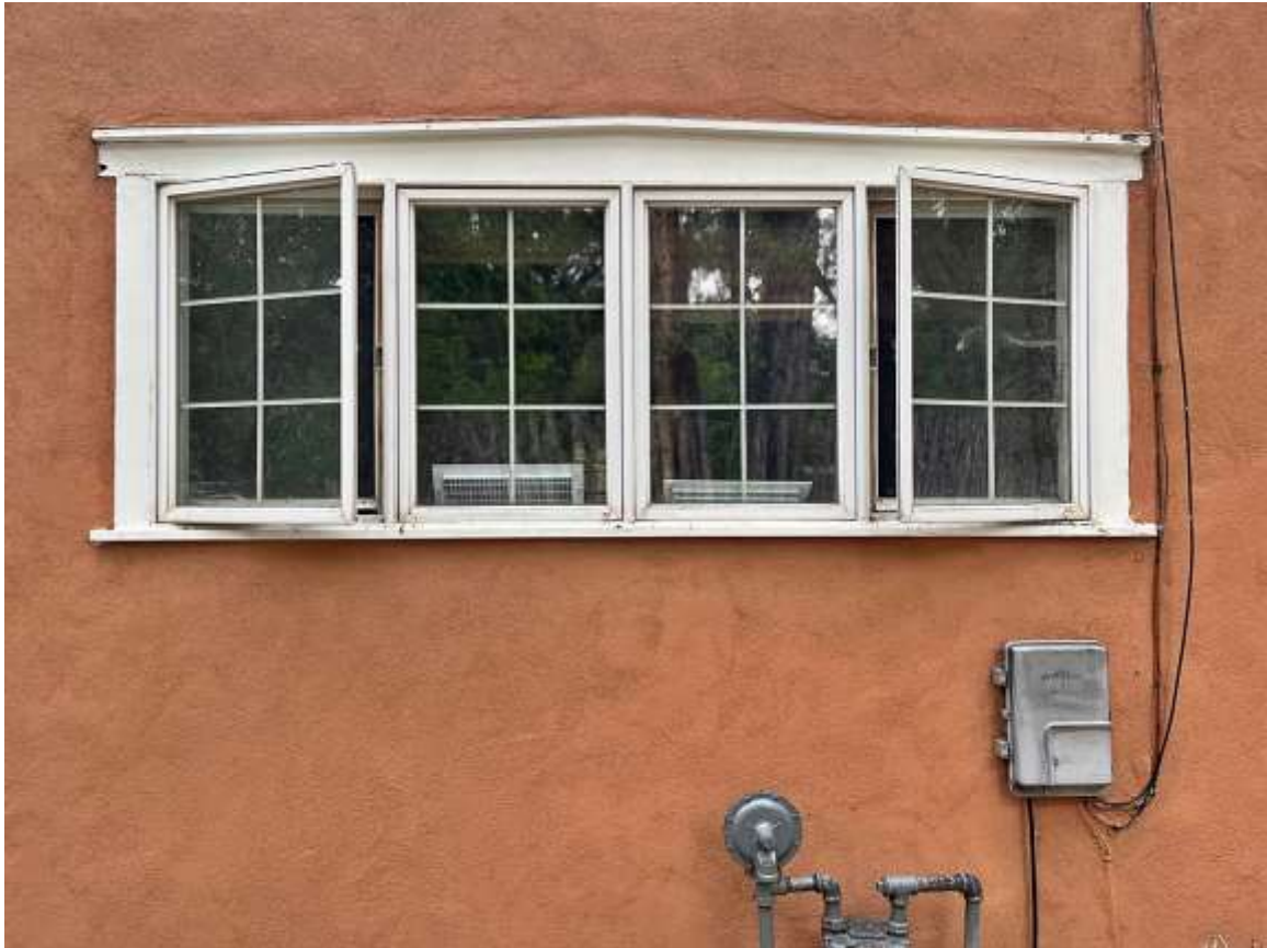
Photo 8: East elevation, casement windows. Camera facing west.
