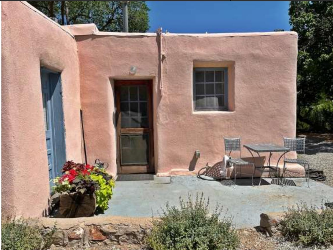
Photo 9: South elevation, assumed core block. Camera facing north.
