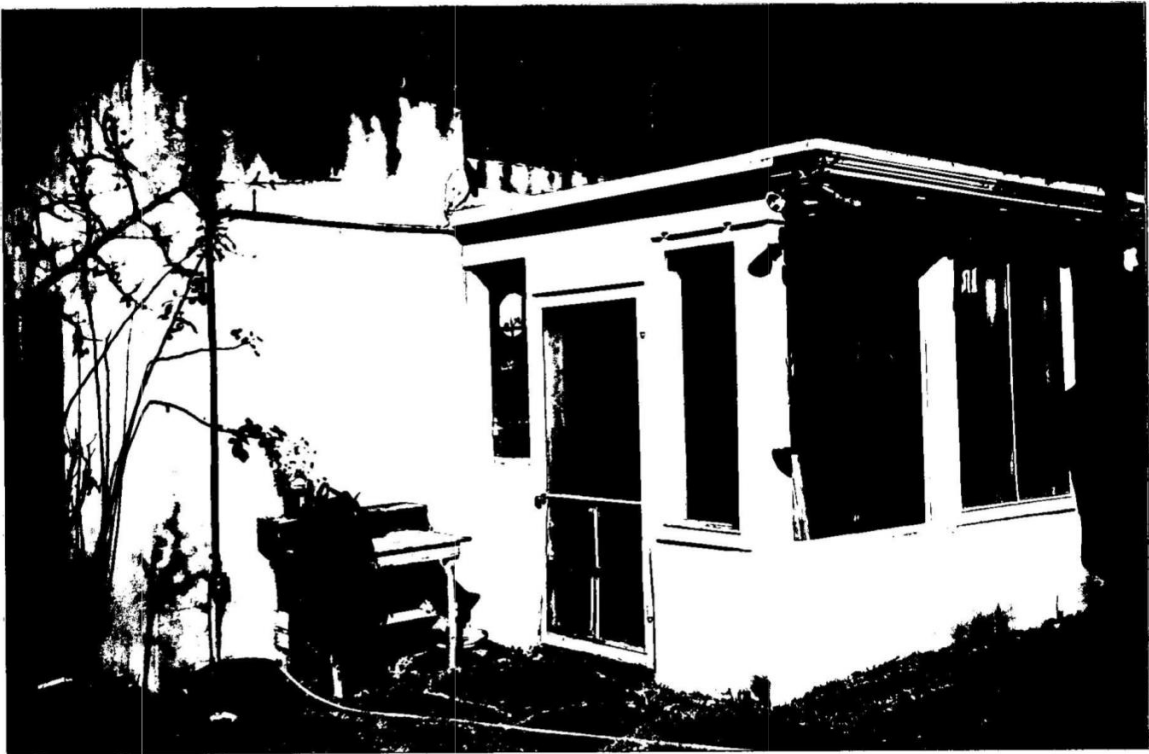
South elevation, west end
