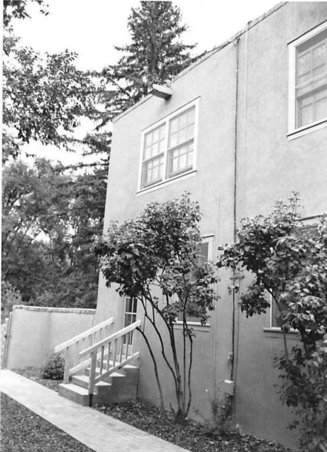
#6 north part of west elevation
