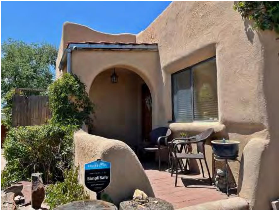
Photo 4: East façade, entry porch. Camera facing southwest. Note exaggerated window reveals and sill. Compare to Figure 1.
