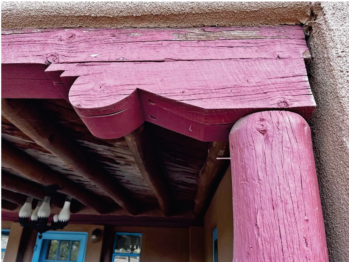
Photo 6: Porch corbel. Camera facing up. October 4, 2023, JWM.
