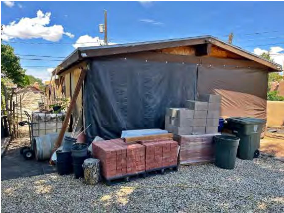
Photo 11: Carport, front (east) elevation. Camera facing northwest.
