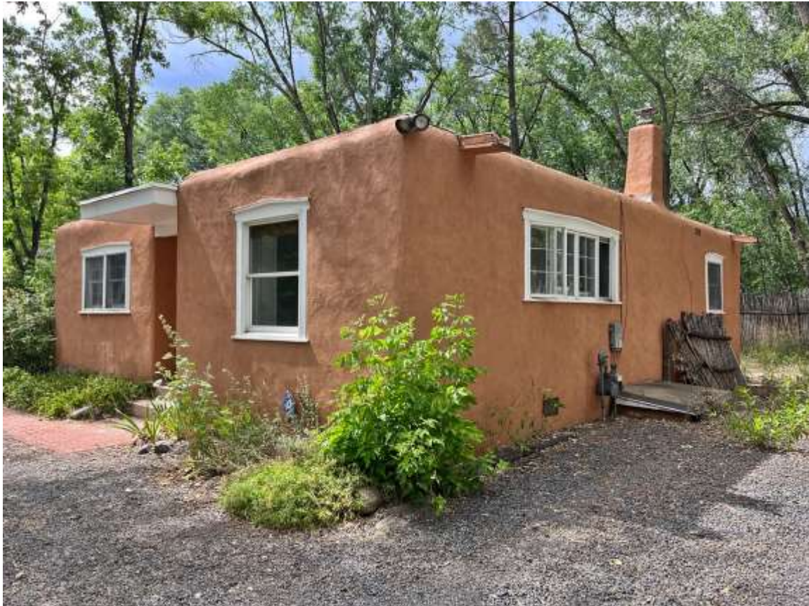
Photo 7: South and east elevations. Camera facing northwest.
