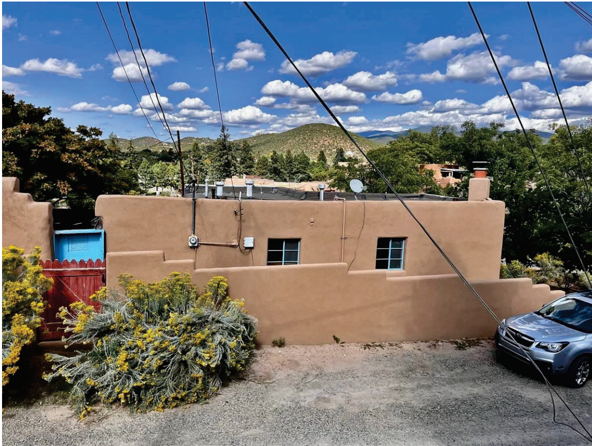
Photo 12: South elevation. Camera facing northeast. October 4, 2023, JWM.
