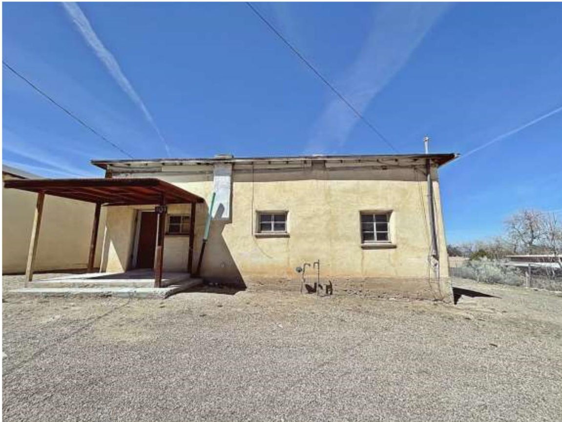
Photo 3: East elevation, camera facing west.
