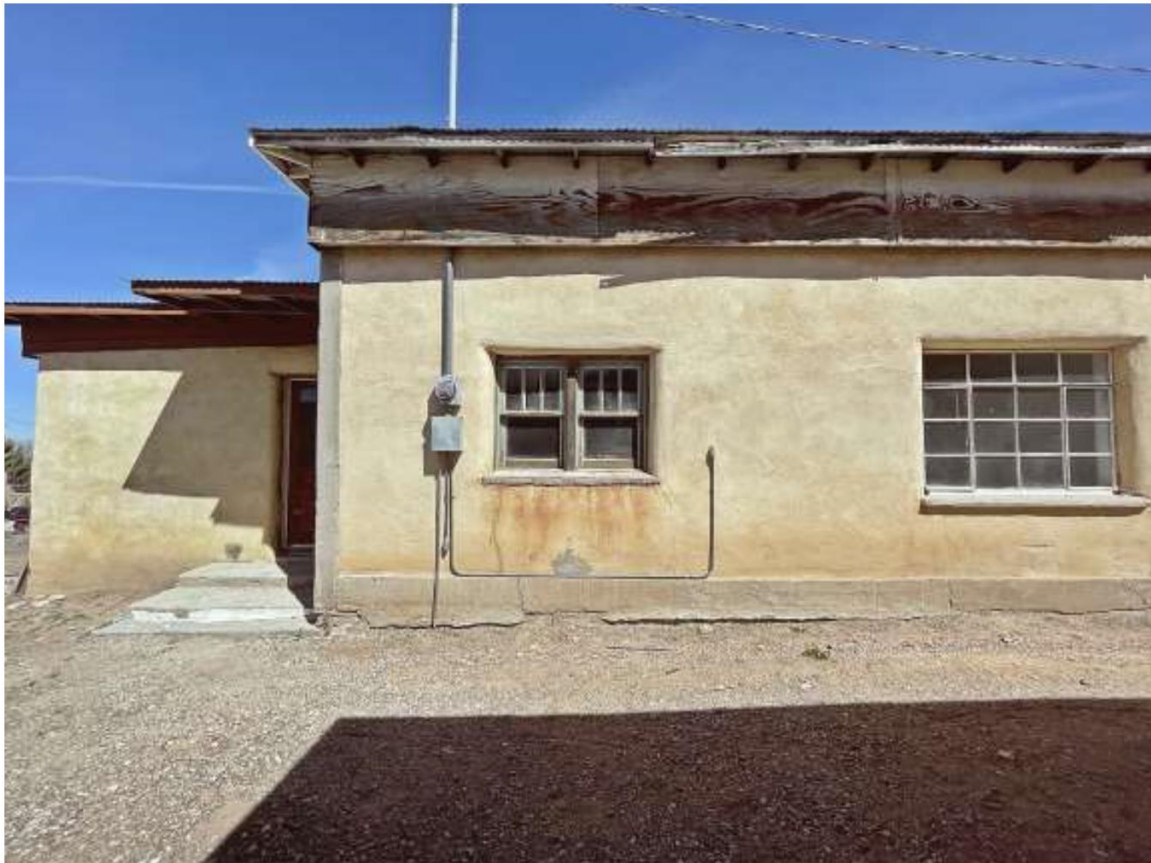
Photo 5: West end of south elevation; addition at left. Camera facing north.
