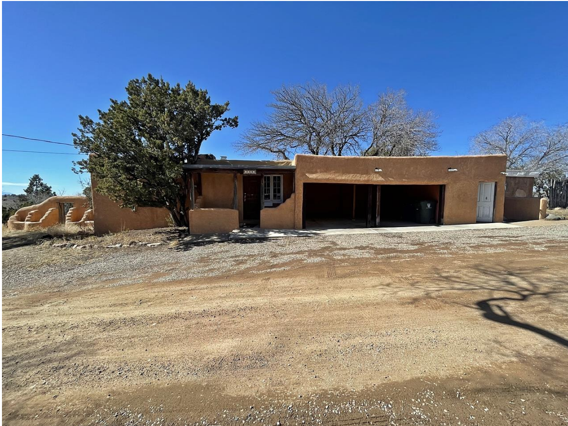
Photo 12: East elevation: older core (left), garage (right). Camera facing west.
