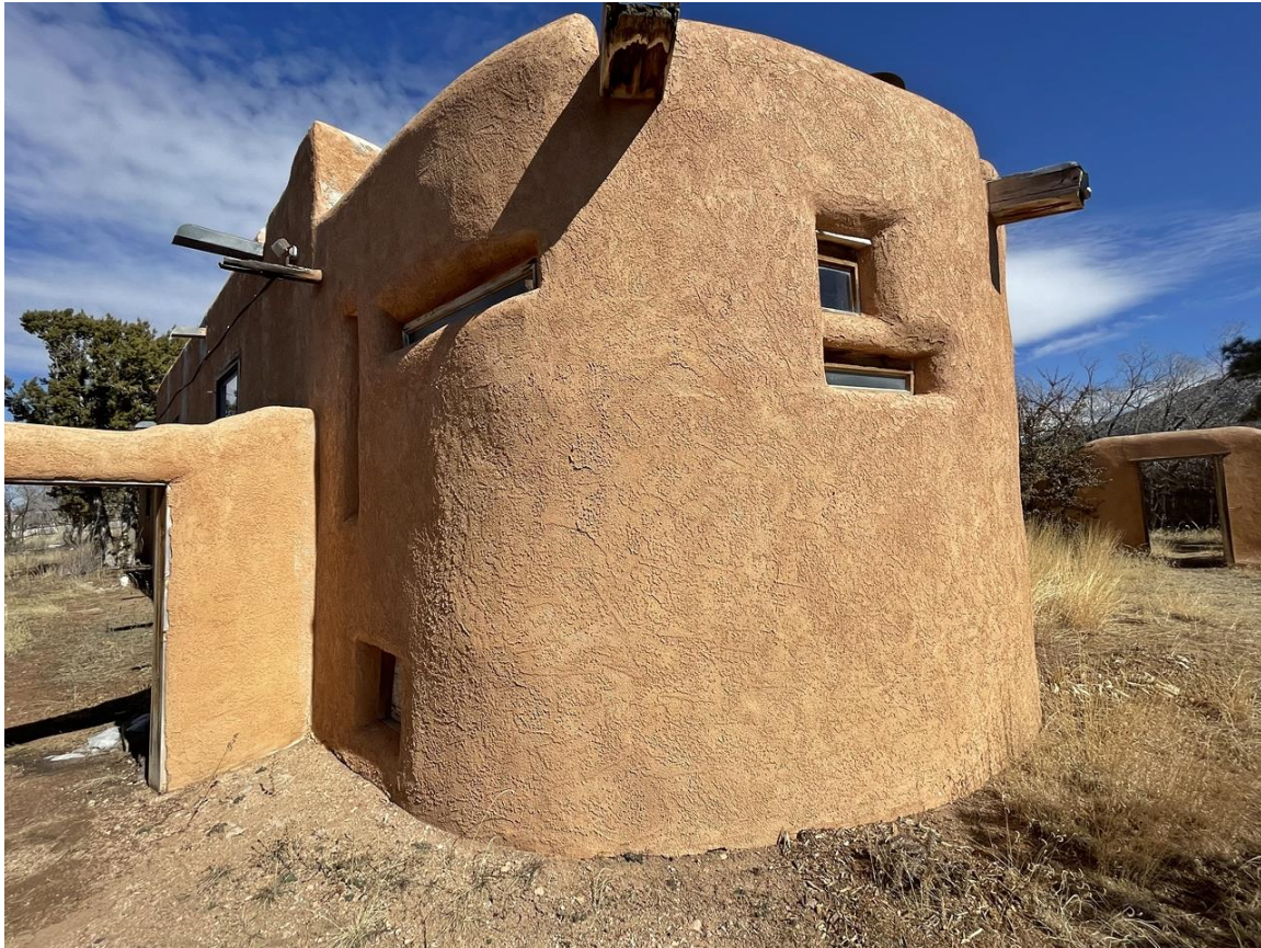
Photo 4: Sewing Room. Camera facing northeast.
