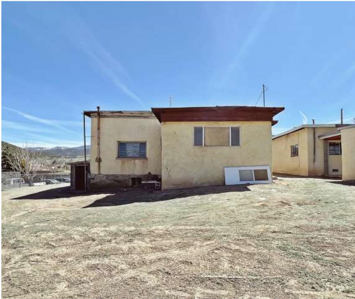
Photo 6: West elevation. Camera facing east.
