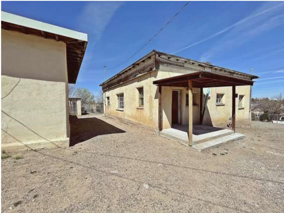
Photo 4: South elevation. Camera facing northwest.
