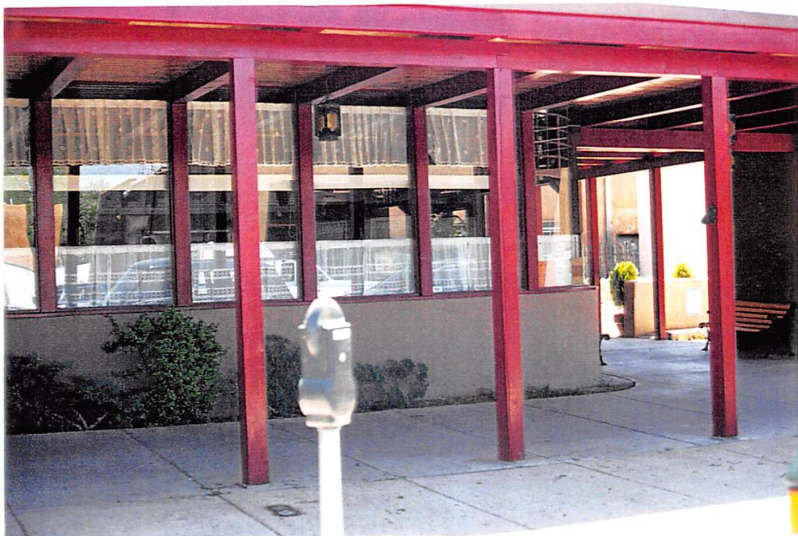
Another view of the area where the planter wall would be installed.
