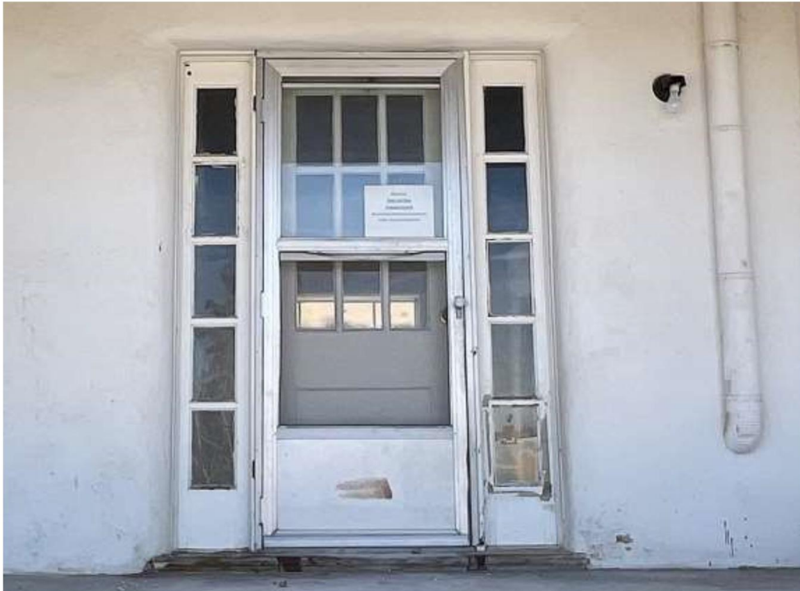
Photo 9: North elevation. Front entry door. Camera facing east.
