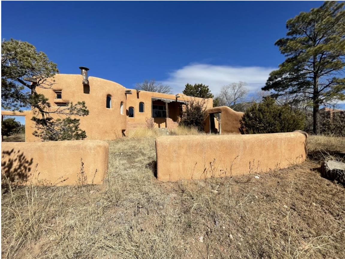
Photo 19: Perimeter wall. Camera facing northeast.
