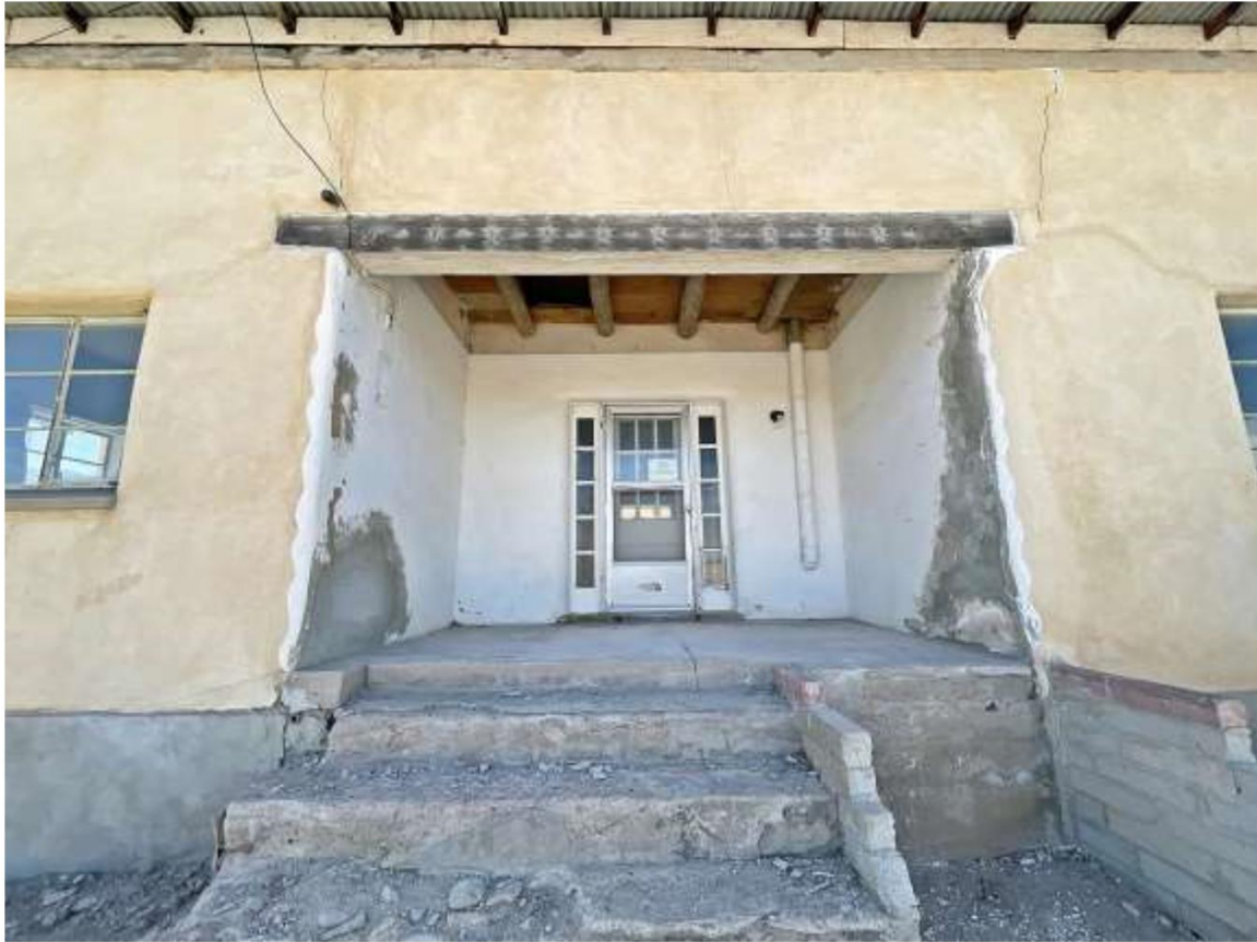
Photo 8: North elevation. Porch. Camera facing up.
