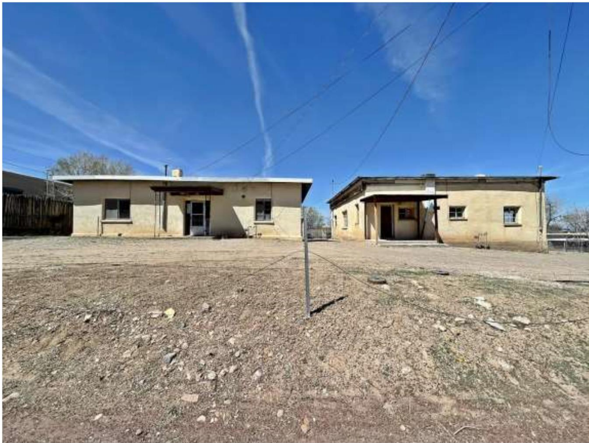
Photo 2: 406 (left) and 404 (right). Camera facing northwest.
