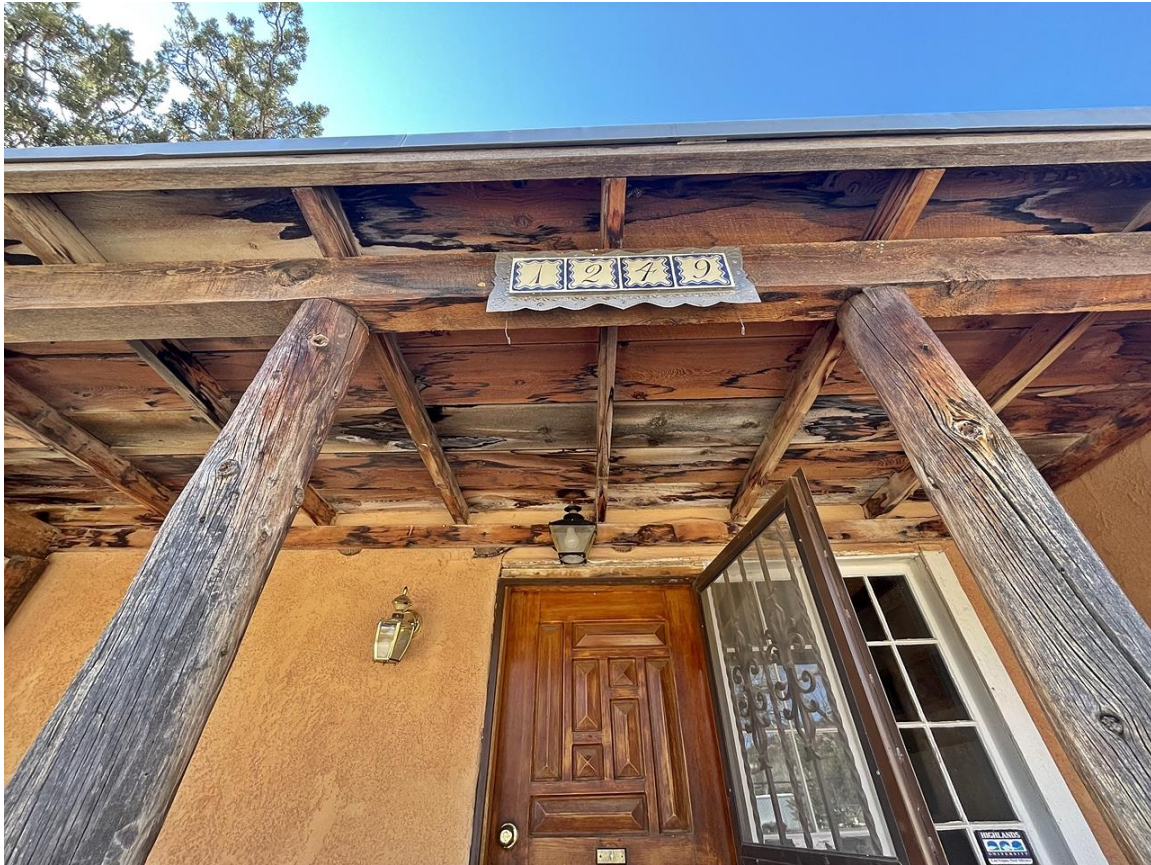
Photo 13: East elevation, introduced portal at older core. Camera facing up.
