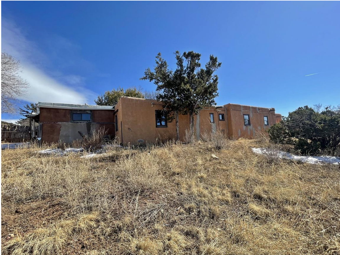
Photo 6: West elevation. Camera facing southeast.
