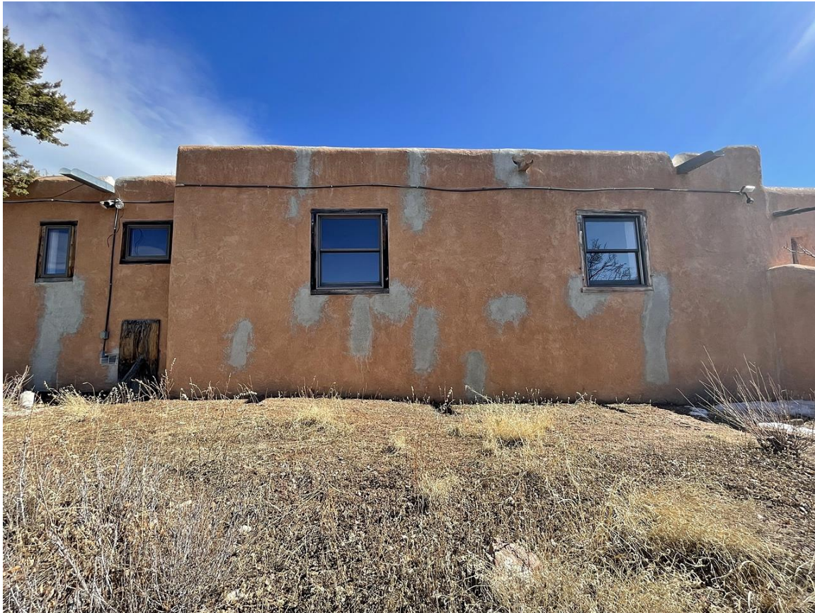
Photo 7: South half of west elevation. Camera facing east.
