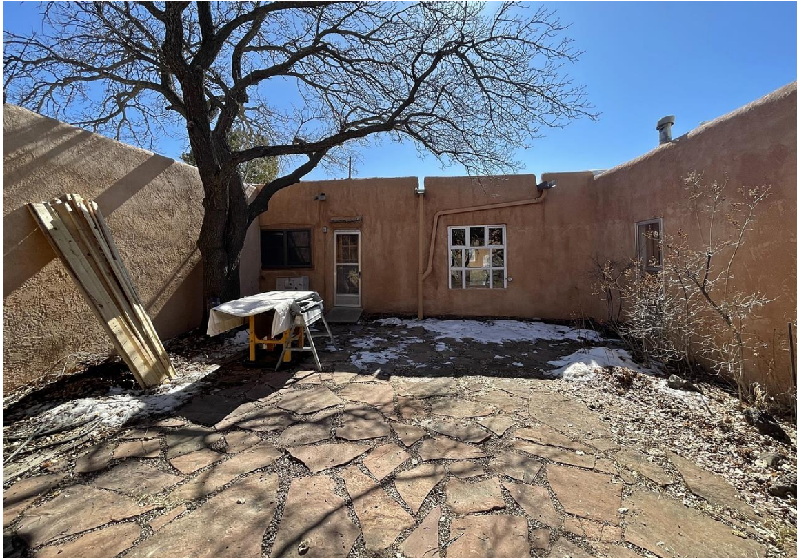
Photo 17: Courtyard, older core at center. Camera facing south.
