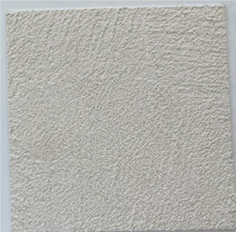
EXTERIOR STUCCO COLOR UNDER PORTAL AREA AT 213 WASHINGTON AVENUE
