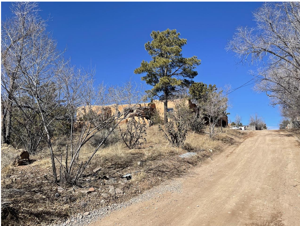
Photo 2: Approaching property from dirt road. Camera facing northwest.
