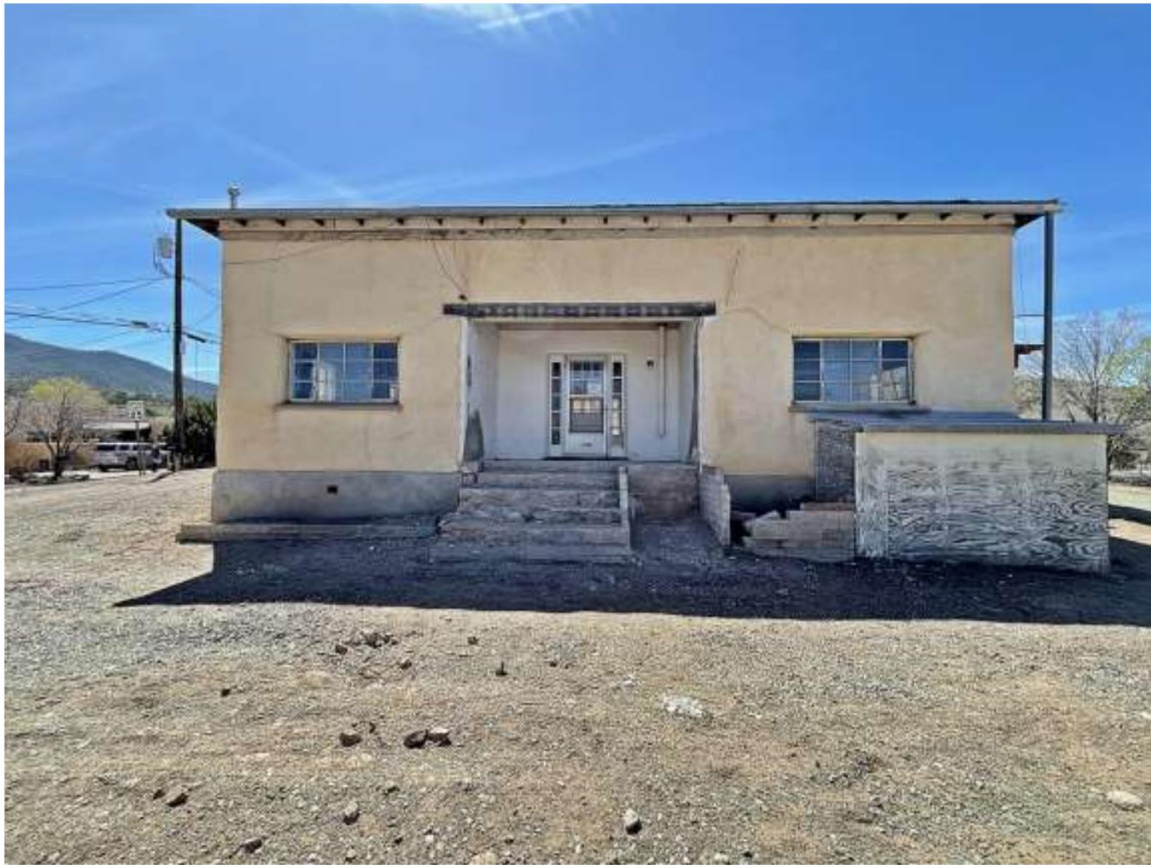
Photo 7: North elevation. Camera facing south.
