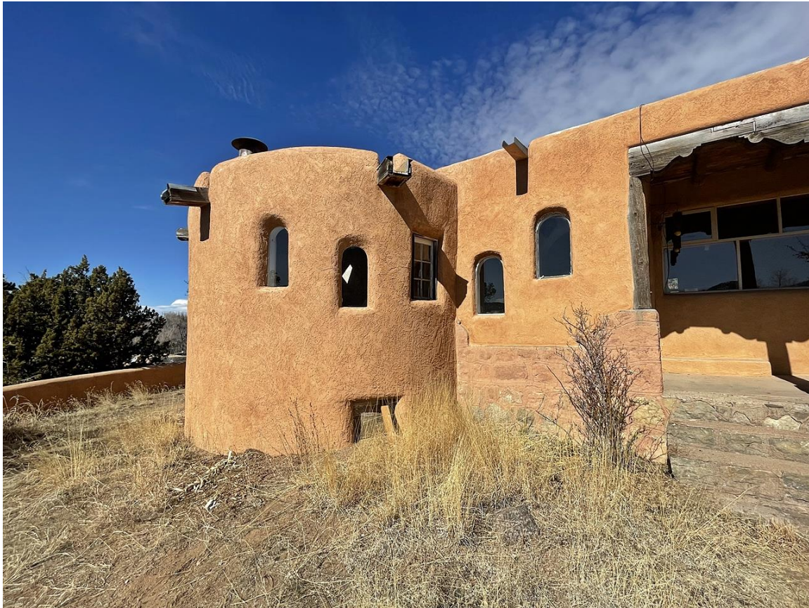
Photo 5: Partial south elevation with porch addition. Camera facing northwest.
