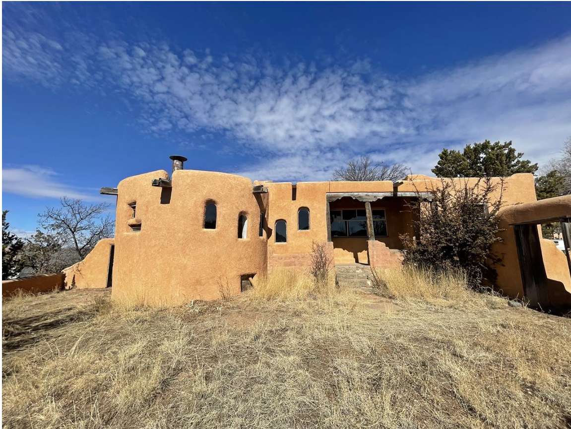
Photo 3: South elevation with Sewing Room and porch addition. Camera facing north.
