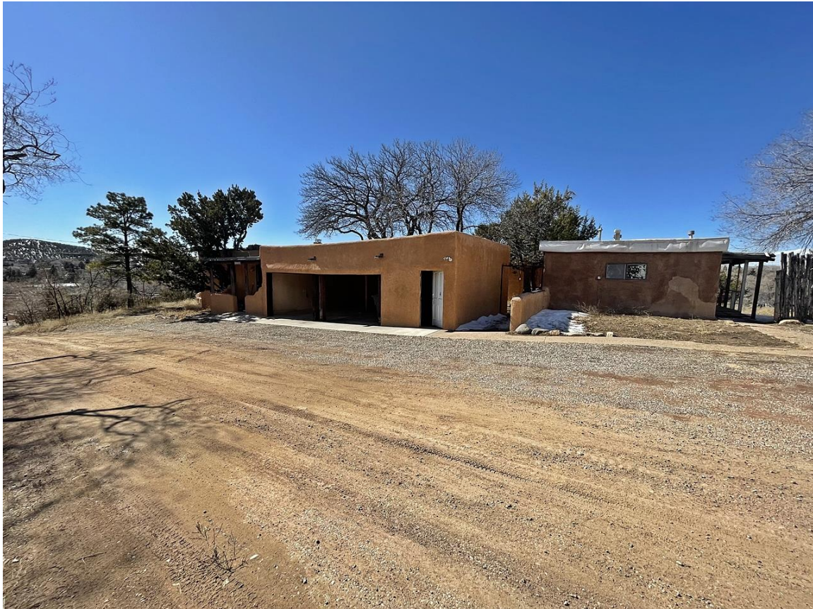
Photo 11: East elevation. Camera facing southwest.
