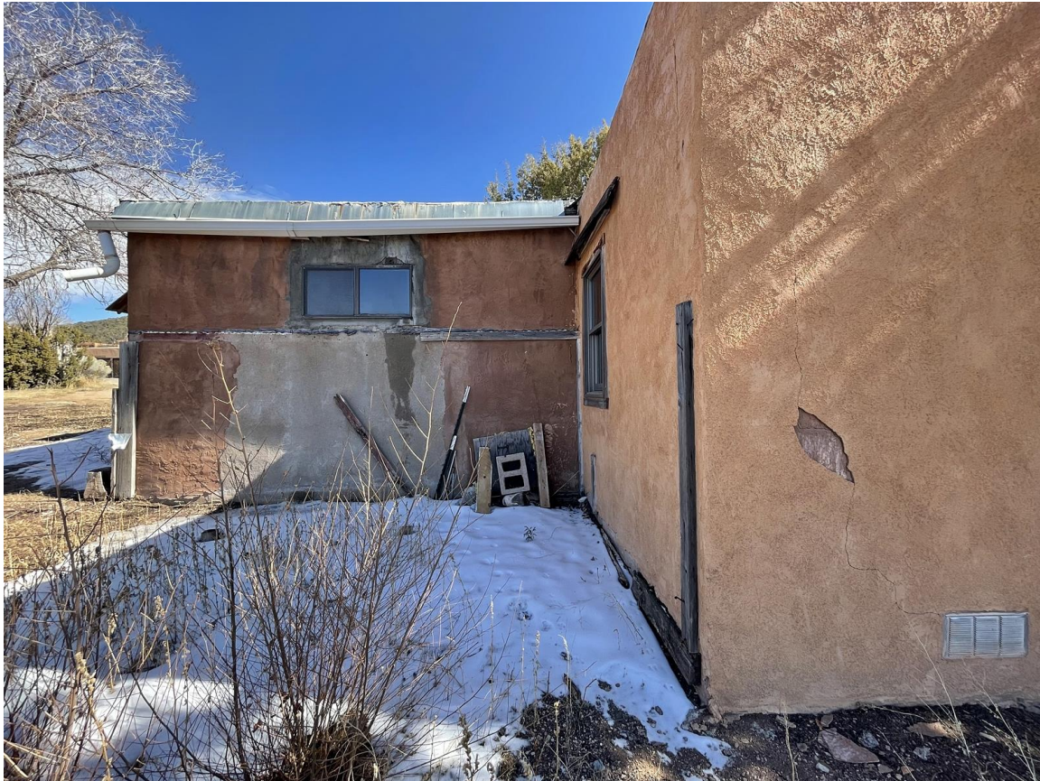
Photo 9: Joining of west wing and apartment/utility room. Camera facing east.
