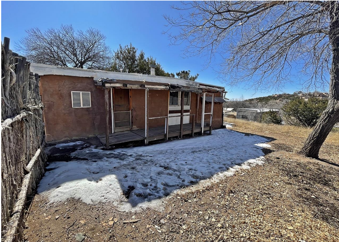
Photo 10: Apartment/utility room, north elevation. Camera facing southwest.
