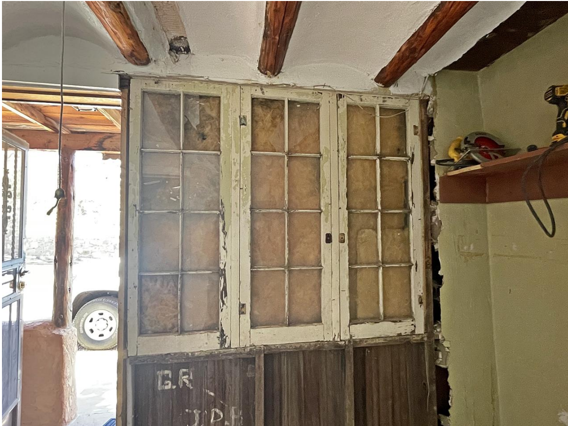
Photo 14: East elevation, older core interior, original enclosed porch. Camera facing northeast.
