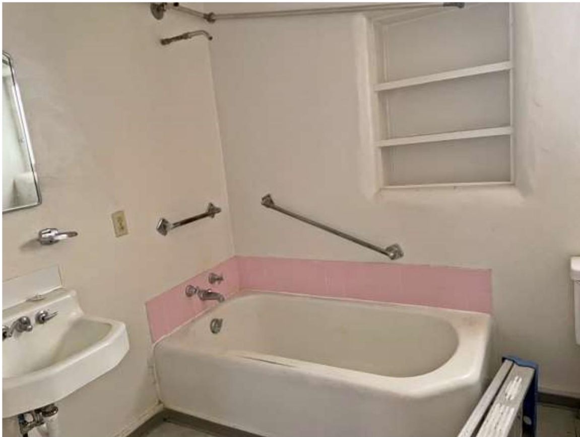
Photo 11: Main bathroom. Fixtures. Richard Van Sickle. April 2023.
