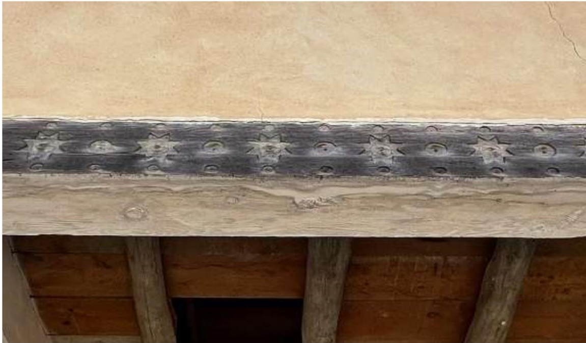
Photo 10: North elevation. Beam above entry vestibule. Camera facing up.
