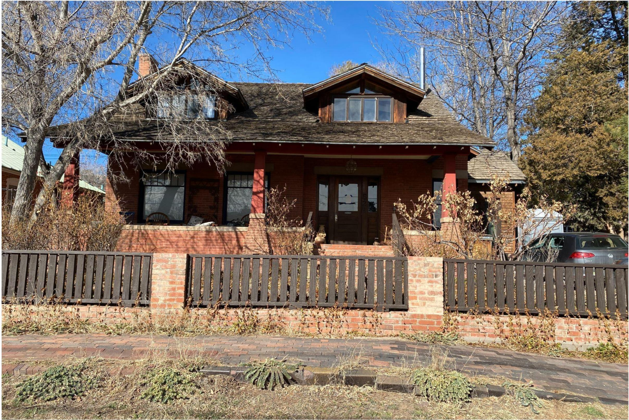
529 E. Palace Ave - South Facade
