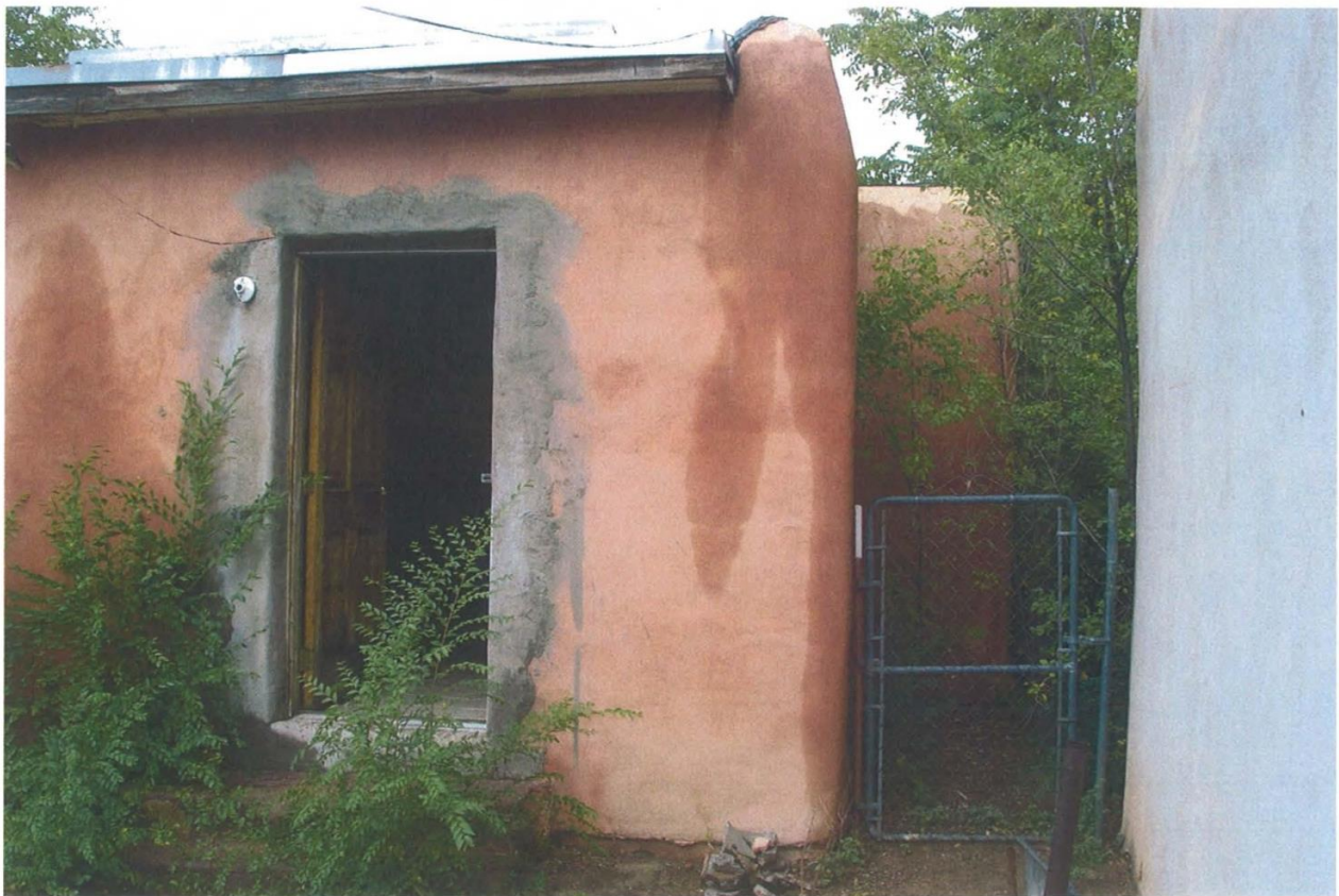
South Elevation with portion of East Facade
