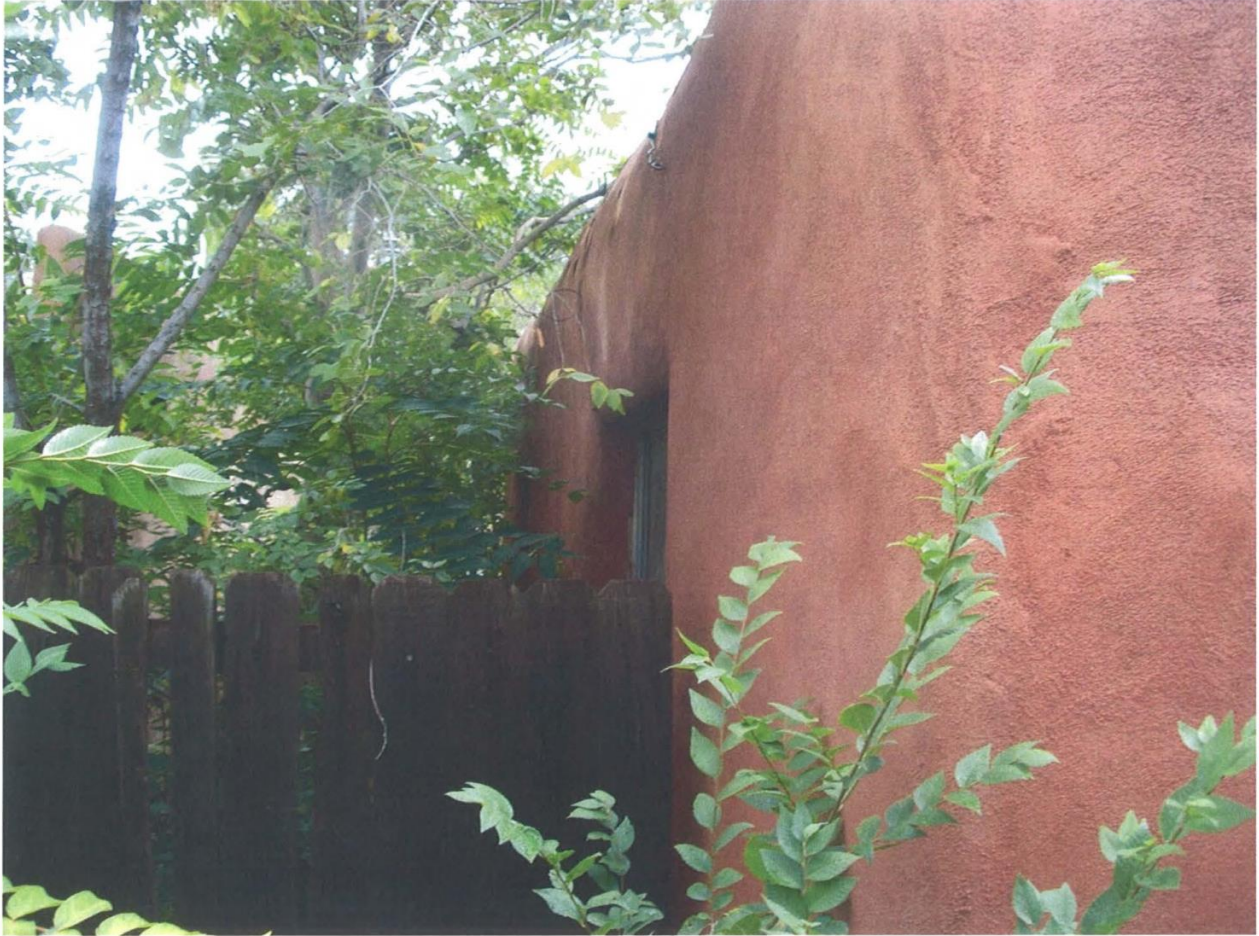
portion of East Façade from NE Corner
