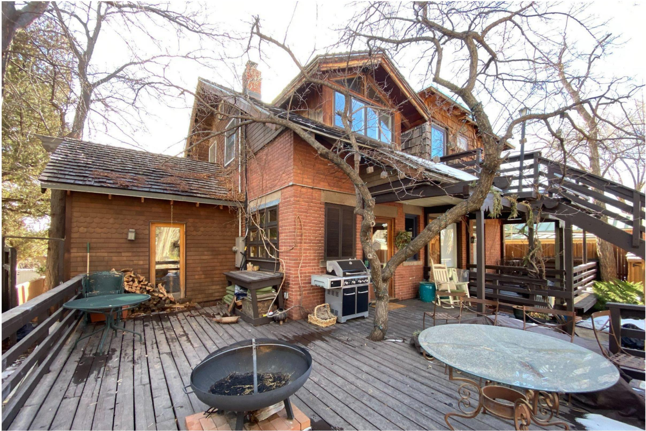
529 E. Palace Ave - North East Facade
