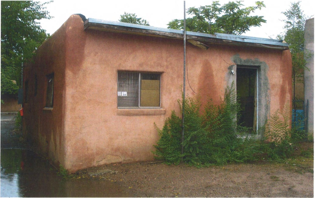
Rear South Elevation with West Elevation
