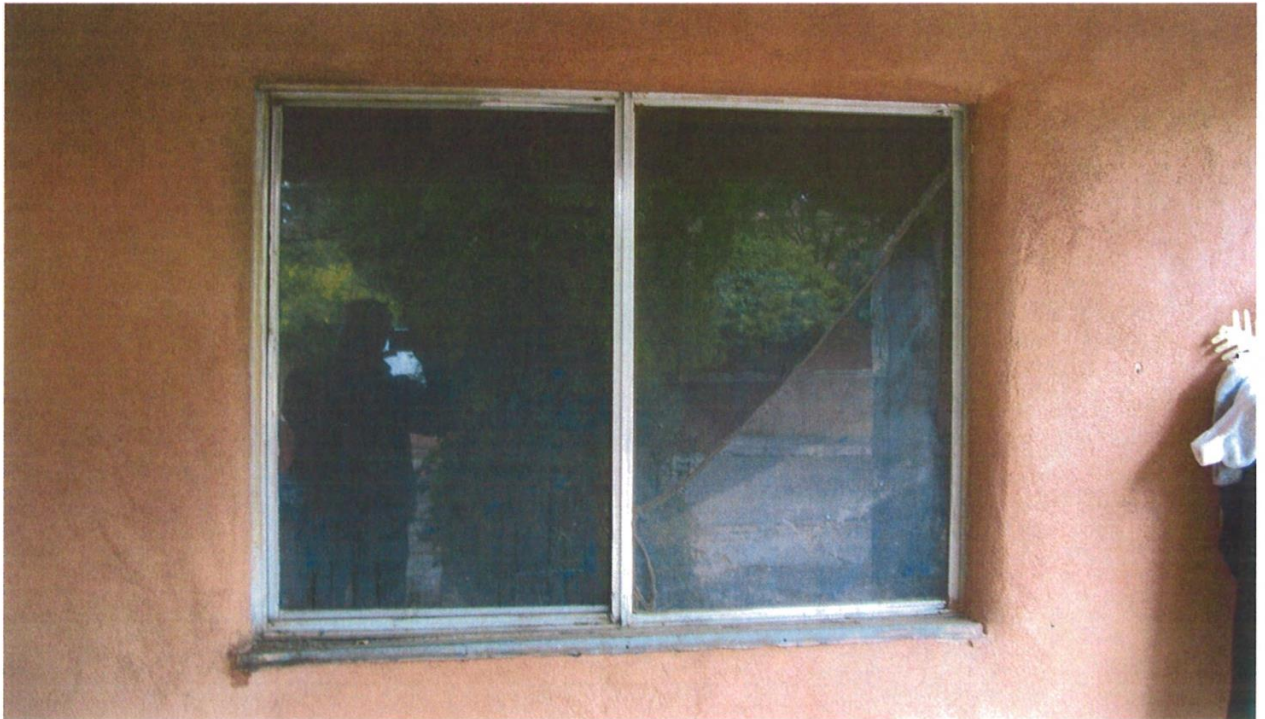
North Elevation Window under Porch
