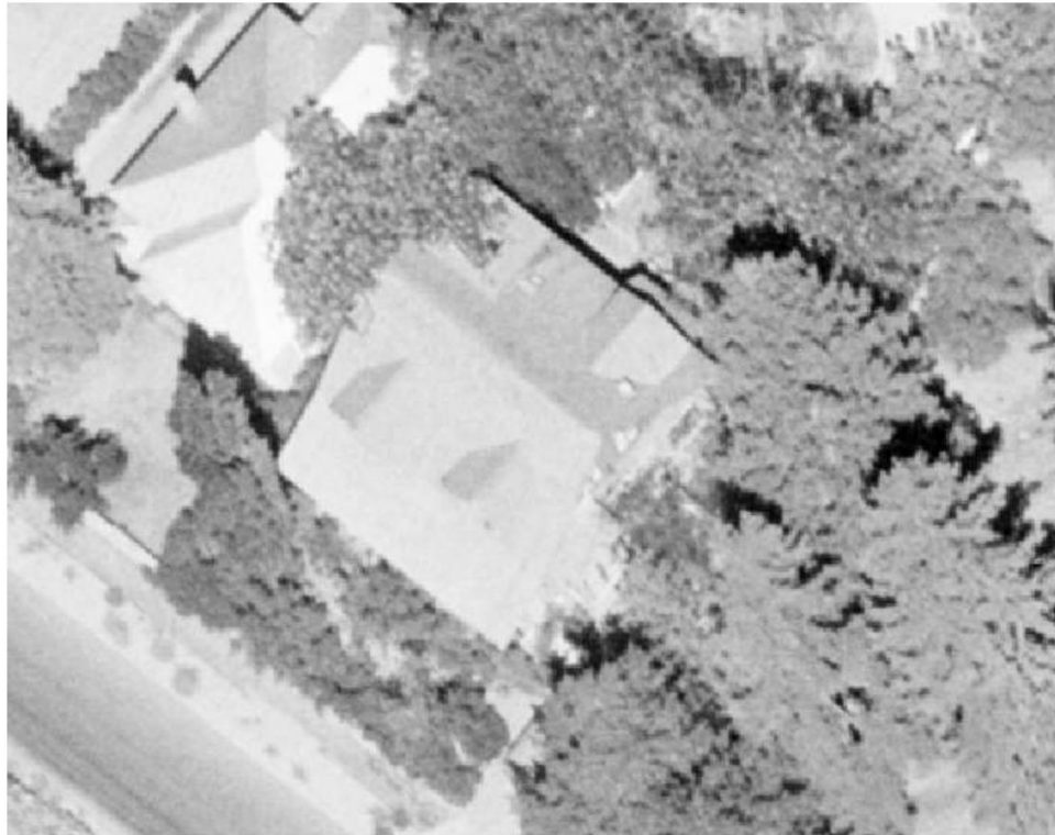
Figure 5: September 11, 1978, aerial photograph. Note there are the dormers and the east, west, and north additions.
