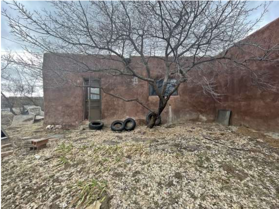
Photo 6: East elevation. Camera facing southwest.
