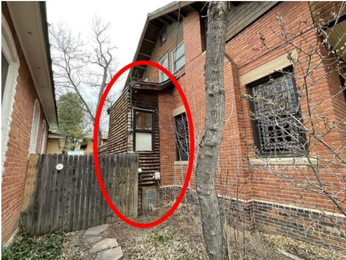
Photo 13: West elevation with 1970s addition circled. Camera facing northeast.
