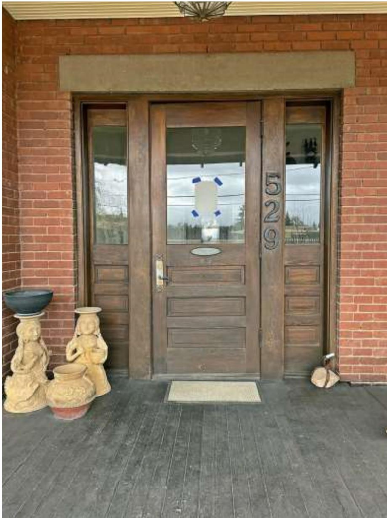
Photo 4: Entry door at porch. Camera facing north.
