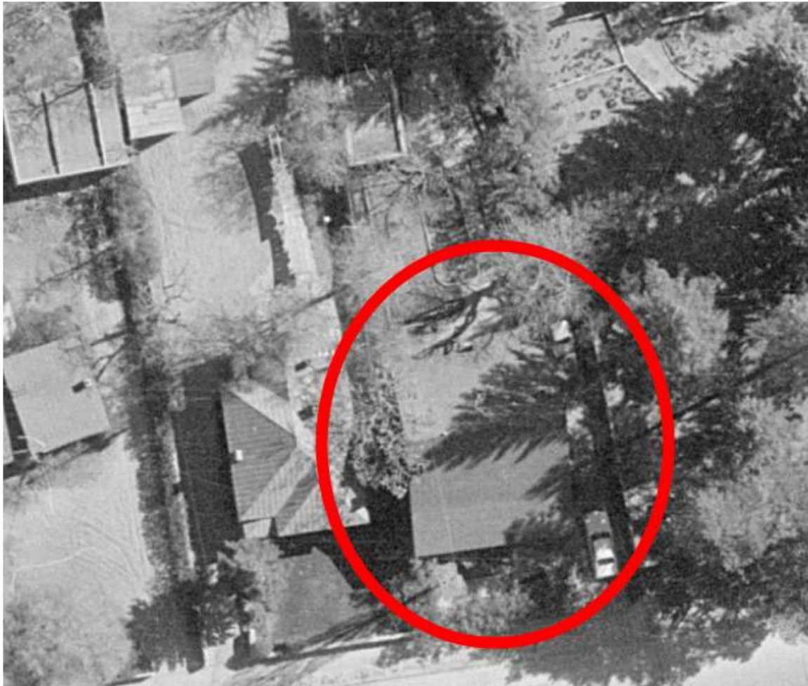
Figure 4: May 1, 1973, aerial photograph. Note there are no dormers or east, west, and north additions.
