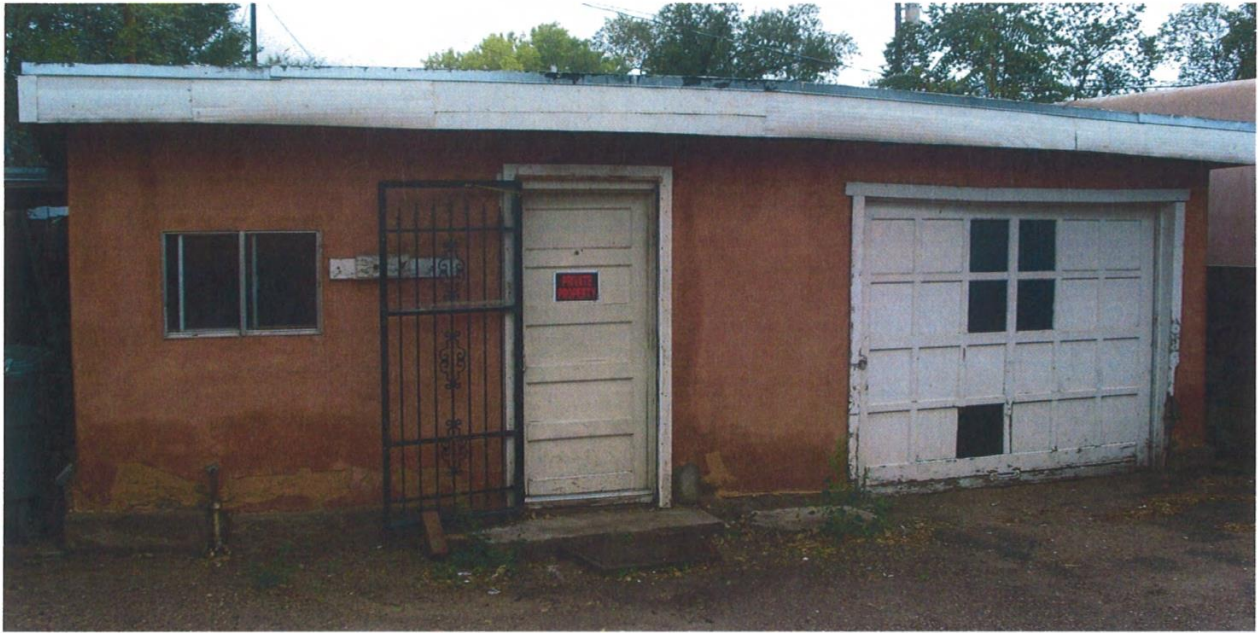
Rear Casita and Garage North Elevation
