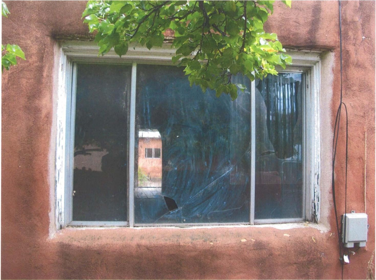
Front North Elevation Window
