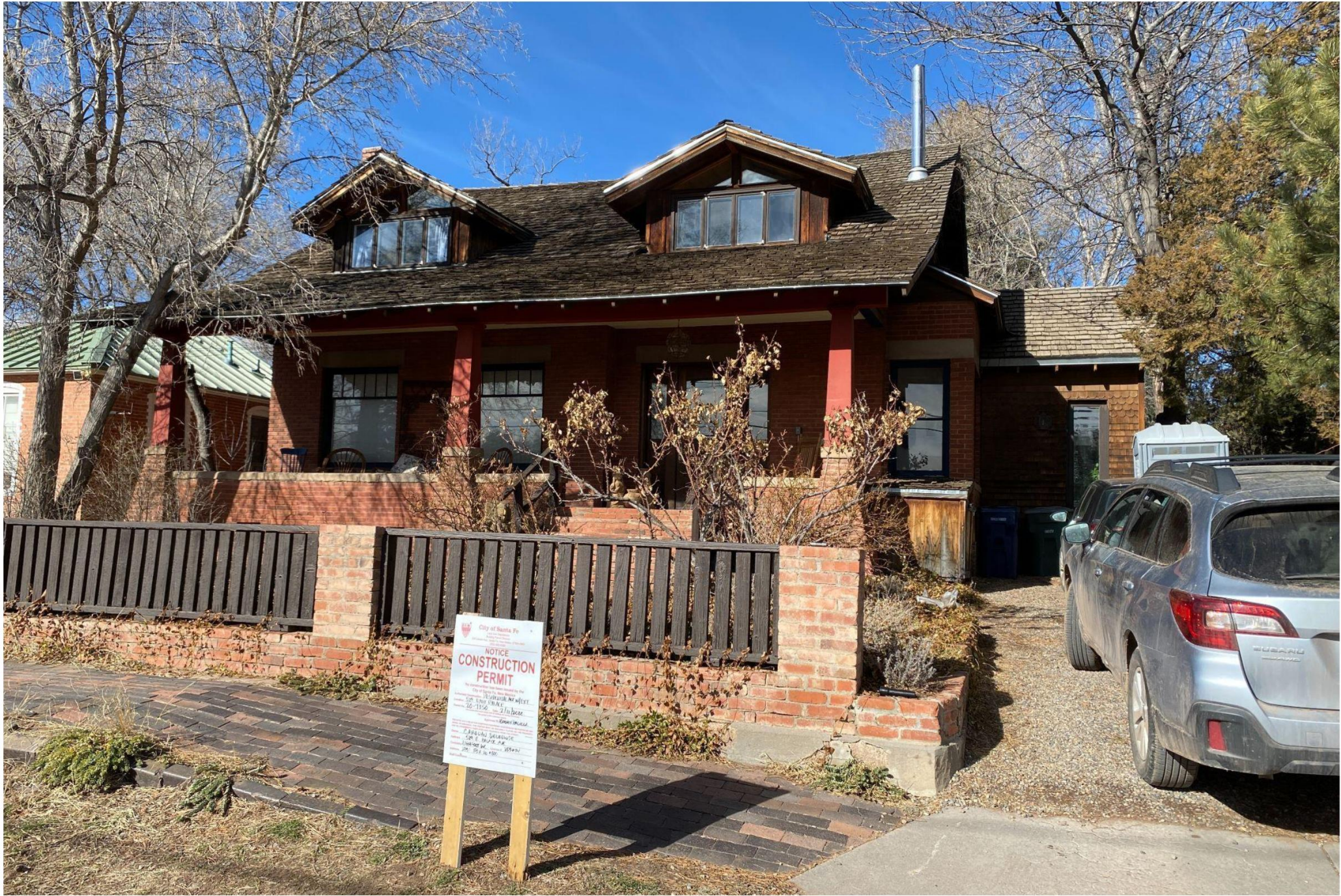
529 E. Palace Ave - South East Facade
