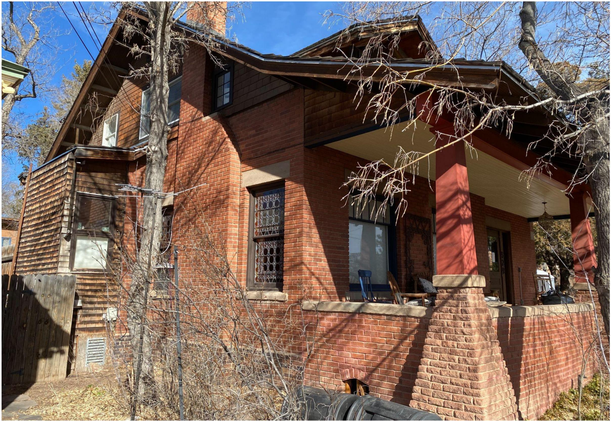
529 E. Palace Ave - South West Facade
