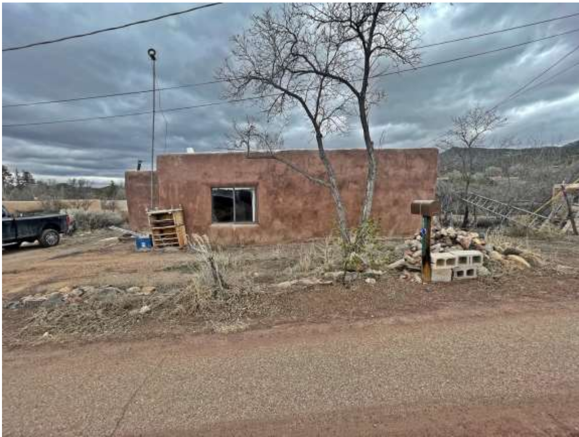
Photo 2: Façade taken from street centerline. Camera facing northeast.
