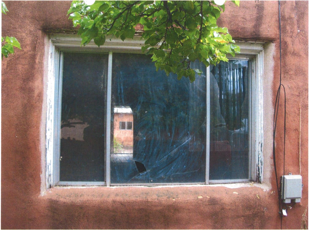
Front North Elevation Window
