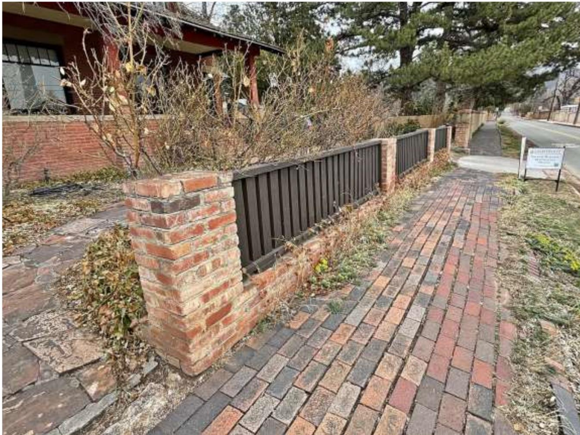
Photo 14: Front property fence. Camera facing east.
