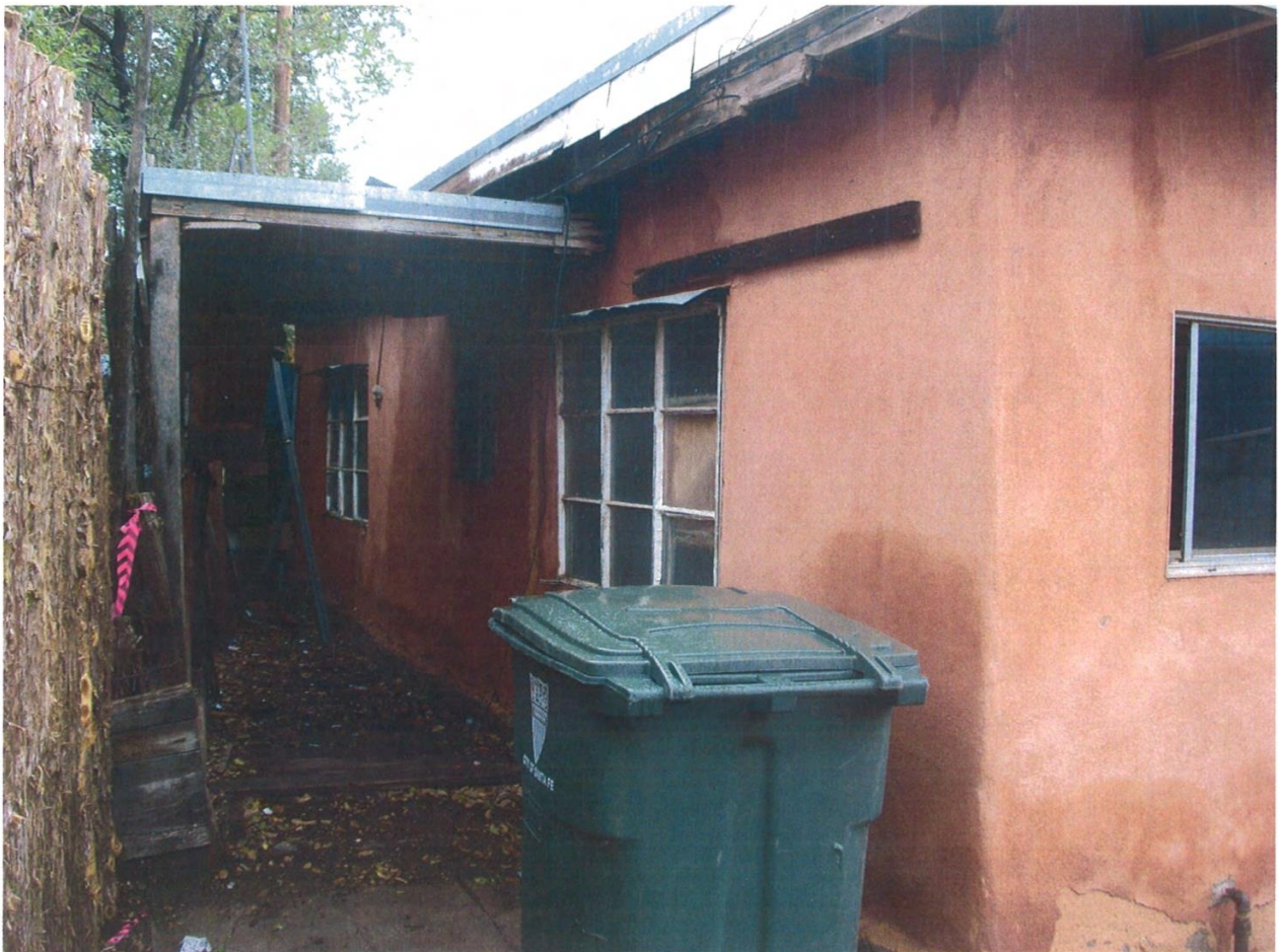
Rear Casita East Elevation
