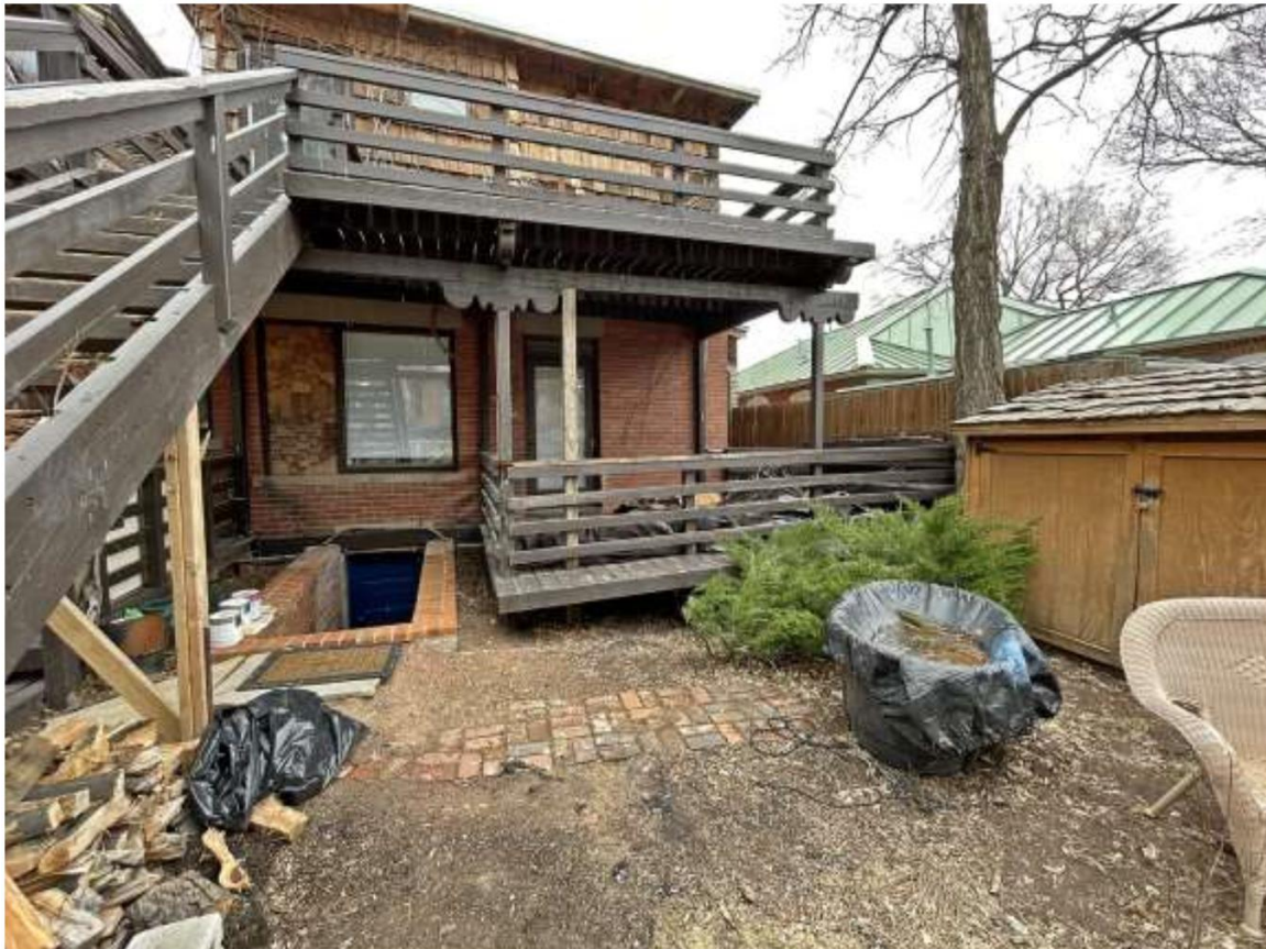
Photo 12: North elevation with altered fenestration at ground level. Camera facing southwest.
