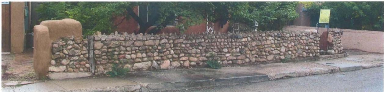
Yardwall North Elevation with Pedestrian Gate and NW Corner
