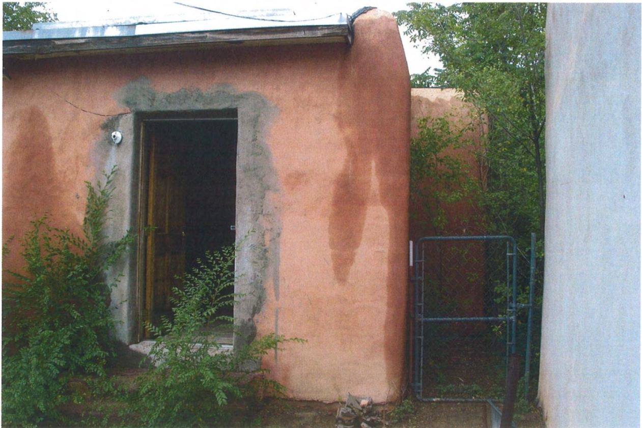
South Elevation with portion of East Facade
