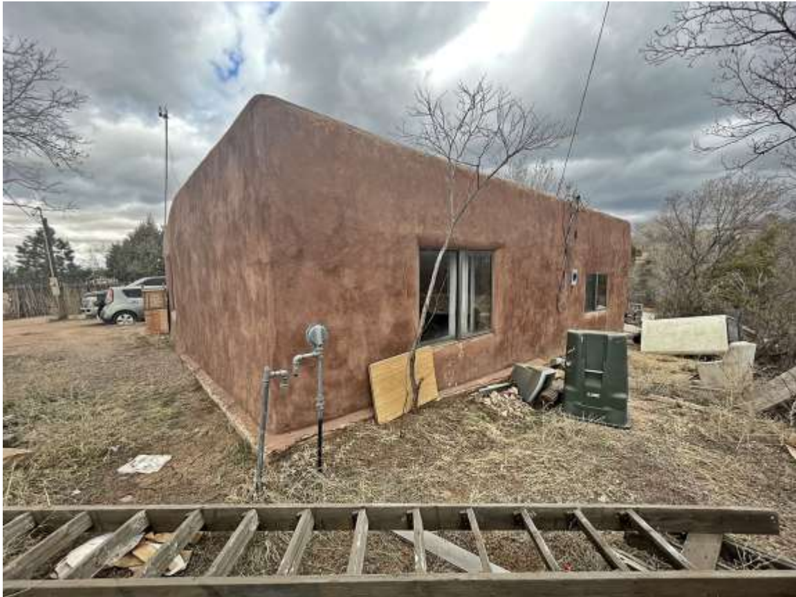
Photo 7: West and south elevations. Camera facing north.
