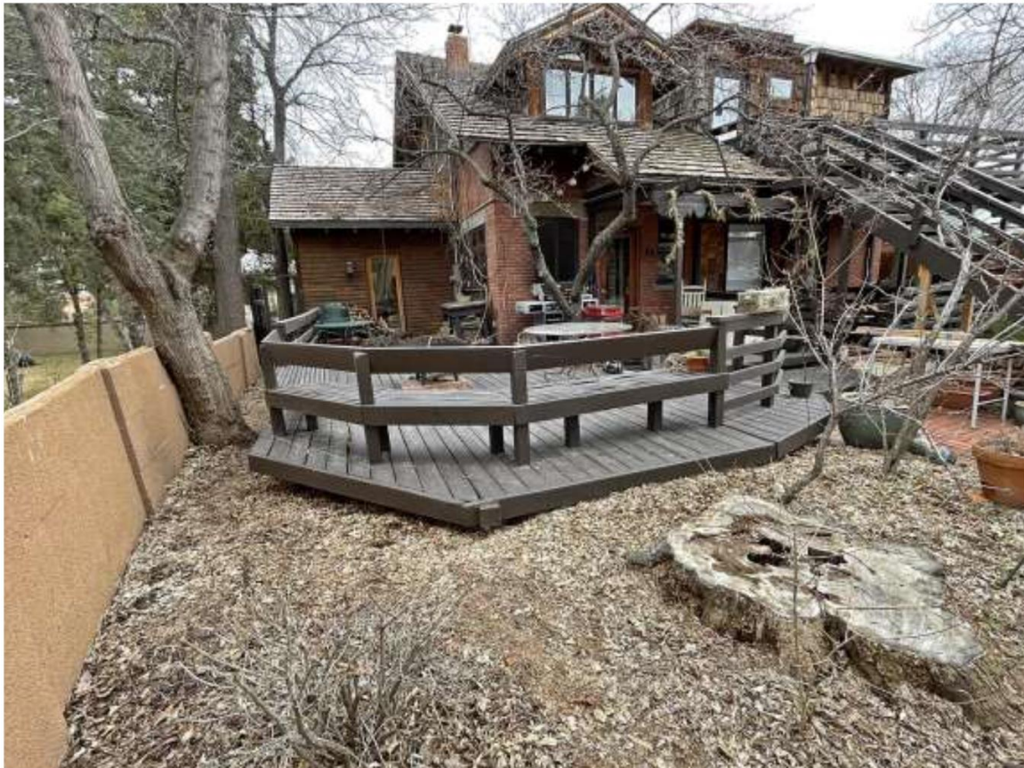
Photo 9: North elevation. Camera facing south.
