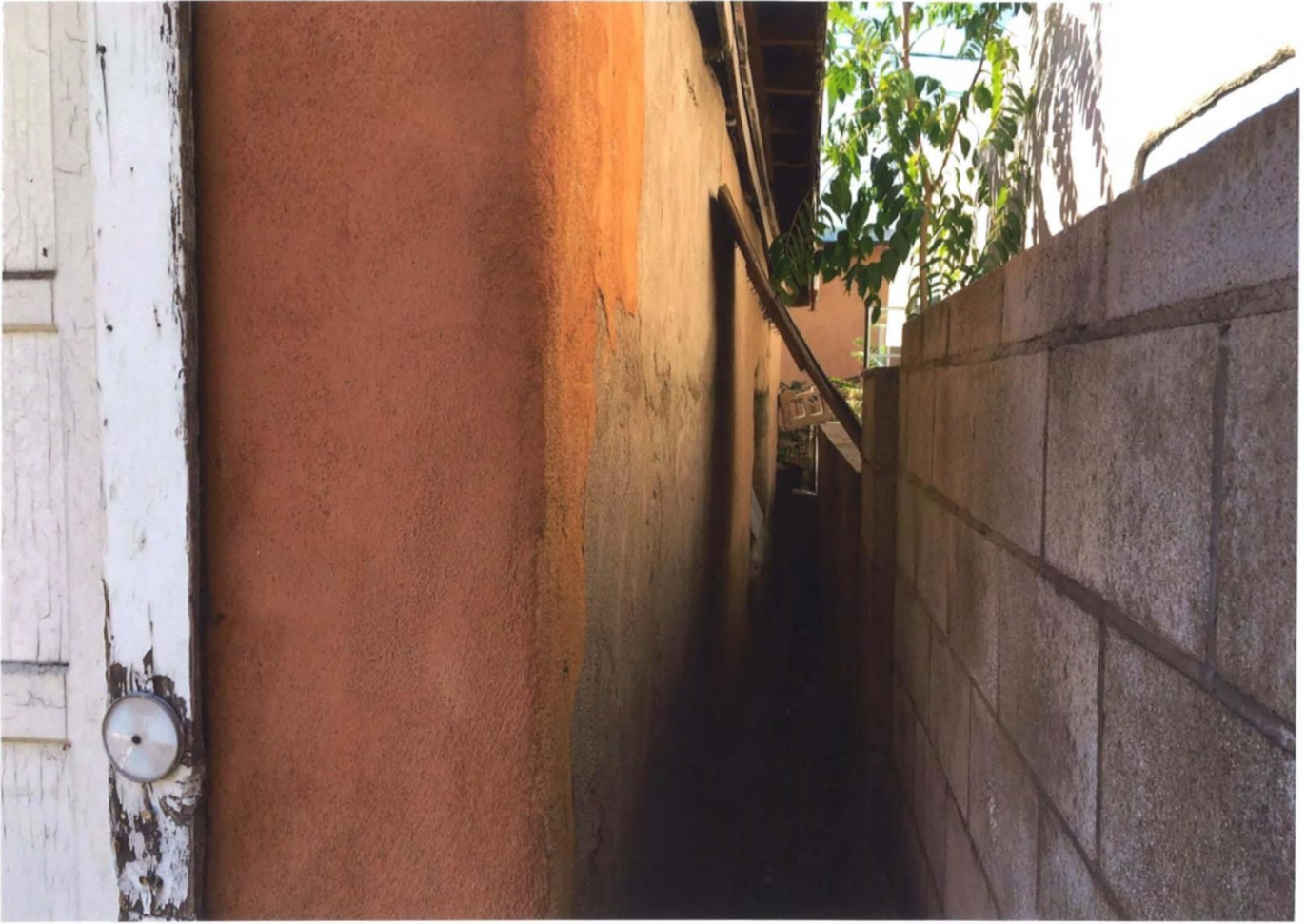
EAST SIDE OF GUEST HOUSE LOOKING AT IT
