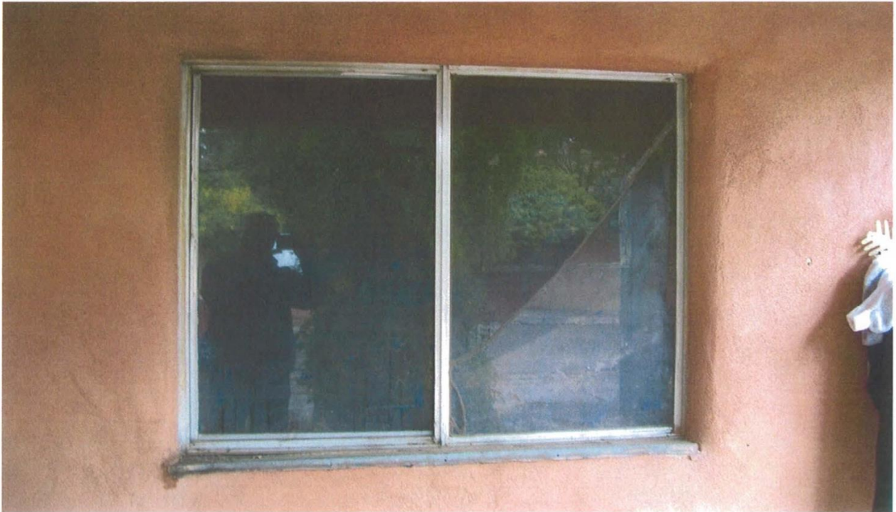
North Elevation Window under Porch
