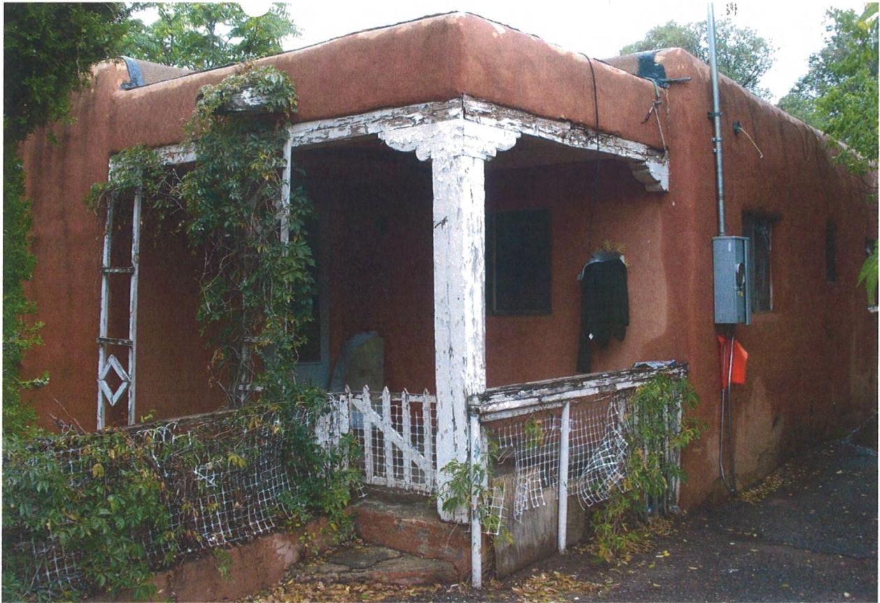
NW Corner Elevation
