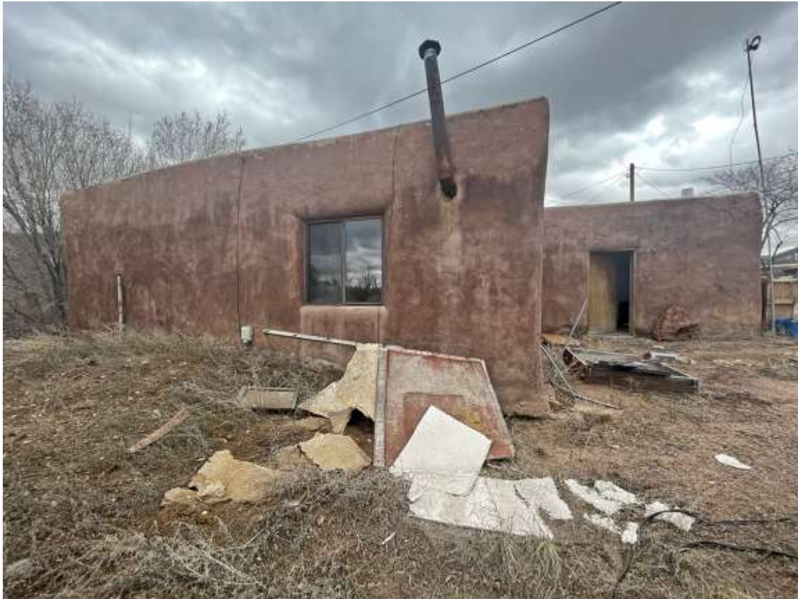
Photo 4: North elevation. Camera facing southeast.
