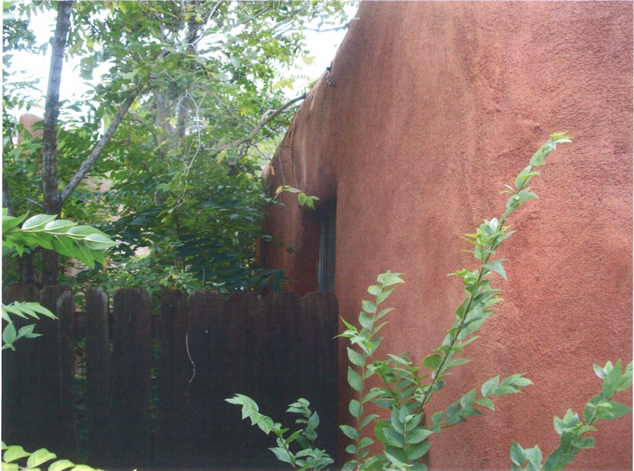
portion of East Façade from NE Corner
