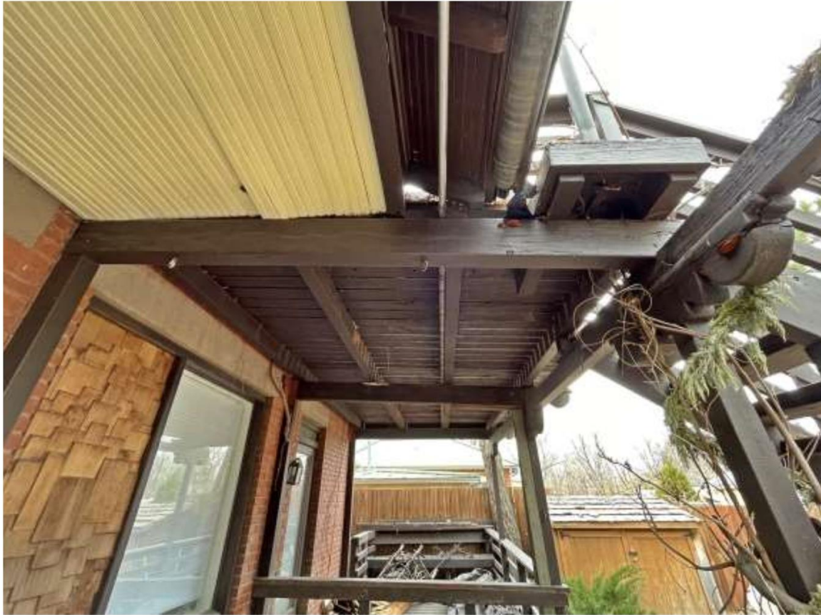
Photo 11: North elevation, porch decking. Camera facing west.
