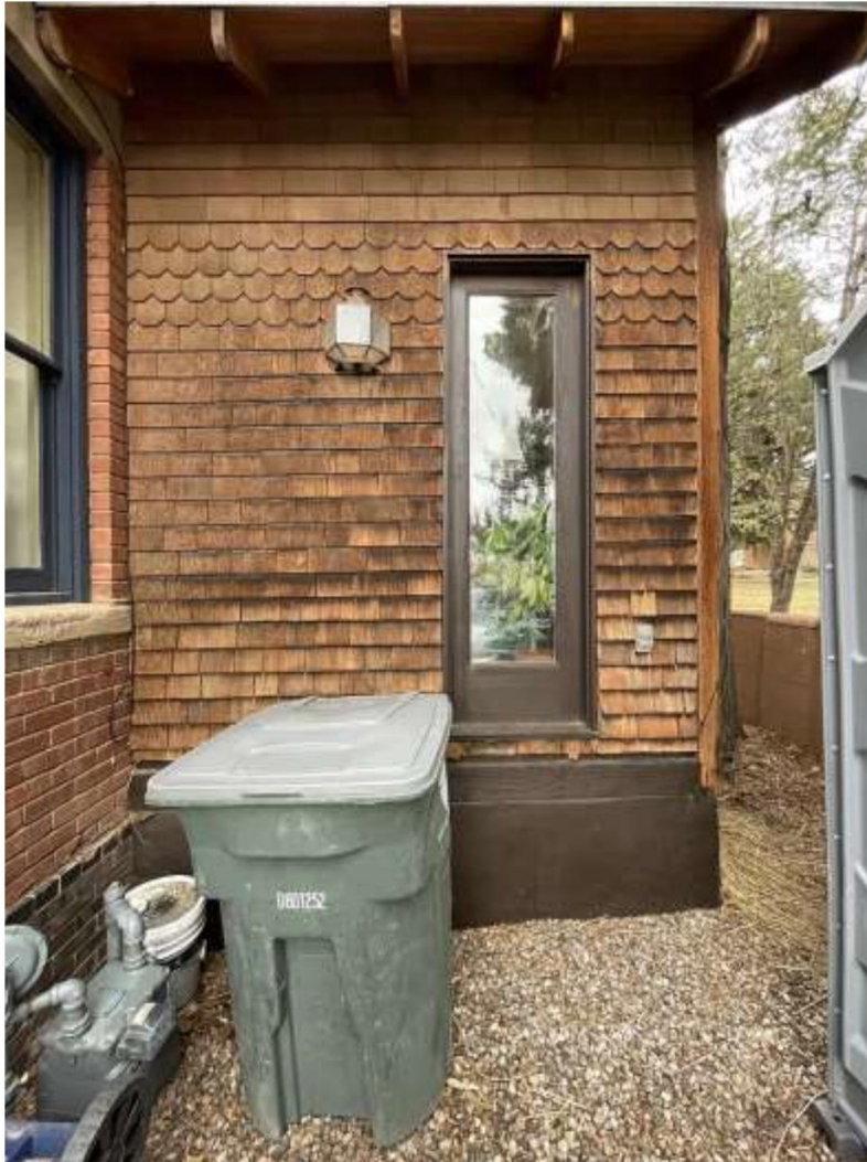
Photo 6: East addition, south elevation. Camera facing north.
