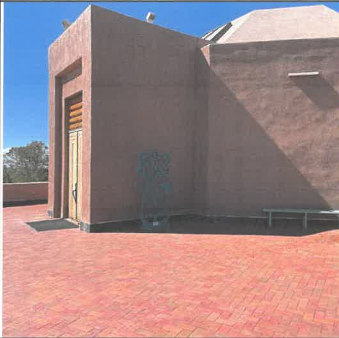
1a. This view shows the existing stucco condition.
