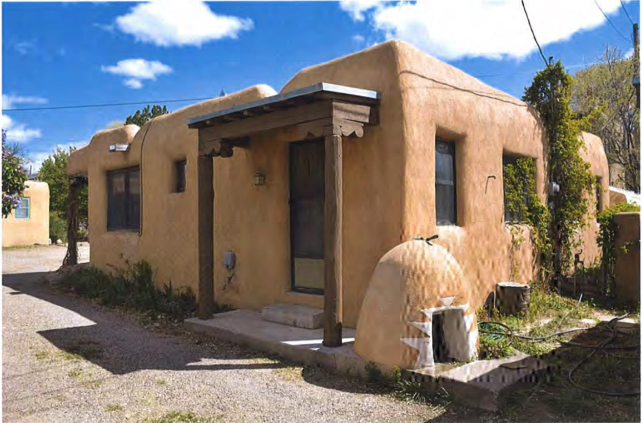
Photo 4: North and west elevations, facing southeast.
