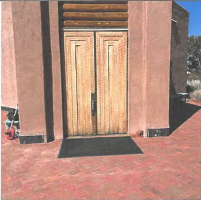
5a. This shows the existing wood entry door.
