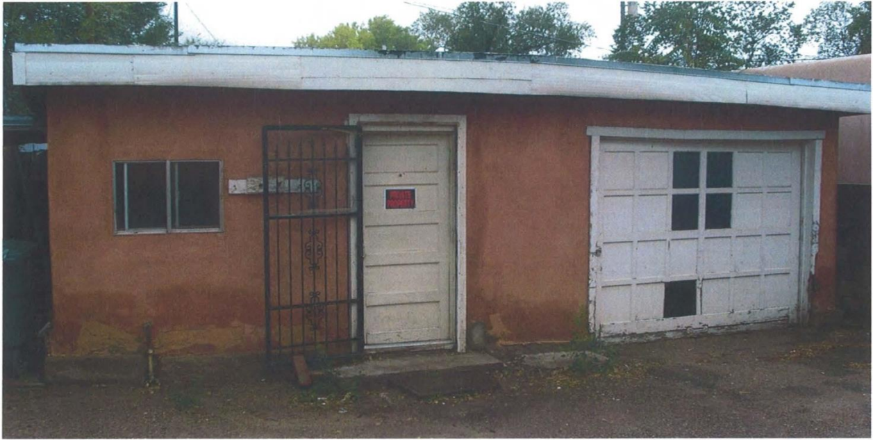
Rear Casita and Garage North Elevation
