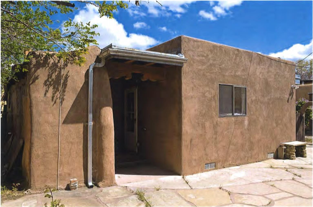
Photo 5: West elevation, post-1978 addition, facing southeast.
