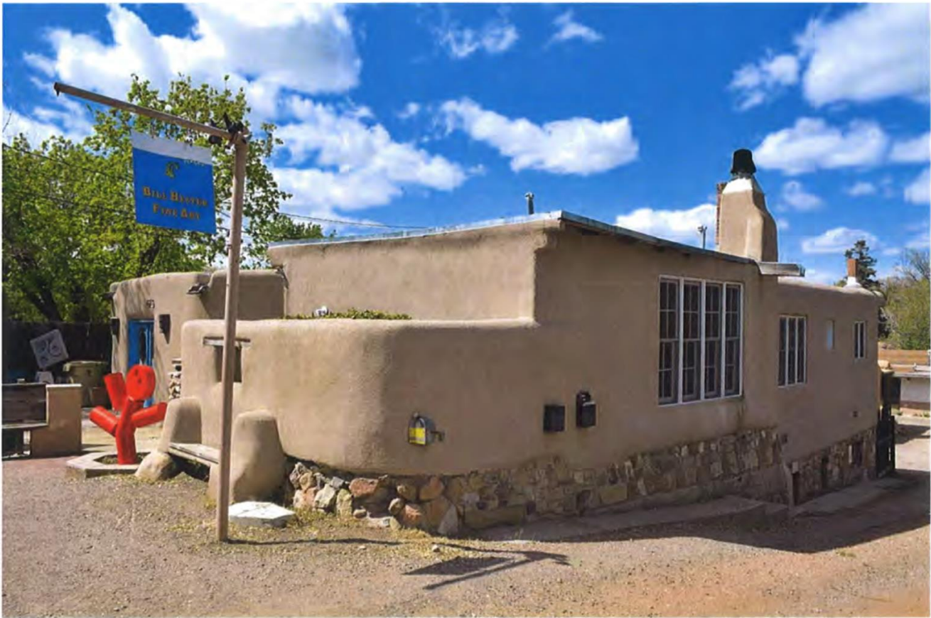
Photo 1: South and east elevations, facing northwest.
