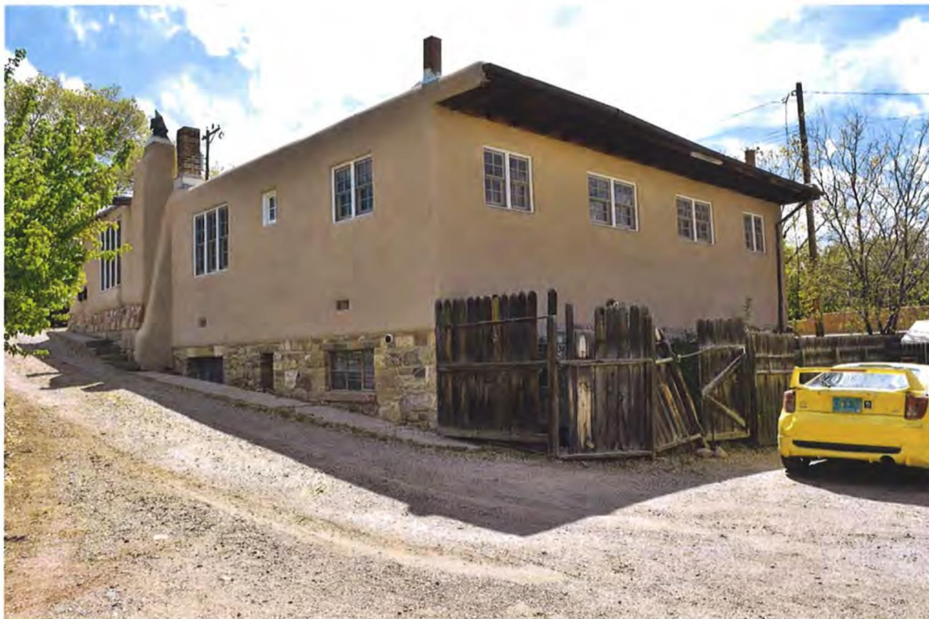
Photo 3: East and North elevations, facing southwest.
