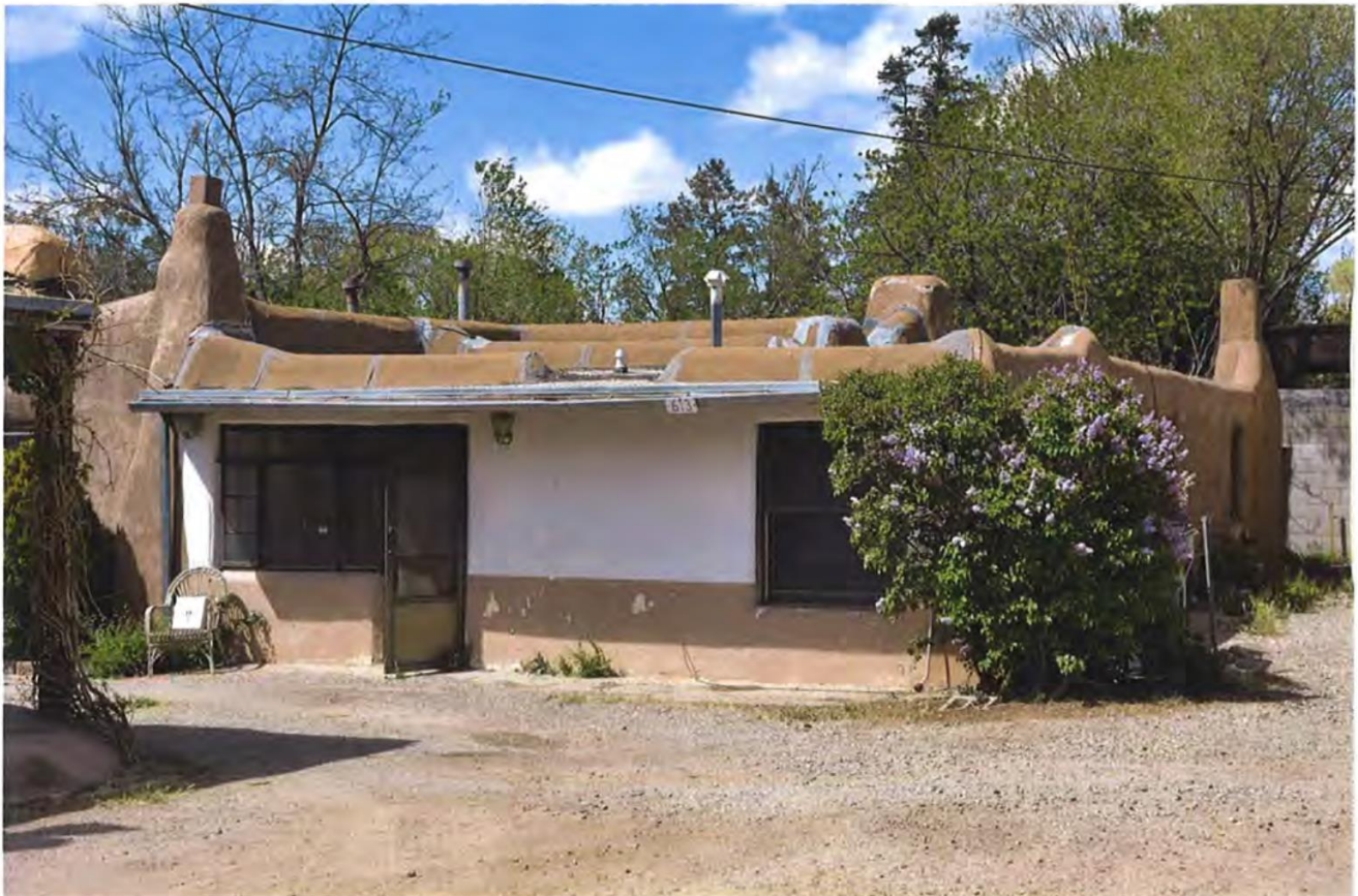
Photo 1: Portion of front (south) façade, facing north.
