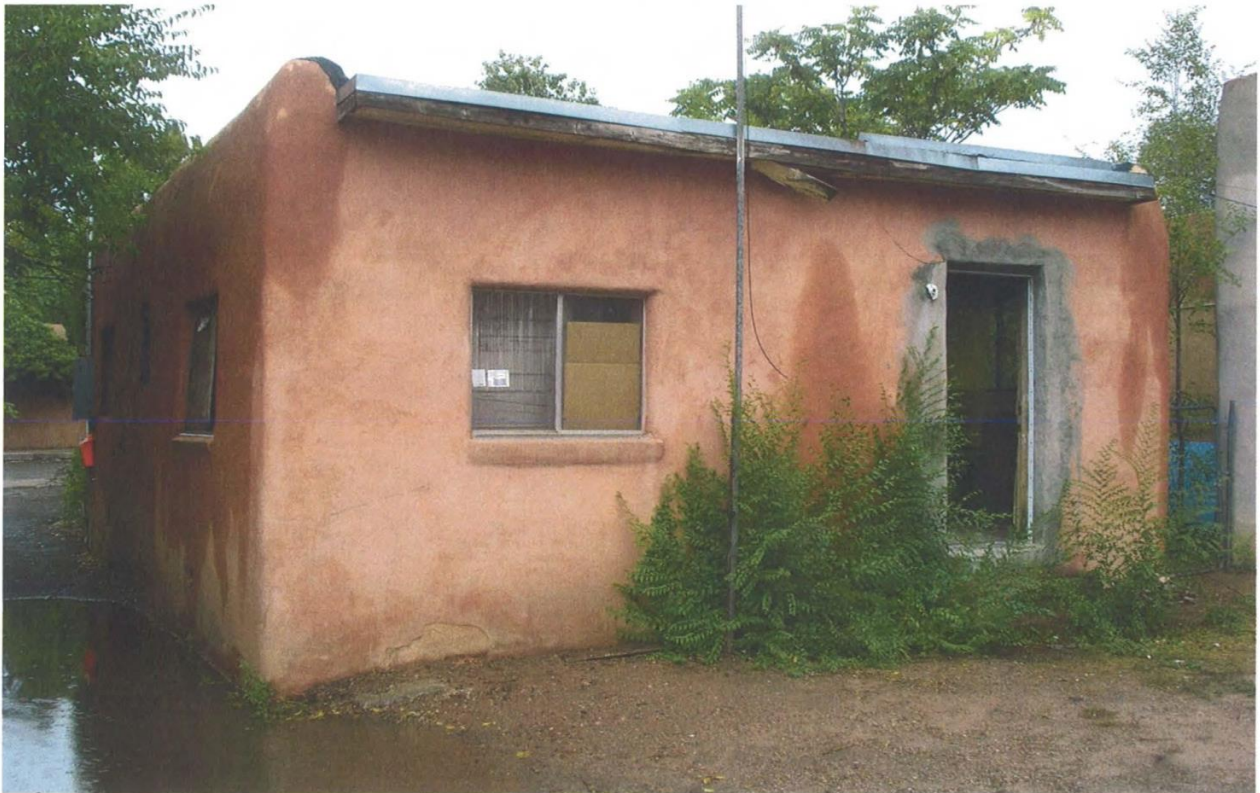
Rear South Elevation with West Elevation
