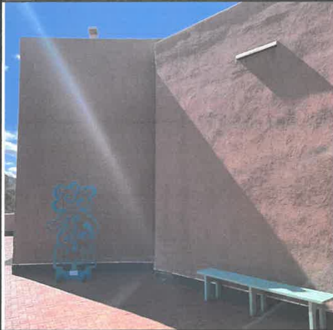
2a. This view shows the existing wall flashing with term bar.
