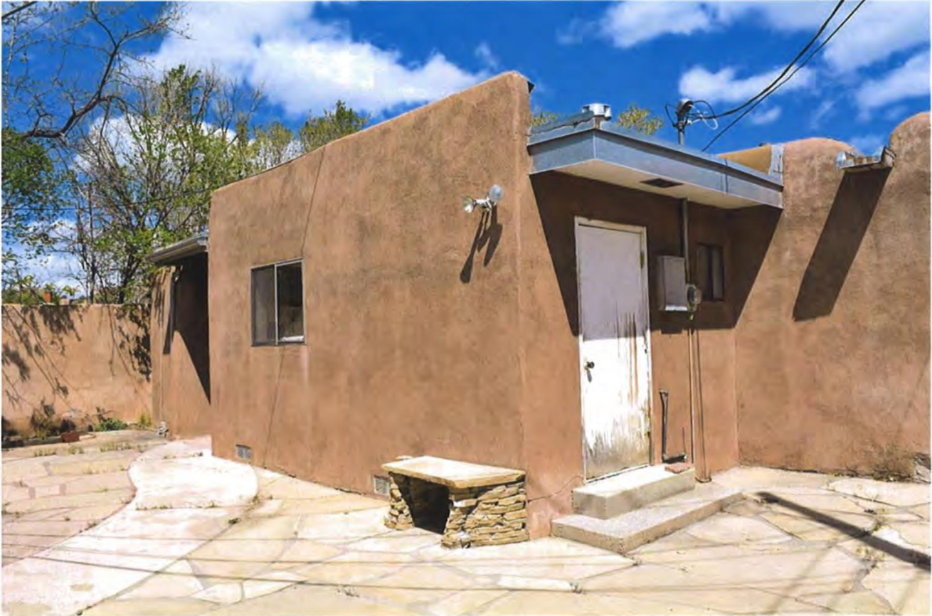
Photo 4: West elevation, post-1978 addition, facing northeast.
