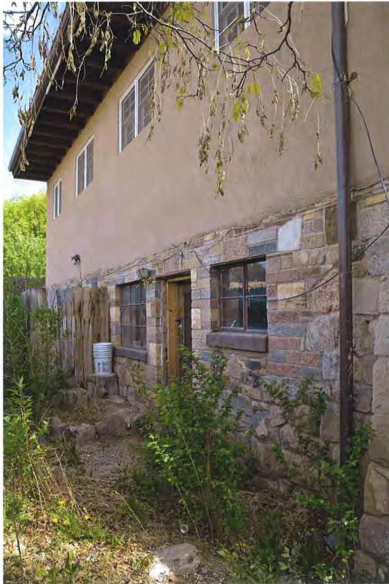
Photo 4: North elevation, facing southeast.
