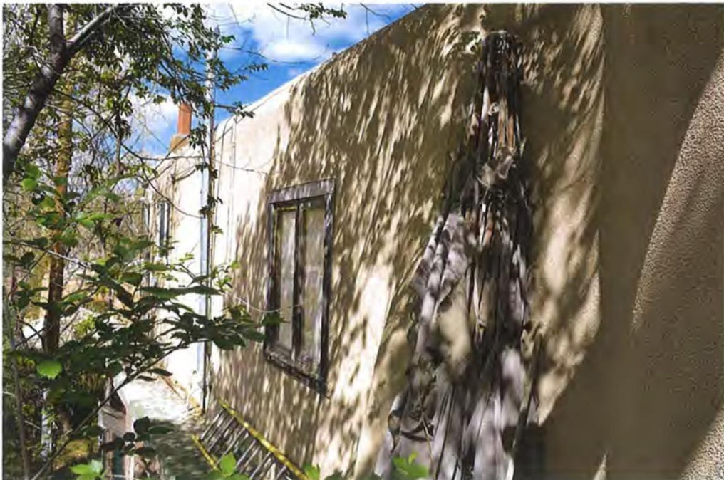
Photo 5: West elevation sequence, starting from Canyon Road, facing northeast.
