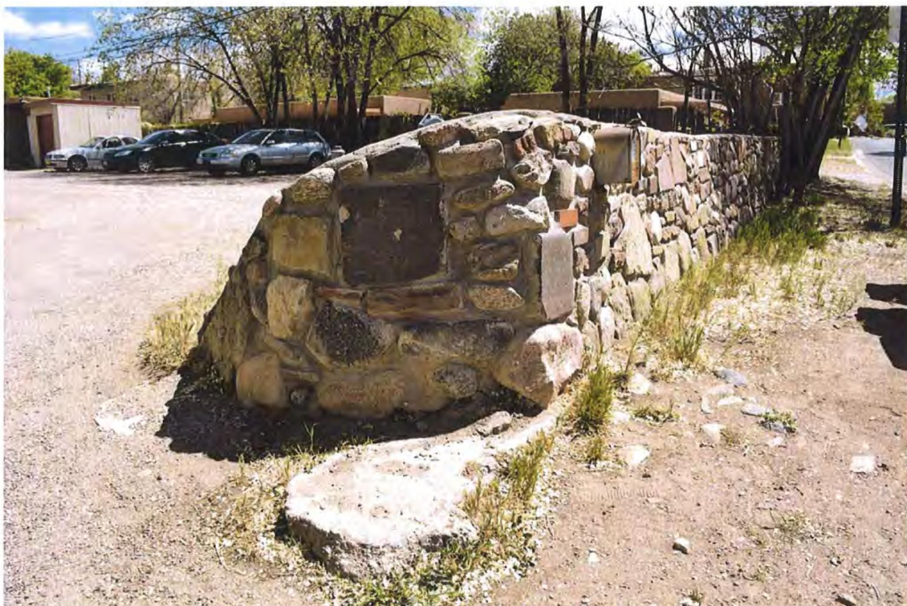
Photo 7: Stone street wall, at Camino Escondido, facing south.
