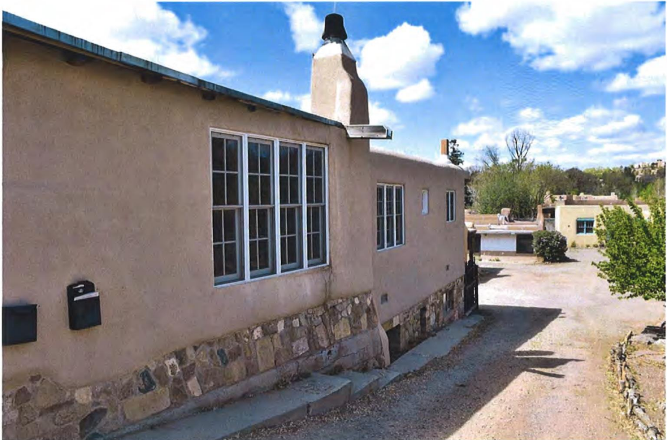
Photo 2: East elevation, facing north.
