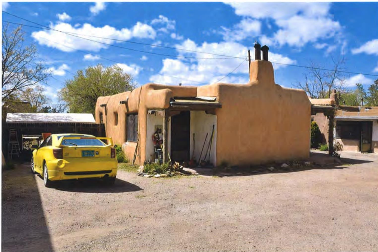
Photo 2: South and east elevations, facing northwest.
