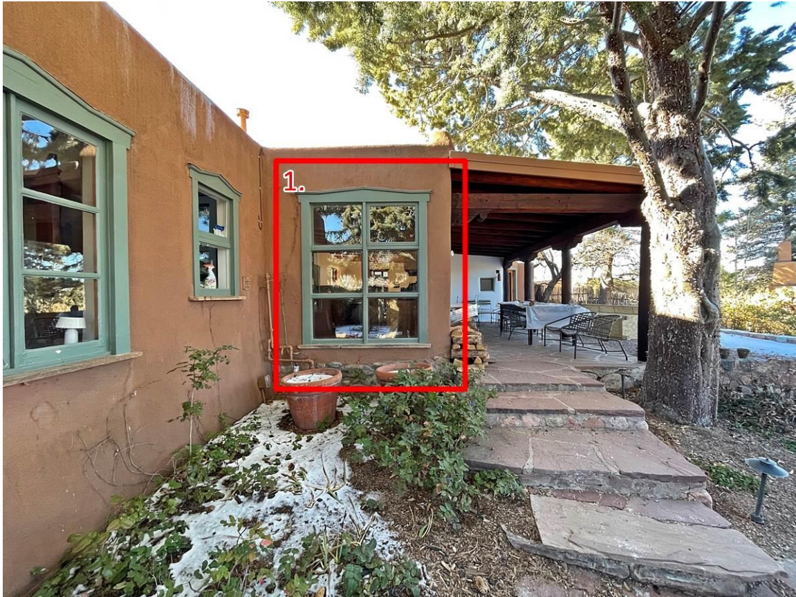
Photo 10: East elevation at portal. Camera facing west. 1. c.1982 addition.
