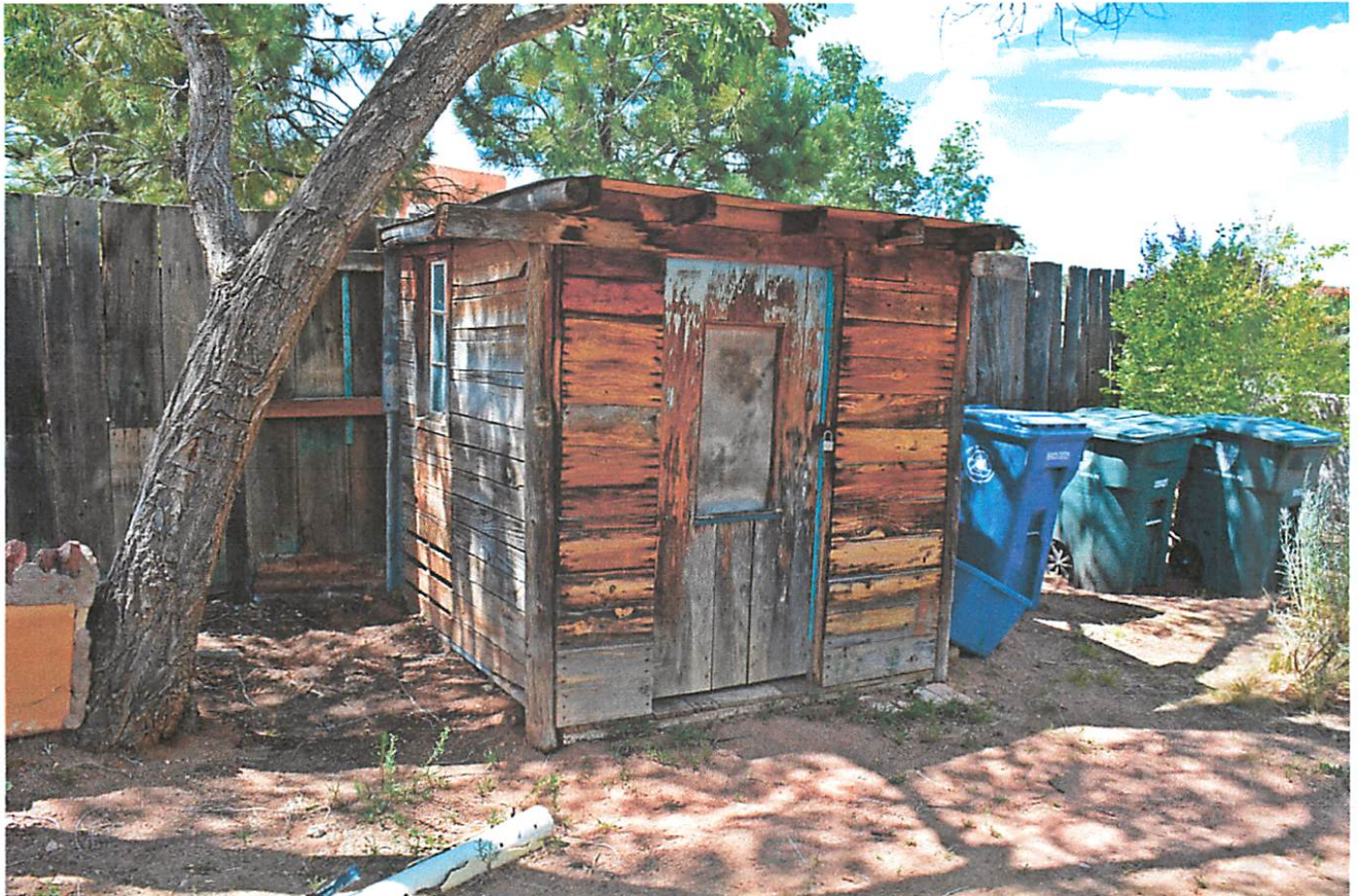
Photo 20: Building E: East elevation, facing northwest.
