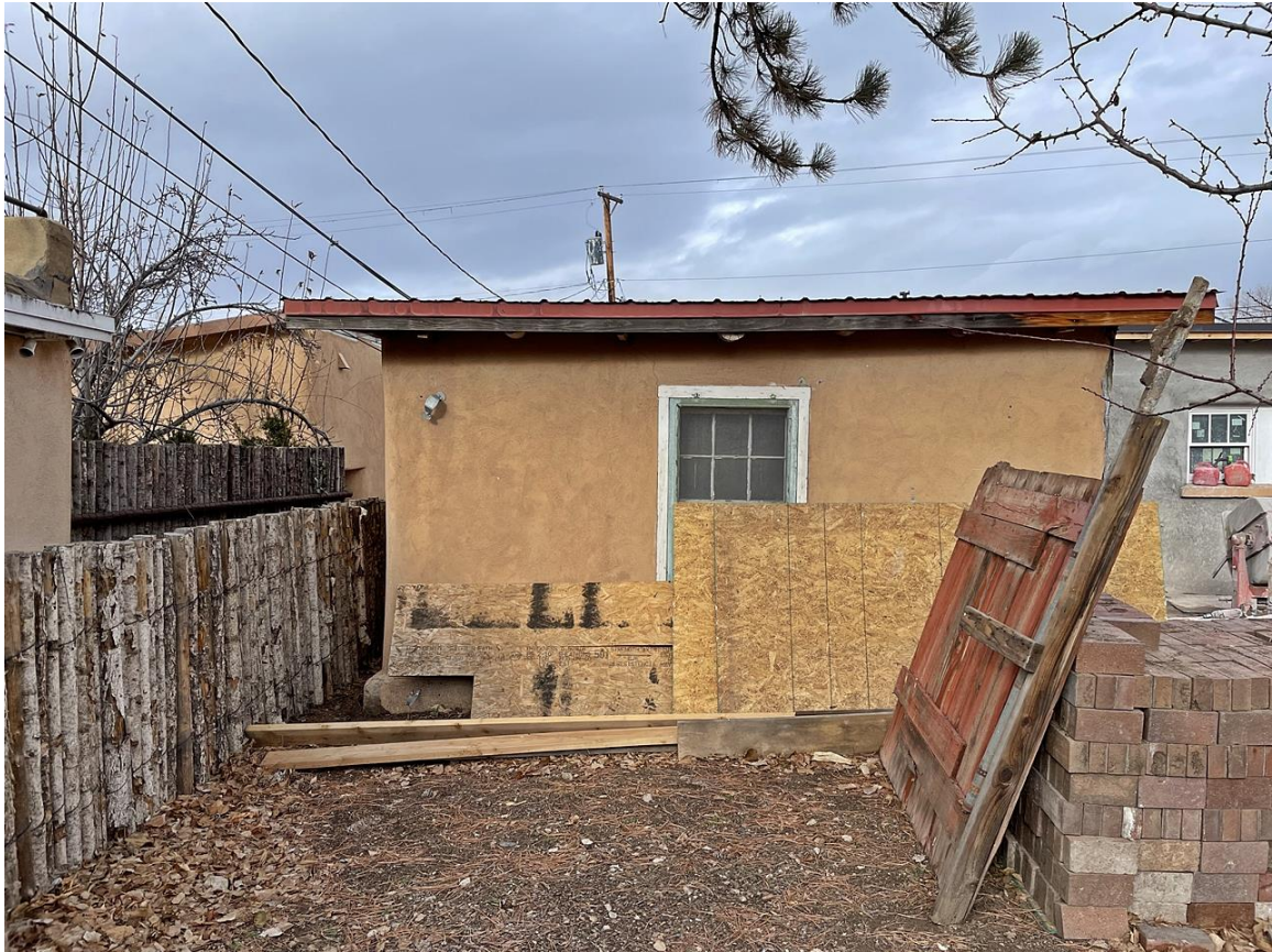
Photo 6: South elevation. Camera facing north.
