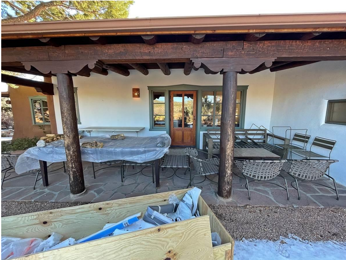
Photo 6: Detail of portal. Camera facing south.
