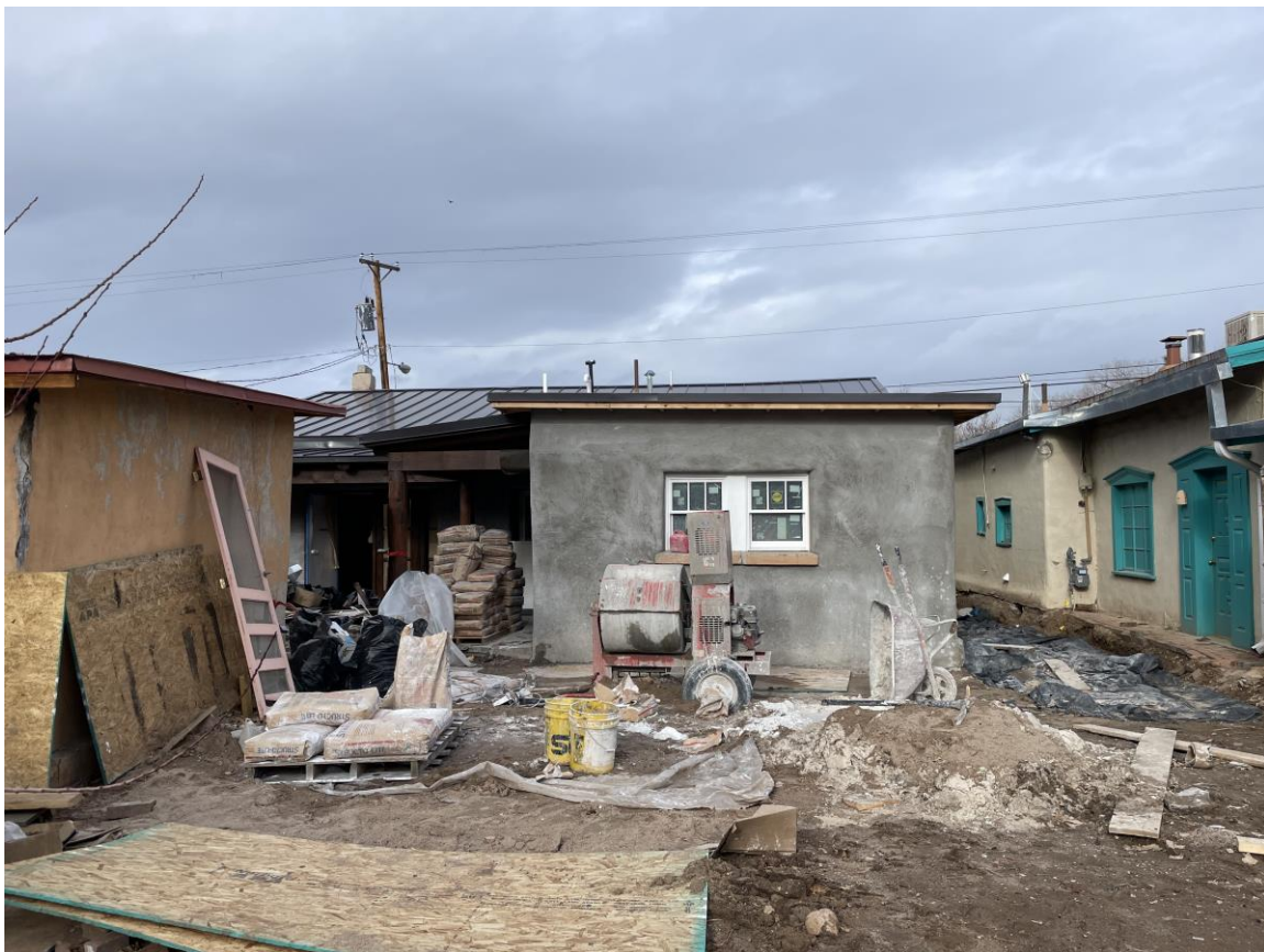
Photo 2: Shed (left) in context with house under renovation. Camera facing north.
