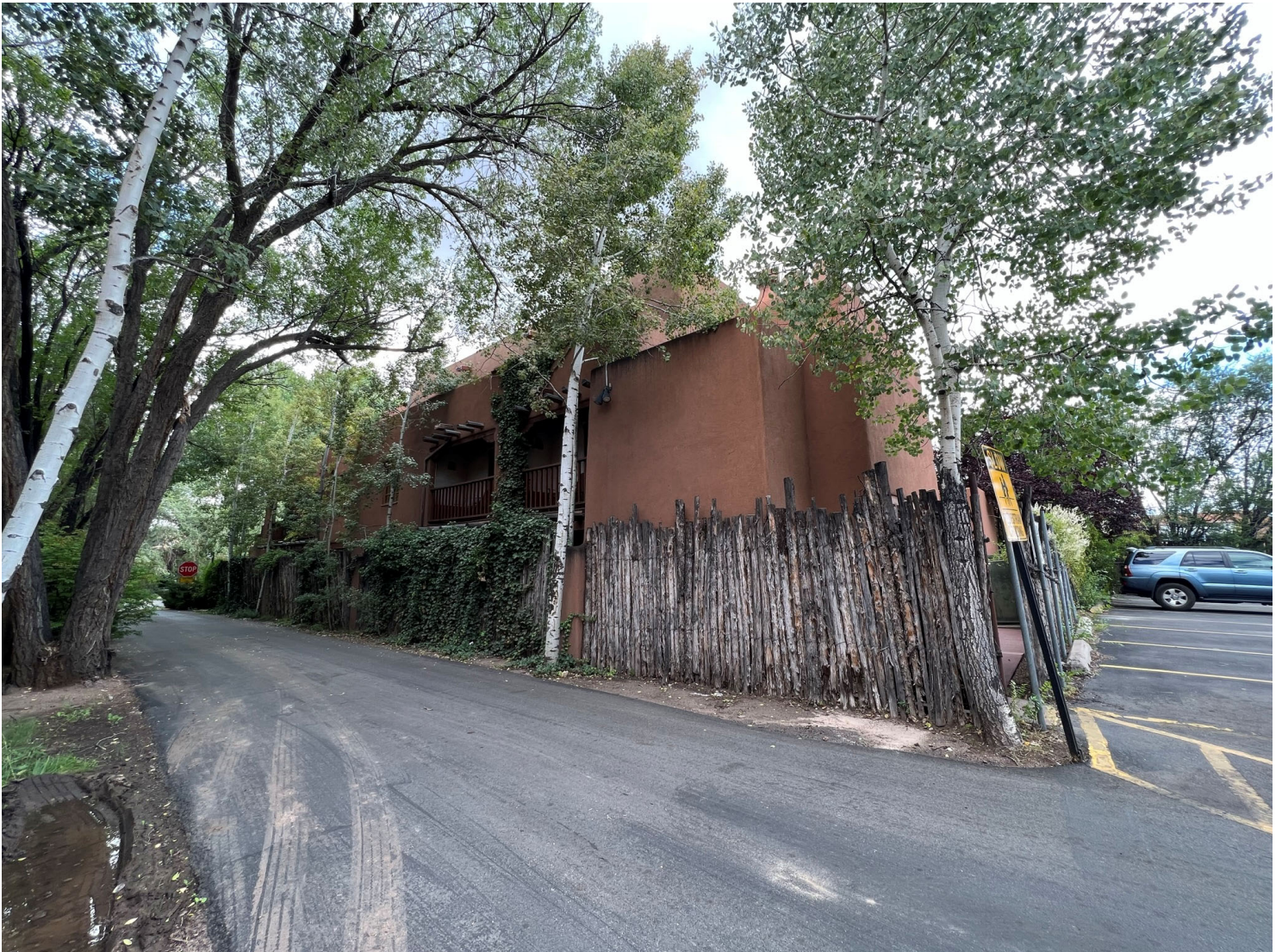
303 E ALAMEDA ST. NORTHEAST VIEW OF BUILDING
