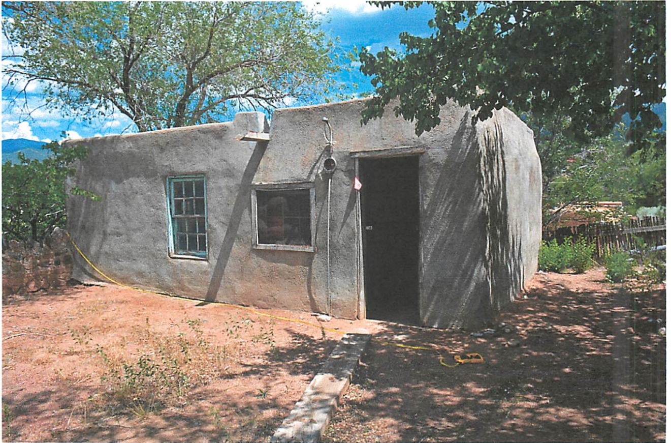
Photo 16: Building D: West elevation, facing northeast.
