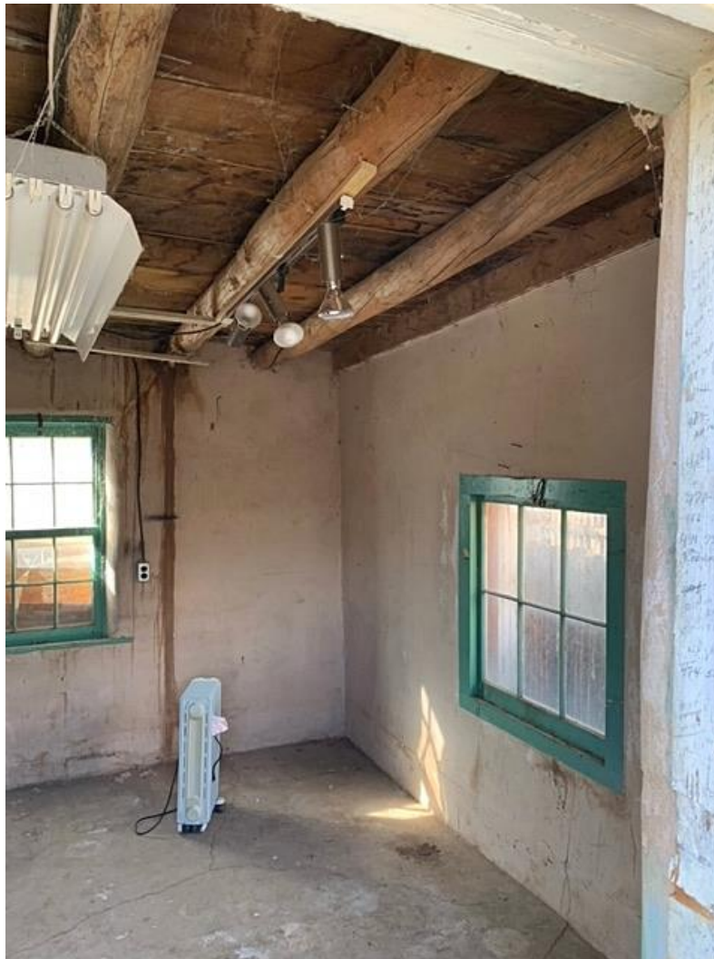
Photo 7: Interior. Camera facing south. Douglas Maahs, February 6, 2023.
