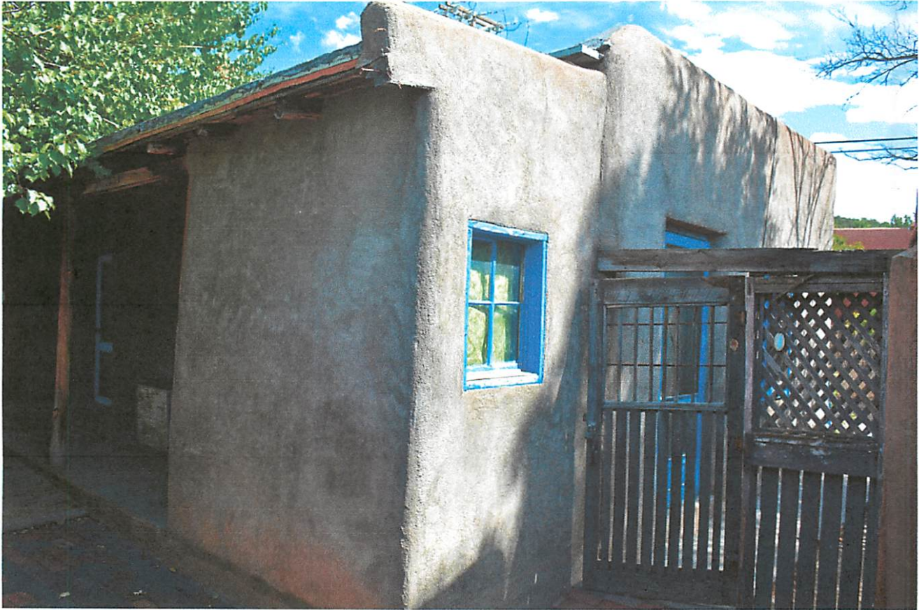
Photo 9: Building B: West elevation, facing northeast.
