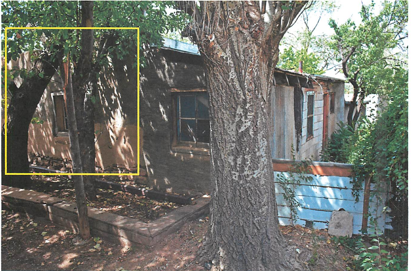
Photo 15: Building C: East elevation, facing northwest. Box indicates probable earlier dwelling incorporated into wing (SP 3).
