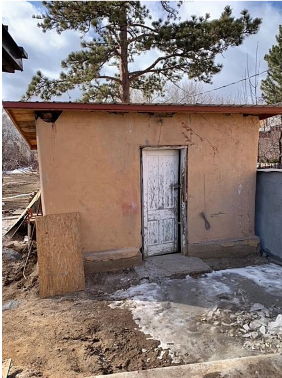
Photo 5: North façade. Camera facing south. Douglas Maahs, February 6, 2023.
