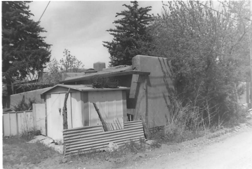
3#25 SE CORNER CONVERTED GARAGE
