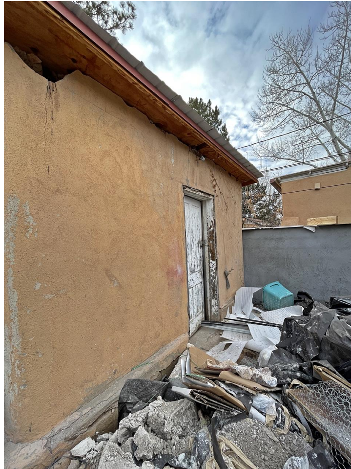
Photo 4: Partial north façade. Camera facing southwest.
