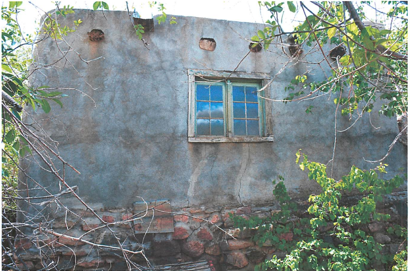
Photo 18: Building D: North elevation, facing southwest.
