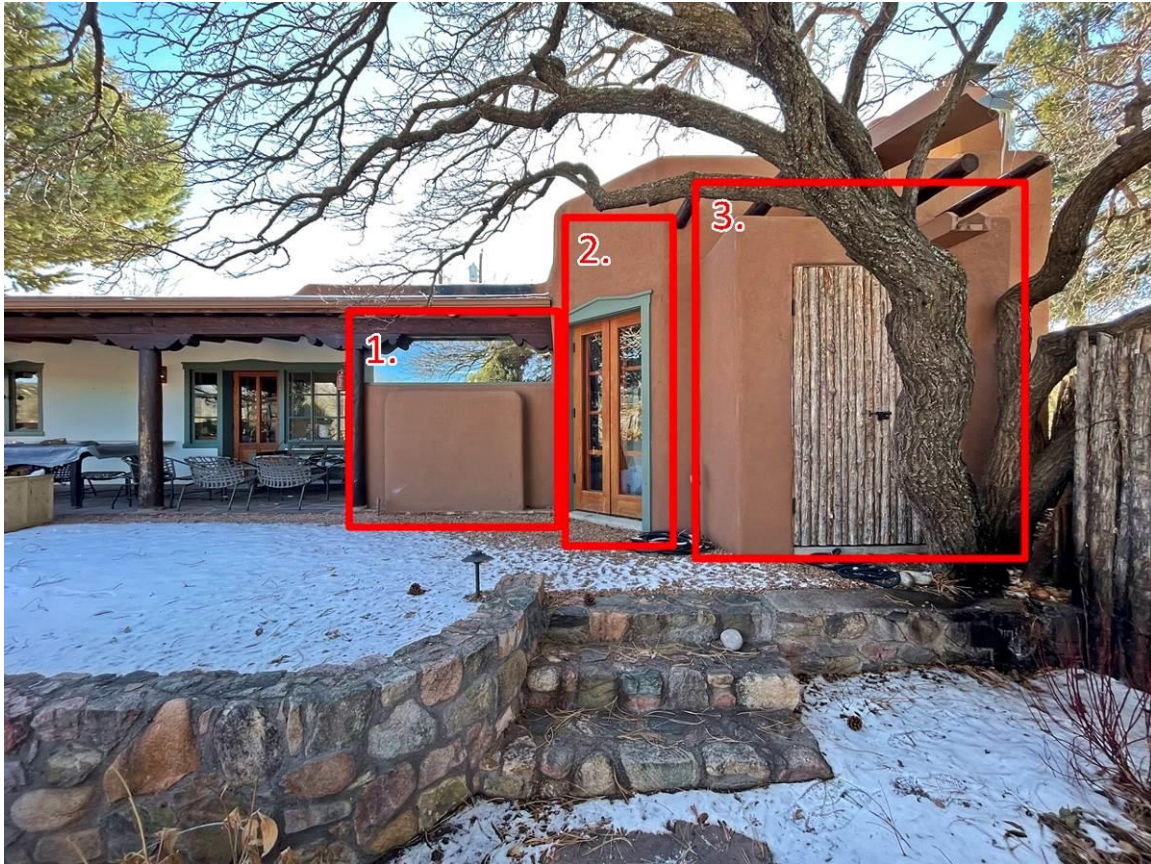
Photo 8: West end of north elevation. Camera facing southeast. 1. c.1982 enclosure to create caretaker's room; 2. 2012 change of window to door; 3. 2012 utility room addition.
