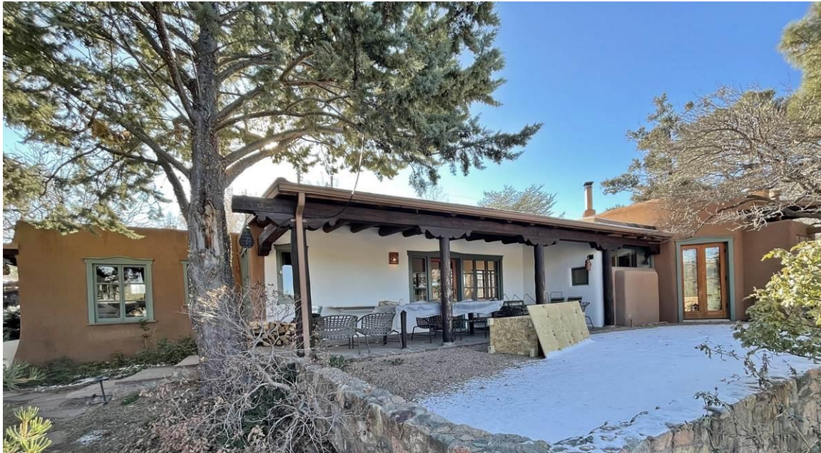
Photo 4: North (rear) elevation. Camera facing northwest.
