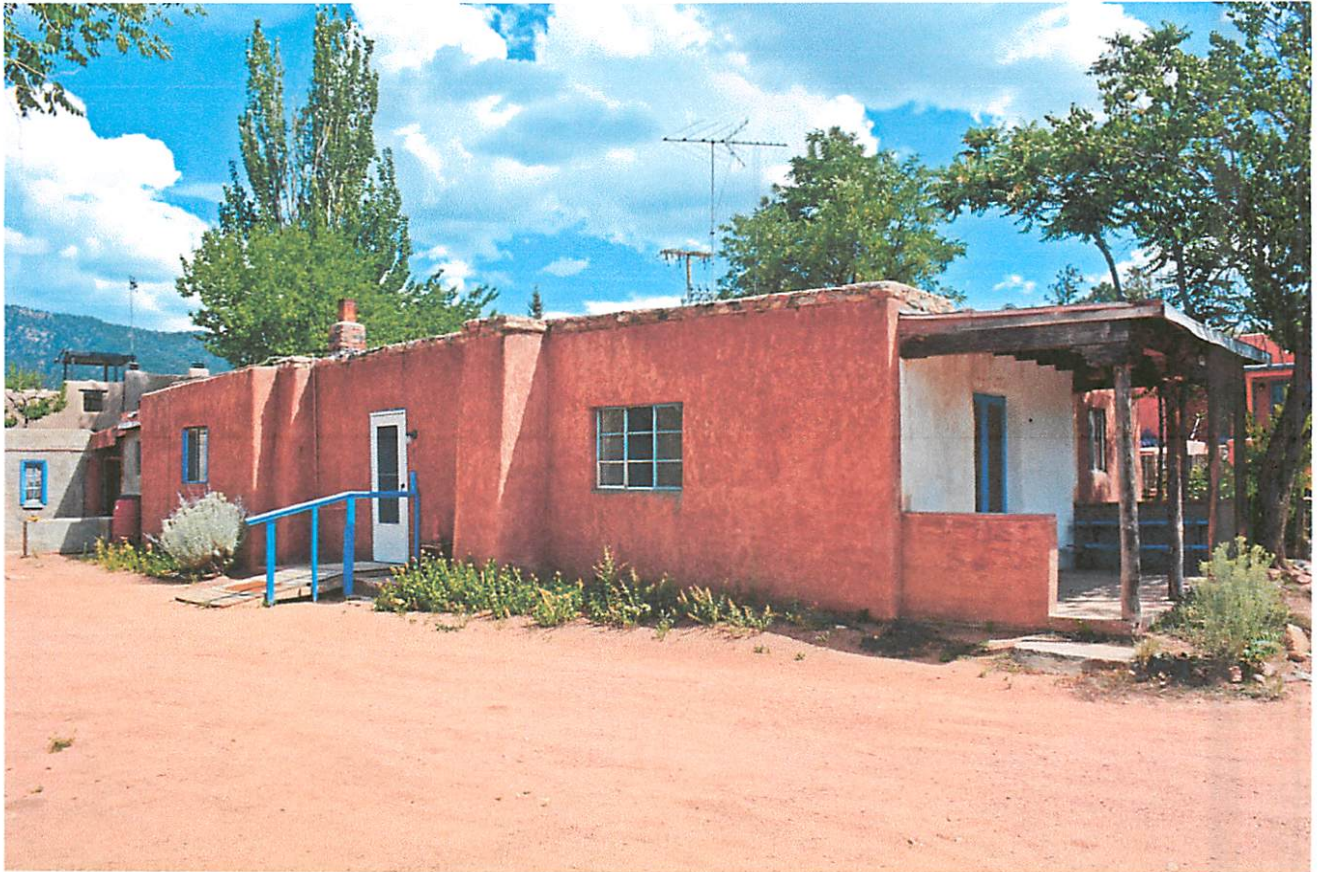
Photo 2: Building A: North and west elevations, facing northeast.
