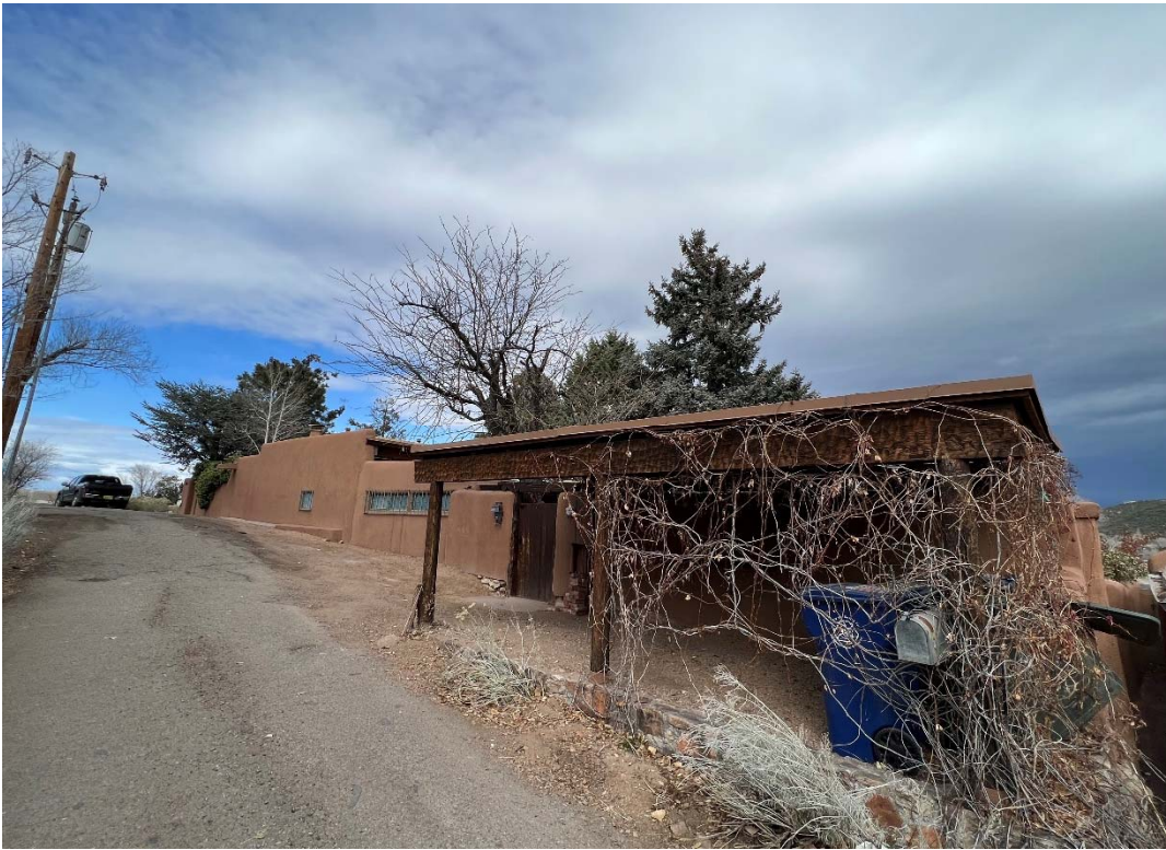
Street View – Looking West
