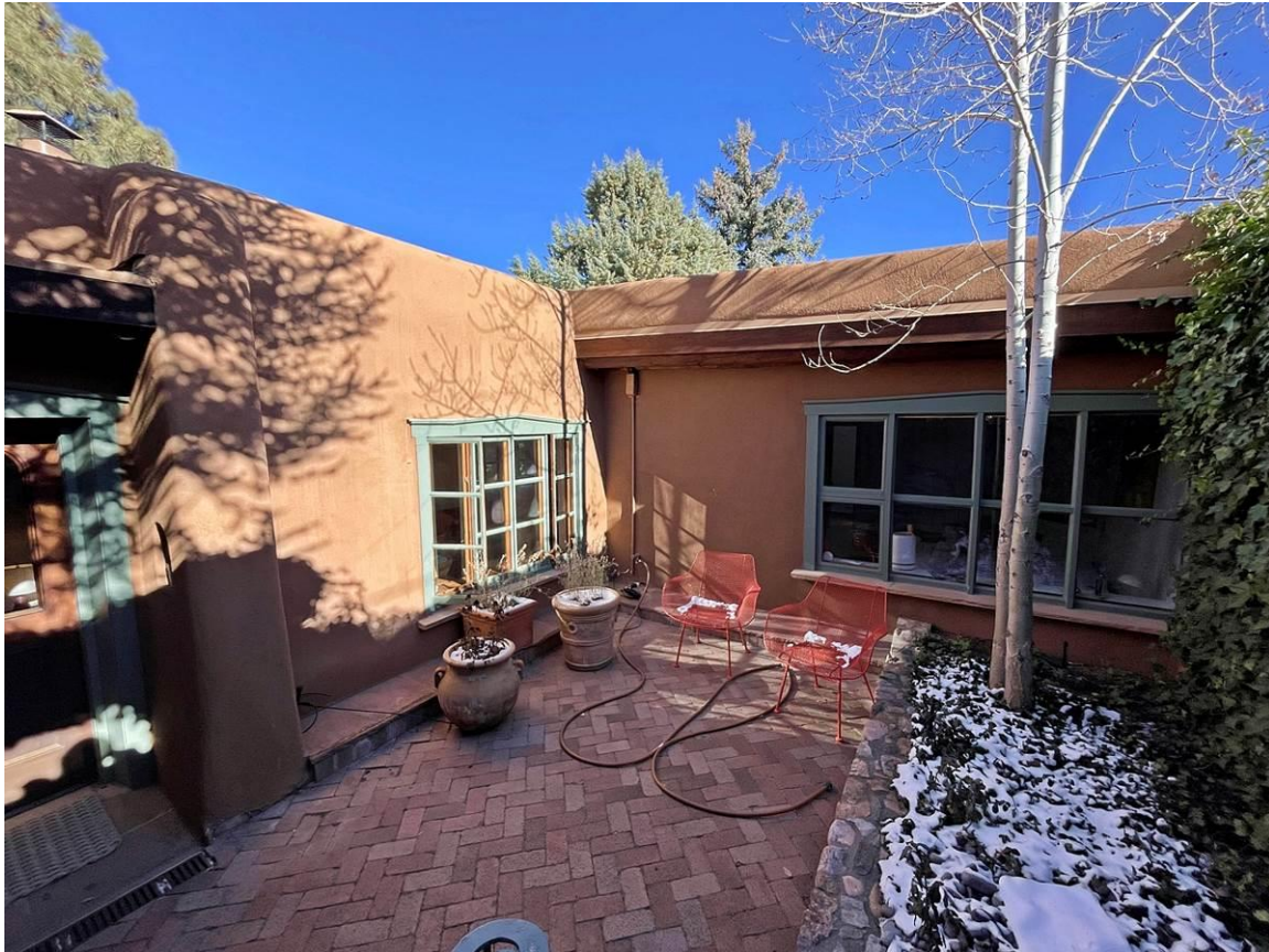
Photo 13: East and south elevations of courtyard. Camera facing northeast.
