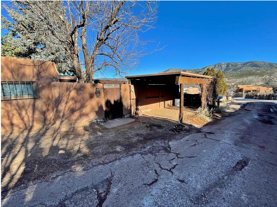
Photo 3: South (front) façade along Camino Delora, and carport. Camera facing northeast.
