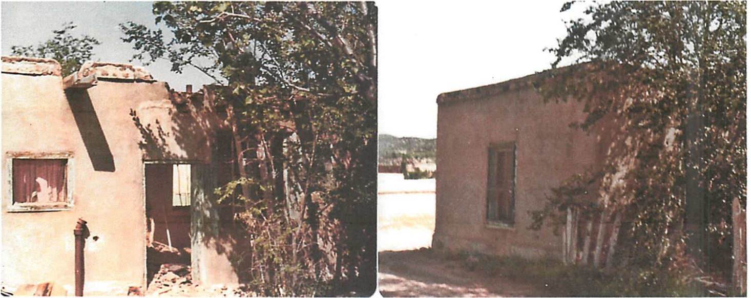
Figure 5: Mid-1970s composite image of Mateo and Teodorita Tafoya House before demolition. Notice similar use of stone at parapet. Source: Tafoya Family.
