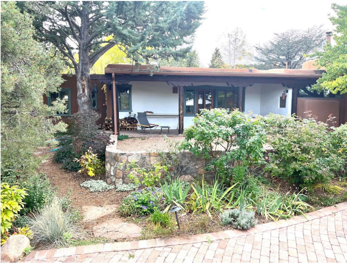
North Side - Rear Elevation
