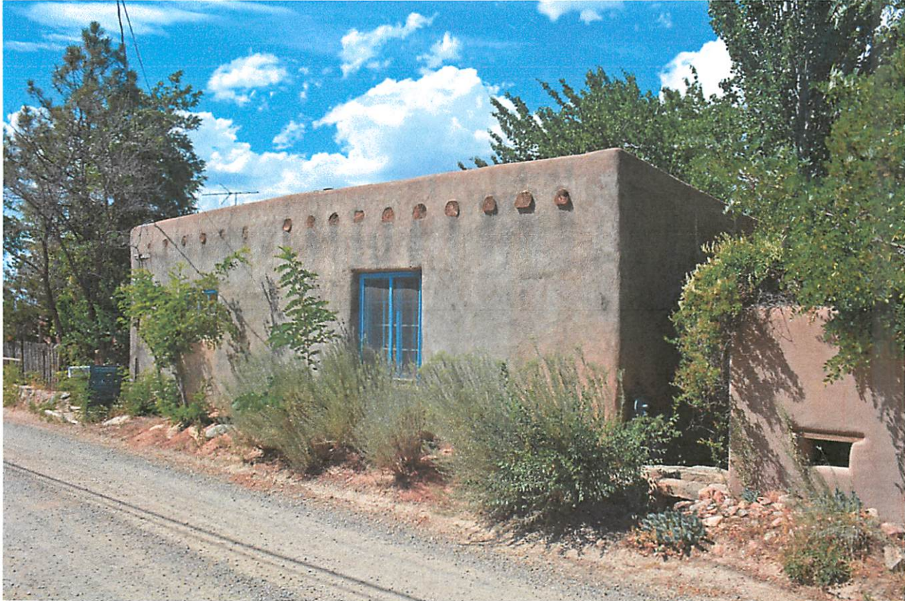
Photo 8: Building B: North elevation, facing northwest.
