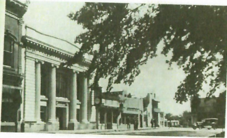
Figure 63. Shelby Street at the Plaza with the First National Bank in foreground, La Florida in background to the left, c. 1928. Courtesy of Museum of New Mexico #51875.
