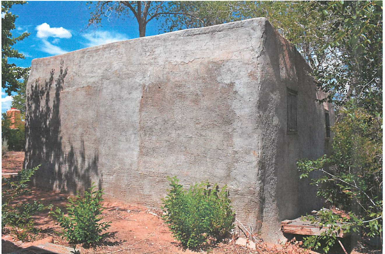
Photo 17: Building D: South and east elevations, facing northwest.
