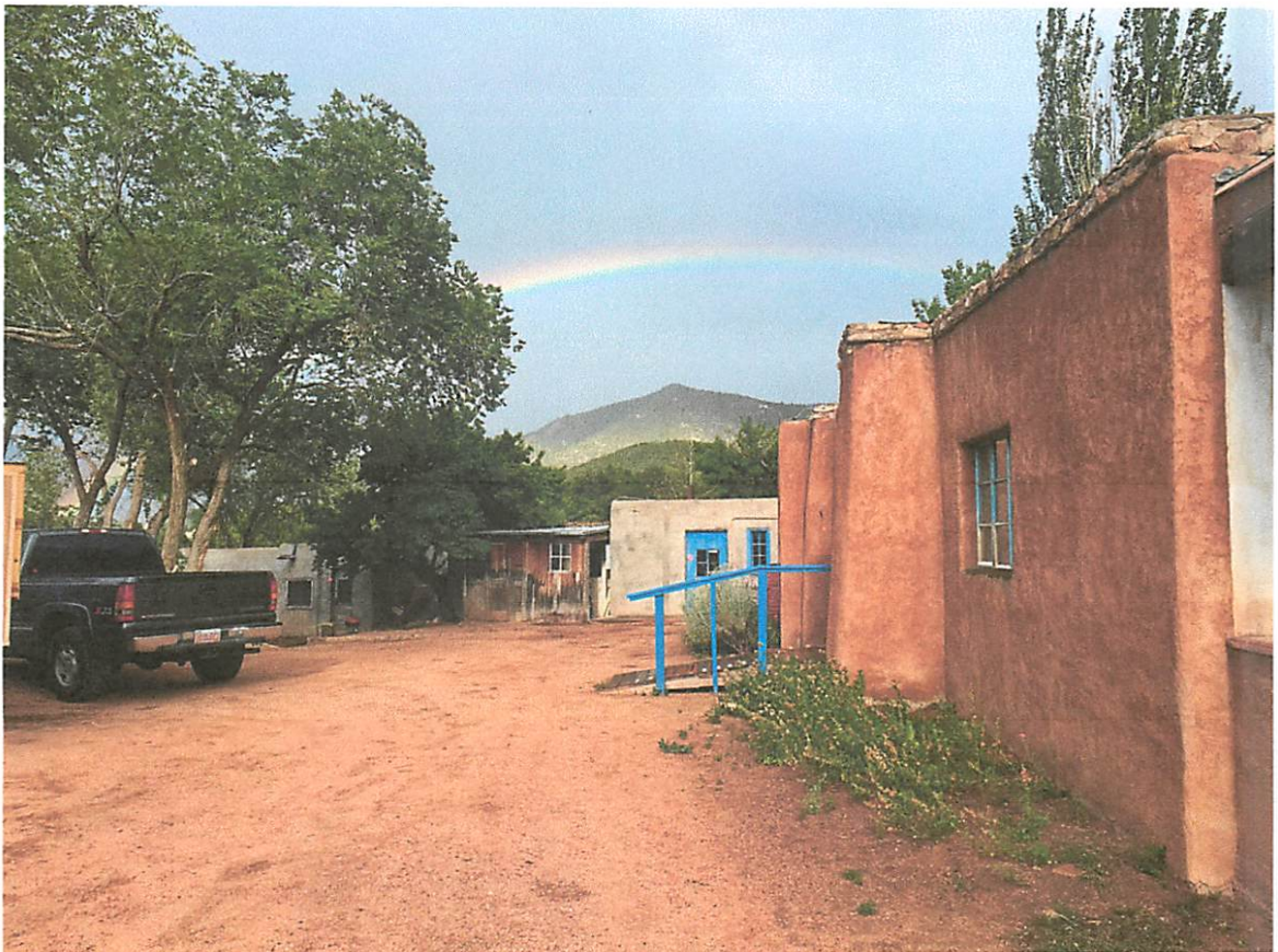
Photo 1: Layout of buildings, as viewed from auto court, facing east.
