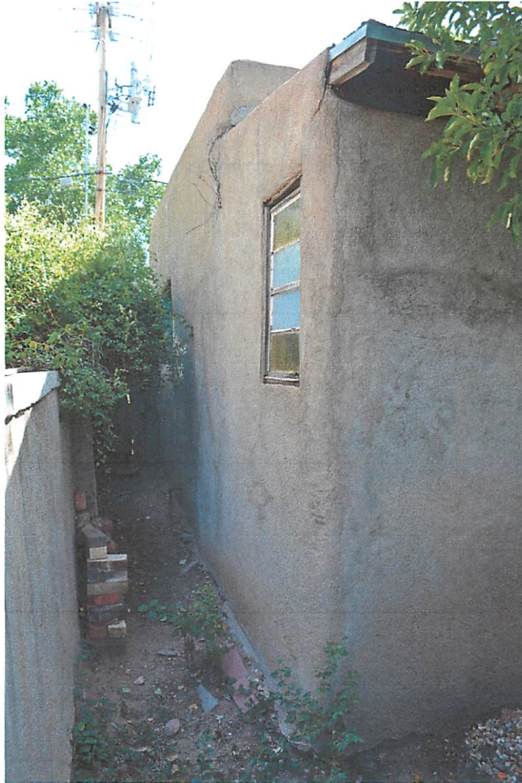
Photo 11: Building B: East elevation, facing southeast.
