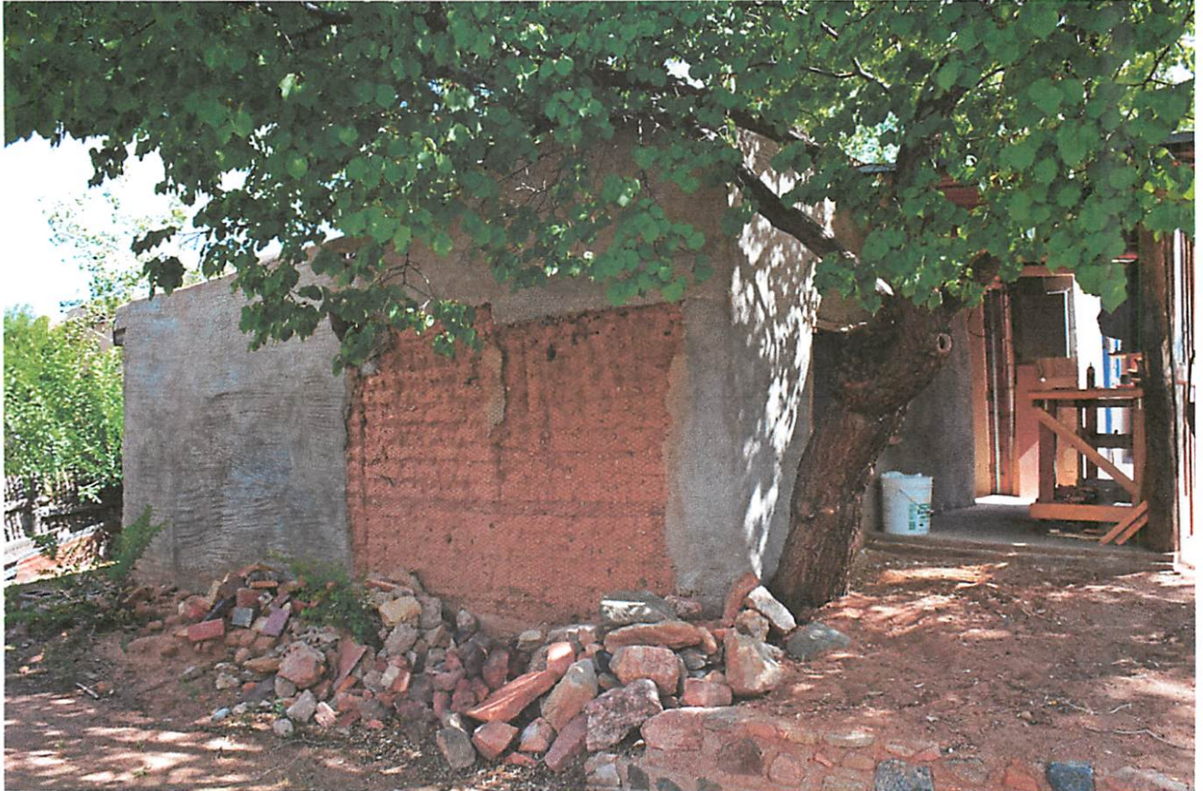
Photo 13: Building C: North elevation, facing northeast.
