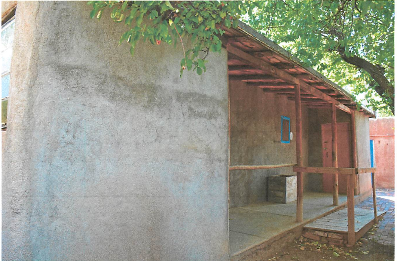
Photo 10: Building B: North elevation with non-historic portal (SP 5), facing southeast.
