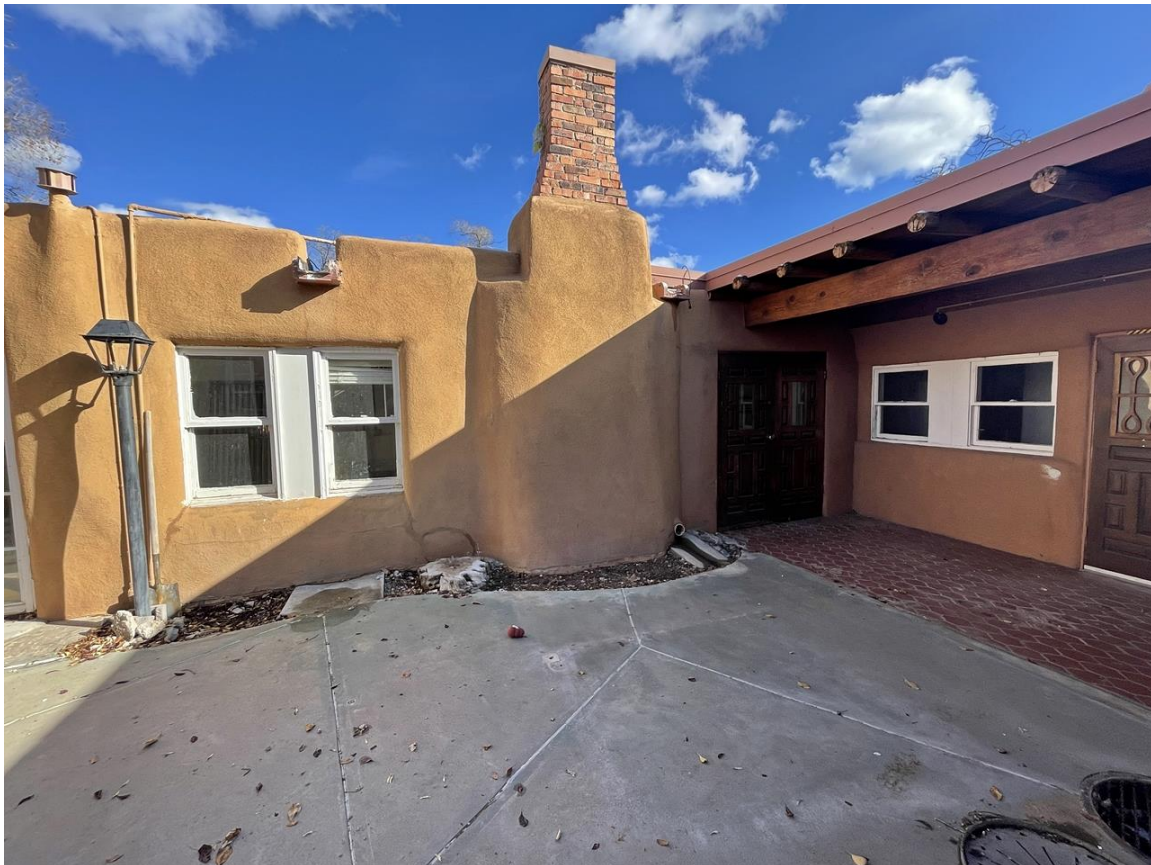
Photo 10: Courtyard, north elevation. Camera facing southeast.
