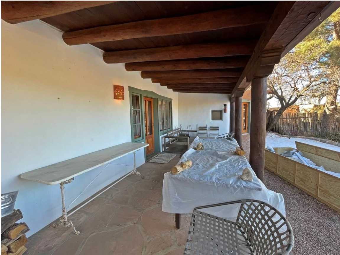
Photo 5: Detail of portal. Camera facing west.
