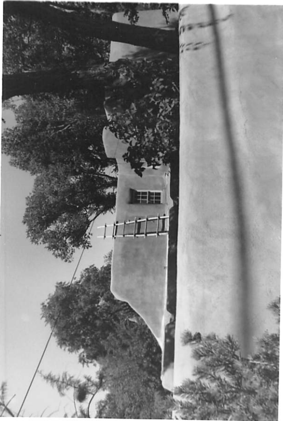
#15 south portion of east elevation
