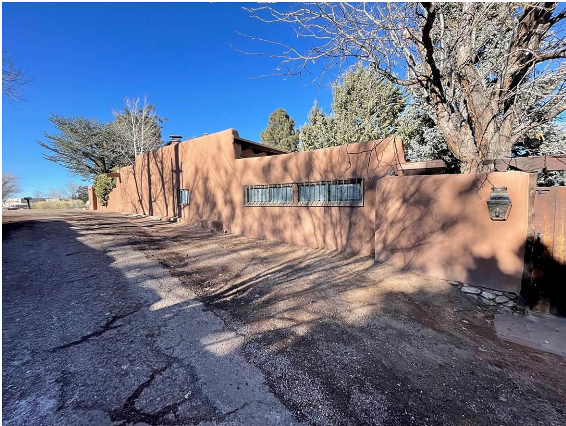
Photo 2: South (front) façade along Camino Delora. Camera facing northwest.
