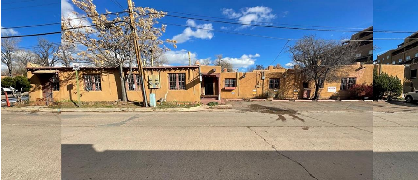
Photo 3: West elevation, composite view. Camera facing east. Chapelle Street view.
