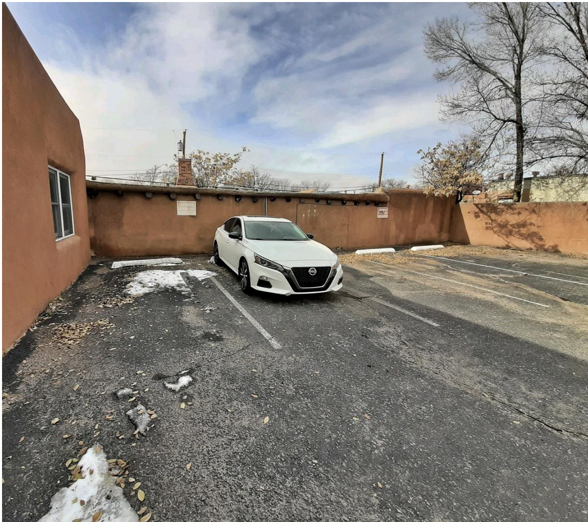
Photo 7: East elevation (center wall). Camera facing northeast. Parking lot view. November 17, 2022.
