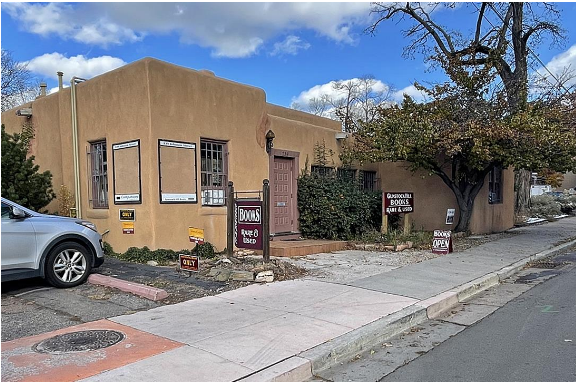
Photo 2: Front (south) façade. Camera facing northeast. Johnson Street view.
