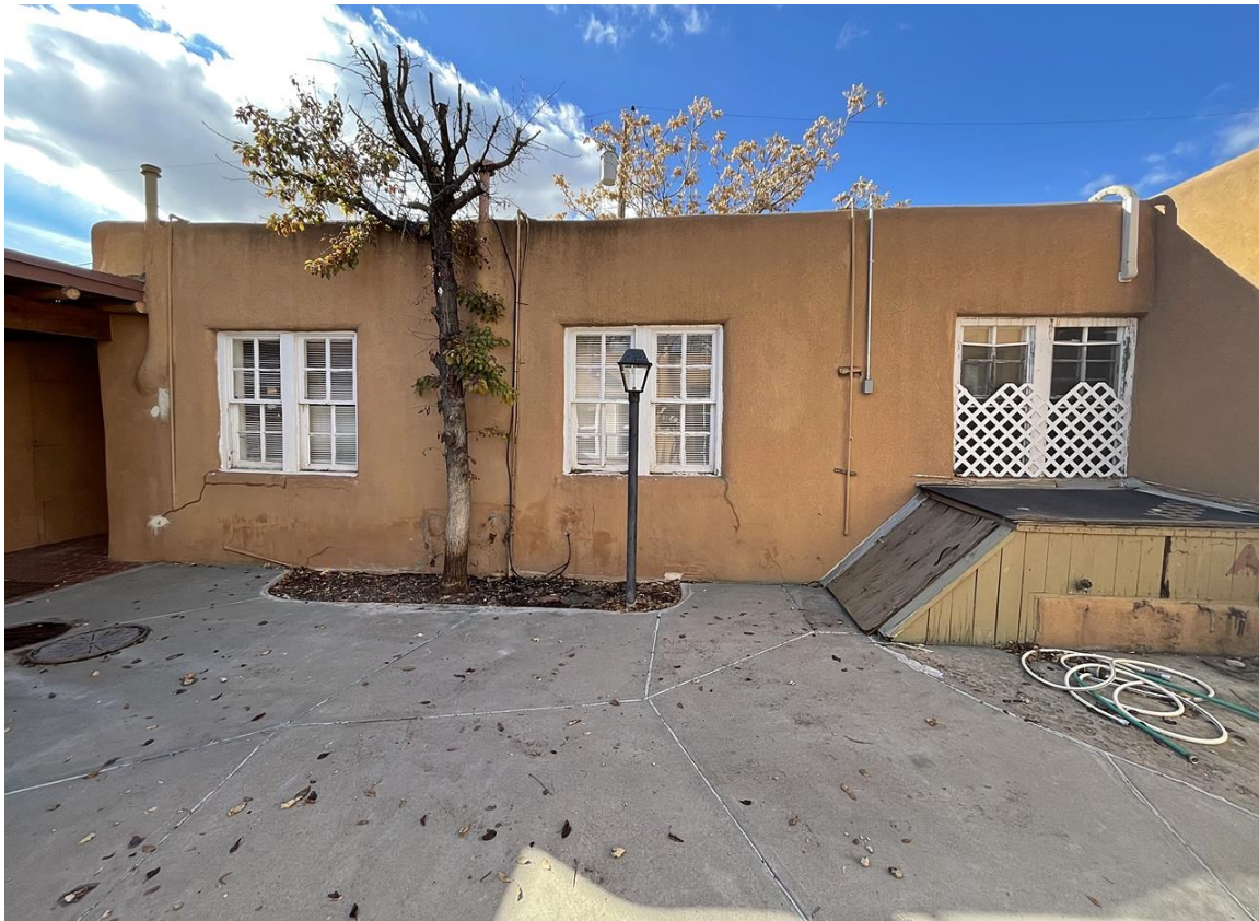
Photo 11: Courtyard, east elevation. Camera facing west.
