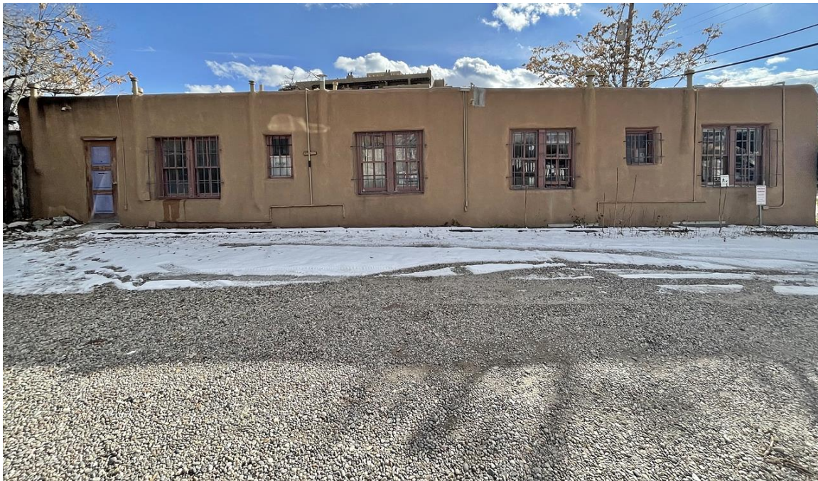
Photo 6: North elevation. Camera facing south. Parking lot view.
