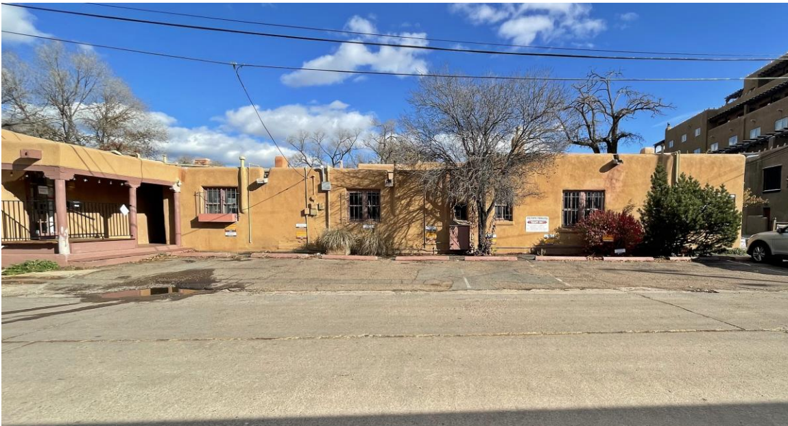
Photo 4: West elevation, south half. Camera facing east. Chapelle Street view.
