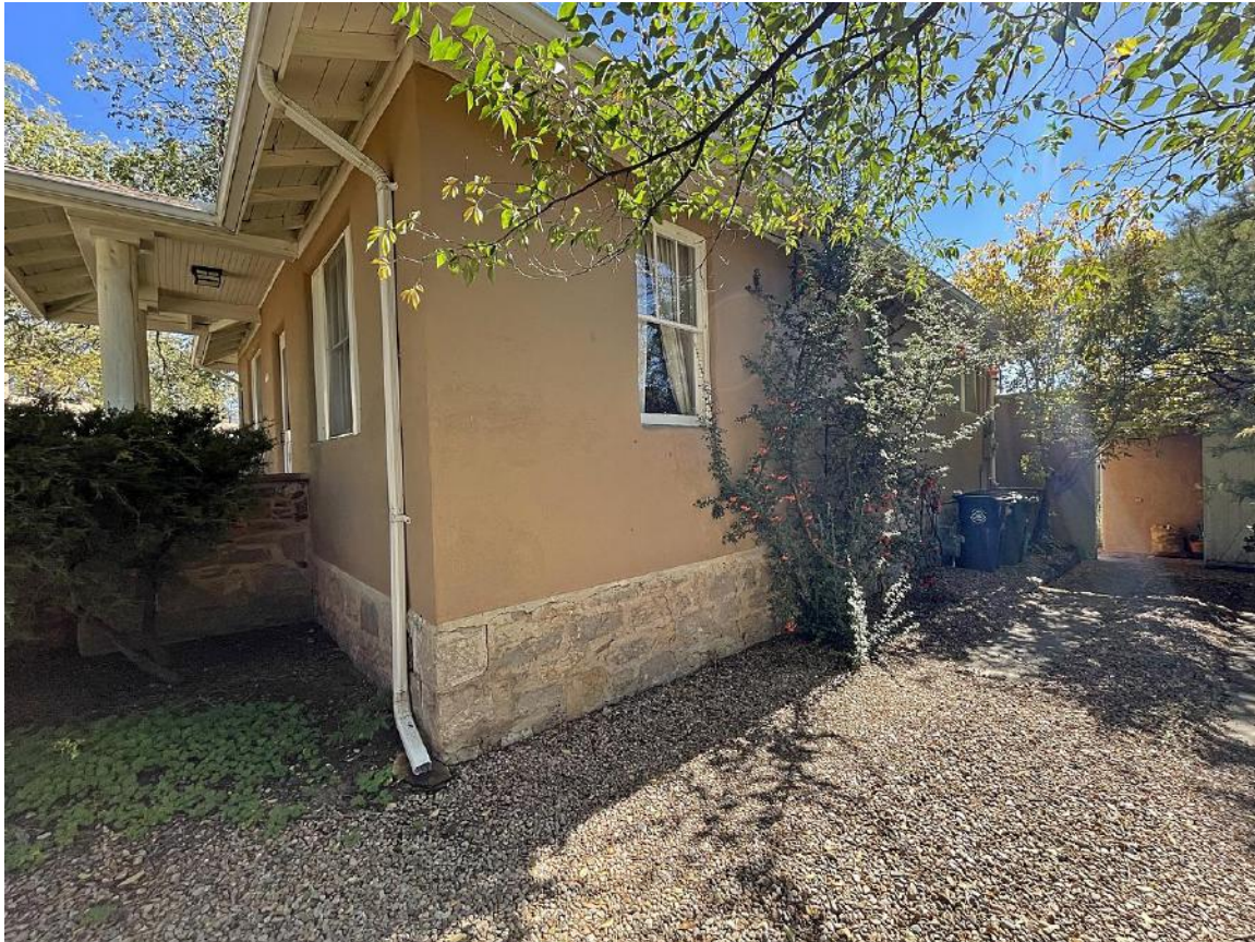
Photo 7: Northwest corner. Camera facing southeast.
