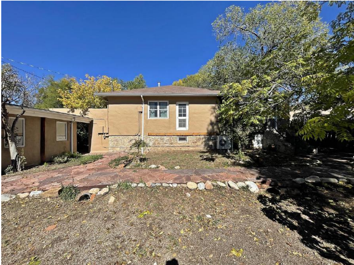
Photo 15: House and Studio. Camera facing north.
