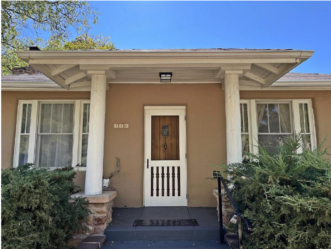
Photo 3: North façade entry. Camera facing south.
