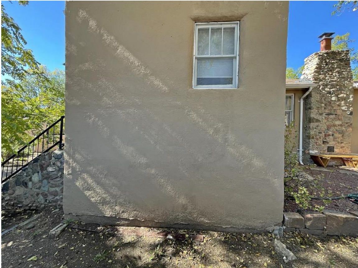
Photo 11: Addition, east elevation. Camera facing west.
