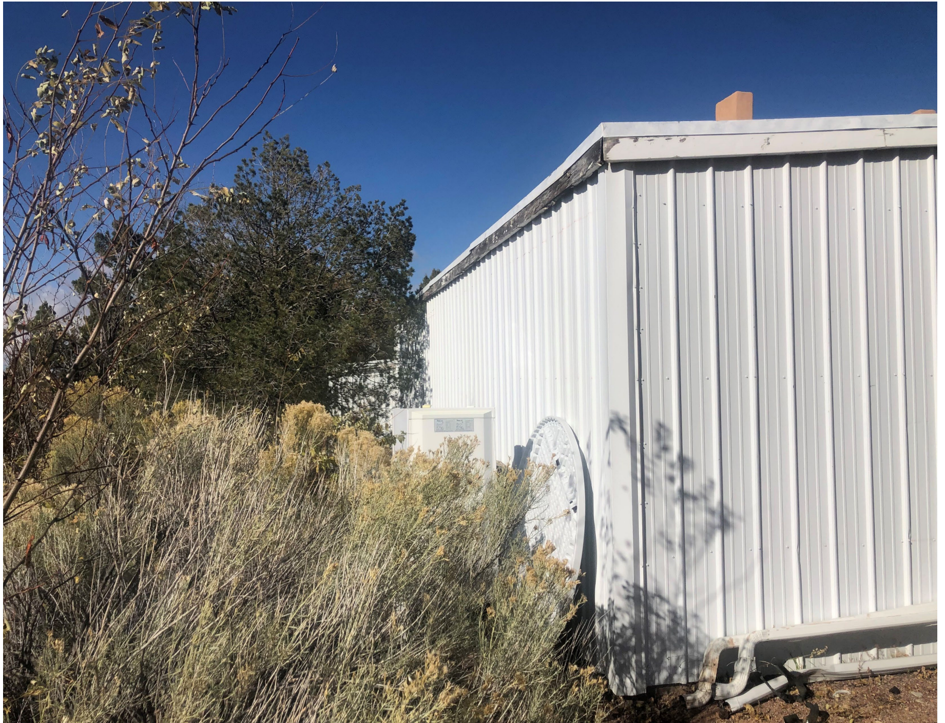
Carport/Shed – South façade
