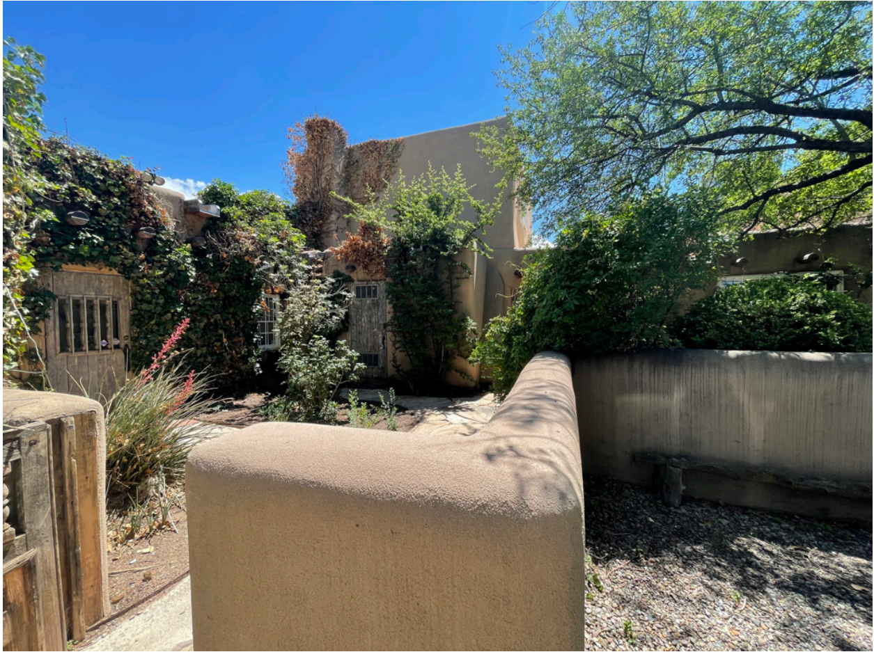
Second floor addition and mechanical room at Courtyard, likely added in 1984.
