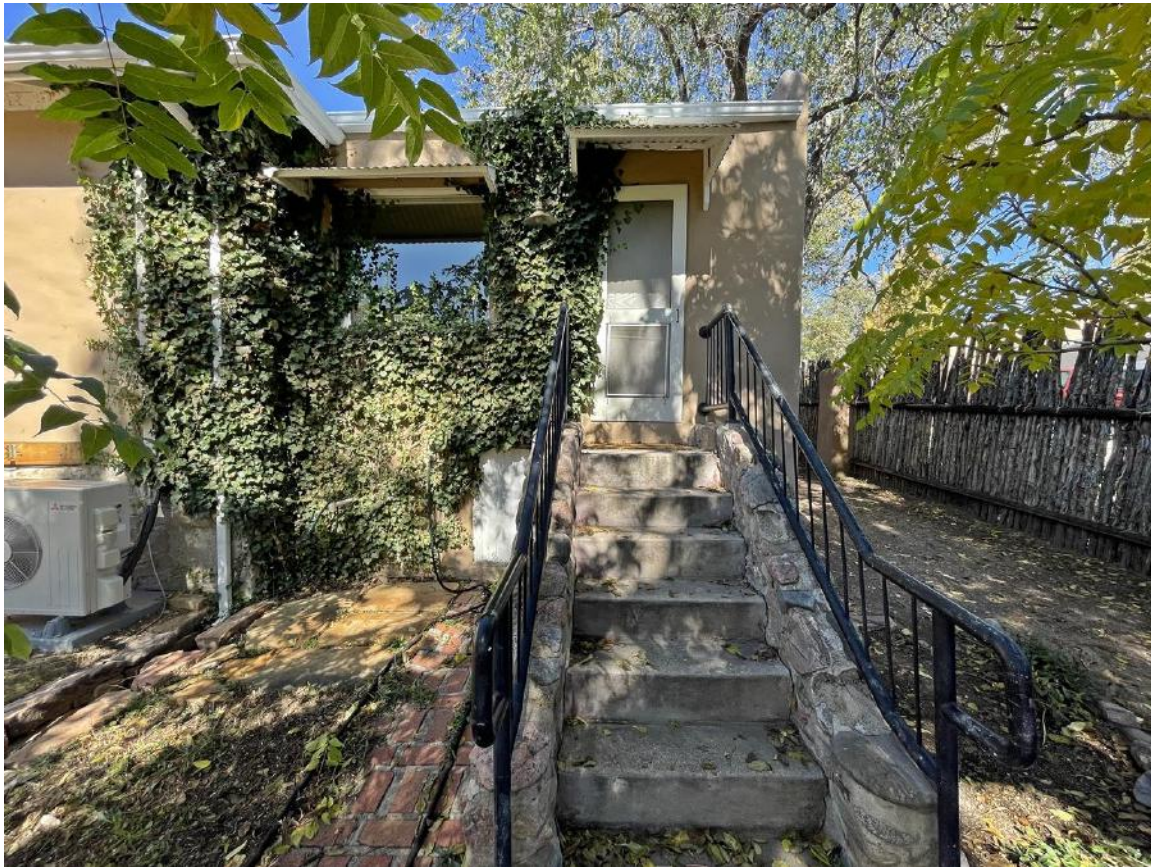
Photo 10: Addition, south elevation. Camera facing north.
