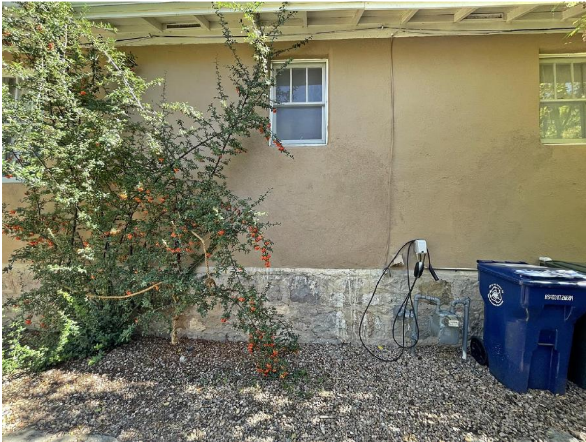
Photo 8: Partial west elevation. Camera facing east.
