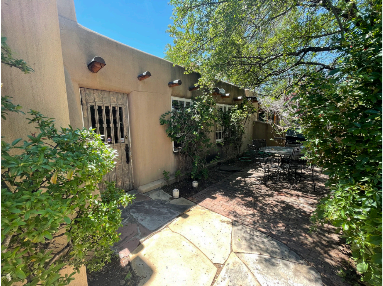
West façade at kitchen and office. Vigas are continuous with interior.
