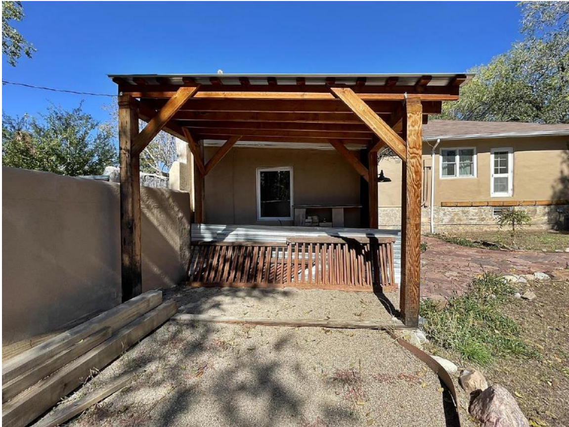
Photo 17: Studio, south elevation. Camera facing north.
