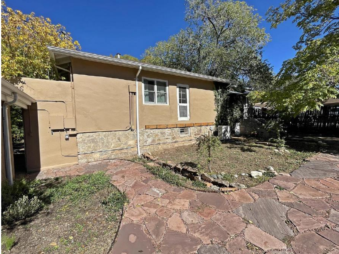
Photo 9: South elevation. Camera facing northeast.
