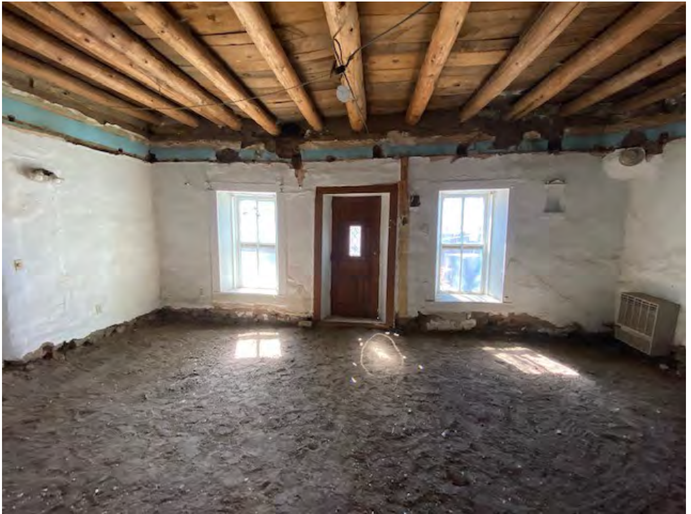
Interior of Southwest Room after removal of wood boards and ceiling.
