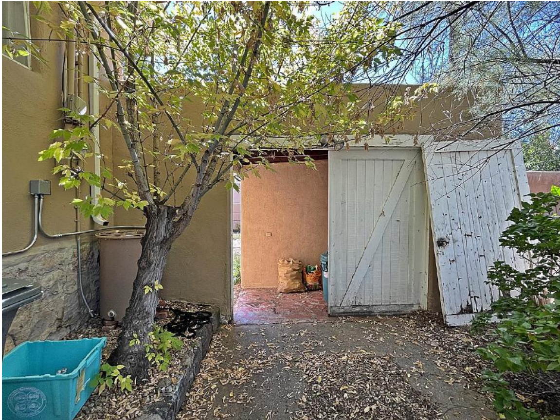
Photo 14: Former garage, north elevation. Camera facing south.
