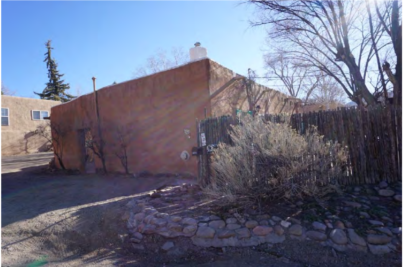
WEST FACADE WITH ONE DOOR OPENING, SLIGHTLY BELOW GRADE, CHIMNEY IS EXPOSED, INSIDE THE FIREPLACE WAS REMOVED. EXISTING ROCK WALLS AND COYOTE FENCE- NO DATES AVAILABLE.
