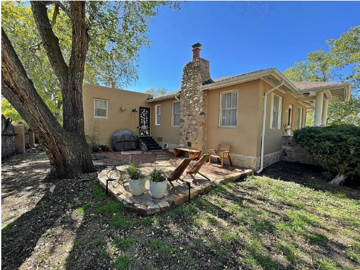
Photo 13: East elevation. Camera facing southwest.
