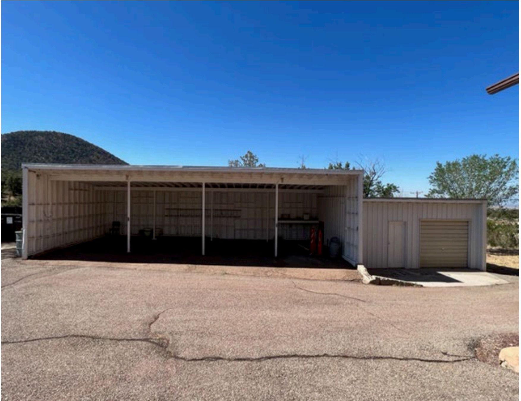
Carport/Shed – North façade
