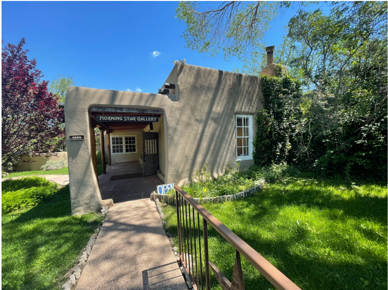
South Façade facing Canyon Road, the oldest part of the structure
