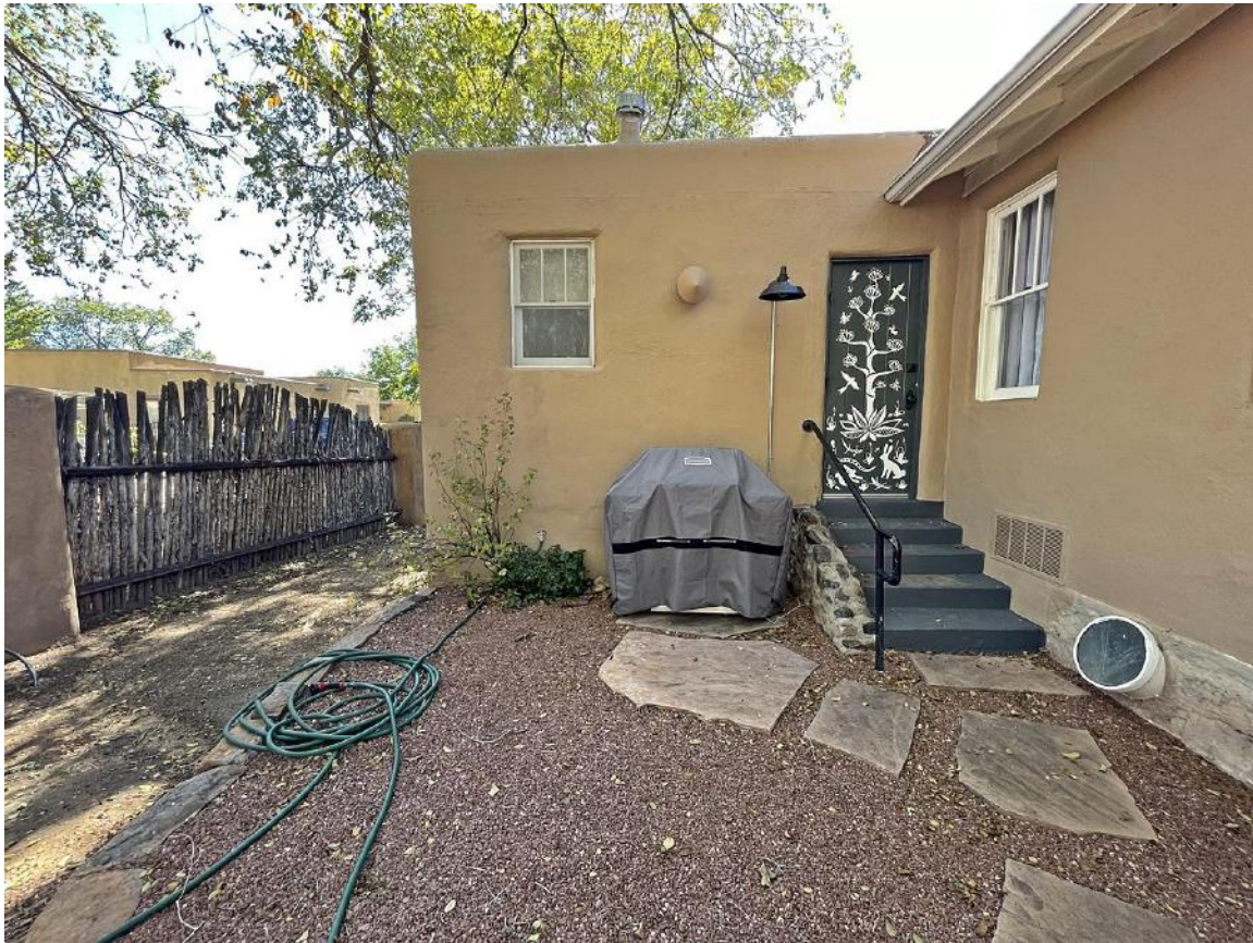
Photo 12: Addition, north elevation. Camera facing south.
