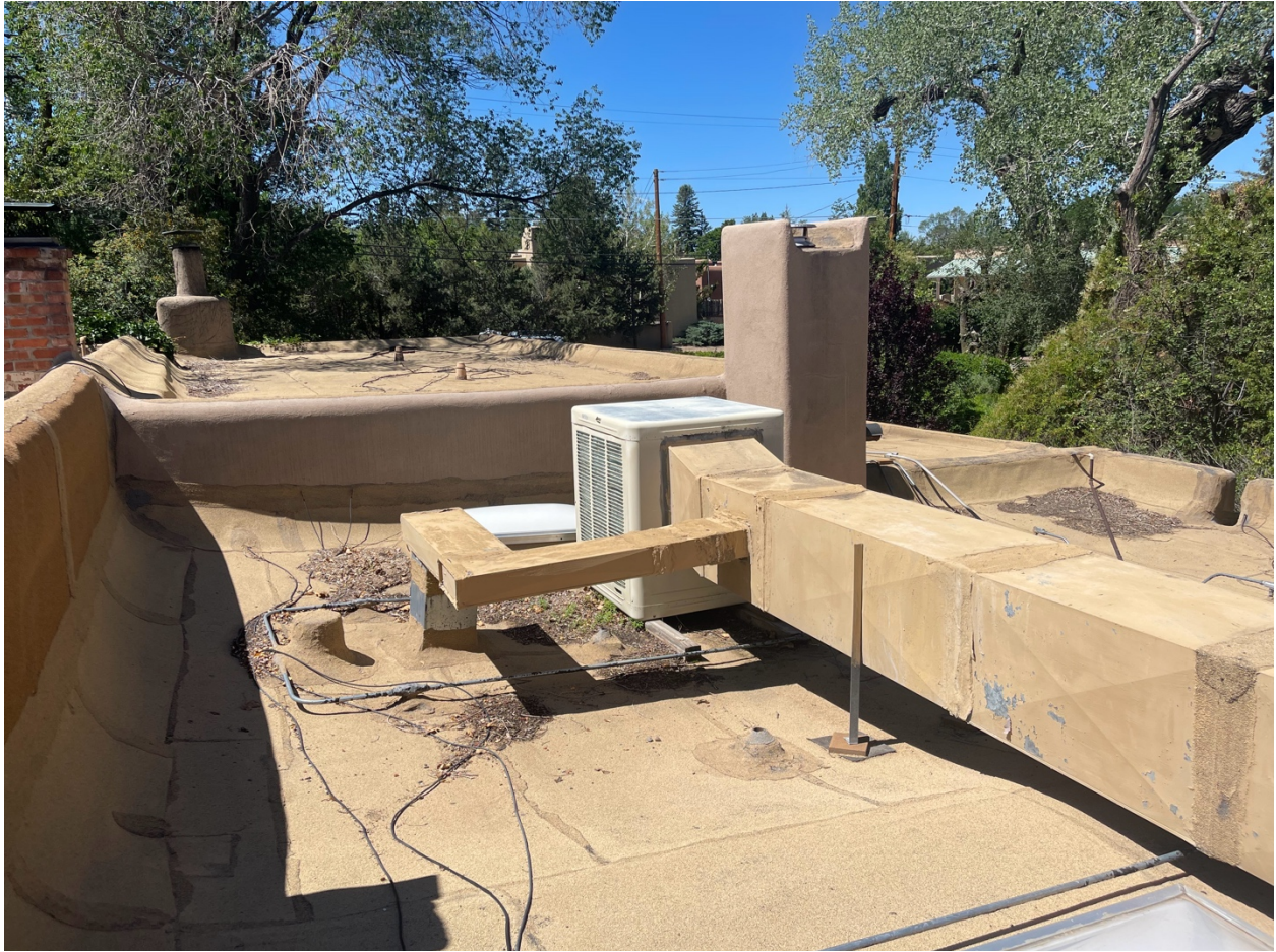
Roof top view looking south
