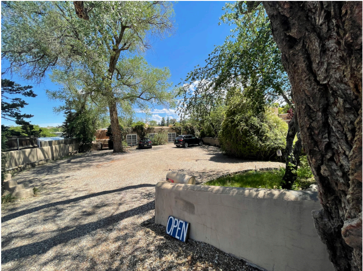
View from Canyon Road. This wall appears in the 1978 Aerial photos. The structure is 3-4' below Canyon Road.
