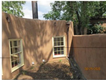
WEST VIEW COURTYARD
