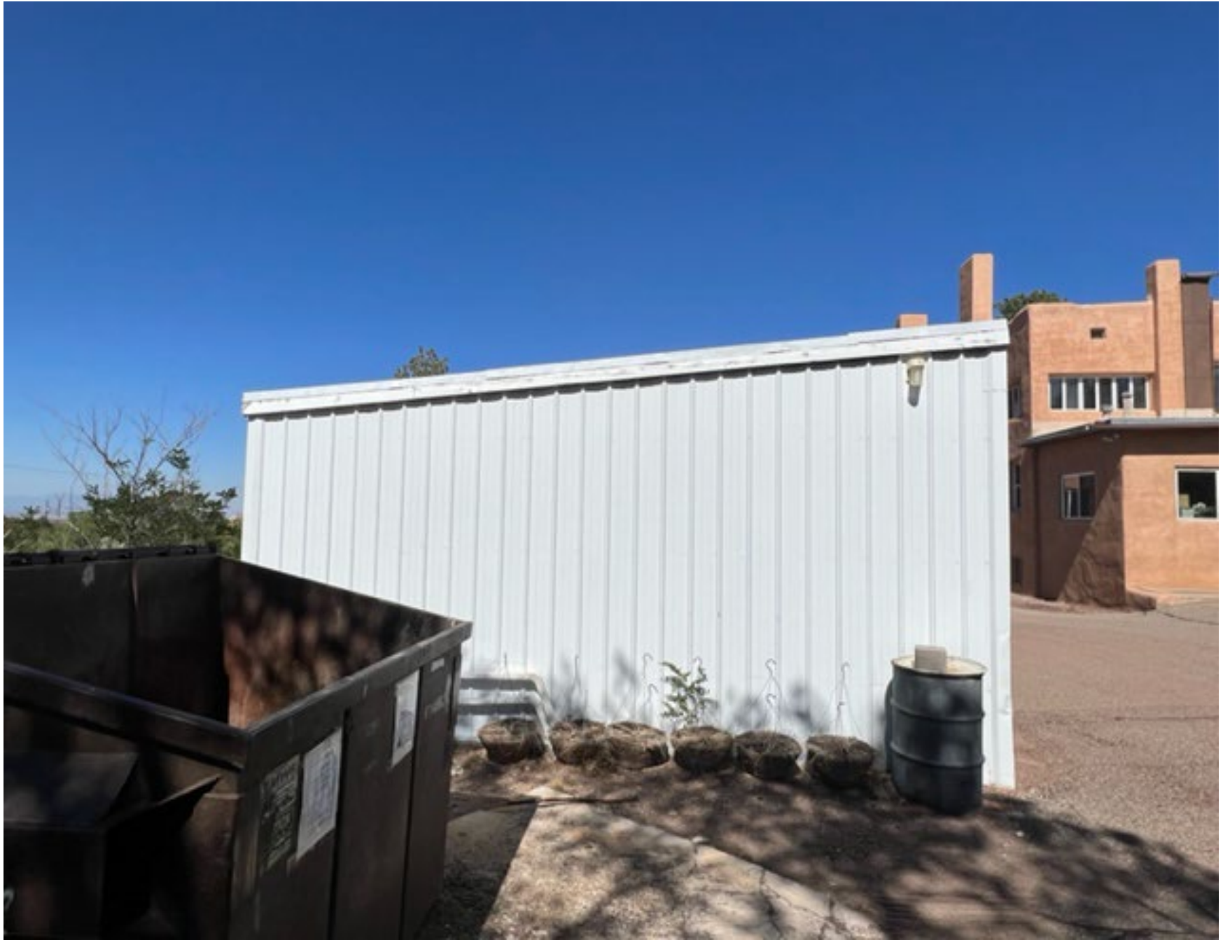
Carport/Shed – East façade
