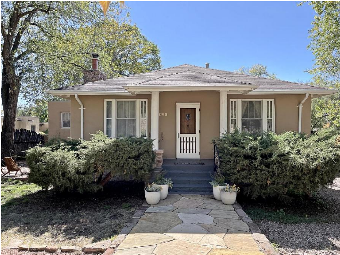
Photo 1: Front (north) façade. Camera facing south.
