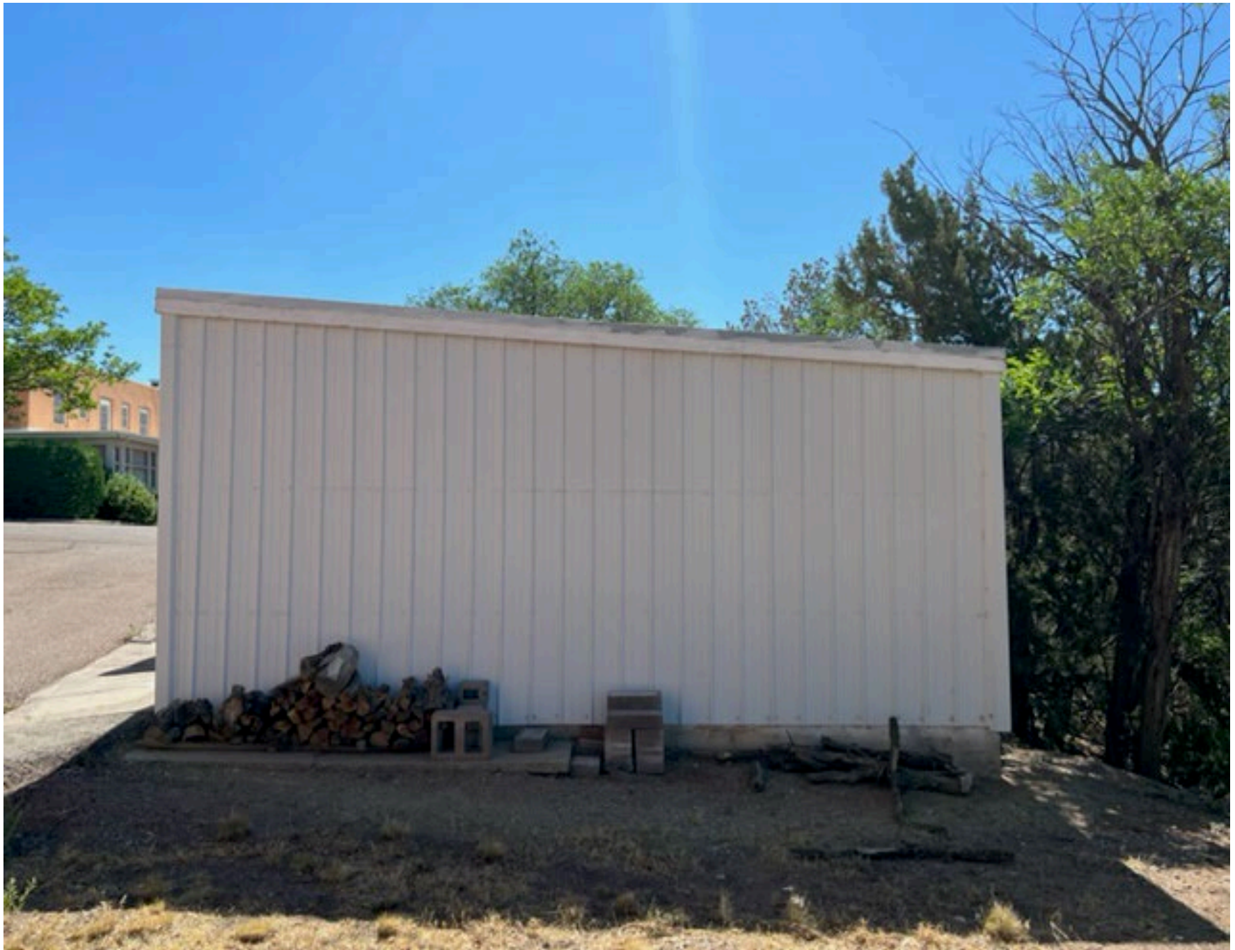
Carport/Shed – West façade
