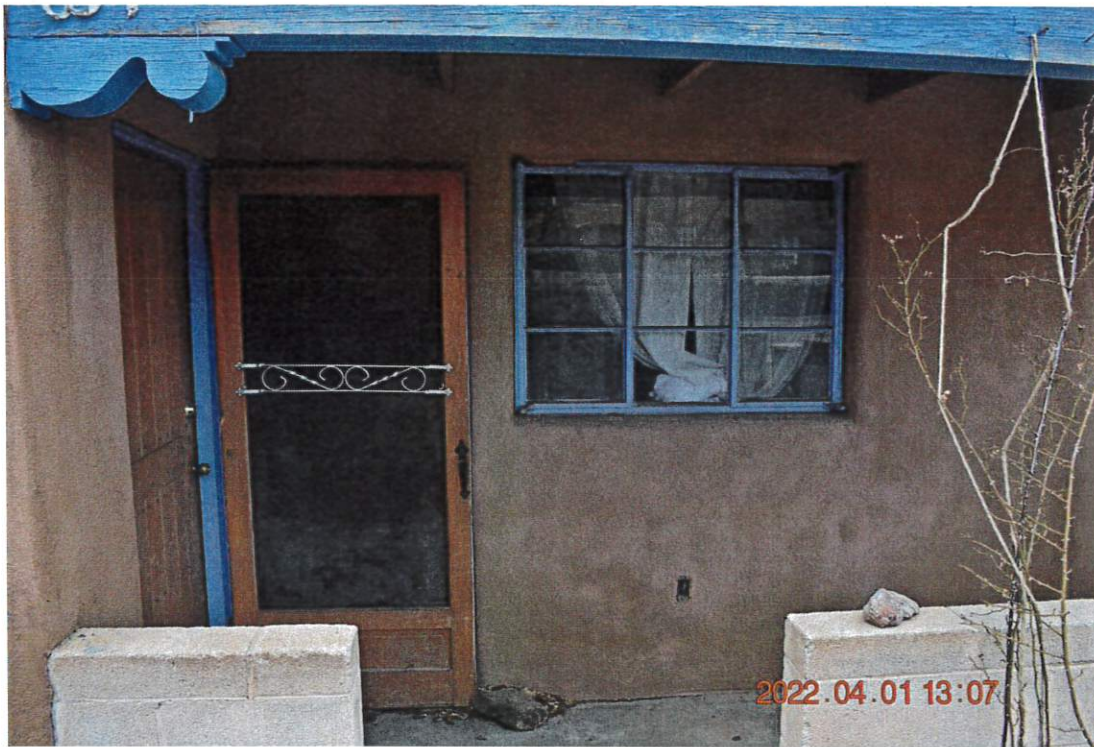
Photo 2: Front (east) façade. Portal. Camera facing west.
