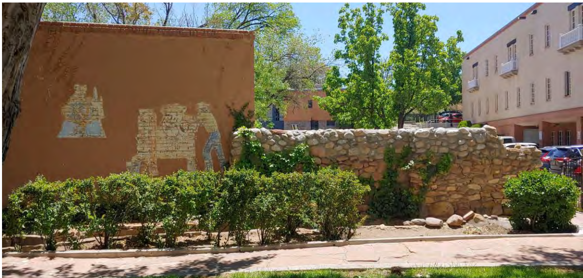
Photo 12: Potentially older stone wall at northwest corner. Camera facing south.
