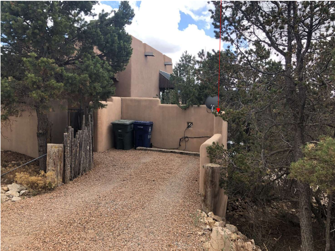
Fig. 2 Main Residence – North Façade (streetscape) at Camino Militar. The façade the height is approx. 14'.
