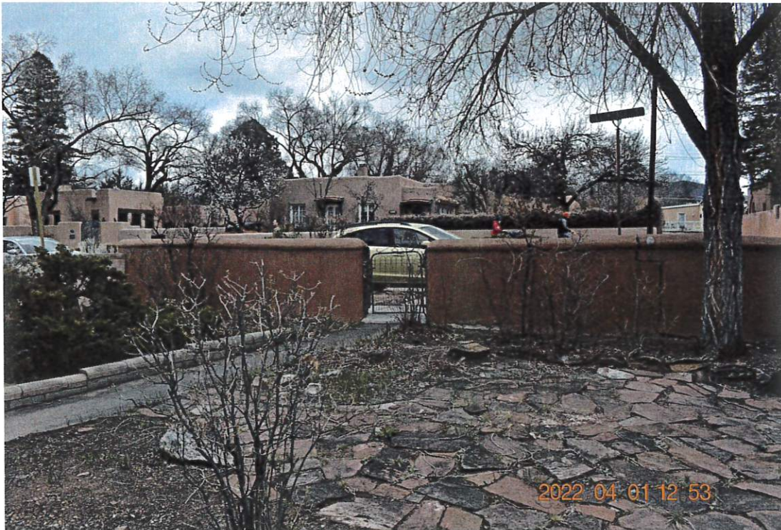
Photo 12: Front Wall. Camera facing northeast.
