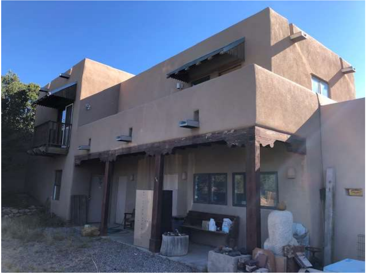
Fig. 6 Main Residence – West Façade (max height at 24')
