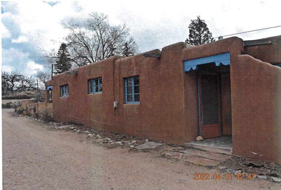
Photo 3: View of north elevation. Camera facing southeast.
