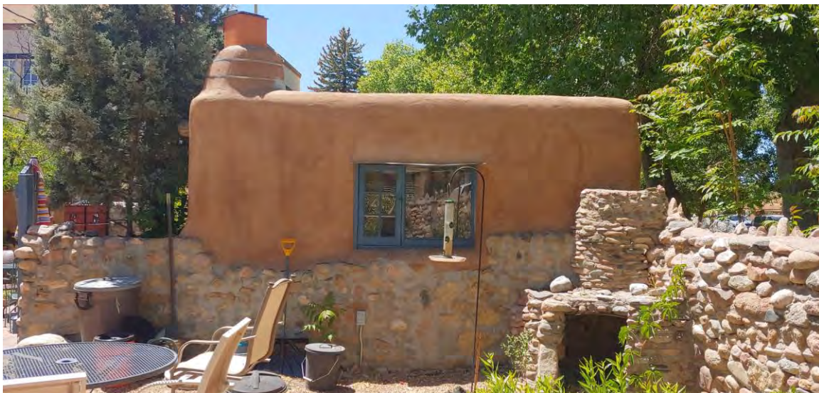
Photo 6: Cider Press, east elevation, c.1950s addition. Camera facing west.
