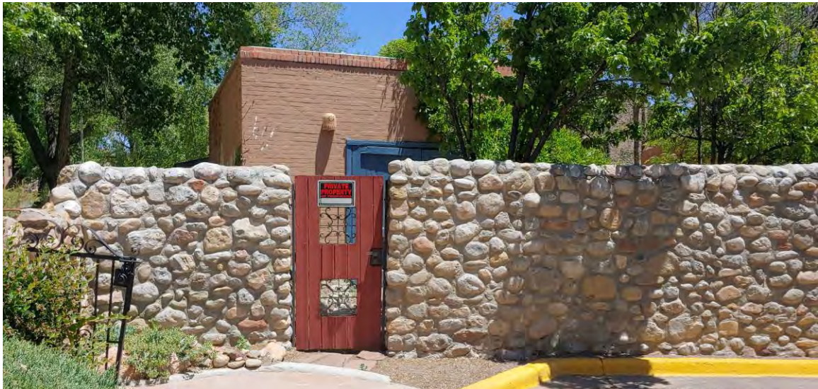
Photo 11: Post-1988 stone wall in front of Cider Press. Camera facing east.
