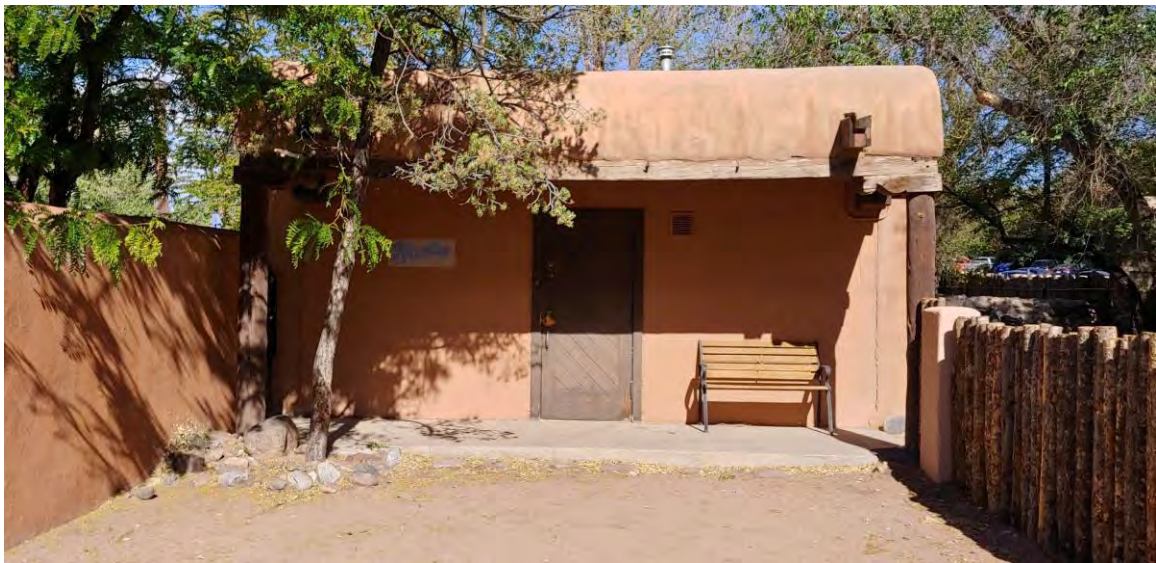
Photo 8: Studio, west (front) elevation. Camera facing east.
