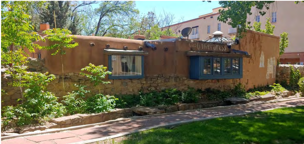
Photo 7: Cider Press, north elevation, full façade. Camera facing southwest.
