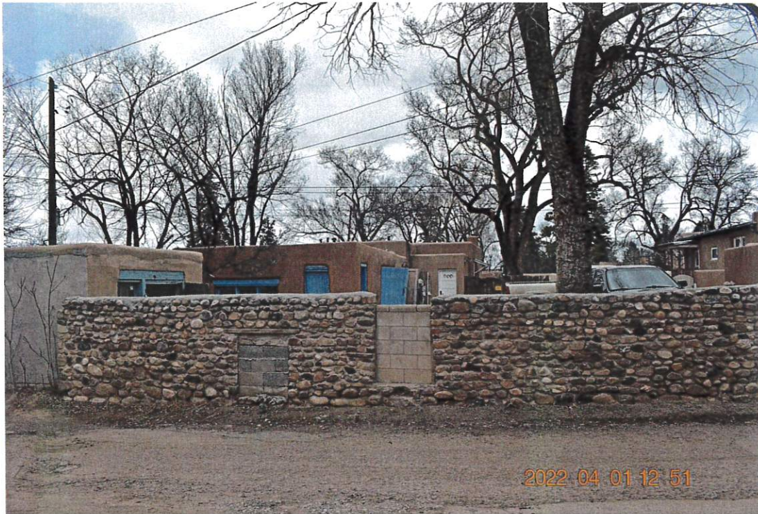
Photo 11: Alley Wall. Blocked in openings. Camera facing north.
