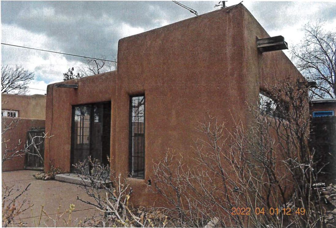
Photo 5: West and south elevations. Post-1983 dining room addition at right. Camera facing northwest.
