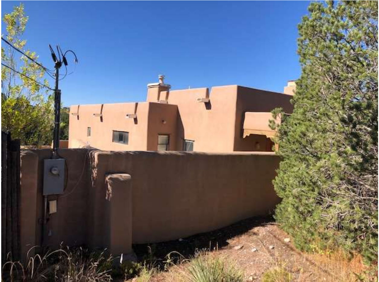
Fig. 3 Main Residence - North Façade (streetscape) at Camino Militar
