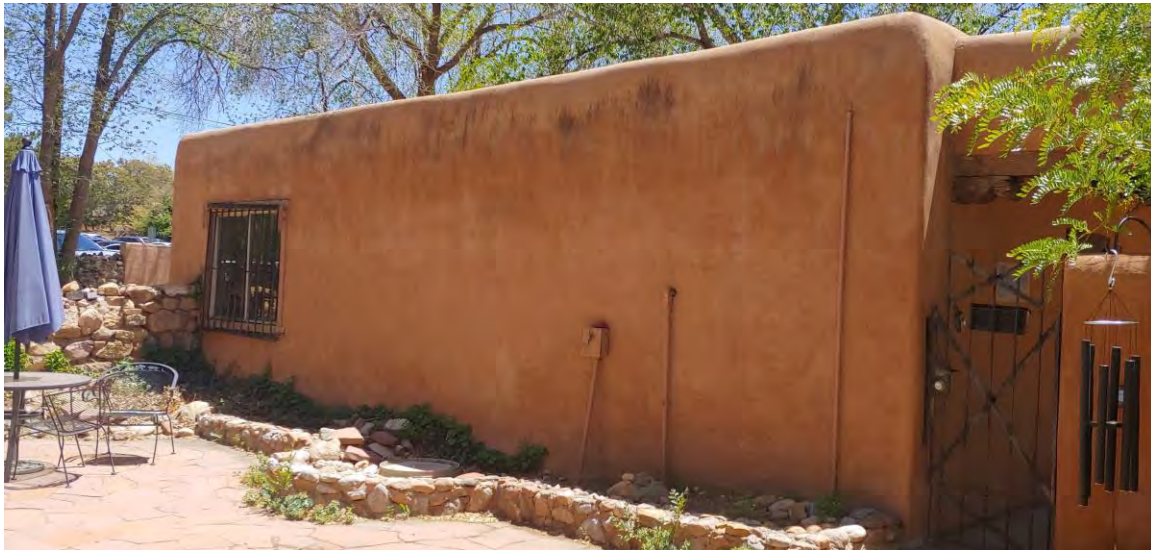
Photo 9: Studio, north elevation Camera facing southeast.
