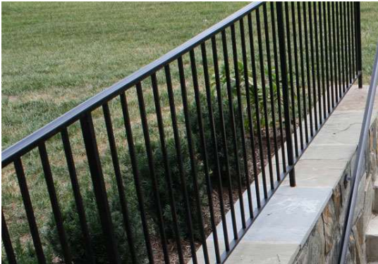
Fig. 12 Power coated metal railing attached between stucco walls at west portal
