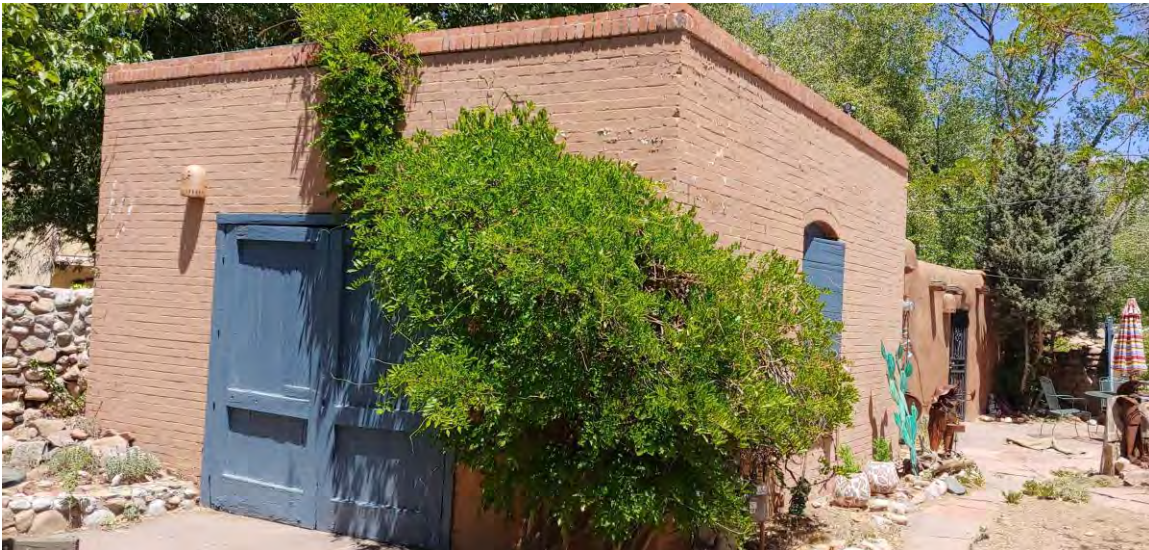
Photo 4: View of Cider Press, west and south elevations, original garage portion. Camera facing northeast.
