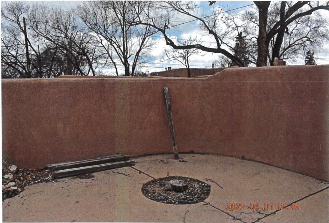
Photo 14: Back Wall. Camera facing northwest.
