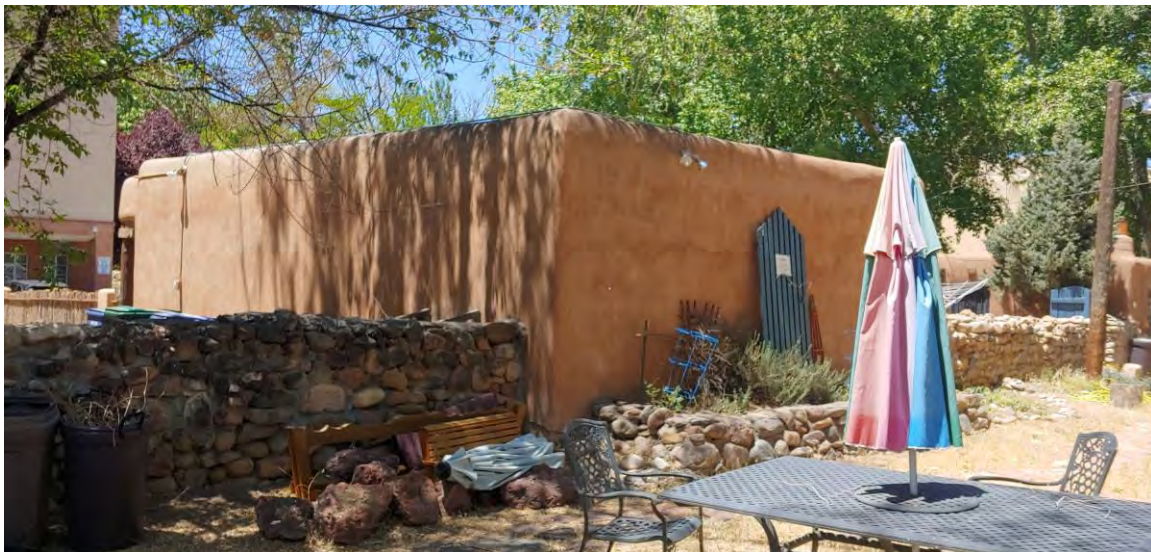
Photo 10: Studio, south and east elevations. Camera facing southwest.
