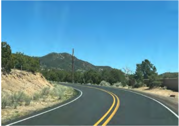
Figure 18. Old Santa Fe Trail is a two-lane roadway that has rural design features and several curves along the corridor. Chevrons and advanced curve warning signs are not located
