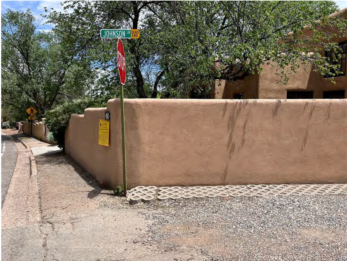
Photo 13: Garcia Street and Johnson Lane walls. Camera facing north.
