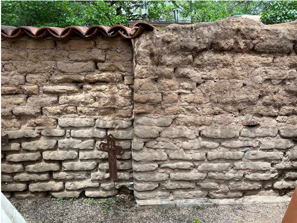
Photo 14: Adobe wall on adjacent property. Camera facing north.
