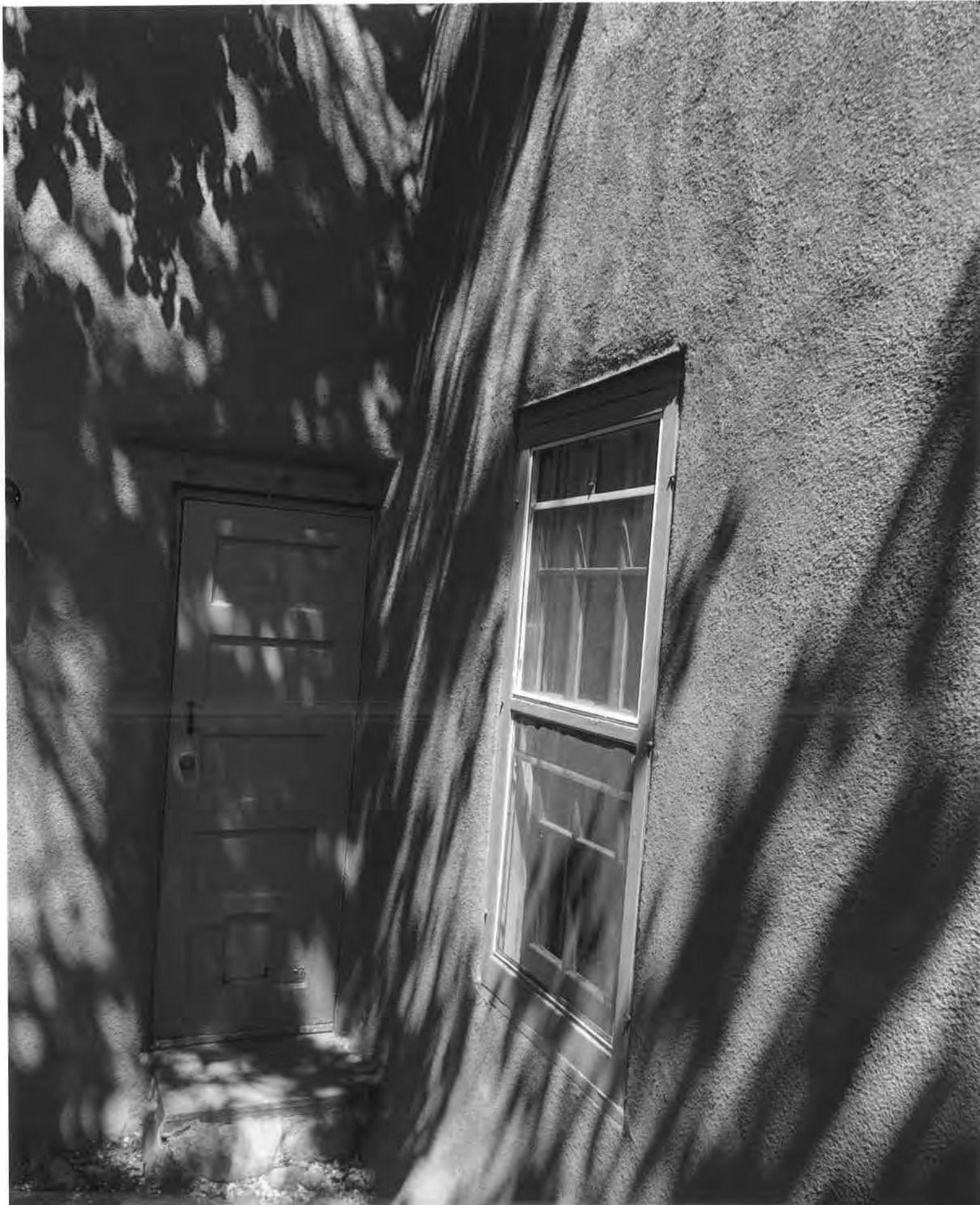
634 GARCIA #19-EAST & NORTH ELEVATION BACK PATIO
