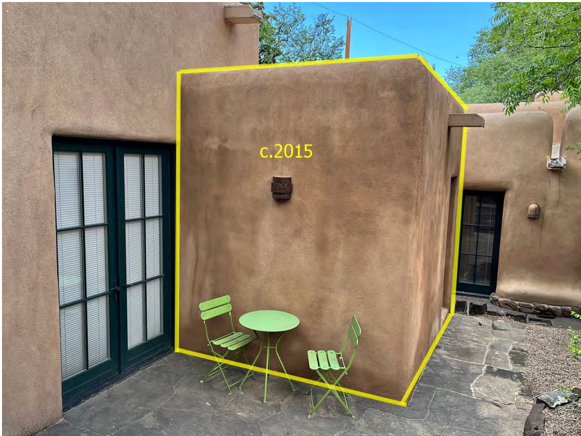
Photo 9: North, 2015 addition highlighted. Camera facing southwest.
