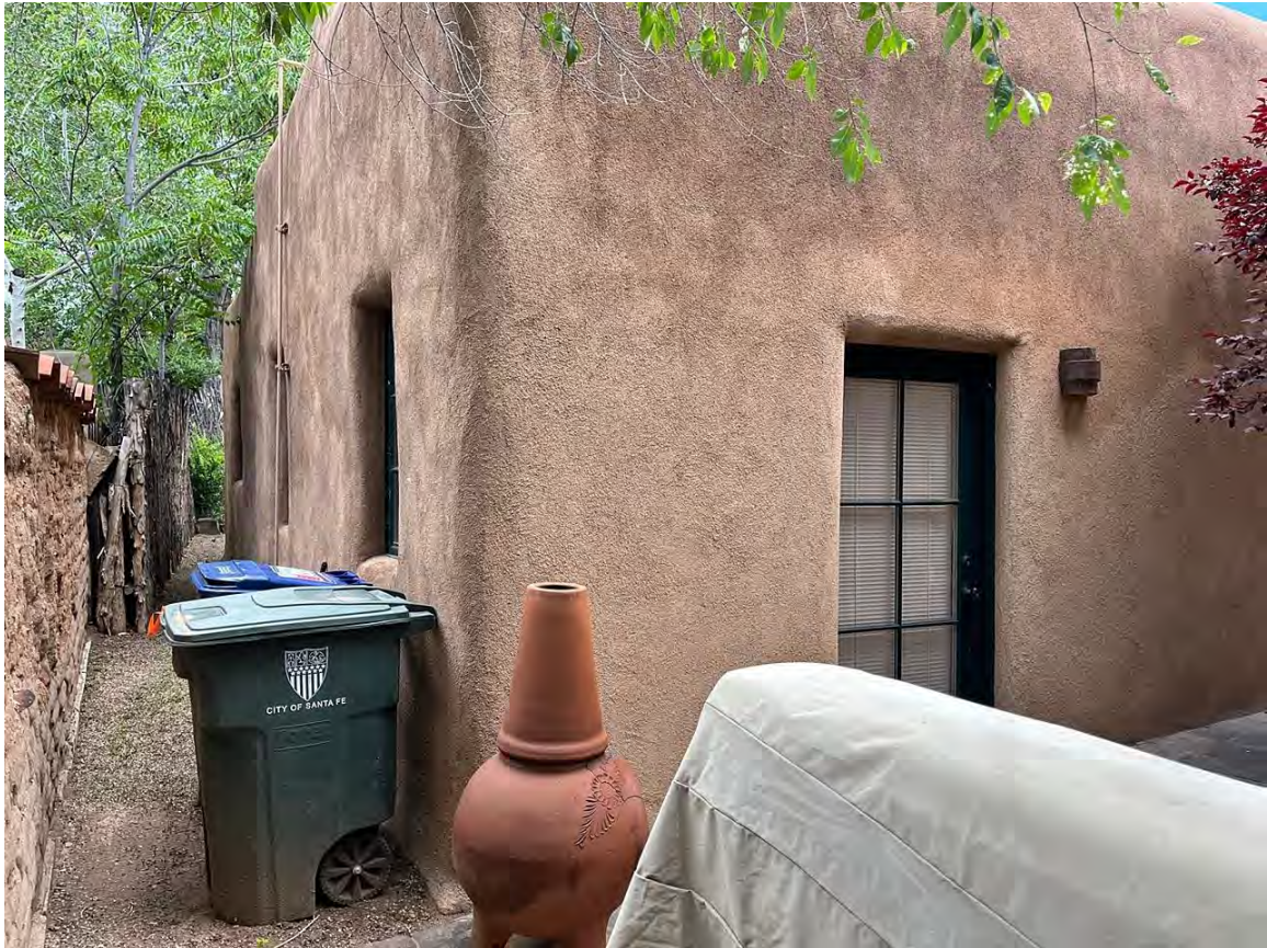
Photo 11: North elevation. Camera facing east.
