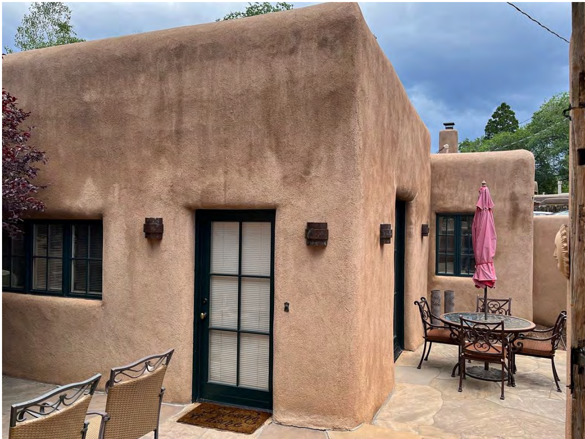
Photo 4: Partial west elevation. Camera facing east.
