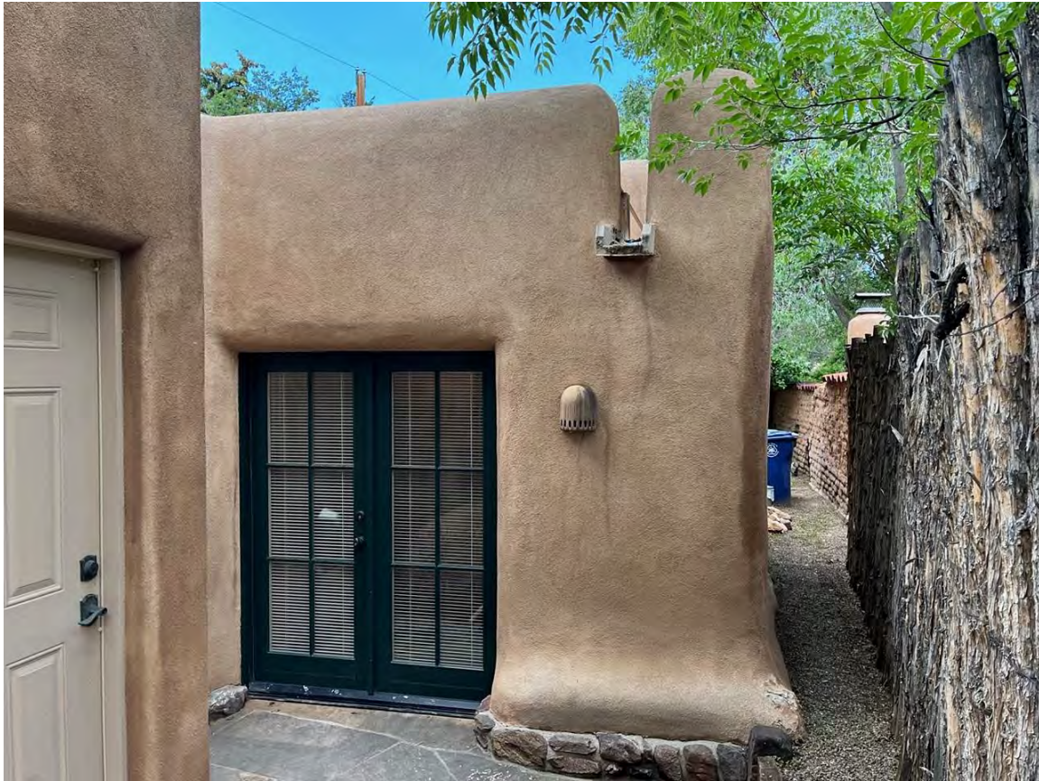
Photo 10: North elevation, 2015 addition at left. Camera facing southwest.
