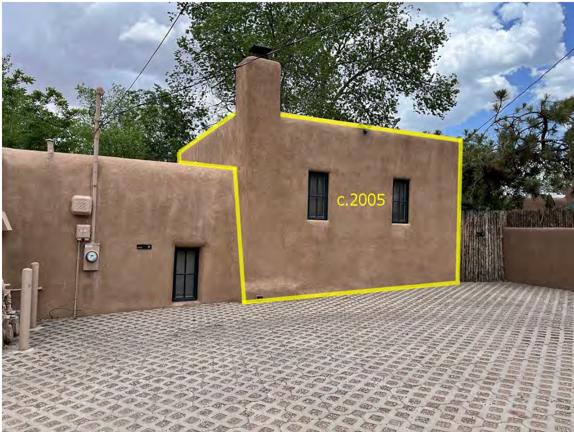
Photo 7: South elevation, upper section, 2005 addition highlighted. Camera facing northeast. June 16, 2022.
