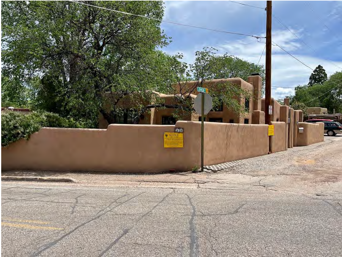
Photo 3: Full south elevation, viewed from Garcia Street. Camera facing east.
