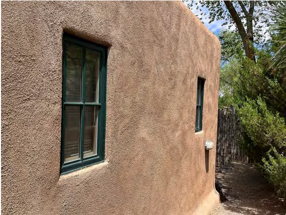
Photo 8: 2005 east elevation. Camera facing northwest.
