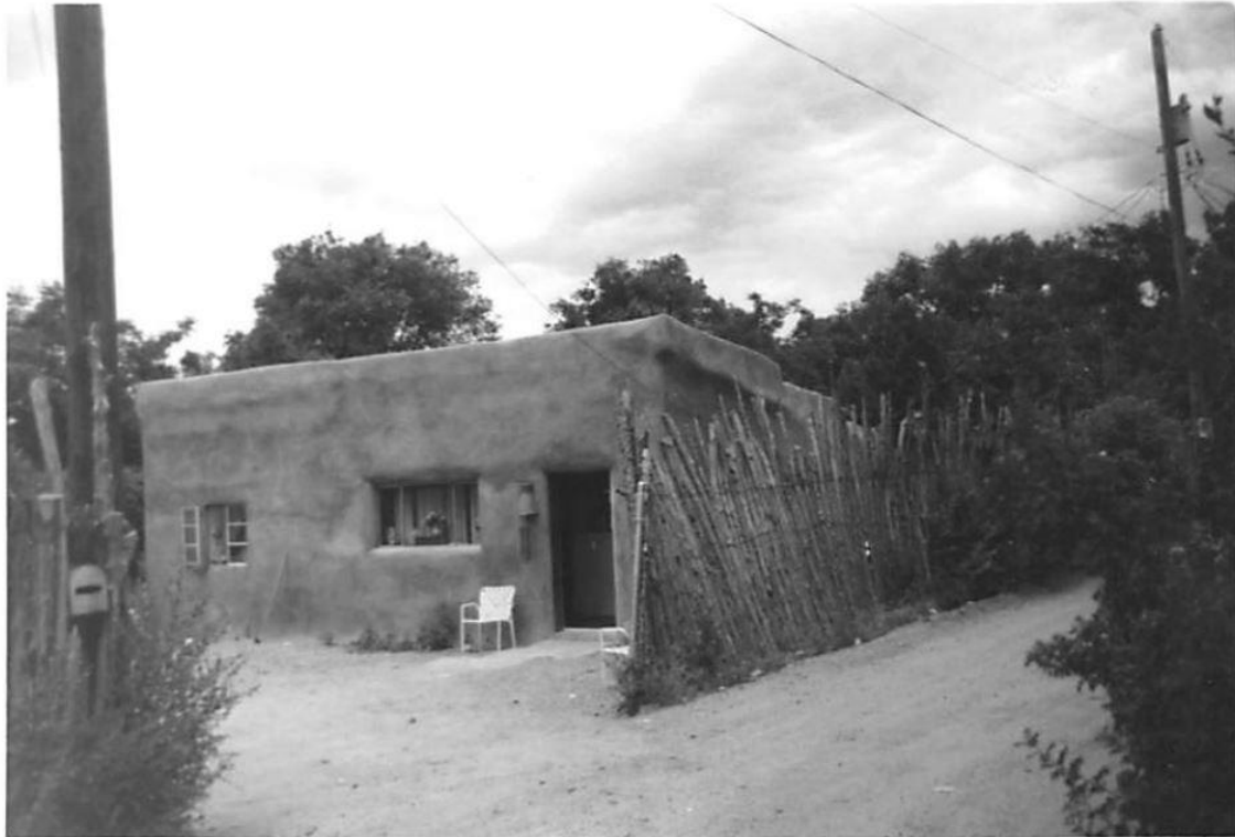
Figure 2: West façade, 1993. August 30, 1993, Historic Building Inventory.
