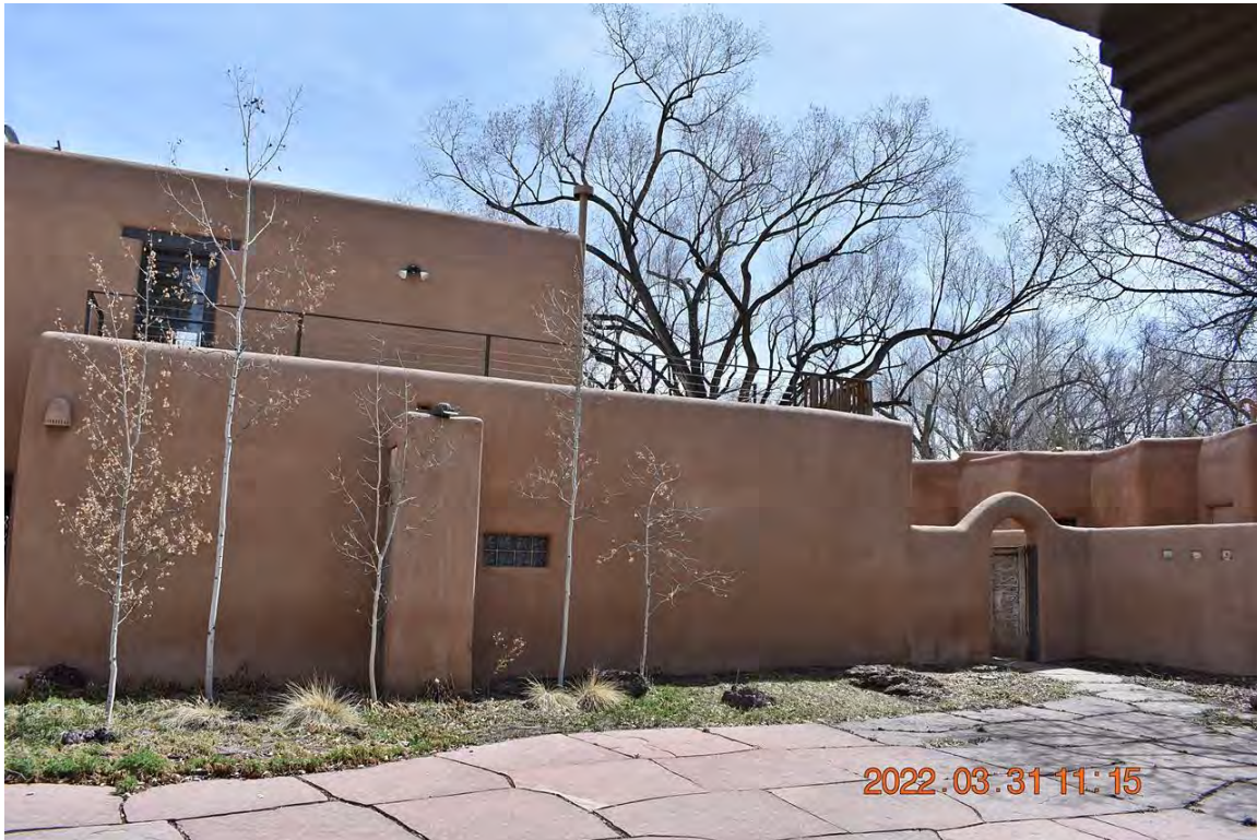
Photo 18: East Wing, west elevation. Camera facing southeast.
