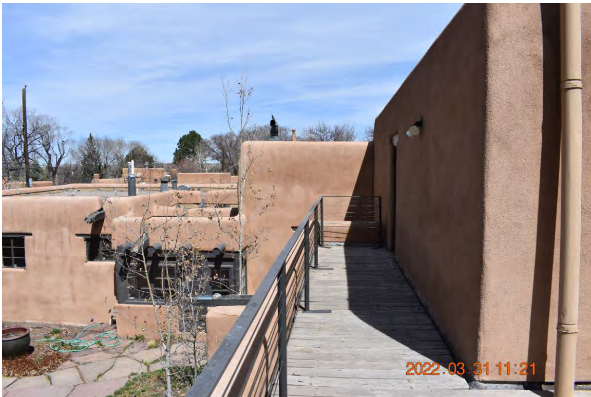
Photo 11: East Wing, west elevation. Balcony. Camera facing north.
