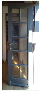
WOOD UPSTAIRS BALCONY DOOR
