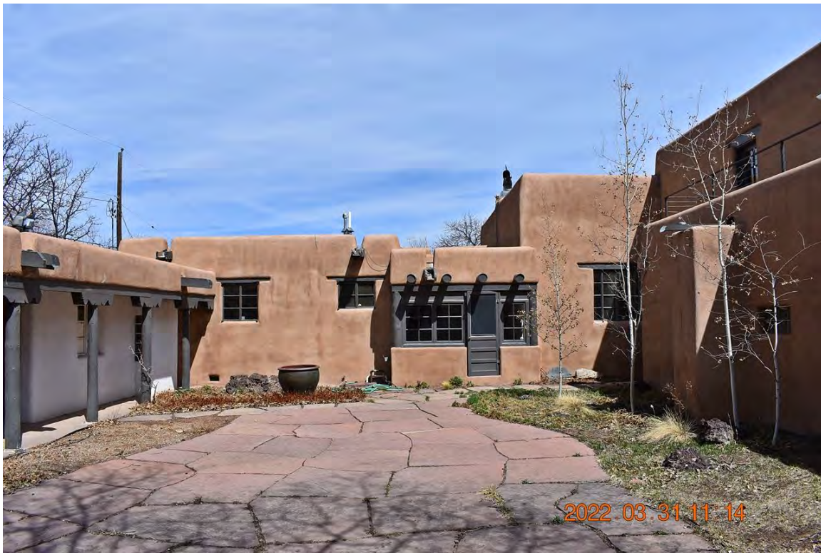
Photo 12: Courtyard. 1950s Casita (left), original 1942 home (center), 1950s East Wing (right). Camera facing north.
