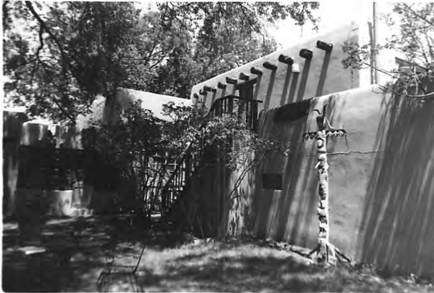
#1 E. facade of courtyard
