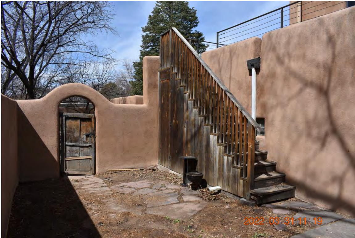
Photo 10: East Wing, south elevation. Stairs. Camera facing west.
