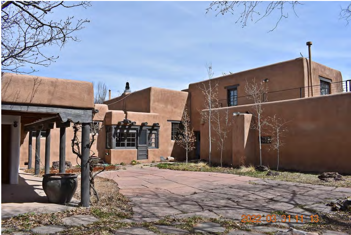
Photo 13: Courtyard. Camera facing southeast.
