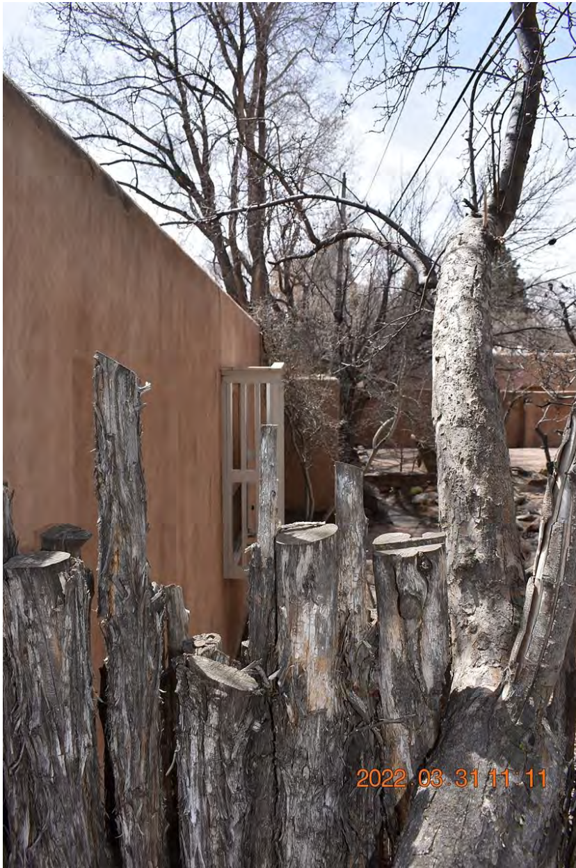
Photo 14: Casita, west elevation. Camera facing south.
