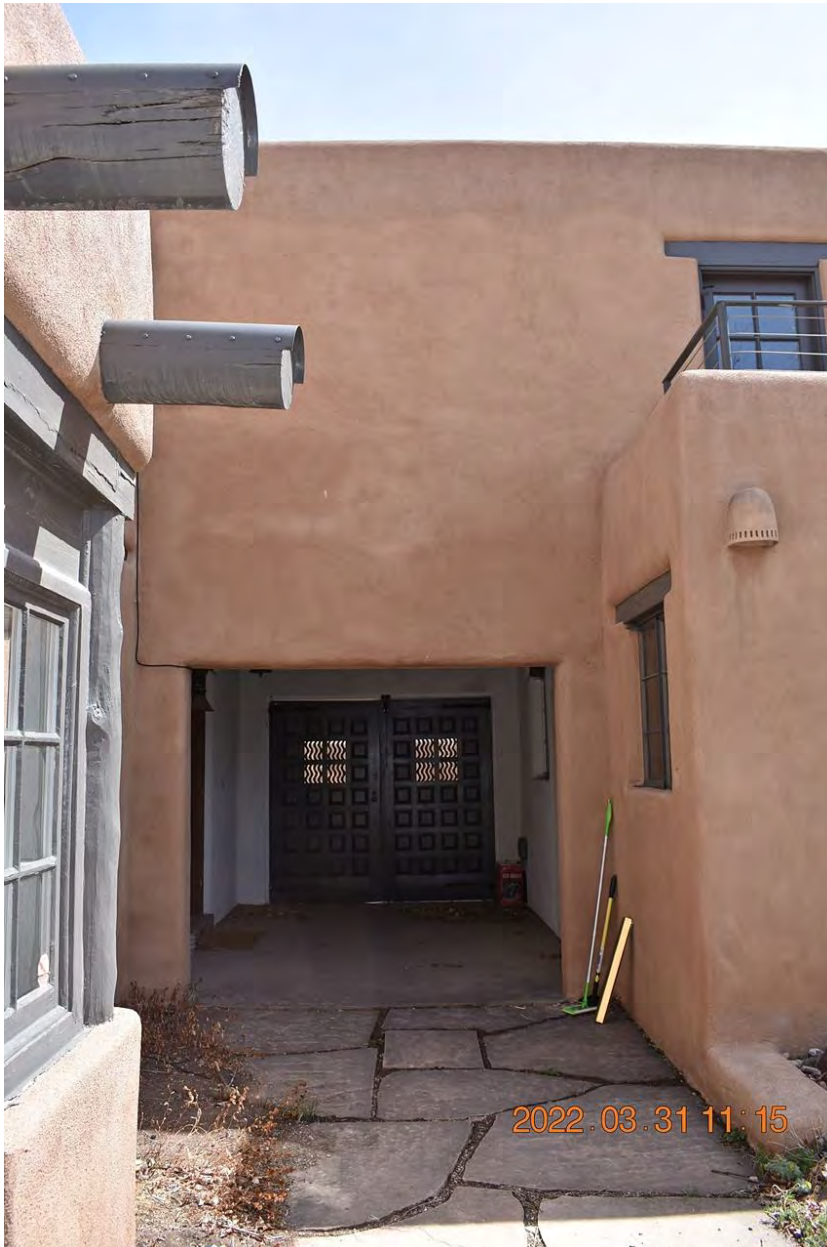
Photo 17: East Wing, west elevation. Zaguan. Camera facing east.
