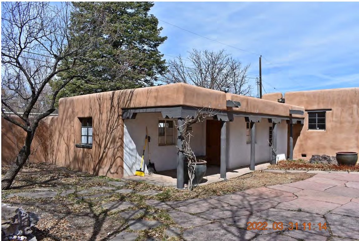
Photo 14: Casita, south and east elevations. Camera facing northeast.
