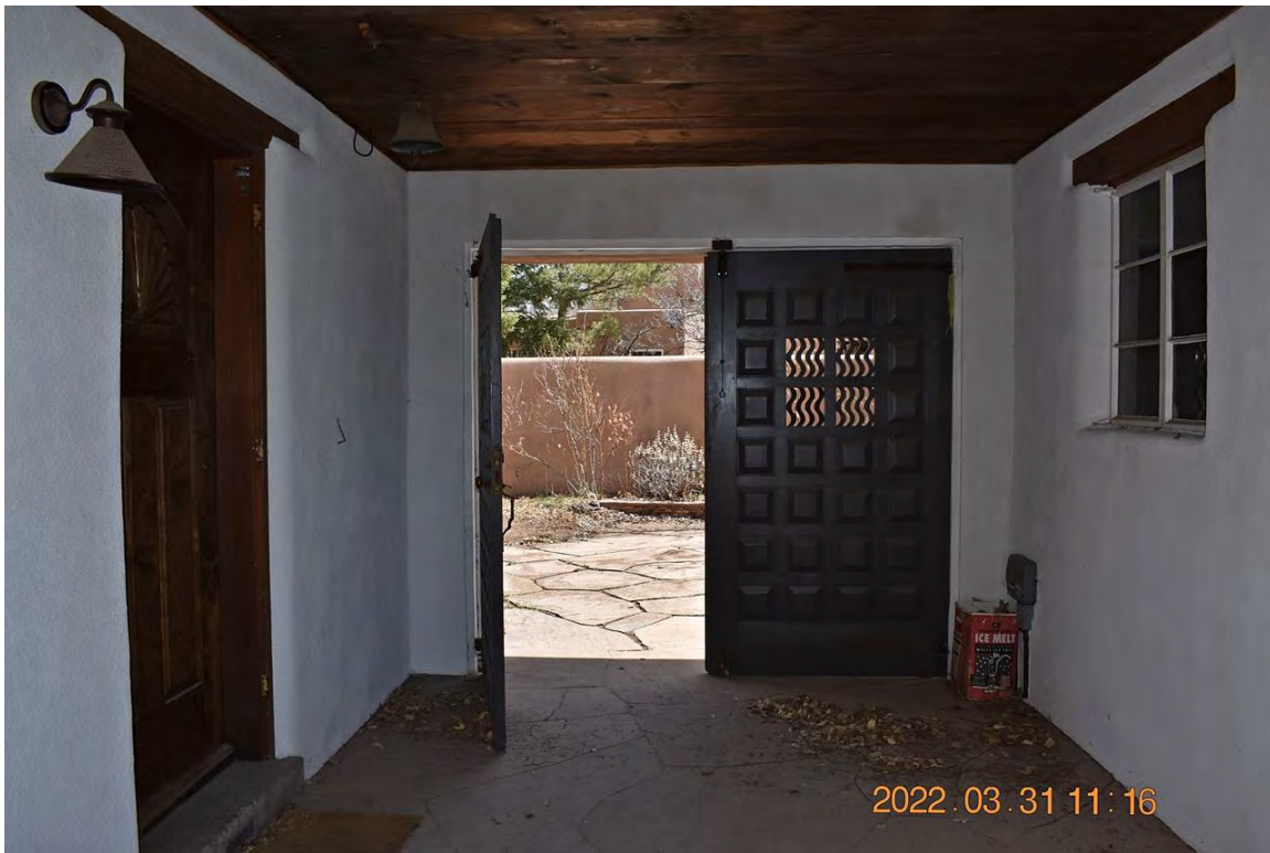
Photo 7: East Wing. Zaguan. Camera facing east.
