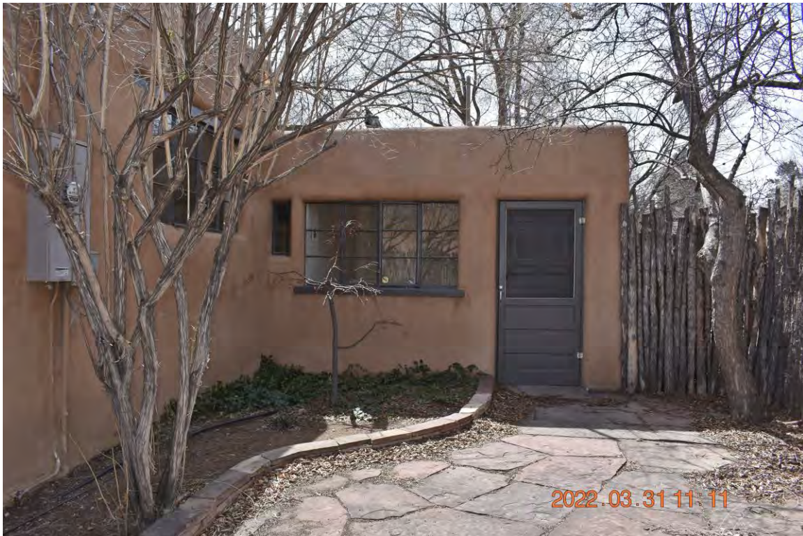
Photo 1: Casita, north elevation. Camera facing south.
