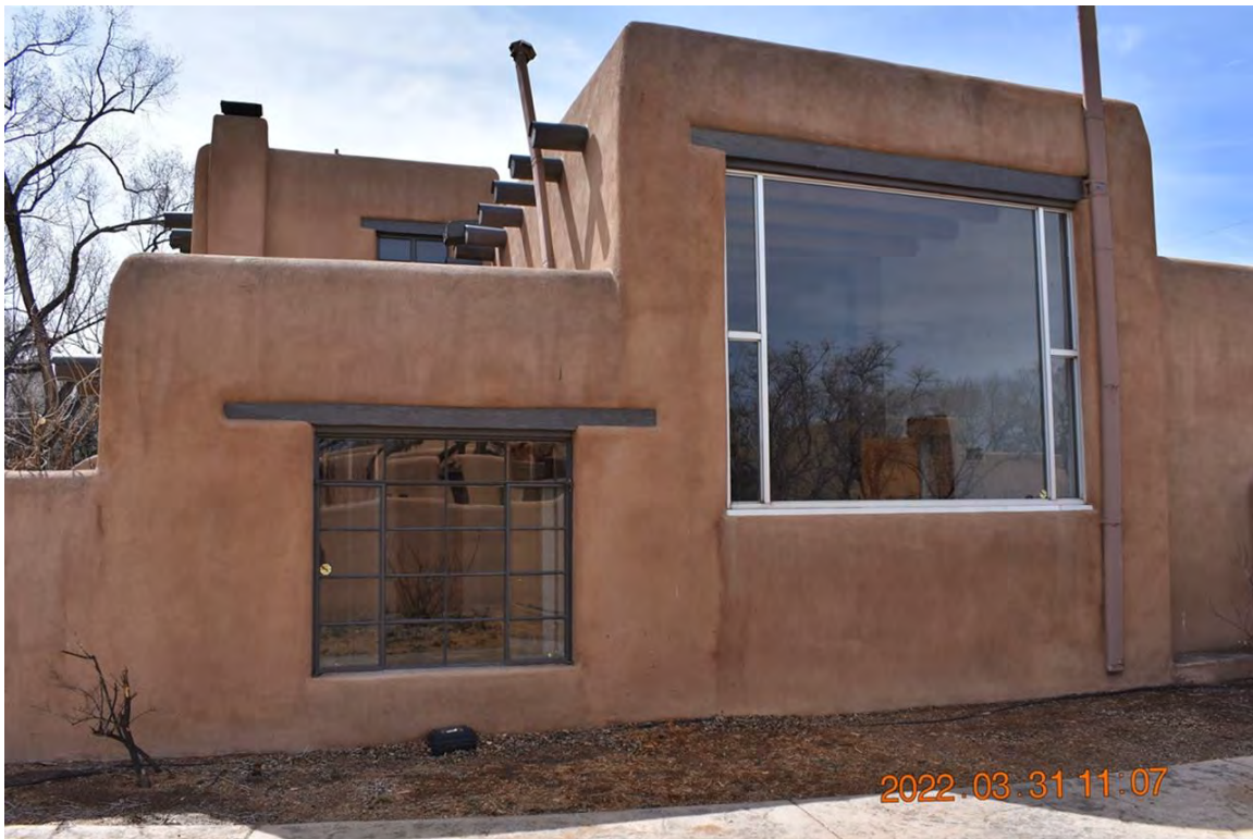
Photo 4: View of north elevation. Studio room (right), post-1958 enclosure (left). Camera facing southwest.
