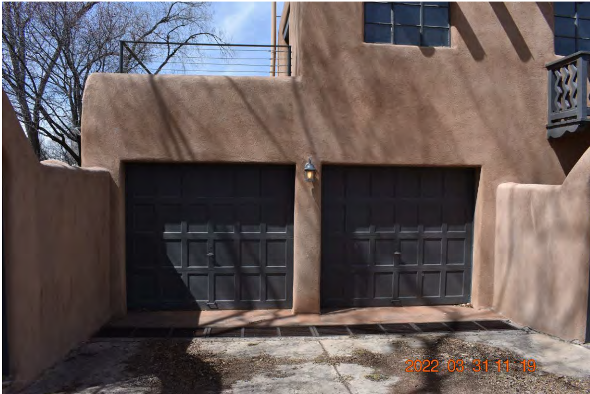
Photo 9: East Wing, east elevation. Garage. Camera facing west.
