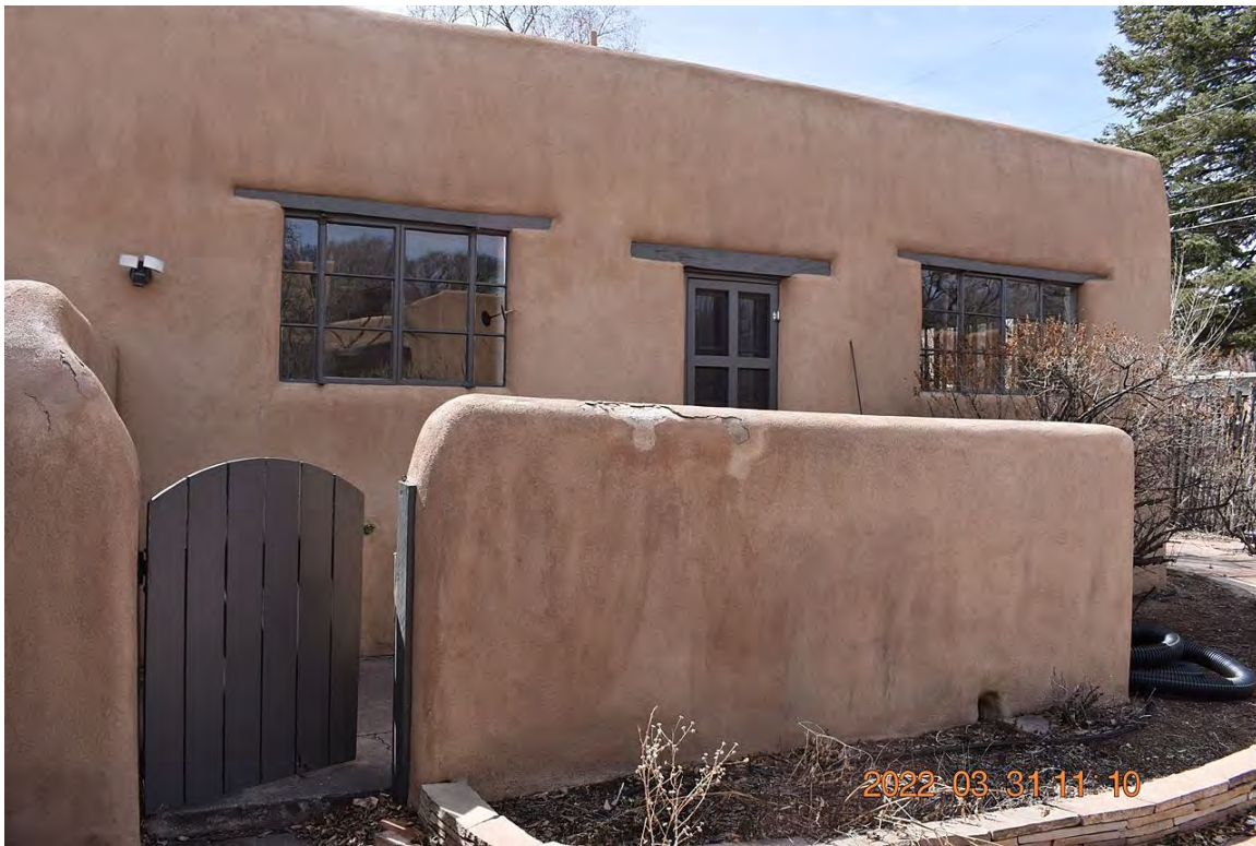
Photo 3 North elevation. 1942 section. Camera facing southwest.
