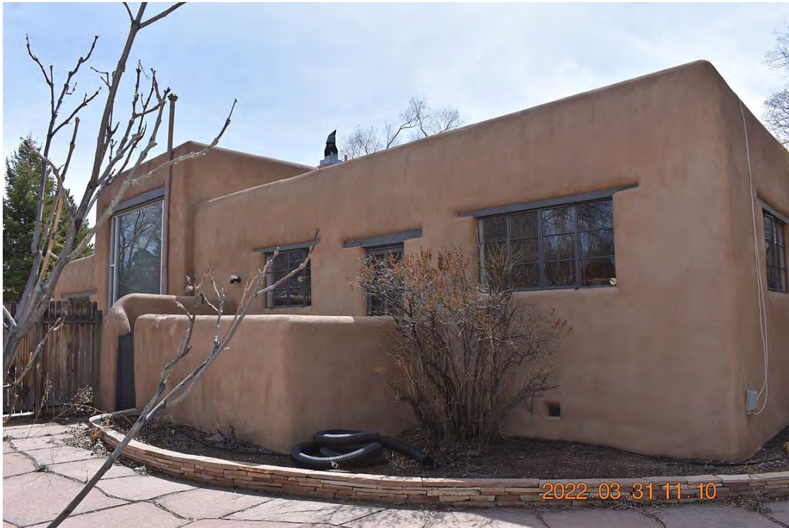
Photo 2: North elevation. 1942 house in foreground. Camera facing southeast.
