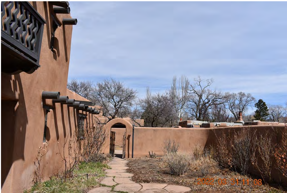
Photo 6: East Wing, east elevation. Courtyard. Camera facing north.
