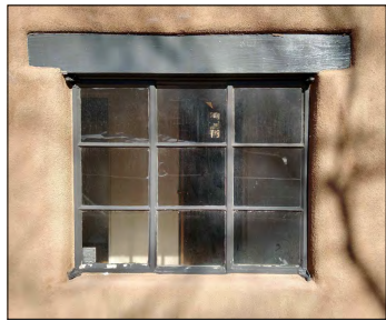
STEEL WINDOW WITH LINTEL
