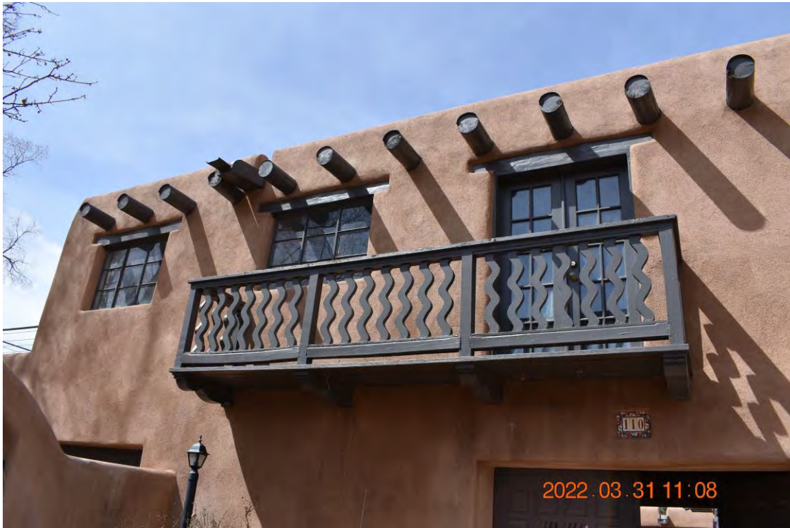
Photo 8: East Wing, east elevation. Balcony. Camera facing up.
