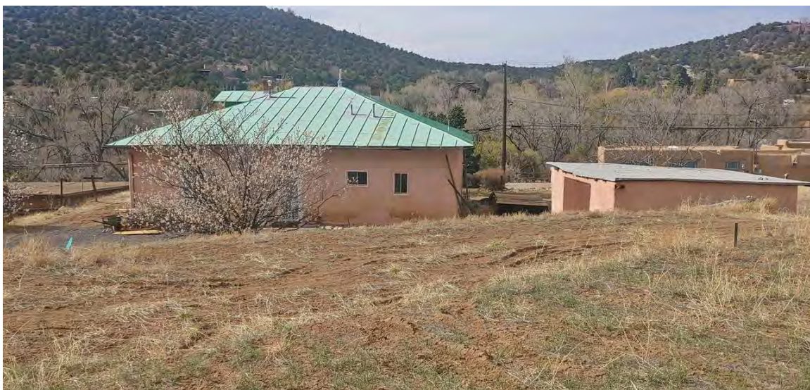
Photo 2: House and garage. Camera facing north.
