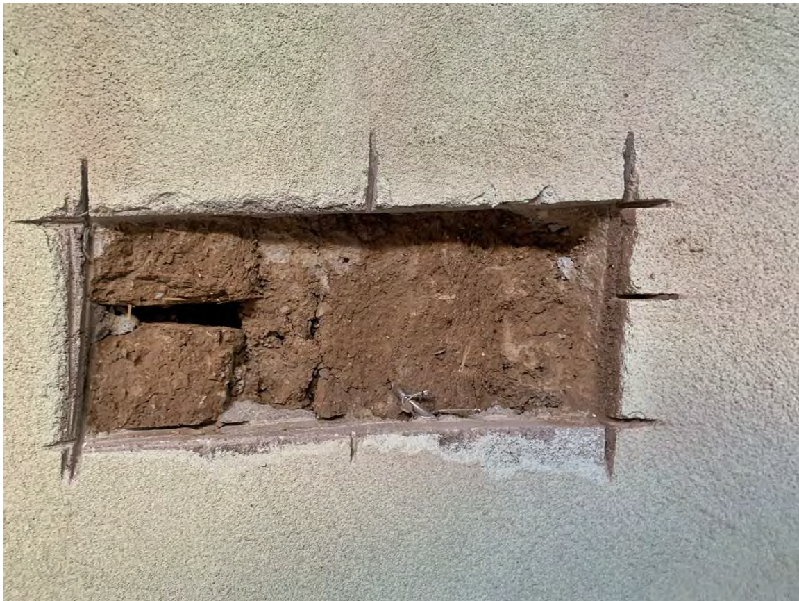
Photo 11: Interior, south wall, core sample (adobe). William Powell. May 3, 2022.
