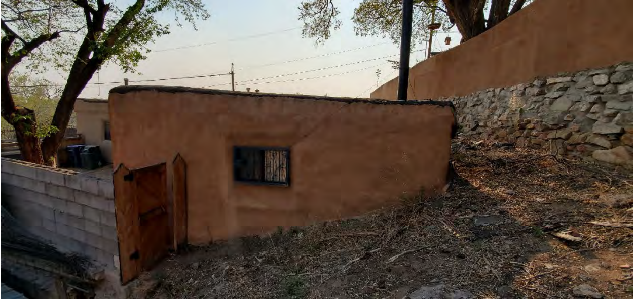
East Elevation – from adjacent property
