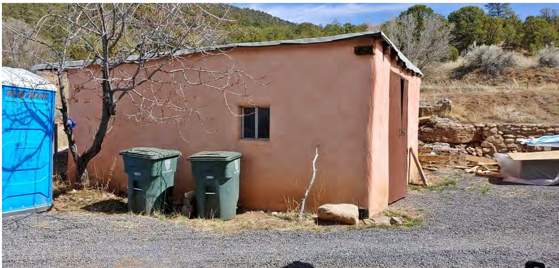
Photo 4: North and west elevations Camera facing southeast.
