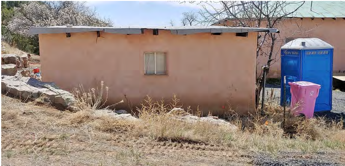
Photo 5: East elevation. Camera facing west.
