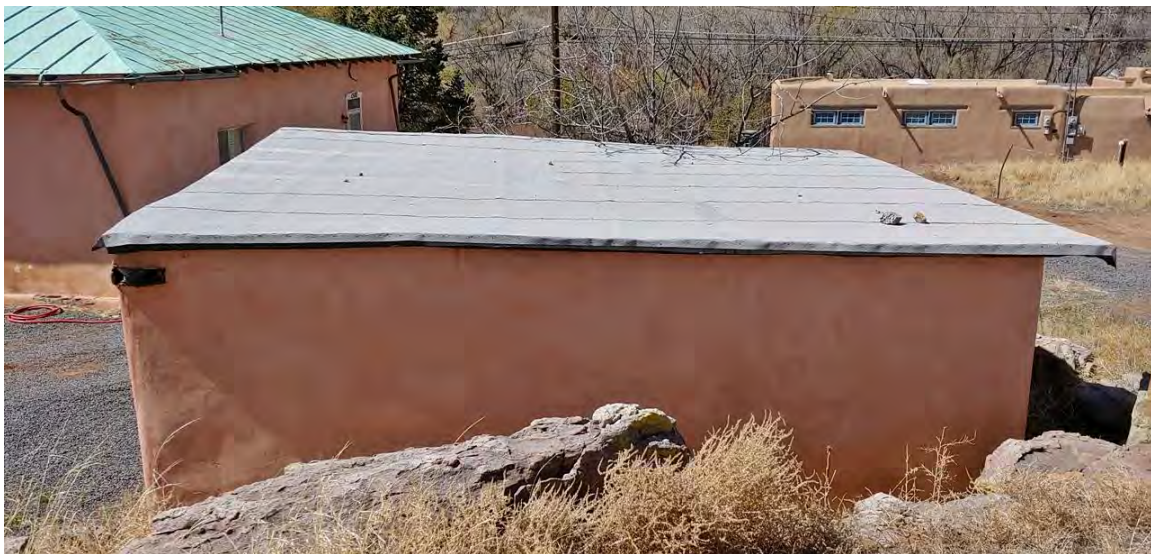
Photo 6: South elevation. Camera facing north.
