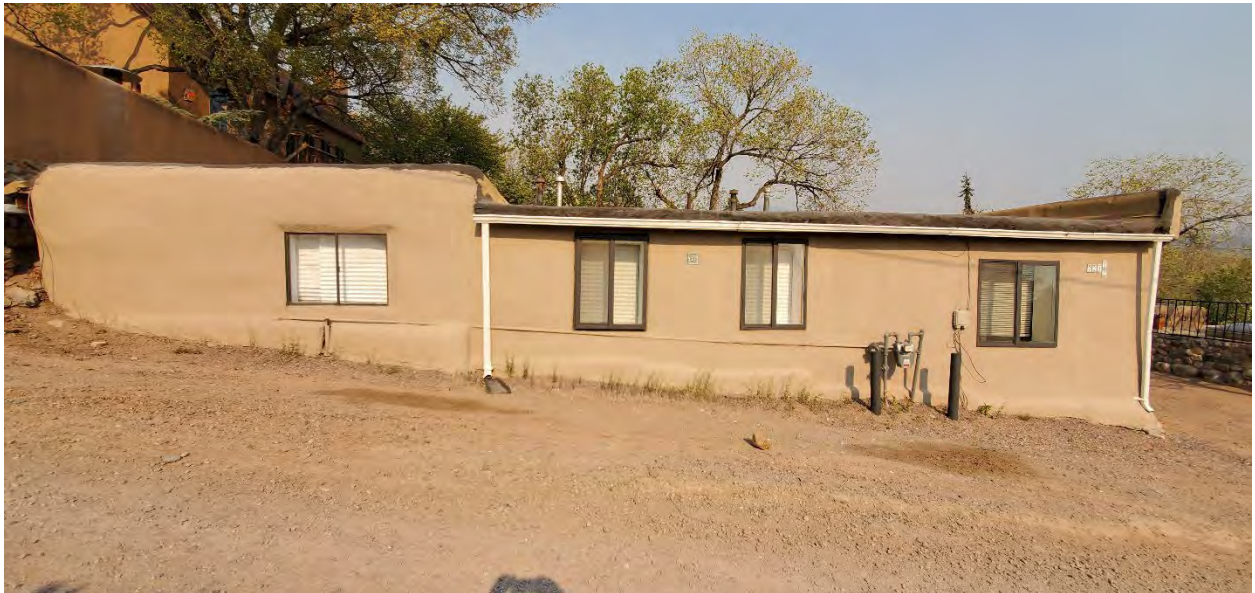
West Elevation – on Rodriguez Street
