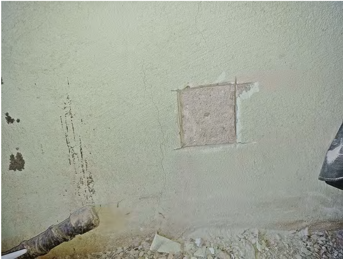
Photo 10: Interior, north wall, core sample (CMU). Richard Horcasitas. April 30, 2022.
