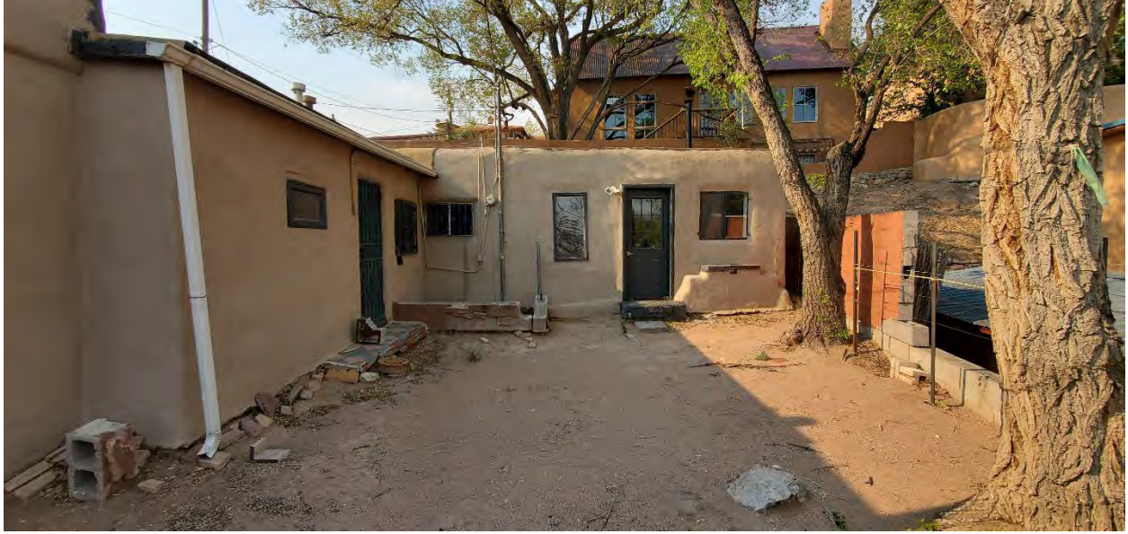
South Elevation – inside the east courtyard
