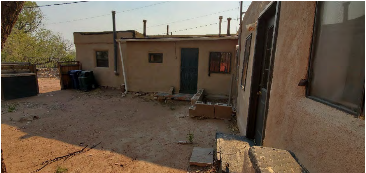
East Elevation – inside the east courtyard
