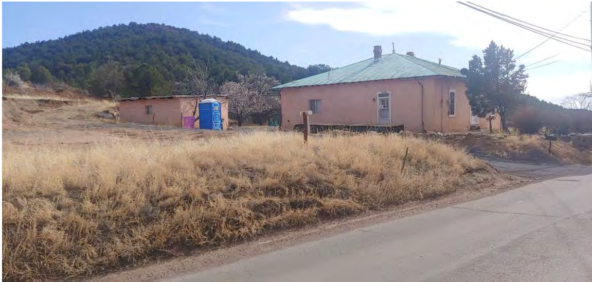
Photo 3: View of publicly visible façades from Upper Canyon Road. Camera facing southwest.
