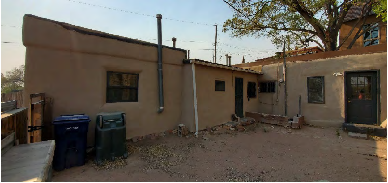
East Elevation – inside the east courtyard
