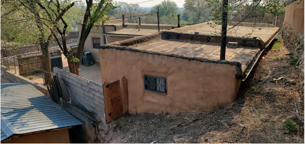
East Elevation – from adjacent property
