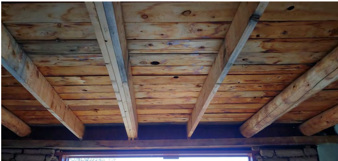
Photo 8: Roof structure and decking. Camera facing up toward west elevation opening.
