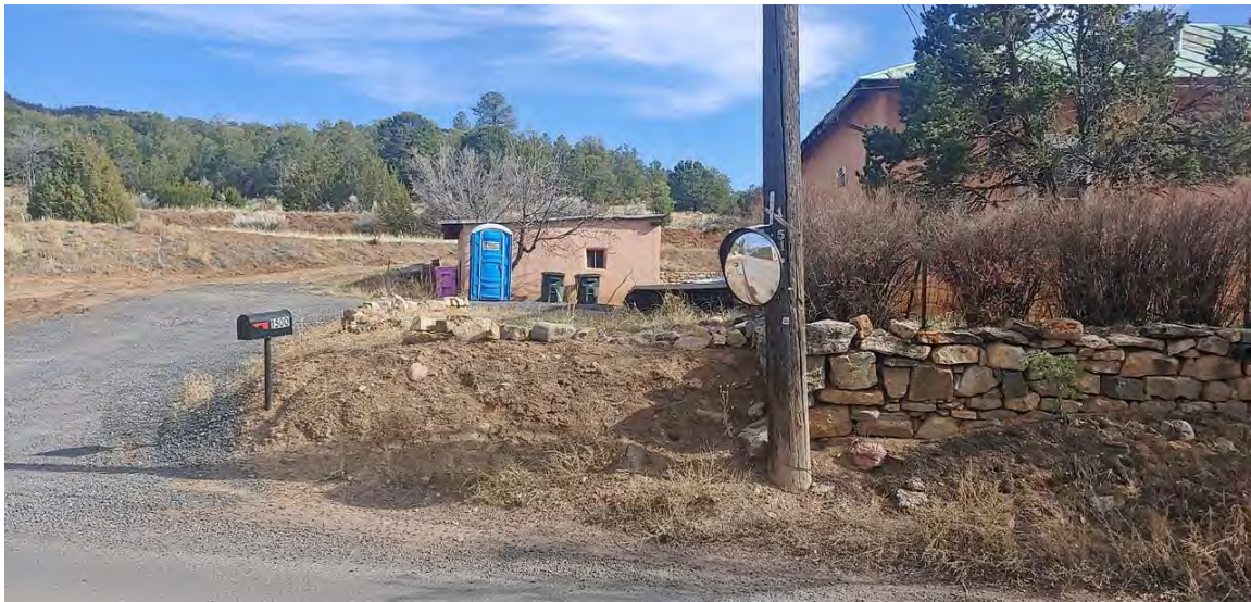
Photo 1: View of building from Upper Canyon Road. Camera facing south.
