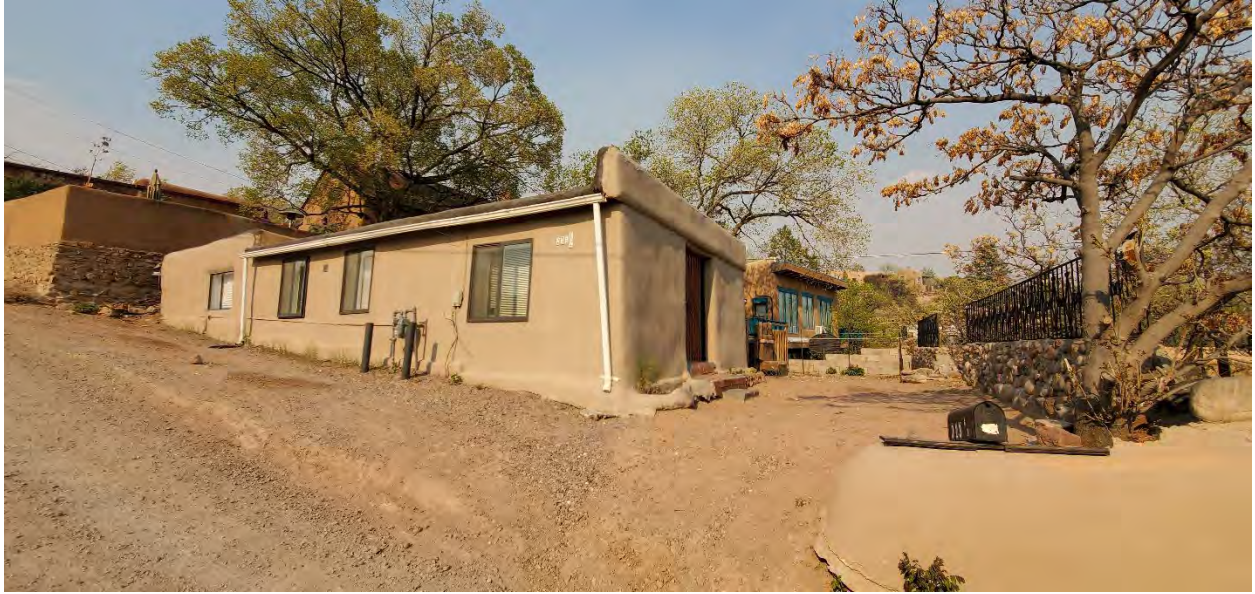
West Elevation on Rodriguez Street - looking northeast
