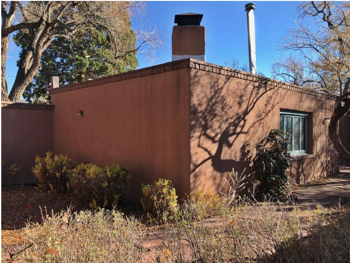
Photo 11: North and west elevations, Great Room. Camera facing southeast.
