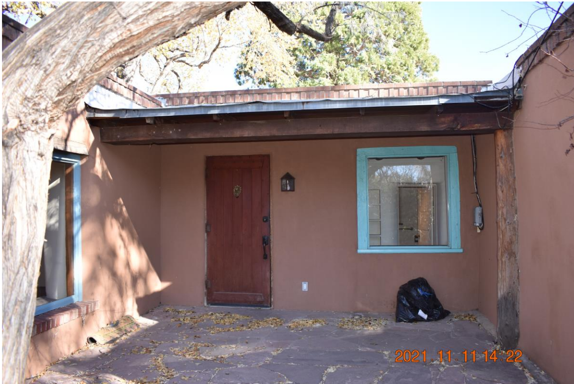
Photo 9: West elevation, entry portal. Camera facing east. Sharon Joyce, November 11, 2021.
