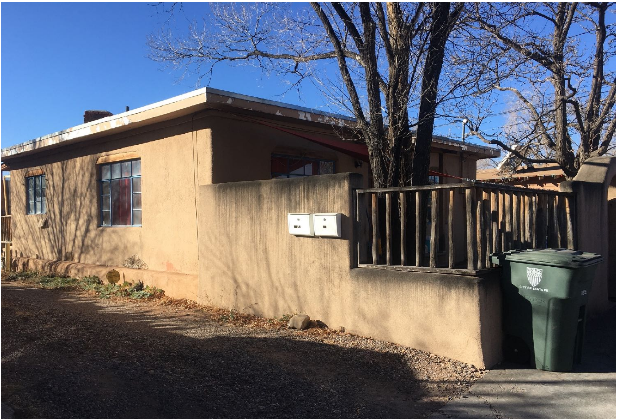
620 W San Francisco Front House Northeast corner viewed from street
