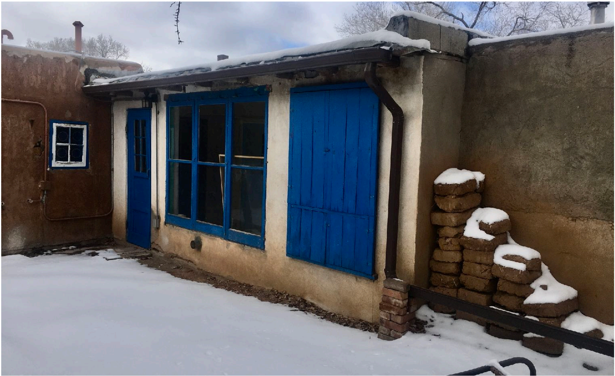
1149 Camino San Acacio Partial South Façade
