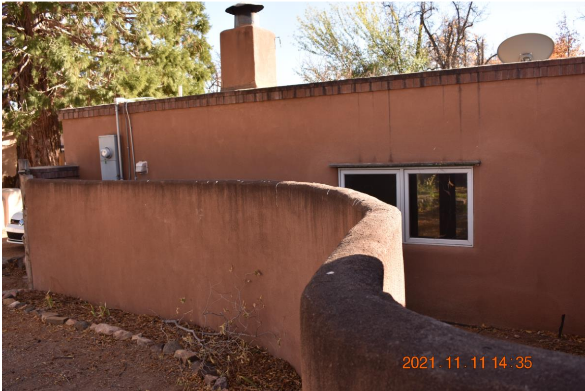
Photo 12: North elevation. Camera facing southeast. Sharon Joyce, November 11, 2021.
