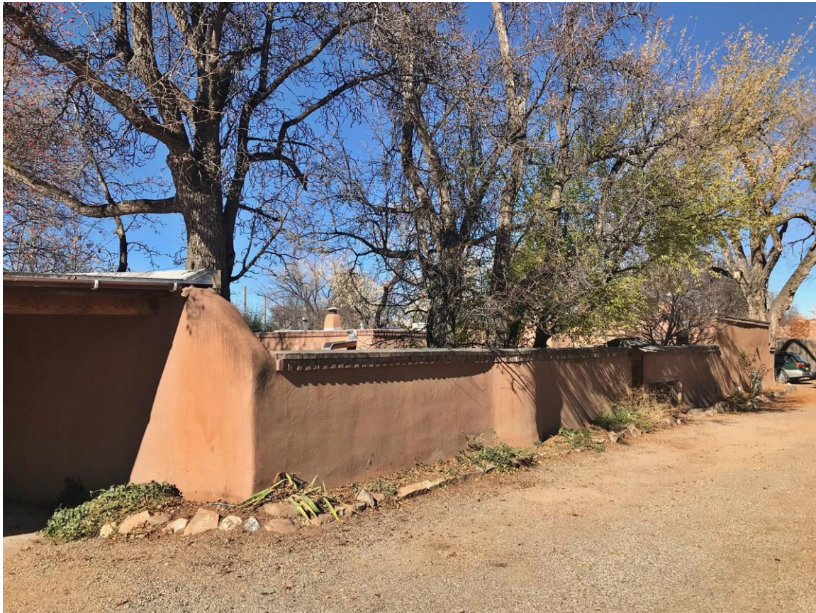
Photo 18: Yard wall. Camera facing northwest.
