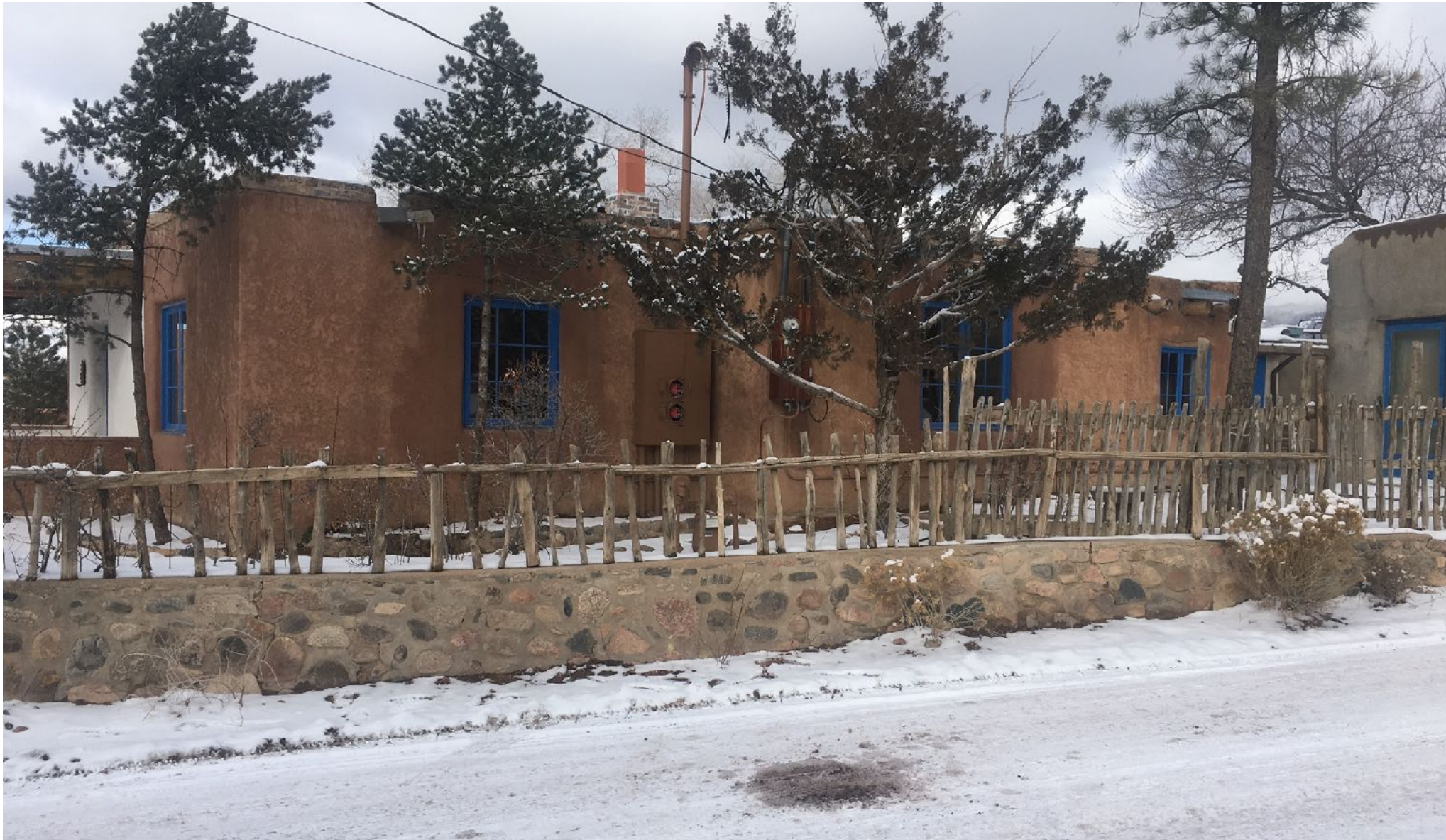
1149 Camino San Acacio South Façade Street facing
