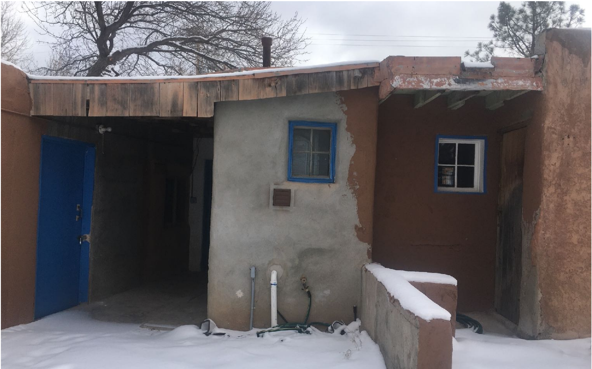
1149 Camino San Acacio East end of North Façade
