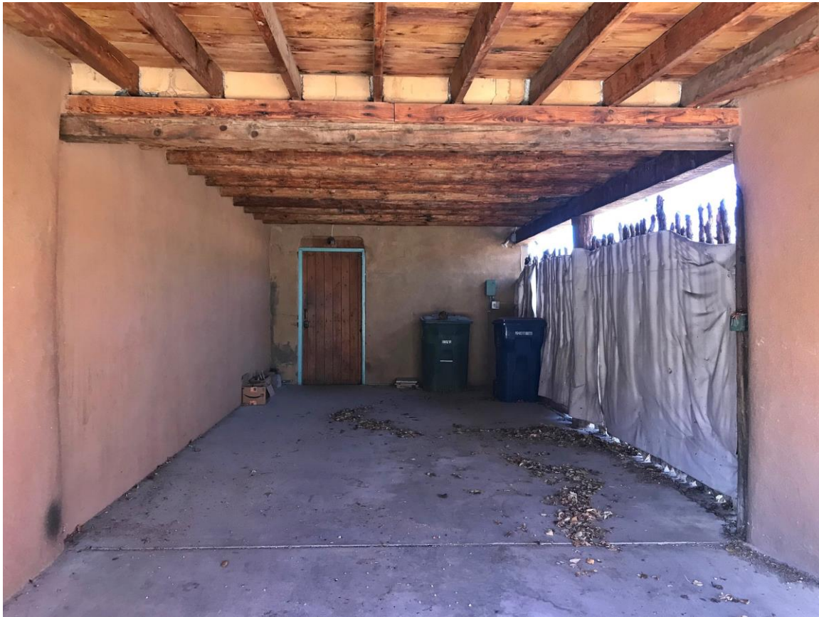
Photo 3: View of Carport. Camera facing west.
