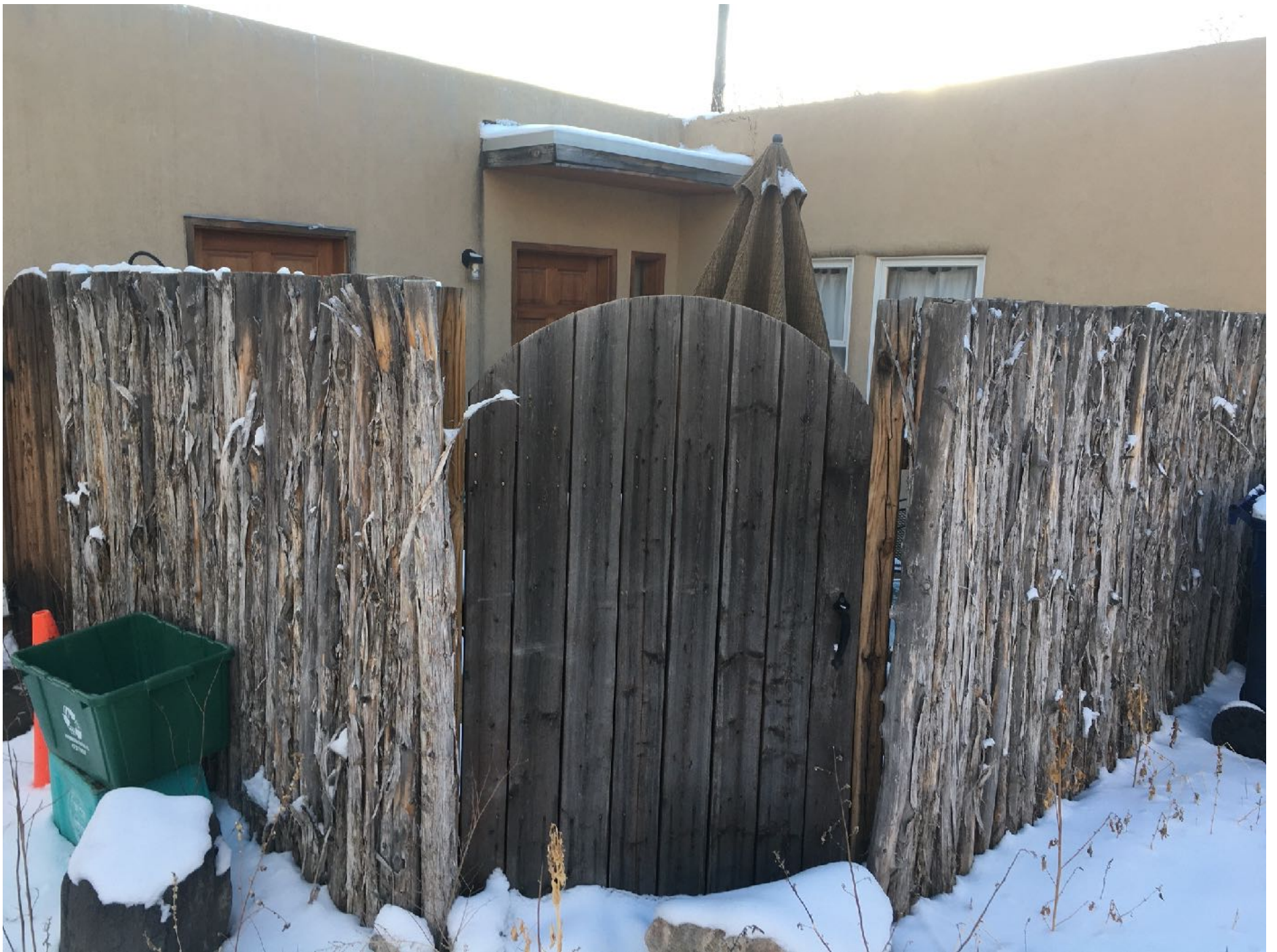
620 W San Francisco Rear House North courtyard detail
