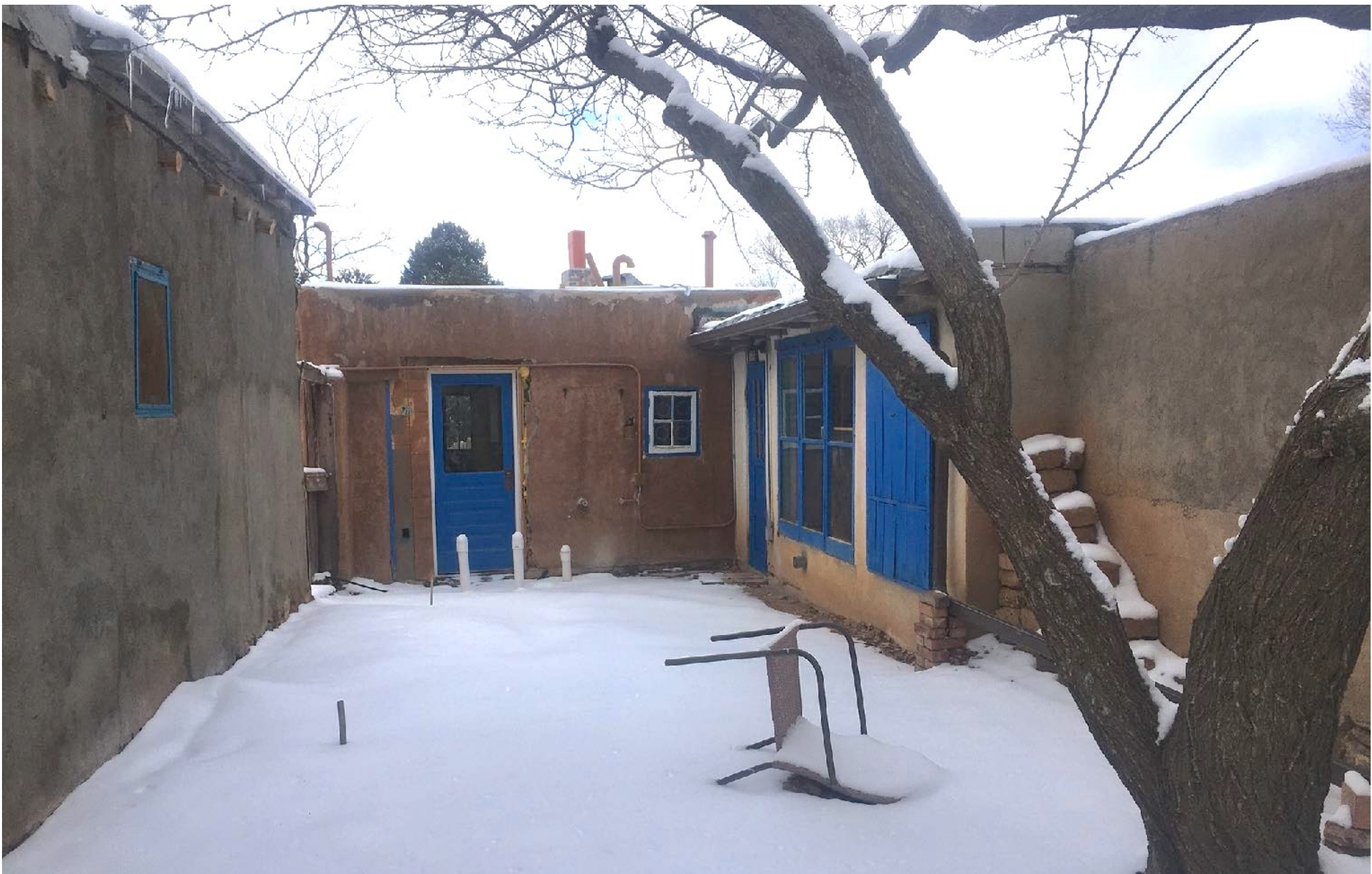
1149 Camino San Acacio Partial West and South Façade
