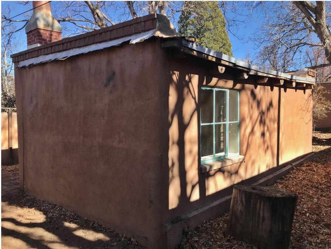
Photo 15: Casita, west and south elevations. Camera facing northeast.
