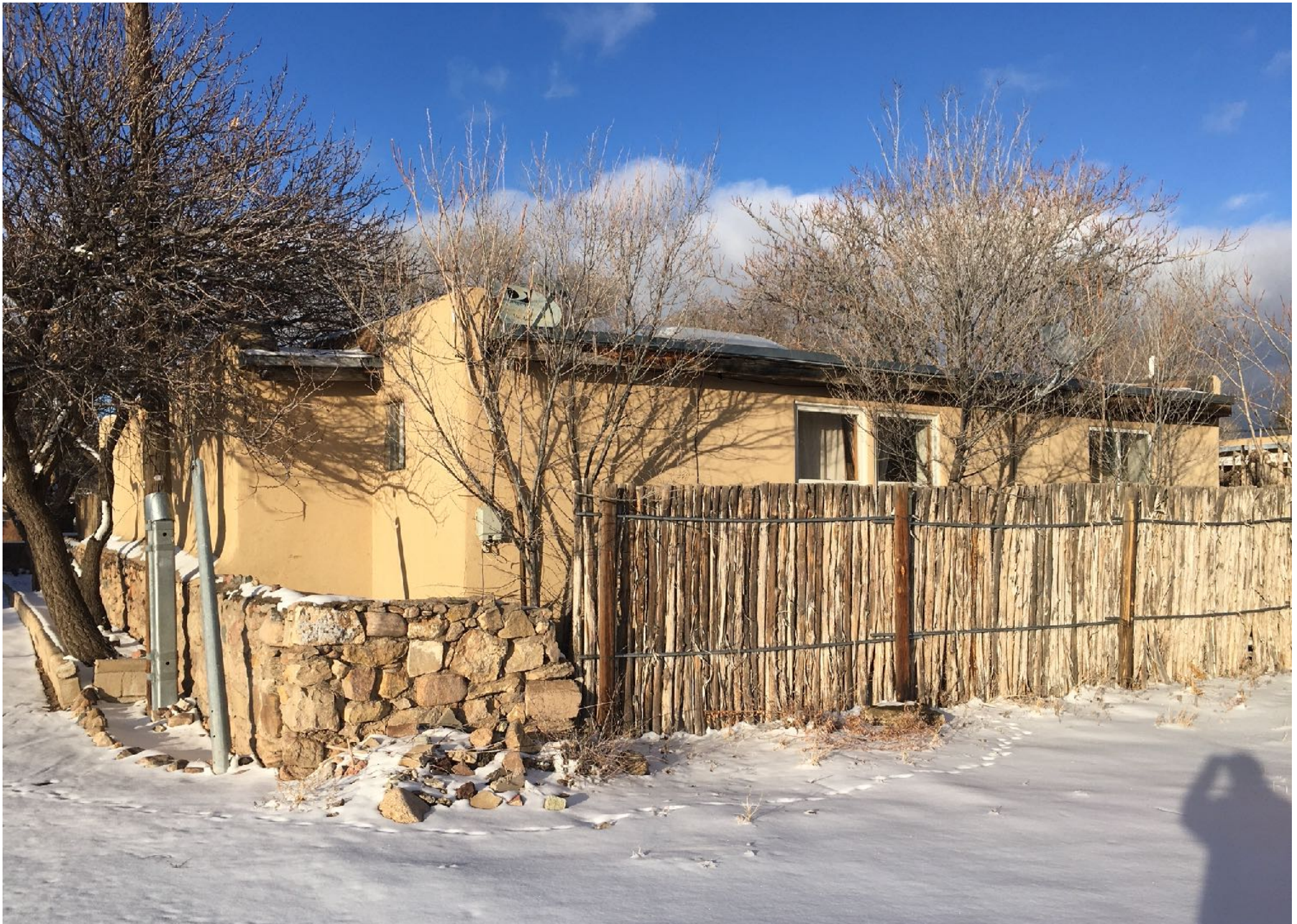
620 W San Francisco Rear House South Façade
