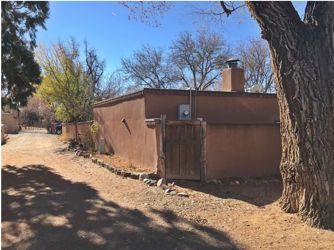
Photo 13: North and east elevations. Camera facing southwest.
