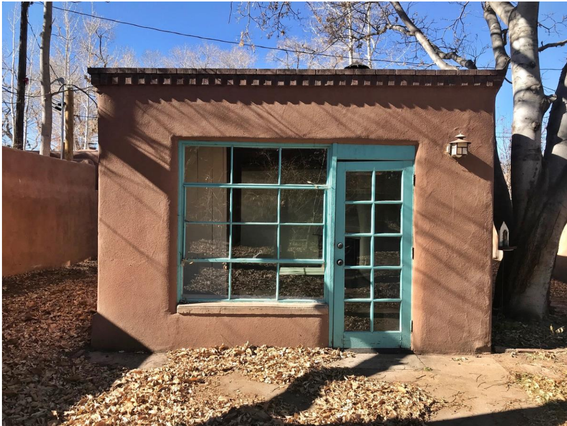
Photo 14: Casita, east elevation. Camera facing west.
