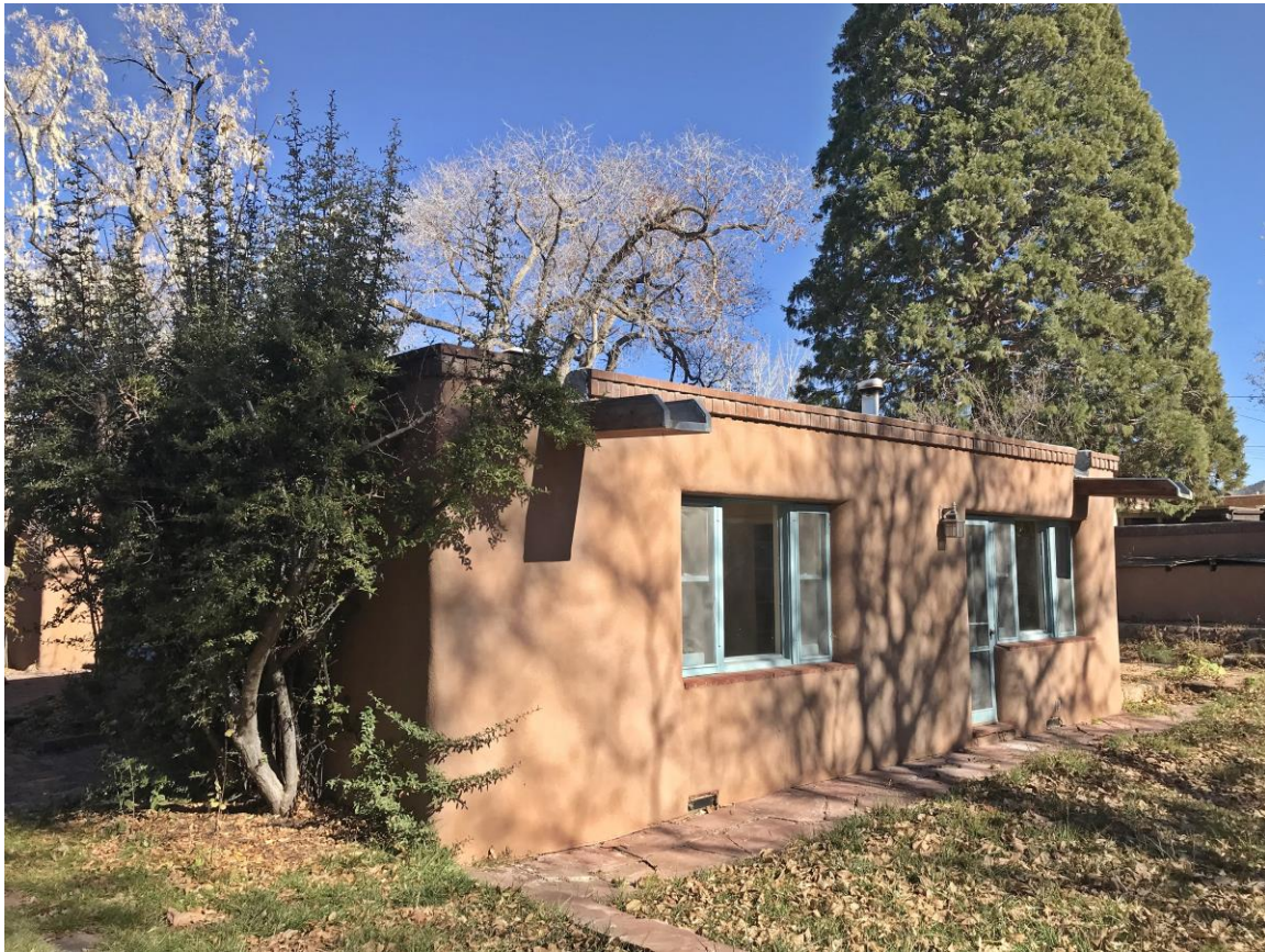
Photo 4: South elevation. Camera facing northeast.
