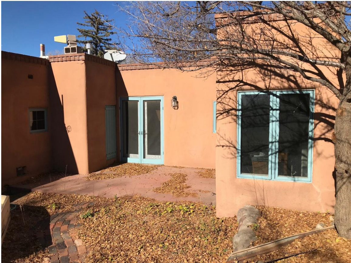
Photo 6: South elevation. Camera facing northwest.
