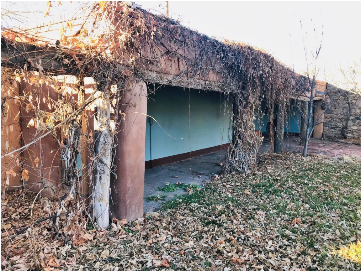
Photo 16: Portal/Pergola, west elevation. Camera facing northwest.
