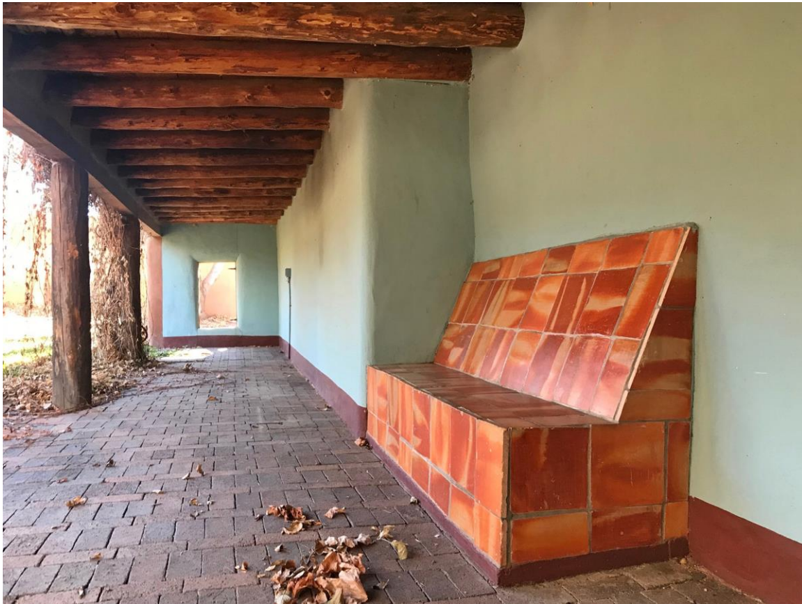
Photo 17: Portal/Pergola, interior. Camera facing south.
