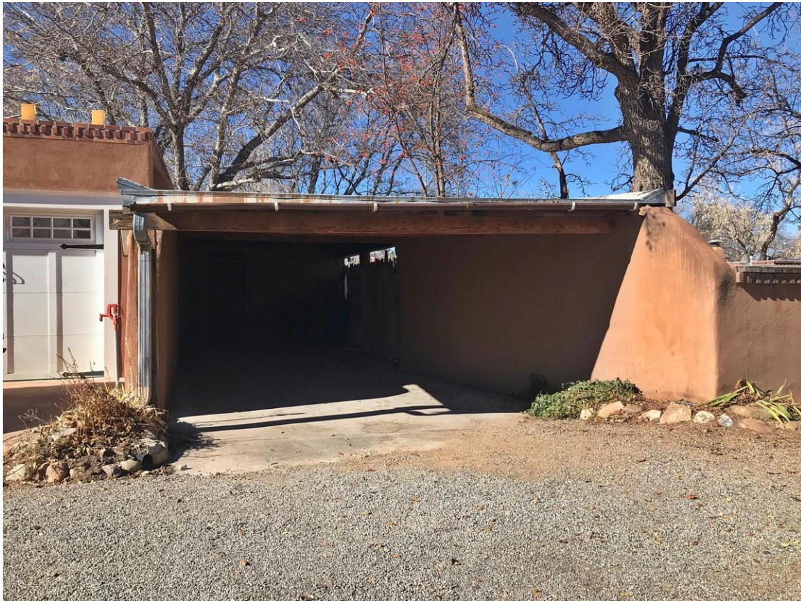
Photo 2: Carport. Camera facing northwest.
