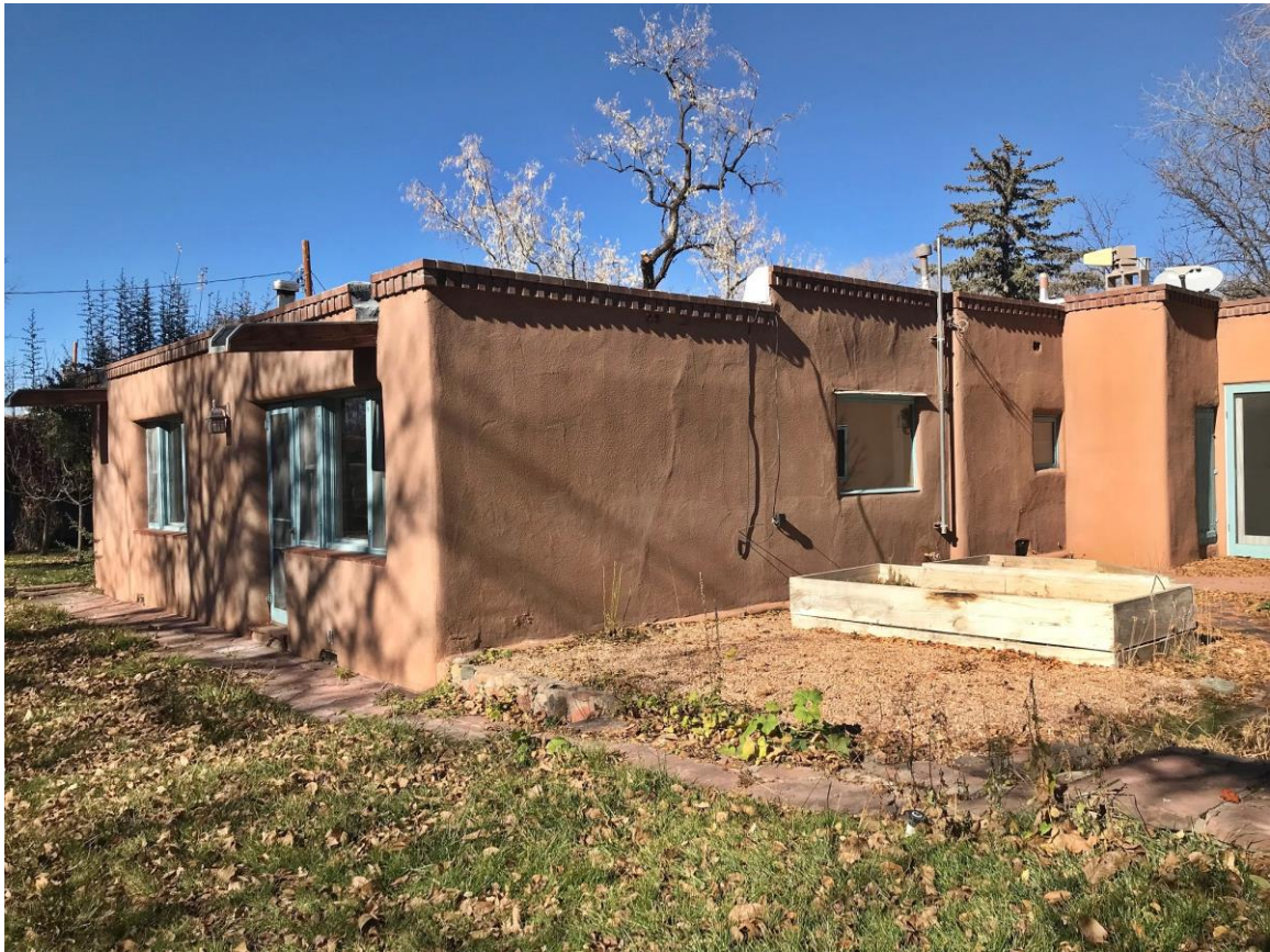
Photo 5: South and east elevations. Camera facing northwest.
