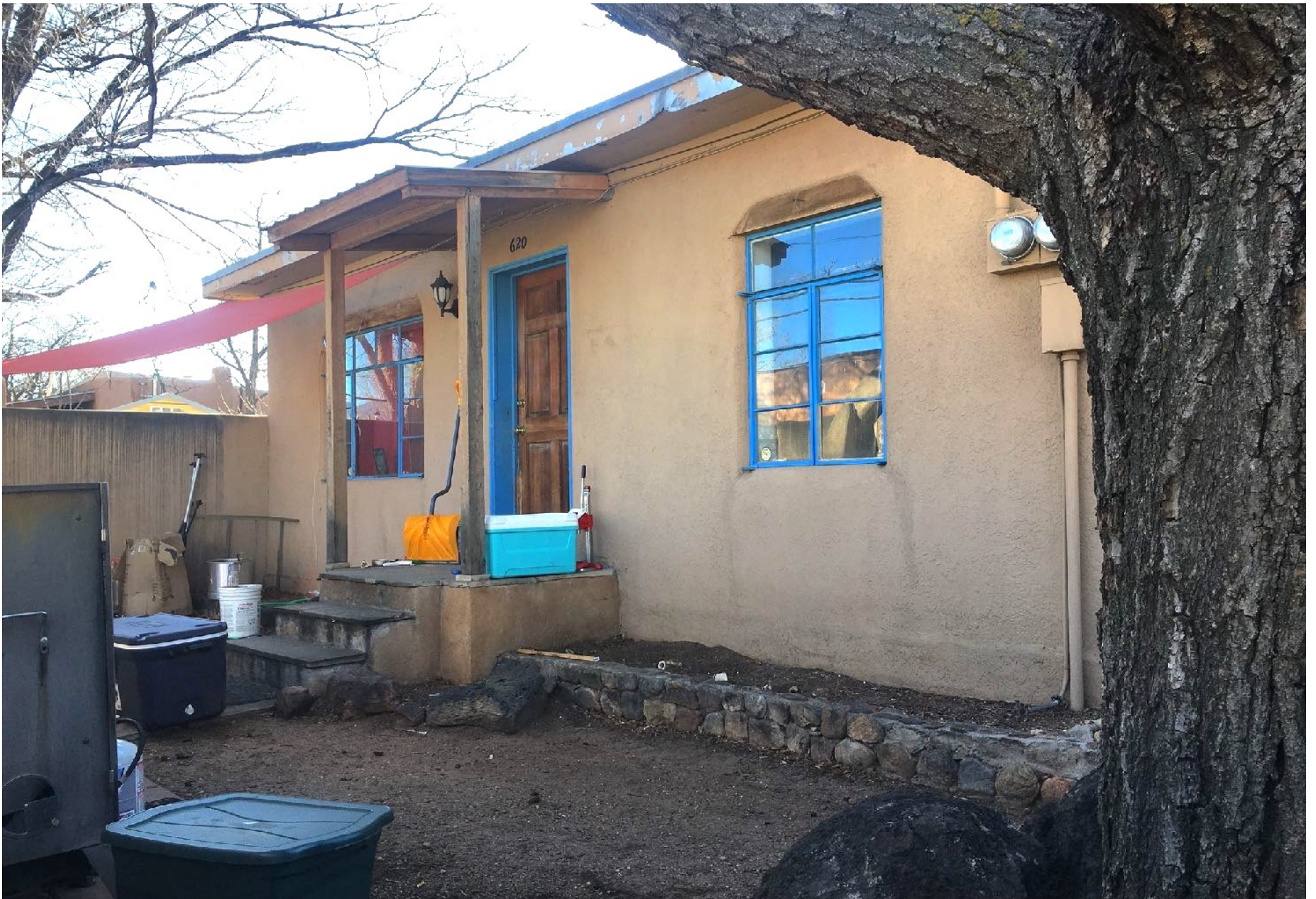
620 W San Francisco Front House North Façade
