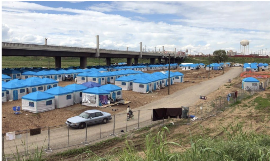
Modesto Emergency Outdoor Shelter (MOES) (Modesto, CA, 2019)
