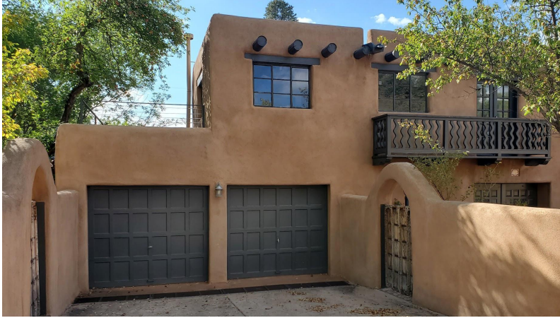
Inconspicuous cable based railing (above left garage door) and highly visible wooden railing at 110 Calle La Pena (off of Acequia Madre)
