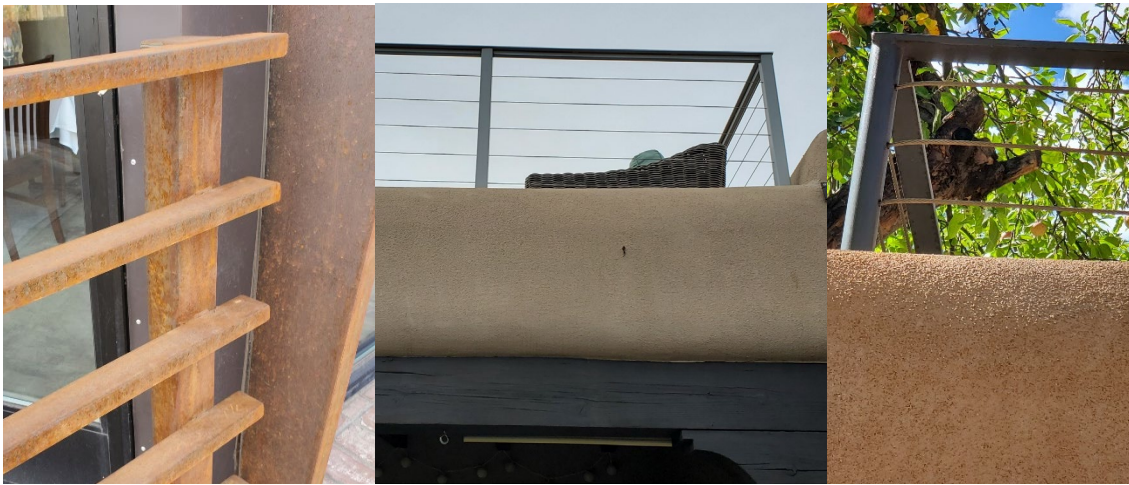
Figure 1: Fabricated steel rusty finish (left) will be used for vertical and top horizontal members of rail, with horizontal cable as shown in deck rails on nearby home (center) and at 110 Calle La Pena (right).
