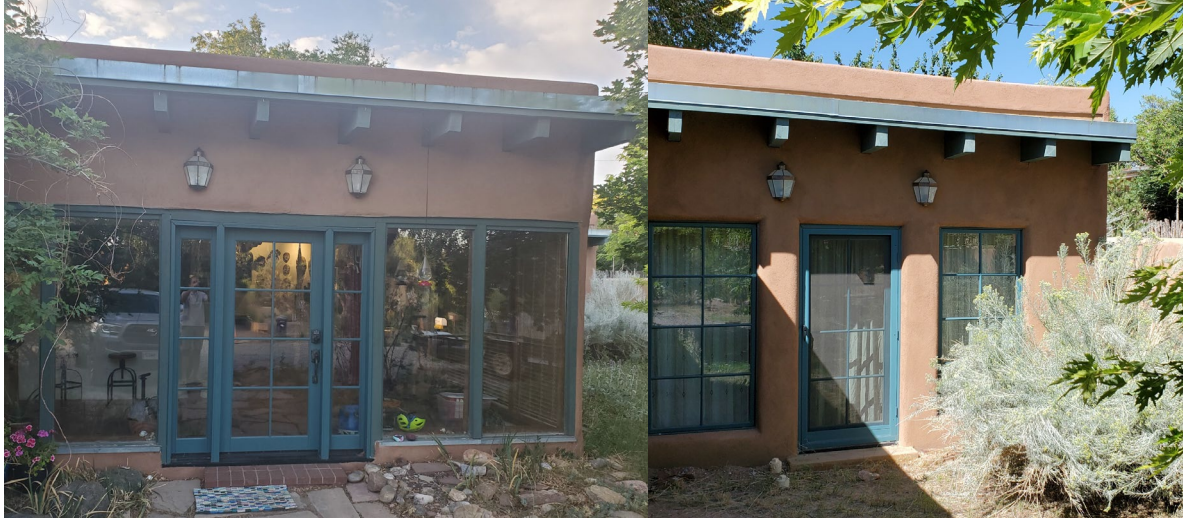
Figure 3: Overhang detail on south walls of existing home.
