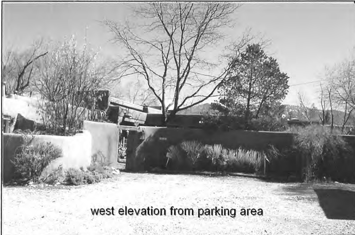
PHOTOGRAPH VIEW: west elevation
