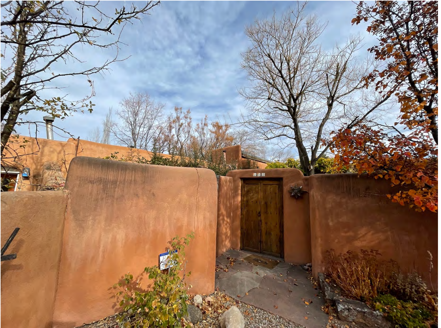
Pedestrian Entrance Gate on East wall
