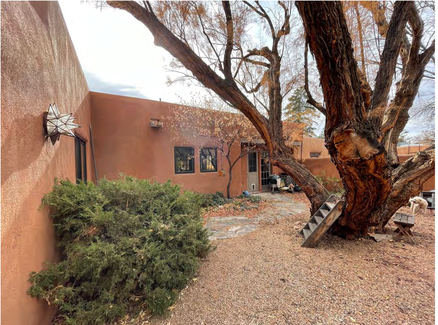
North yard looking southwest. The back wall of the kitchen will be changed. The ancient salt cedar tree remains.
