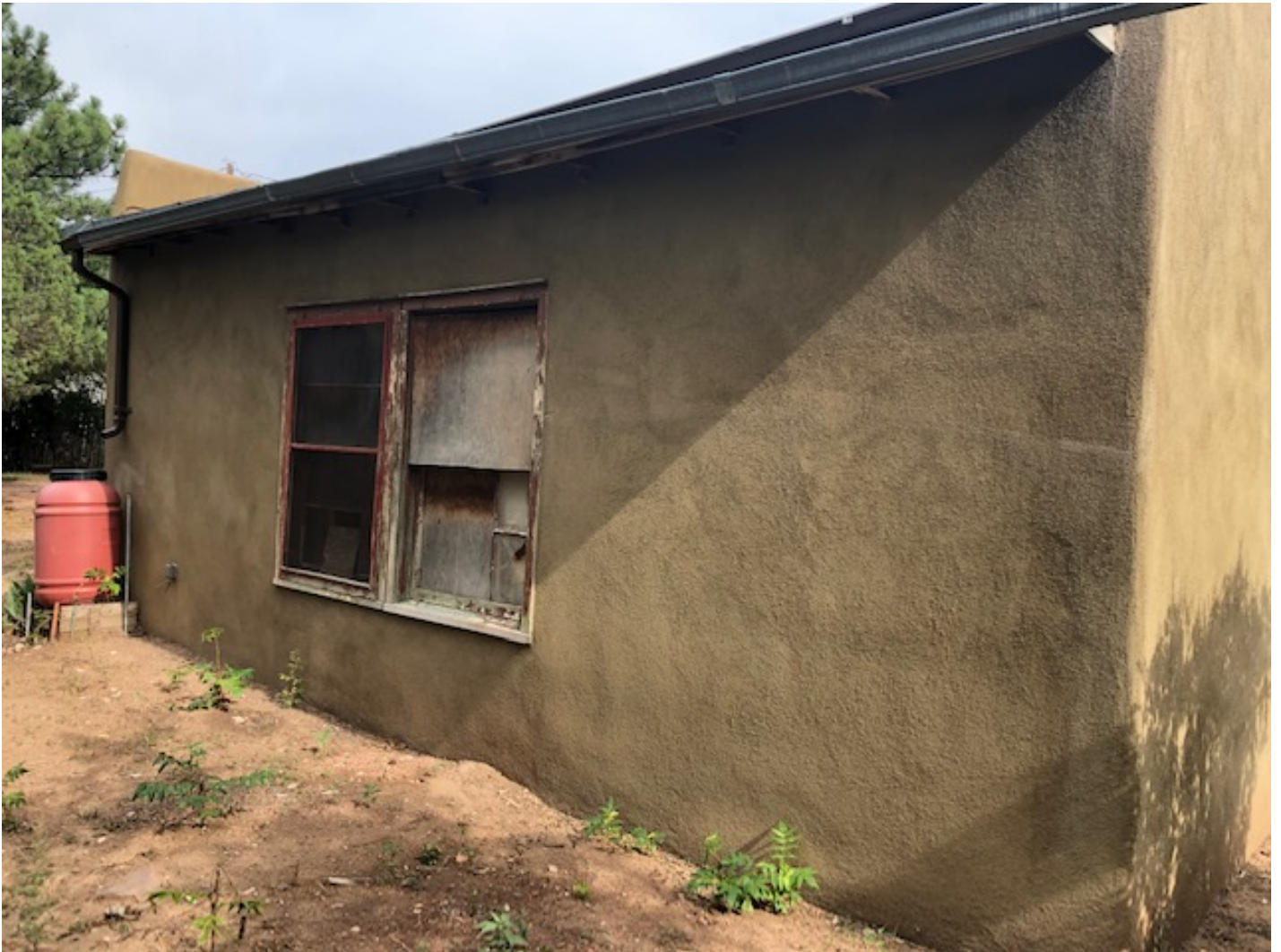
Northwest Corner of Garage
