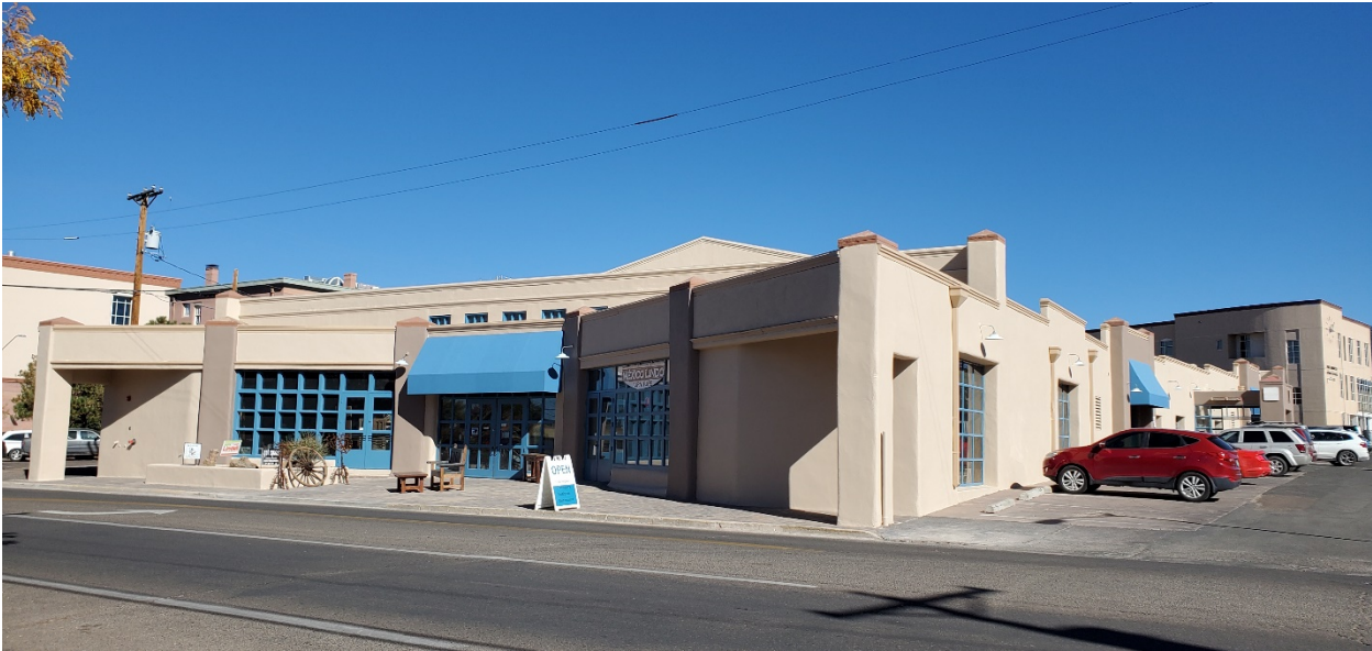
VIEW FROM SANDOVAL (SOUTHWEST CORNER)
