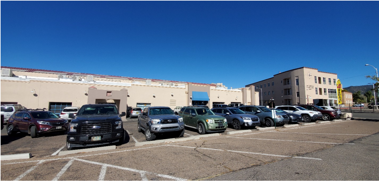
VIEW FROM PARKING LOT (SOUTH ELEVATION)
