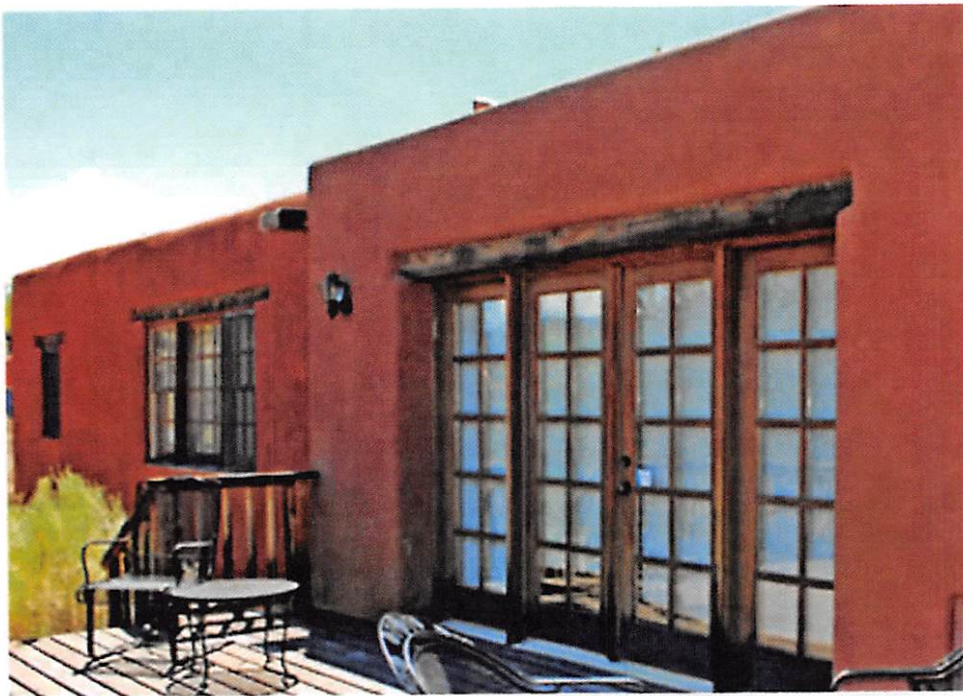
Windows, railing and doors at deck on the north side from the northwest
