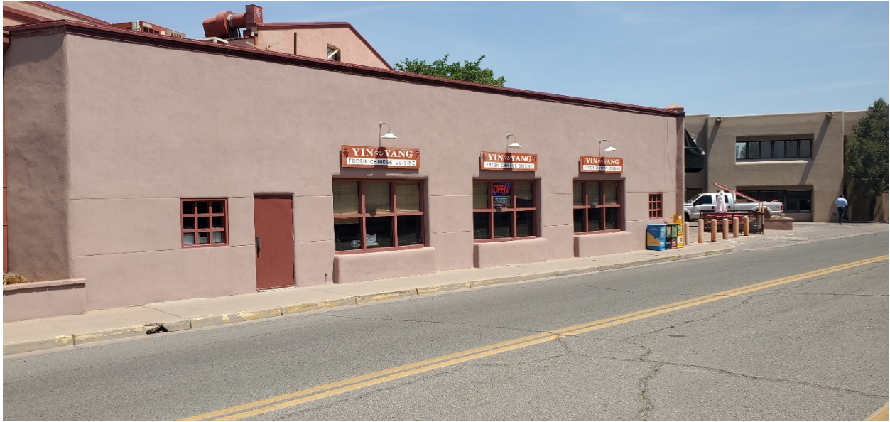
418 Cerrillos Road – Design Center Southeast Elevation
