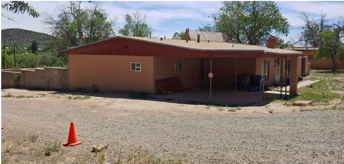
Photo 2: North and east elevations. Camera facing southeast.
