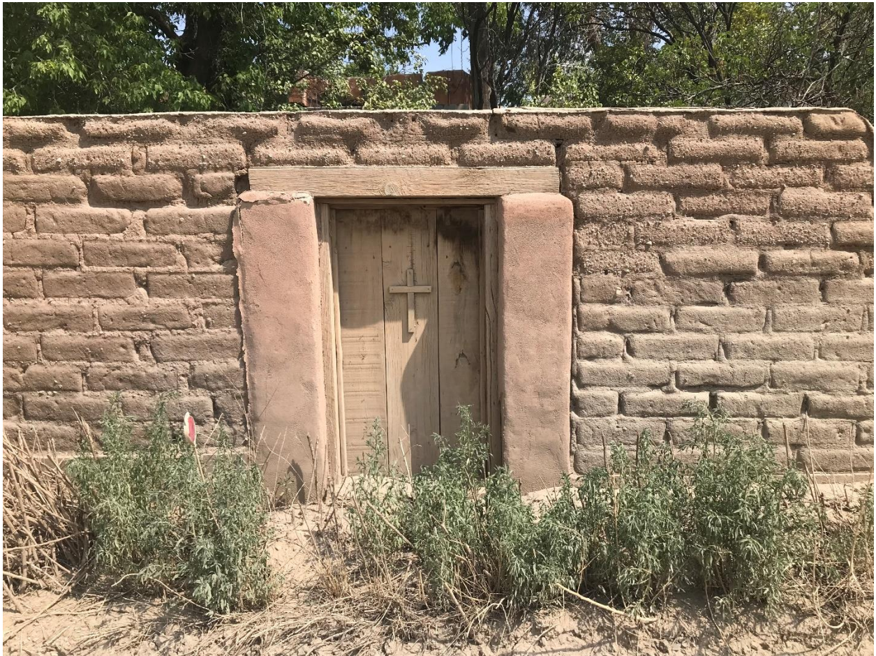
Photo 3: Stabilized adobe wall and wood gate. 1325 Cerro Gordo Road.
