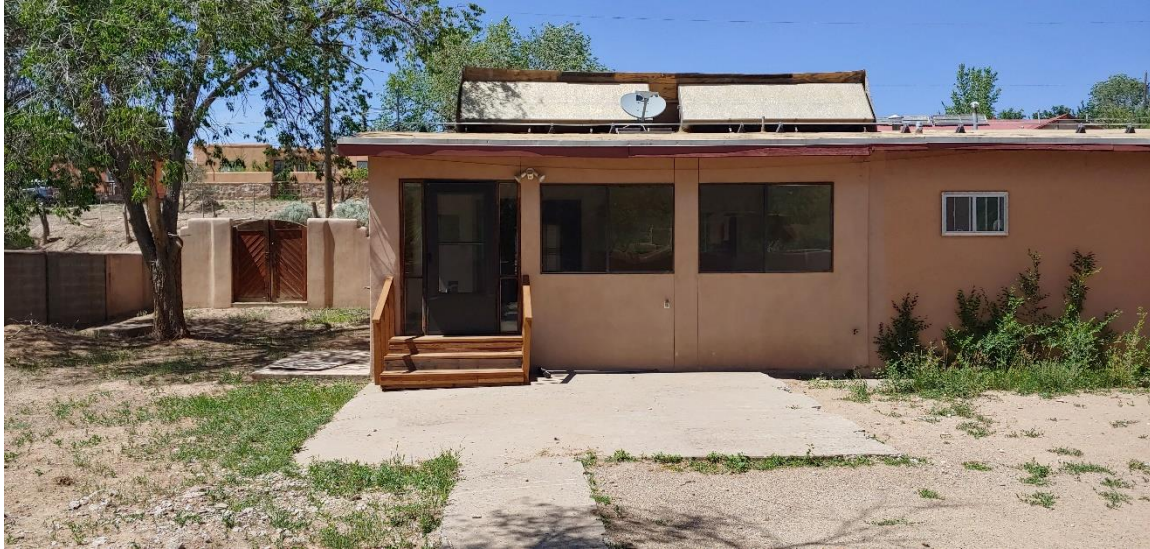
Photo 9: West end of south elevation. Camera facing north.
