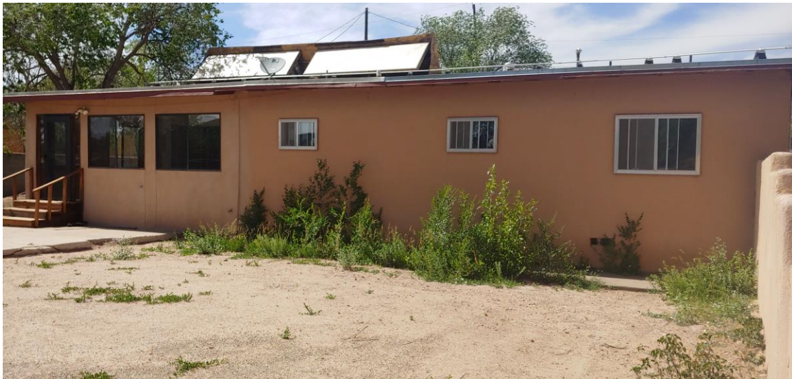
Photo 5: South elevation. Camera facing northwest.
