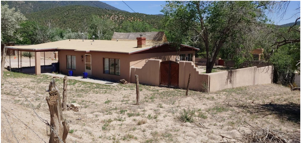
Photo 2: North and west elevations and front yard. Camera facing southeast.
