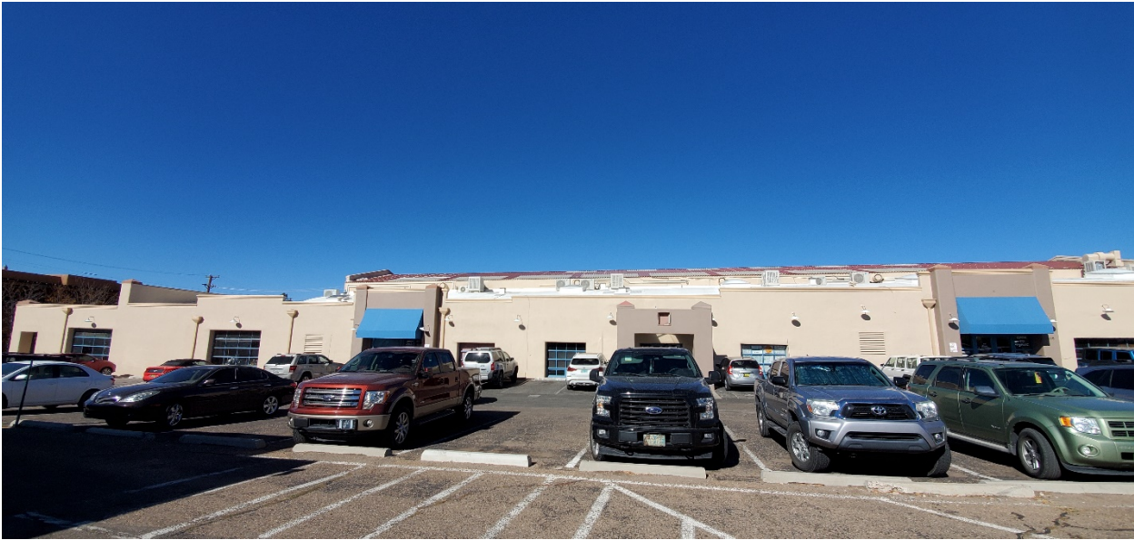
VIEW FROM PARKING LOT (SOUTH ELEVATION)
