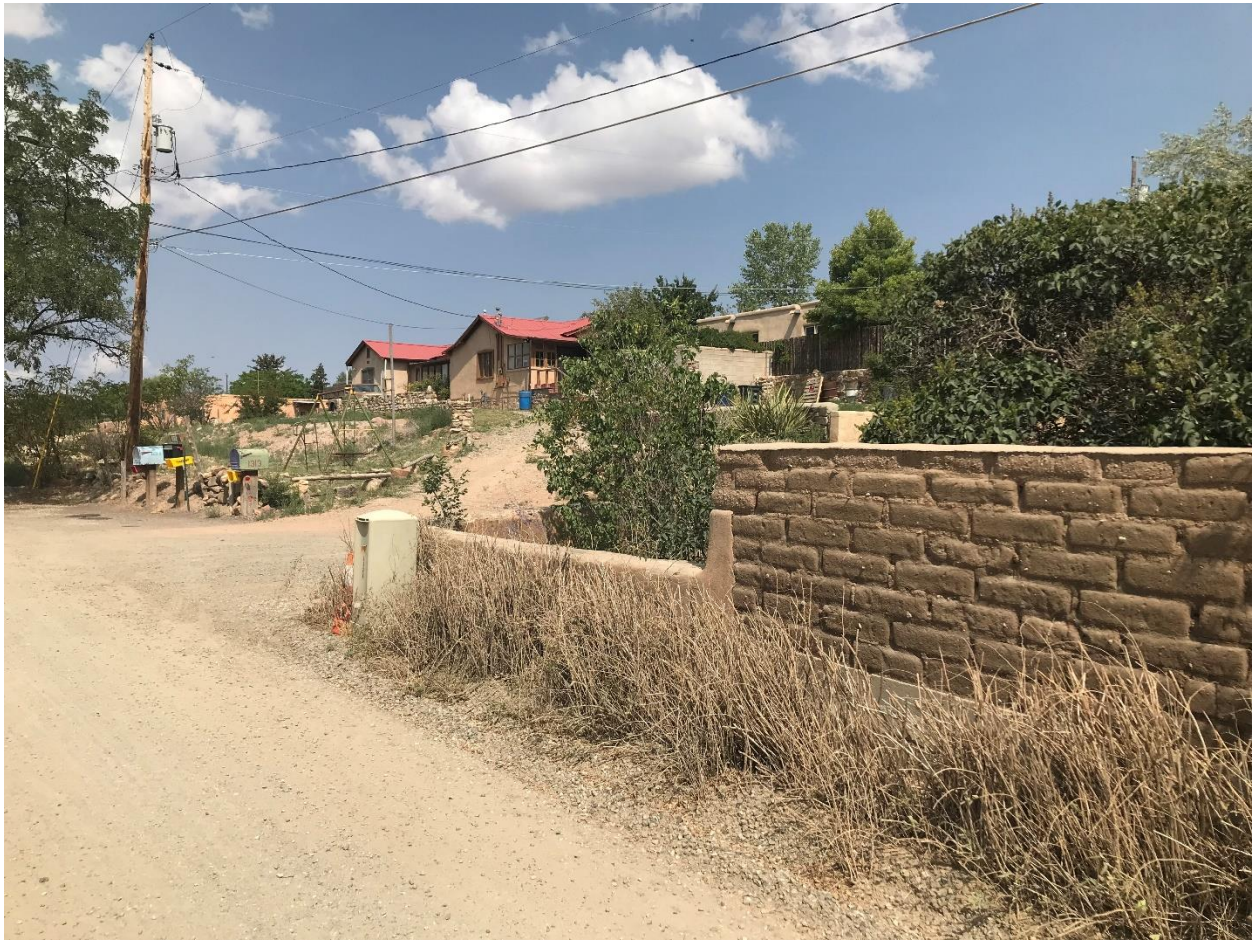
Photo 2: Stabilized adobe and low stucco-on-block wall. 1325 Cerro Gordo Road.
