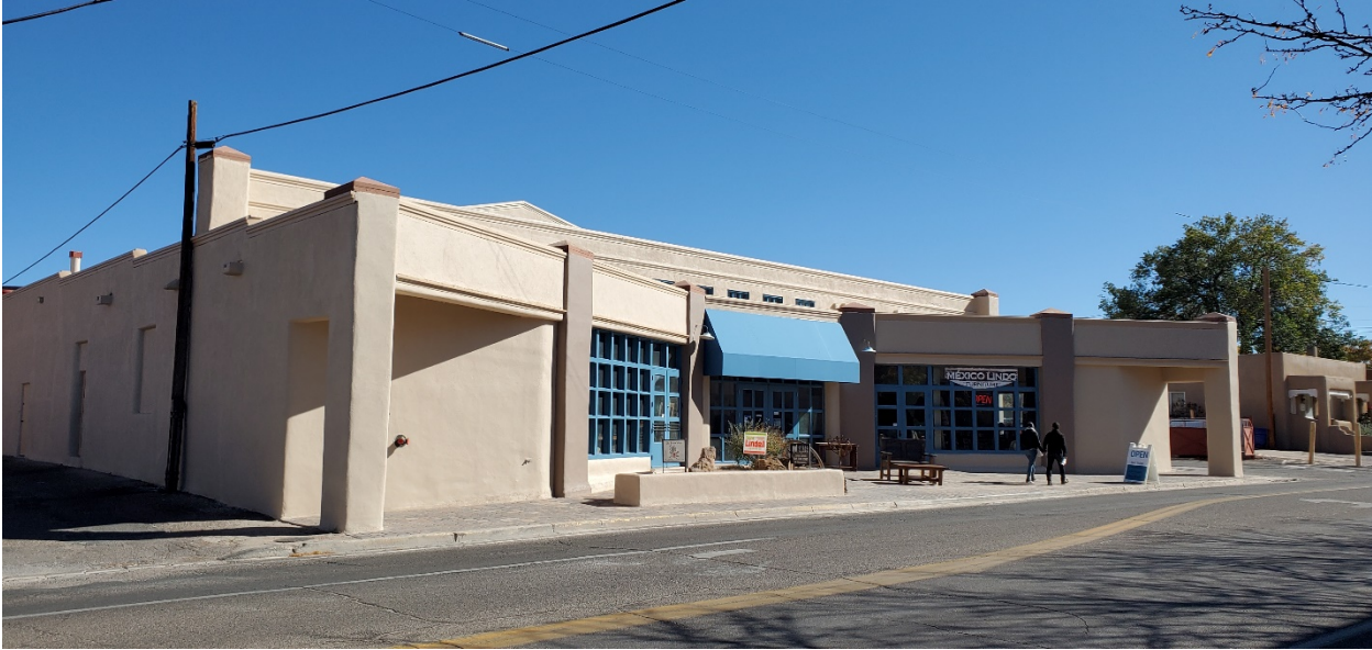
VIEW FROM SANDOVAL (NORTHWEST CORNER)
