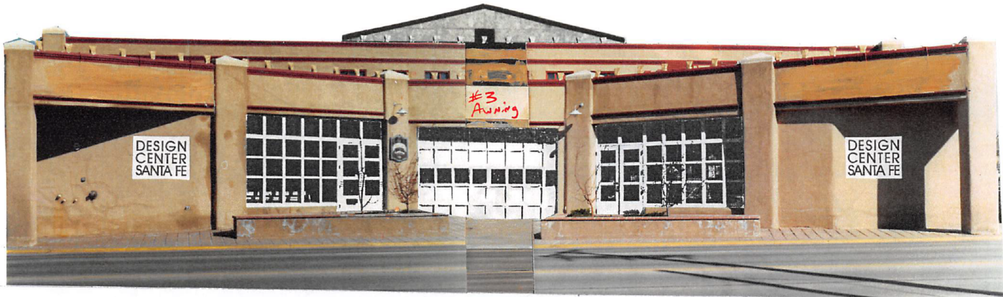
West Elevation (from Sandoval Street)
