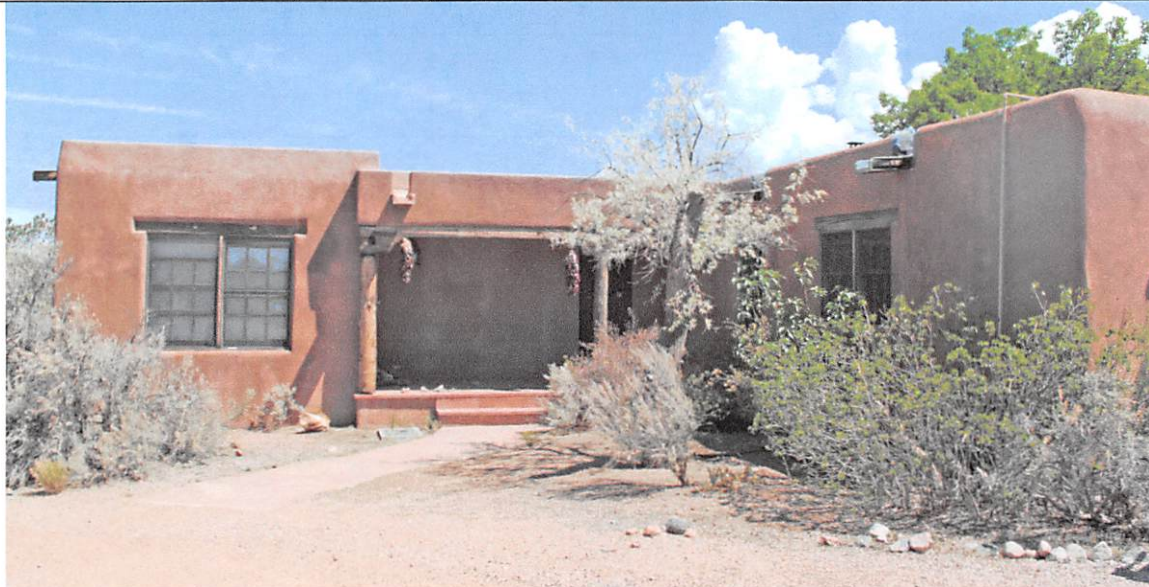
West addition and porch at left and the south end of the ell-shaped house at right
