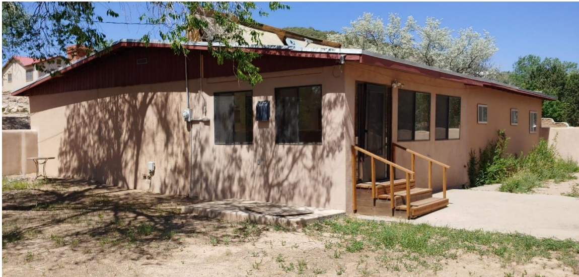
Photo 10: West elevation. Camera facing northeast.
