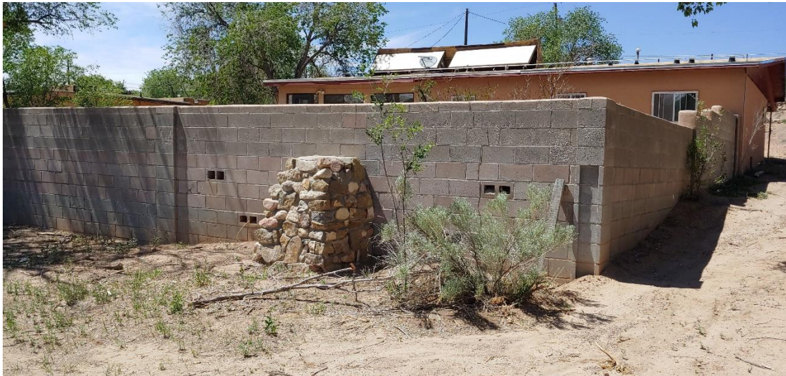
Photo 13: Backyard perimeter wall. Camera facing northwest.
