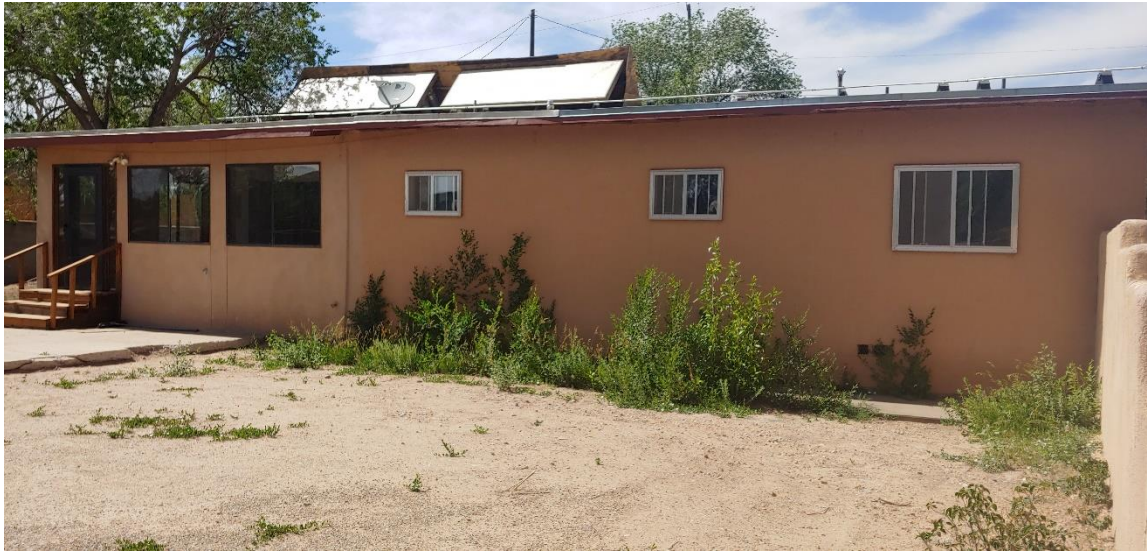
Photo 8: South elevation. Camera facing northwest.
