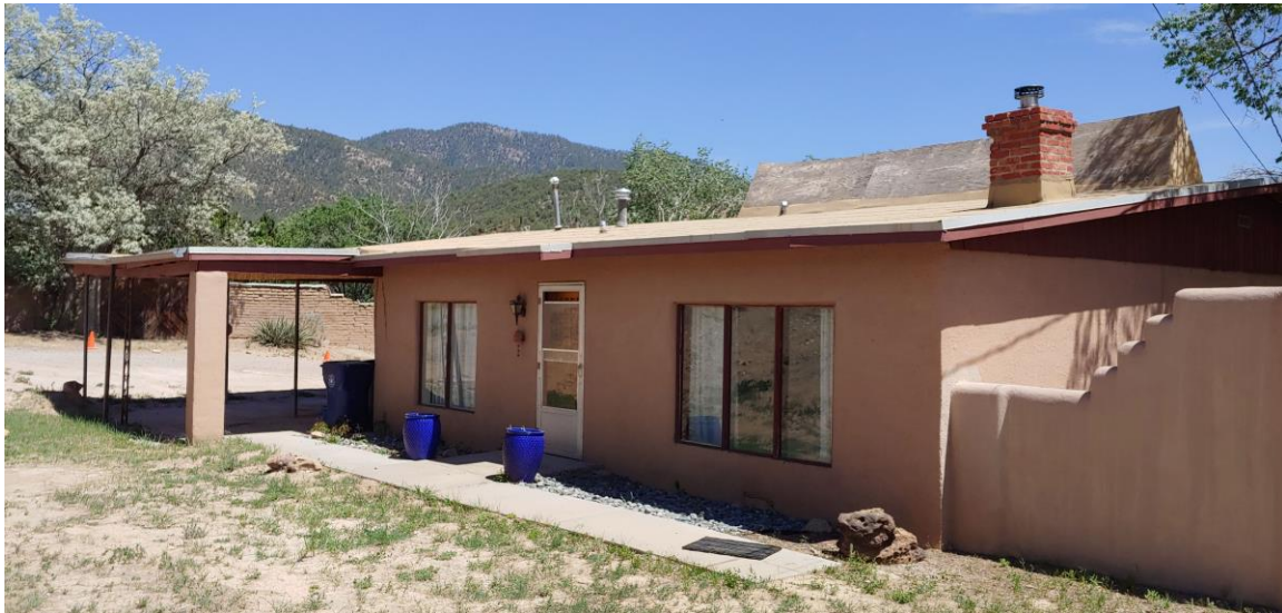
Photo 3: North elevation. Camera facing southeast.
