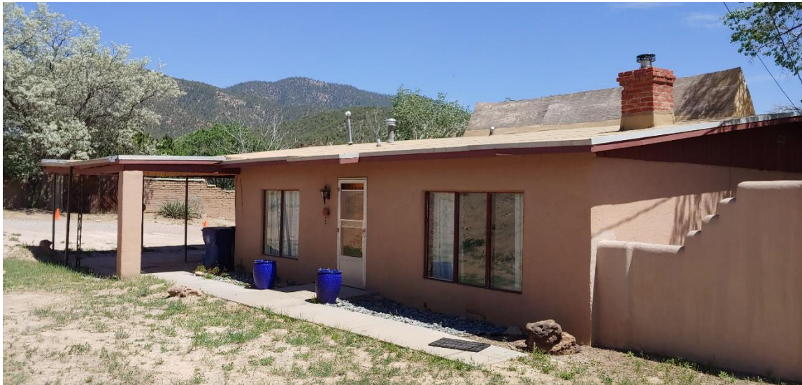
Photo 4: North elevation. Camera facing southeast.
