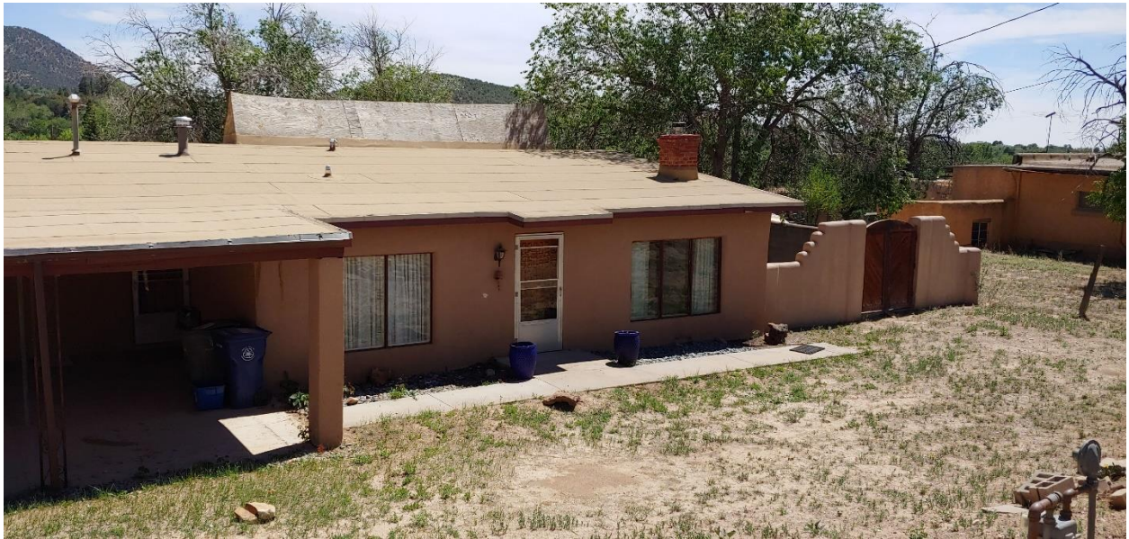
Photo 3: North elevation Camera facing southwest.
