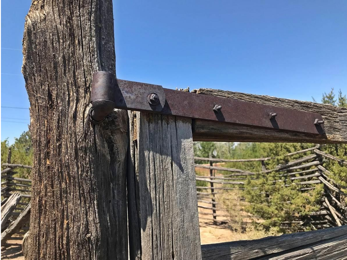
Photo 10: Screw-hook strap hinge.
