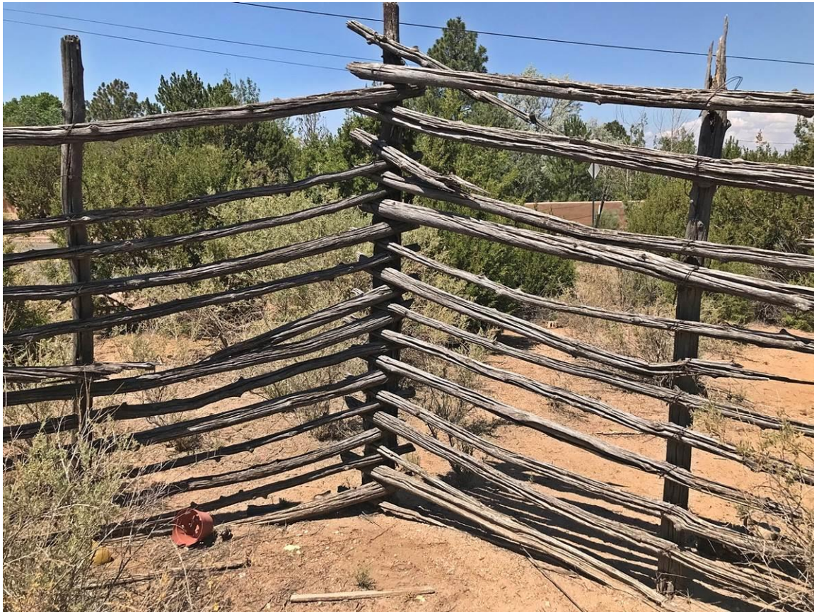
Photo 14: Small Corral-Round Pen, interlocking panels. Camera facing west.
