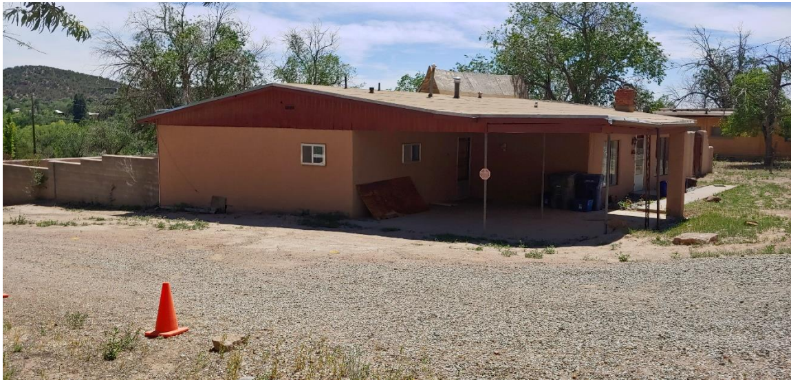
Photo 7: East and north elevations. Camera facing southwest.
