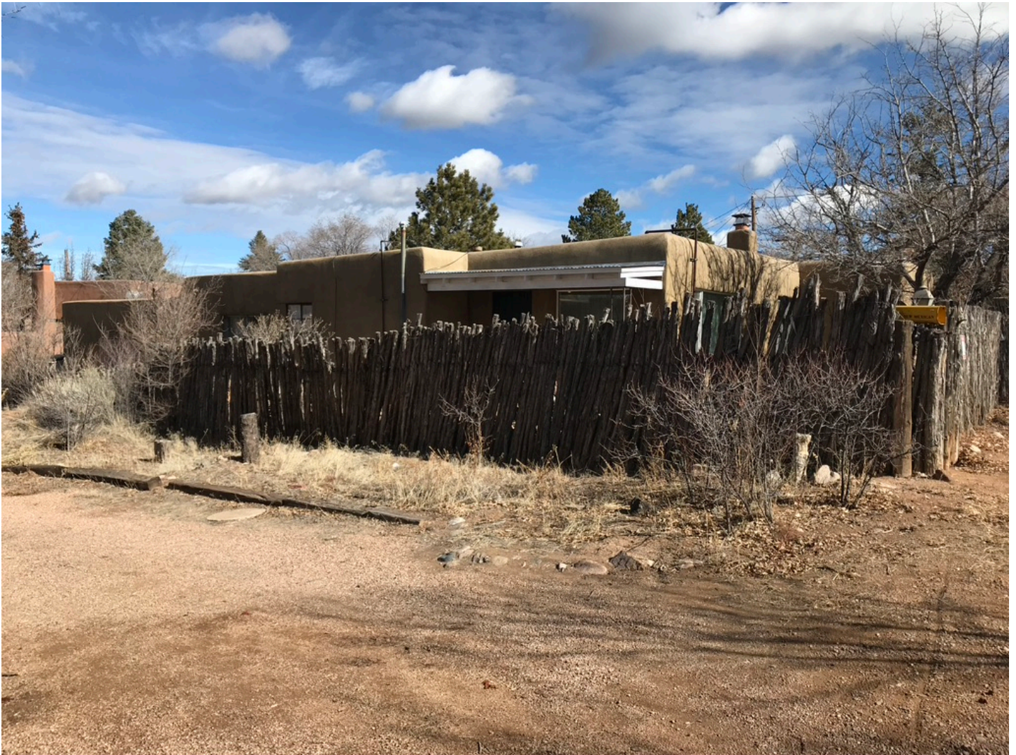
Southwest Corner from the Easement
