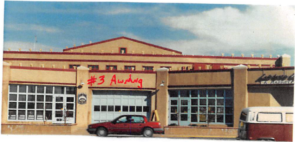
West Elevation (from Sandoval Street)
