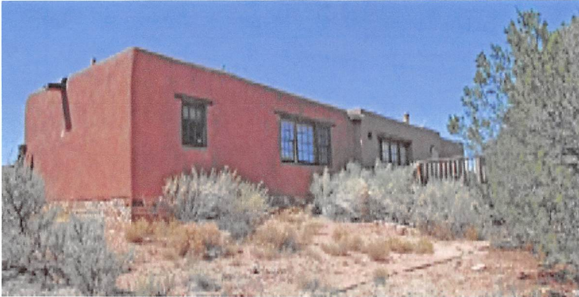
North elevation from northeast
