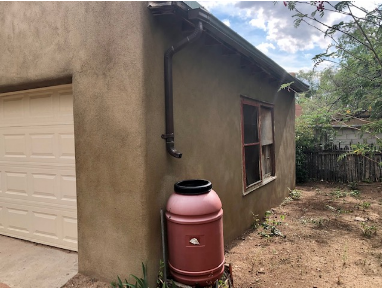
Northeast corner of Garage
