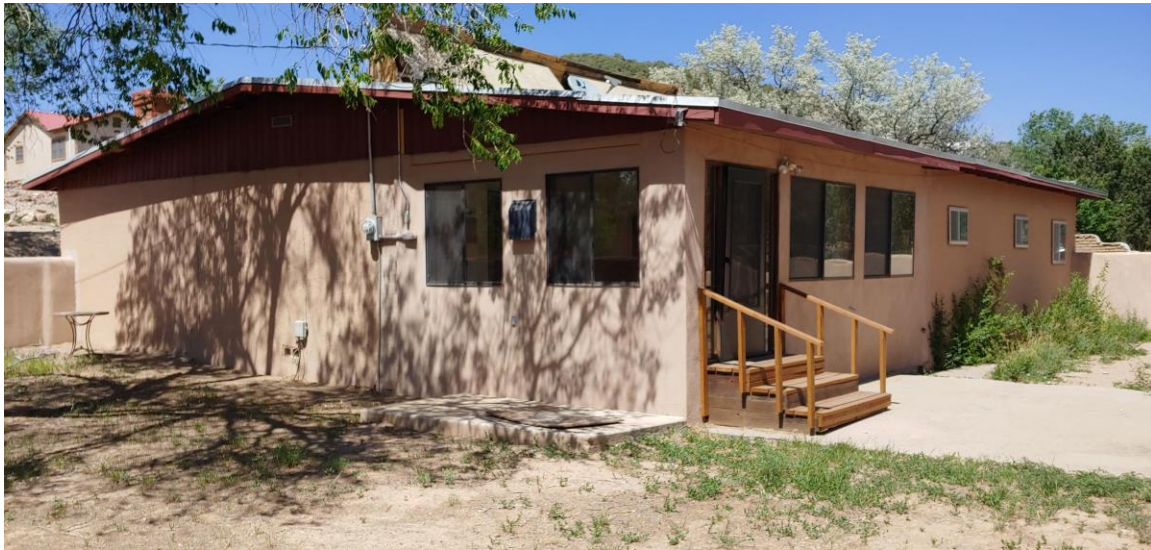
Photo 7: West elevation; enclosed porch, right. Camera facing northeast.
