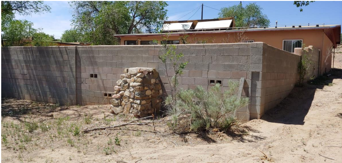
Photo 8: Backyard perimeter wall. Camera facing northwest.
