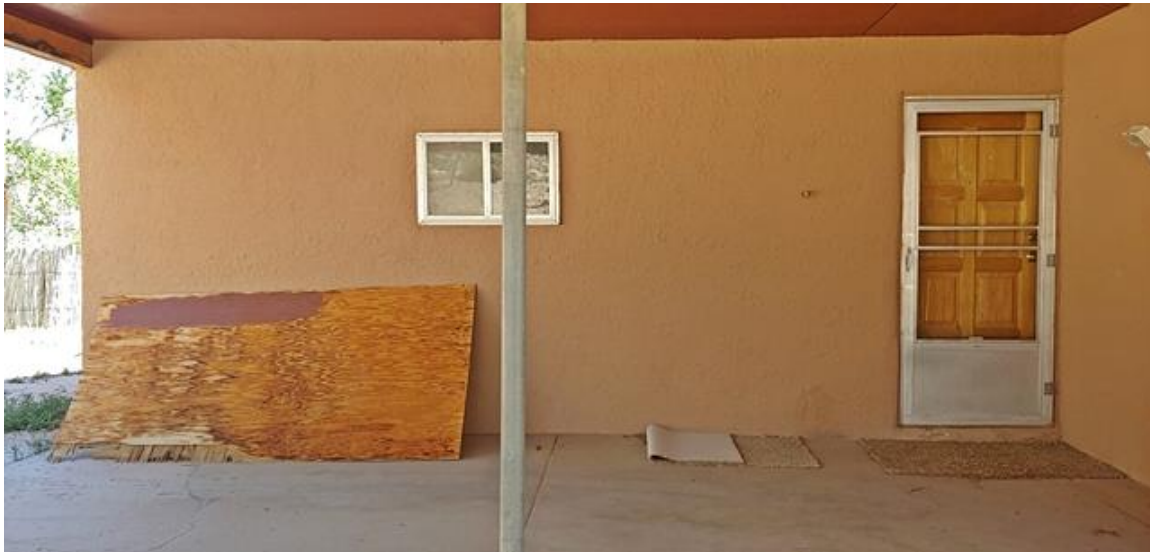
Photo 6: Carport, north elevation. Camera facing south
