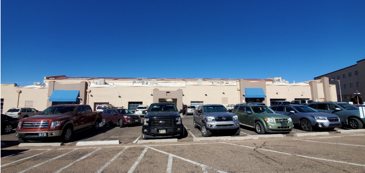
VIEW FROM PARKING LOT (SOUTH ELEVATION)
