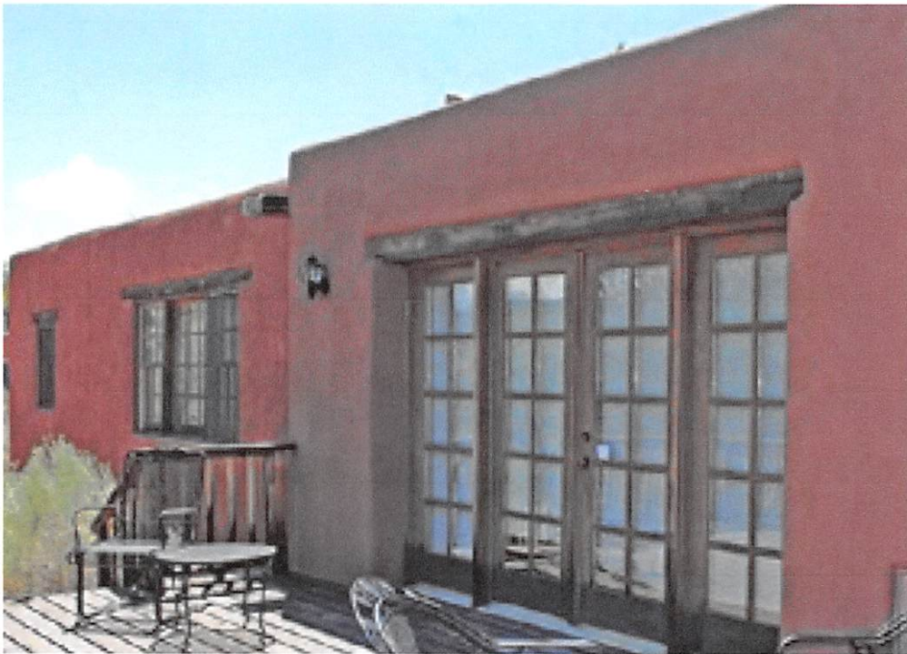
Windows, railing and doors at deck on the north side from the northwest
