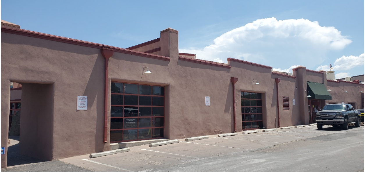
418 Cerrillos Road – Design Center Southwest Corner View
