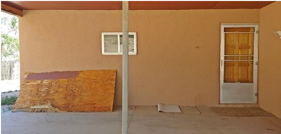
Photo 4: Carport, north elevation. Camera facing south.
