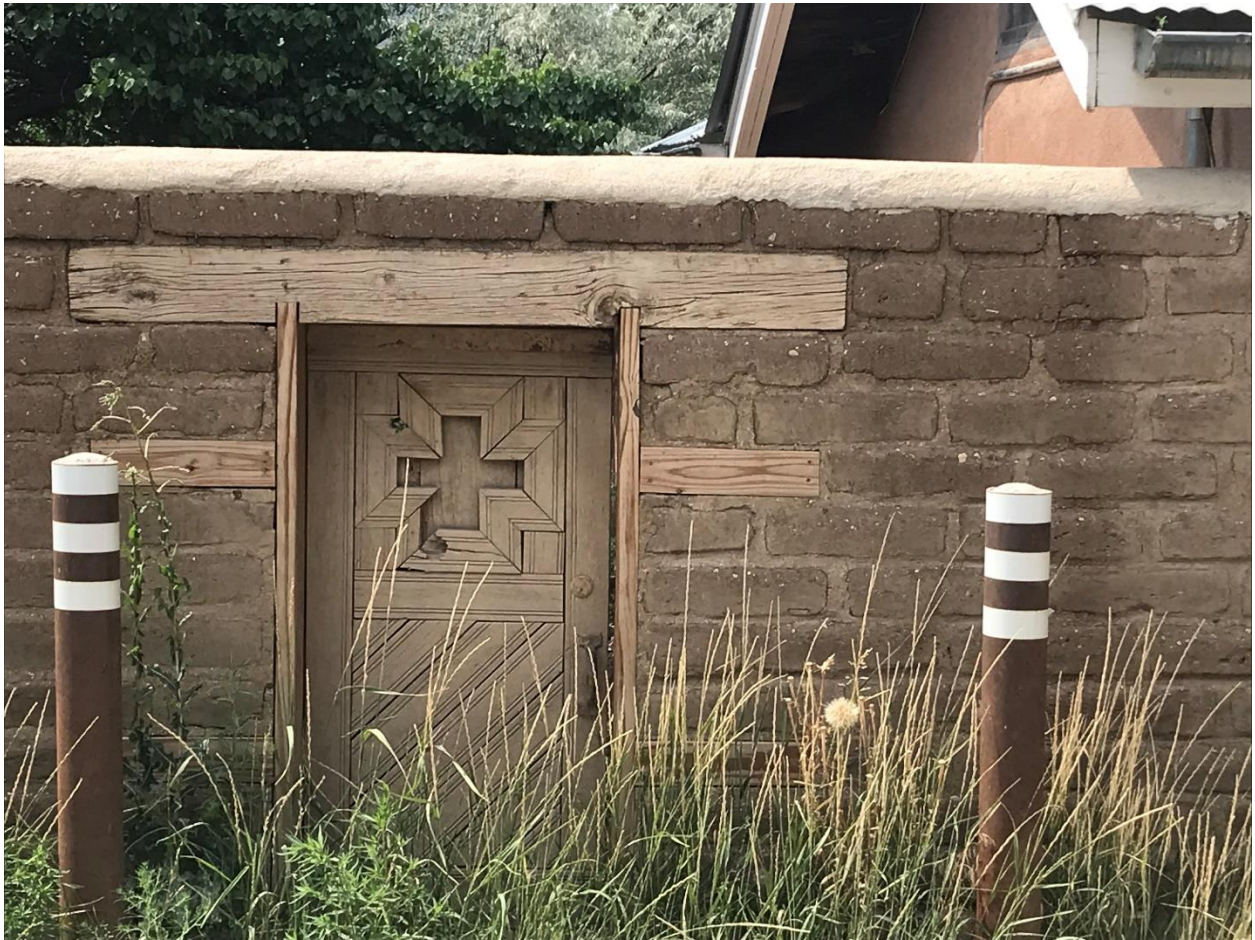
Photo 1: Stabilized adobe wall and wood gate. 1320 Cerro Gordo Road.
