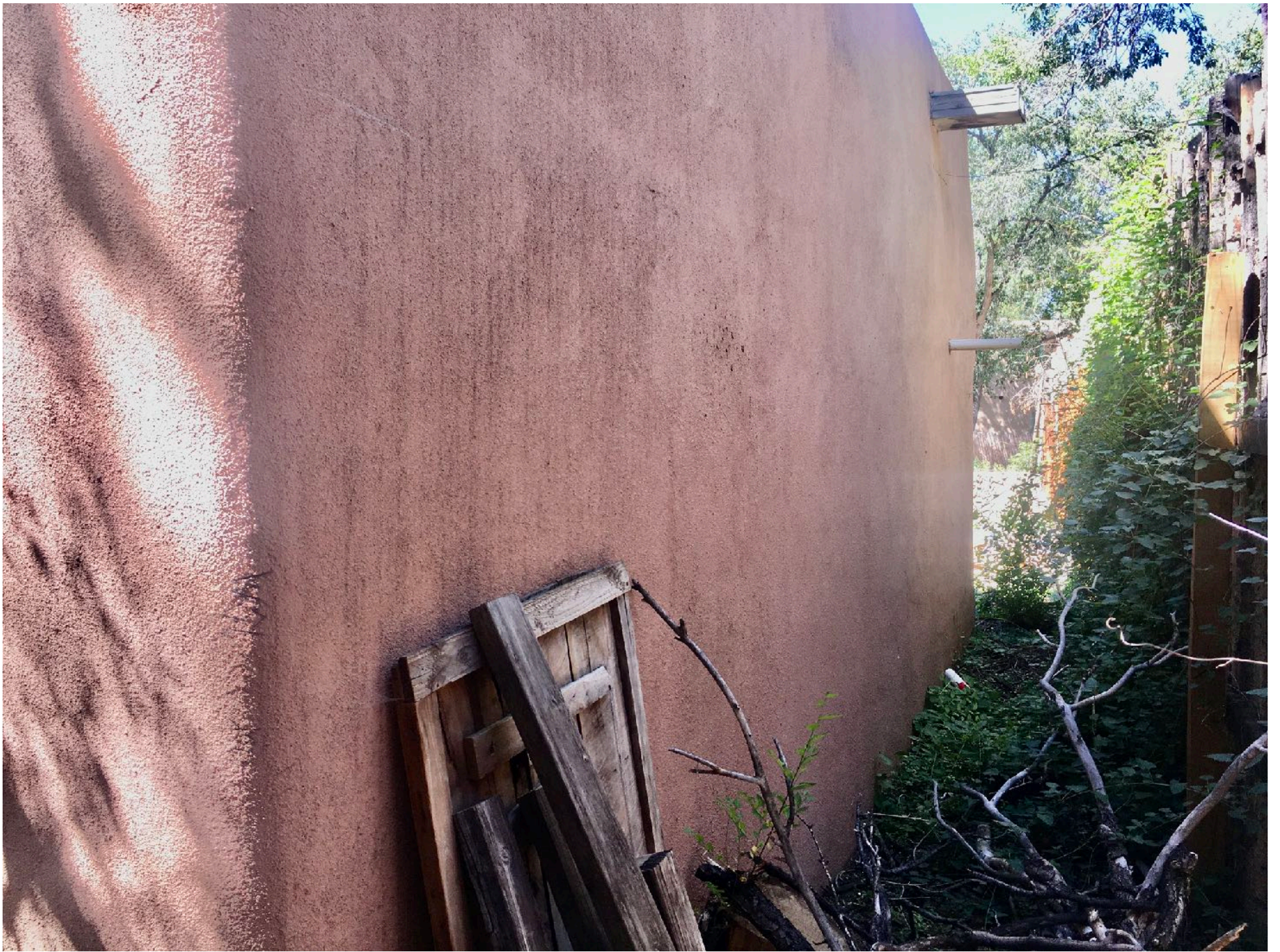
107 VICTORIA STREET ADU NORTH FAÇADE
