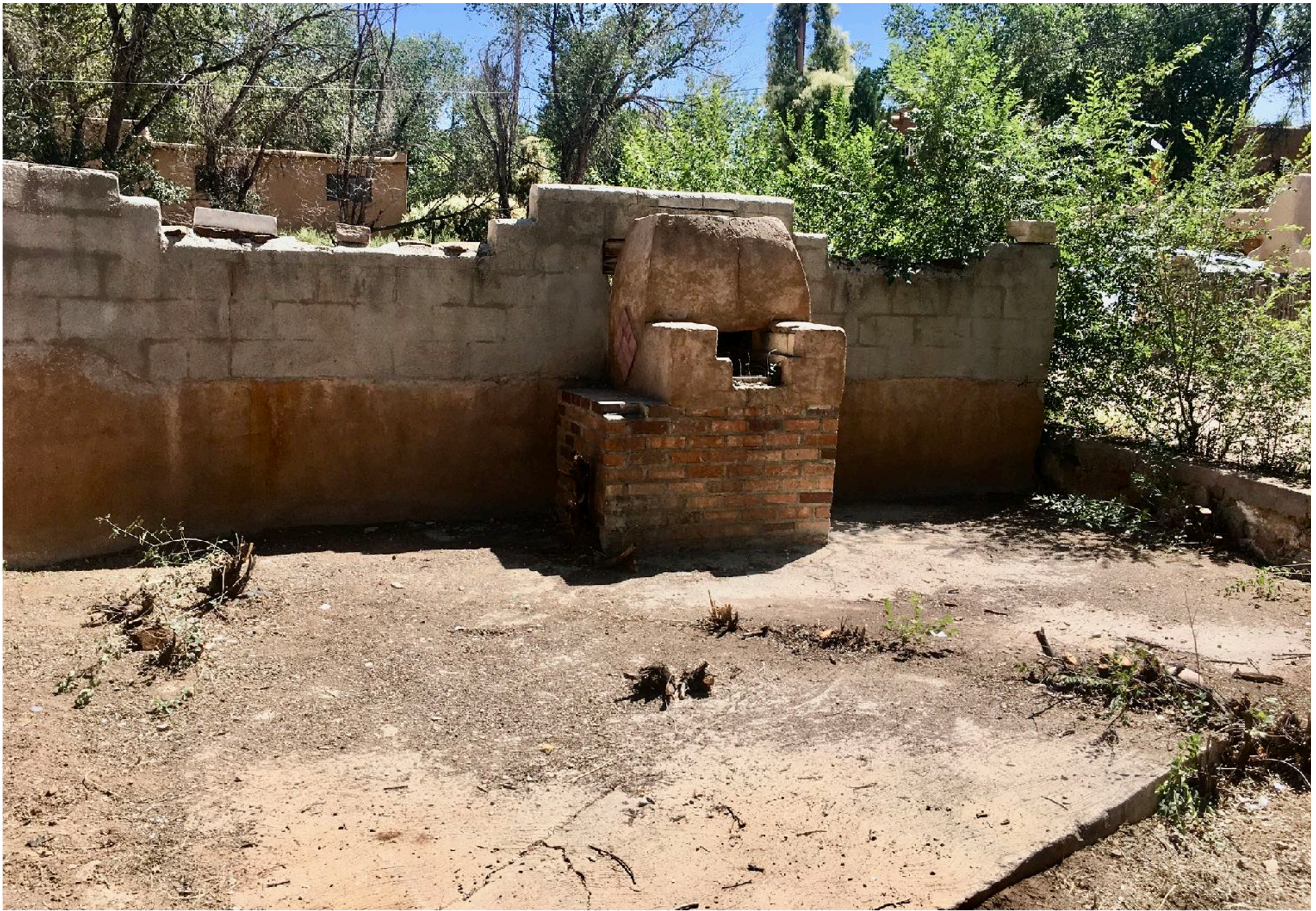
107 VICTORIA STREET GRILL & YARDWALL, NORTH SIDE
