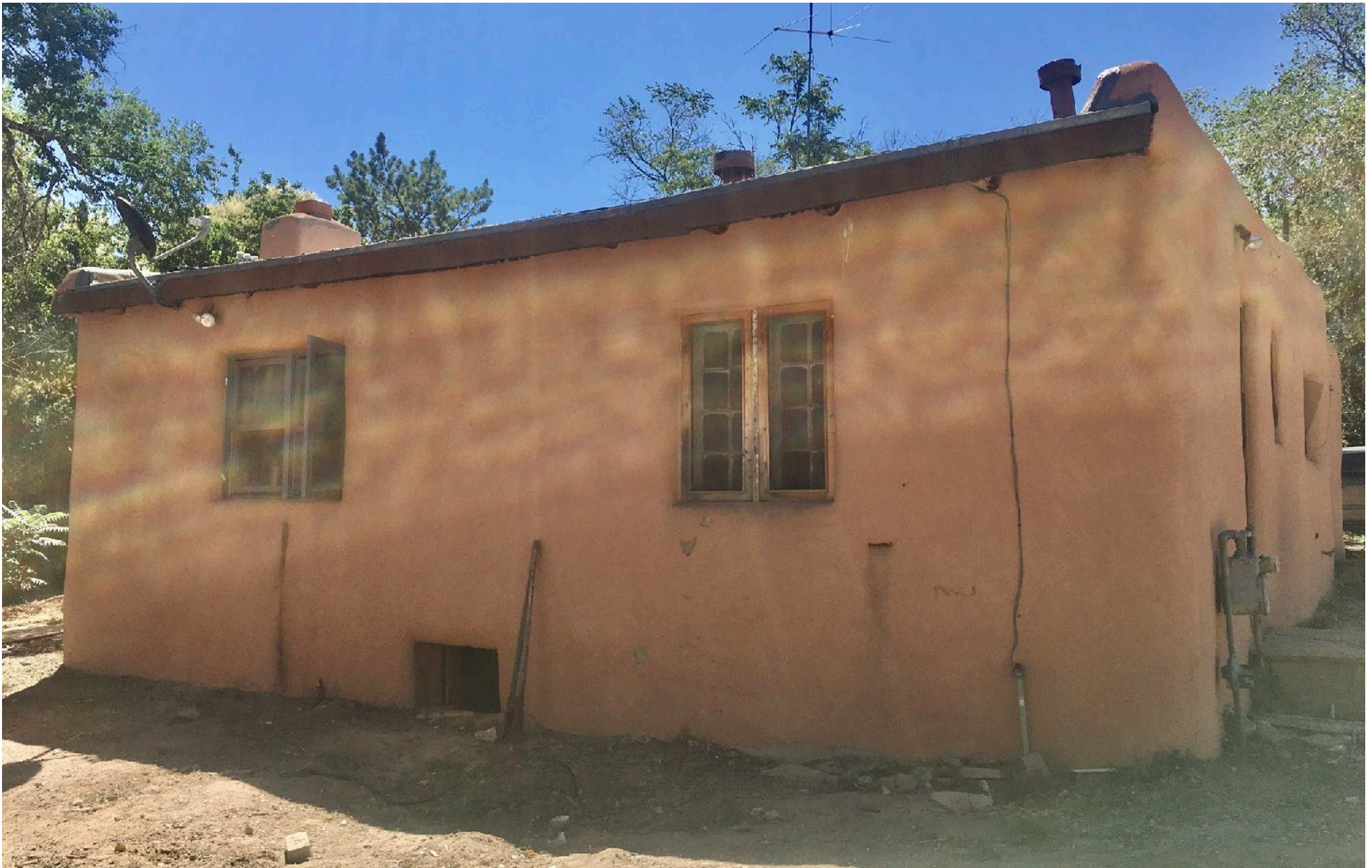
107 VICTORIA STREET NORTH FAÇADE
