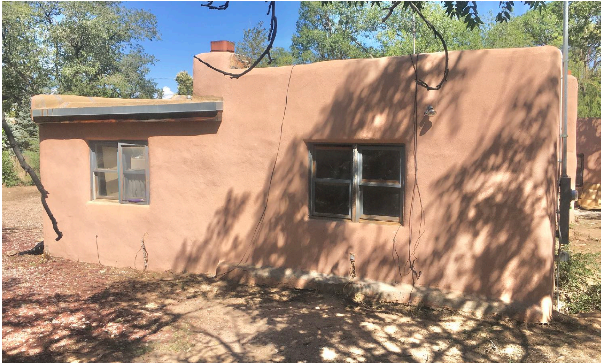
107 VICTORIA STREET SOUTH FAÇADE
