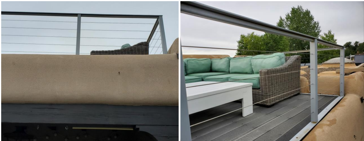
Figure 1: Metal & cable deck rail on nearby home.
