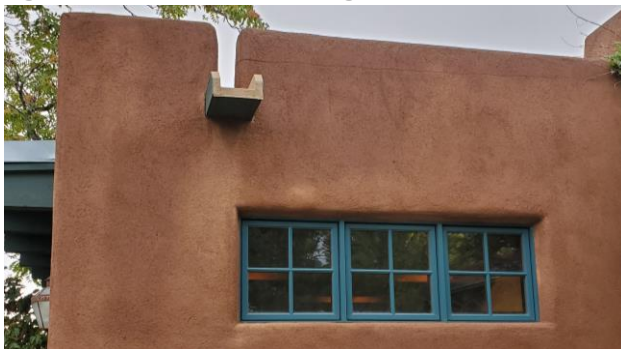
Figure 2: Windows on existing home
