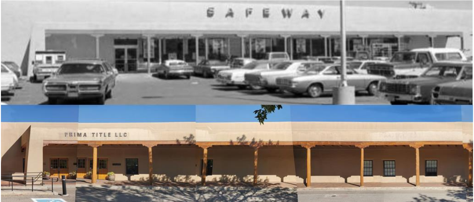
Figure 24: Composite image showing c.1977 and 2020 photographs of front (west) façade.
