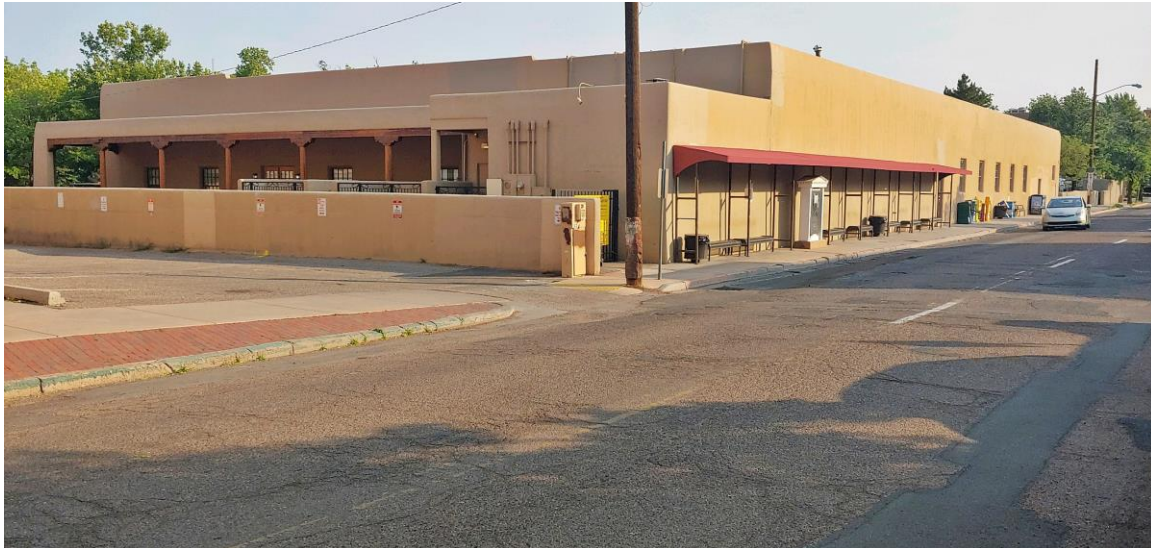
Photo 8: South and east elevations. Camera facing northwest. Robyn Powell: June 13, 2021.
