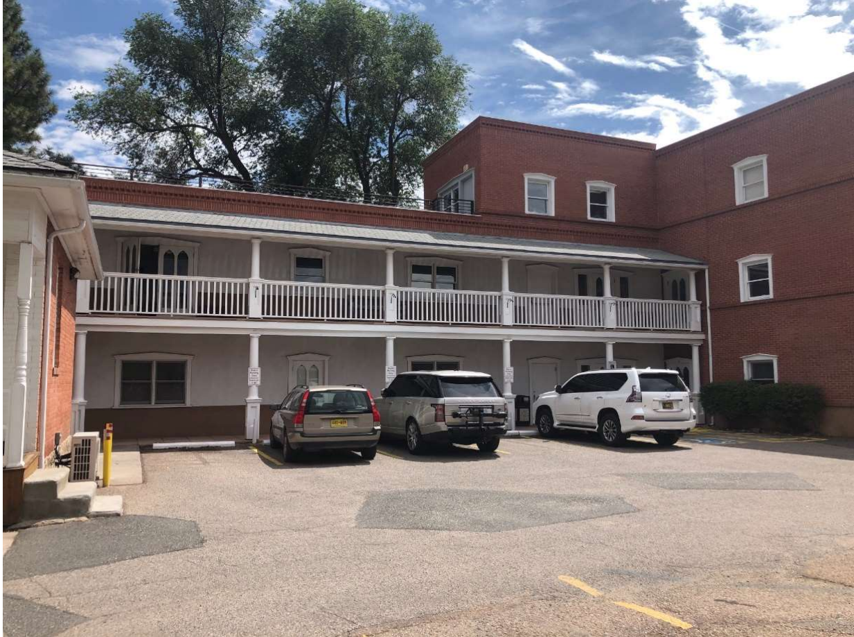
FIG 07 - PARKING LOT WITH 128 GRANT AVE SHOWING BALCONY ON 2 ND FLOOR
