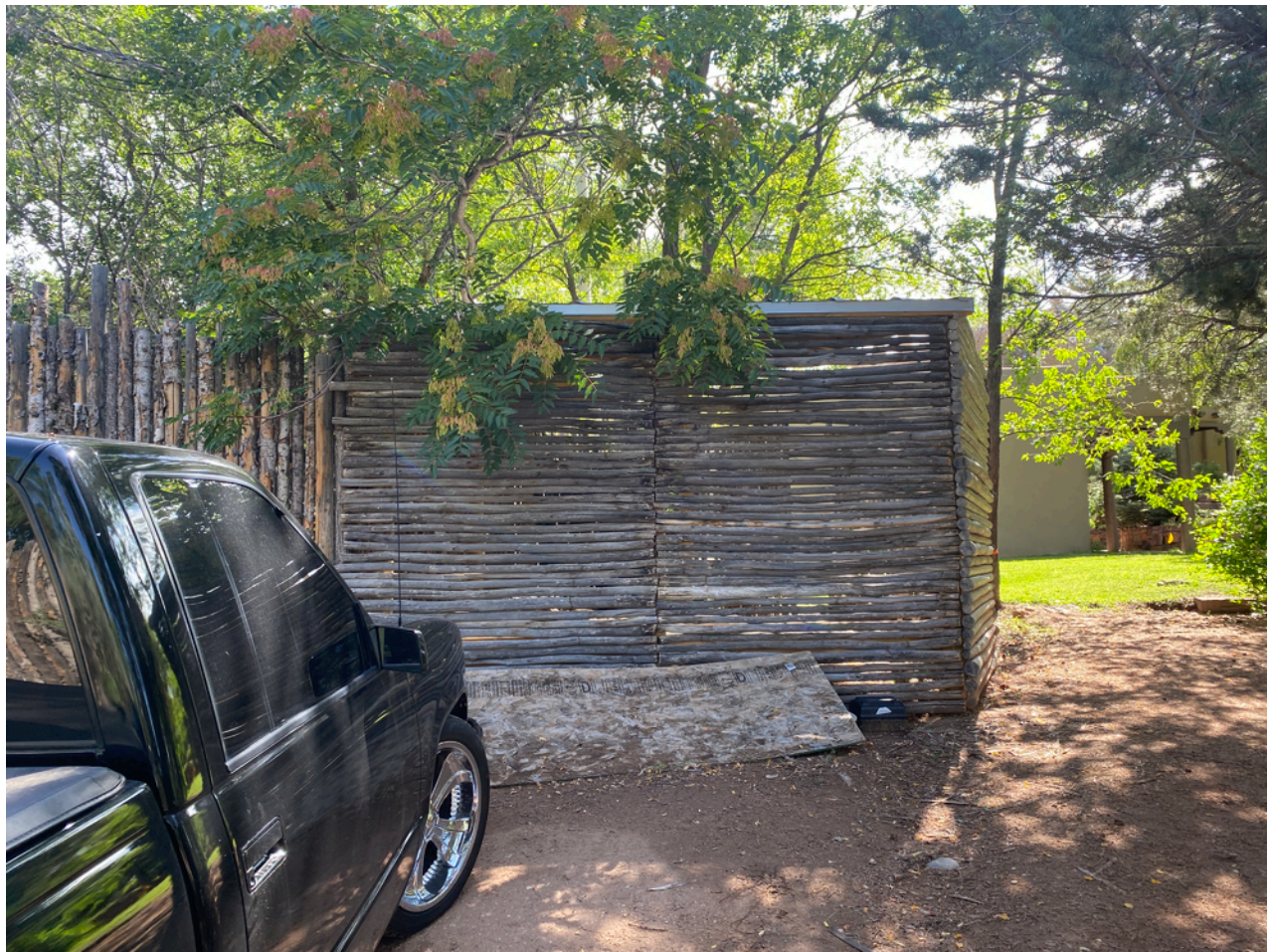
SHED — Removal of existing shed
