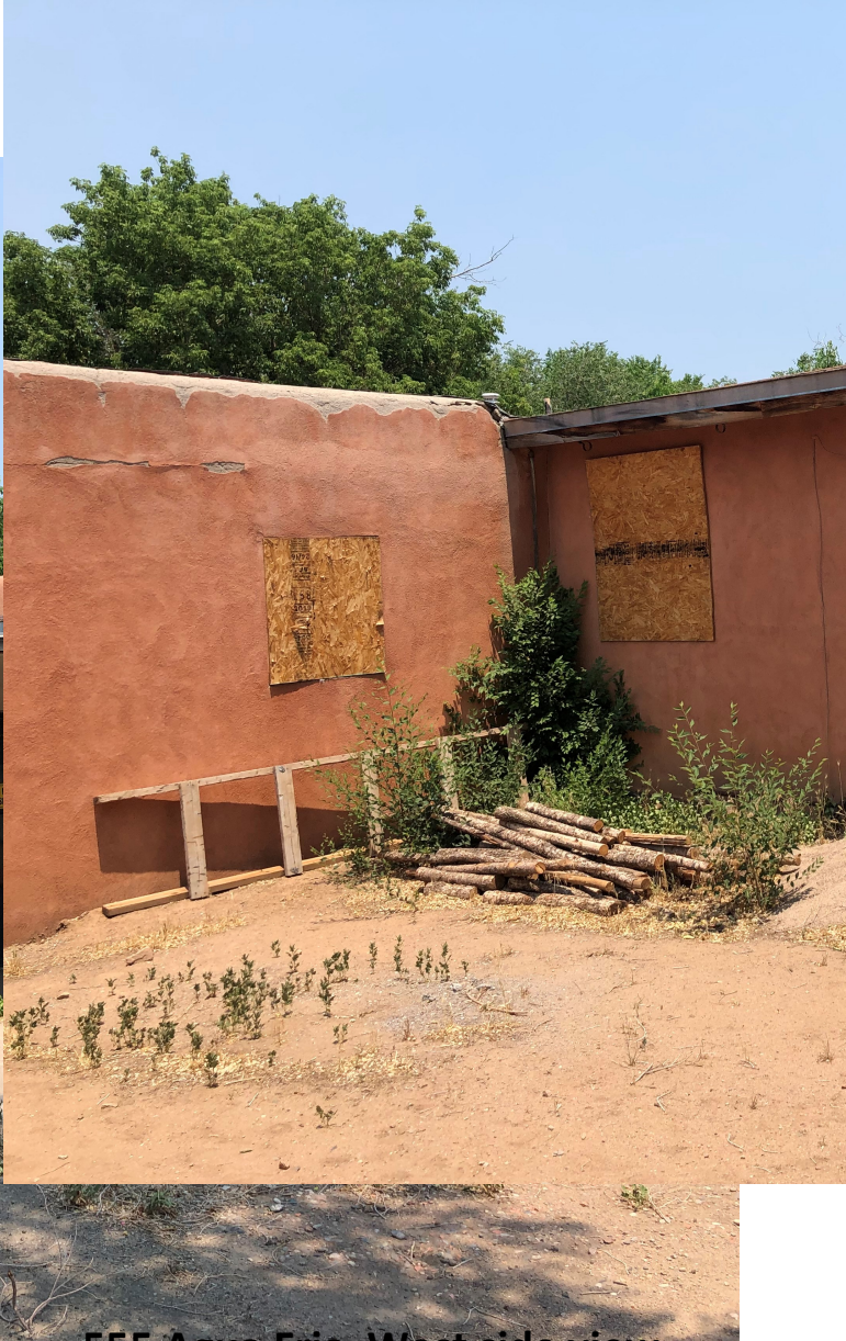
555 Agua Fria West side view
