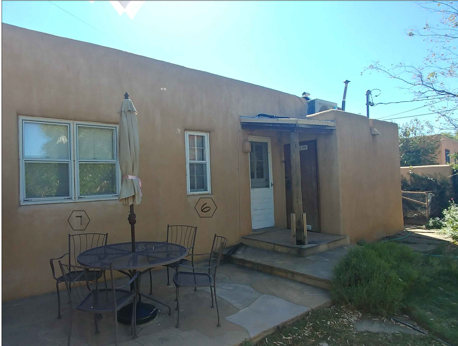
Partial east elevation w/ windows #6 and #7
