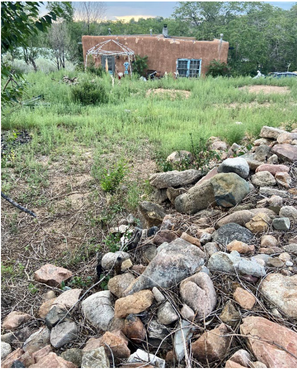
Figure 8. Location of west retaining wall looking north
