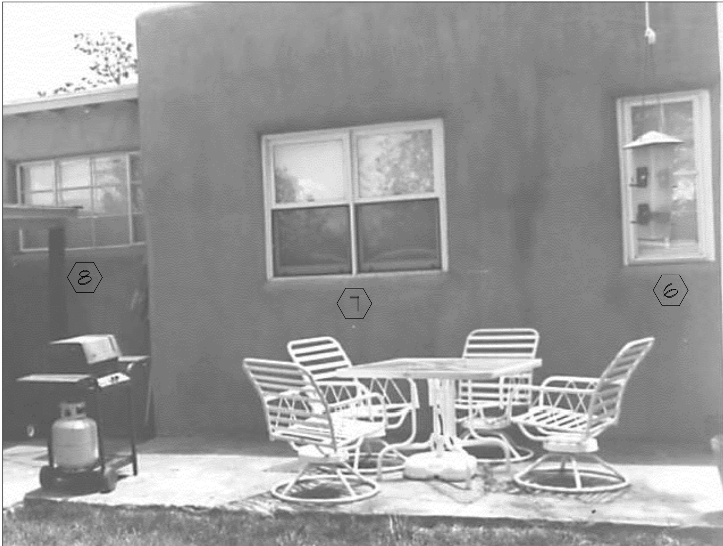
Partial west elevation from 1995 w/ windows #6, #7 and #8
