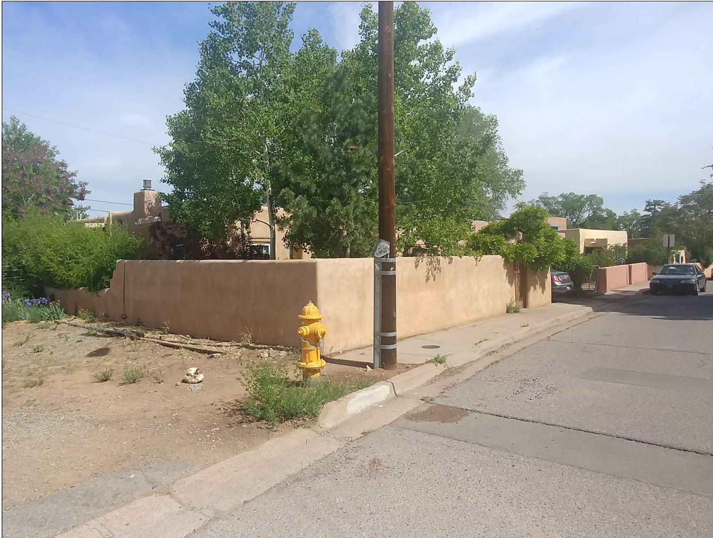
Partial east and south elevations
