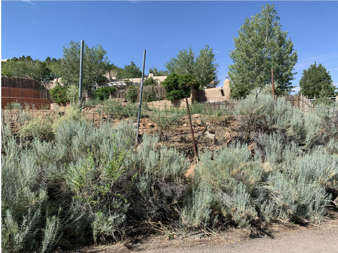
MID PROPERTY LINE - EXISTING WIRE FENCE / EROSION
