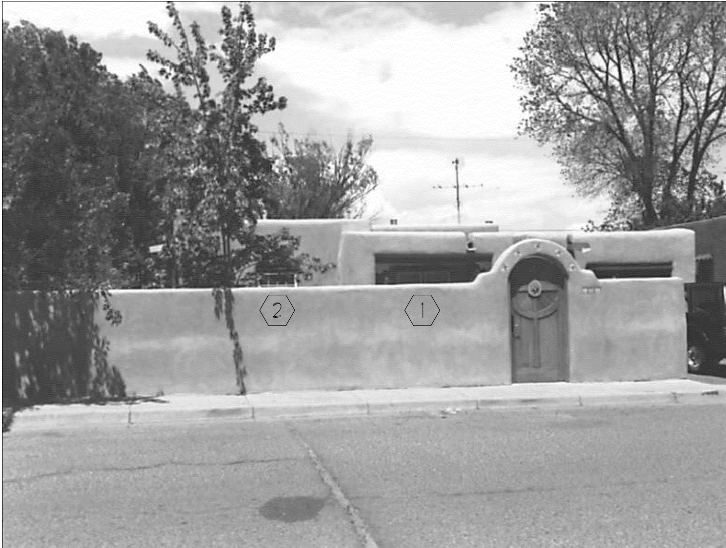
East elevation from 1995
