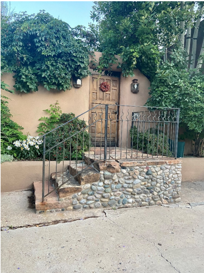
Figure 10. Stairs from parking area w/ rock façade. We will construct brick steps
