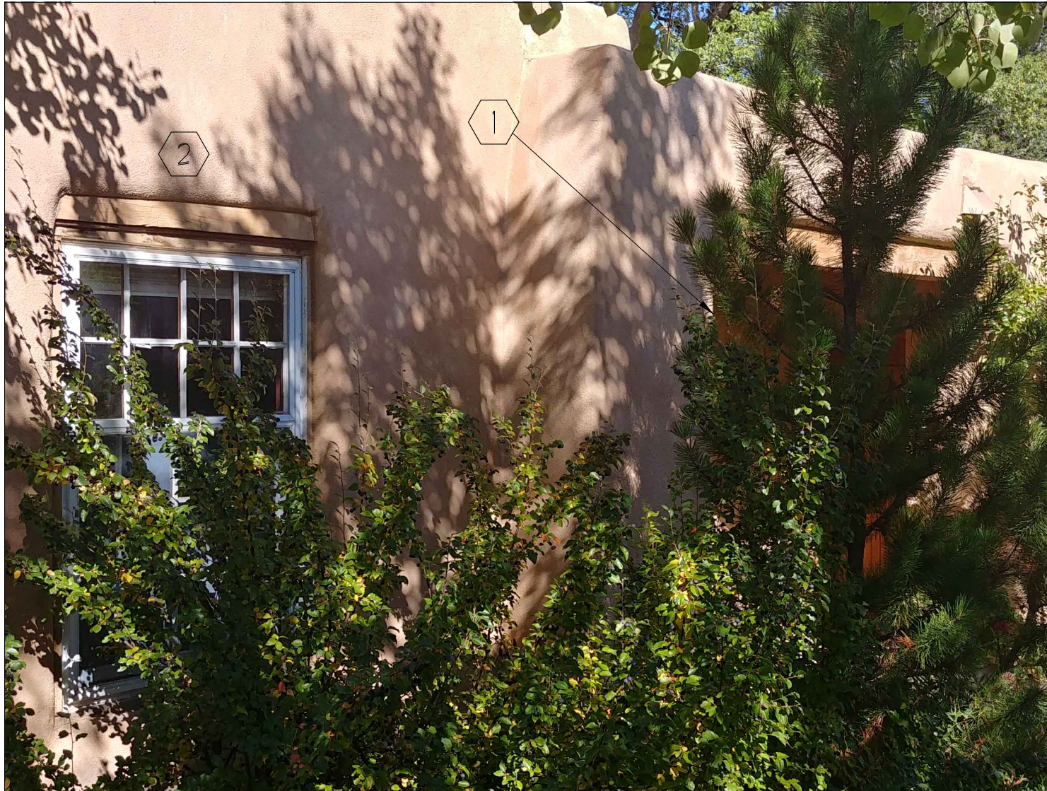
Partial east elevation w/ windows #1 and #2
