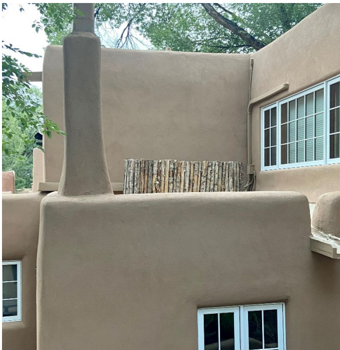
Figure 6. HVAC Screening w/ parapet and coyote fence
