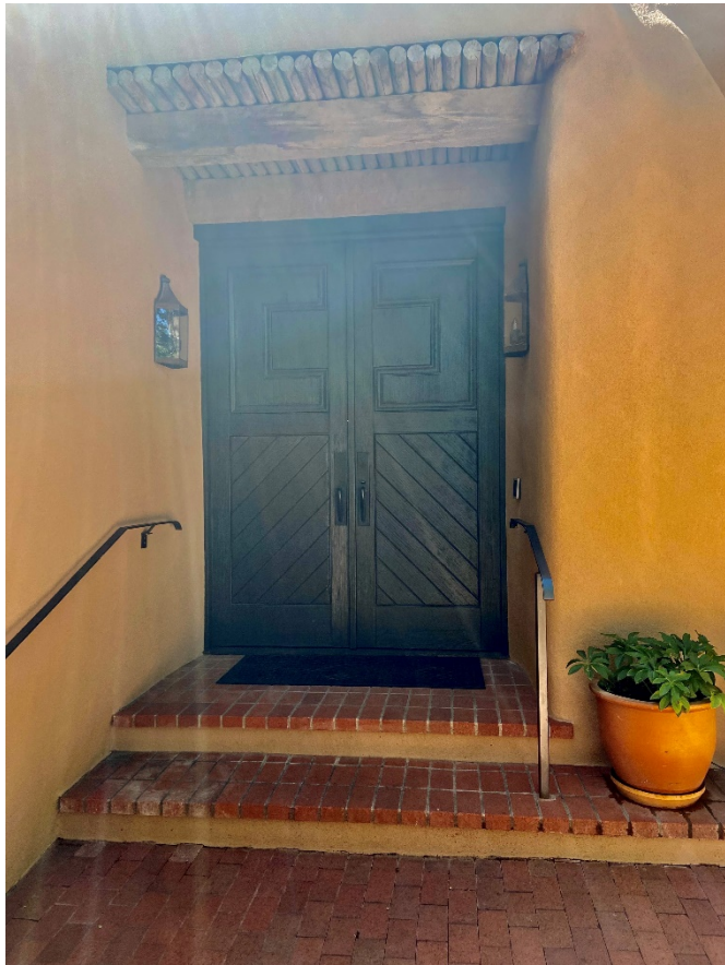
Figure 4. Beam, latillas, brick stairs & hand rail
