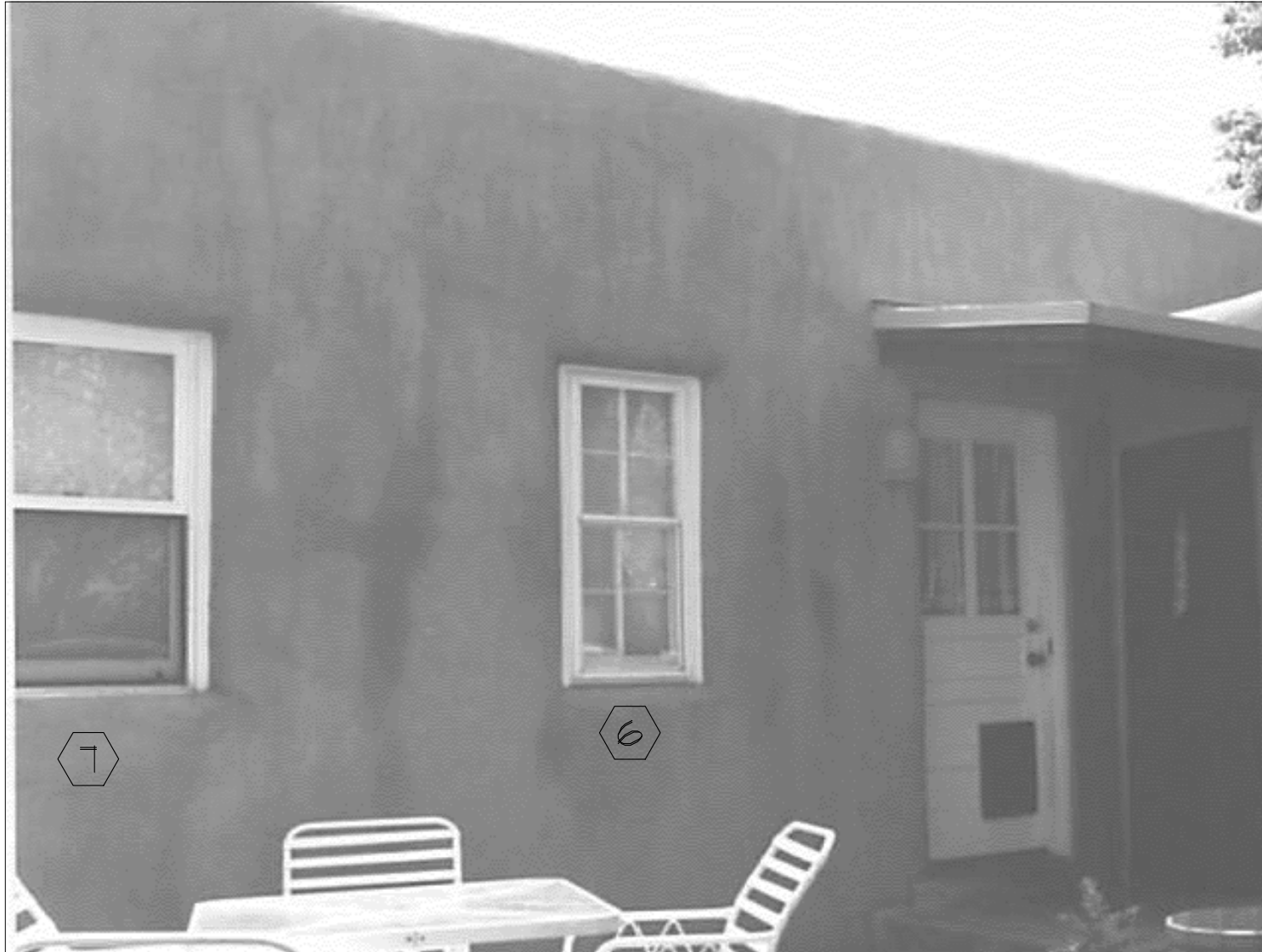
Partial west elevation from 1995 w/ windows #6 and #7
