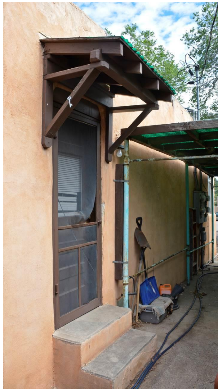
Photo 11: 1950s duplex, east elevation. Camera facing northwest.
