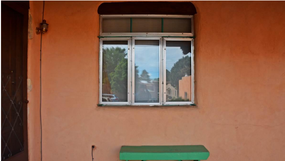
Photo 6: 1950s duplex, portal windows. Camera facing south.
