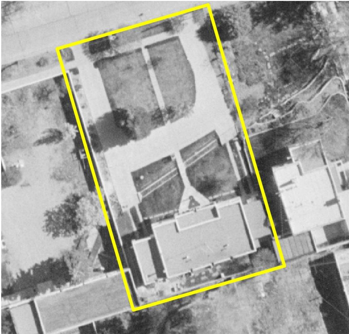
Figure 5: May 11, 1973, aerial photograph. Note maturing of formal landscape. Courtesy New Mexico Department of Transportation.
