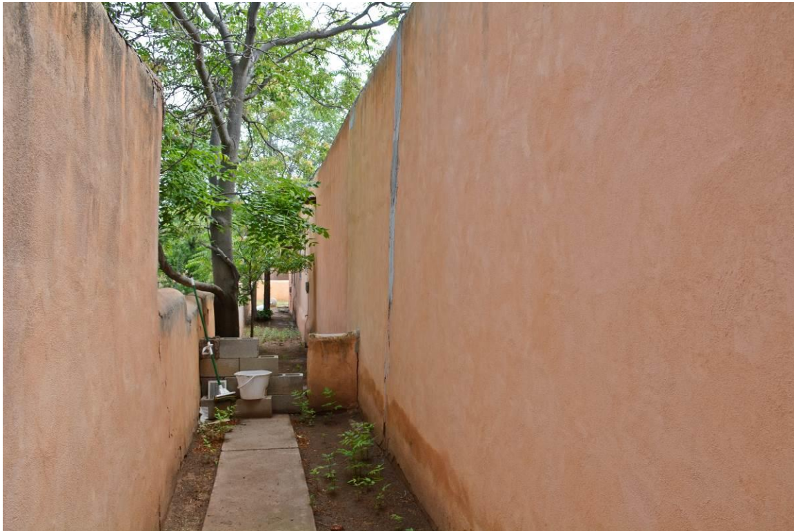
Photo 14: 1950sduplex, west elevation. Camera facing northeast.
