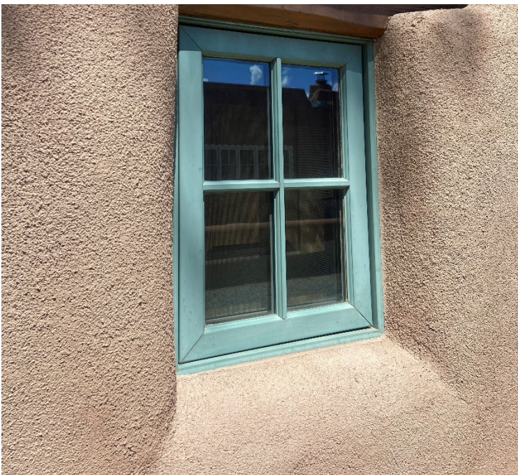
Figure 3. Window with divided light, inset and lintel beam
