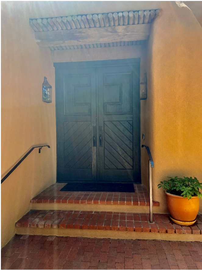
Figure 4. Beam, latillas, brick stairs & hand rail
