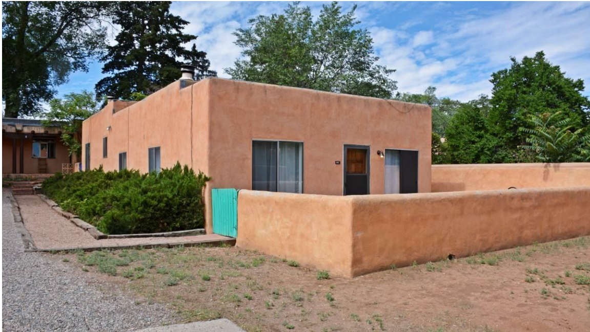
Photo 15: 1980s duplex, yard walls. Camera facing southwest.
