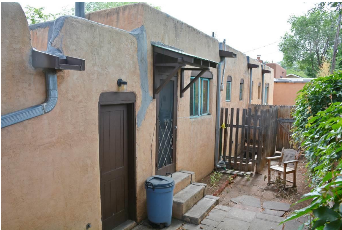
Photo 13: 1950s duplex, south elevation. Former garage at left. Camera facing northeast.
