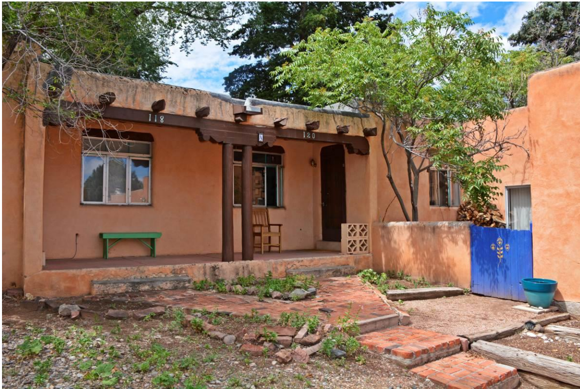
Photo 5: 1950s duplex, north elevation. Camera facing southwest.
