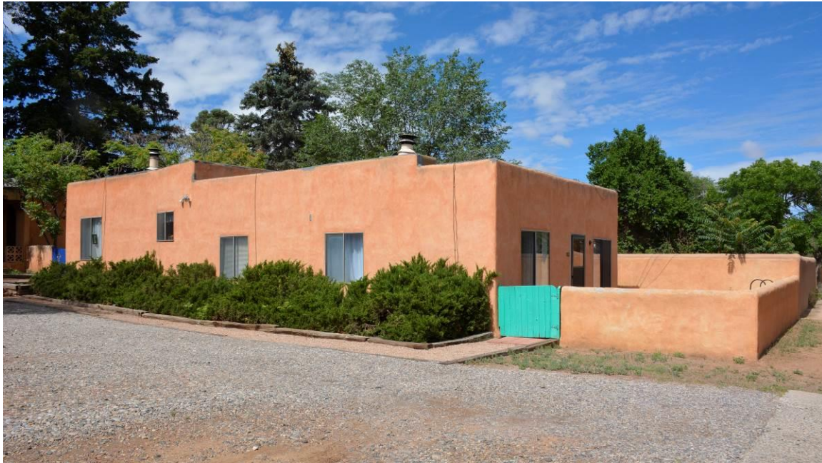
Photo 2: 1980s duplex, east elevation. Camera facing southwest.
