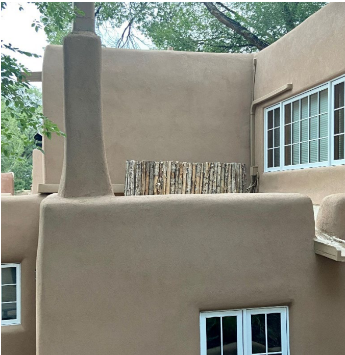
Figure 6. HVAC Screening w/ parapet and coyote fence
