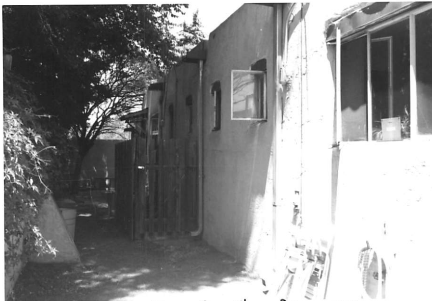
#33 south elevation from SE
