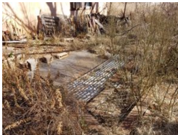
Figure 6-2 Septic tank improperly covered by plywood and corrugated tin. Courtesy of NMED Liquid Waste Program.
