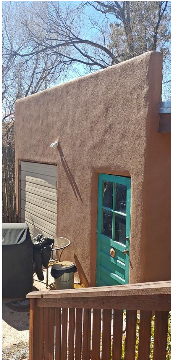
Photo 12: Garage, east elevation. Note extended parapet. Camera facing southwest.
