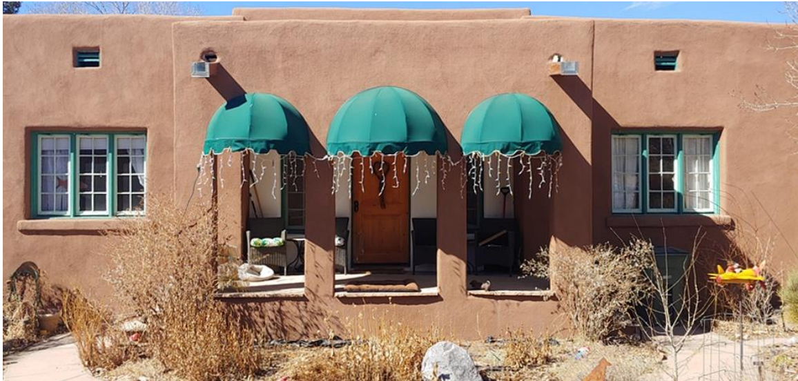
Photo 2: Front, east façade. Camera facing west.
