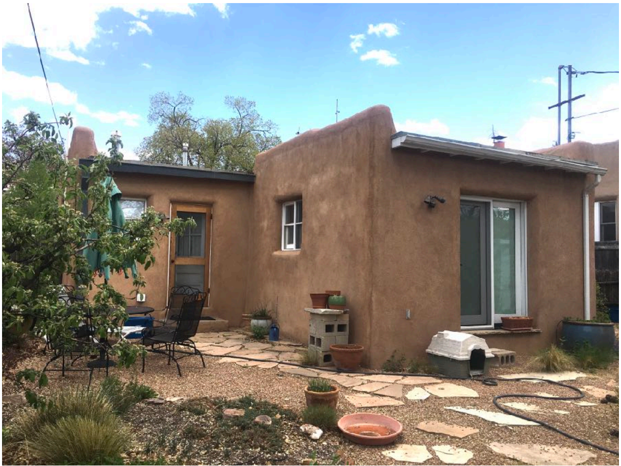
West and North Elevation viewed from northwest corner
