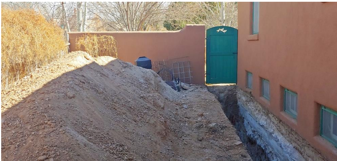
Photo 9: East half of north elevation. Camera facing east.
