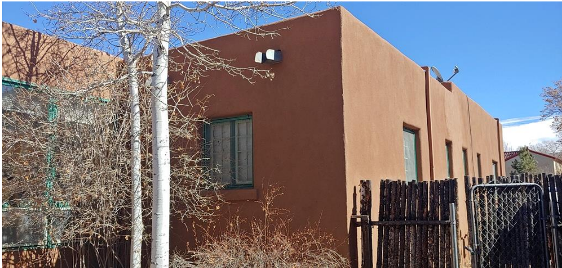
Photo 5: West and south elevations; addition at left. Camera facing northwest.
