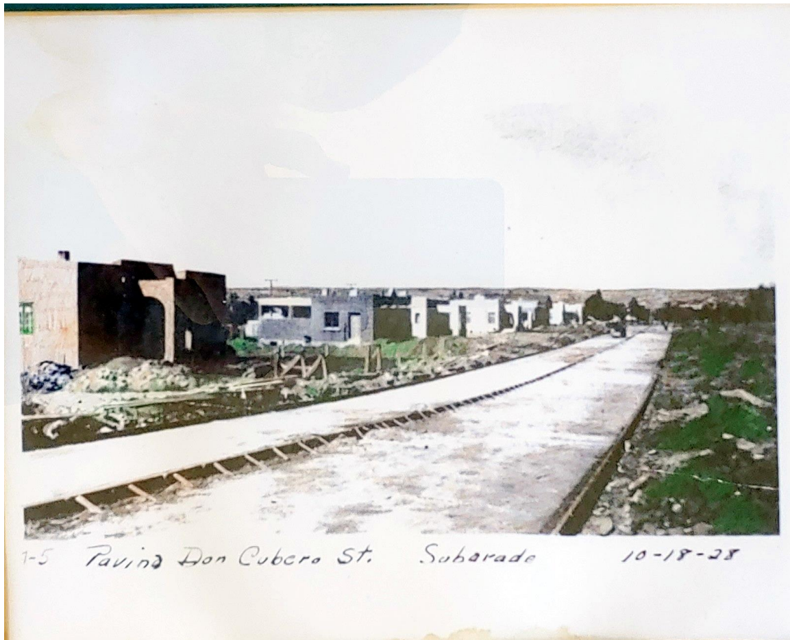
Figure 4: Don Cubero Avenue Under Construction, October 18, 1928. Courtesy Tim and Evelyne Taylor.
