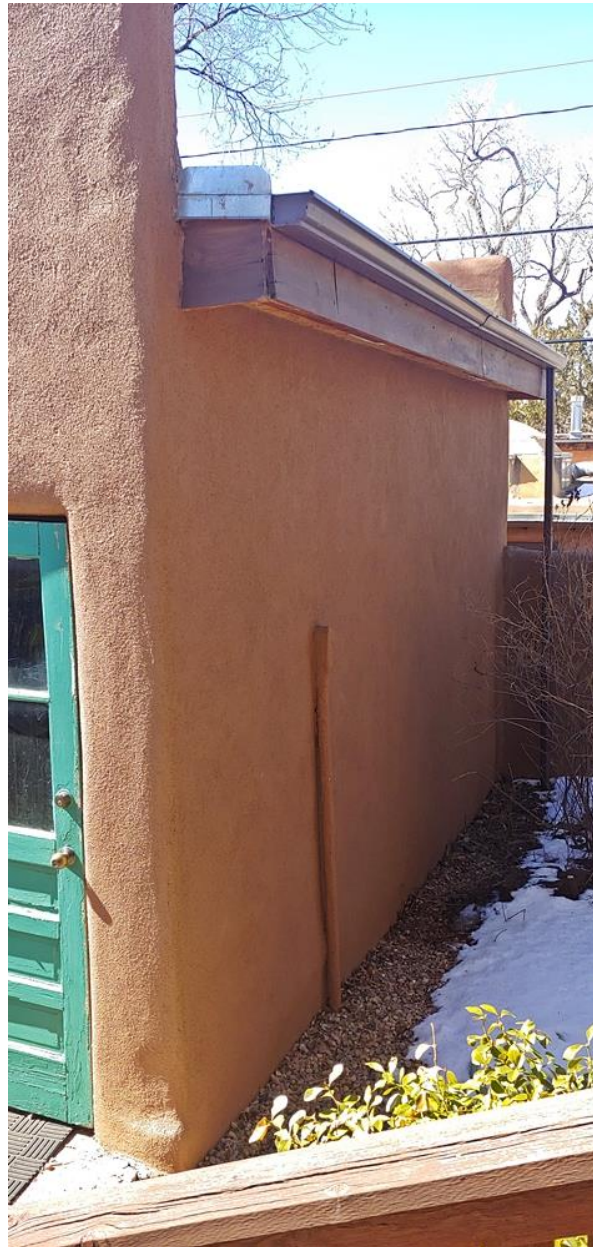
Photo 14: Garage, north elevation. Note removed parapet and addition of overhang. Camera facing southwest.
