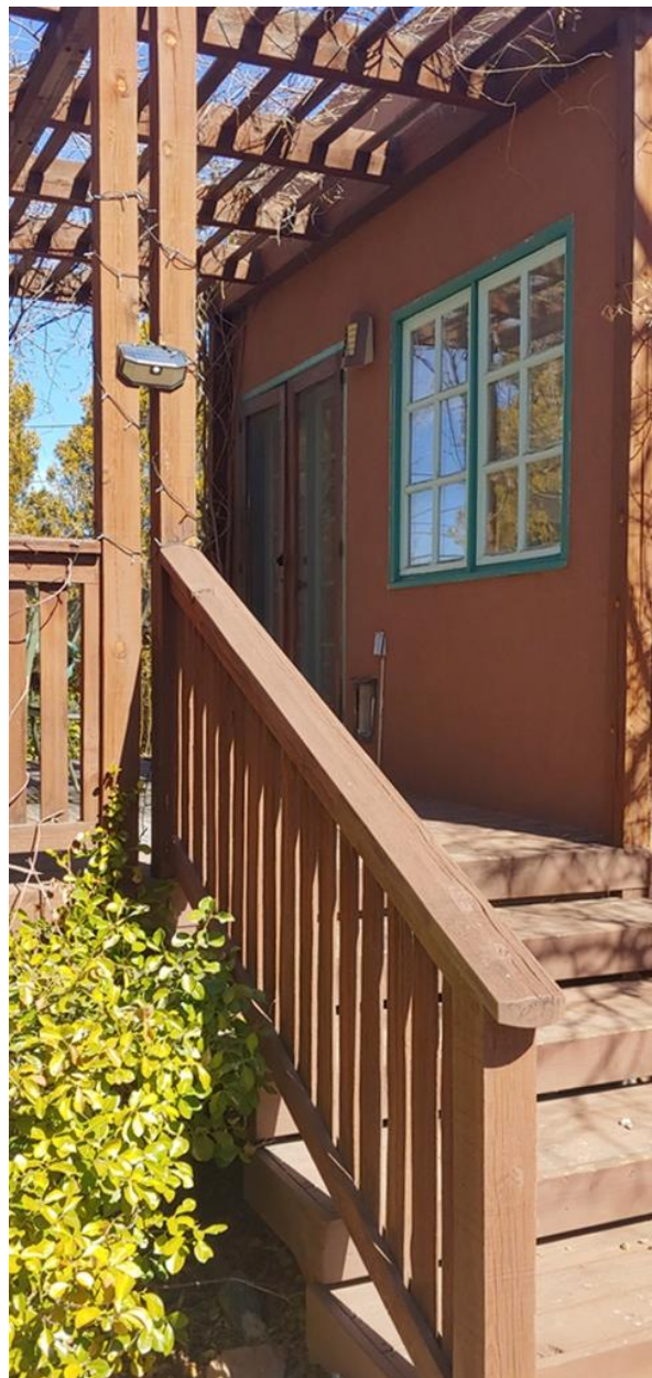
Photo 7: Addition, west elevation. Camera facing northeast.
