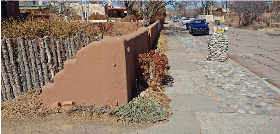
Photo 16: Yard Wall at street. Camera facing north.
