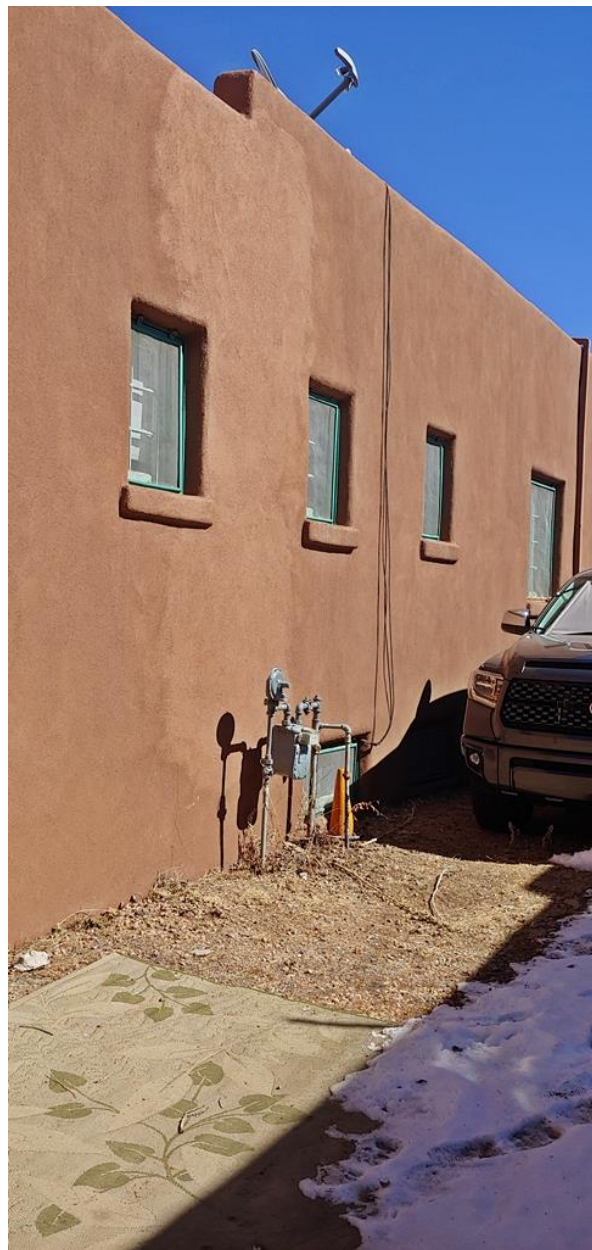
Photo 4: South elevation. Camera facing northeast.
