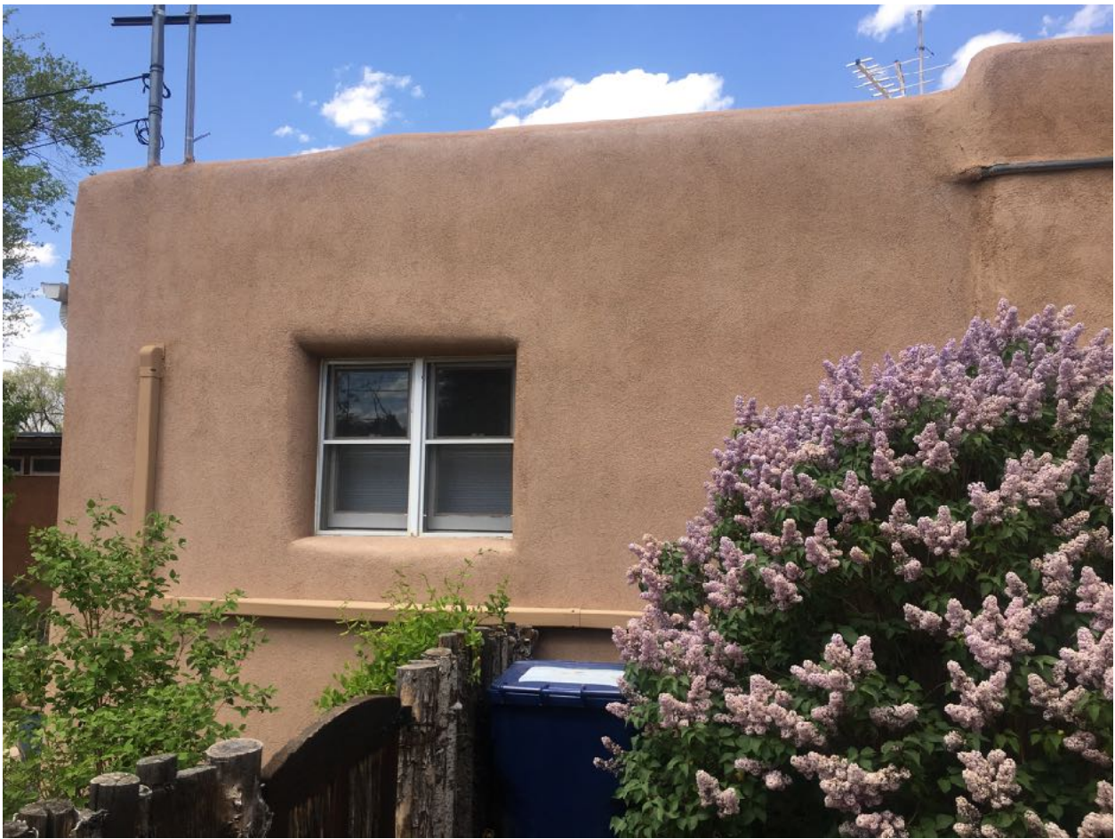
West end of South Elevation
