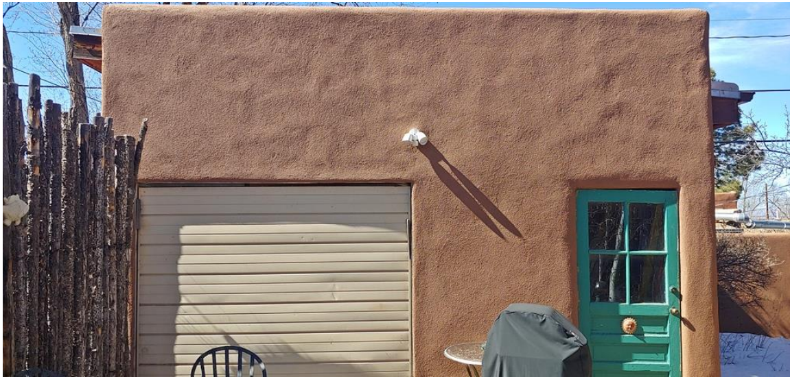
Photo 11: Garage, east elevation. Camera facing west.
