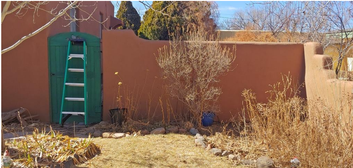
Photo 17: Interior Yard Wall. Camera facing west.
