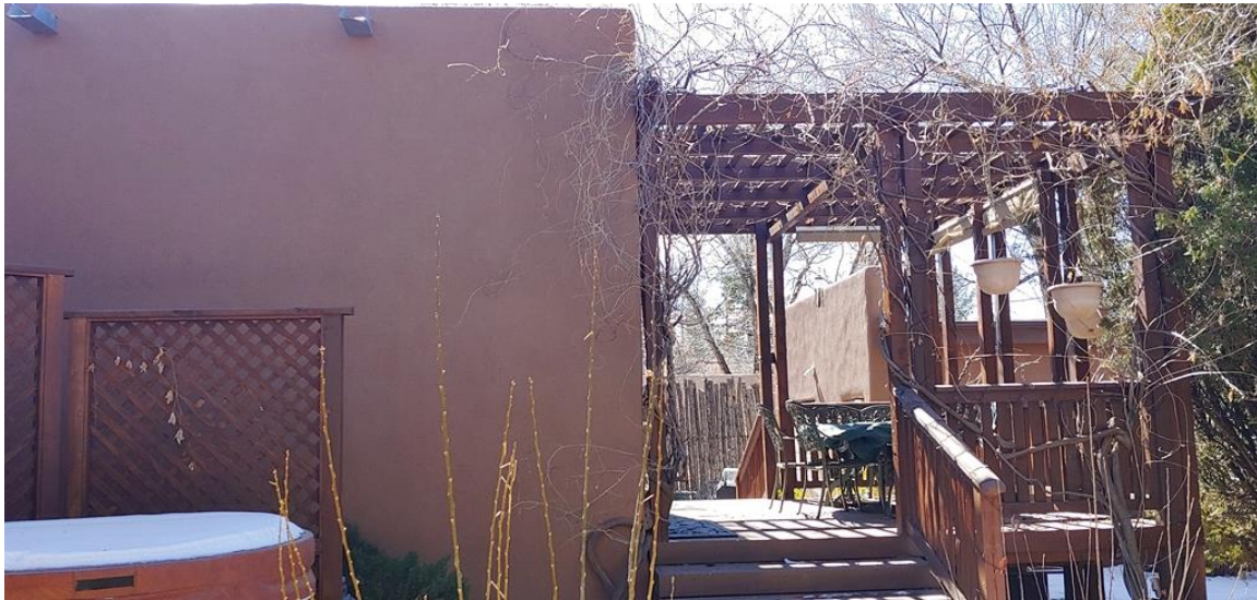
Photo 8: Addition, north elevation. Camera facing southwest.
