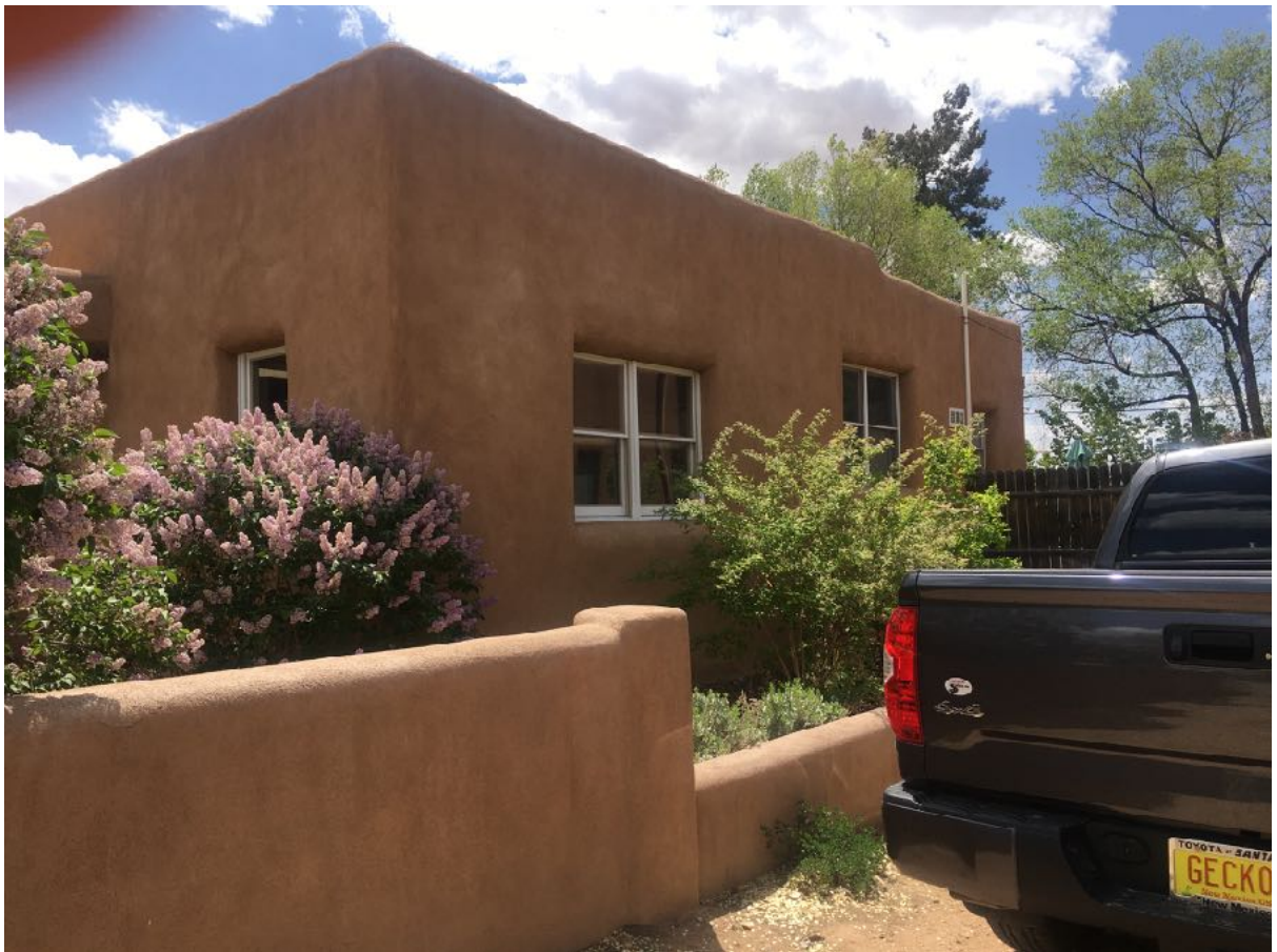
West Elevation viewed from northeast corner
