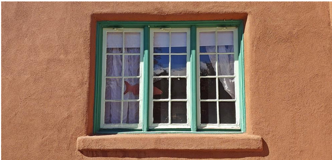
Photo 3: Typical casement windows. Camera facing west.
