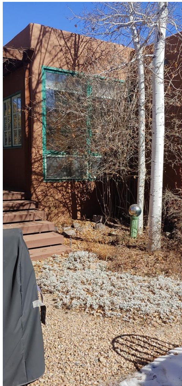
Photo 6: Addition, south elevation. Camera facing northeast.
