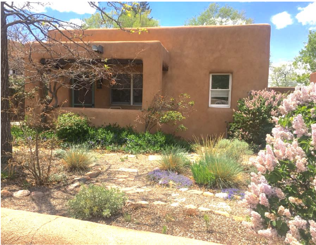
East Elevation-Street facing
