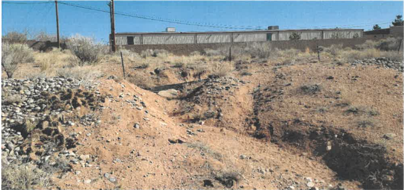
An arroyo created by runoff from the upper level with Mini U Storage (also Santa Fe Wine Storage) in background.
