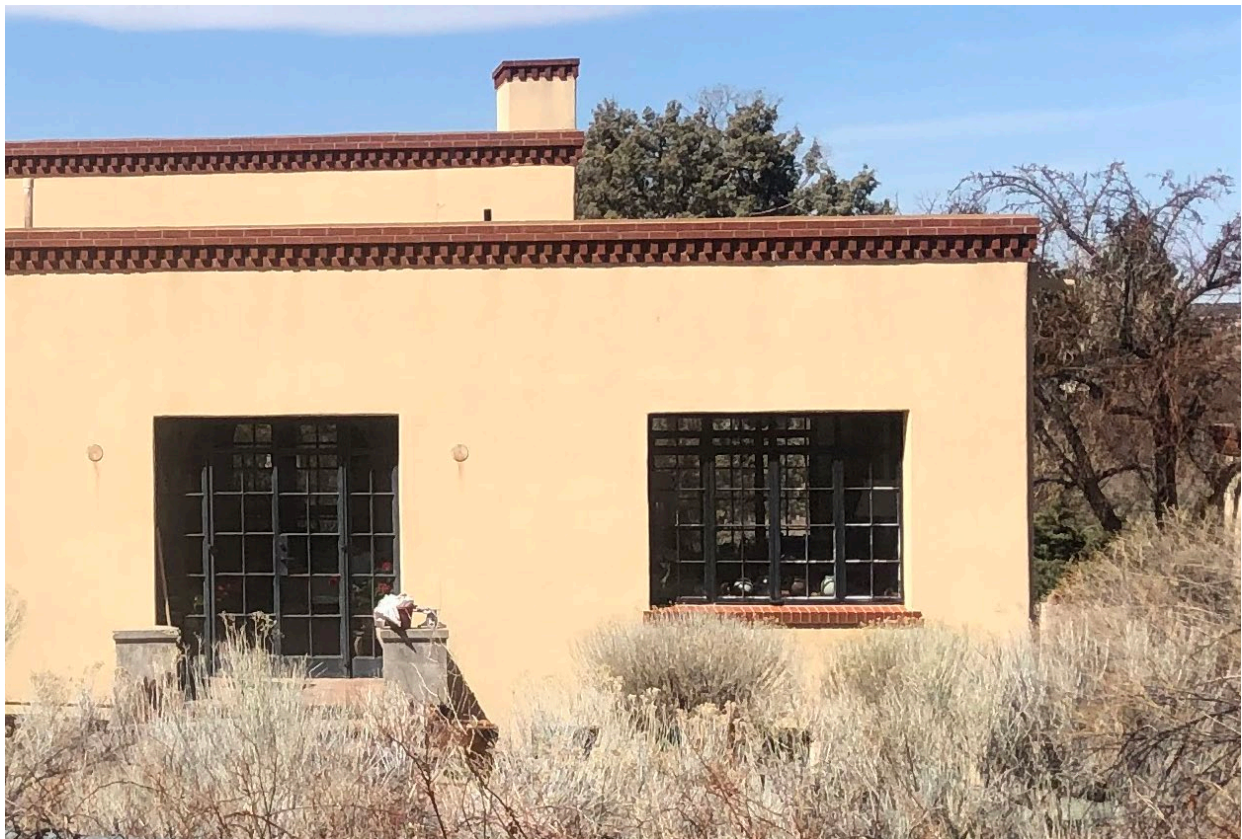
Steel Windows at 803 Camino Atalaya, designed by John Gaw Meem
