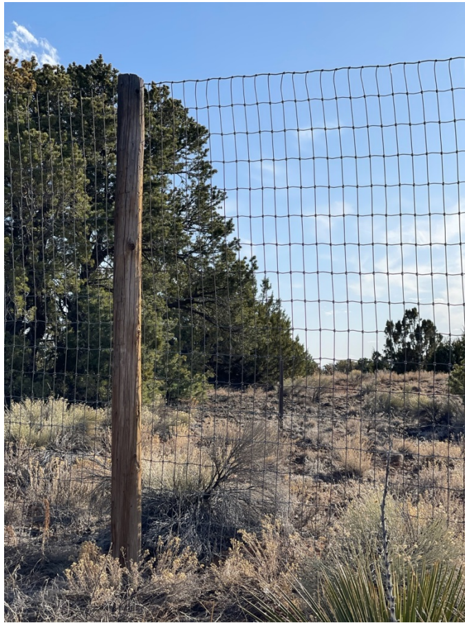
Example of rabbit fencing for in-kind replacement along eastern property boundary
