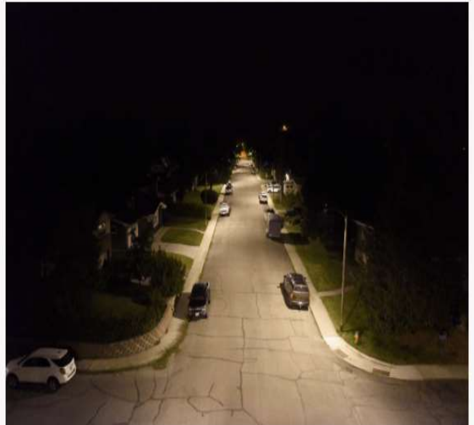
Fairview Ave. LED #2
